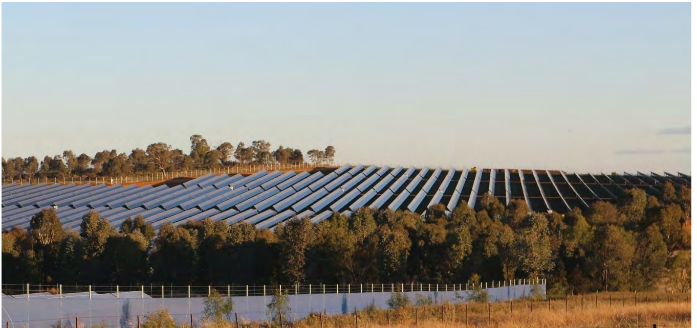
Figure 3.1 Solar array example – Wagga Wagga Solar Farm (source: Terrain Solar)
