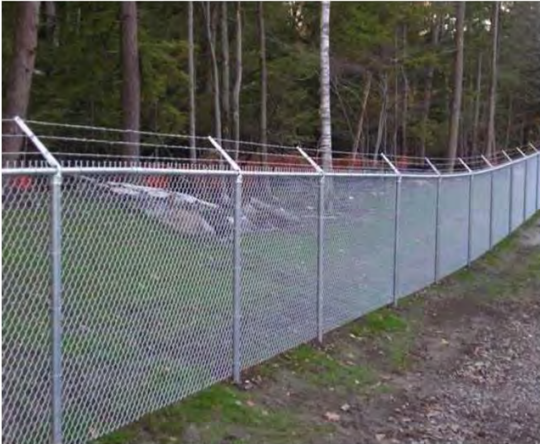
Figure 3.3 Security fencing example
