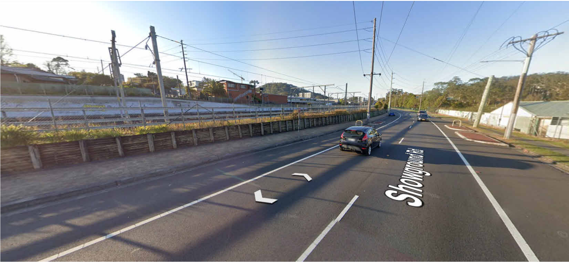
59: CORNER OF SITE FROM SHOWGROUND ROAD
