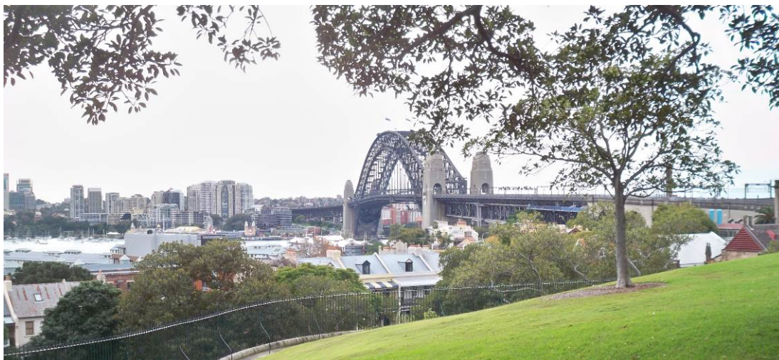
Fig 2.9 – Sydney Harbour Bridge viewed from Observatory Hill
