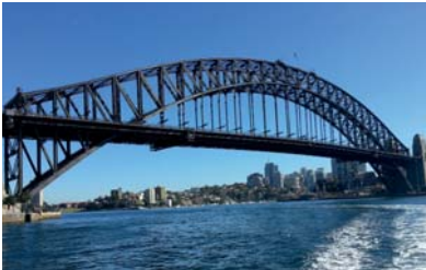
Sydney Harbour Bridge
