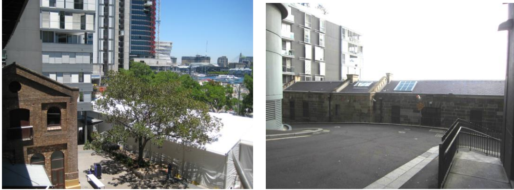
Figure 36 Open space resulting from the courtyard in front of the MSB group extends visually to Darling Harbour. This aspect of the setting of the items will be affected by the Concept Plan (left) as will views looking west from Gas Lane to the group (right). The appreciation of the group when viewed from Gas Lane will be obscured to some extent because the building will no longer be read clearly against the sky.
