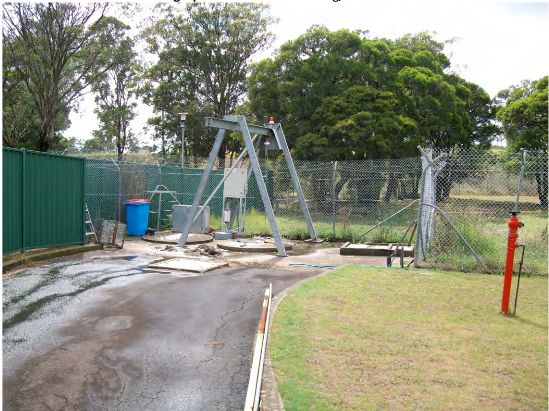
Photograph 6 – The effluent collection point in the eastern part of the Dog/Cat section.
