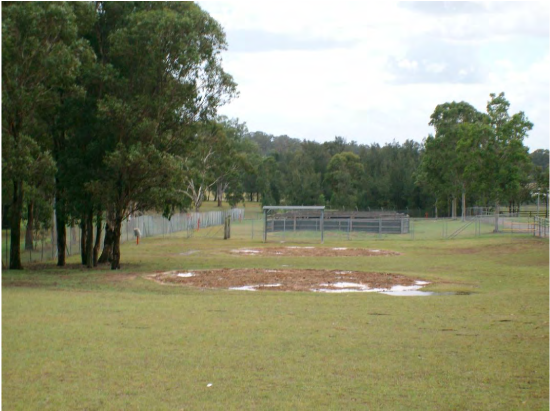
Photograph 7 – View northwards of areas of building waste in the vicinity of former buildings
