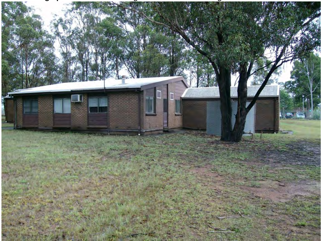
Photograph 4 –The Bee House building with water tank.
