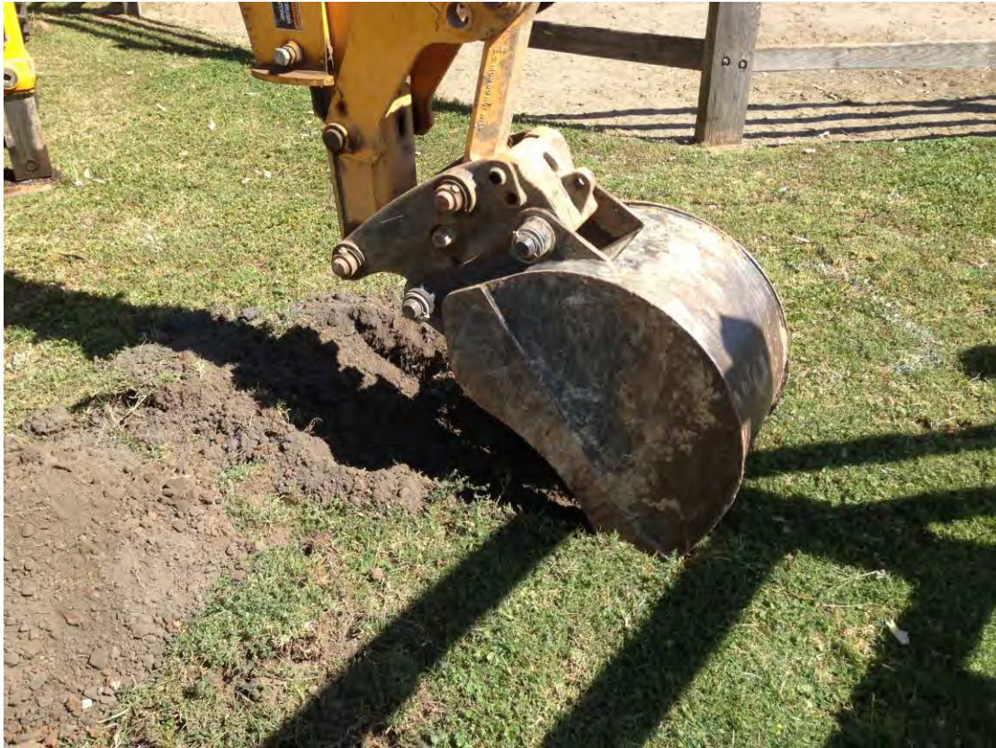
Photograph 11 – Excavation of TP01
