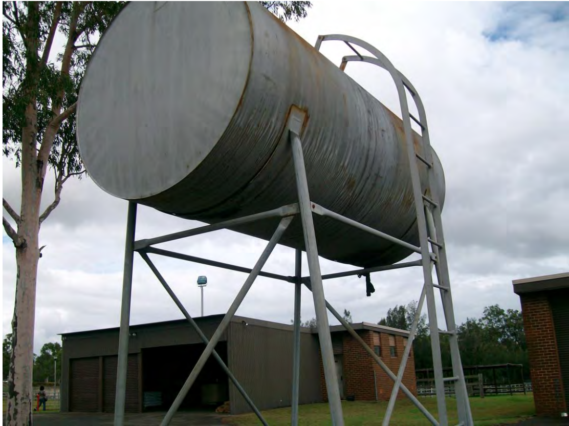
Photograph 9 – The decommissioned aboveground storage tank
