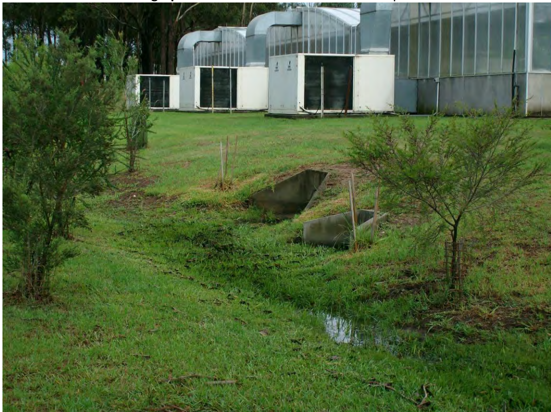
Photograph 2 –Glass greenhouses with attached temperature control units, and surface water drainage channel in foreground.
