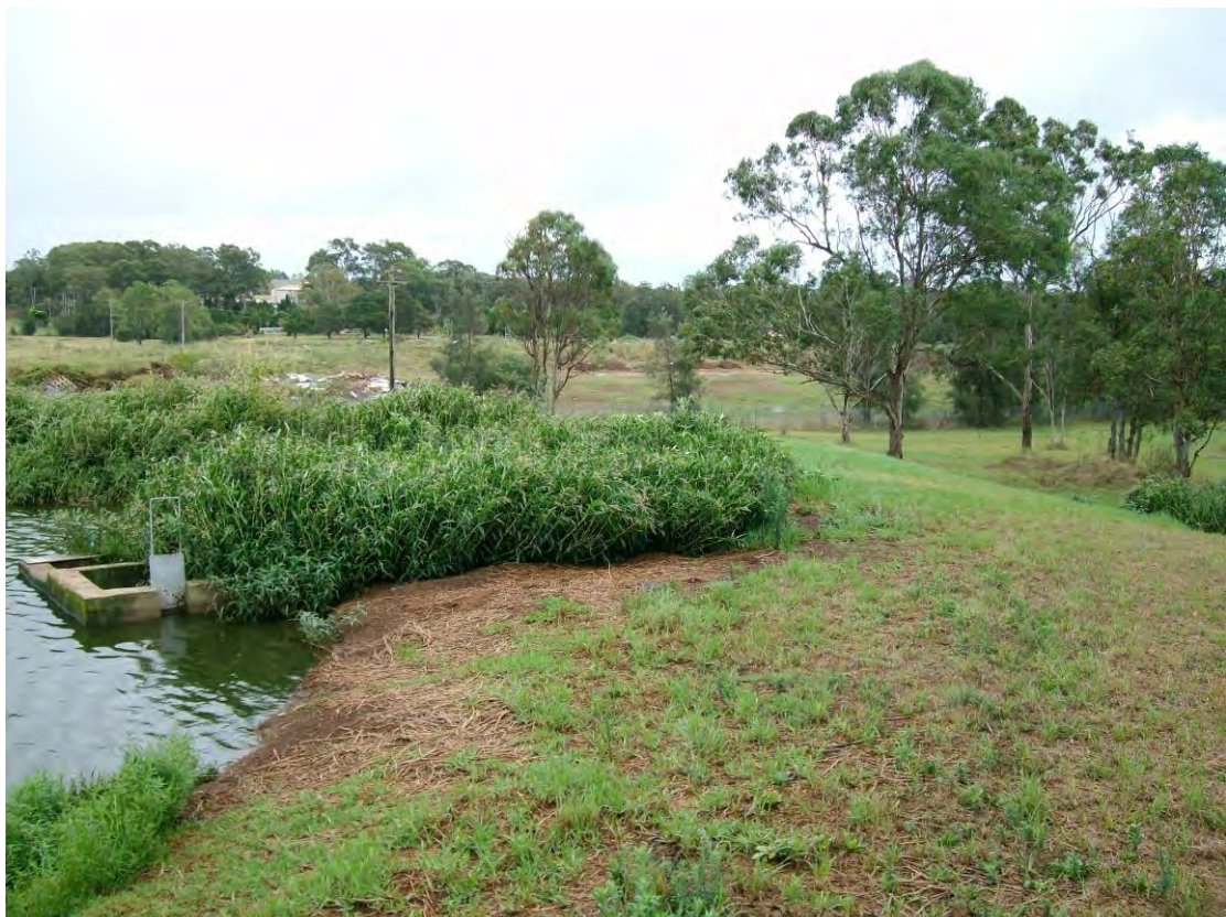
Photograph 10 –The settling pond and embankment of fill
