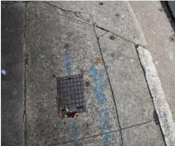
Figure 427 - General condition of service pit
