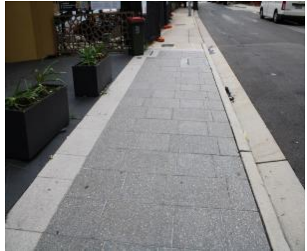
Figure 32 - General condition of footpath pavers heading East
