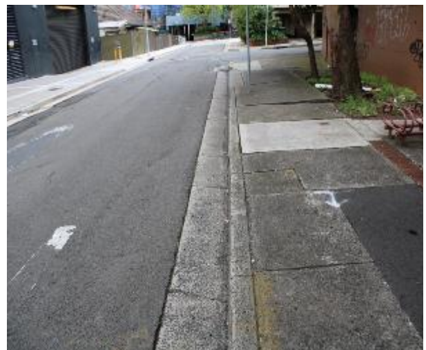
Figure 468 - General condition of kerb and gutter heading North
