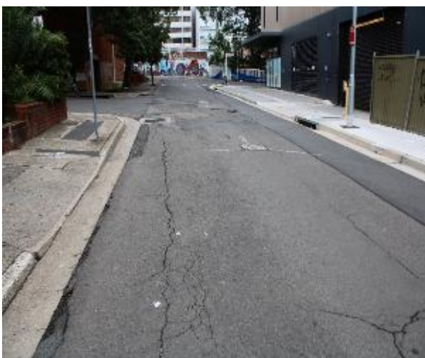
Figure 611 - General condition of road surface heading South
