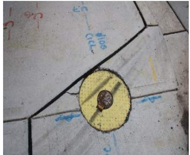
Figure 400 - General condition of service pit
