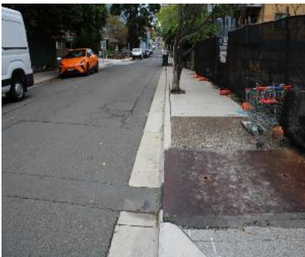
Figure 89 - General condition of kerb and gutter heading West
