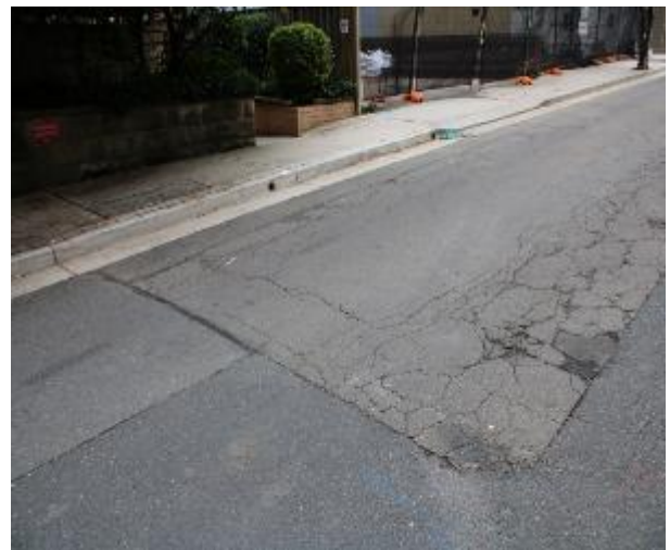
Figure 196 - General condition of road surface heading East
