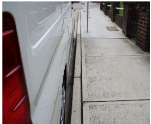
Figure 328 - General condition of kerb and gutter heading East
