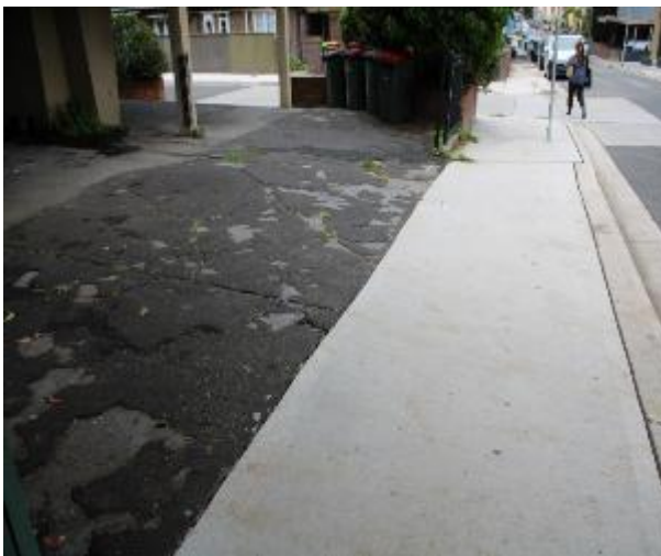
Figure 225 - General condition of footpath pavement heading West
