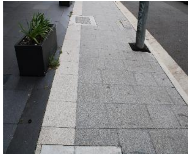
Figure 28 - General condition of footpath pavers heading East
