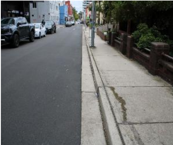
Figure 139 - General condition of kerb and gutter heading West
