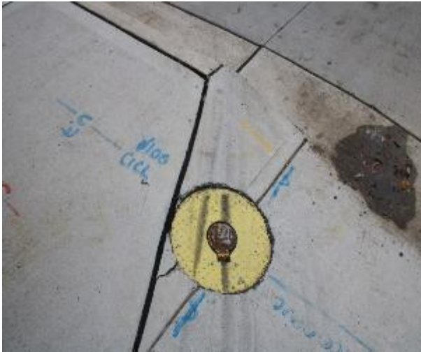
Figure 229 - General condition of service pit
