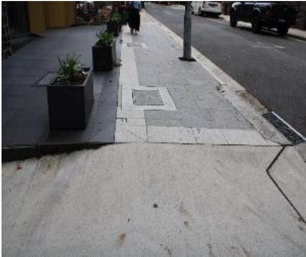
Figure 25 - General condition of footpath pavers heading East
