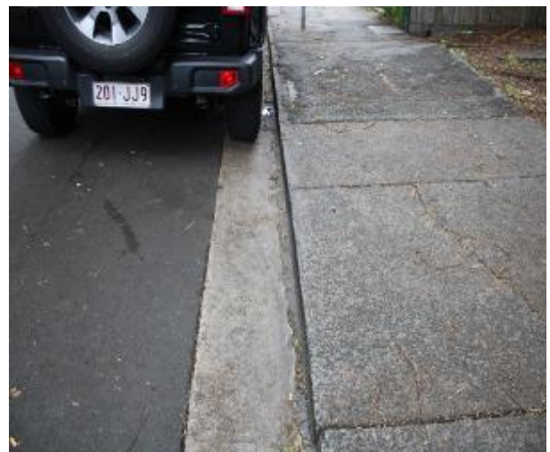
Figure 306 - General condition of kerb and gutter heading East
