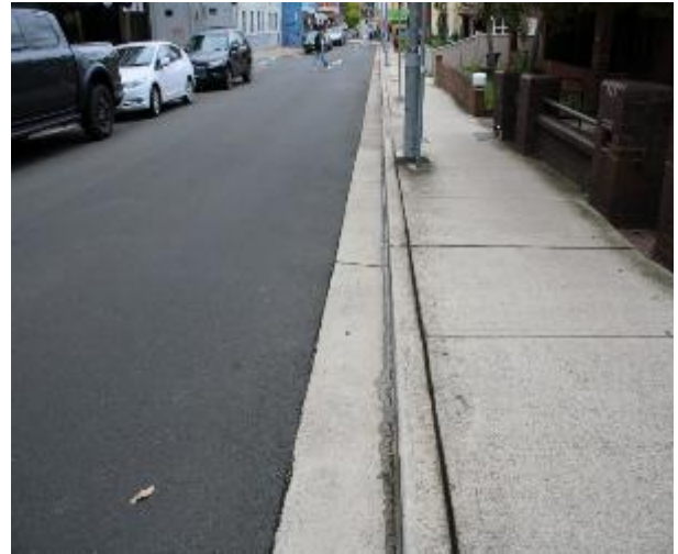
Figure 140 - General condition of kerb and gutter heading West
