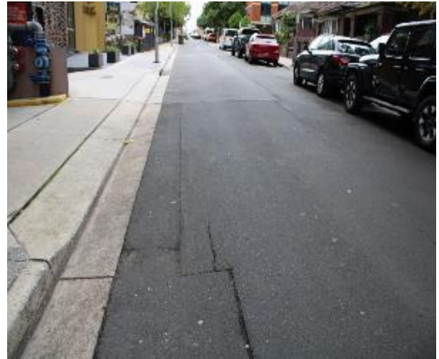
Figure 164 - General condition of road surface heading East
