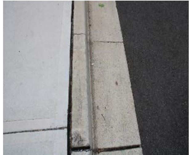
Figure 584 - General condition of kerb and gutter heading North
