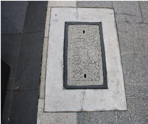
Figure 27 - General condition of service pit
