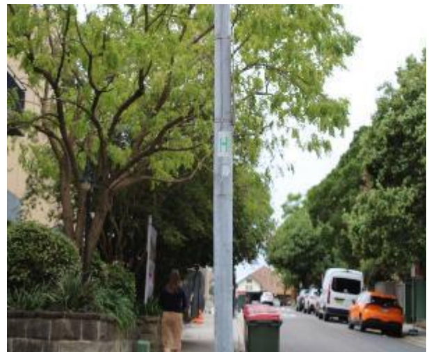
Figure 376 - General condition of street light post Identification No. SVHP62252
