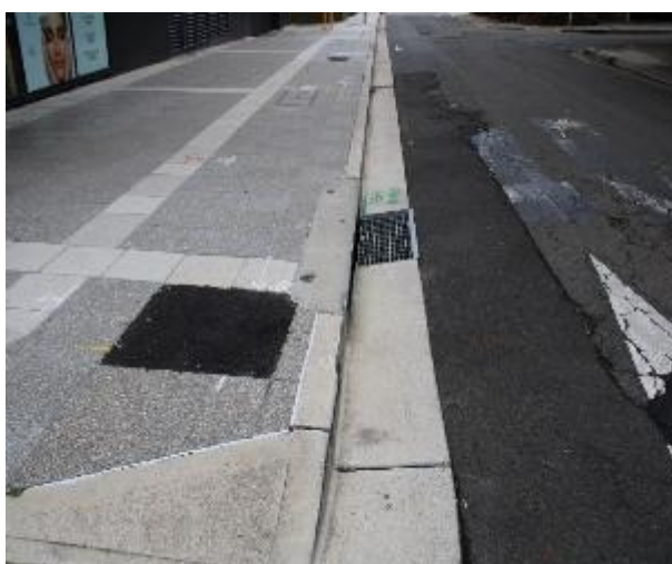
Figure 557 - General condition of kerb and gutter heading North
