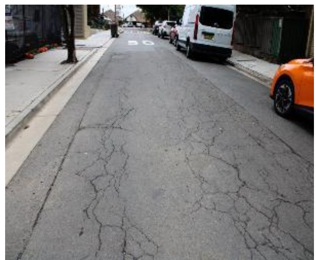
Figure 204 - General condition of road surface heading East
