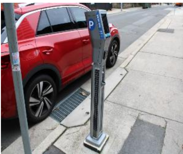
Figure 395 - General condition of parking meter identification No. GEO8
