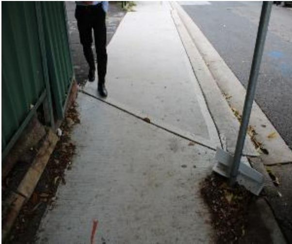
Figure 223 - General condition of footpath pavement heading West
