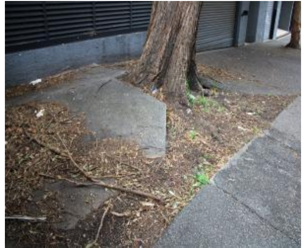
Figure 266 - General condition of footpath pavement heading West
