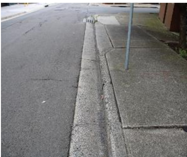
Figure 473 - General condition of kerb and gutter heading North
