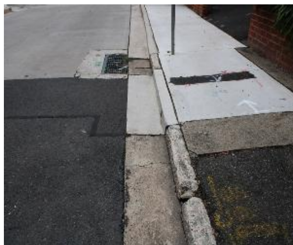
Figure 502 - General condition of kerb and gutter heading North
