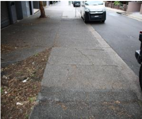
Figure 267 - General condition of footpath pavement heading West
