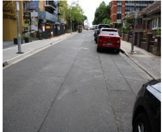
Figure 170 - General condition of road surface heading East
