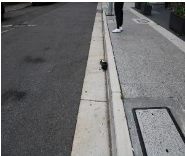
Figure 117 - General condition of kerb and gutter heading West
