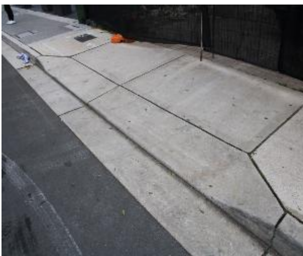
Figure 113 - General condition of driveway layback and gutter heading West
