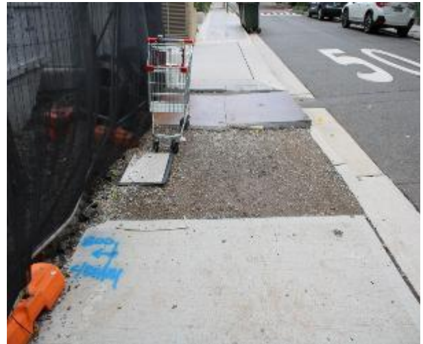
Figure 82 - General condition of footpath pavement heading East
