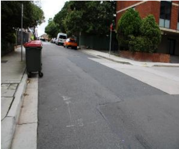
Figure 187 - General condition of road surface heading East
