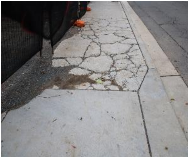
Figure 75 - General condition of footpath pavement heading East
