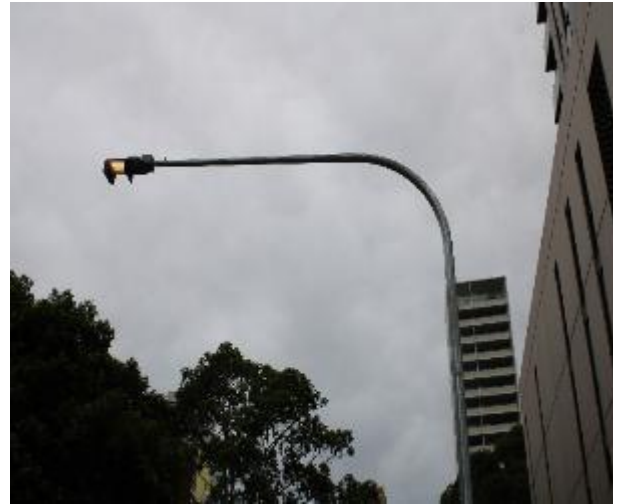
Figure 650 - General condition of street light post identification No. LE32119
