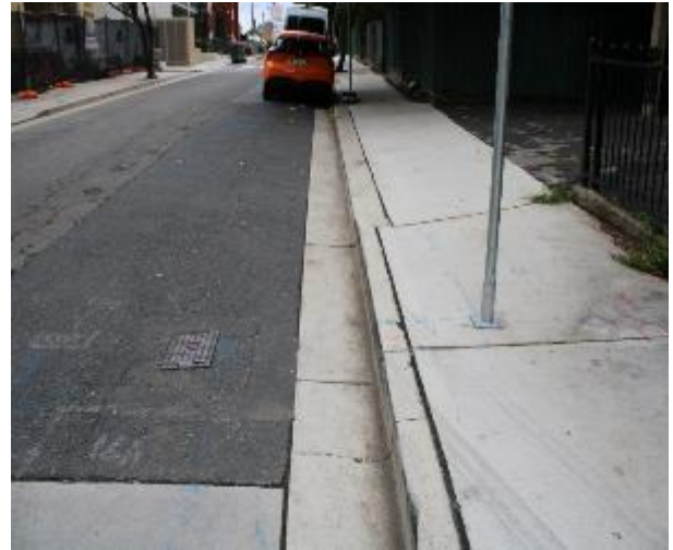
Figure 338 - General condition of kerb and gutter heading East
