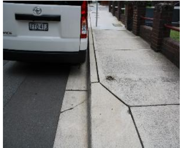
Figure 326 - General condition of kerb and gutter heading East
