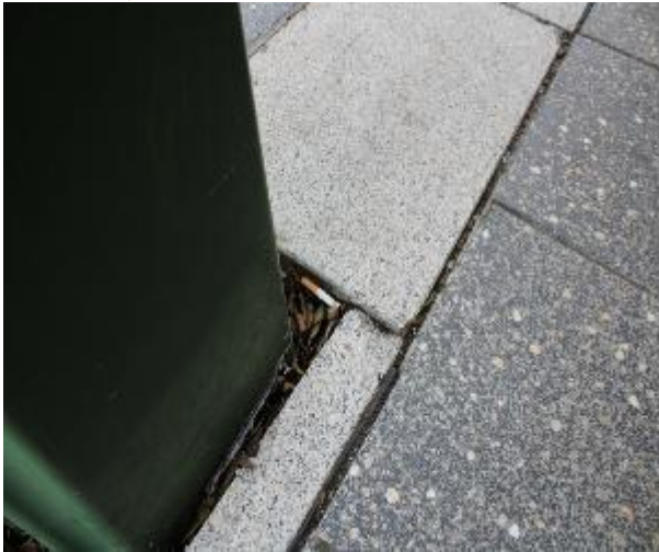
Figure 13 - General condition of footpath pavers heading East
