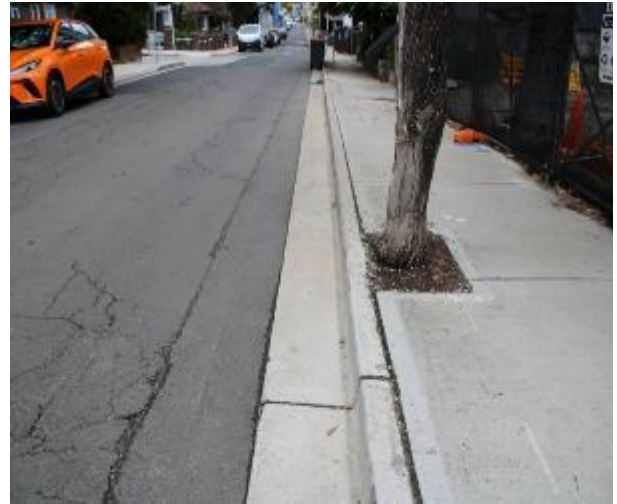
Figure 92 - General condition of kerb and gutter heading West
