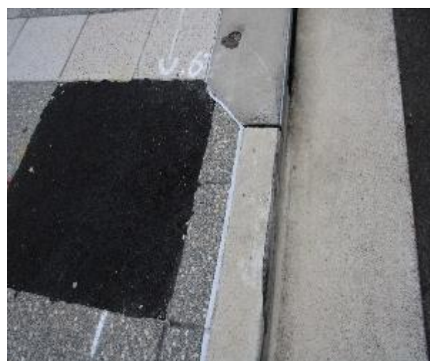
Figure 558 - General condition of kerb and gutter heading North
