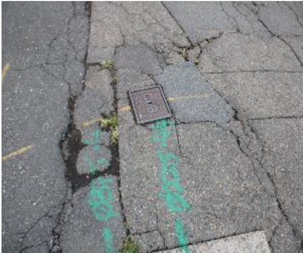
Figure 619 - General condition of service pit
