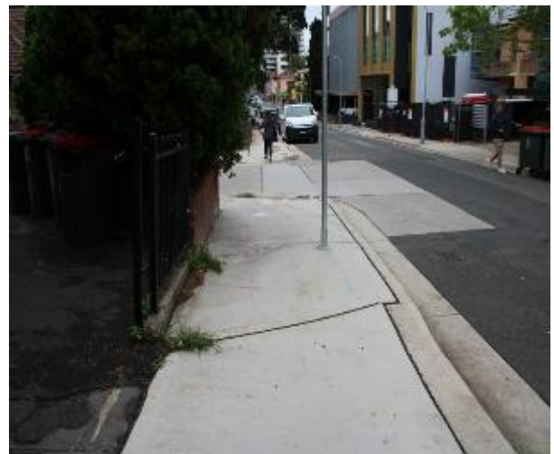
Figure 226 - General condition of footpath pavement heading West
