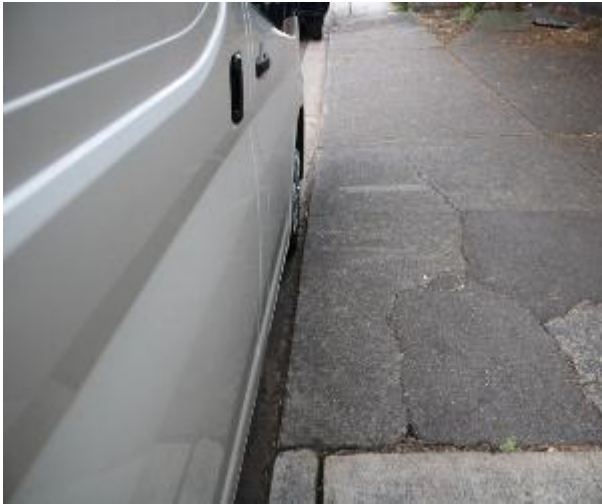
Figure 301 - General condition of kerb and gutter heading East
