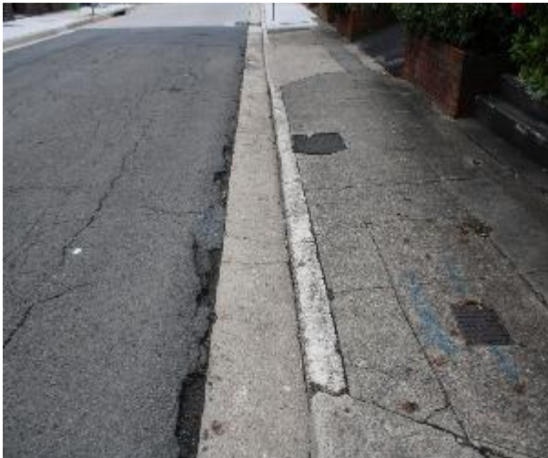
Figure 489 - General condition of kerb and gutter heading North
