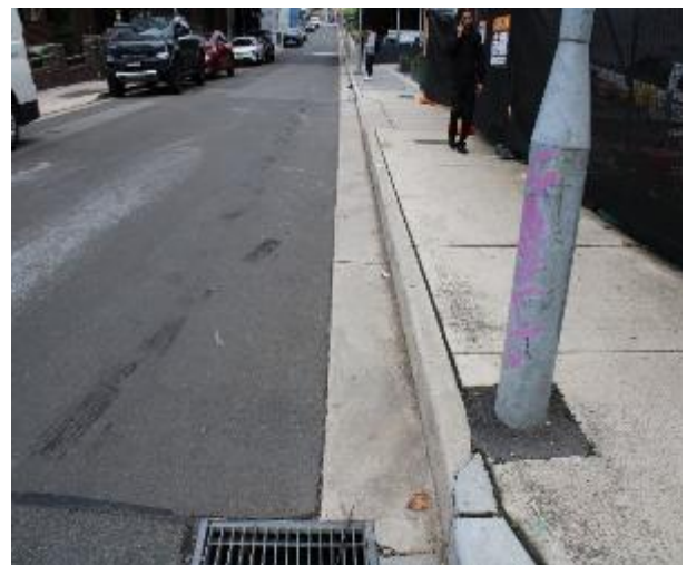
Figure 108 - General condition of kerb and gutter heading West
