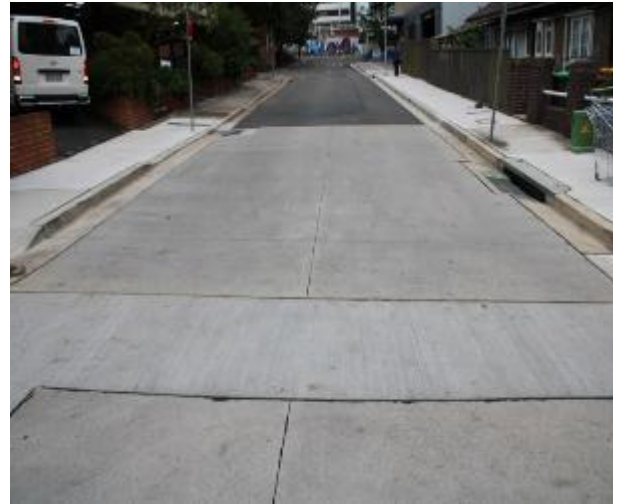
Figure 596 - General condition of road surface heading South
