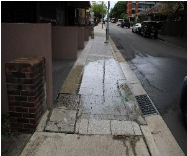
Figure 3 - General condition of footpath pavers heading East
