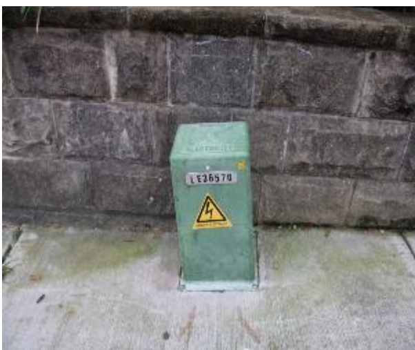
Figure 371 - General condition of electricity box identification No. LE36570
