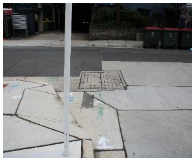
Figure 594 - General condition of kerb and gutter heading North
