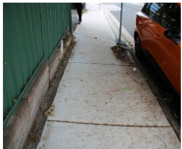
Figure 222 - General condition of footpath pavement heading West
