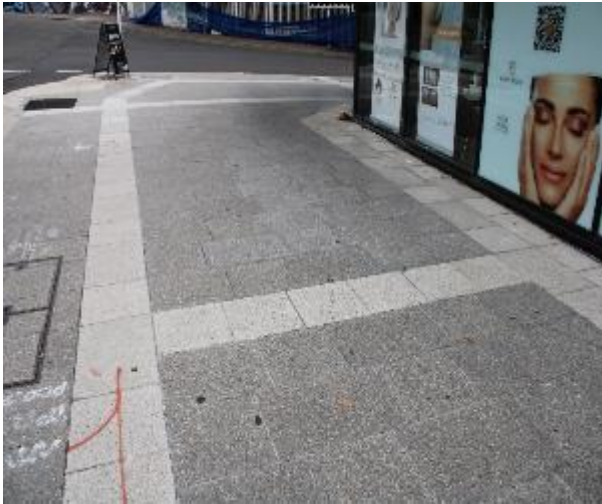
Figure 547 - General condition of footpath pavers heading South
