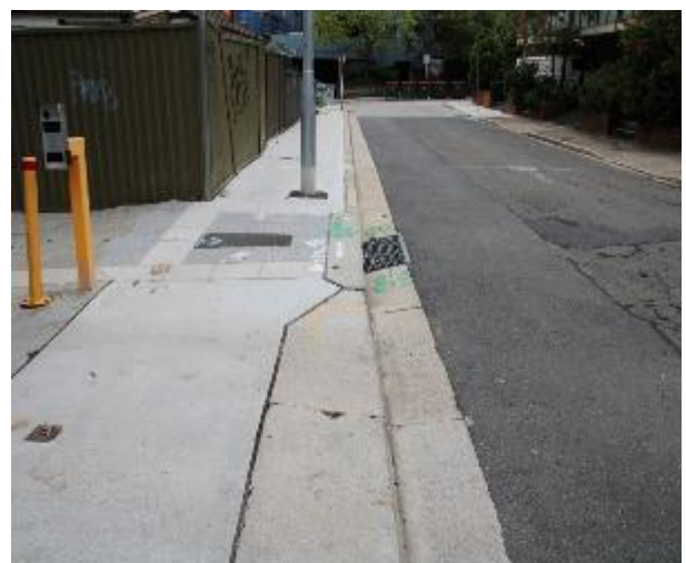
Figure 570 - General condition of driveway layback and gutter heading North
