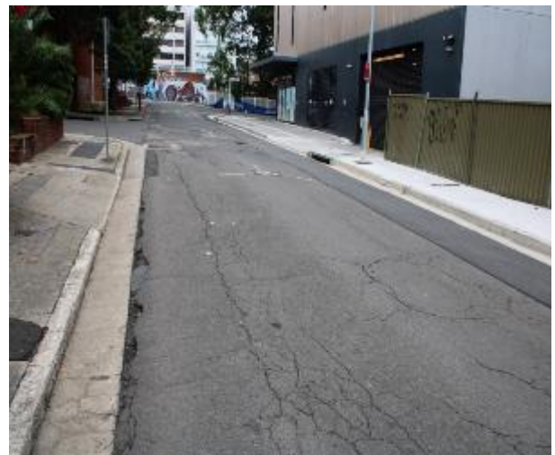
Figure 610 - General condition of road surface heading South
