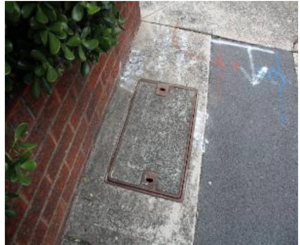
Figure 434 - General condition of service pit
