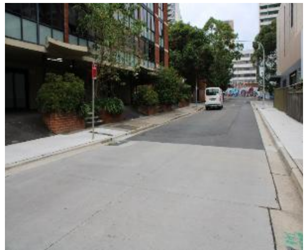
Figure 598 - General condition of road surface heading South
