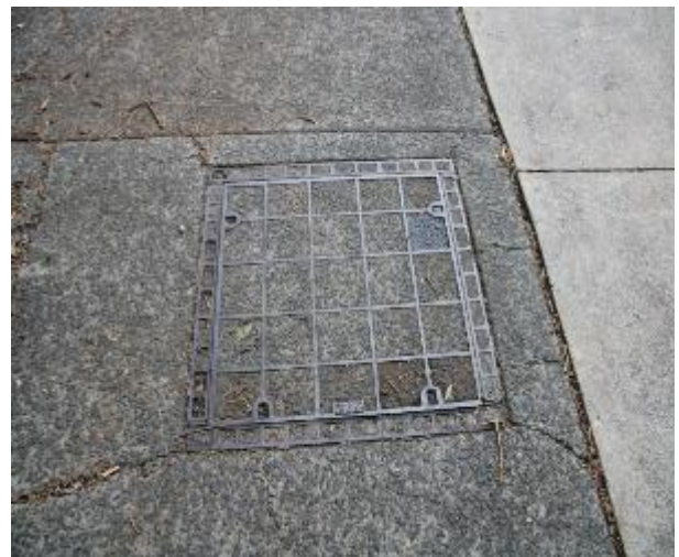
Figure 280 - General condition of service pit
