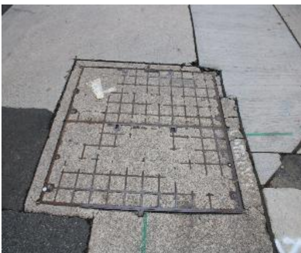
Figure 191 - General condition of service pit
