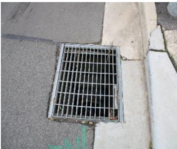
Figure 107 - General condition of stormwater inlet pit
