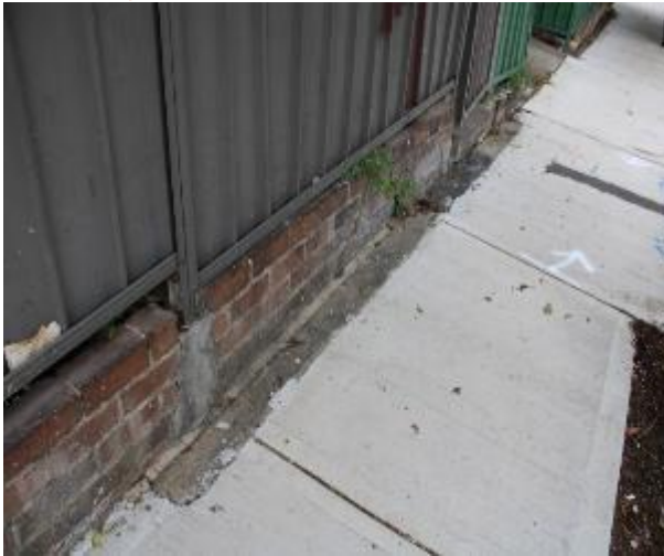
Figure 217 - General condition of footpath pavement heading West
