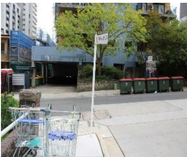
Figure 653 - General condition of street signage
