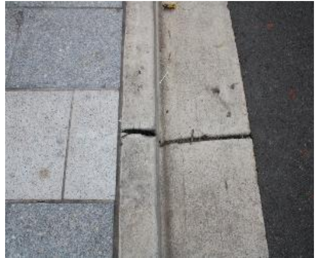
Figure 566 - General condition of kerb and gutter heading North
