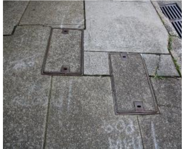
Figure 442 - General condition of service pits
