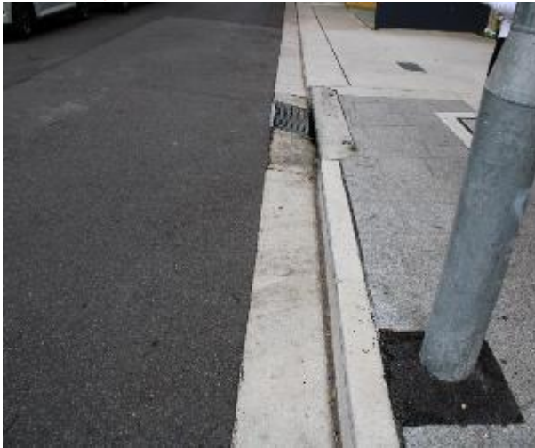
Figure 121 - General condition of kerb and gutter heading West
