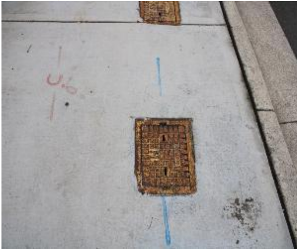
Figure 235 - General condition of service pit
