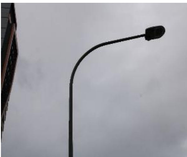
Figure 377 - General condition of street light post Identification No. SVHP62252
