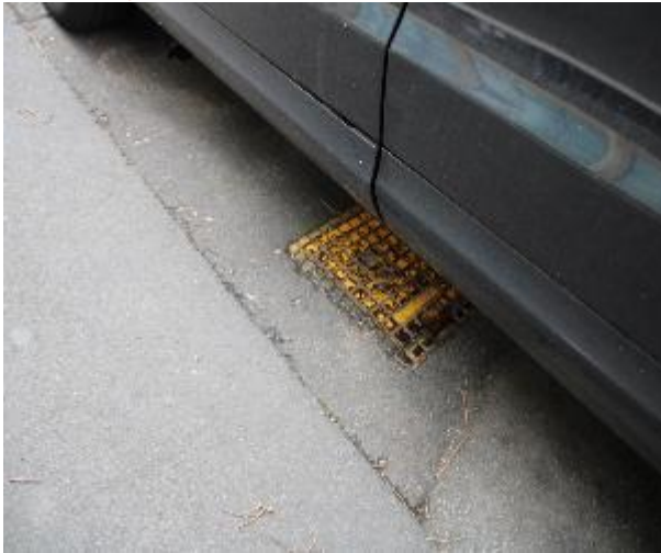
Figure 169 - General condition of service pit
