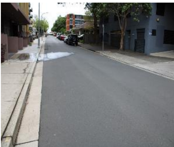
Figure 149 - General condition of road surface heading East
