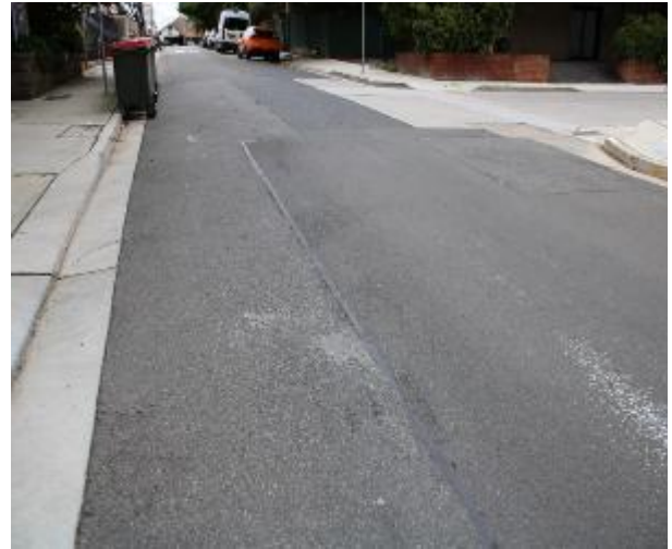
Figure 182 - General condition of road surface heading East
