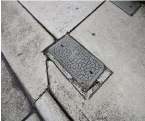
Figure 145 - General condition of service pit
