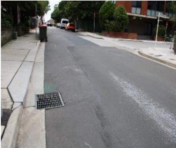
Figure 181 - General condition of road surface heading East
