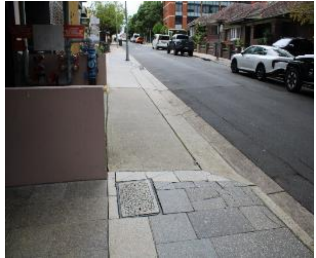
Figure 14 - General condition of footpath pavers heading East
