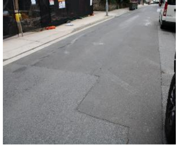
Figure 176 - General condition of road surface heading East
