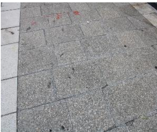
Figure 539 - General condition of footpath pavers heading South
