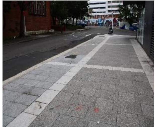
Figure 542 - General condition of footpath pavers heading South
