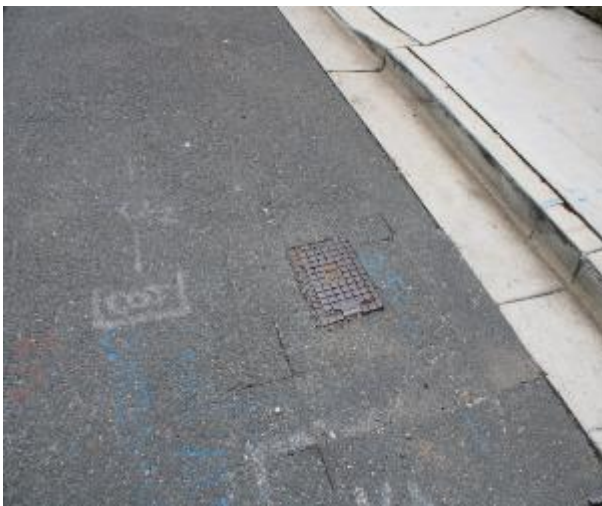
Figure 195 - General condition of service pit
