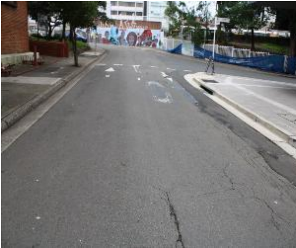
Figure 631 - General condition of road surface heading South
