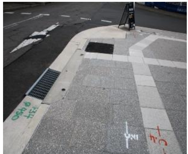
Figure 550 - General condition of footpath pavers heading South
