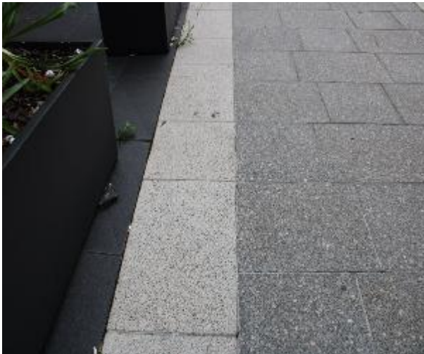
Figure 33 - General condition of footpath pavers heading East
