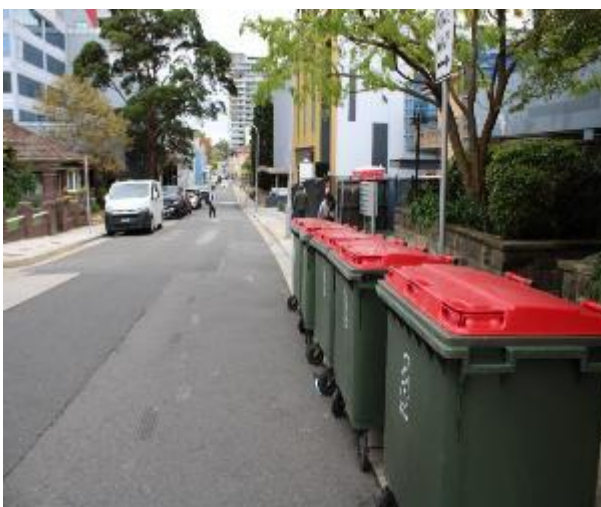
Figure 101 - General condition of kerb and gutter heading West
