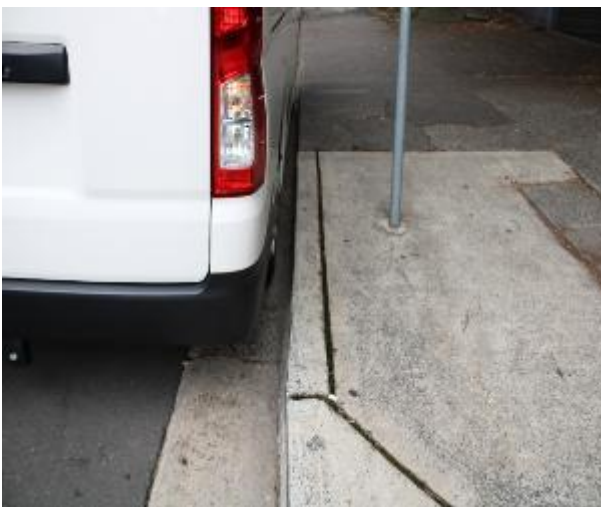
Figure 299 - General condition of kerb and gutter heading East
