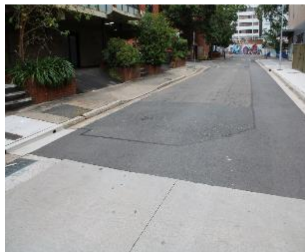
Figure 600 - General condition of road surface heading South
