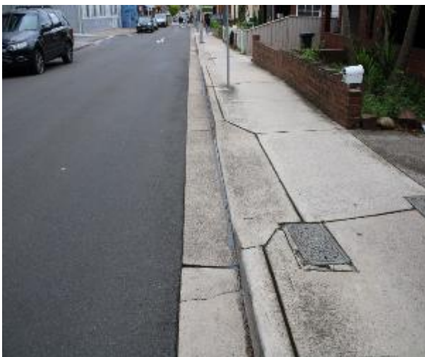
Figure 143 - General condition of kerb and gutter heading West
