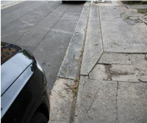
Figure 313 - General condition of kerb and gutter heading East
