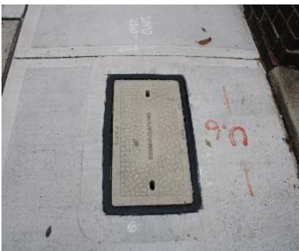
Figure 515 - General condition of service pit
