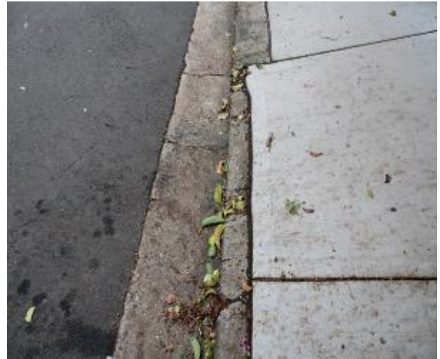
Figure 350 - General condition of kerb and gutter heading East
