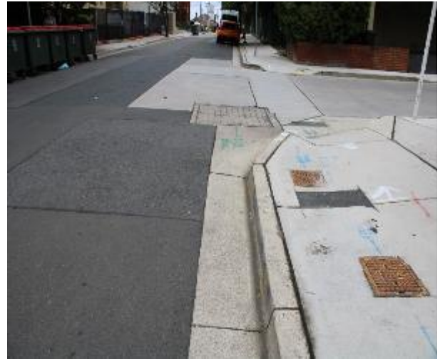
Figure 332 - General condition of kerb and gutter heading East
