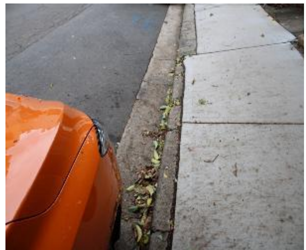
Figure 348 - General condition of kerb and gutter heading East
