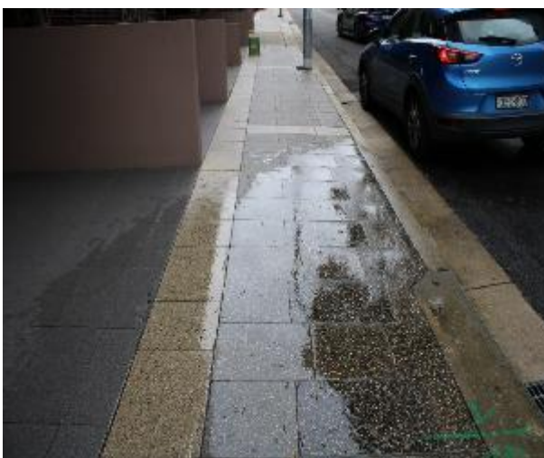
Figure 5 - General condition of footpath pavers heading East
