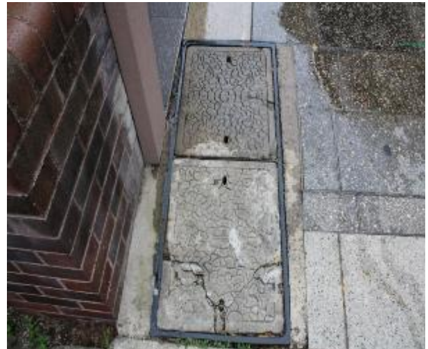
Figure 4 - General condition of service pit
