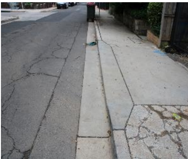
Figure 95 - General condition of driveway layback and gutter heading West
