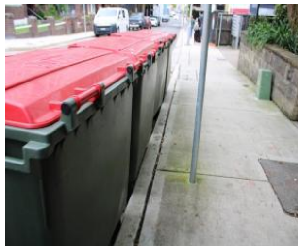
Figure 102 - General condition of kerb and gutter heading West
