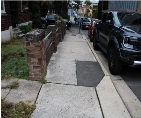
Figure 247 - General condition of footpath pavement heading West
