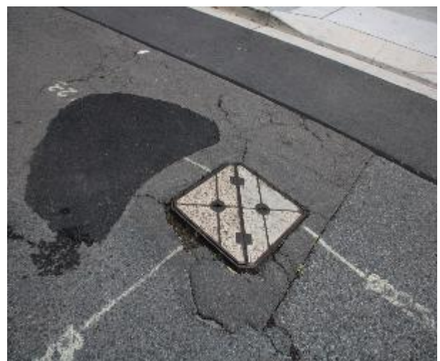
Figure 624 - General condition of service pit
