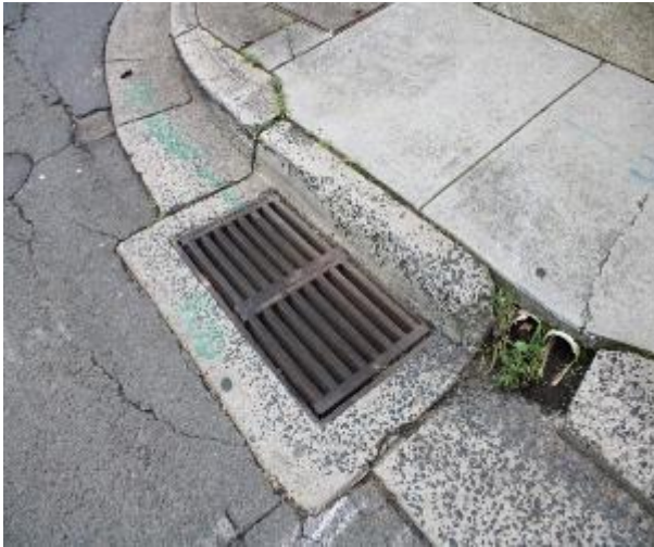
Figure 481 - General condition of stormwater inlet pit
