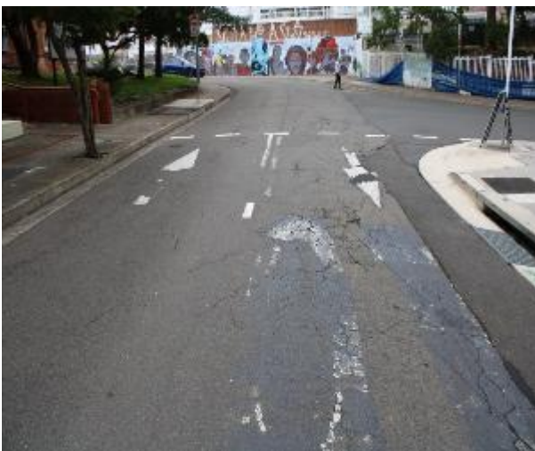
Figure 635 - General condition of road surface heading South
