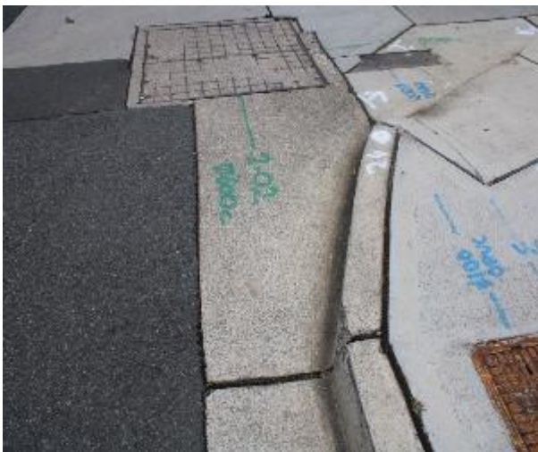
Figure 333 - General condition of kerb and gutter heading East
