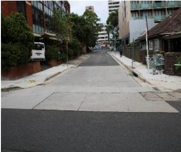
Figure 595 - General condition of road surface heading South
