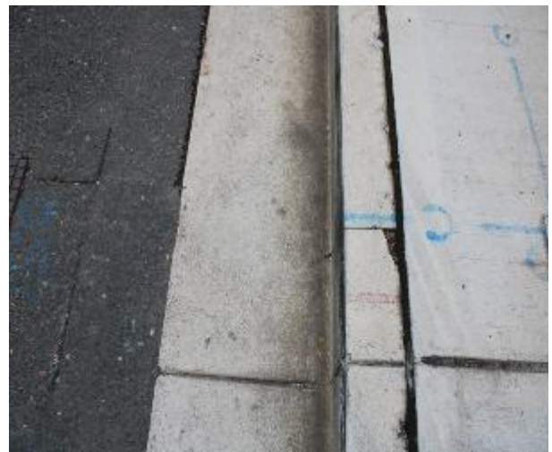
Figure 340 - General condition of kerb and gutter heading East
