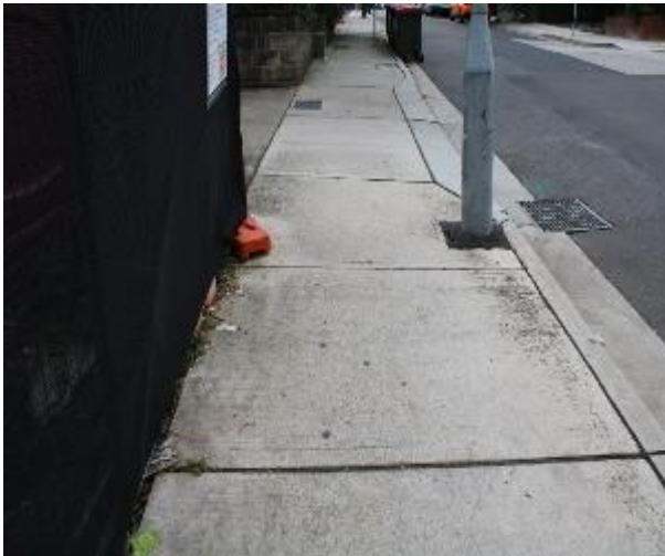
Figure 51 - General condition of footpath pavement heading East
