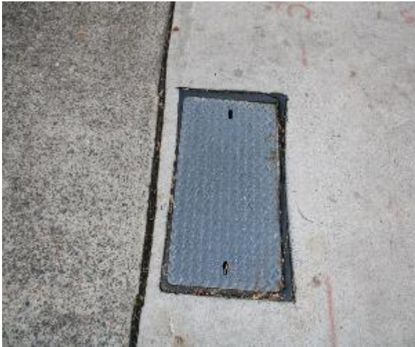
Figure 55 - General condition of service pit
