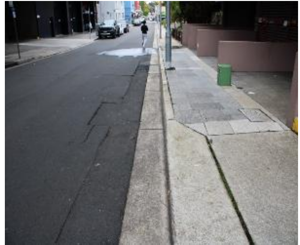
Figure 128 - General condition of kerb and gutter heading West
