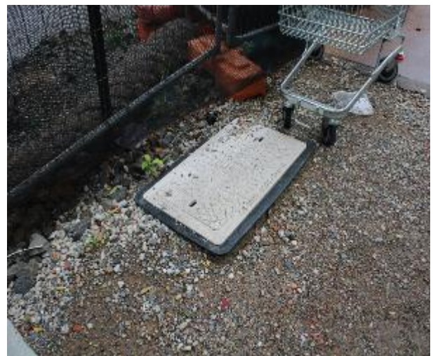
Figure 84 - General condition of service pit
