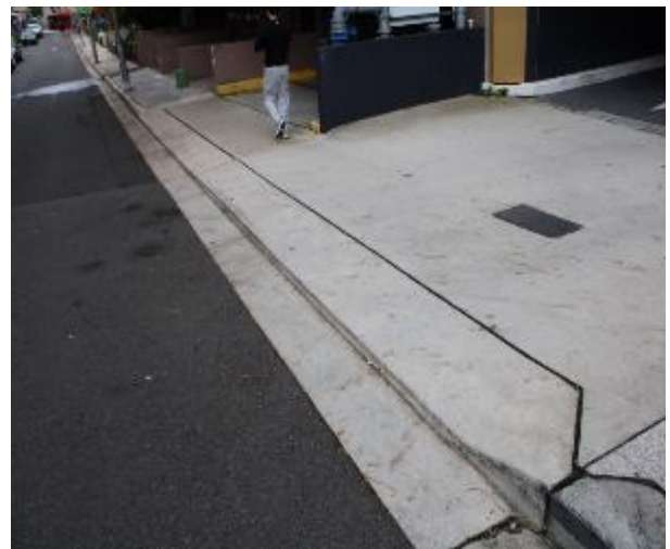
Figure 124 - General condition of driveway layback and gutter heading West
