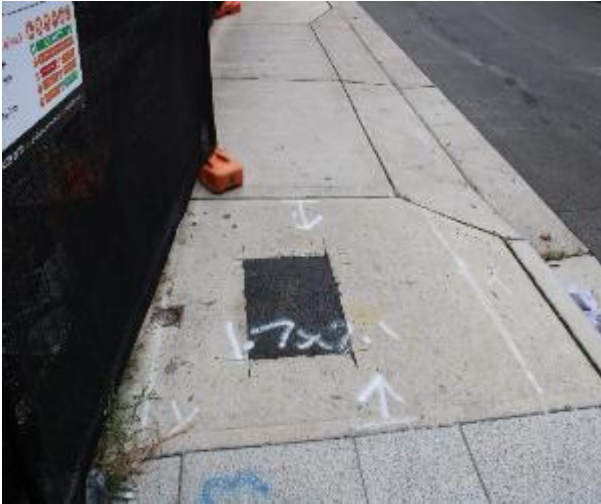
Figure 39 - General condition of footpath pavers heading East
