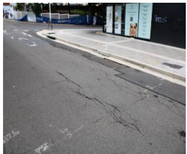
Figure 630 - General condition of road surface heading South
