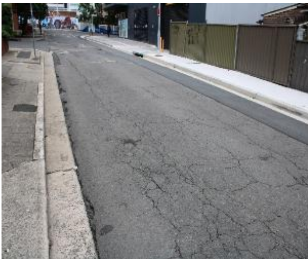
Figure 609 - General condition of road surface heading South
