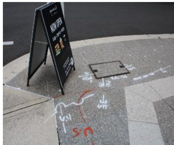
Figure 554 - General condition of footpath pavers heading South
