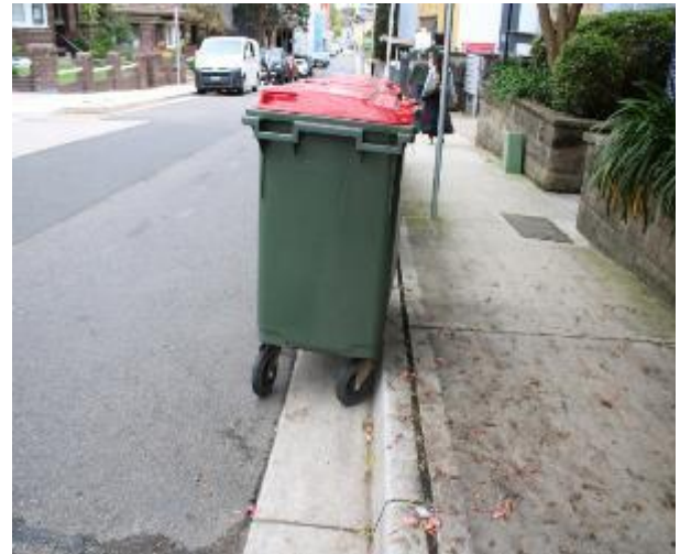
Figure 100 - General condition of kerb and gutter heading West
