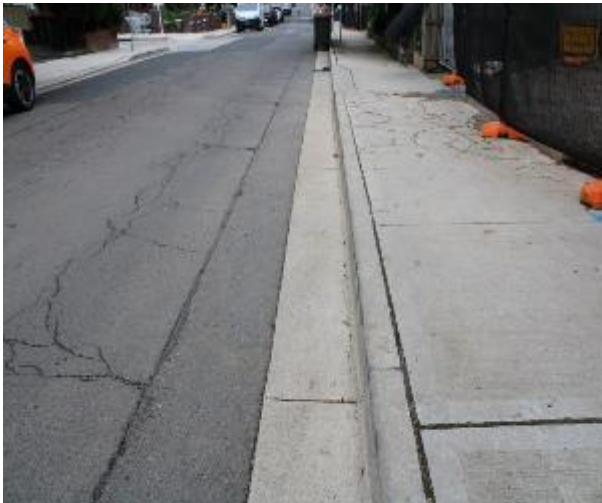
Figure 93 - General condition of kerb and gutter heading West
