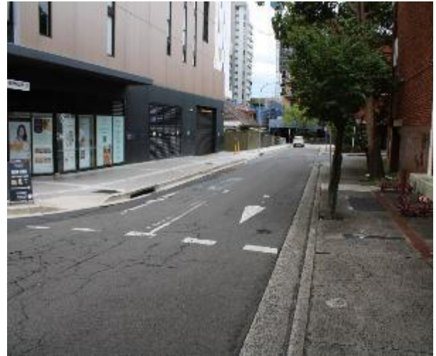
Figure 464 - General condition of kerb and gutter heading North
