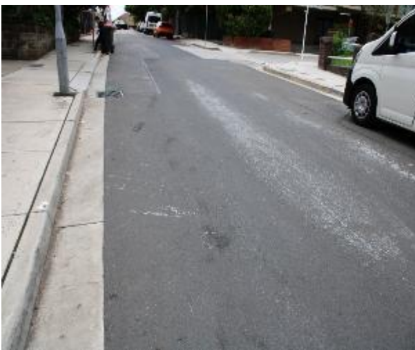
Figure 179 - General condition of road surface heading East
