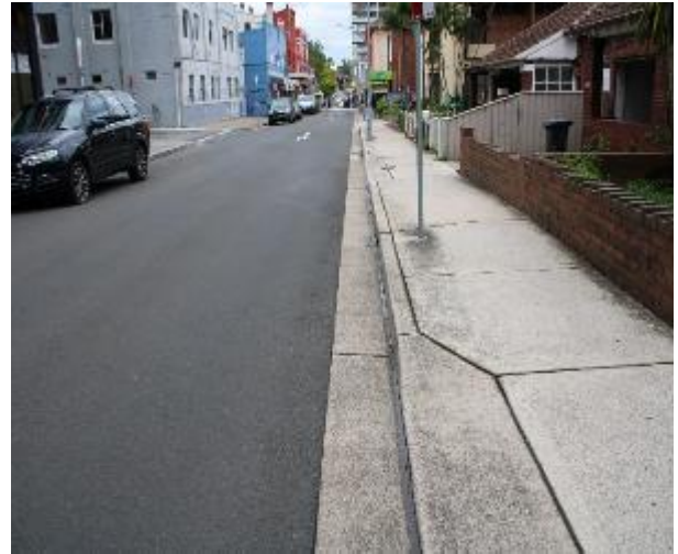
Figure 146 - General condition of kerb and gutter heading West
