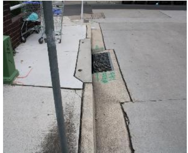
Figure 590 - General condition of kerb and gutter heading North
