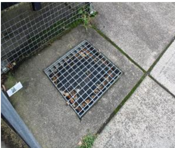
Figure 53 - General condition of stormwater inlet pit
