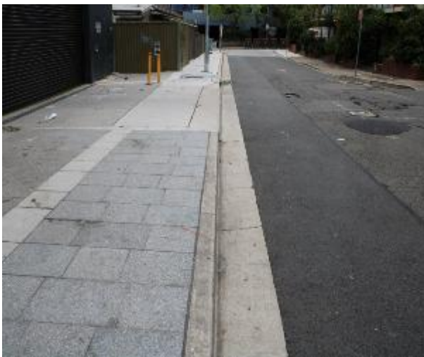
Figure 567 - General condition of kerb and gutter heading North
