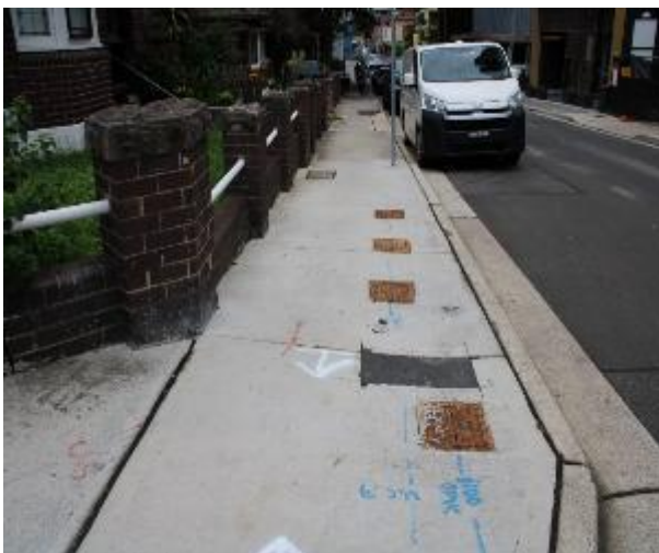
Figure 233 - General condition of footpath pavement heading West
