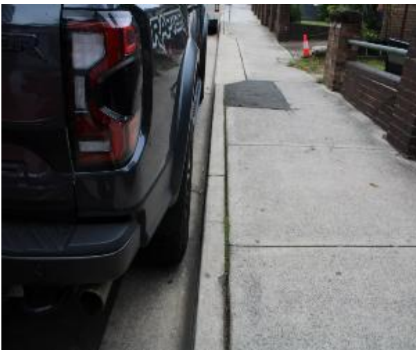
Figure 321 - General condition of kerb and gutter heading East
