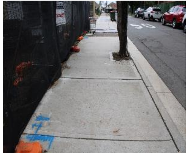
Figure 80 - General condition of footpath pavement heading East
