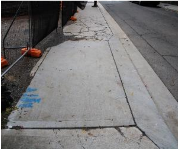
Figure 73 - General condition of footpath pavement heading East
