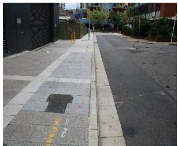
Figure 564 - General condition of kerb and gutter heading North
