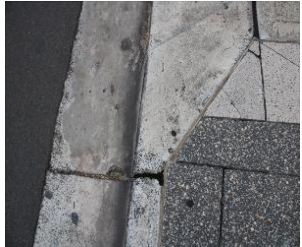
Figure 290 - General condition of kerb and gutter heading East
