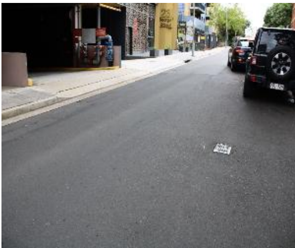
Figure 159 - General condition of road surface heading East
