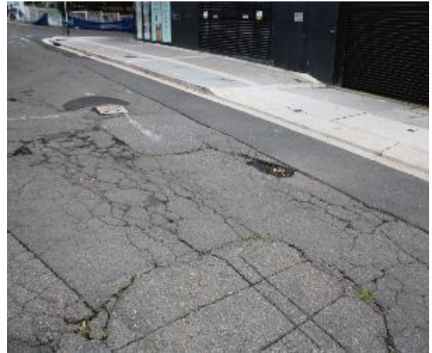
Figure 620 - General condition of road surface heading South
