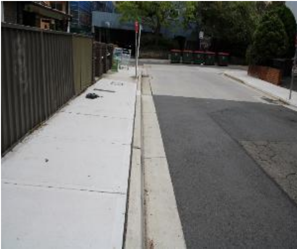
Figure 583 - General condition of kerb and gutter heading North
