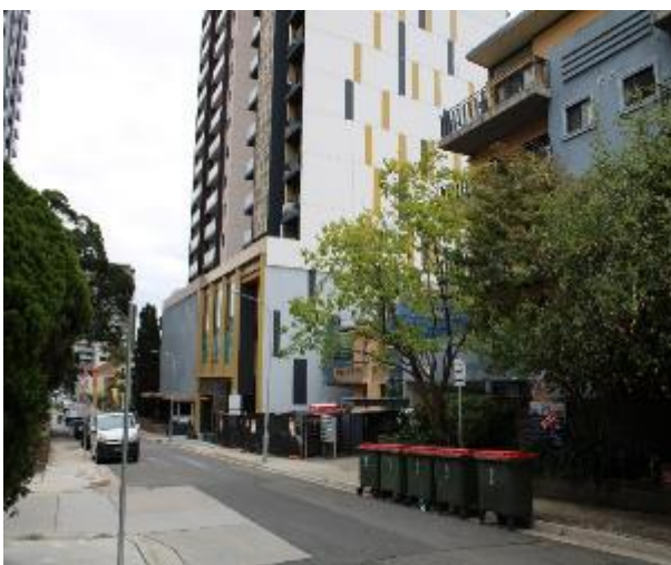
Figure 365 - General condition of street tree
