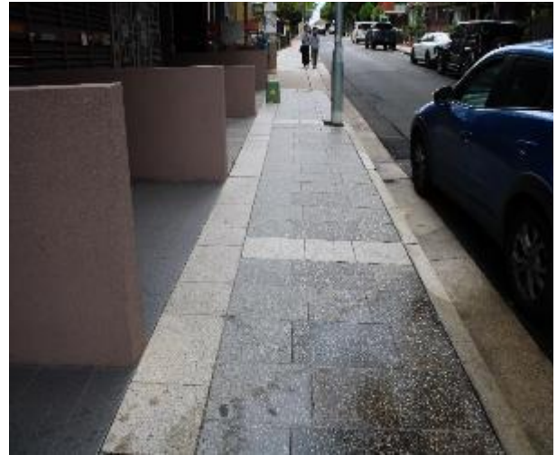
Figure 8 - General condition of footpath pavers heading East
