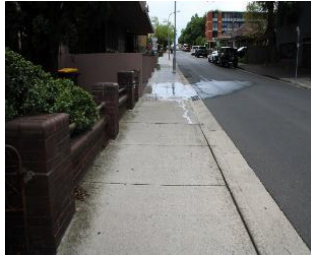
Figure 2 - General condition of footpath pavement heading East
