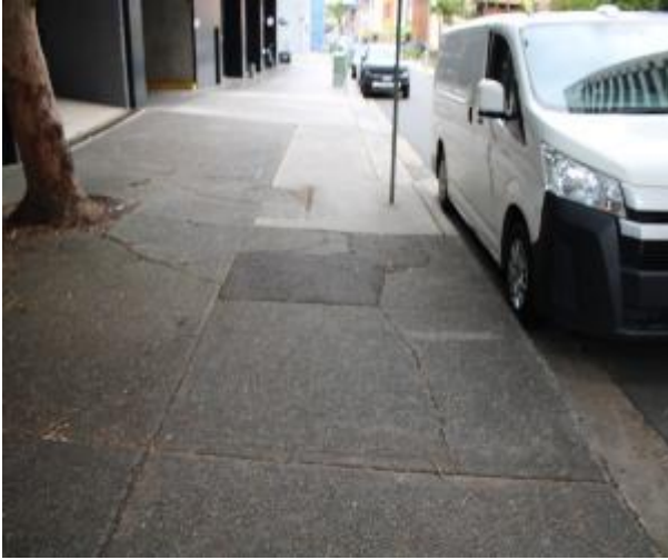
Figure 271 - General condition of footpath pavement heading West
