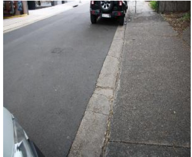
Figure 302 - General condition of kerb and gutter heading East
