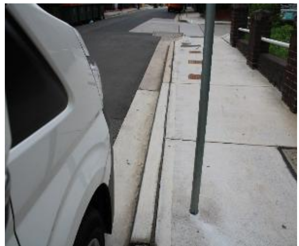
Figure 330 - General condition of kerb and gutter heading East
