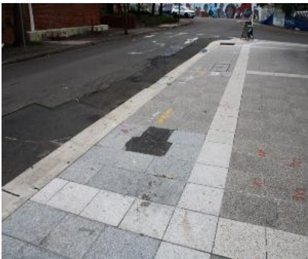
Figure 543 - General condition of footpath pavers heading South
