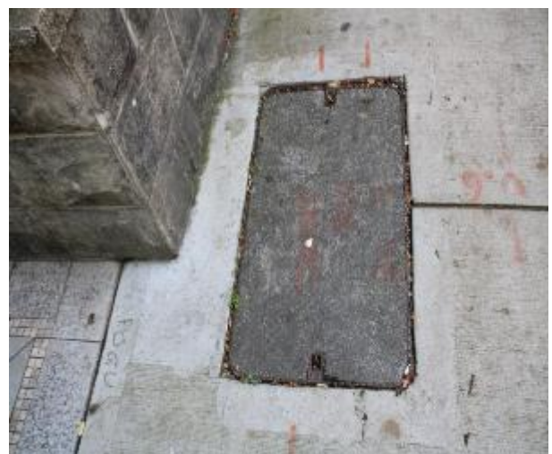
Figure 60 - General condition of service pit
