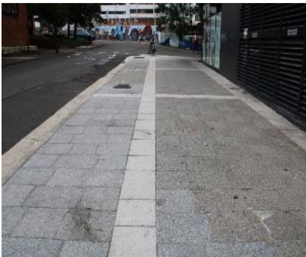
Figure 537 - General condition of footpath pavers heading South
