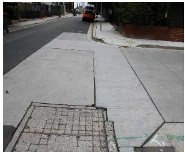
Figure 334 - General condition of road surface heading East
