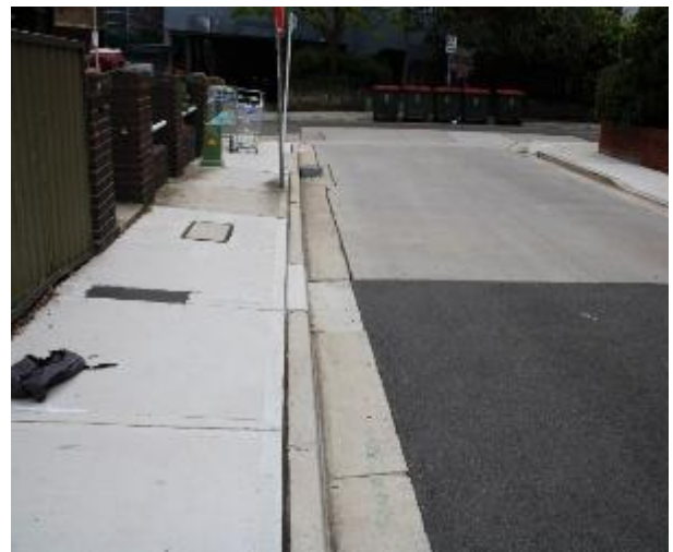
Figure 586 - General condition of kerb and gutter heading North
