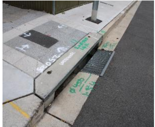
Figure 572 - General condition of stormwater inlet pit
