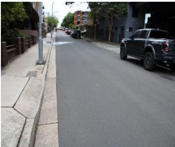
Figure 147 - General condition of road surface heading East
