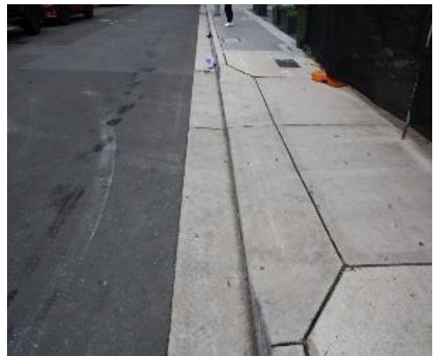
Figure 112 - General condition of driveway layback and gutter heading West
