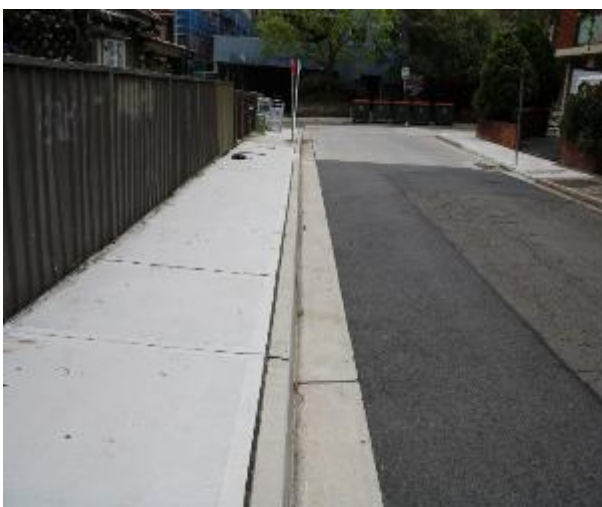
Figure 581 - General condition of kerb and gutter heading North
