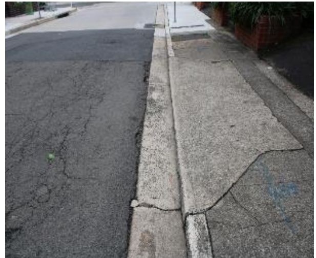
Figure 496 - General condition of driveway layback and gutter heading North
