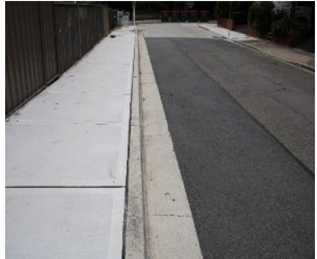
Figure 578 - General condition of kerb and gutter heading North
