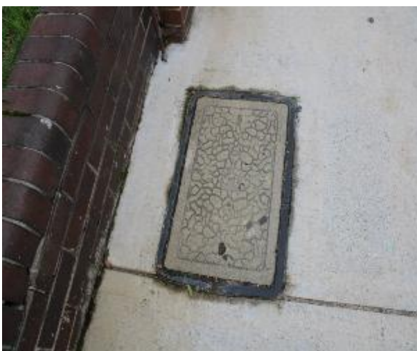
Figure 239 - General condition of service pit
