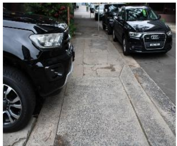
Figure 258 - General condition of footpath pavement heading West
