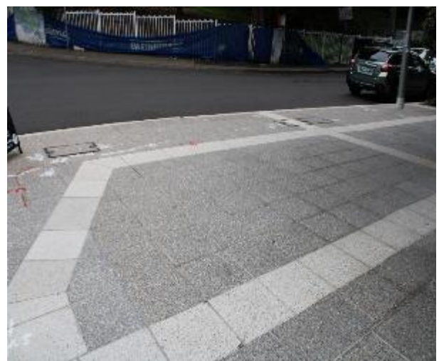
Figure 552 - General condition of footpath pavers heading South
