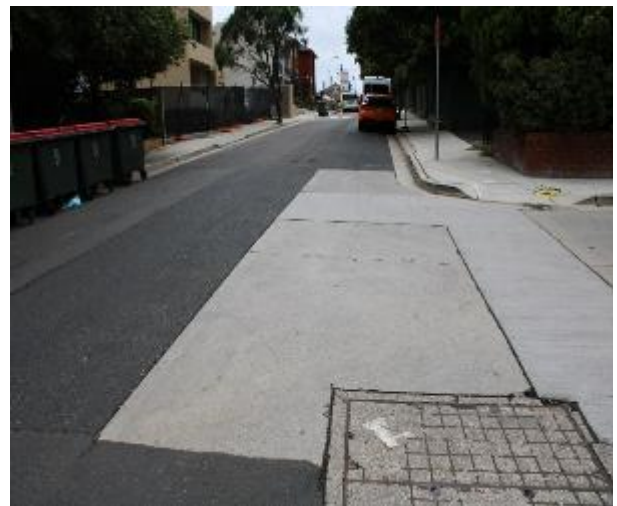
Figure 190 - General condition of road surface heading East
