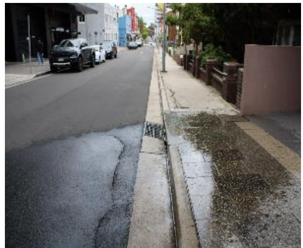
Figure 136 - General condition of kerb and gutter heading West
