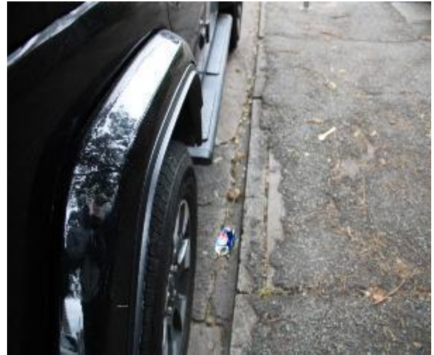
Figure 308 - General condition of kerb and gutter heading East
