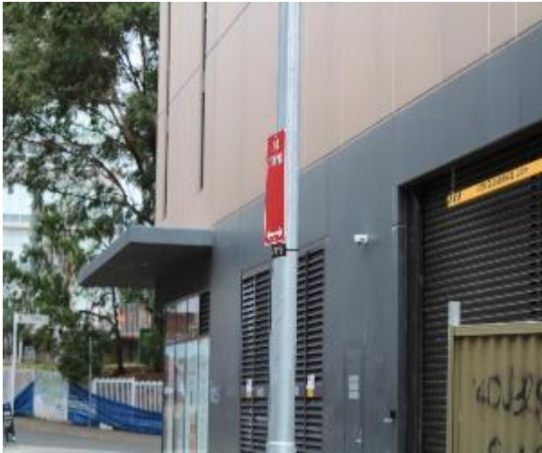
Figure 649 - General condition of street light post identification No. LE32119
