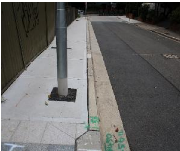
Figure 573 - General condition of kerb and gutter heading North
