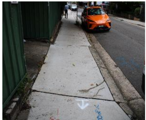
Figure 220 - General condition of footpath pavement heading West
