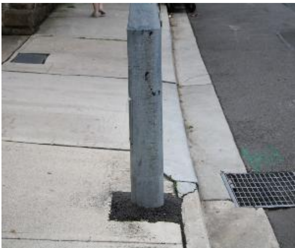
Figure 375 - General condition of street light post Identification No. SVHP62252
