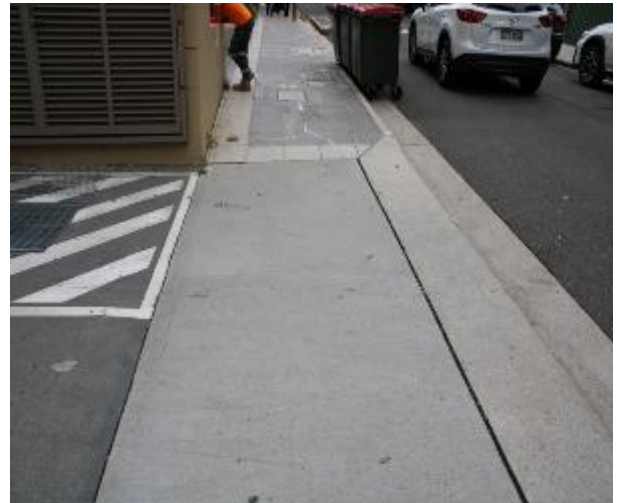
Figure 88 - General condition of footpath pavement heading East
