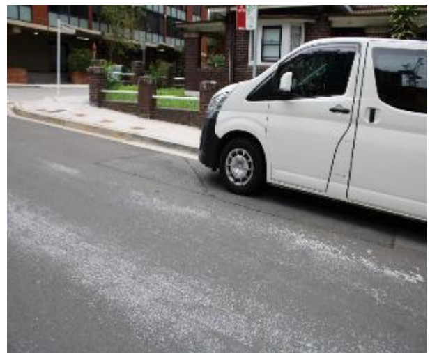
Figure 180 - General condition of road surface heading East
