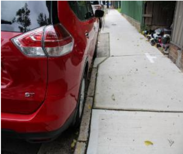
Figure 361 - General condition of kerb and gutter heading East
