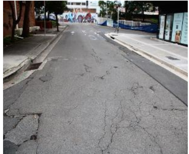
Figure 626 - General condition of road surface heading South
