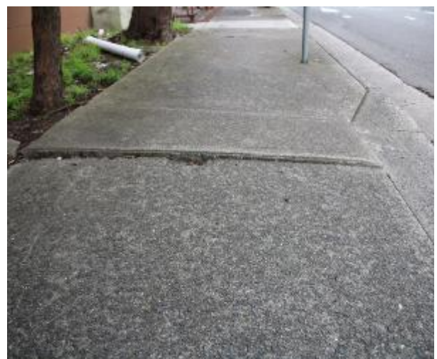
Figure 450 - Differential settlement evident through footpath pavement heading South
