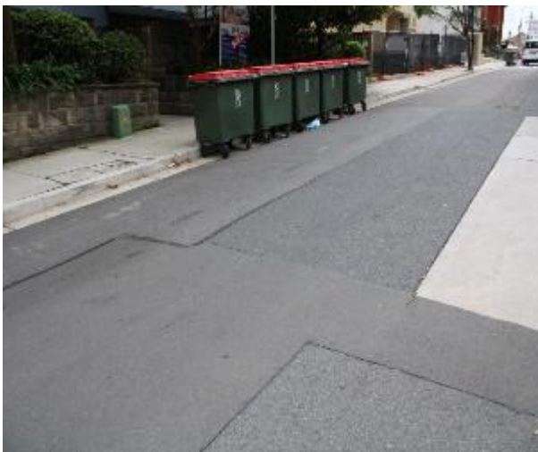
Figure 189 - General condition of road surface heading East
