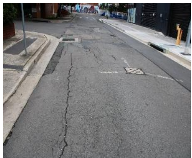
Figure 612 - General condition of road surface heading South
