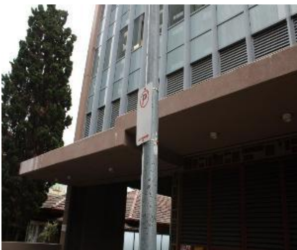
Figure 389 - General condition of streetlight post
