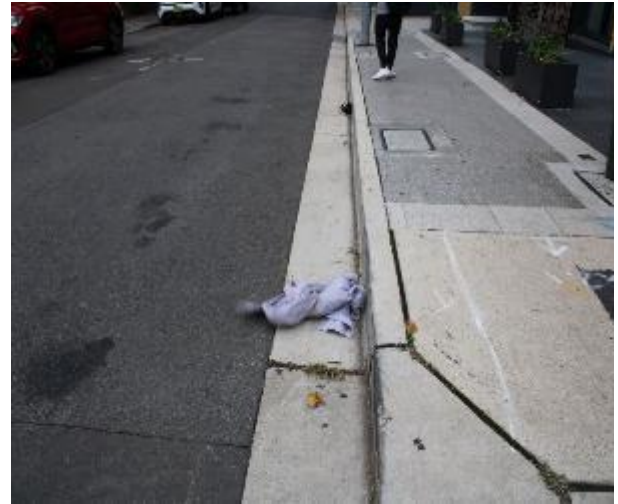
Figure 116 - General condition of kerb and gutter heading West
