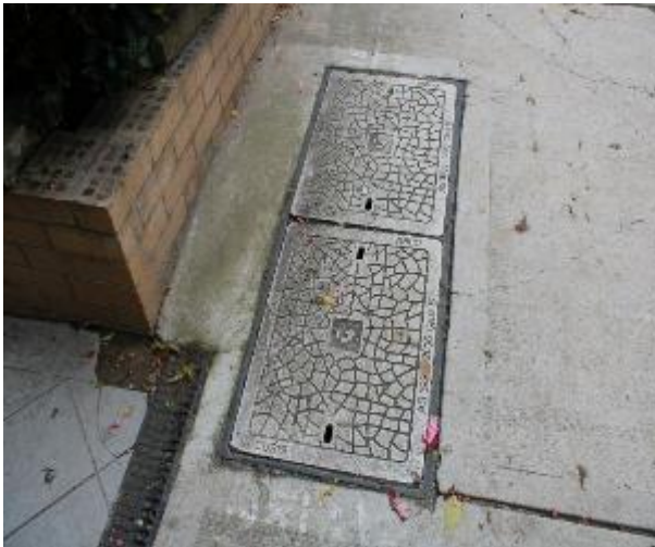
Figure 69 - General condition of service pit
