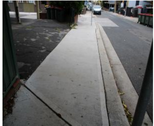
Figure 224 - General condition of footpath pavement heading West
