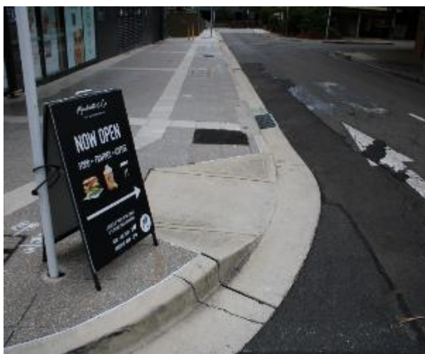
Figure 555 - General condition of kerb and gutter heading North
