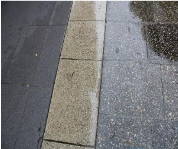
Figure 7 - General condition of footpath pavers heading East
