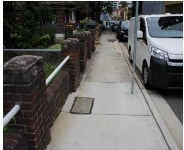
Figure 238 - General condition of footpath pavement heading West
