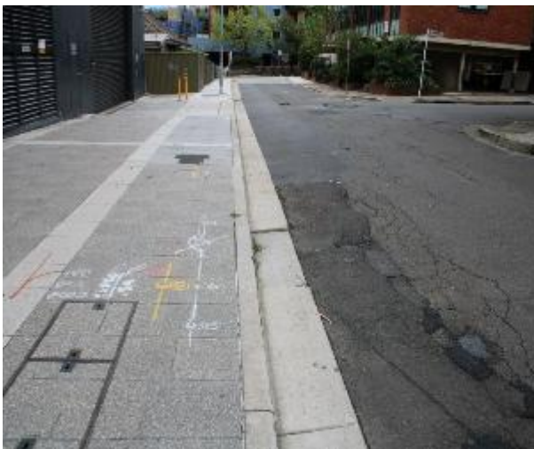
Figure 561 - General condition of kerb and gutter heading North
