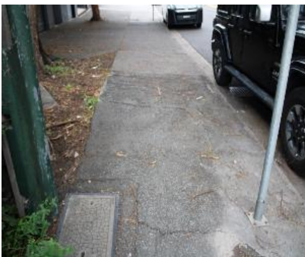
Figure 263 - General condition of footpath pavement heading West
