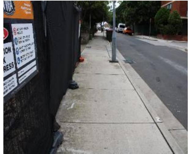
Figure 50 - General condition of footpath pavement heading East
