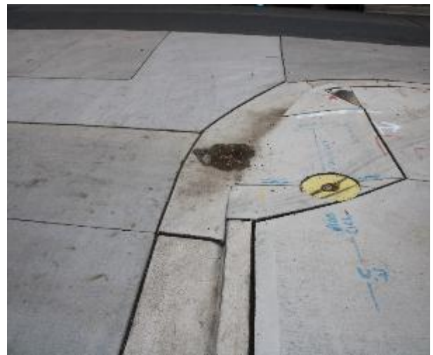
Figure 508 - General condition of kerb and gutter heading North
