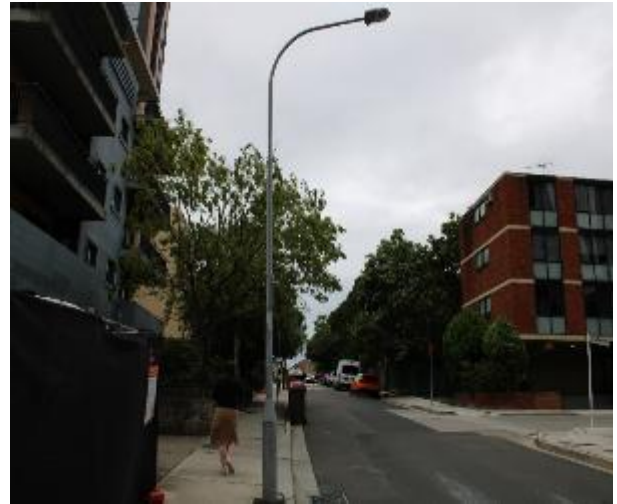
Figure 374 - General condition of street light post Identification No. SVHP62252
