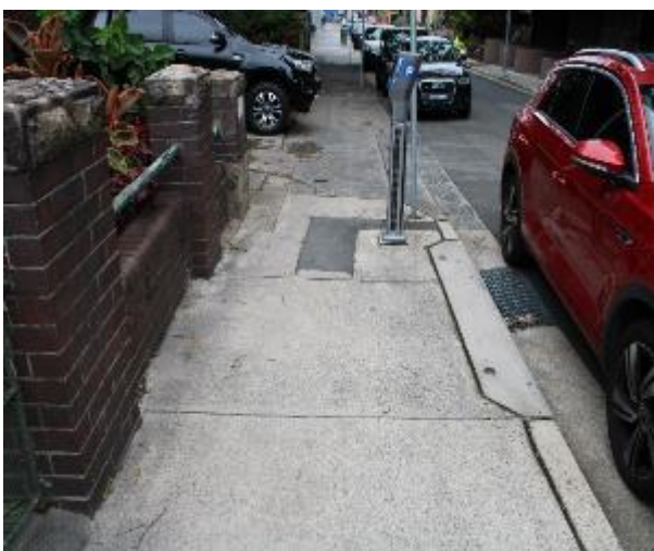
Figure 251 - General condition of footpath pavement heading West
