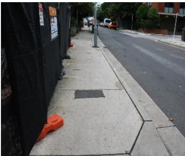
Figure 47 - General condition of footpath pavement heading East
