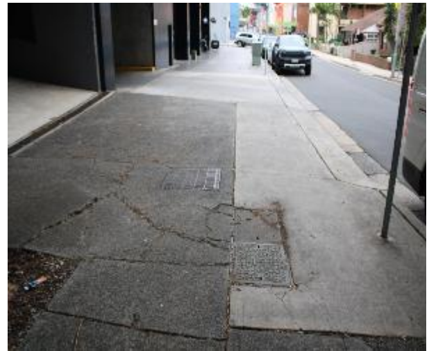
Figure 274 - General condition of footpath pavement heading West
