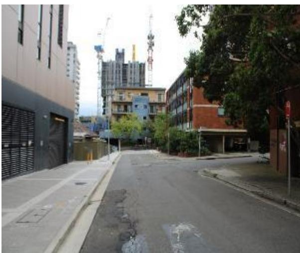
Figure 641 - General condition of road surface
