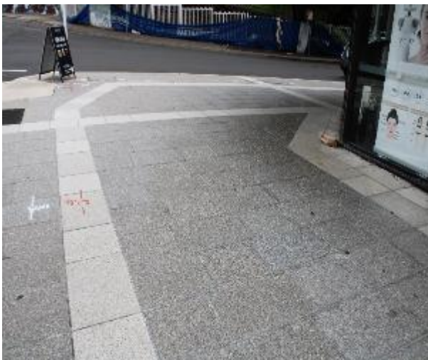
Figure 549 - General condition of footpath pavers heading South
