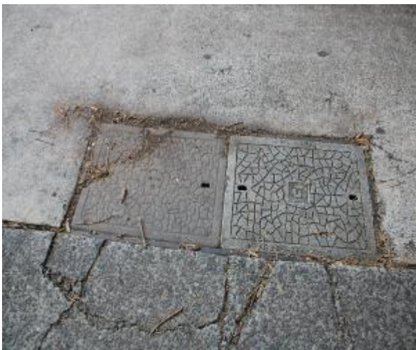
Figure 279 - General condition of service pit
