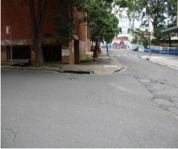
Figure 439 - General condition of road surface heading South
