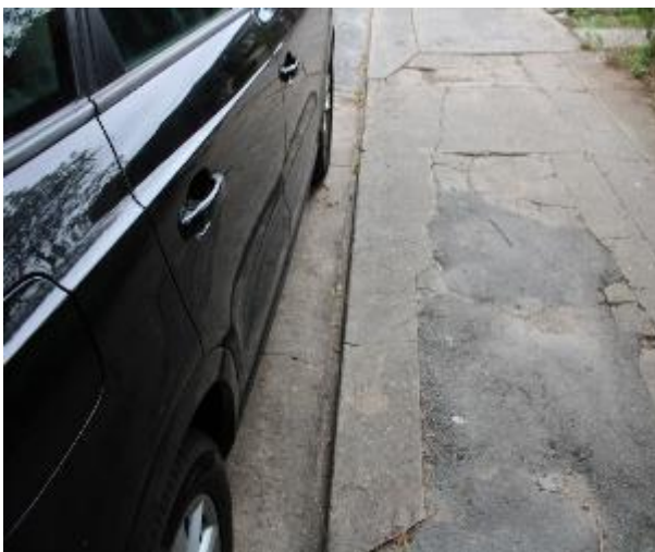
Figure 311 - General condition of kerb and gutter heading East
