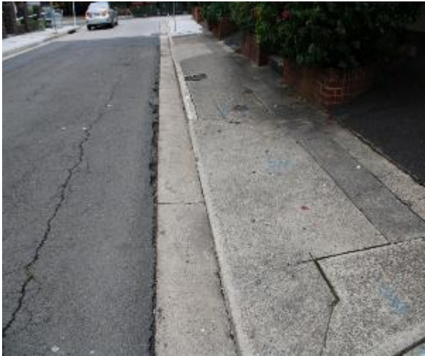
Figure 487 - General condition of kerb and gutter heading North
