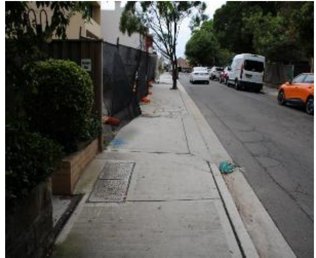
Figure 68 - General condition of footpath pavement heading East
