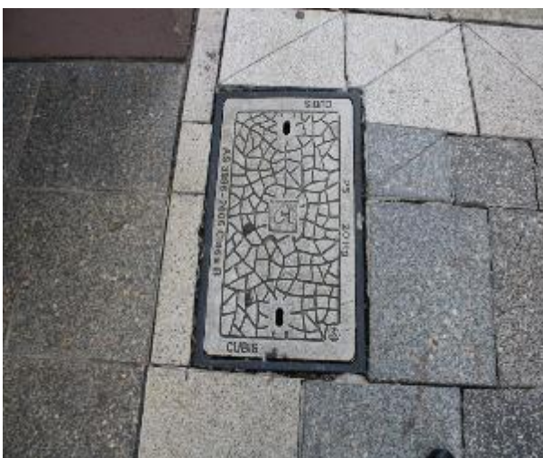
Figure 17 - General condition of service pit
