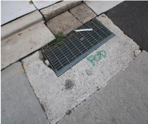
Figure 601 - General condition of stormwater inlet pit
