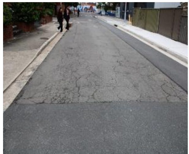
Figure 606 - General condition of road surface heading South
