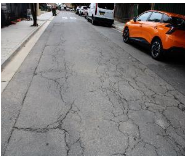
Figure 203 - General condition of road surface heading East
