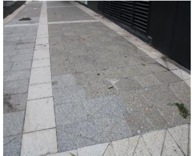
Figure 536 - General condition of footpath pavers heading South
