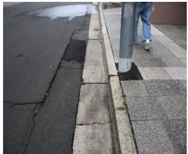
Figure 130 - General condition of kerb and gutter heading West
