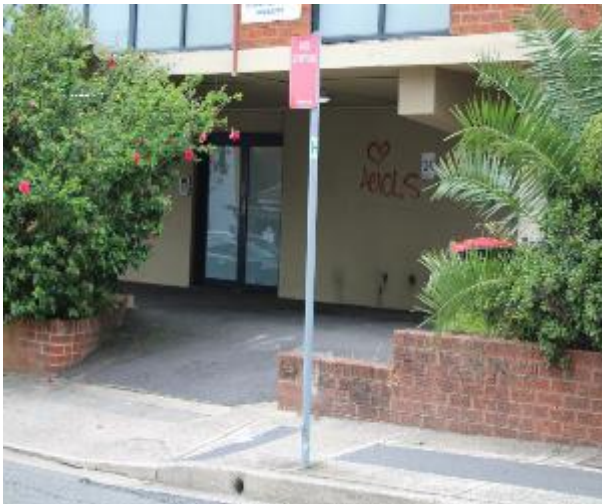
Figure 645 - General condition of street signage
