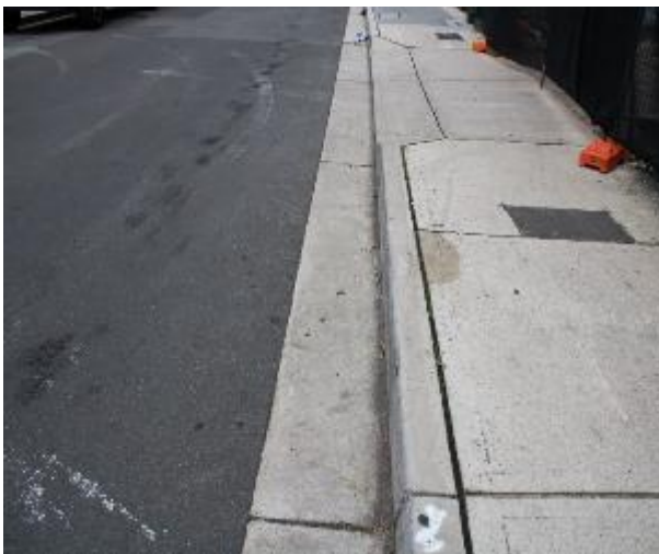
Figure 111 - General condition of kerb and gutter heading West
