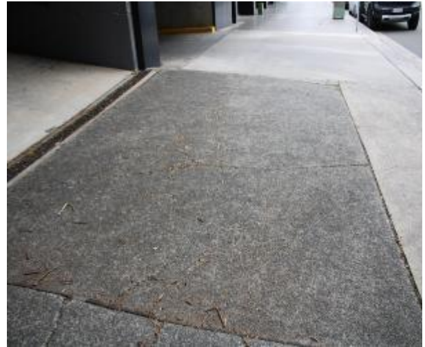
Figure 278 - General condition of footpath pavement heading West
