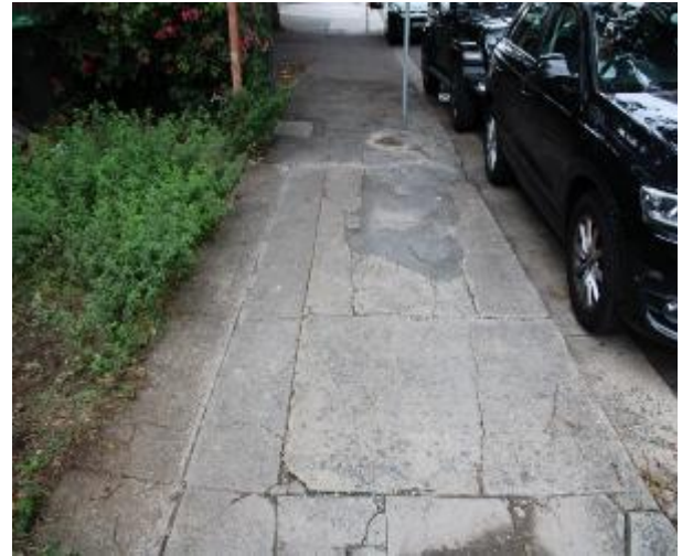
Figure 260 - General condition of footpath pavement heading West
