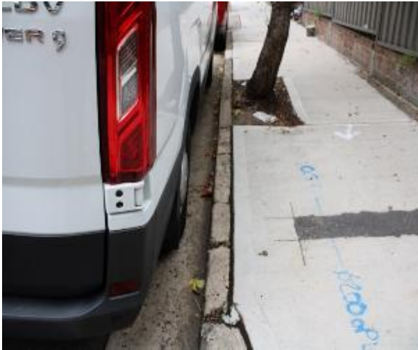
Figure 355 - General condition of kerb and gutter heading East
