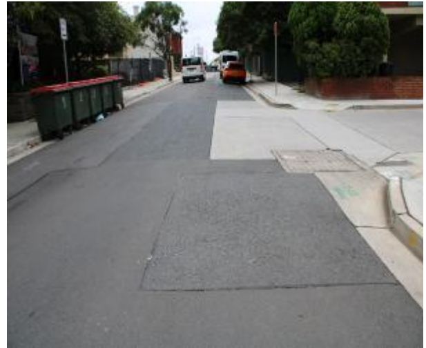
Figure 188 - General condition of road surface heading East
