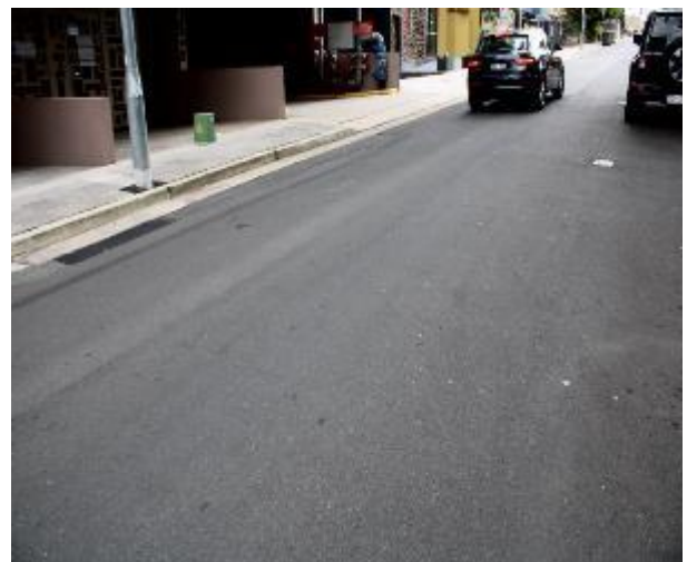
Figure 156 - General condition of road surface heading East
