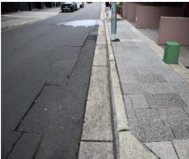
Figure 129 - General condition of kerb and gutter heading West
