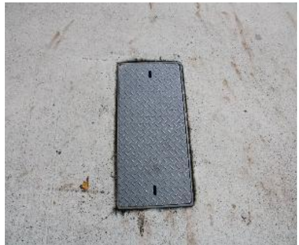
Figure 24 - General condition of service pit
