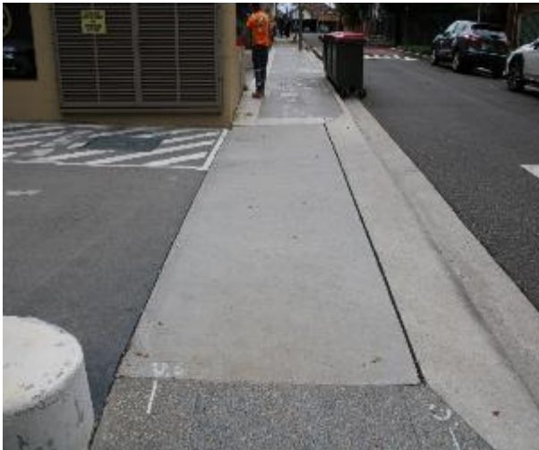
Figure 87 - General condition of footpath pavement heading East
