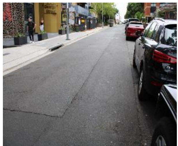
Figure 168 - General condition of road surface heading East
