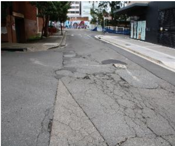
Figure 621 - General condition of road surface heading South
