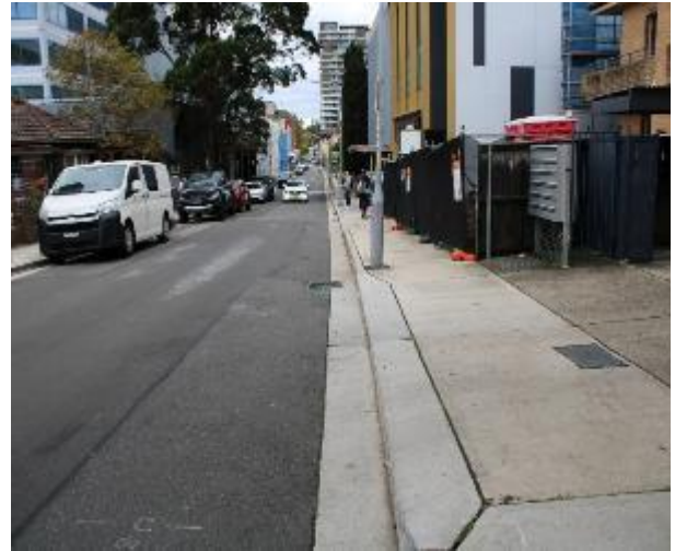
Figure 104 - General condition of kerb and gutter heading West
