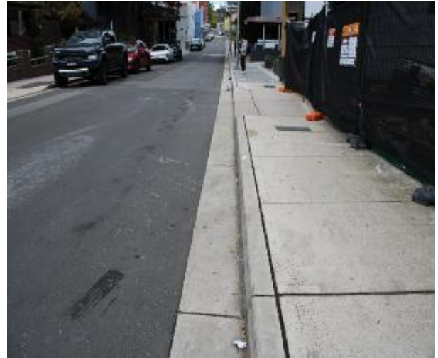
Figure 110 - General condition of kerb and gutter heading West
