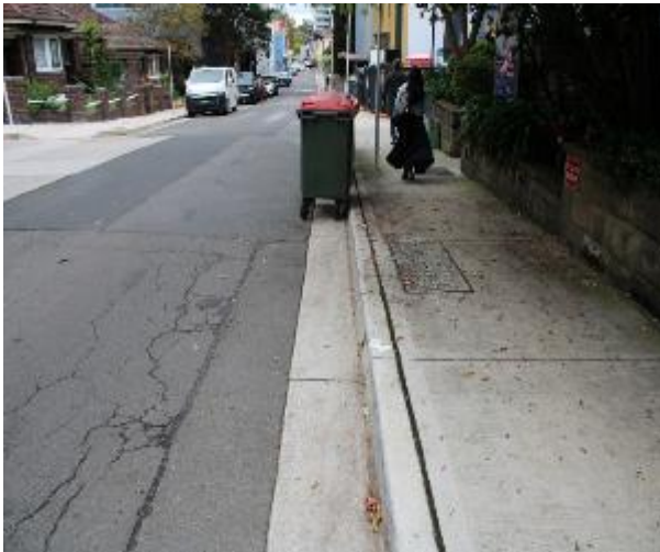
Figure 99 - General condition of kerb and gutter heading West
