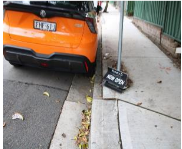
Figure 344 - General condition of kerb and gutter heading East
