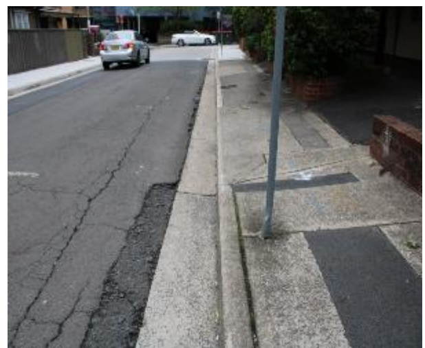
Figure 486 - General condition of kerb and gutter heading North
