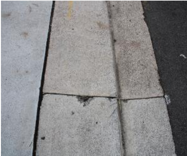
Figure 571 - General condition of driveway layback and gutter heading North
