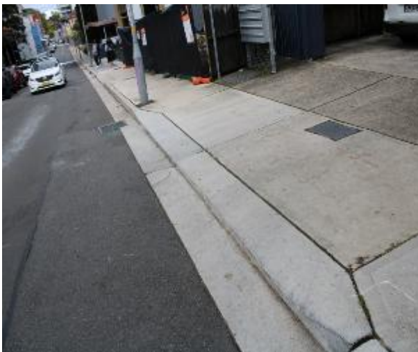
Figure 105 - General condition of driveway layback and gutter heading West
