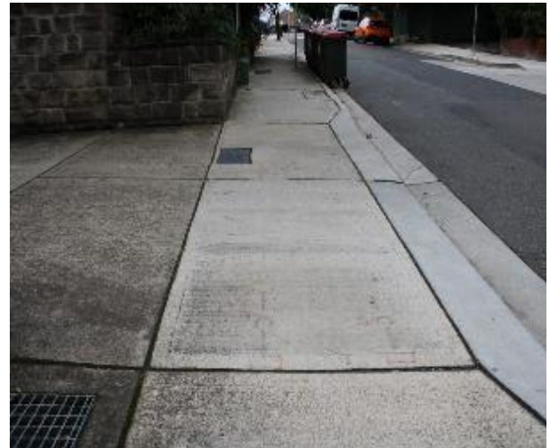
Figure 52 - General condition of footpath pavement heading East
