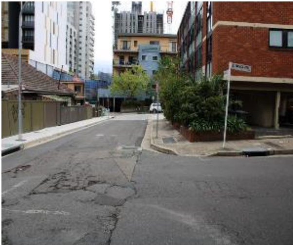
Figure 483 - General condition of road surface heading North
