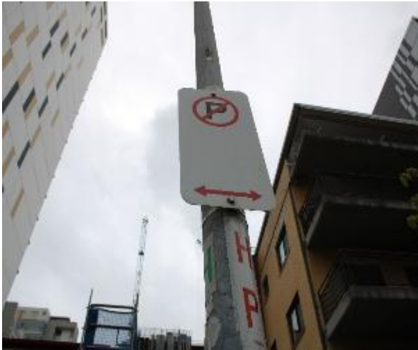
Figure 373 - General condition of street light post Identification No. SVHP62252
