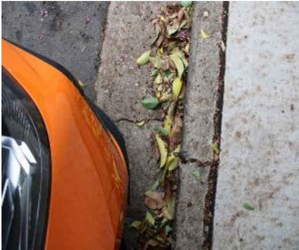
Figure 349 - Crack propagation through kerb and gutter heading East
