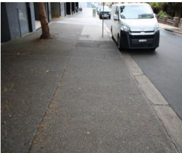
Figure 269 - General condition of footpath pavement heading West
