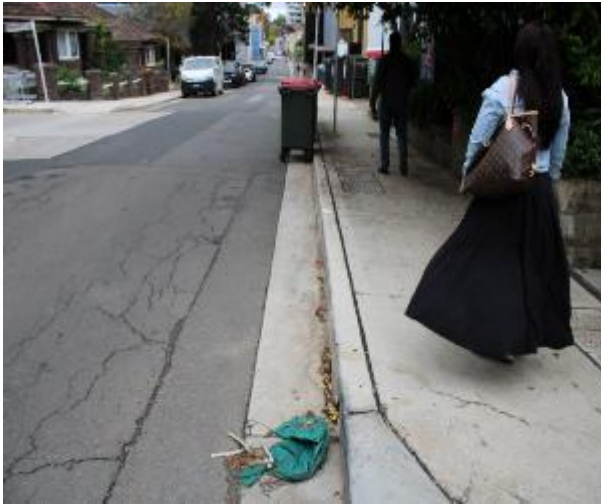
Figure 97 - General condition of kerb and gutter heading West
