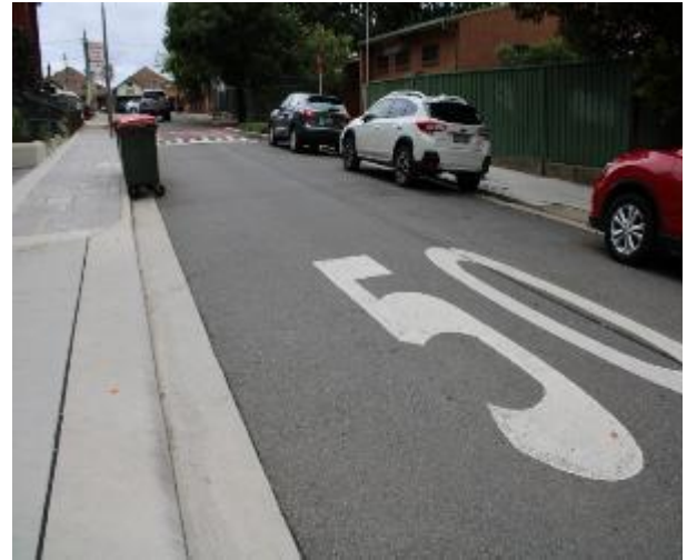
Figure 212 - General condition of
