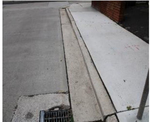
Figure 506 - General condition of kerb and gutter heading North
