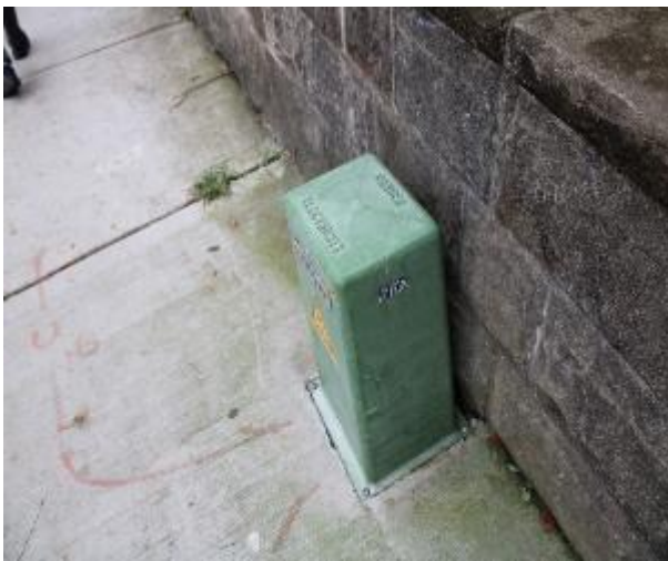
Figure 369 - General condition of electricity box identification No. LE36570
