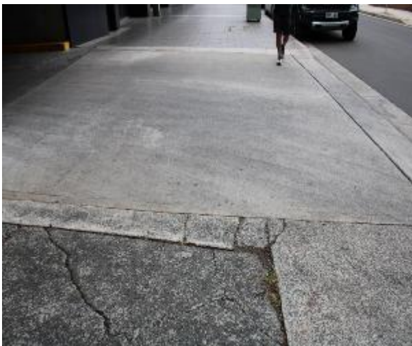
Figure 285 - General condition of footpath pavement heading West
