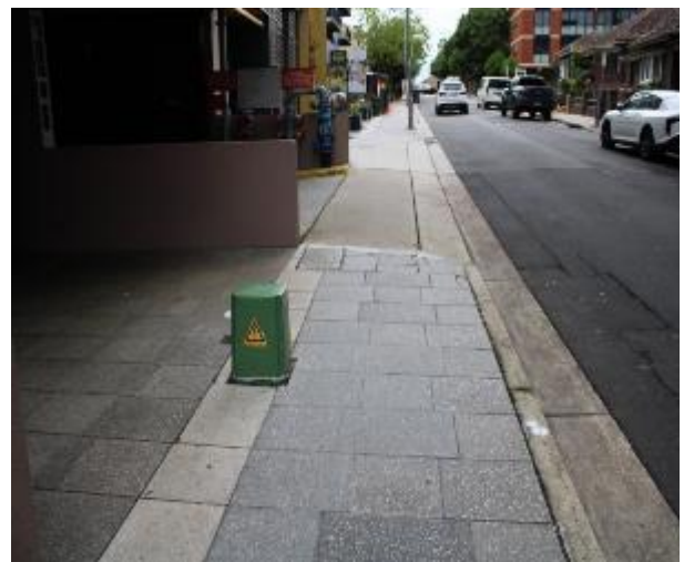
Figure 12 - General condition of footpath pavers heading East
