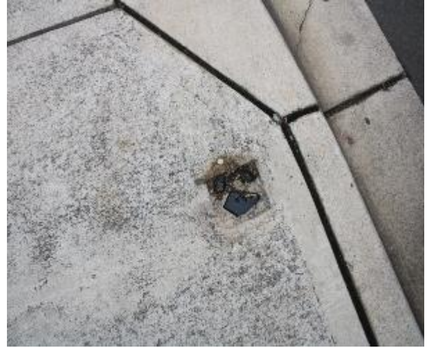
Figure 242 - General condition of service pit
