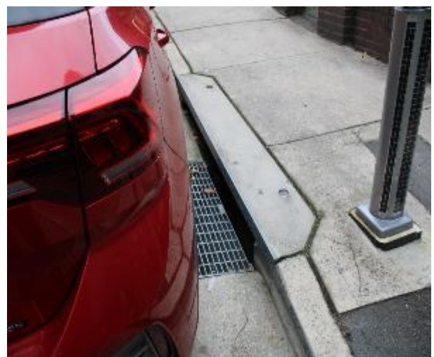
Figure 318 - General condition of stormwater inlet pit
