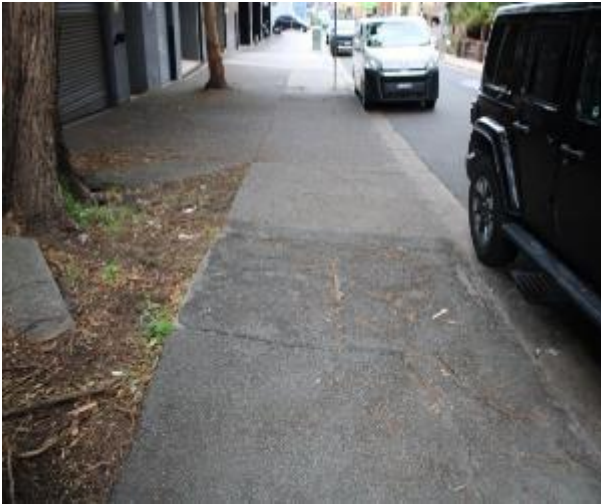
Figure 265 - General condition of footpath pavement heading West
