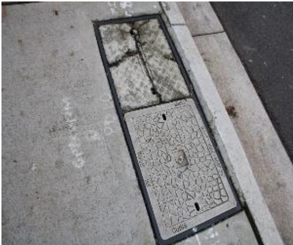
Figure 57 - General condition of service pit
