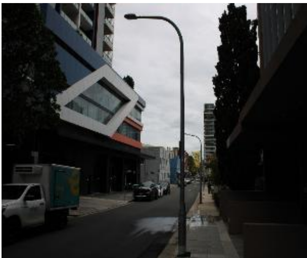
Figure 387 - General condition of streetlight post
