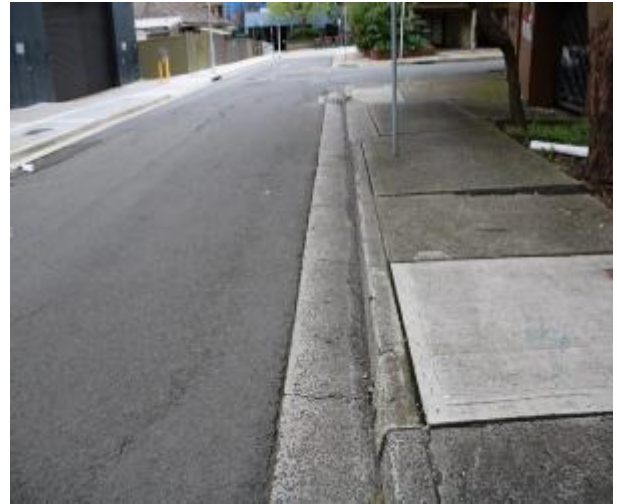
Figure 470 - General condition of kerb and gutter heading North
