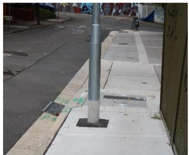
Figure 648 - General condition of street light post identification No. LE32119
