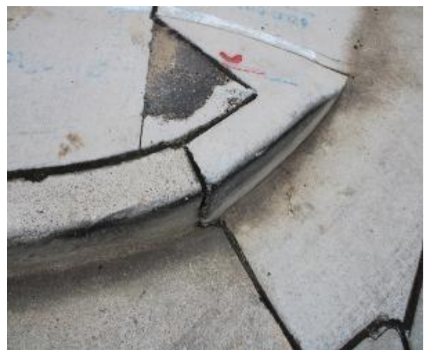
Figure 336 - General condition of kerb and gutter heading East
