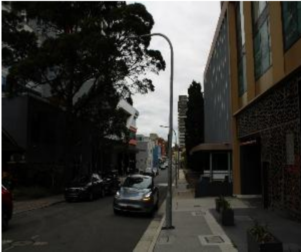
Figure 379 - General condition of street light post Identification No. HR13804
