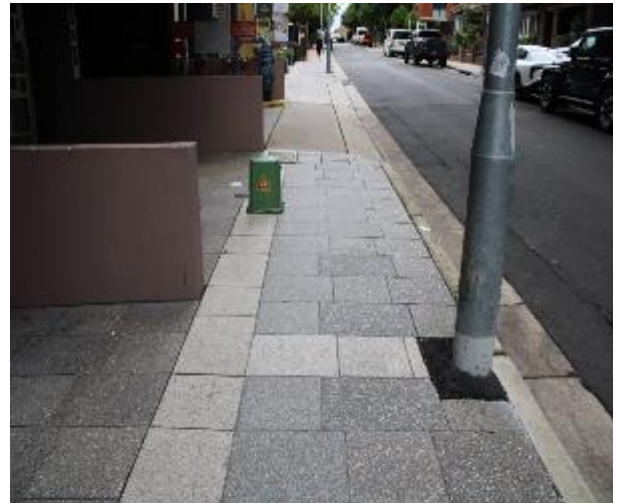
Figure 10 - General condition of footpath pavers heading East
