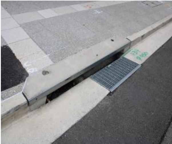
Figure 559 - General condition of stormwater inlet pit
