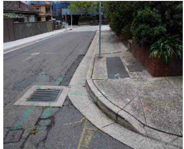
Figure 484 - General condition of kerb and gutter heading North
