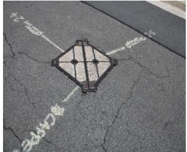
Figure 614 - General condition of service pit
