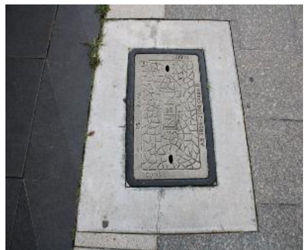
Figure 30 - General condition of service pit
