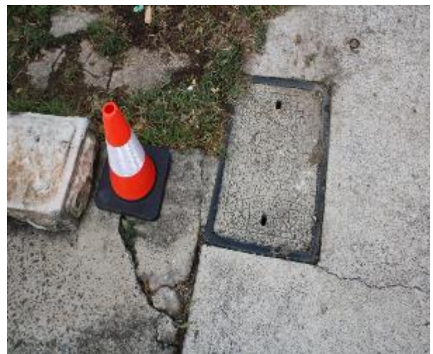
Figure 246 - General condition of service pit
