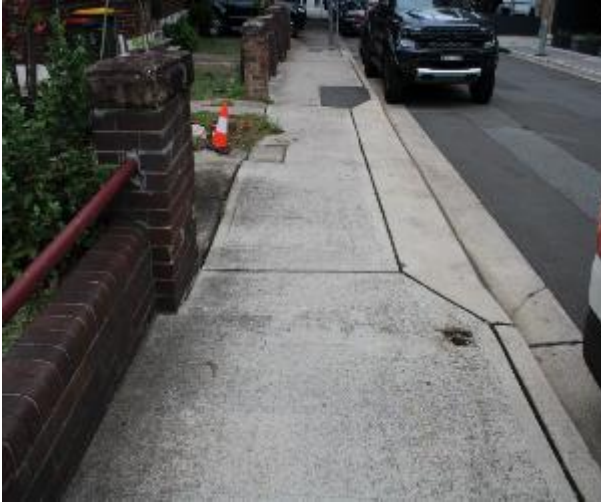
Figure 241 - General condition of footpath pavement heading West
