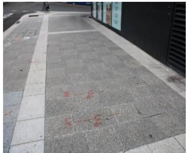
Figure 544 - General condition of footpath pavers heading South
