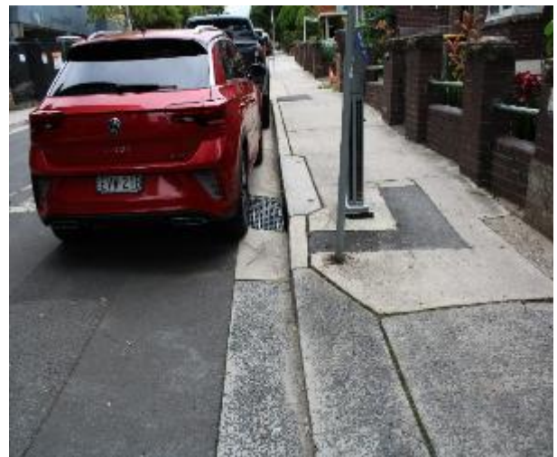
Figure 316 - General condition of kerb and gutter heading East
