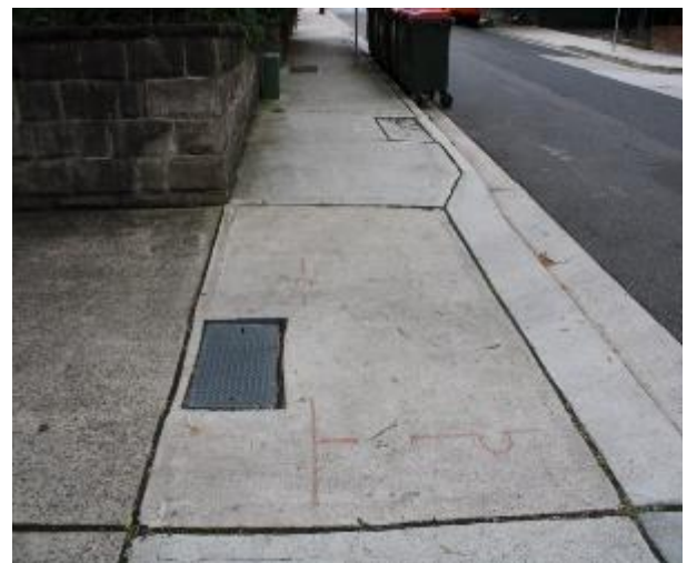
Figure 54 - General condition of footpath pavement heading East
