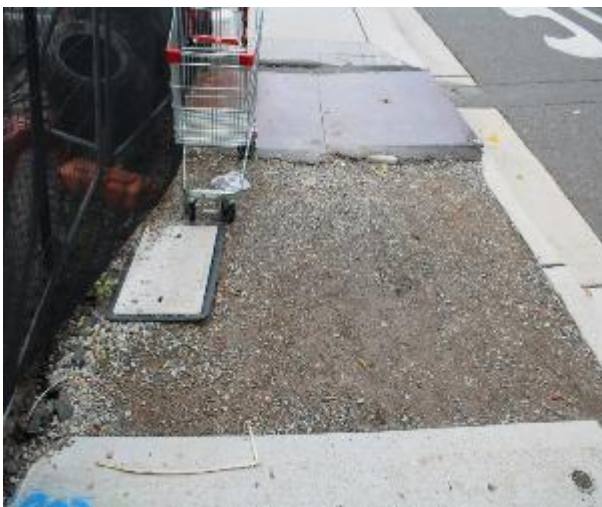
Figure 83 - General condition of footpath pavement heading East
