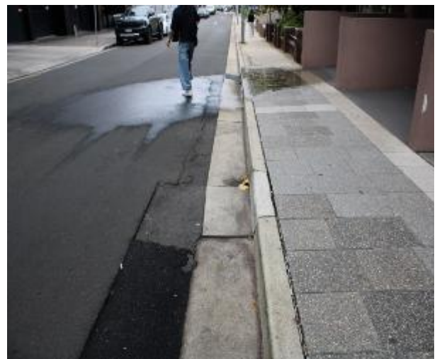
Figure 132 - General condition of kerb and gutter heading West
