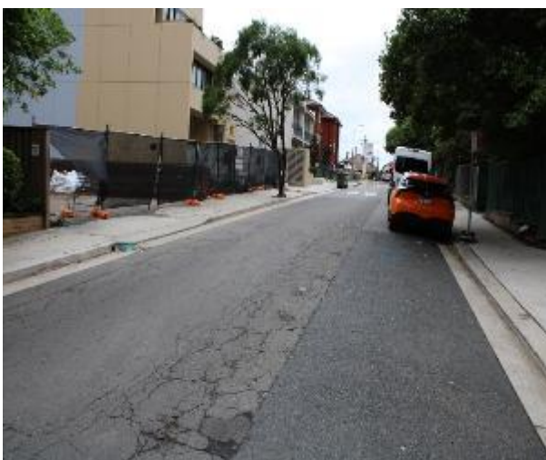
Figure 197 - General condition of road surface heading East
