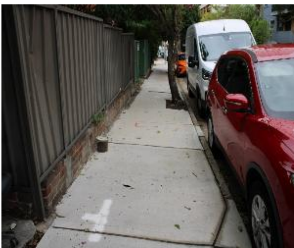
Figure 215 - General condition of footpath pavement heading West
