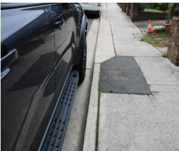
Figure 323 - General condition of kerb and gutter heading East
