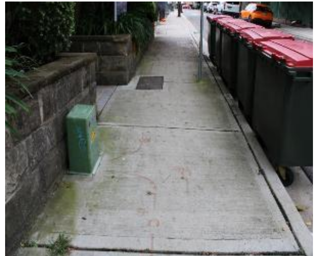
Figure 58 - General condition of footpath pavement heading East
