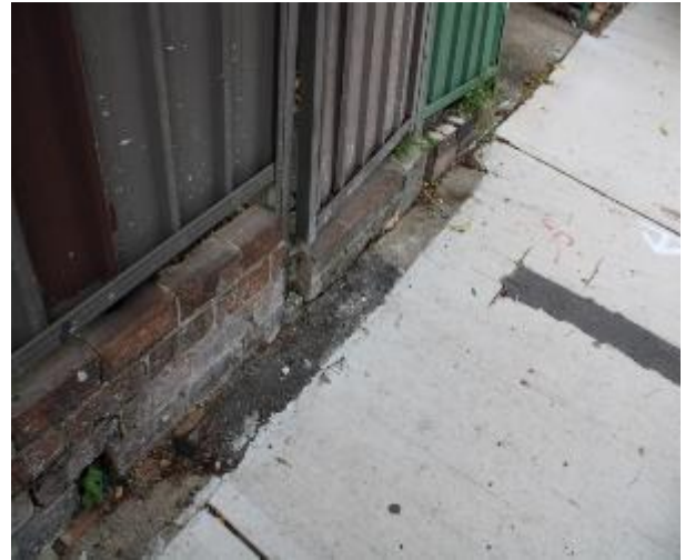
Figure 218 - General condition of footpath pavement heading West
