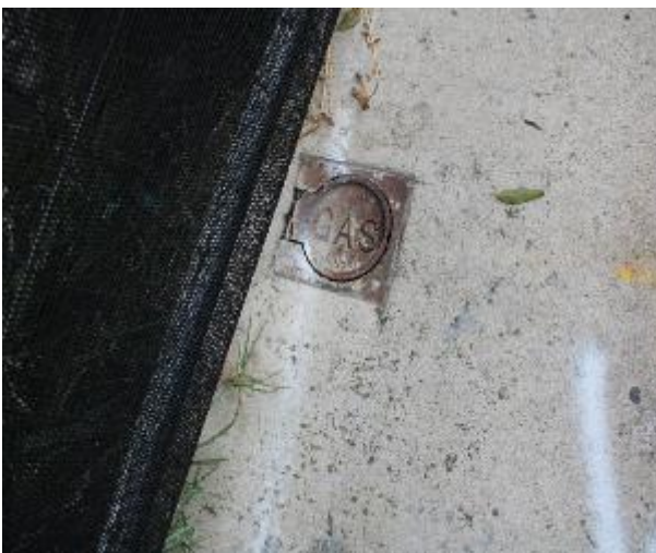
Figure 41 - General condition of service pit
