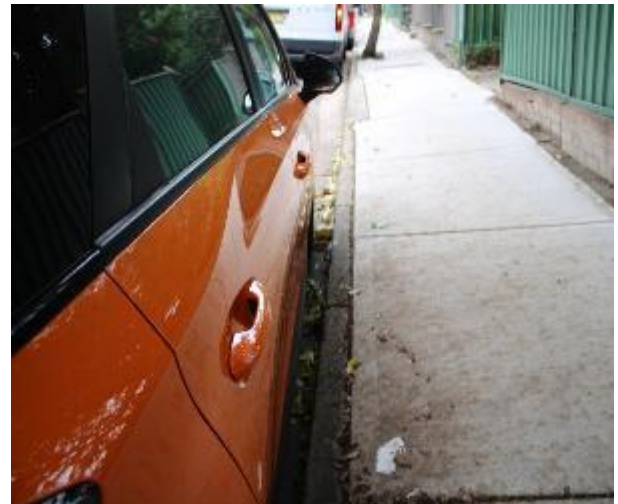
Figure 346 - General condition of kerb and gutter heading East
