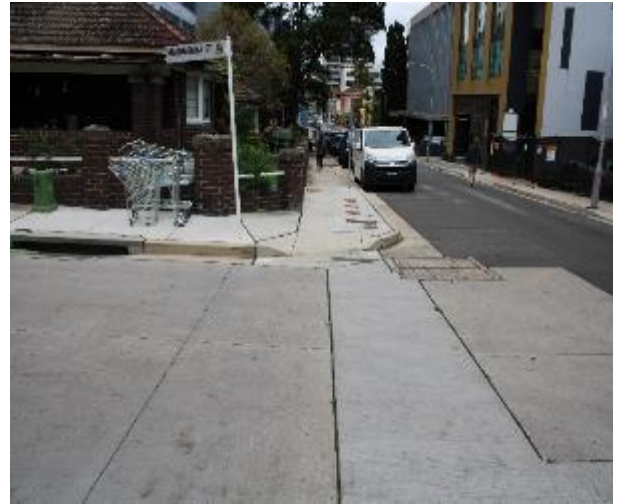
Figure 230 - General condition of footpath pavement heading West
