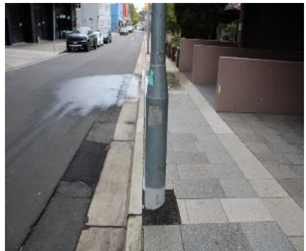
Figure 388 - General condition of streetlight post
