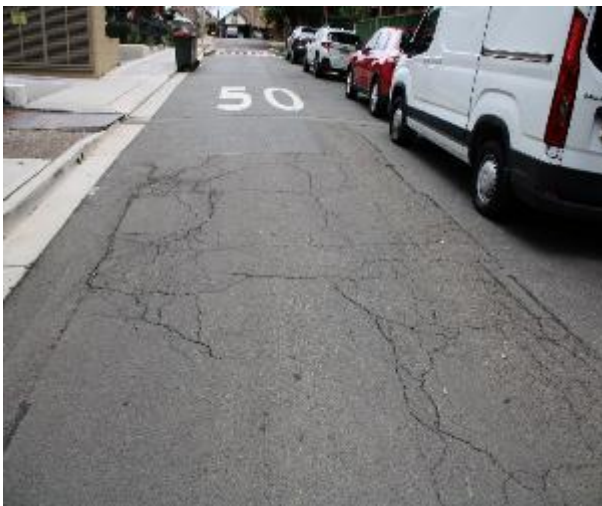
Figure 207 - General condition of road surface heading East
