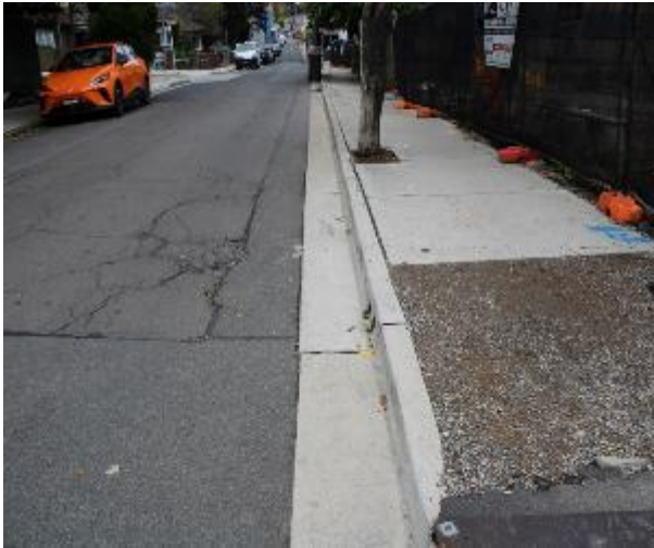
Figure 91 - General condition of kerb and gutter heading West
