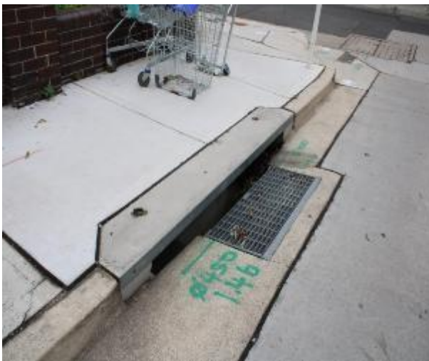
Figure 591 - General condition of stormwater inlet pit
