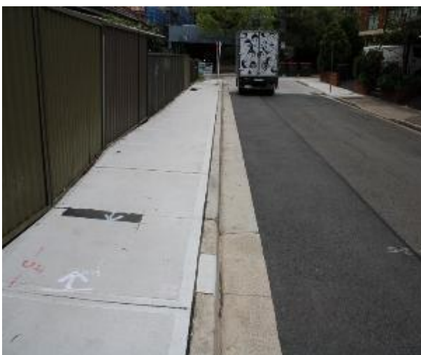
Figure 575 - General condition of kerb and gutter heading North
