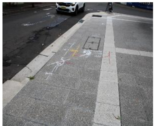
Figure 546 - General condition of footpath pavers heading South
