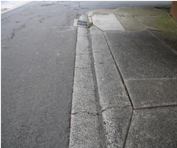
Figure 477 - General condition of driveway layback and gutter heading North
