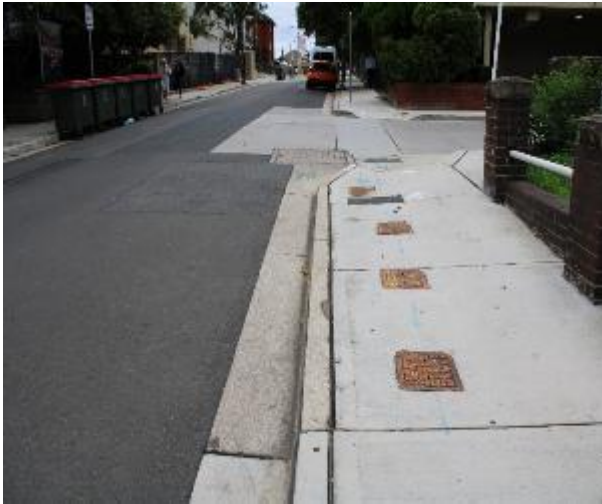
Figure 331 - General condition of kerb and gutter heading East
