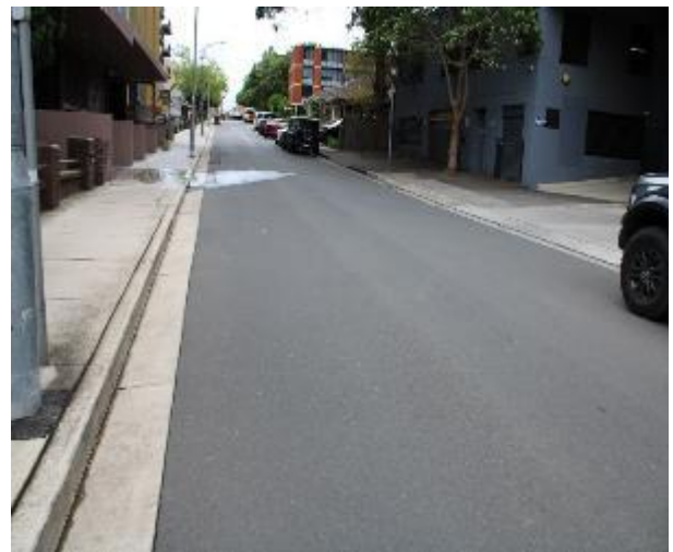
Figure 148 - General condition of road surface heading East
