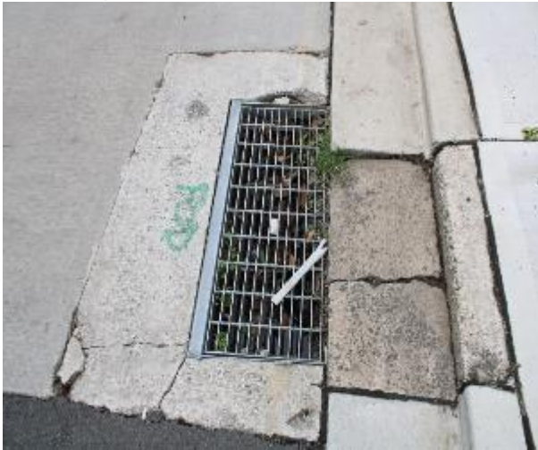
Figure 505 - General condition of stormwater inlet pit
