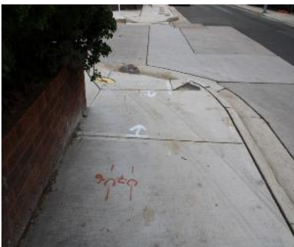
Figure 227 - General condition of footpath pavement heading West
