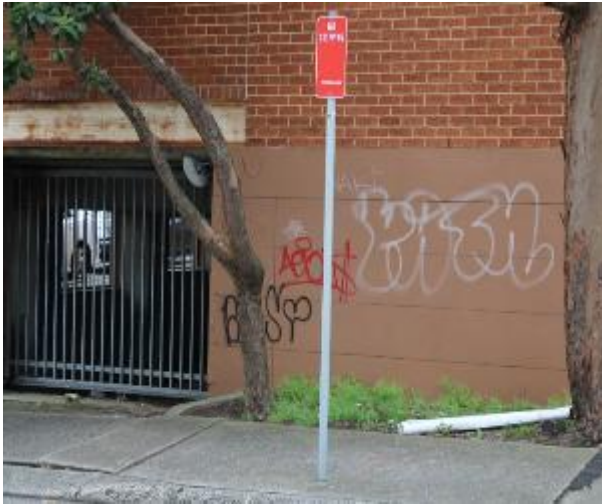
Figure 643 - General condition of street signage
