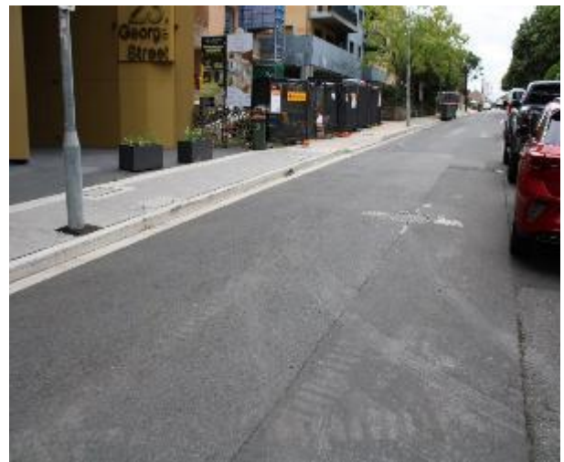
Figure 172 - General condition of road surface heading East
