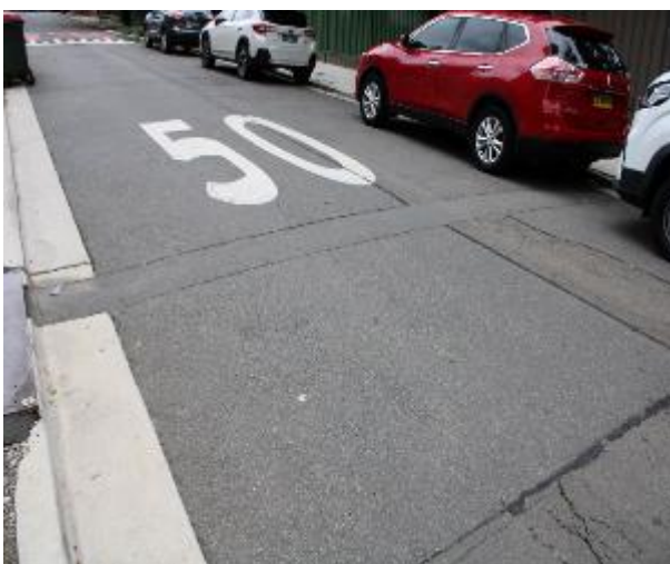
Figure 209 - General condition of road surface heading East
