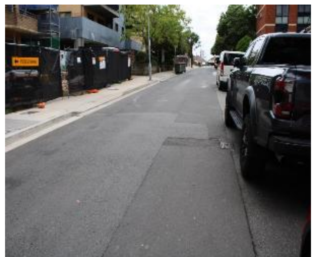
Figure 174 - General condition of road surface heading East
