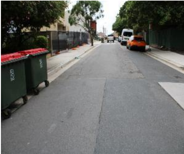
Figure 193 - General condition of road surface heading East
