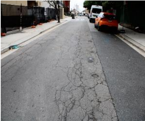
Figure 199 - General condition of road surface heading East
