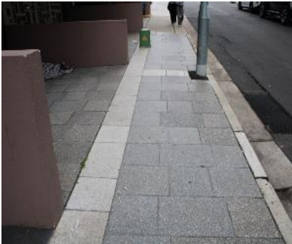
Figure 9 - General condition of footpath pavers heading East
