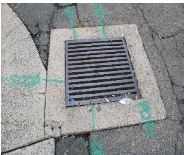
Figure 617 - General condition of stormwater inlet pit
