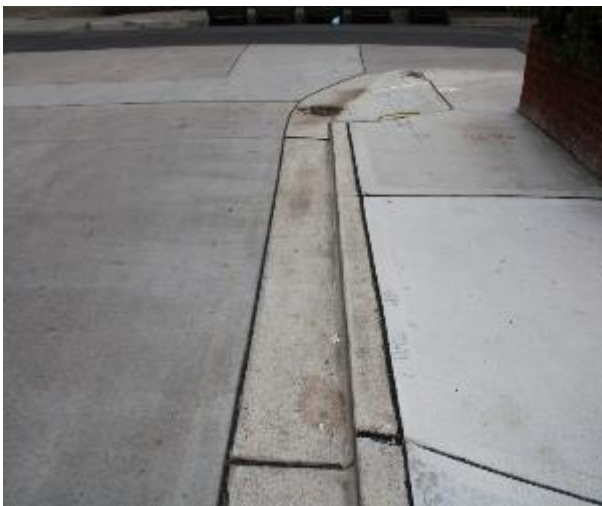
Figure 507 - General condition of kerb and gutter heading North
