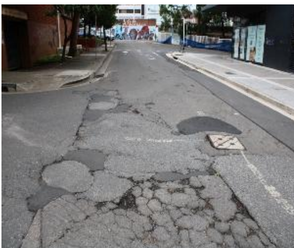
Figure 623 - General condition of road surface heading South
