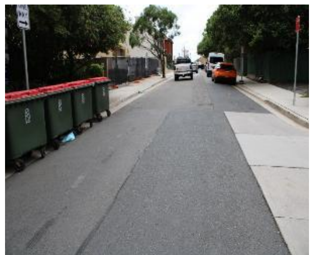
Figure 192 - General condition of road surface heading East
