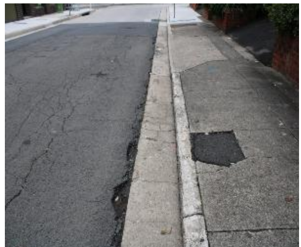
Figure 492 - General condition of kerb and gutter heading North
