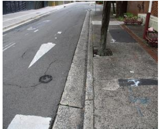
Figure 466 - General condition of kerb and gutter heading North
