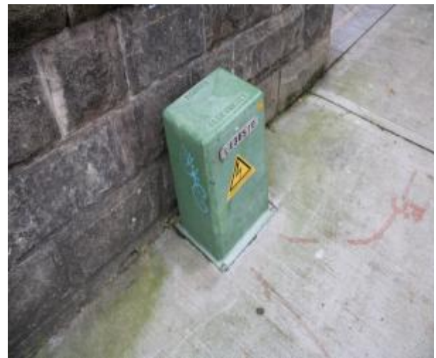
Figure 370 - General condition of electricity box identification No. LE36570
