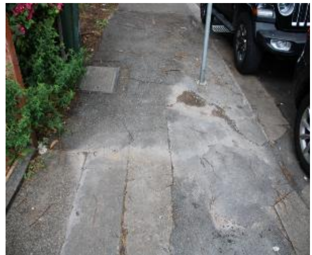
Figure 262 - General condition of footpath pavement heading West
