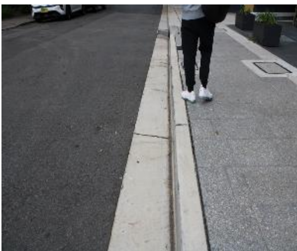
Figure 119 - General condition of kerb and gutter heading West
