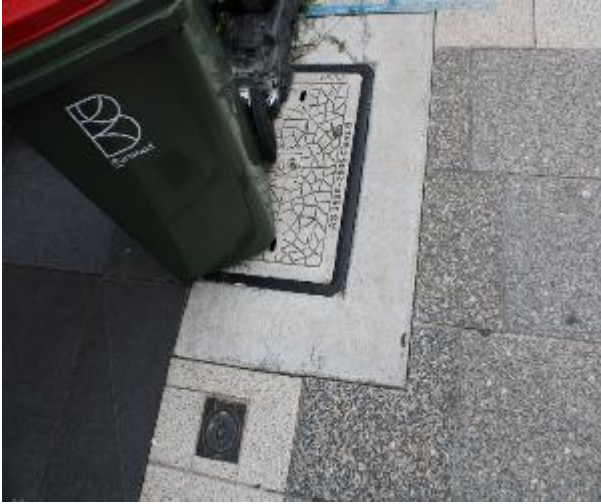
Figure 37 - General condition of service pit
