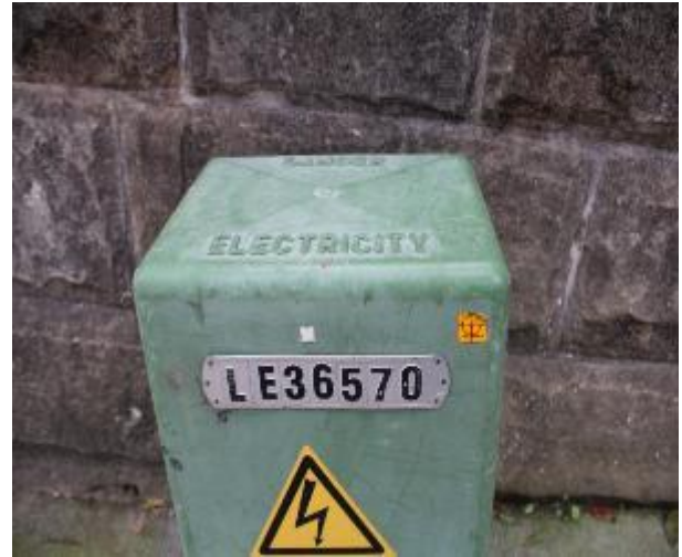
Figure 368 - The following images display the condition of electricity box identification No. LE36570
