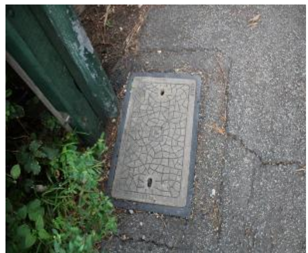
Figure 264 - General condition of service pit
