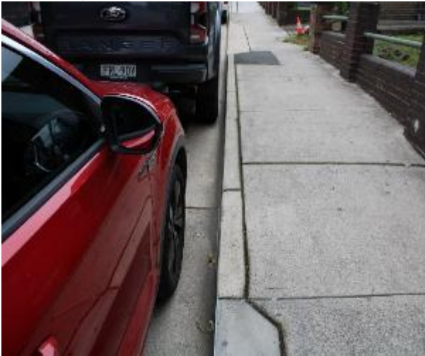
Figure 319 - General condition of kerb and gutter heading East
