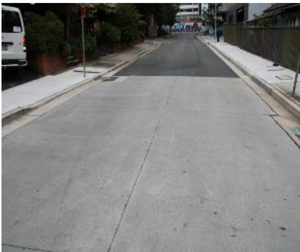
Figure 597 - General condition of road surface heading South
