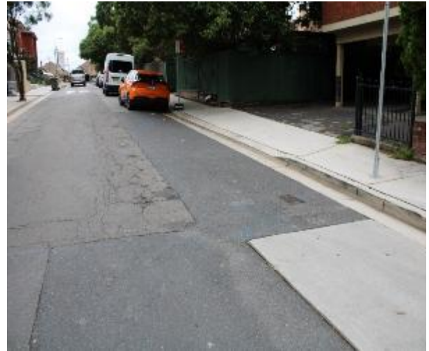
Figure 194 - General condition of road surface heading East
