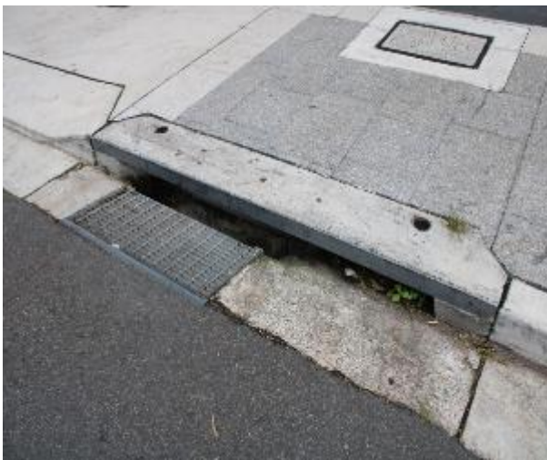
Figure 123 - General condition of stormwater inlet pit
