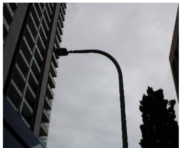
Figure 390 - General condition of streetlight post
