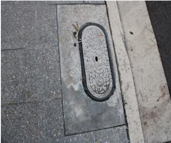
Figure 31 - General condition of service pit
