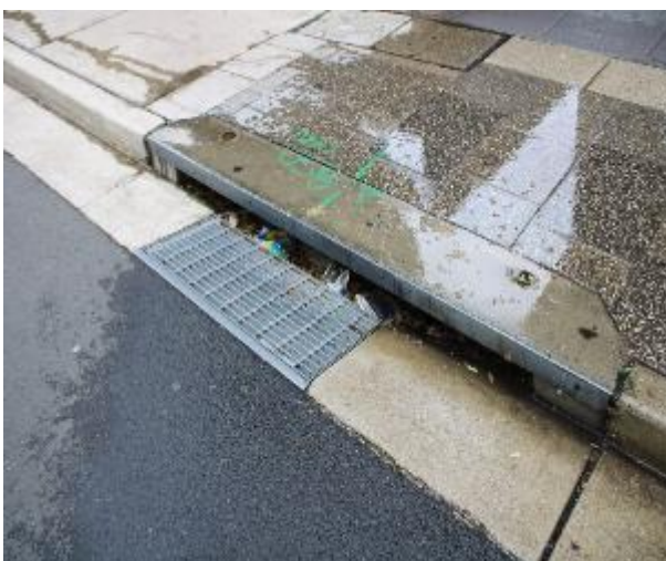
Figure 137 - General condition of stormwater inlet pit
