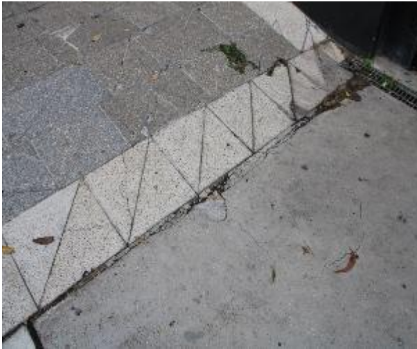
Figure 535 - General condition of footpath pavers heading South
