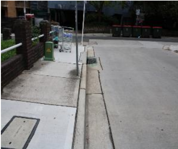
Figure 589 - General condition of kerb and gutter heading North
