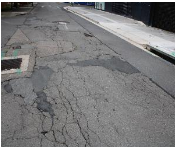
Figure 615 - General condition of road surface heading South
