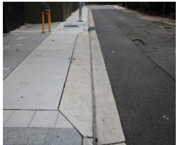
Figure 568 - General condition of driveway layback and gutter heading North
