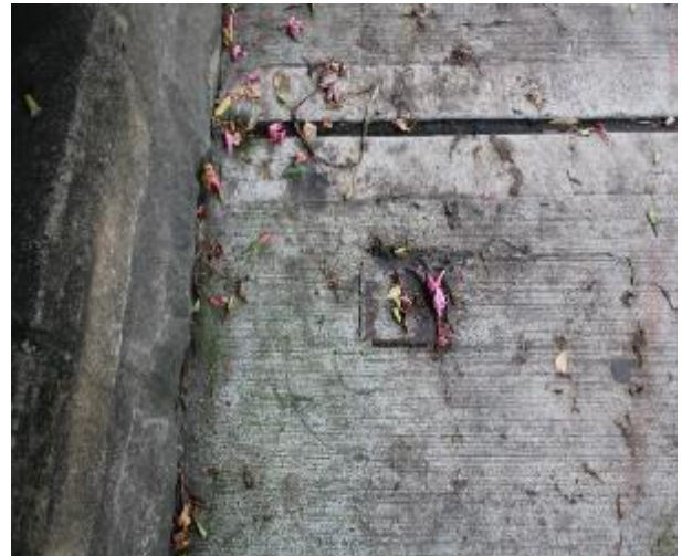
Figure 64 - General condition of service pit
