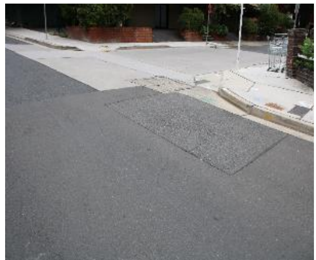
Figure 186 - General condition of road surface heading East
