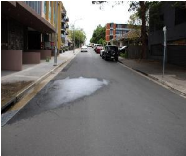
Figure 151 - General condition of road surface heading East
