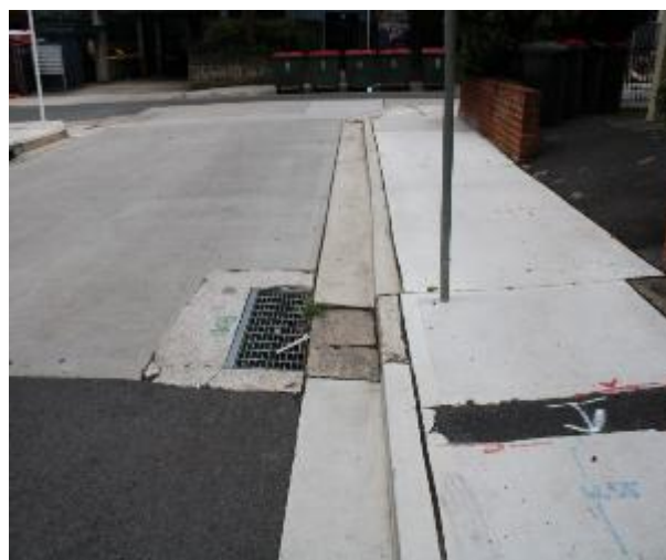
Figure 504 - General condition of kerb and gutter heading North
