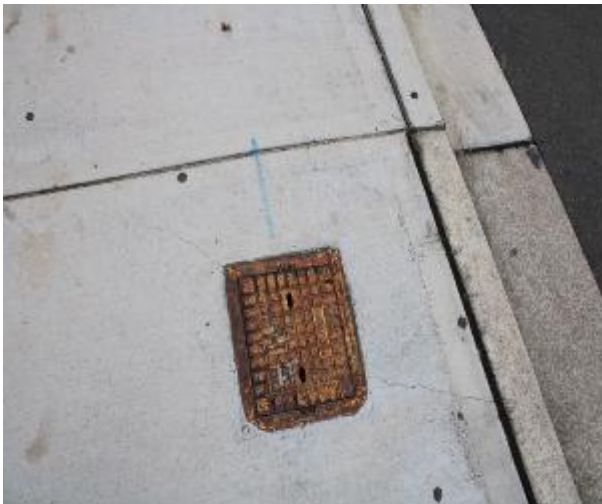
Figure 237 - General condition of service pit
