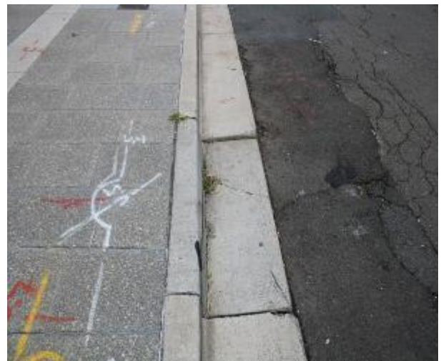
Figure 562 - General condition of kerb and gutter heading North
