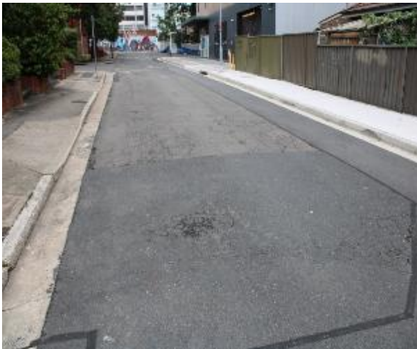
Figure 603 - General condition of road surface heading South
