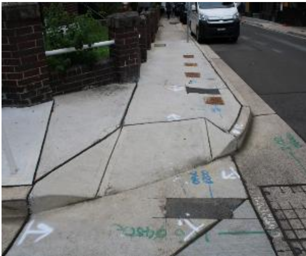
Figure 231 - General condition of footpath pavement heading West
