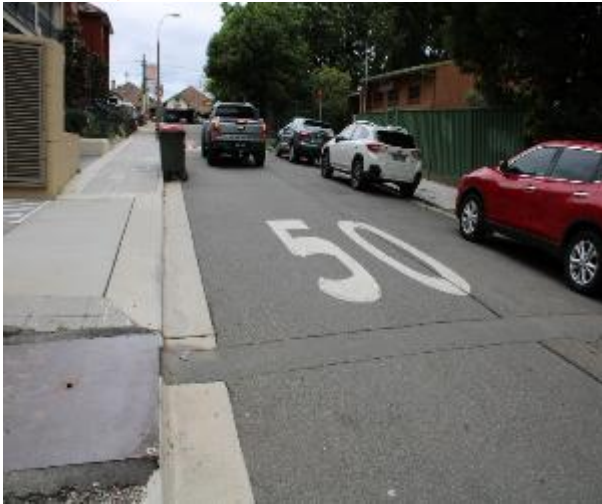
Figure 211 - General condition of road surface heading East
