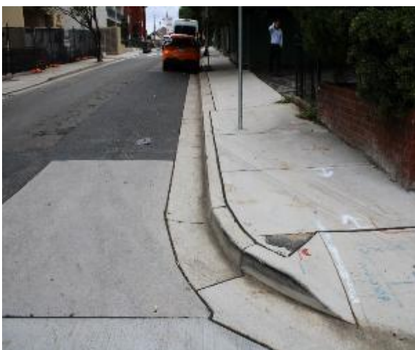
Figure 335 - General condition of kerb and gutter heading East
