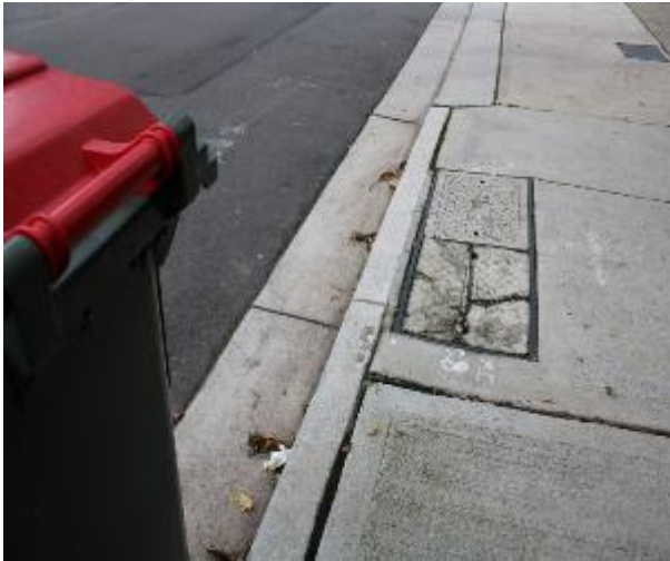
Figure 103 - General condition of kerb and gutter heading West
