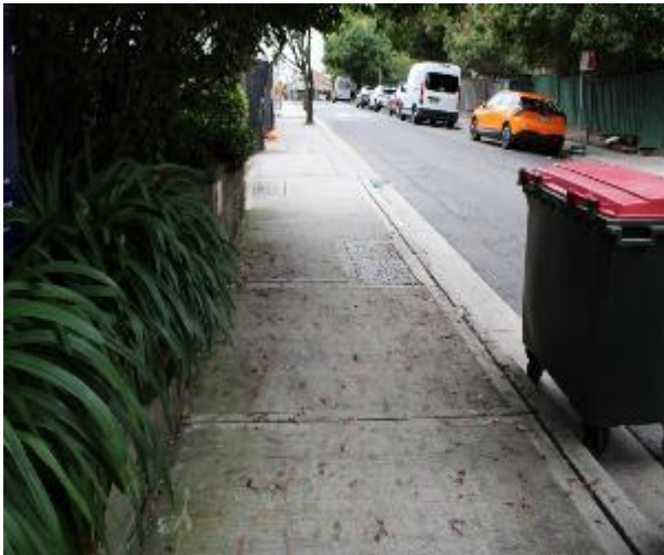
Figure 63 - General condition of footpath pavement heading East
