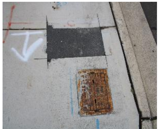
Figure 234 - General condition of service pit
