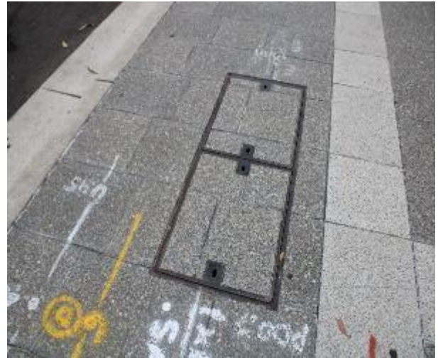
Figure 548 - General condition of service pit
