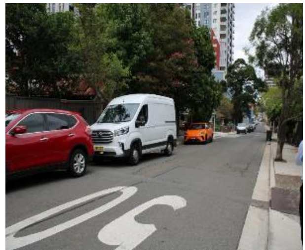
Figure 214 - General condition of road surface heading East
