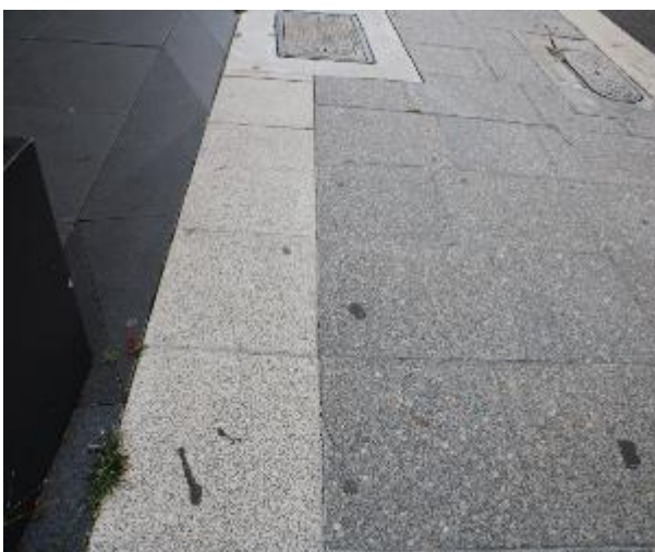
Figure 29 - General condition of footpath pavers heading East
