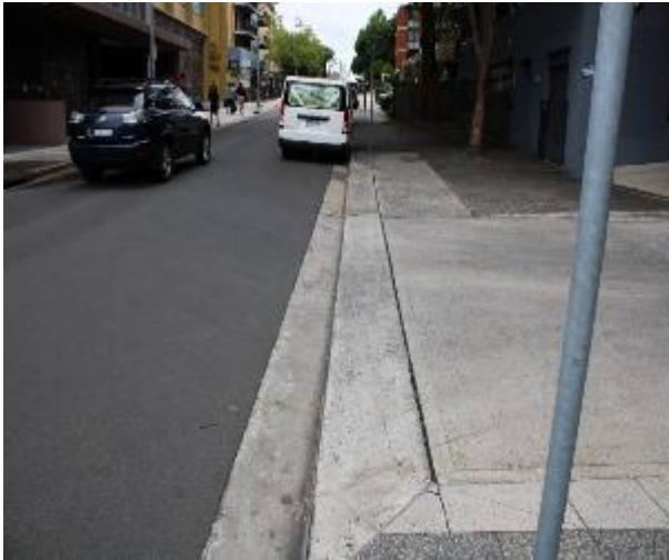
Figure 289 - General condition of kerb and gutter heading East
