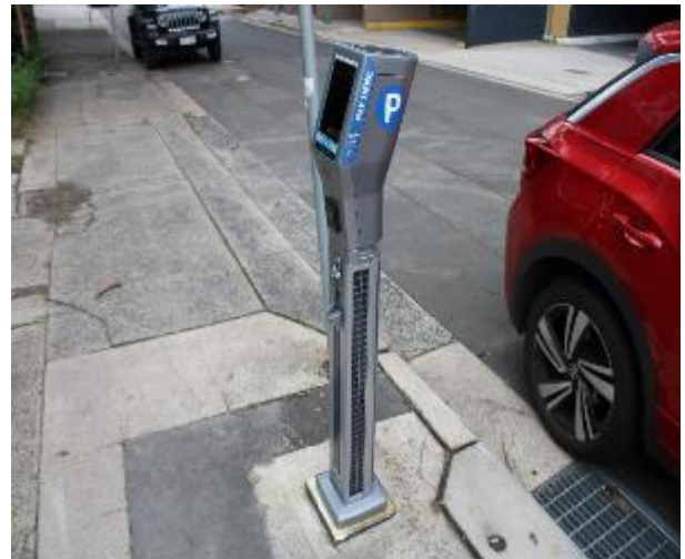
Figure 394 - General condition of parking meter identification No. GEO8
