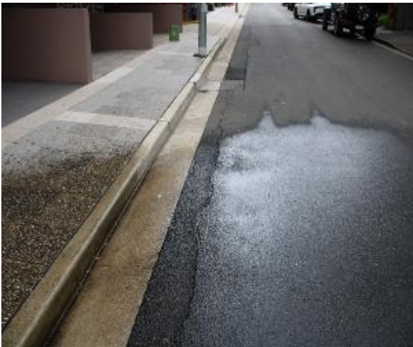
Figure 153 - General condition of road surface heading East
