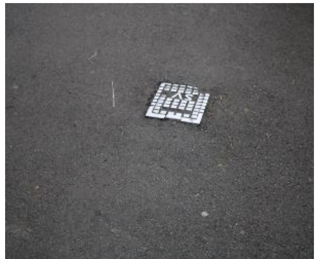
Figure 160 - General condition of service pit
