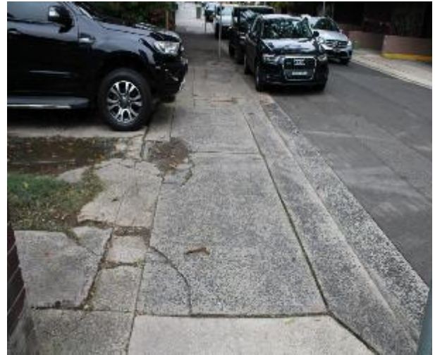
Figure 254 - General condition of footpath pavement heading West
