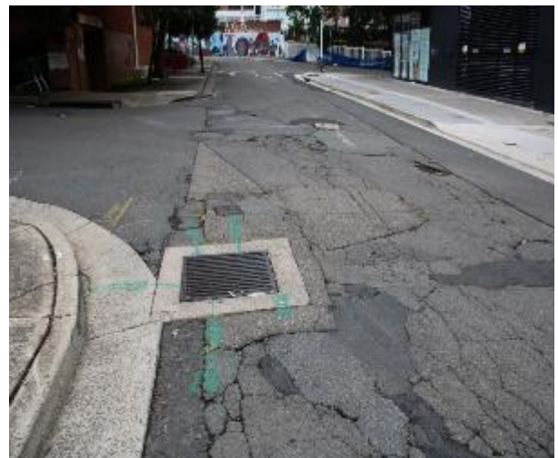
Figure 616 - General condition of road surface heading South
