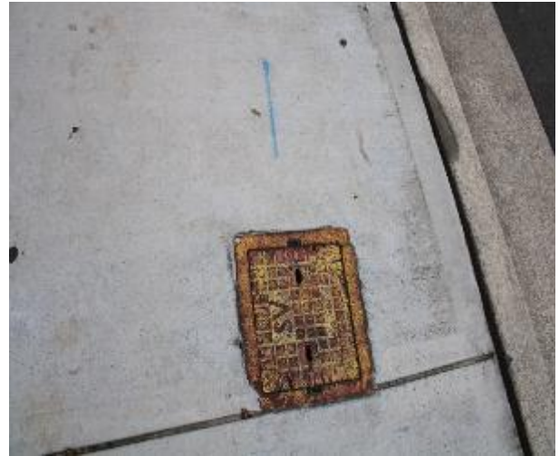
Figure 236 - General condition of service pit
