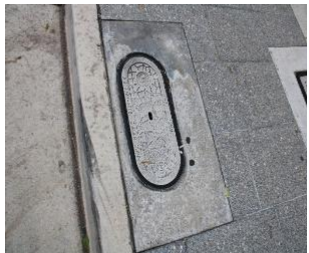
Figure 120 - General condition of service pit
