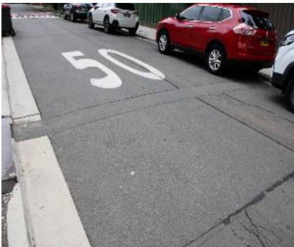
Figure 213 - General condition of road surface heading East
