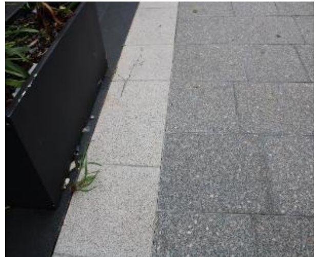
Figure 34 - General condition of footpath pavers heading East
