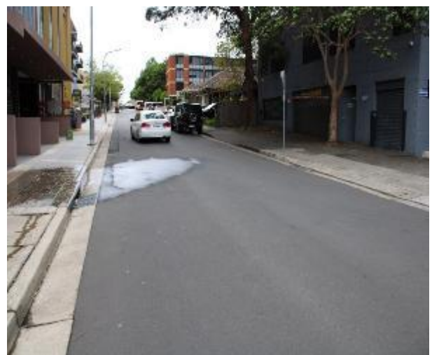
Figure 150 - General condition of road surface heading East
