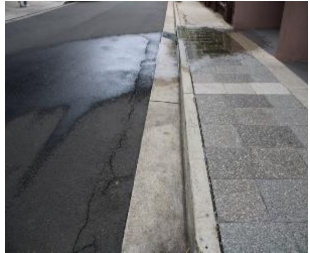
Figure 134 - General condition of kerb and gutter heading West
