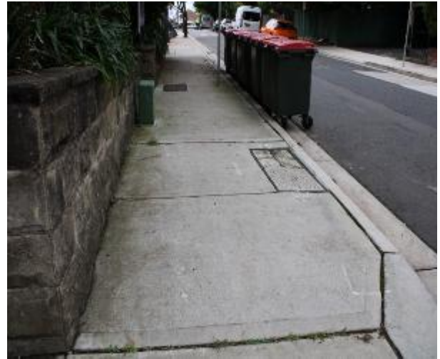
Figure 56 - General condition of footpath pavement heading East
