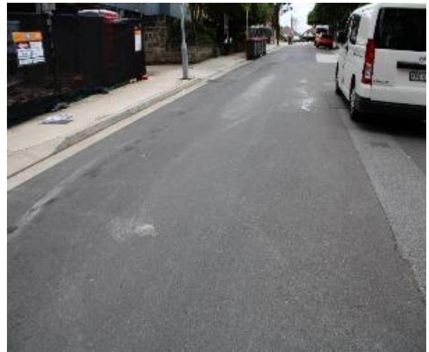
Figure 178 - General condition of road surface heading East
