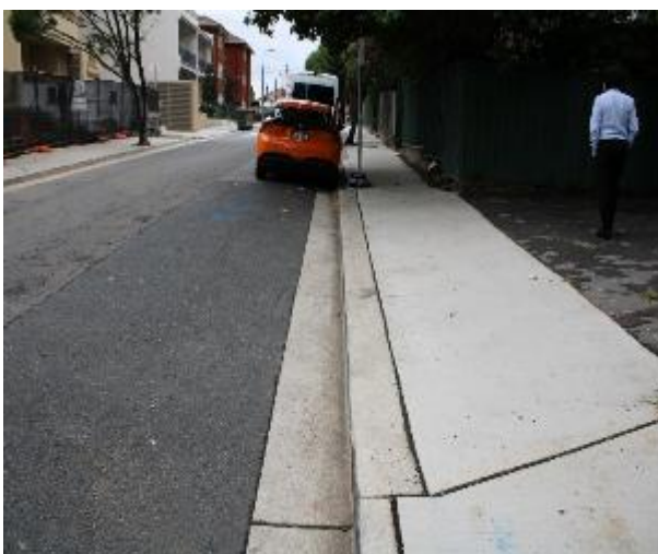
Figure 341 - General condition of kerb and gutter heading East
