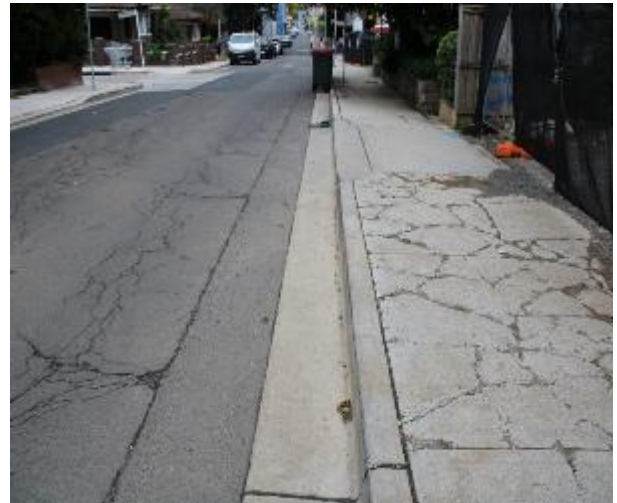
Figure 94 - General condition of kerb and gutter heading West
