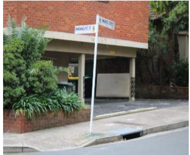
Figure 644 - General condition of street signage
