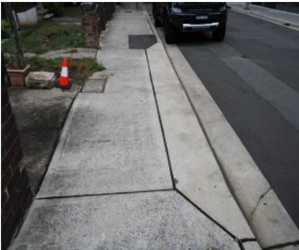
Figure 243 - General condition of footpath pavement heading West
