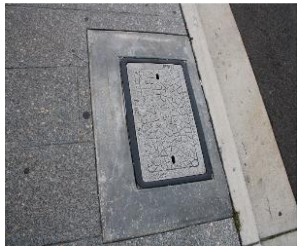
Figure 36 - General condition of service pit
