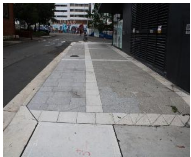
Figure 534 - General condition of footpath pavers heading South
