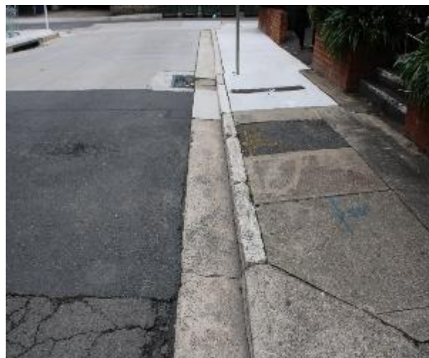
Figure 500 - General condition of kerb and gutter heading North
