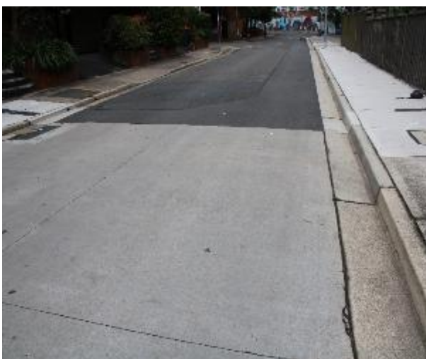
Figure 599 - General condition of road surface heading South
