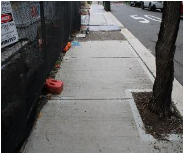
Figure 81 - General condition of footpath pavement heading East
