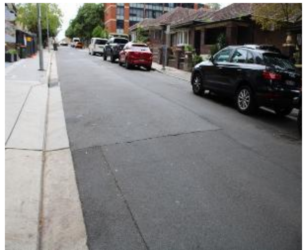
Figure 166 - General condition of road surface heading East
