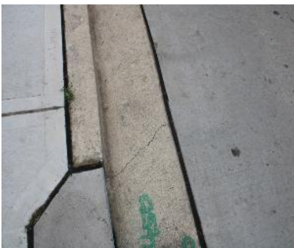
Figure 593 -kerb and gutter heading North
