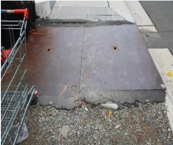
Figure 85 - General condition of service pit
