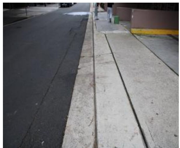
Figure 126 - General condition of driveway layback and gutter heading West
