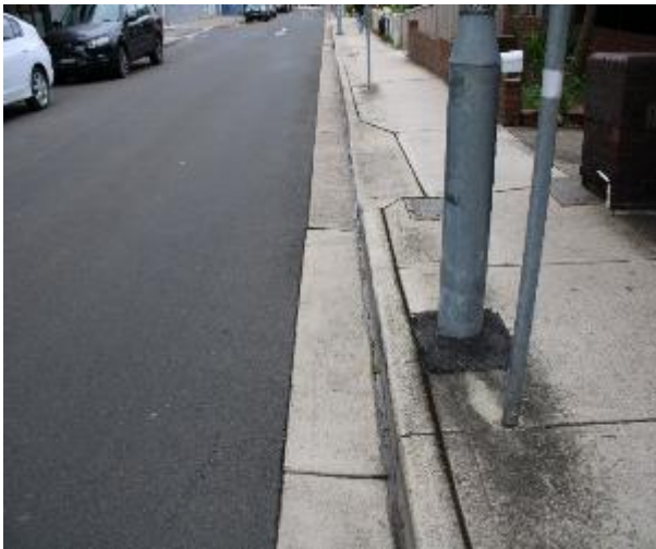
Figure 141 - General condition of kerb and gutter heading West
