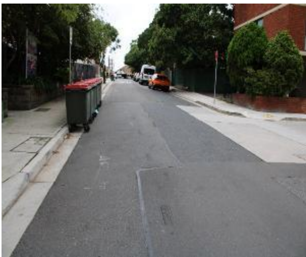
Figure 185 - General condition of road surface heading East
