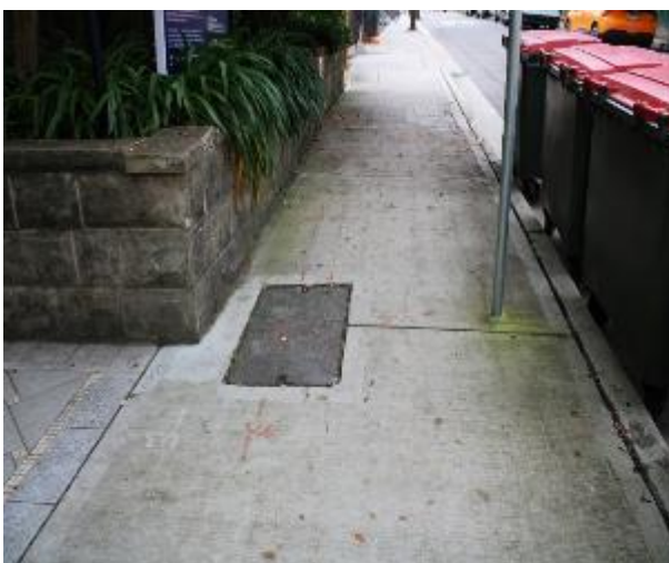
Figure 59 - General condition of footpath pavement heading East
