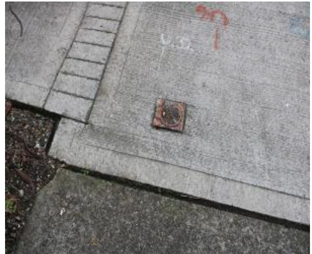
Figure 454 - General condition of service pit
