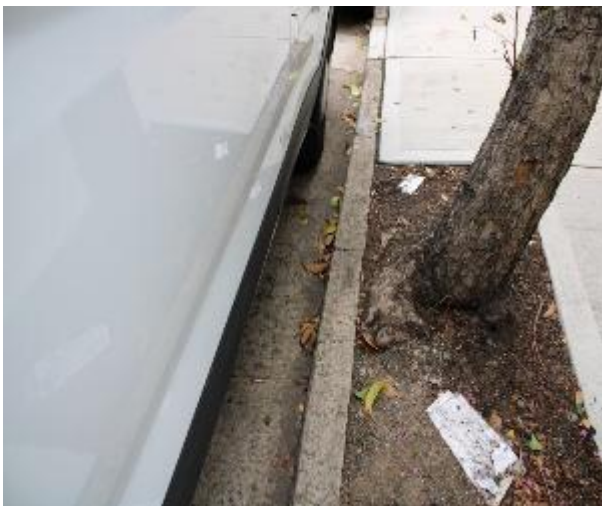
Figure 357 - General condition of kerb and gutter heading East
