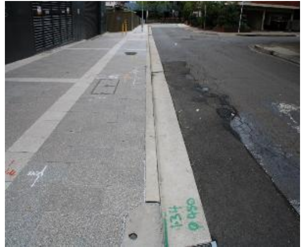
Figure 560 - General condition of kerb and gutter heading North
