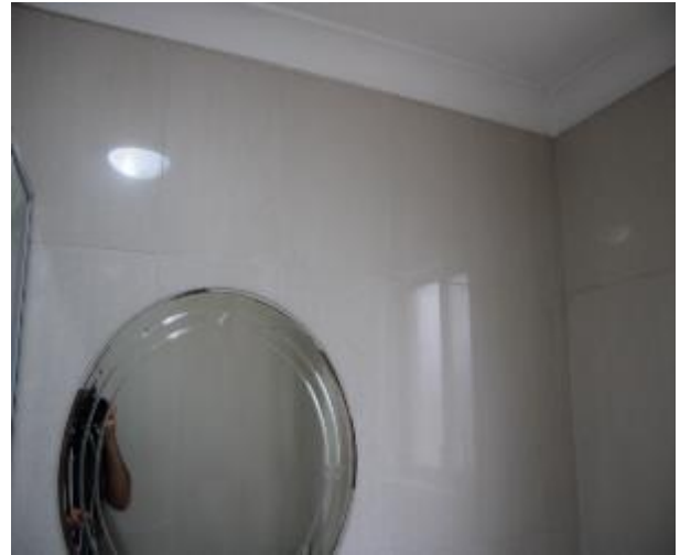
Figure 698 - General condition of bathroom 1 internal wall
