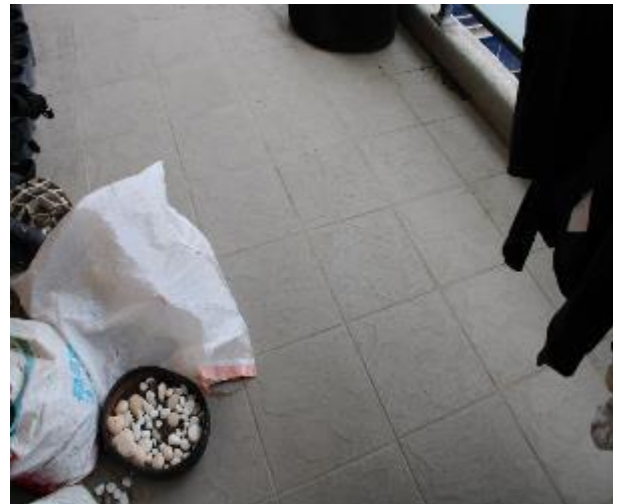
Figure 1433 - General condition of balcony floor tiles
