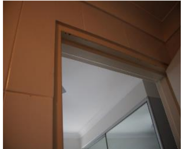
Figure 907 - General condition of ensuite bathroom internal wall
