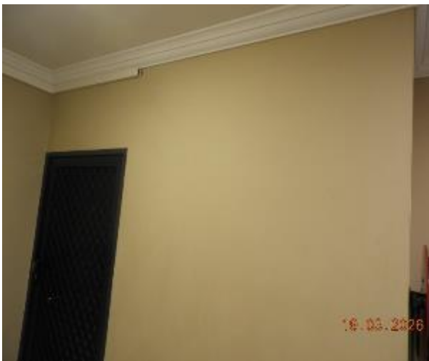
Figure 81 - General condition of level 3 common area internal wall
