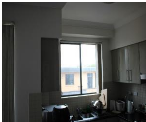
Figure 1466 - General condition of open kitchen/ lounge room internal wall
