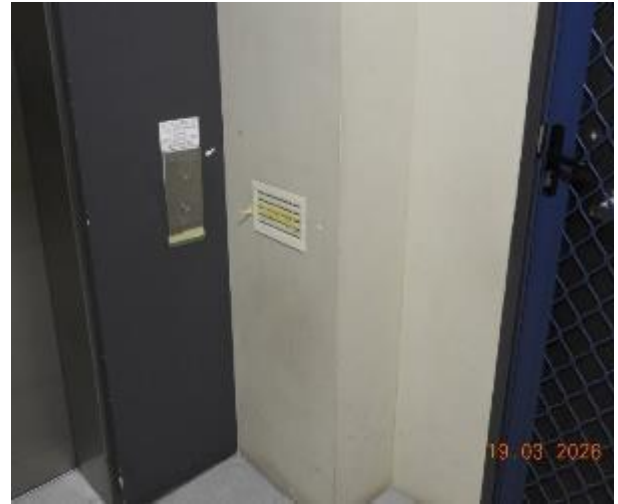
Figure 104 - General condition of level 3 common area internal wall
