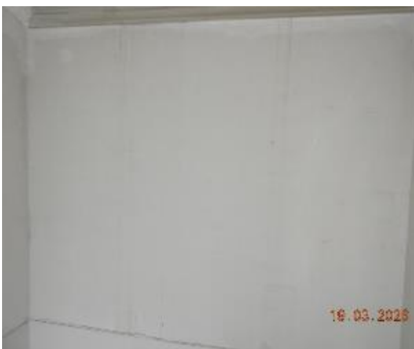
Figure 298 - General condition of level 5 fire stairs internal wall
