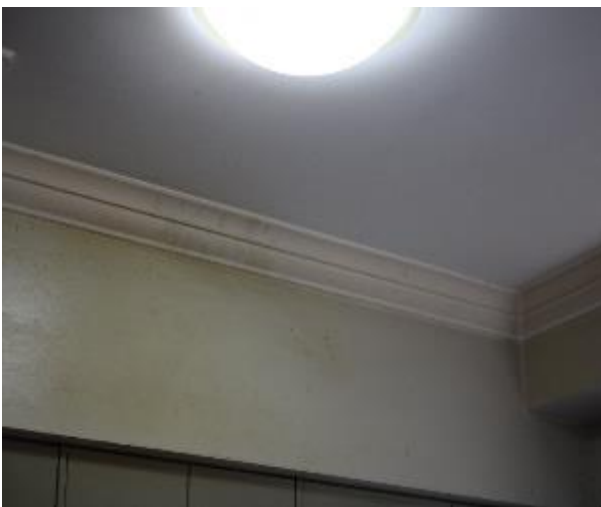
Figure 767 - General condition of open kitchen/ lounge room ceiling
