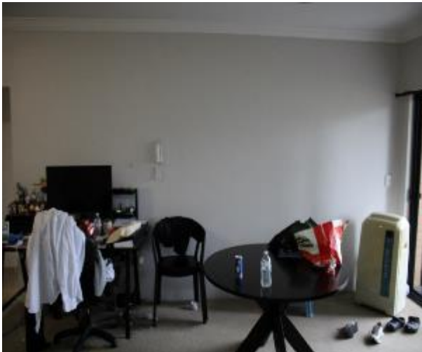
Figure 633 - General condition of lounge room internal wall
