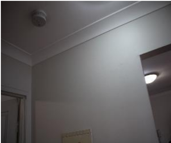
Figure 986 - General condition of corridor internal wall
