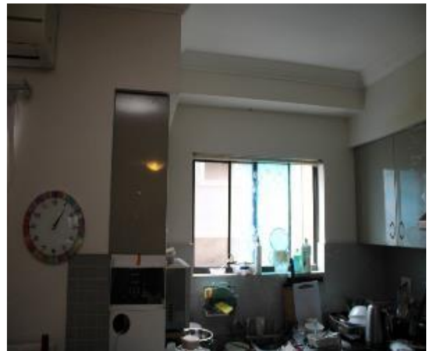
Figure 867 - General condition of kitchen internal wall
