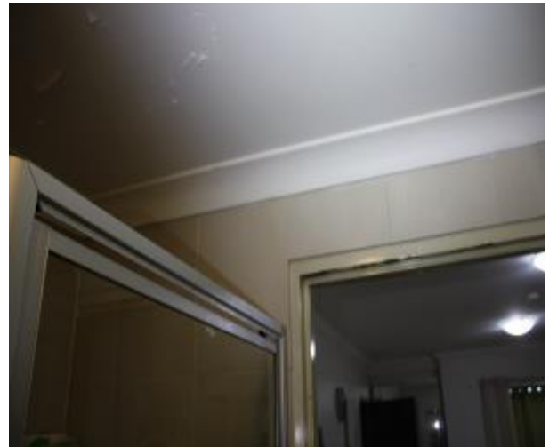
Figure 566 - General condition of bathroom 1 internal wall
