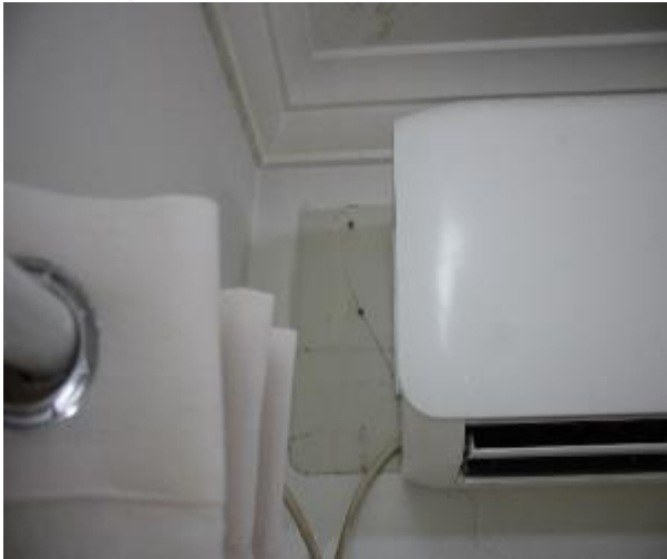
Figure 527 - Crack propagation through open kitchen/ lounge room internal wall
