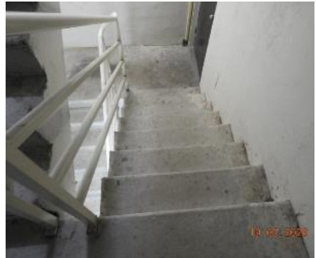
Figure 345 - General condition of level 3 fire stairs
