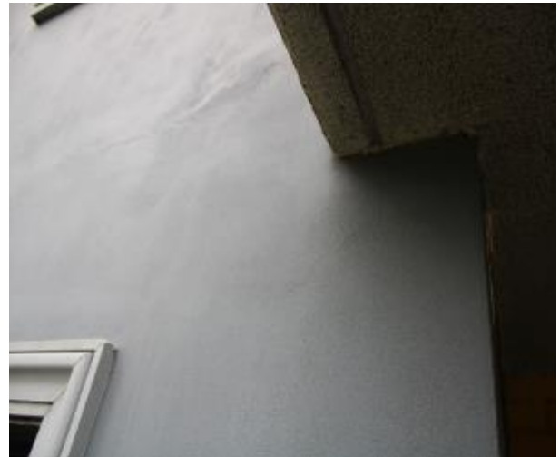
Figure 670 - General condition of external wall
