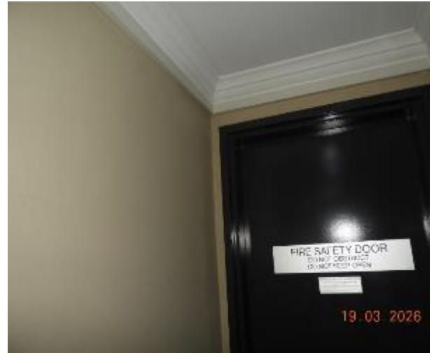
Figure 164 - General condition of level 5 common area internal wall
