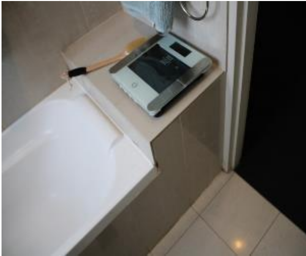
Figure 1583 - General condition of bathroom 1 internal wall
