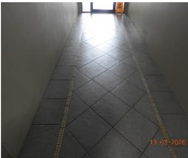
Figure 5 - General condition of level 1 common area floor tiles
