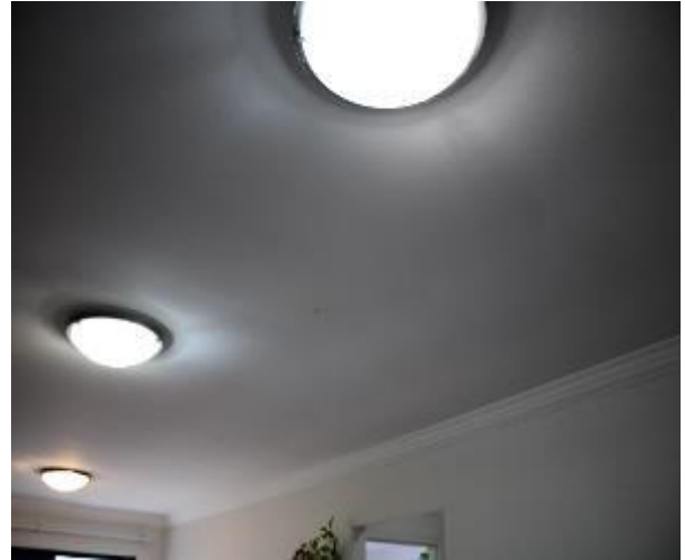
Figure 951 - General condition of lounge room ceiling
