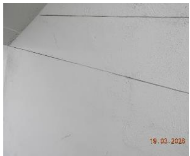
Figure 419 - General condition of level 1 fire stairs internal wall
