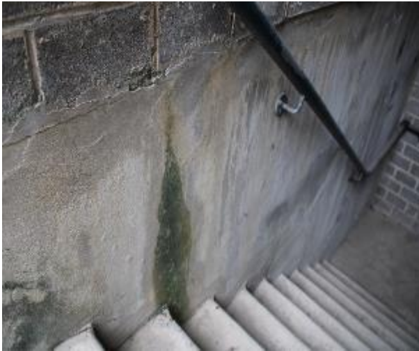
Figure 263 - General condition of level 1 fire stairs internal wall
