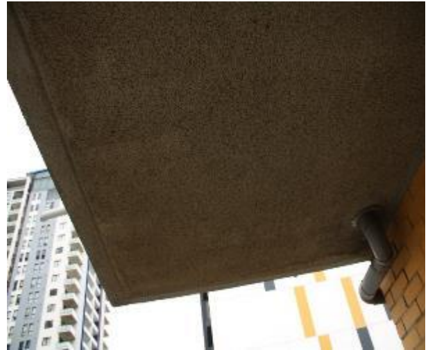
Figure 1093 - General condition of balcony underside slab
