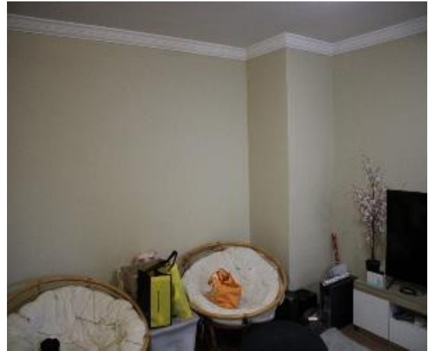
Figure 1269 - General condition of lounge room internal wall
