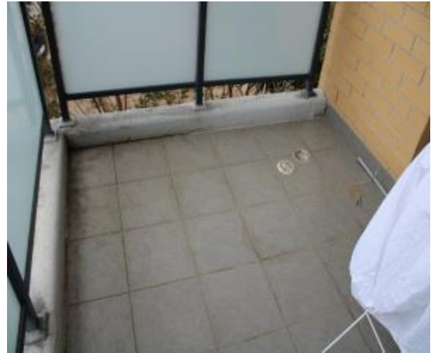
Figure 1254 - General condition of balcony floor tiles
