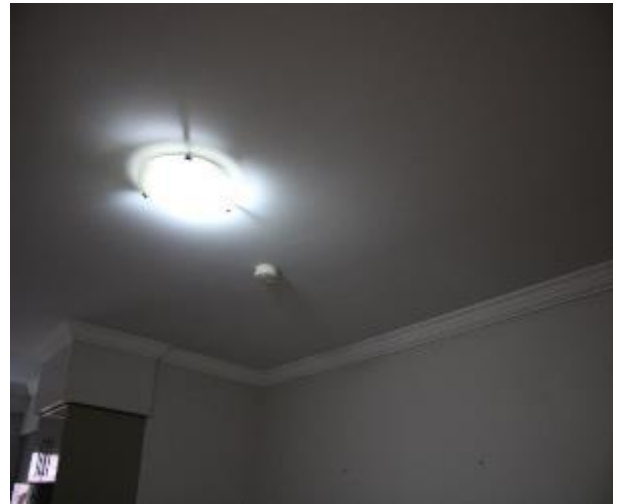
Figure 640 - General condition of lounge room ceiling
