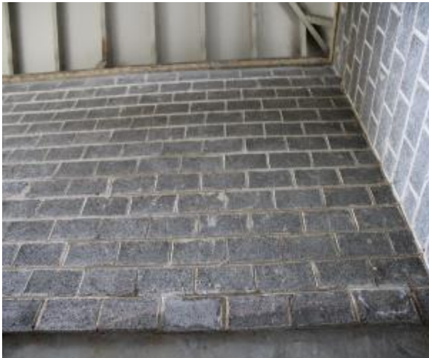
Figure 253 - General condition of level 1 fire stairs internal wall
