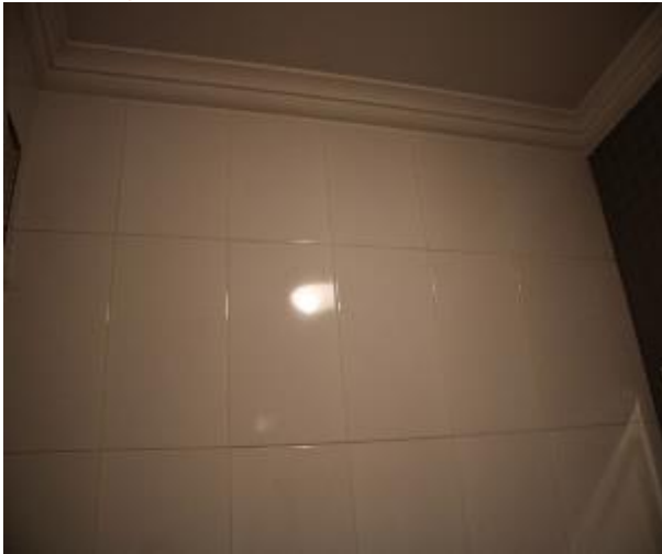
Figure 1631 - General condition of ensuite bathroom internal wall
