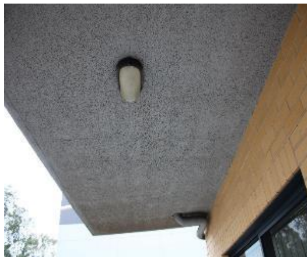
Figure 1266 - General condition of balcony underside slab
