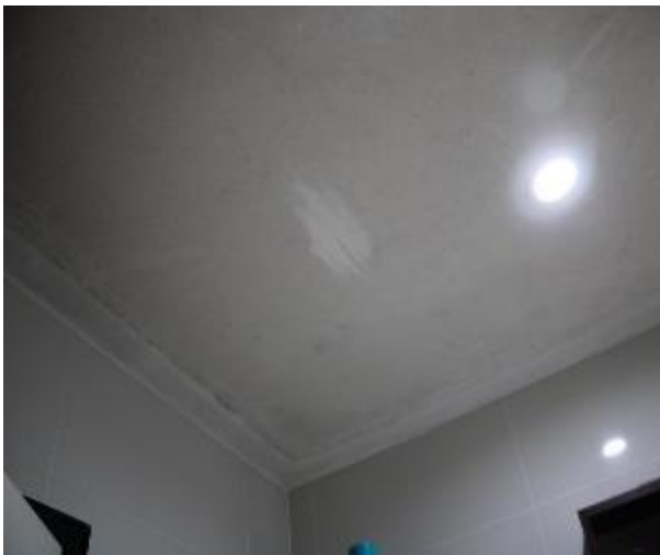
Figure 890 - General condition of bathroom 1 ceiling
