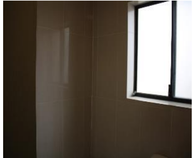
Figure 1347 - General condition of bathroom 1 internal wall
