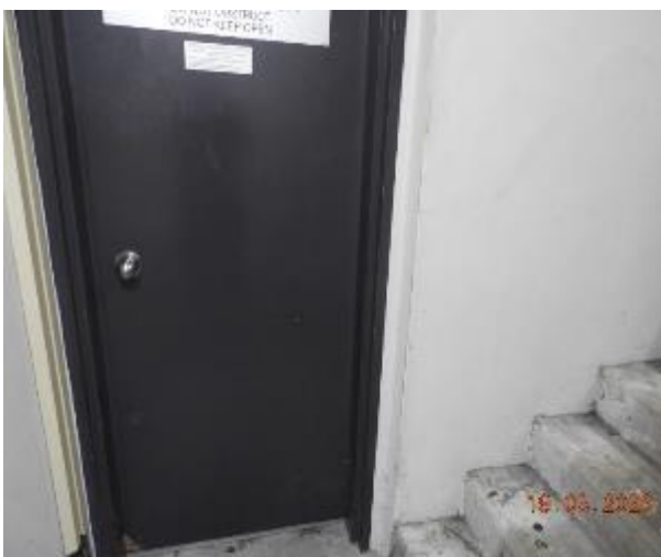
Figure 424 - General condition of level 1 fire stairs internal wall
