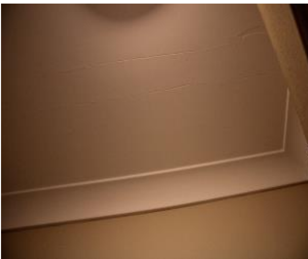
Figure 1326 - General condition of laundry ceiling
