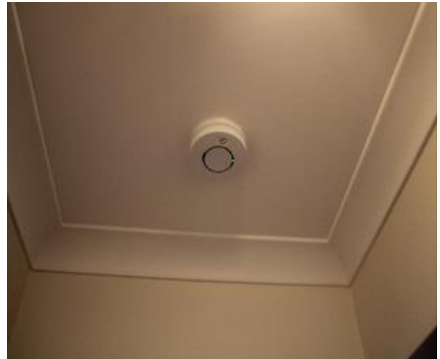
Figure 1154 - General condition of corridor ceiling
