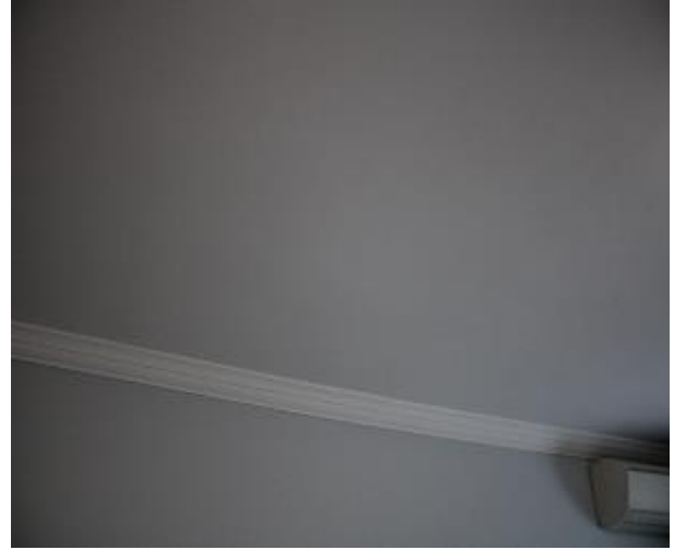
Figure 490 - General condition of open kitchen/ lounge room ceiling
