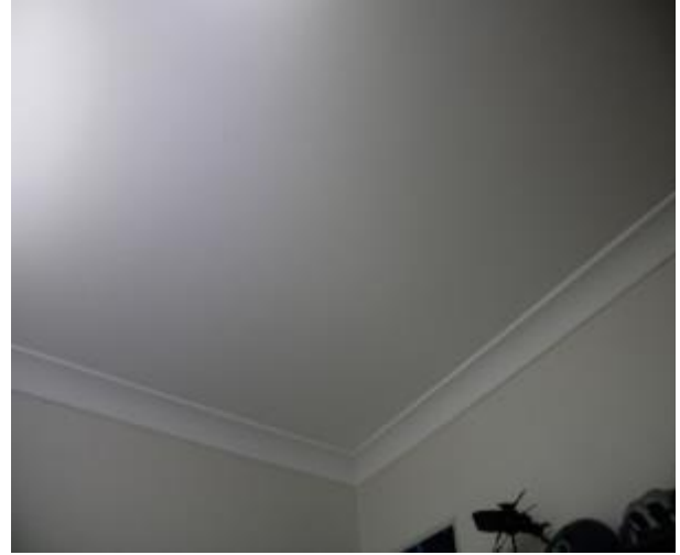
Figure 919 - General condition of bedroom 3 ceiling
