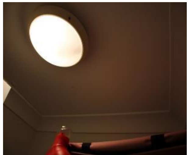
Figure 1138 - General condition of laundry ceiling
