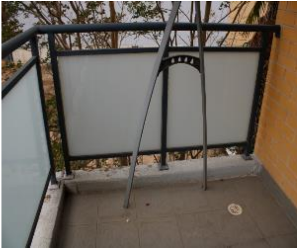
Figure 841 - General condition of balcony balustrade
