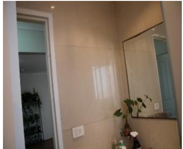
Figure 1017 - General condition of bathroom 1 internal wall
