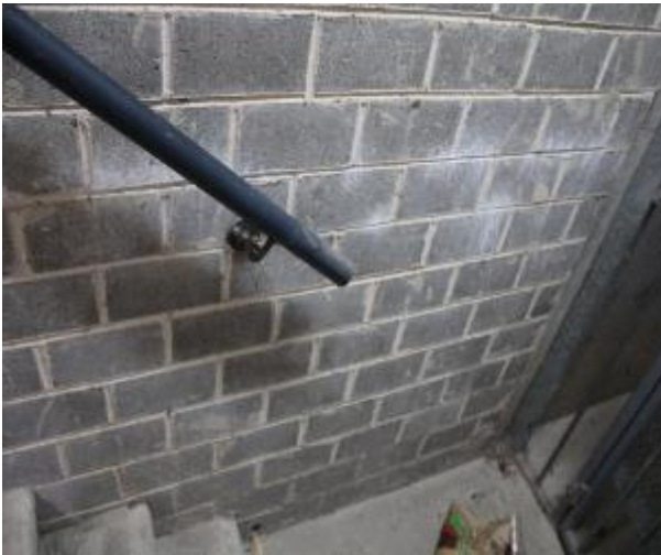
Figure 247 - General condition of level 1 fire stairs internal wall
