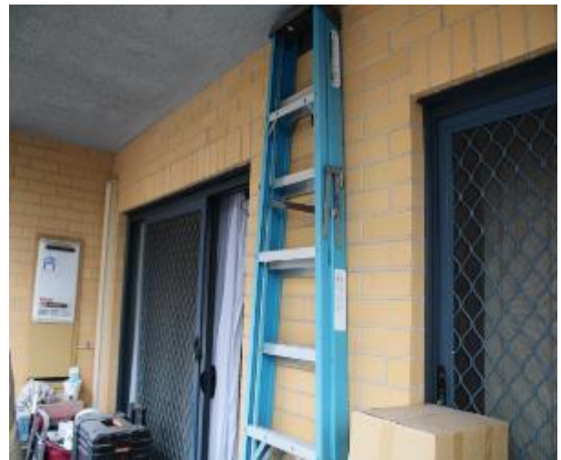
Figure 927 - General condition of external wall
