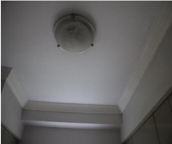
Figure 649 - General condition of kitchen ceiling
