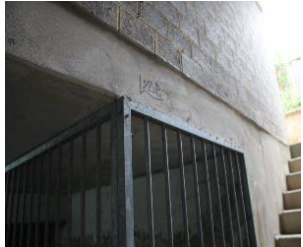
Figure 270 - General condition of fire stairs underside slab
