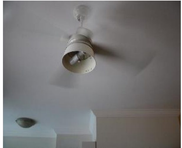
Figure 865 - General condition of bedroom 1 ceiling
