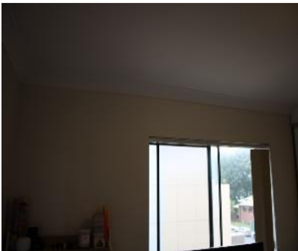
Figure 1237 - General condition of bedroom 2 internal wall
