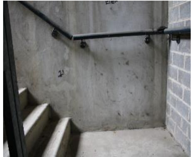
Figure 252 - General condition of level 1 fire stairs internal wall
