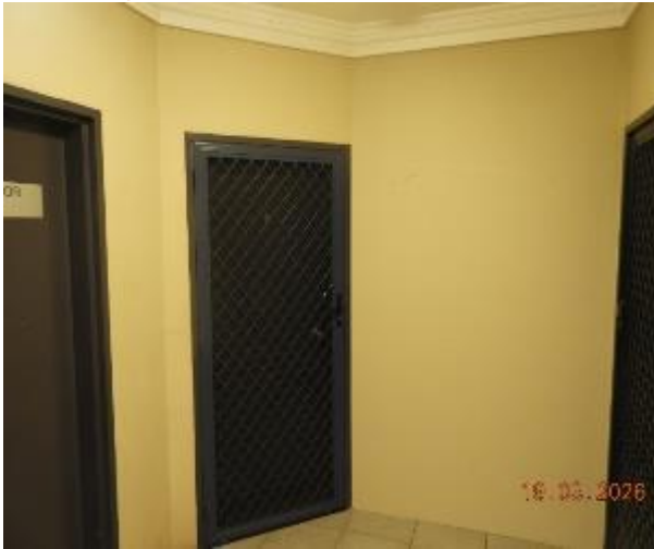
Figure 85 - General condition of level 3 common area internal wall
