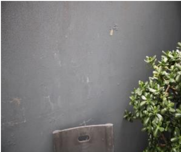
Figure 613 - General condition of courtyard external wall
