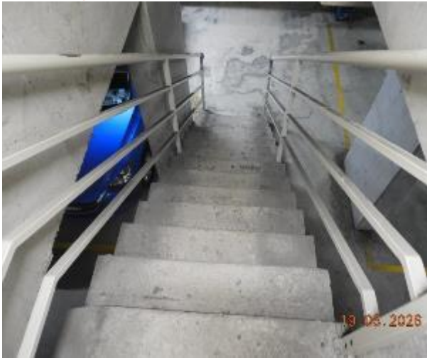
Figure 468 - General condition of basement fire stairs
