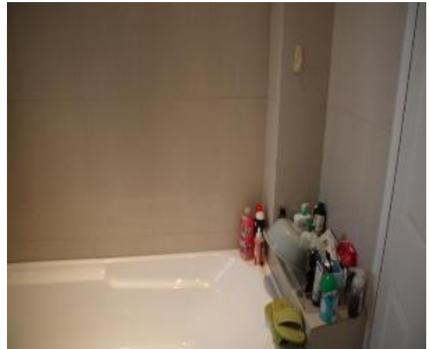
Figure 1011 - General condition of bathroom 1 internal wall
