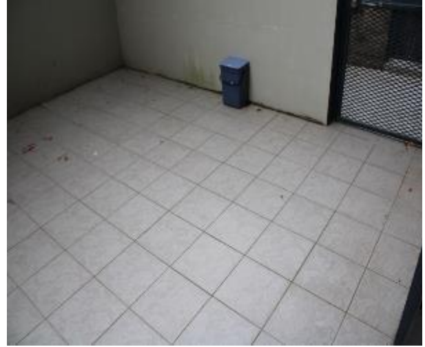
Figure 496 - General condition of courtyard floor tiles
