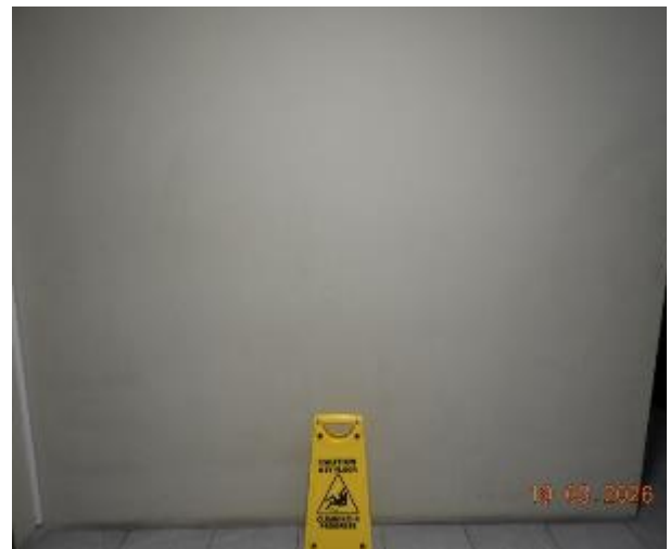
Figure 166 - General condition of level 5 common area internal wall
