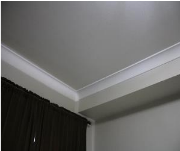
Figure 801 - General condition of bedroom 1 ceiling
