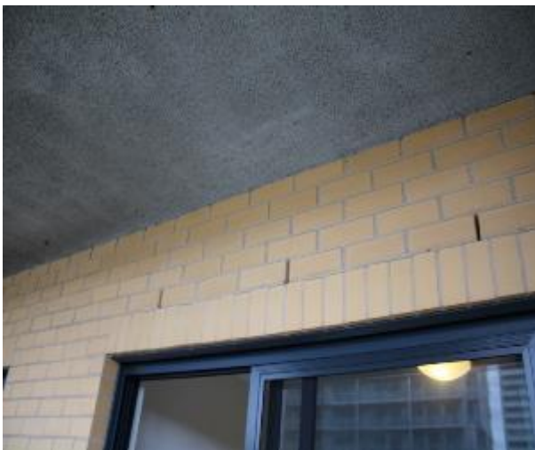
Figure 1088 - General condition of external wall
