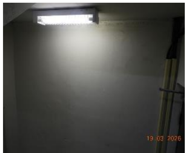
Figure 389 - General condition of level 2 fire stairs internal wall
