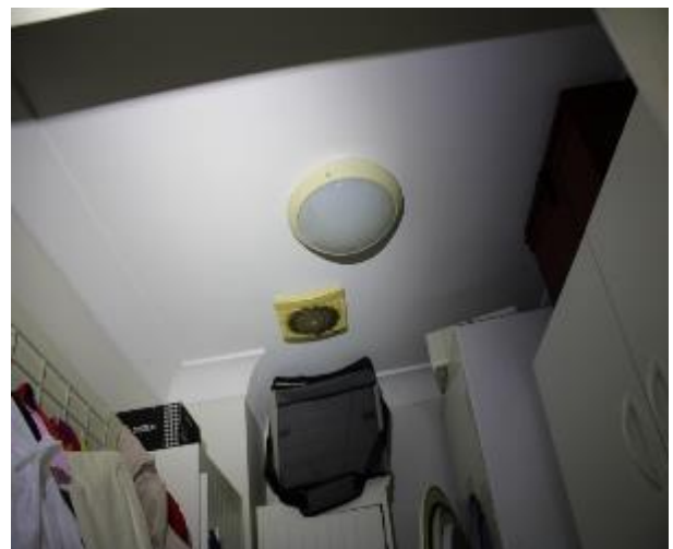
Figure 875 - General condition of laundry ceiling
