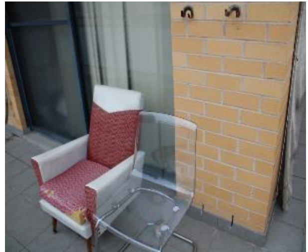
Figure 1526 - General condition of external wall
