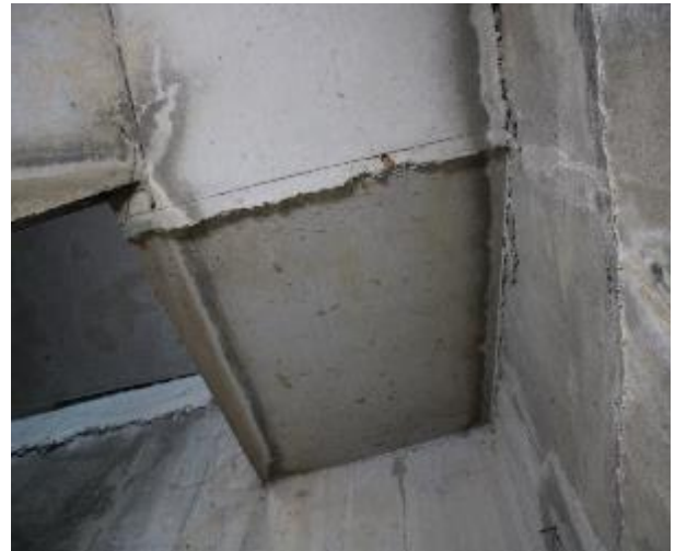
Figure 212 - General condition of B2 fire stairs underside stairs
