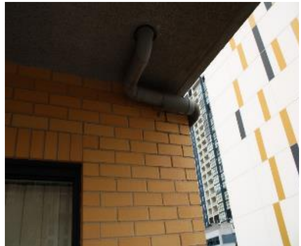
Figure 1445 - General condition of external wall
