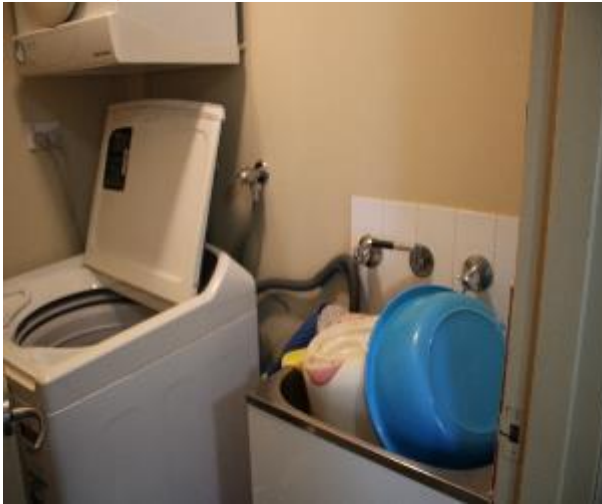
Figure 1316 - General condition of laundry internal wall
