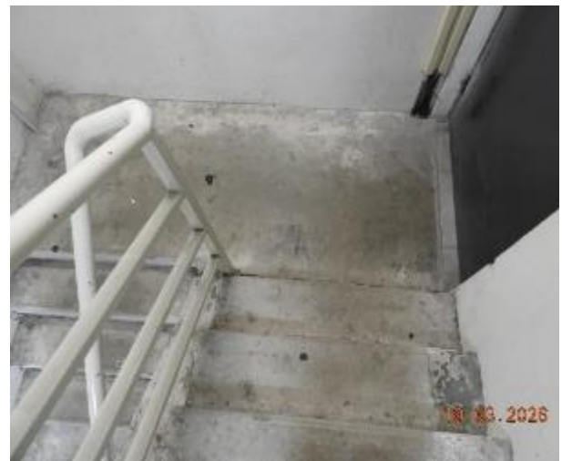
Figure 381 - General condition of level 2 fire stairs
