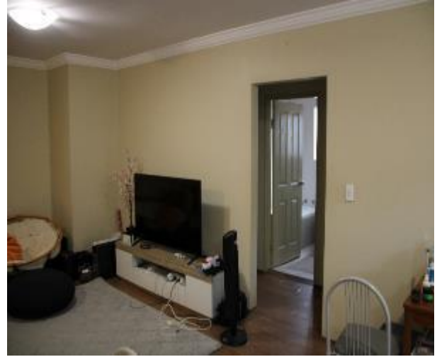
Figure 1287 - General condition of lounge room internal wall
