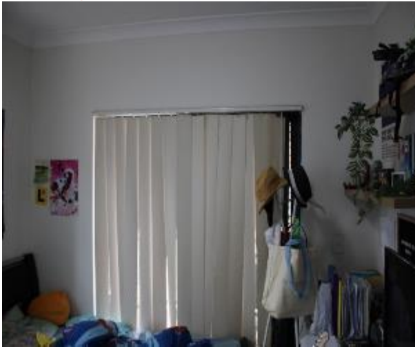
Figure 912 - General condition of bedroom 3 internal wall
