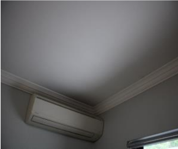
Figure 491 - General condition of open kitchen/ lounge room ceiling
