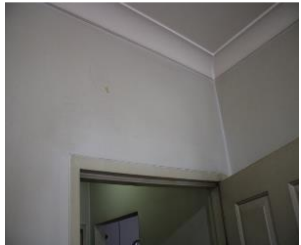
Figure 822 - General condition of study internal wall
