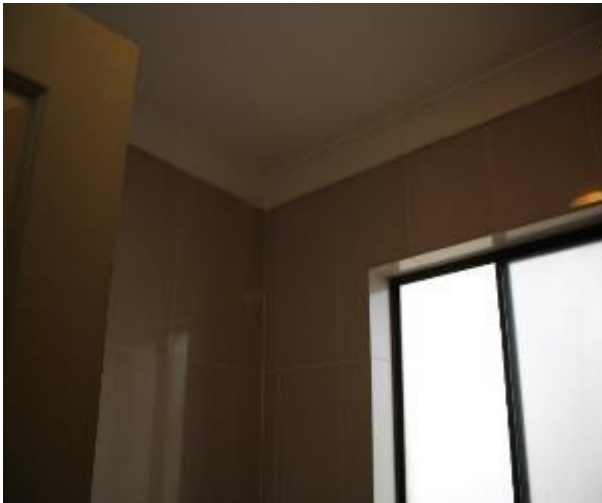
Figure 1348 - General condition of bathroom 1 internal wall
