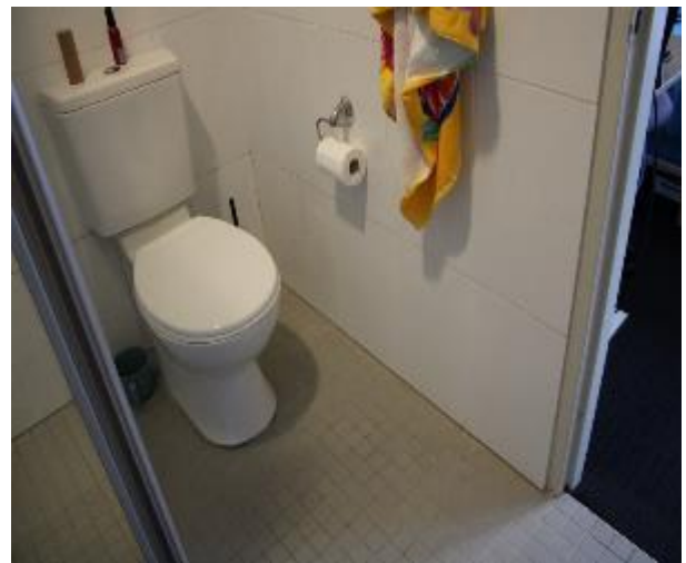
Figure 1622 - General condition of ensuite bathroom internal wall
