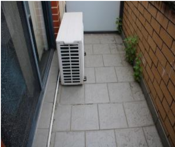
Figure 1513 - General condition of external wall
