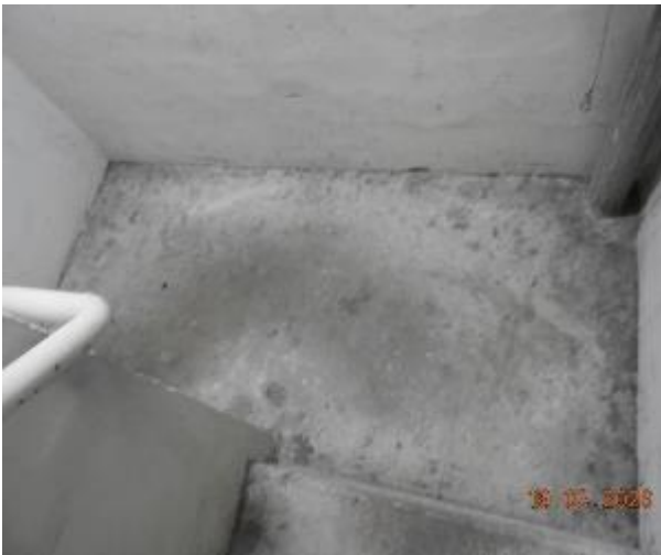
Figure 404 - General condition of level 1 fire stairs
