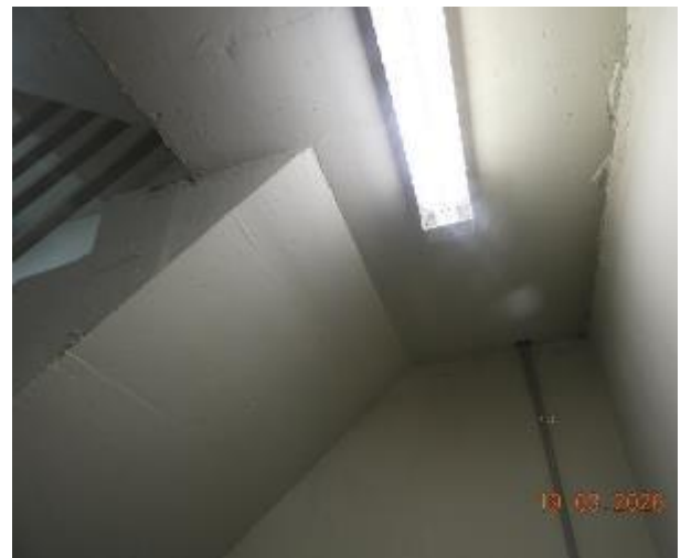
Figure 393 - General condition of level 2 fire stairs underside stairs
