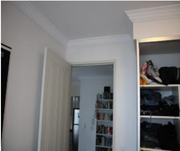
Figure 1565 - General condition of bedroom 2 internal wall
