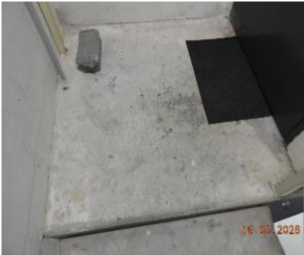
Figure 278 - General condition of level 5 fire stairs concrete floor
