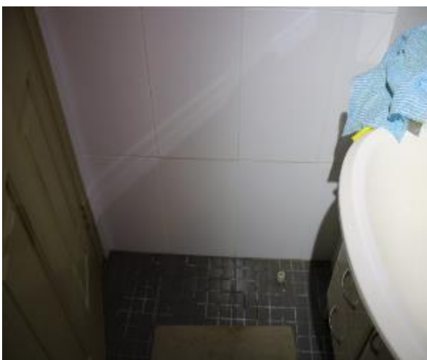
Figure 1404 - General condition of ensuite bathroom internal wall
