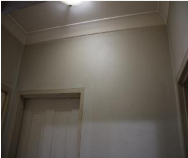
Figure 769 - General condition of corridor internal wall
