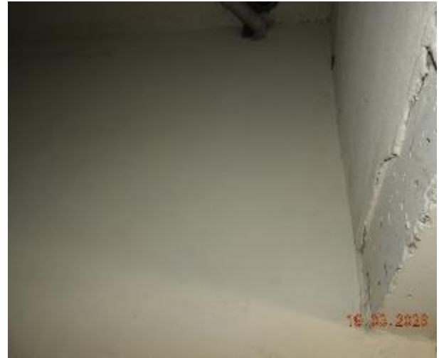
Figure 463 - General condition of basement fire stairs internal wall
