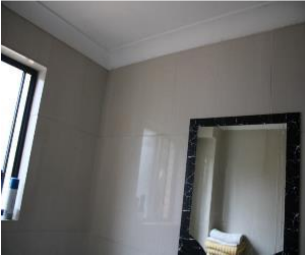
Figure 783 - General condition of bathroom 1 internal wall
