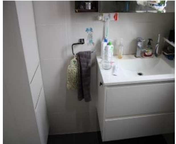
Figure 883 - General condition of bathroom 1 internal wall
