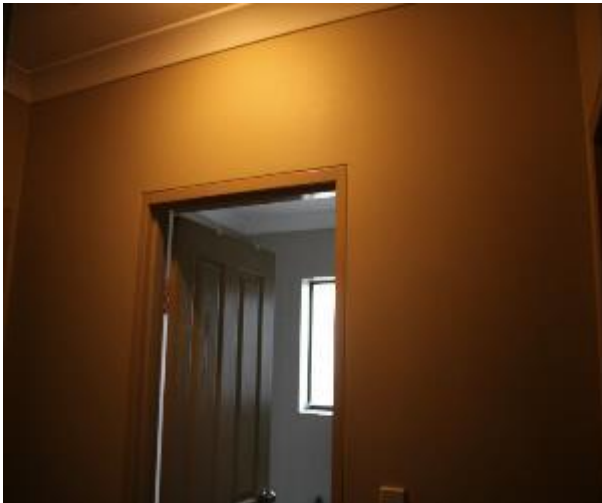
Figure 1330 - General condition of corridor internal wall
