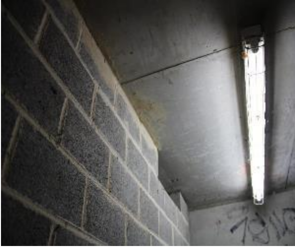
Figure 275 - General condition of fire stairs underside slab
