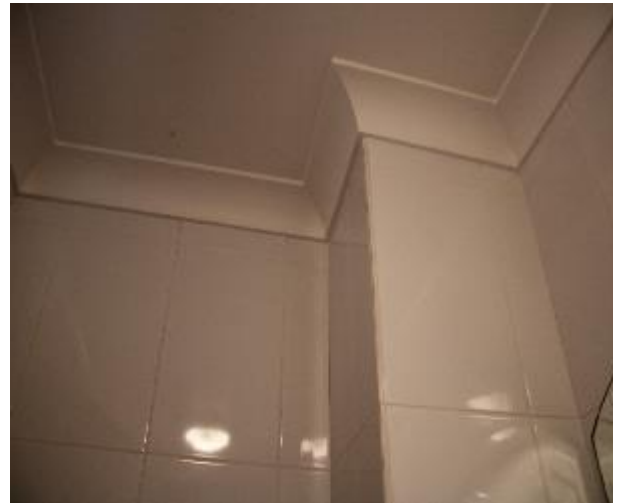
Figure 909 - General condition of ensuite bathroom internal wall
