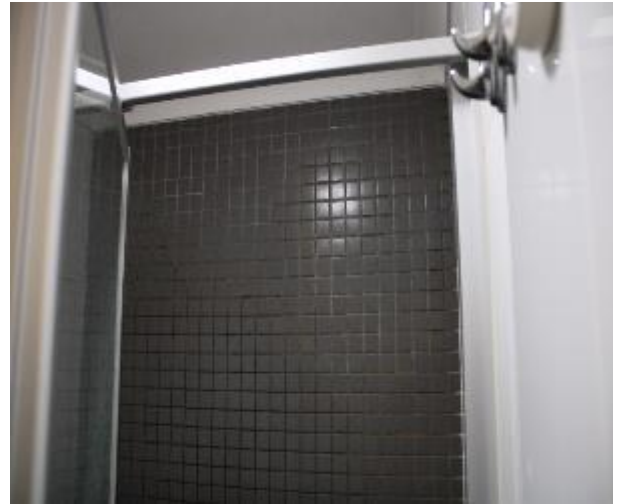
Figure 716 - General condition of ensuite bathroom internal wall
