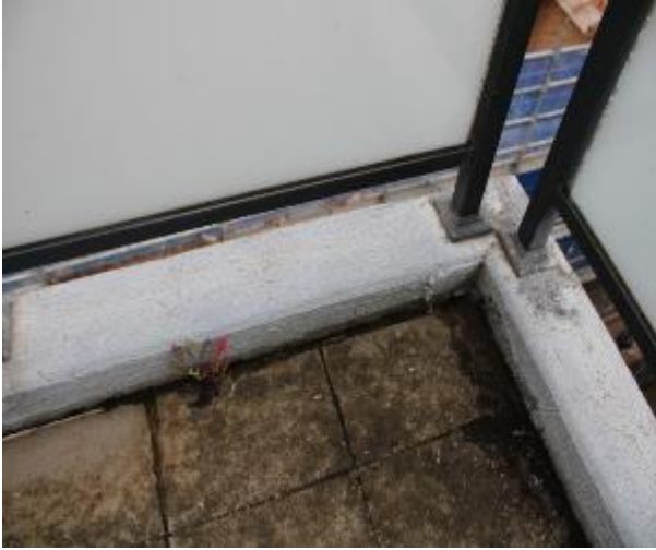
Figure 1505 - General condition of balcony floor tiles
