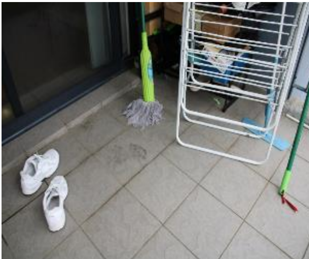
Figure 1082 - General condition of balcony floor tiles
