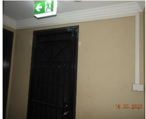
Figure 158 - General condition of level 5 common area internal wall
