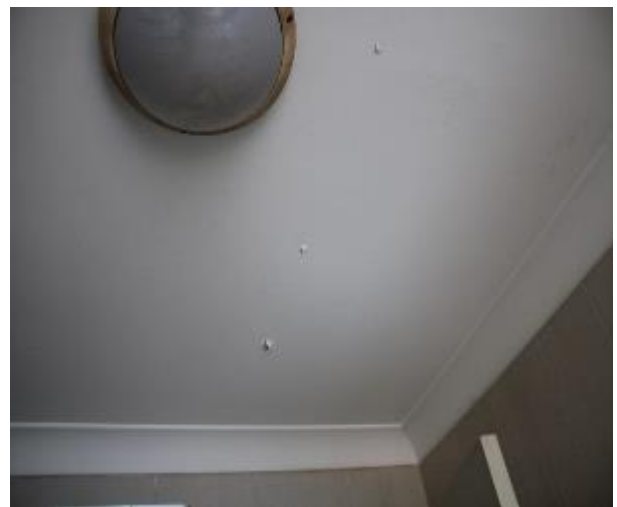
Figure 786 - General condition of bathroom 1 ceiling
