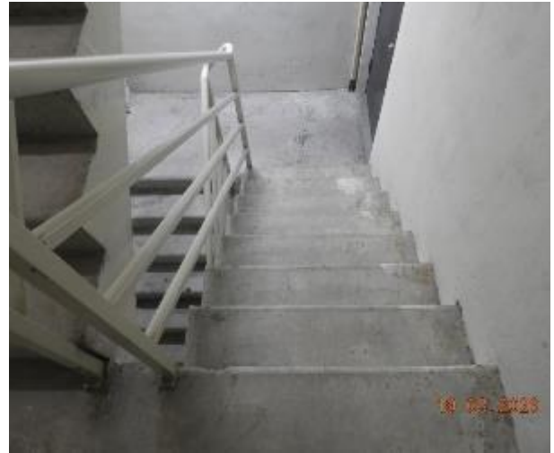
Figure 313 - General condition of level 4 fire stairs
