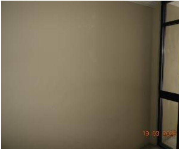
Figure 7 - General condition of level 1 common area internal wall
