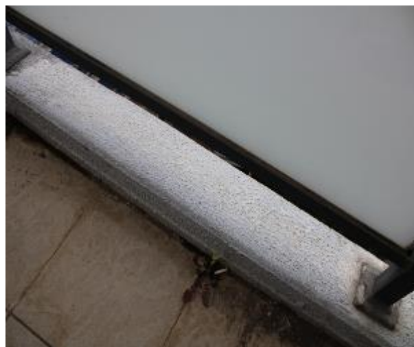
Figure 1502 - General condition of balcony floor tiles
