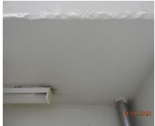
Figure 339 - General condition of level 3 fire stairs underside stairs
