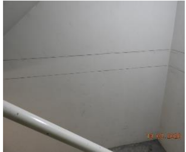
Figure 373 - General condition of level 2 fire stairs internal wall
