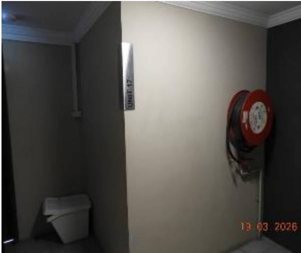
Figure 151 - General condition of level 5 common area internal wall
