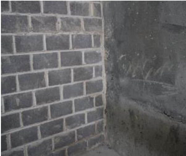
Figure 227 - General condition of B1 fire stairs internal wall
