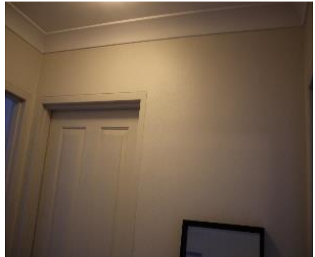
Figure 1148 - General condition of corridor internal wall
