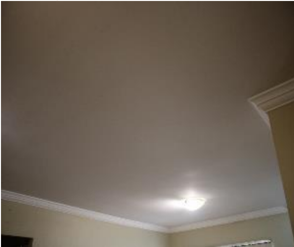
Figure 1298 - General condition of lounge room ceiling
