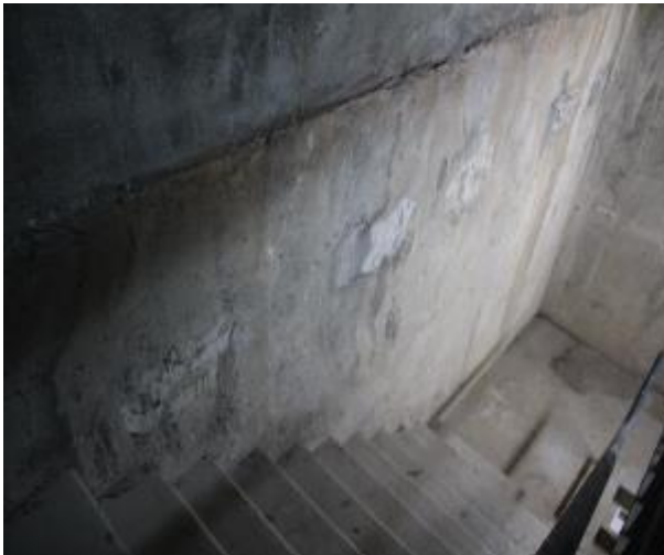
Figure 217 - General condition of B1 fire stairs internal wall
