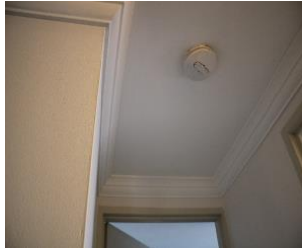
Figure 1578 - General condition of corridor ceiling
