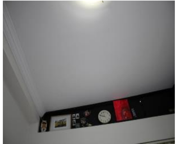
Figure 1560 - General condition of bedroom 1 ceiling
