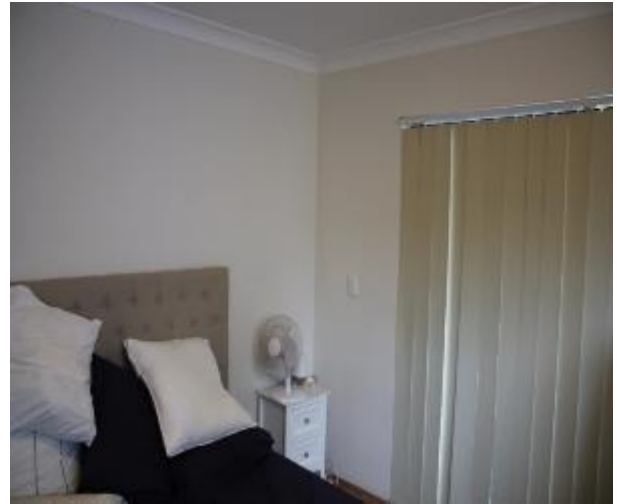
Figure 1230 - General condition of bedroom 2 internal wall
