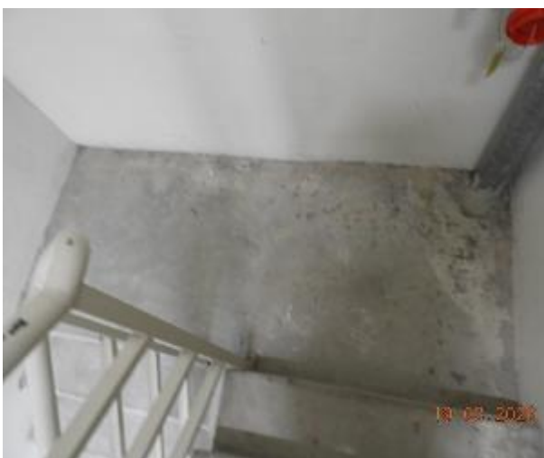
Figure 292 - General condition of level 5 fire stairs
