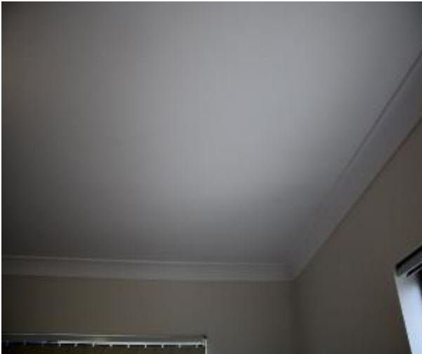
Figure 1243 - General condition of bedroom 2 ceiling
