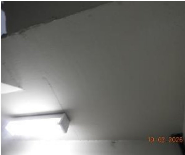
Figure 356 - General condition of level 3 fire stairs underside stairs
