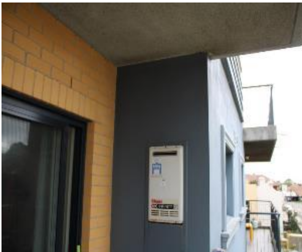
Figure 1084 - General condition of external wall
