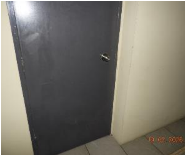
Figure 21 - General condition of level 1 common area internal wall
