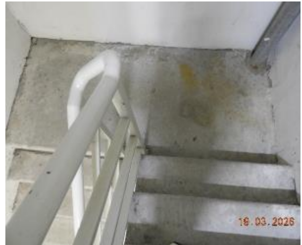
Figure 327 - General condition of level 3 fire stairs
