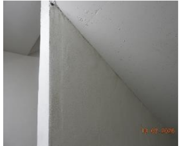
Figure 415 - General condition of level 1 fire stairs internal wall
