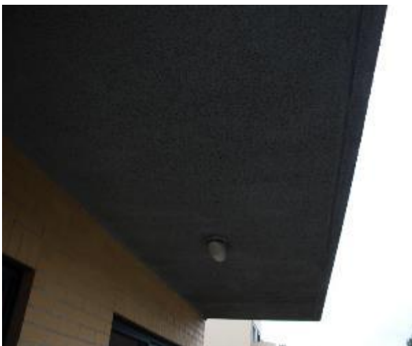
Figure 665 - General condition of balcony underside slab
