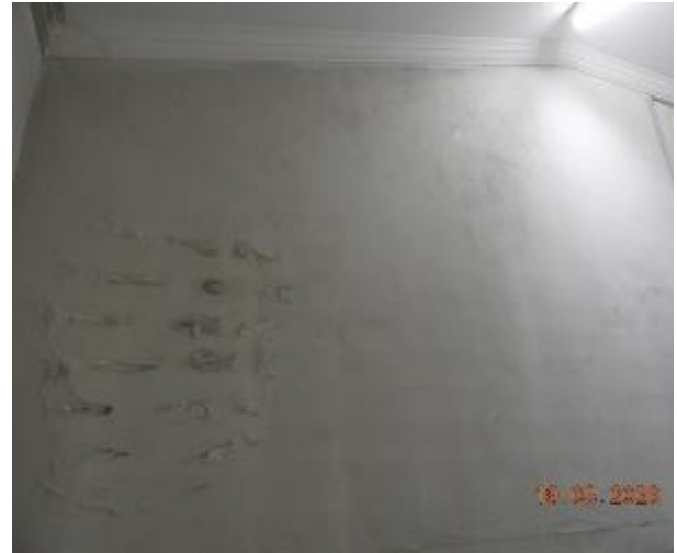
Figure 295 - General condition of level 5 fire stairs internal wall
