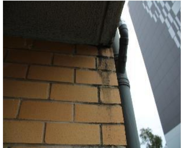
Figure 656 - Crack propagation through external wall
