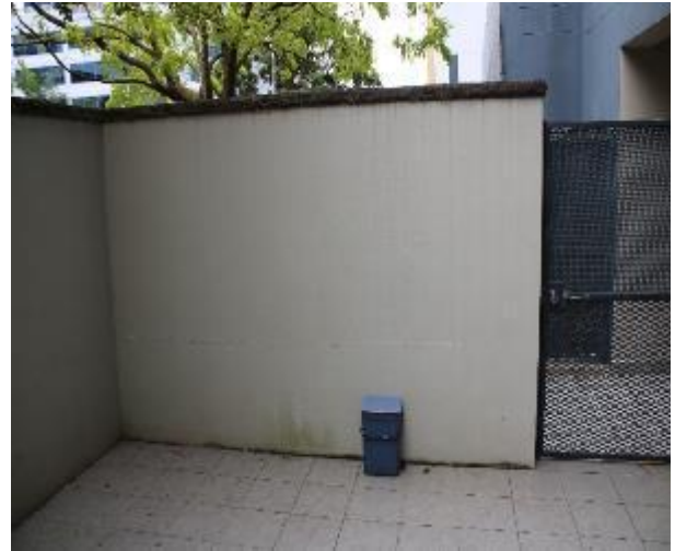
Figure 514 - General condition of courtyard external wall
