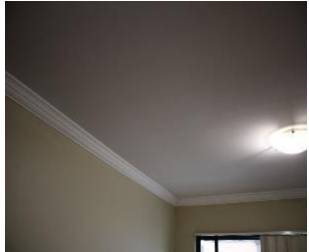
Figure 1299 - General condition of lounge room ceiling
