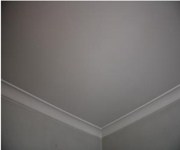
Figure 823 - General condition of study ceiling
