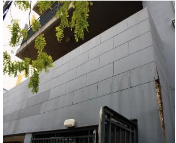
Figure 600 - General condition of external wall
