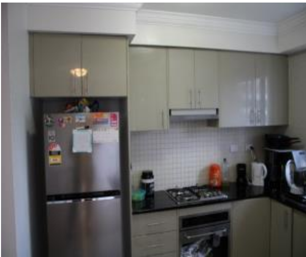
Figure 964 - General condition of kitchen internal wall
