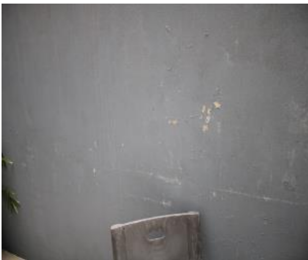
Figure 615 - General condition of courtyard external wall
