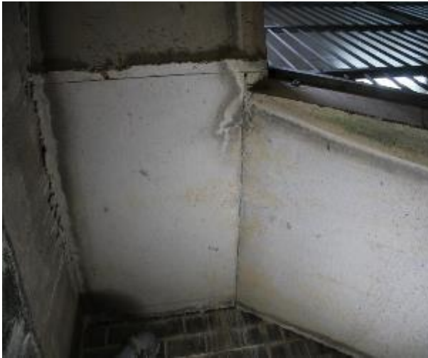
Figure 209 - General condition of B2 fire stairs underside stairs
