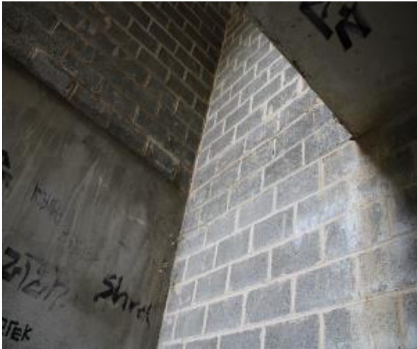
Figure 251 - General condition of level 1 fire stairs internal wall
