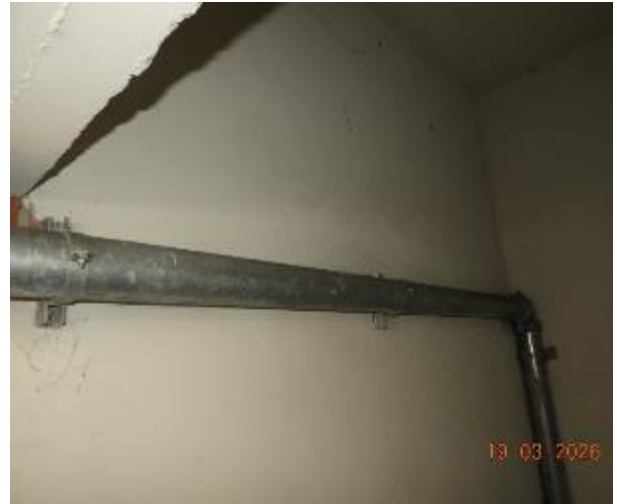
Figure 457 - General condition of basement fire stairs internal wall
