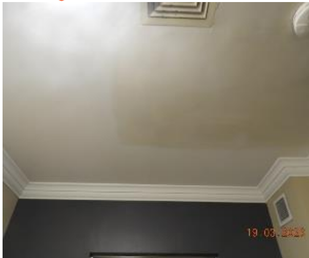
Figure 181 - General condition of level 5 common area ceiling
