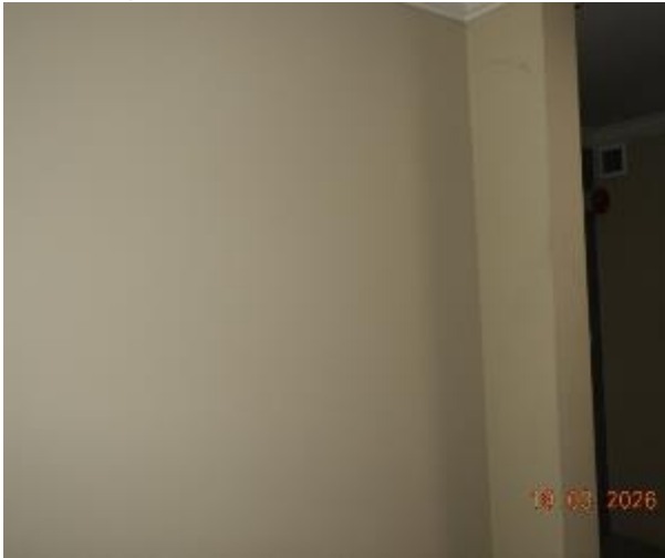
Figure 19 - General condition of level 1 common area internal wall
