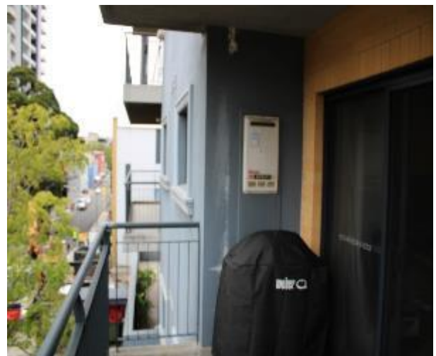
Figure 660 - General condition of external wall
