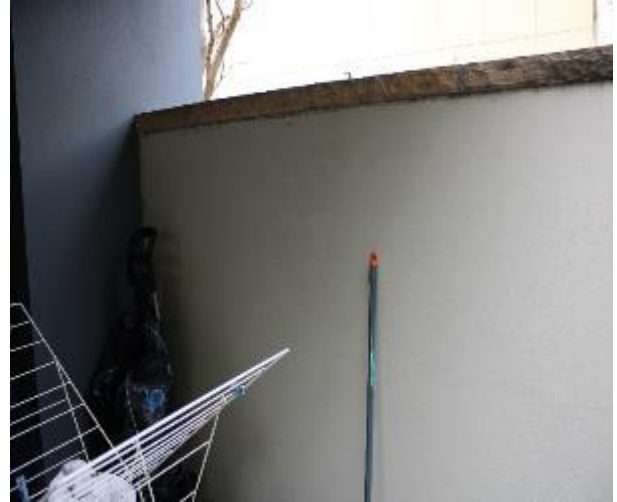
Figure 520 - General condition of courtyard external wall
