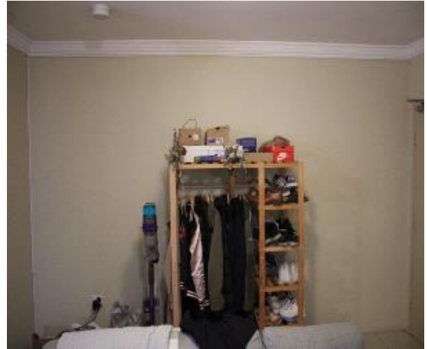
Figure 1277 - General condition of lounge room internal wall
