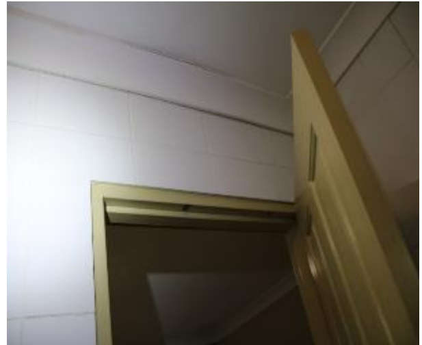
Figure 1407 - General condition of ensuite bathroom internal wall
