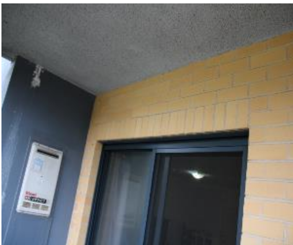
Figure 659 - General condition of external wall
