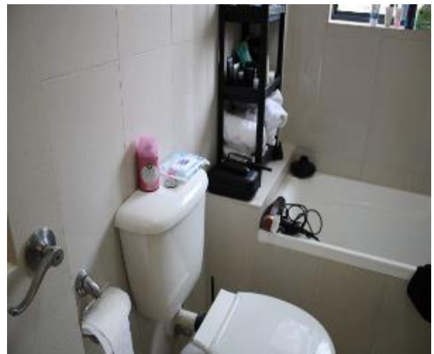
Figure 1166 - General condition of bathroom 1 internal wall
