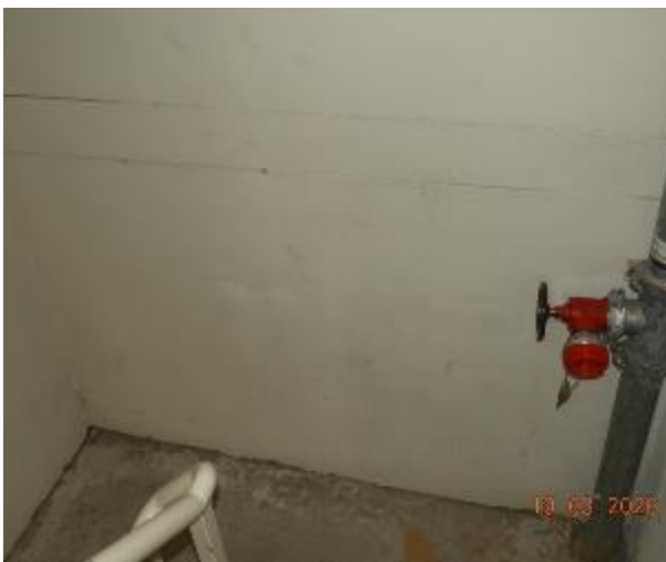
Figure 334 - General condition of level 3 fire stairs internal wall
