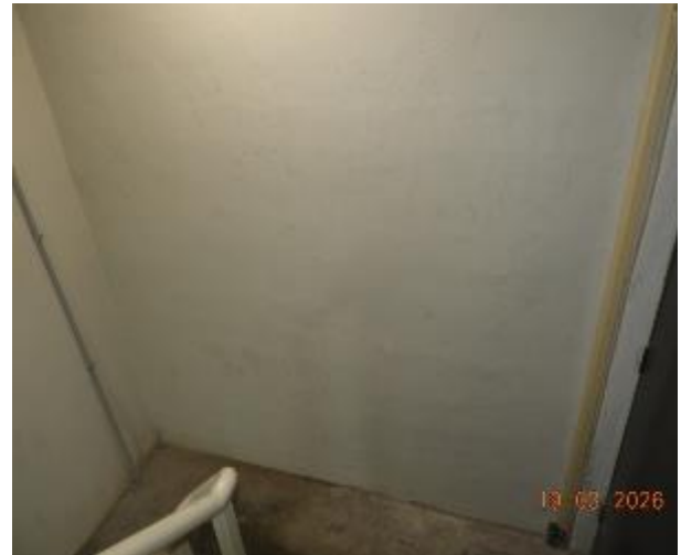
Figure 351 - General condition of level 3 fire stairs internal wall
