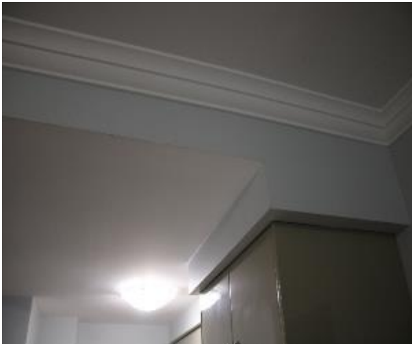
Figure 485 - General condition of open kitchen/ lounge room ceiling
