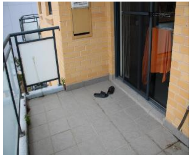
Figure 1528 - General condition of external wall
