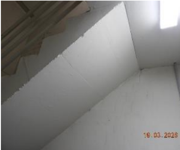
Figure 324 - General condition of level 4 fire stairs underside stairs
