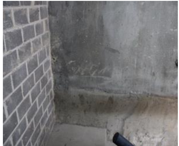
Figure 218 - General condition of B1 fire stairs internal wall
