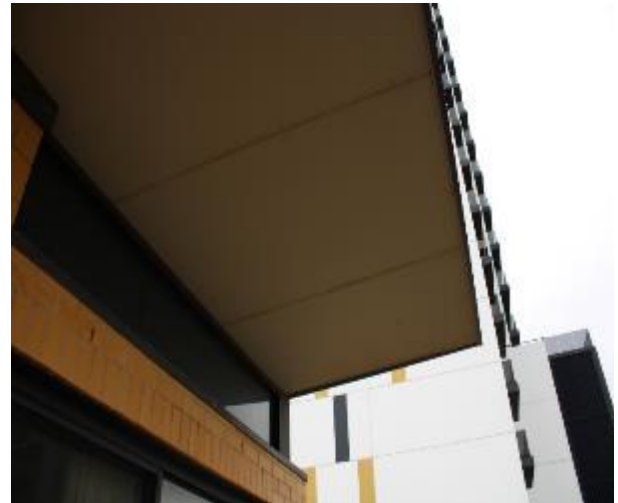
Figure 1532 - General condition of balcony underside slab
