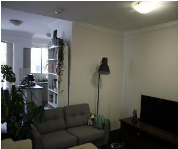
Figure 1453 - General condition of open kitchen/ lounge room internal wall
