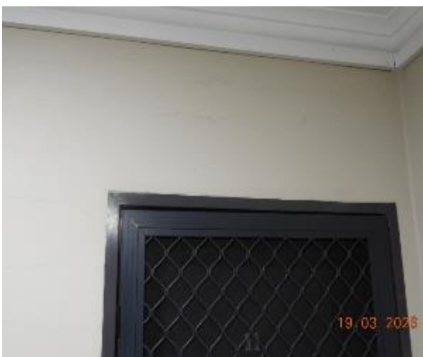
Figure 101 - General condition of level 3 common area internal wall
