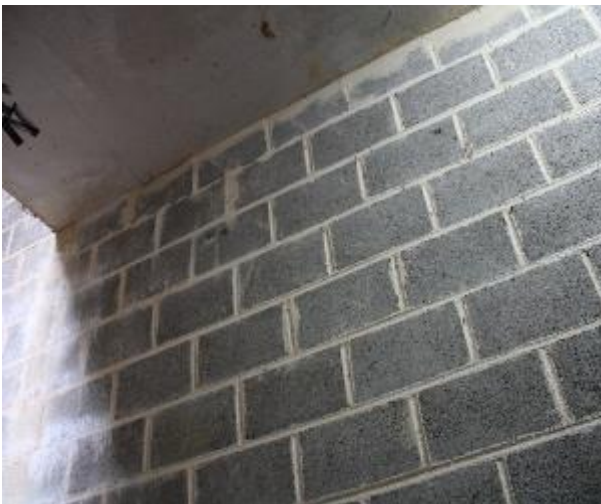
Figure 249 - General condition of level 1 fire stairs internal wall
