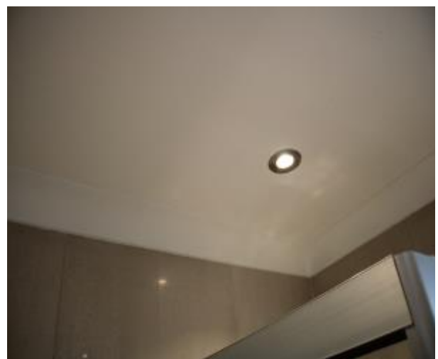
Figure 1025 - General condition of bathroom 1 ceiling
