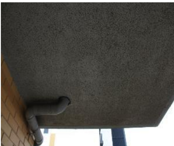
Figure 1446 - General condition of balcony underside slab
