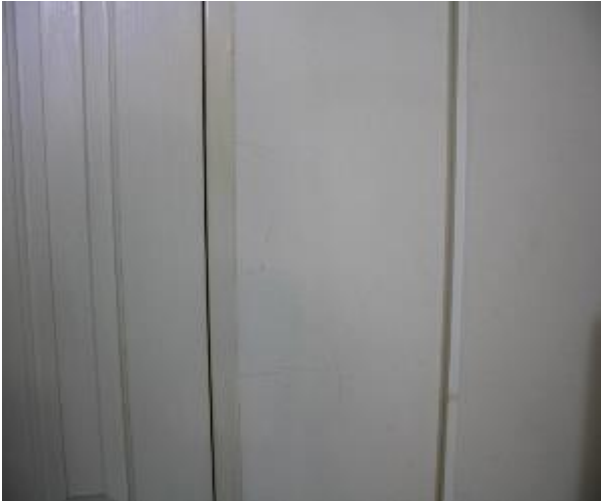
Figure 735 - General condition of open kitchen/ lounge room internal wall
