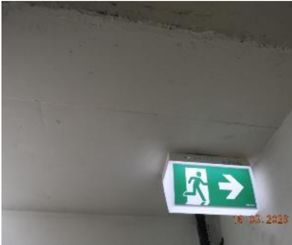
Figure 438 - General condition of level 1 fire stairs underside stairs
