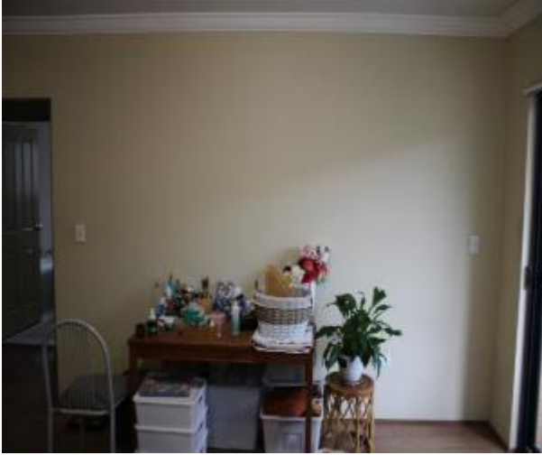
Figure 1286 - General condition of lounge room internal wall
