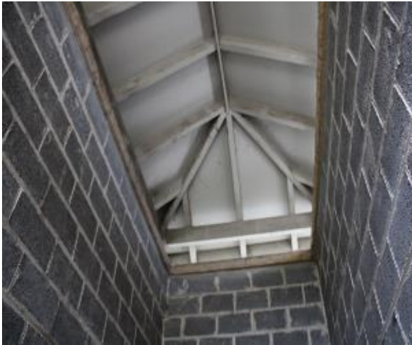
Figure 269 - General condition of level 1 fire stairs roof structure
