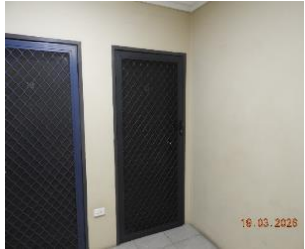
Figure 98 - General condition of level 3 common area internal wall
