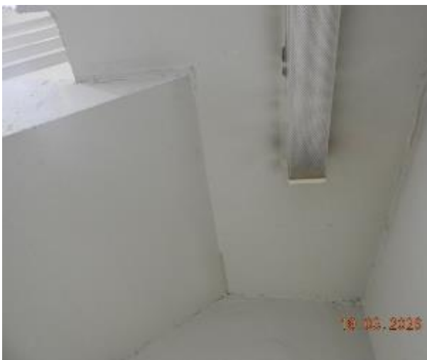
Figure 340 - General condition of level 3 fire stairs underside stairs
