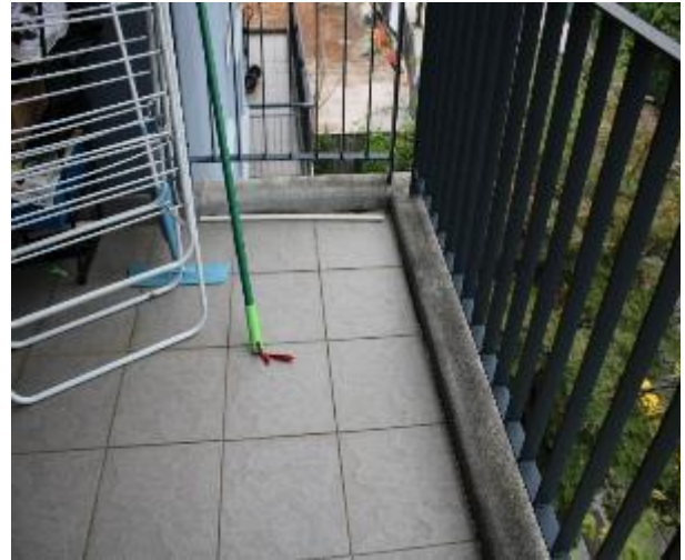
Figure 1081 - General condition of balcony floor tiles
