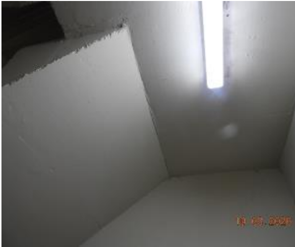
Figure 378 - General condition of level 2 fire stairs underside stairs
