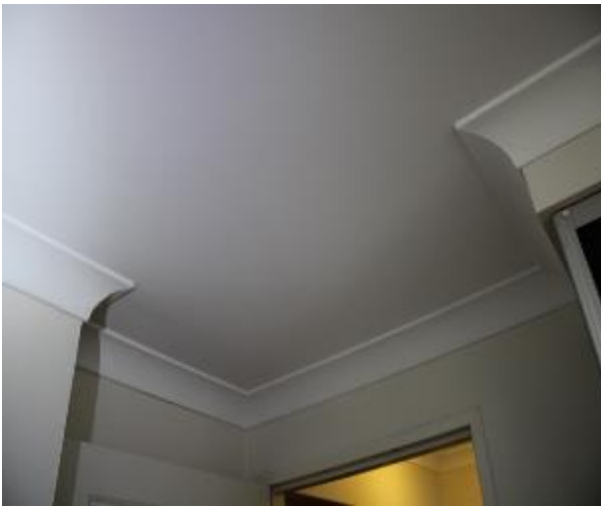
Figure 1201 - General condition of bedroom 1 ceiling
