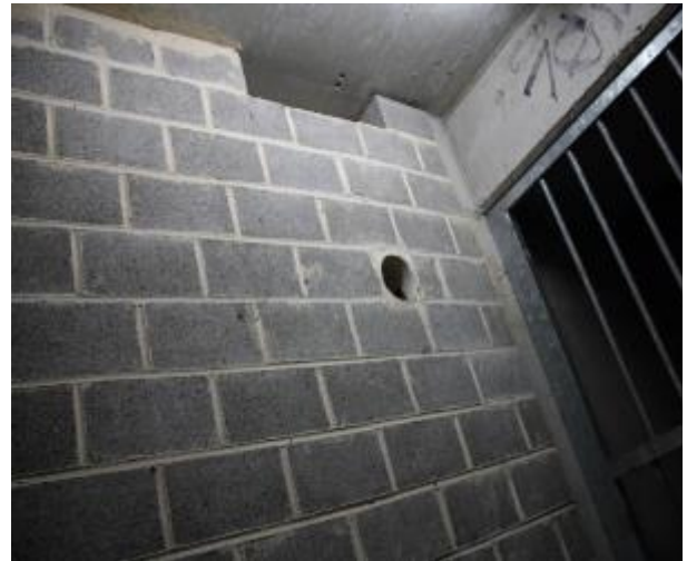
Figure 248 - General condition of level 1 fire stairs internal wall
