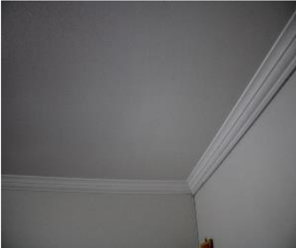
Figure 950 - General condition of lounge room ceiling
