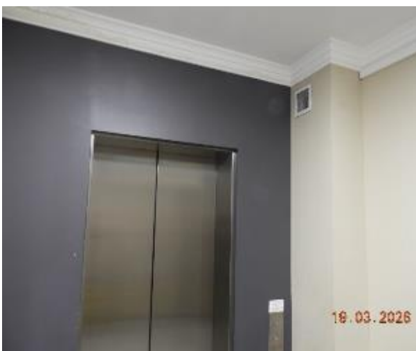
Figure 71 - General condition of level 2 common area internal wall
