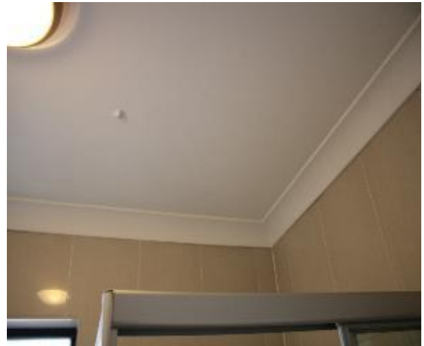
Figure 1361 - General condition of bathroom 1 ceiling
