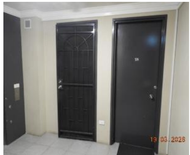
Figure 172 - General condition of level 5 common area internal wall
