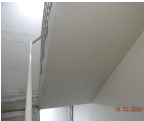
Figure 394 - General condition of level 2 fire stairs underside stairs
