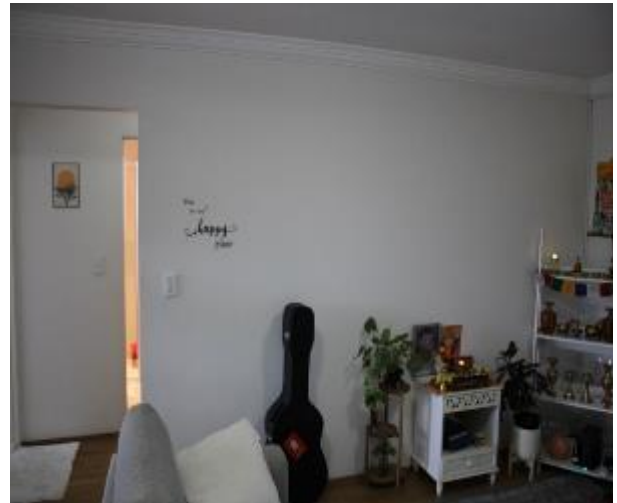
Figure 939 - General condition of lounge room internal wall
