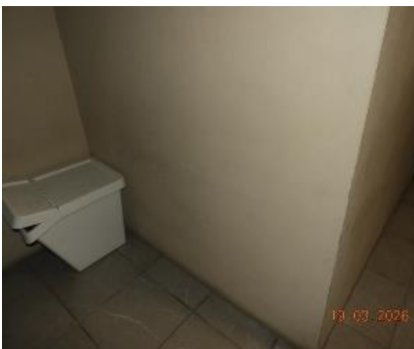
Figure 155 - General condition of level 5 common area internal wall
