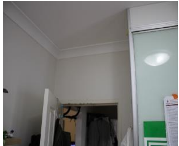
Figure 915 - General condition of bedroom 3 internal wall
