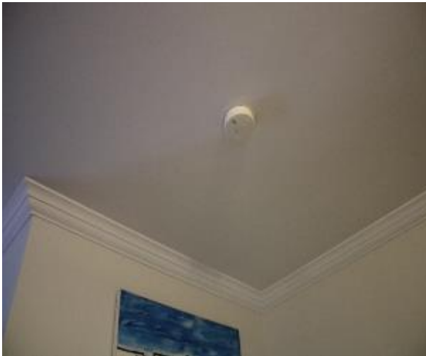
Figure 860 - General condition of bedroom 1 ceiling
