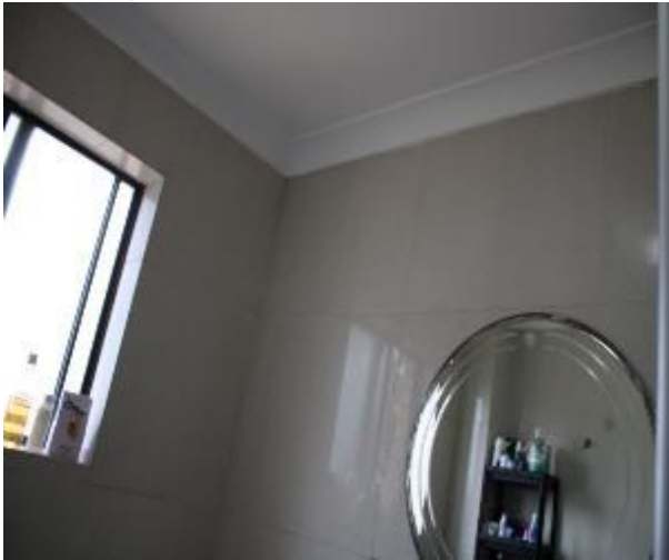
Figure 1169 - General condition of bathroom 1 internal wall
