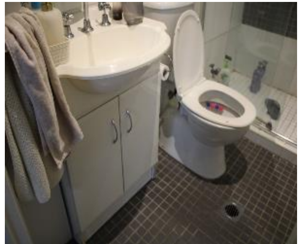
Figure 1041 - General condition of ensuite bathroom floor tiles
