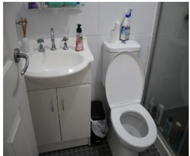
Figure 1208 - General condition of ensuite bathroom internal wall
