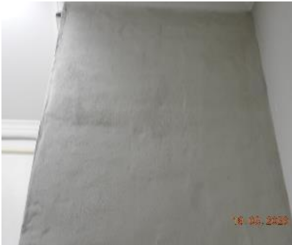
Figure 308 - General condition of level 5 fire stairs internal wall
