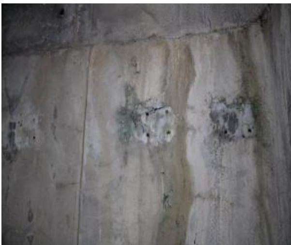
Figure 201 - General condition of B2 fire stairs internal wall
