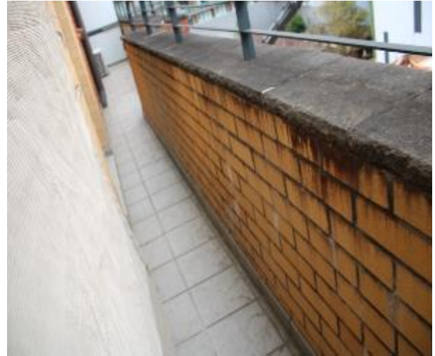
Figure 1538 - General condition of balcony balustrade
