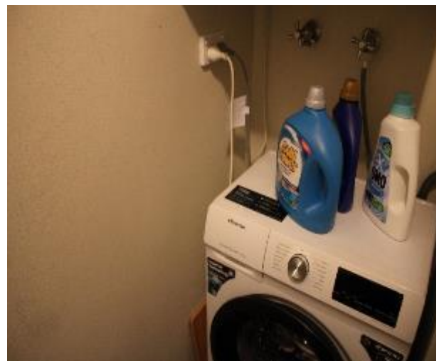
Figure 574 - General condition of laundry internal wall
