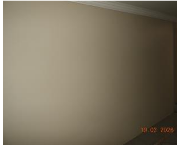
Figure 14 - General condition of level 1 common area internal wall
