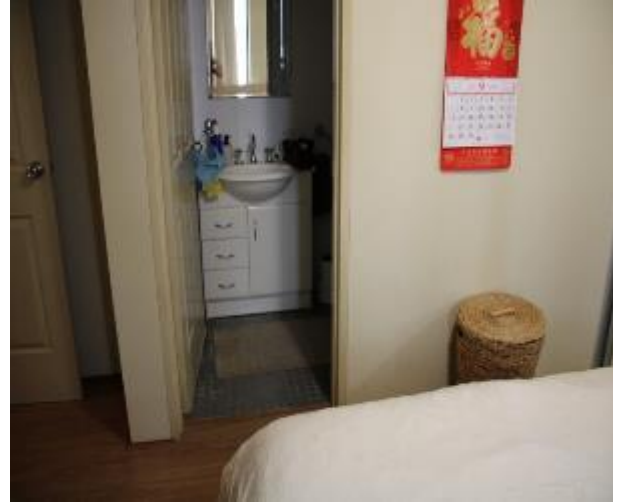
Figure 1371 - General condition of bedroom 1 internal wall
