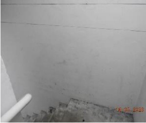
Figure 408 - General condition of level 1 fire stairs internal wall
