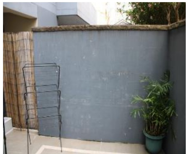
Figure 616 - General condition of courtyard external wall
