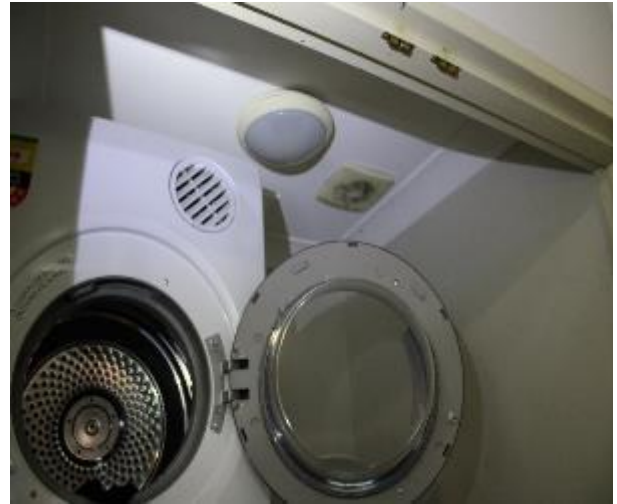
Figure 674 - General condition of laundry ceiling
