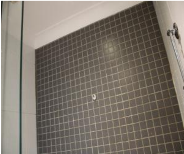
Figure 1044 - General condition of ensuite bathroom internal wall
