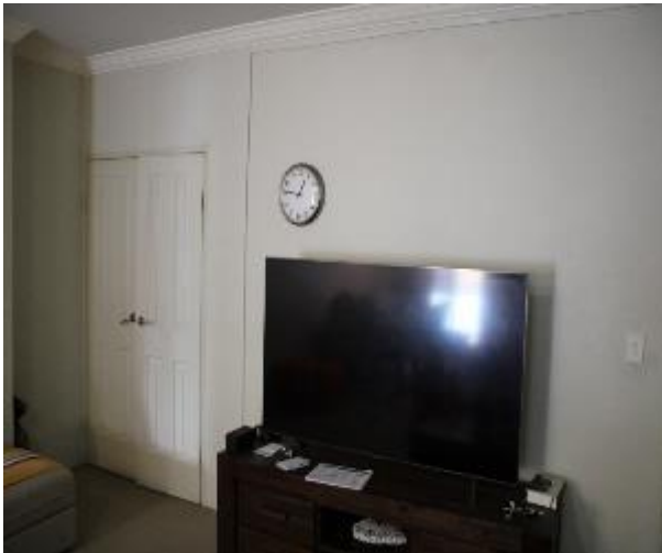
Figure 729 - General condition of open kitchen/ lounge room internal wall
