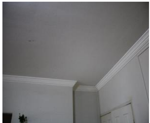
Figure 762 - General condition of open kitchen/ lounge room ceiling
