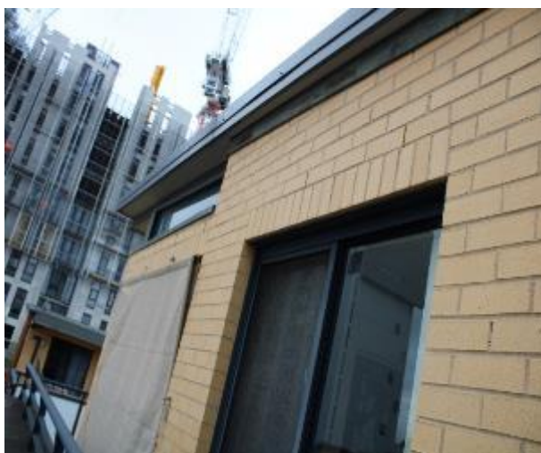
Figure 1521 - General condition of external wall
