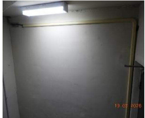
Figure 319 - General condition of level 4 fire stairs internal wall
