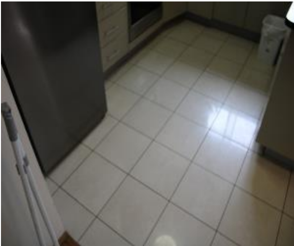
Figure 962 - General condition of kitchen floor tiles
