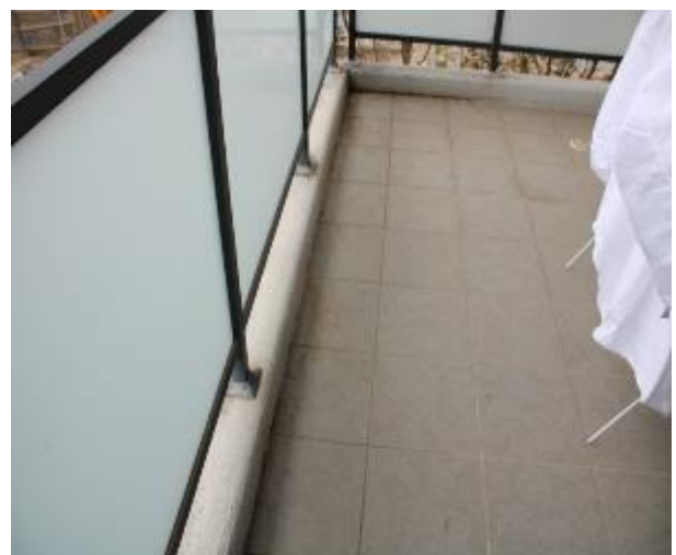
Figure 1252 - General condition of balcony floor tiles
