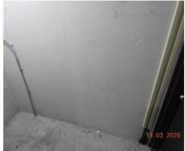
Figure 427 - General condition of level 1 fire stairs internal wall
