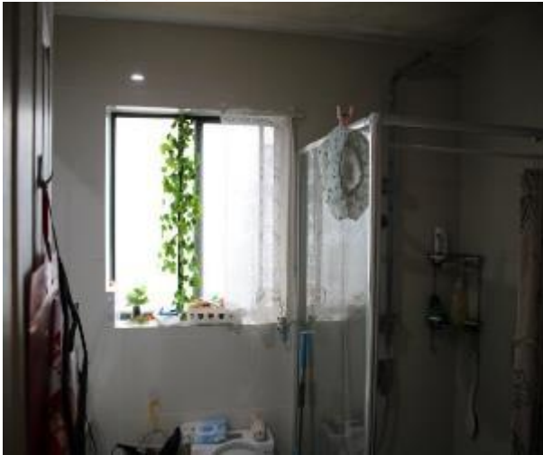
Figure 882 - General condition of bathroom 1 internal wall
