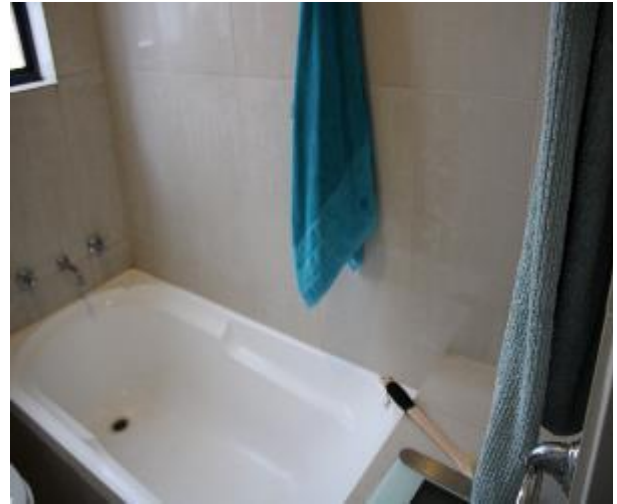
Figure 1584 - General condition of bathroom 1 internal wall
