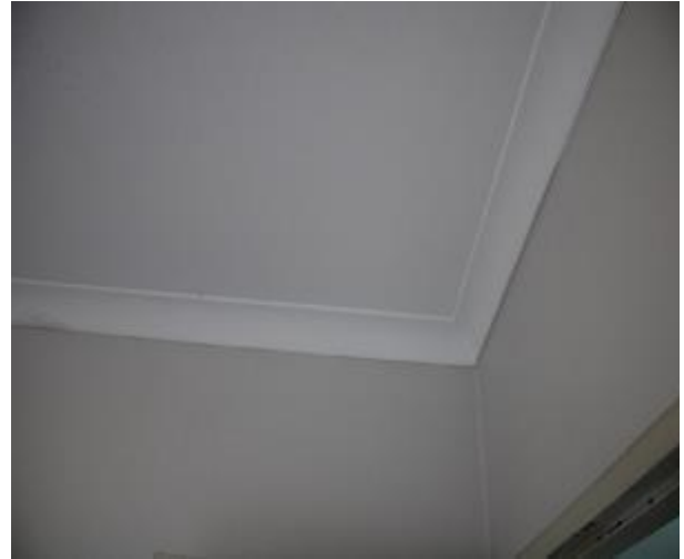
Figure 688 - General condition of bedroom 1 ceiling
