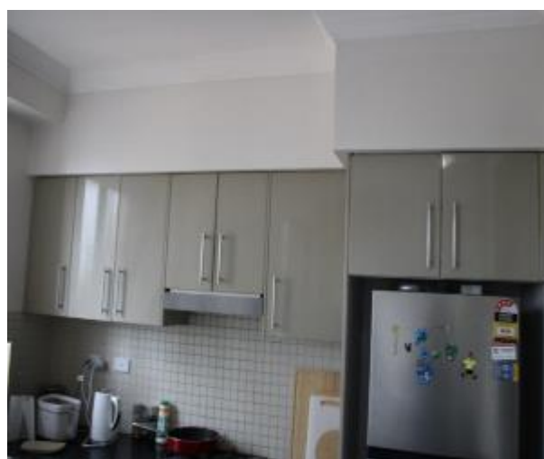
Figure 1468 - General condition of open kitchen/ lounge room internal wall
