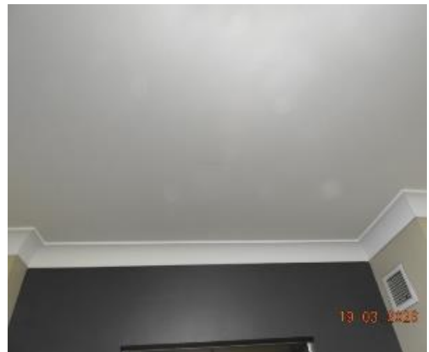
Figure 142 - General condition of level 4 common area ceiling
