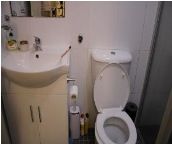
Figure 717 - General condition of ensuite bathroom internal wall
