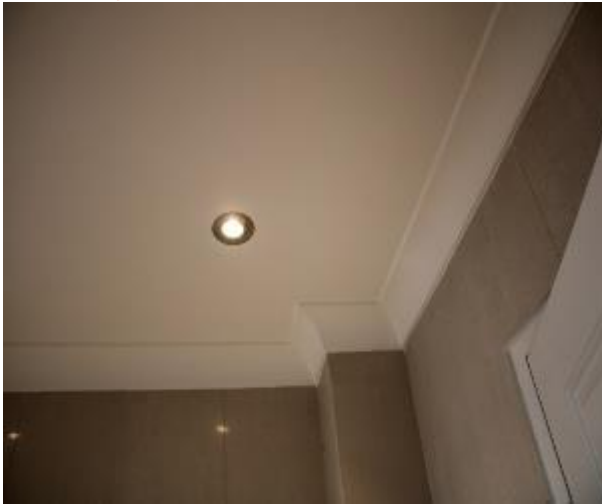
Figure 1026 - General condition of bathroom 1 ceiling
