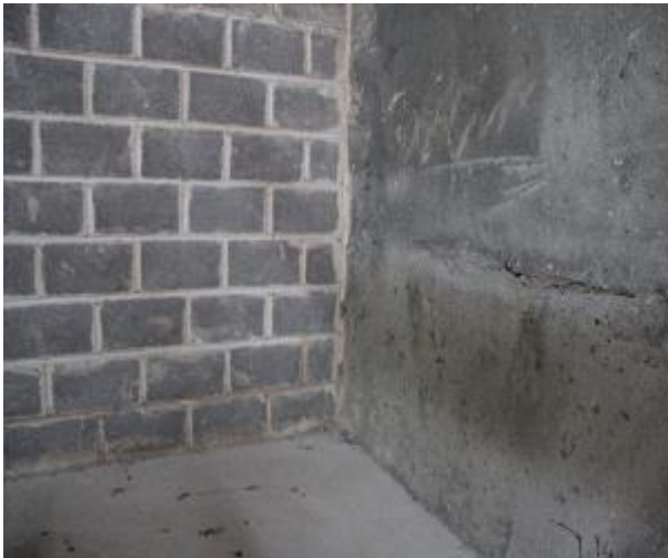
Figure 229 - General condition of B1 fire stairs internal wall
