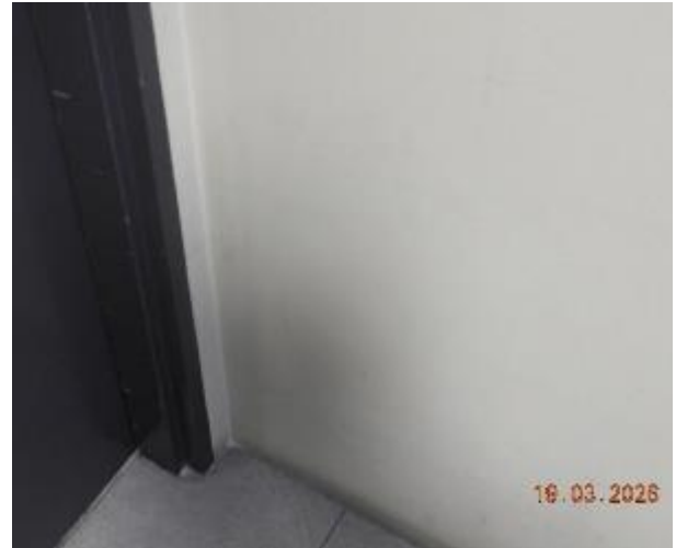
Figure 134 - General condition of level 4 common area internal wall
