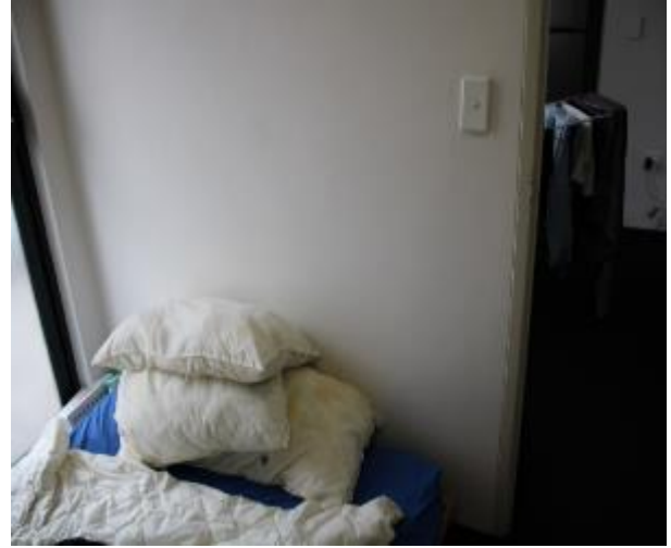
Figure 1554 - General condition of bedroom 1 internal wall
