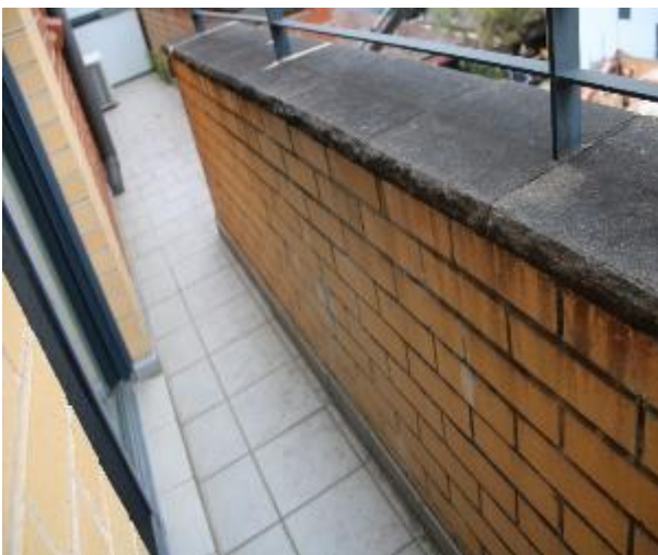
Figure 1539 - General condition of balcony balustrade
