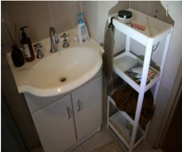
Figure 1358 - General condition of bathroom 1 internal wall
