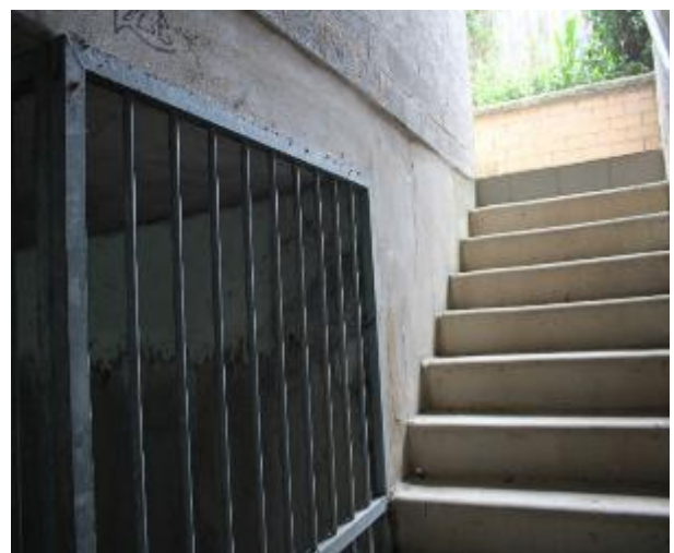
Figure 256 - General condition of level 1 fire stairs internal wall
