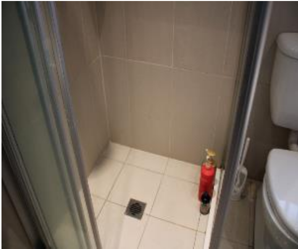
Figure 996 - General condition of bathroom 1 internal wall
