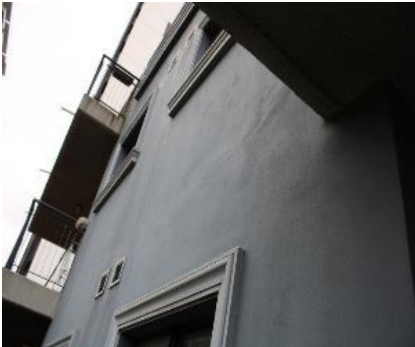
Figure 669 - General condition of external wall
