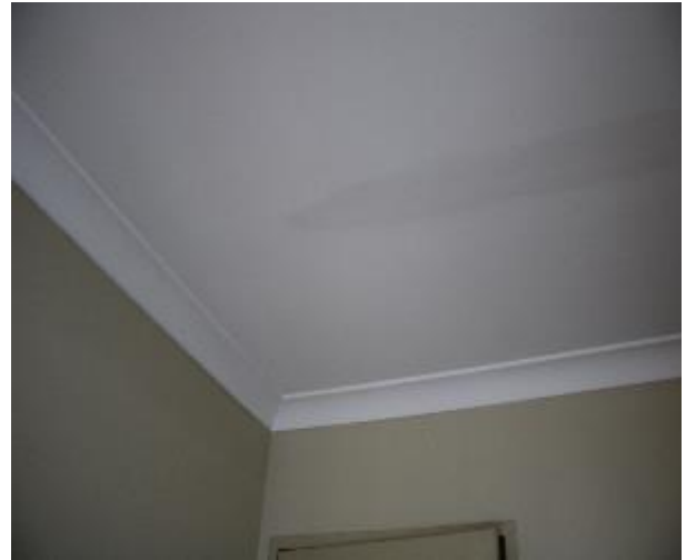
Figure 1425 - General condition of study ceiling
