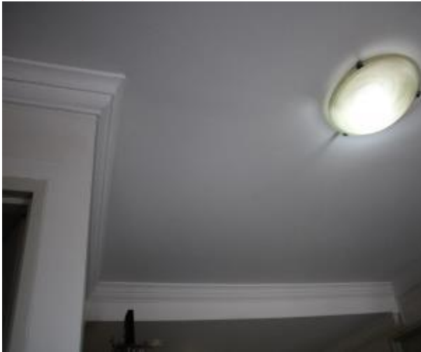
Figure 1475 - General condition of open kitchen/ lounge room ceiling
