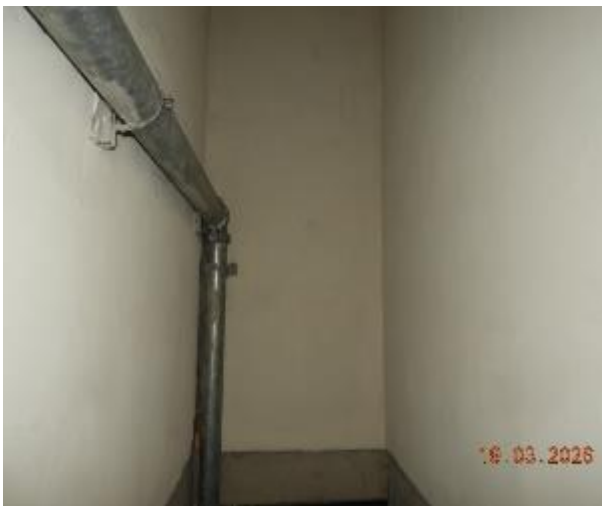
Figure 458 - General condition of basement fire stairs internal wall
