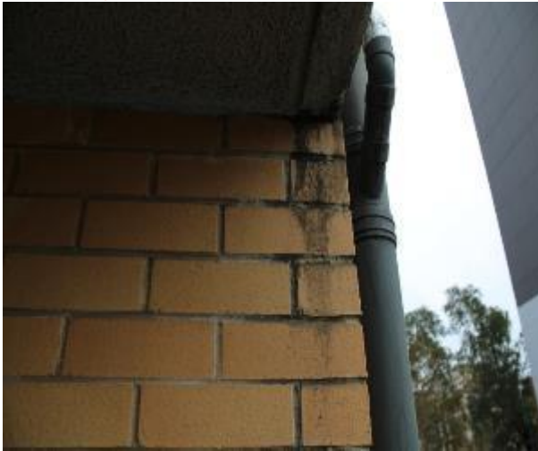
Figure 667 - General condition of balcony underside slab
