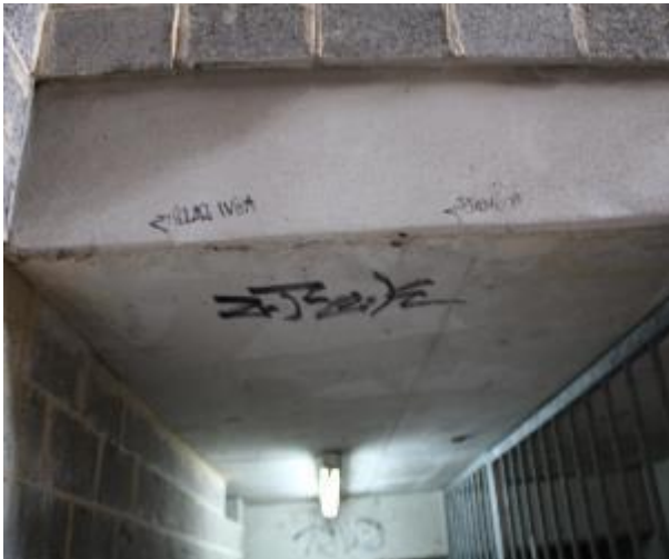
Figure 271 - General condition of fire stairs underside slab
