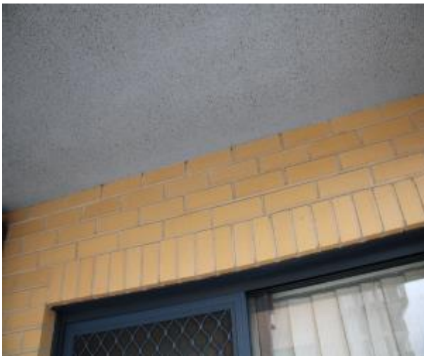
Figure 926 - General condition of external wall
