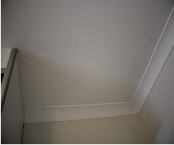
Figure 1241 - General condition of bedroom 2 ceiling
