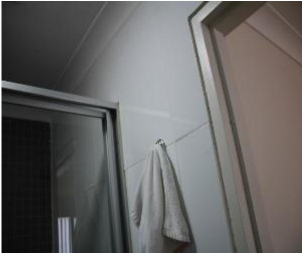
Figure 1223 - General condition of ensuite bathroom internal wall
