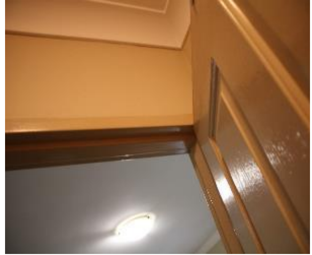
Figure 1323 - General condition of laundry internal wall
