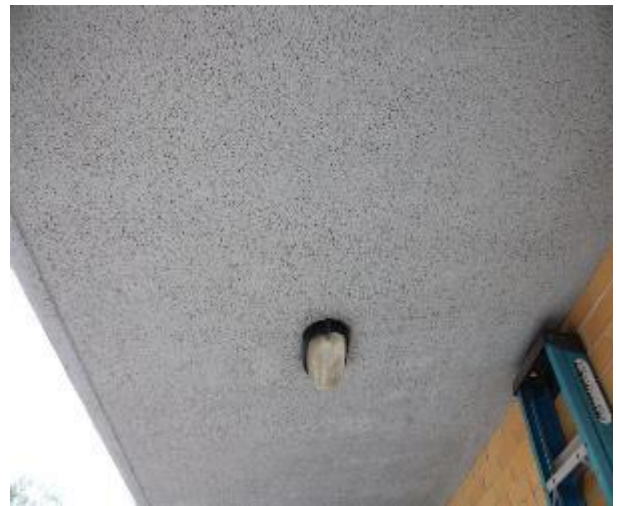
Figure 933 - General condition of balcony underside slab
