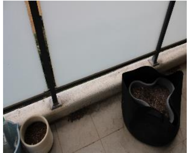
Figure 1437 - General condition of external wall
