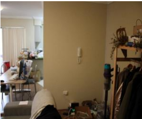
Figure 1278 - General condition of lounge room internal wall
