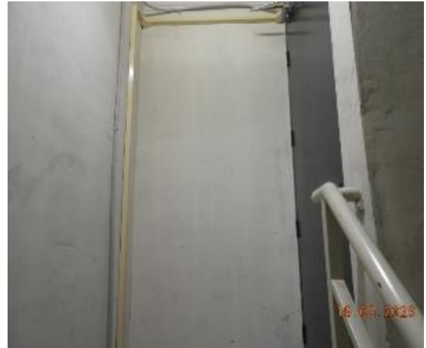
Figure 283 - General condition of level 5 fire stairs internal wall
