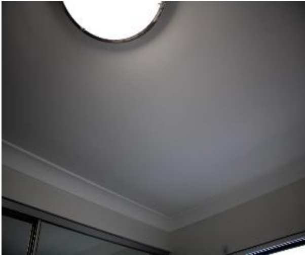
Figure 1038 - General condition of bedroom 1 ceiling
