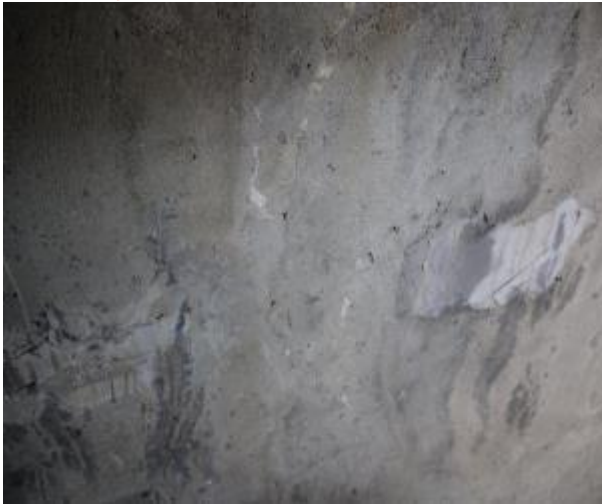
Figure 221 - General condition of B1 fire stairs internal wall
