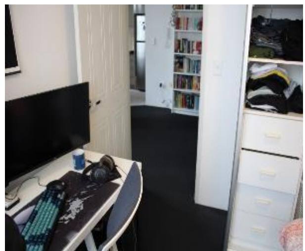
Figure 1564 - General condition of bedroom 2 internal wall
