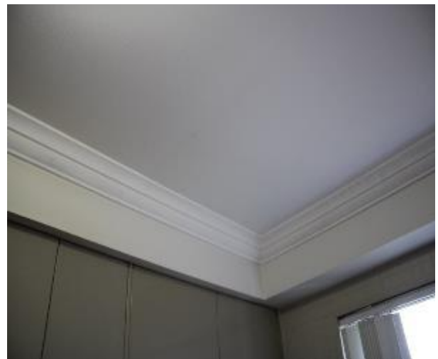
Figure 969 - General condition of kitchen ceiling
