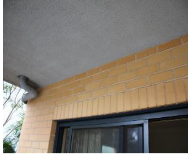
Figure 836 - General condition of external wall
