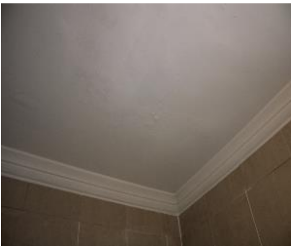
Figure 1599 - General condition of bathroom 1 ceiling
