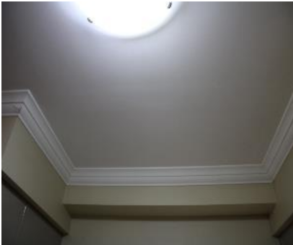
Figure 1312 - General condition of kitchen ceiling
