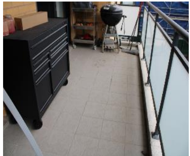
Figure 832 - General condition of balcony floor tiles
