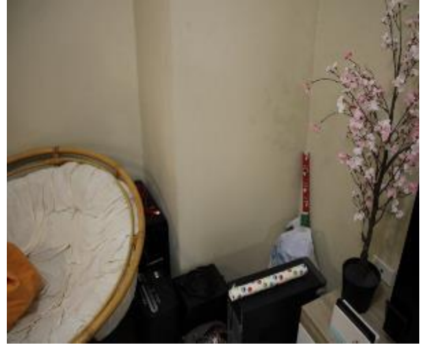
Figure 1293 - General condition of lounge room internal wall
