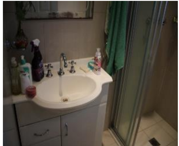
Figure 993 - General condition of bathroom 1 internal wall
