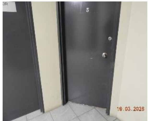
Figure 58 - General condition of level 2 common area internal wall
