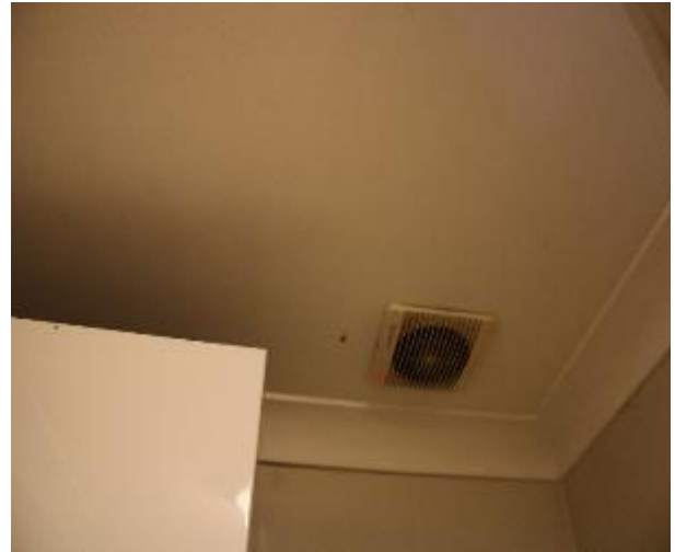
Figure 588 - General condition of laundry ceiling
