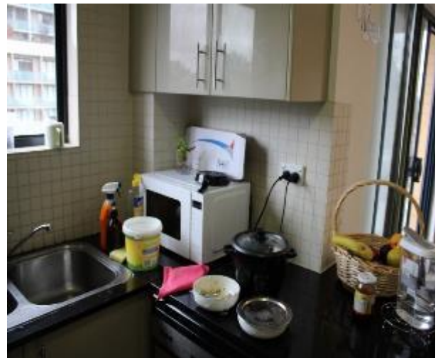
Figure 965 - General condition of kitchen internal wall
