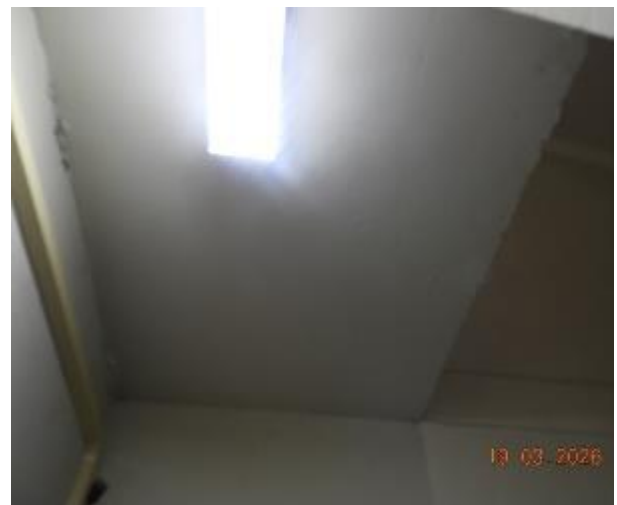
Figure 323 - General condition of level 4 fire stairs underside stairs
