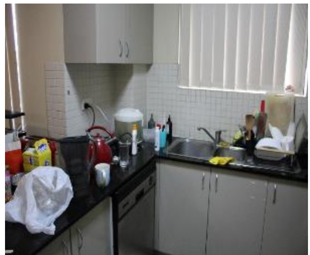
Figure 1303 - General condition of kitchen internal wall
