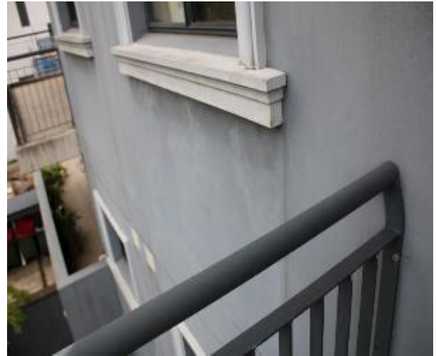
Figure 668 - General condition of external wall
