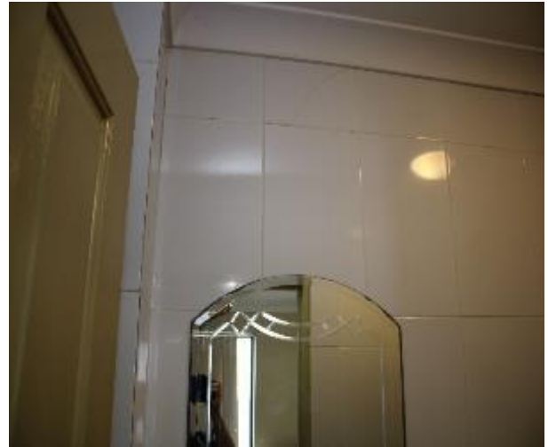
Figure 1401 - General condition of ensuite bathroom internal wall
