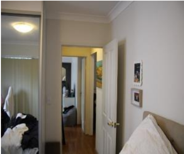
Figure 1235 - General condition of bedroom 2 internal wall
