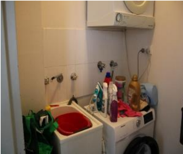
Figure 1487 - General condition of laundry internal wall
