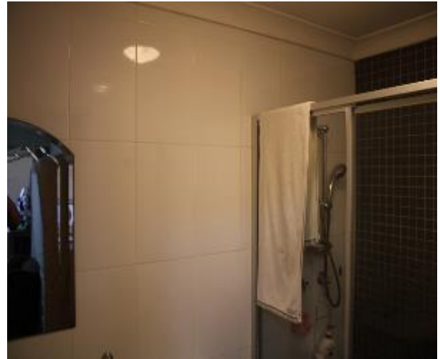
Figure 806 - General condition of ensuite bathroom internal wall
