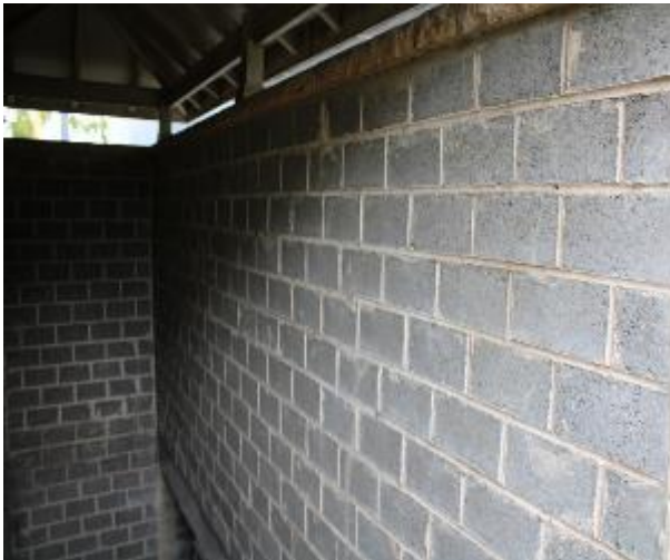
Figure 265 - General condition of level 1 fire stairs internal wall
