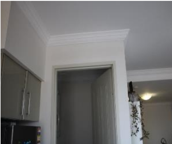
Figure 1471 - General condition of open kitchen/ lounge room internal wall
