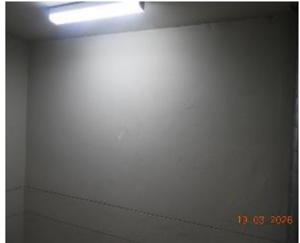
Figure 369 - General condition of level 2 fire stairs internal wall
