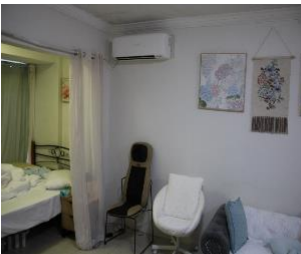
Figure 525 - General condition of open kitchen/ lounge room internal wall
