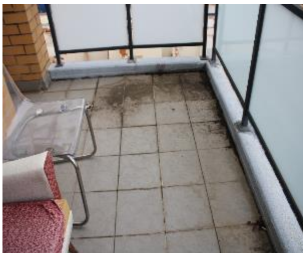
Figure 1501 - General condition of balcony floor tiles
