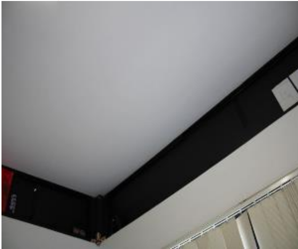
Figure 1559 - General condition of bedroom 1 ceiling
