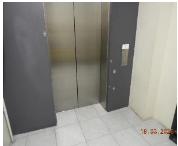
Figure 178 - General condition of level 5 common area internal wall
