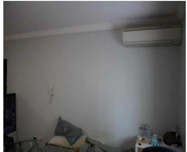
Figure 480 - General condition of open kitchen/ lounge room internal wall
