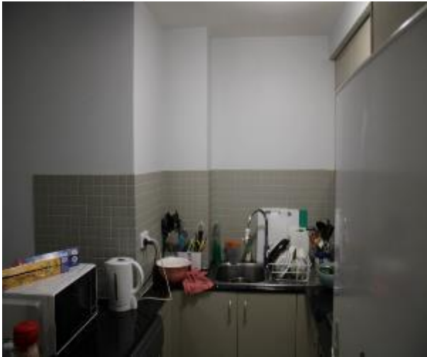
Figure 483 - General condition of open kitchen/ lounge room internal wall
