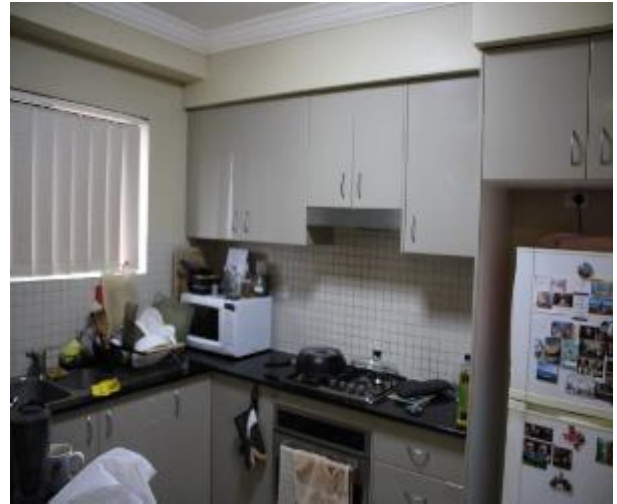
Figure 1305 - General condition of kitchen internal wall
