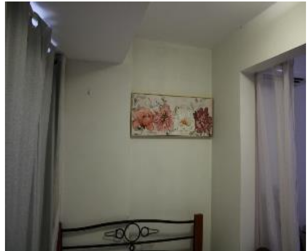
Figure 554 - General condition of bedroom 1 internal wall
