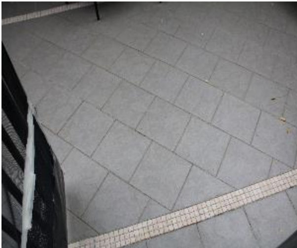
Figure 589 - General condition of courtyard floor tiles
