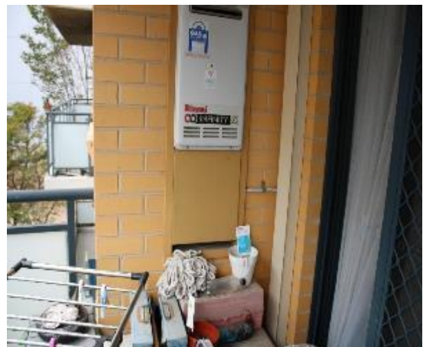
Figure 929 - General condition of external wall
