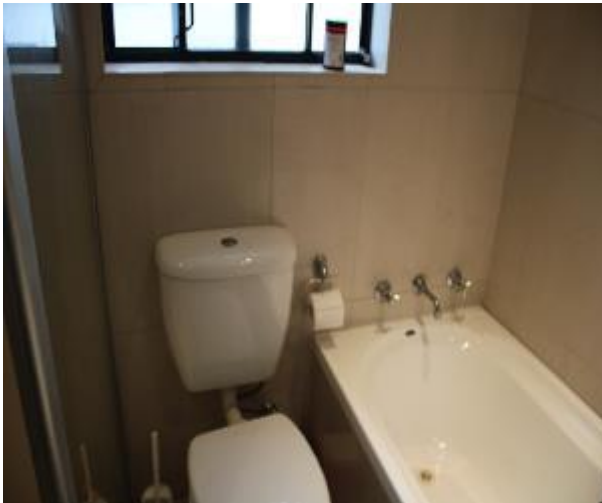
Figure 998 - General condition of bathroom 1 internal wall
