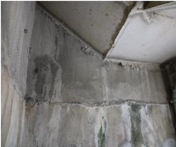
Figure 199 - General condition of B2 fire stairs internal wall
