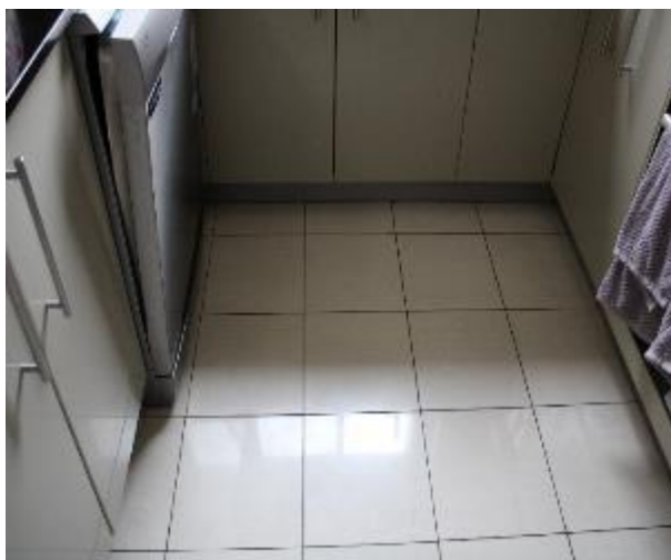
Figure 1465 - General condition of kitchen floor tiles
