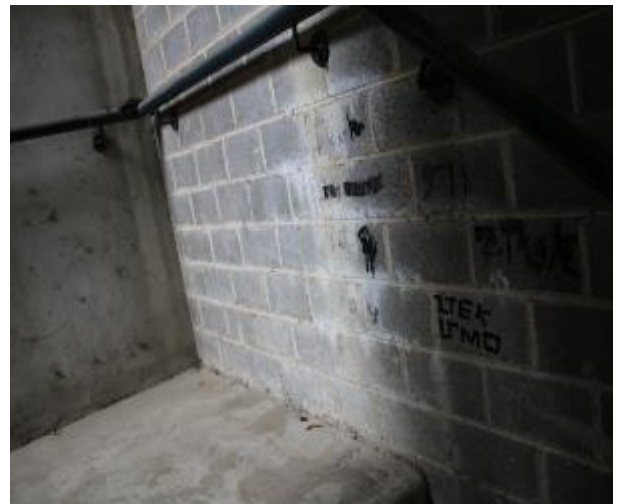
Figure 250 - General condition of level 1 fire stairs internal wall
