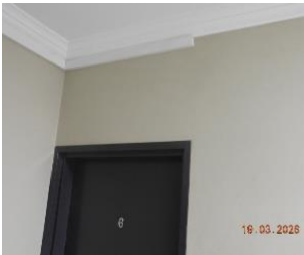
Figure 51 - General condition of level 2 common area internal wall
