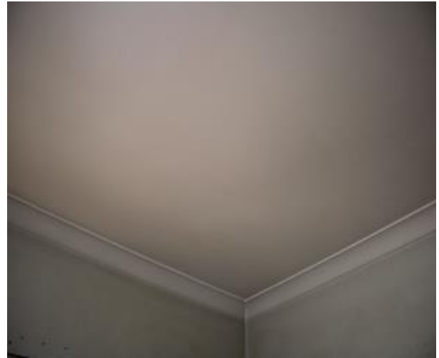
Figure 824 - General condition of study ceiling
