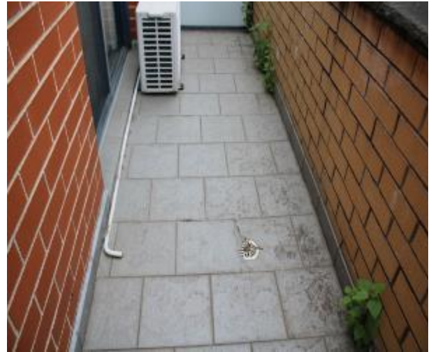
Figure 1512 - General condition of balcony floor tiles
