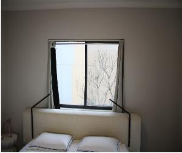
Figure 685 - General condition of bedroom 1 internal wall
