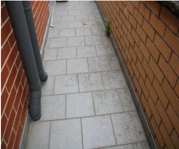
Figure 1511 - General condition of balcony floor tiles
