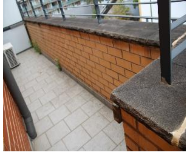
Figure 1542 - General condition of balcony balustrade
