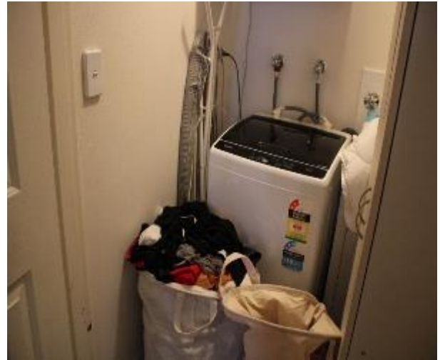
Figure 1134 - General condition of laundry internal wall
