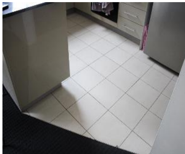
Figure 1464 - General condition of kitchen floor tiles
