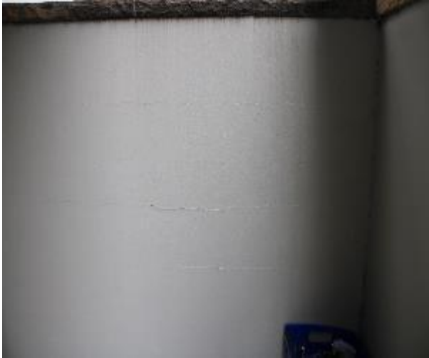
Figure 519 - Crack propagation through courtyard external wall
