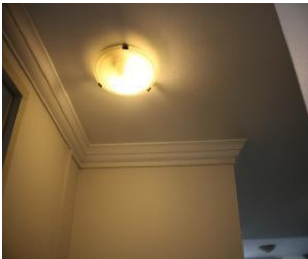
Figure 1579 - General condition of corridor ceiling
