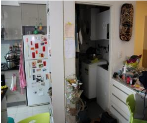
Figure 858 - General condition of bedroom 1 internal wall
