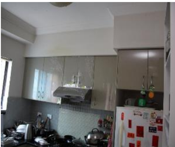
Figure 868 - General condition of kitchen internal wall
