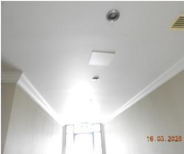
Figure 39 - General condition of level 1 common area ceiling
