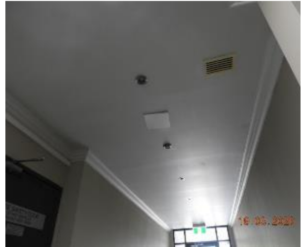
Figure 38 - General condition of level 1 common area ceiling
