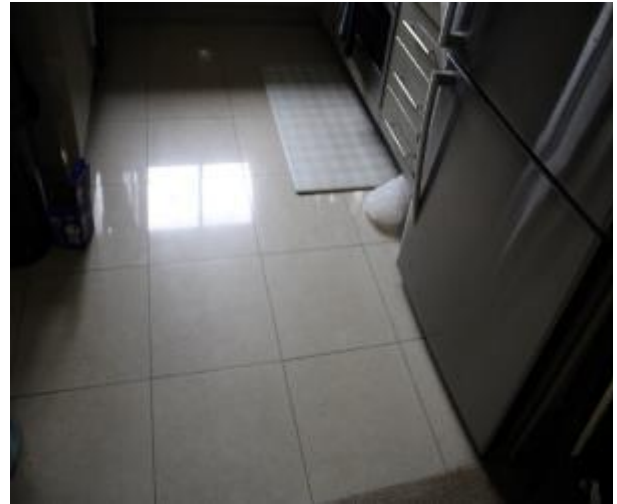
Figure 644 - General condition of kitchen floor tiles
