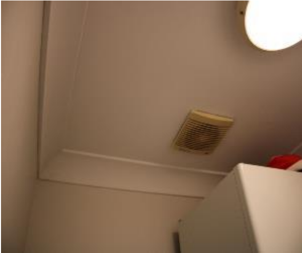
Figure 980 - General condition of laundry ceiling
