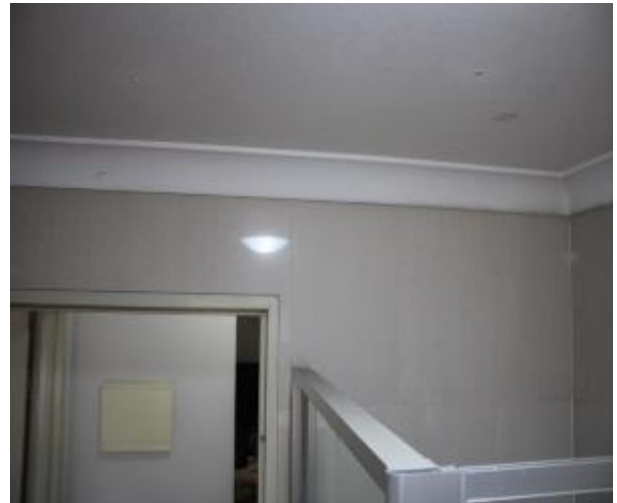
Figure 700 - General condition of bathroom 1 internal wall
