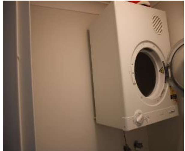
Figure 973 - General condition of laundry internal wall
