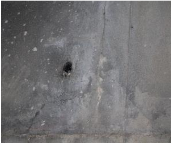
Figure 203 - General condition of B2 fire stairs internal wall
