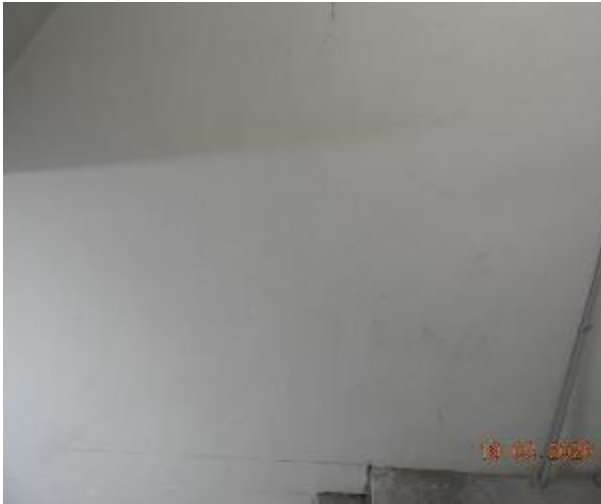
Figure 354 - General condition of level 3 fire stairs internal wall
