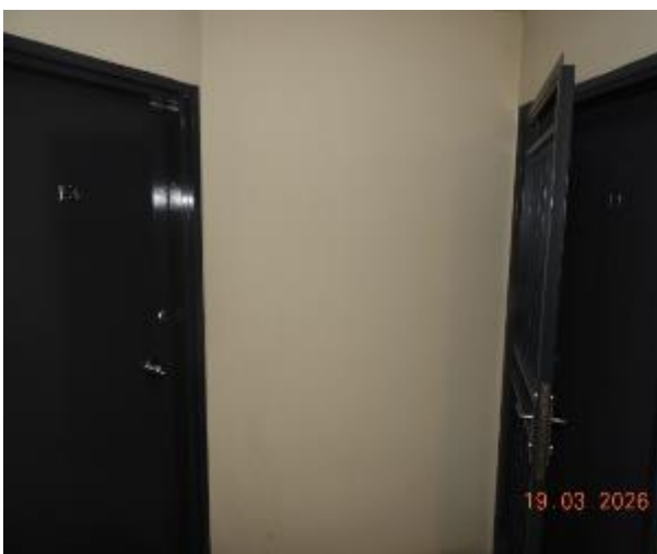
Figure 125 - General condition of level 4 common area internal wall
