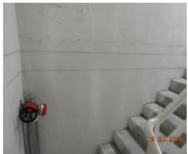
Figure 293 - General condition of level 5 fire stairs internal wall
