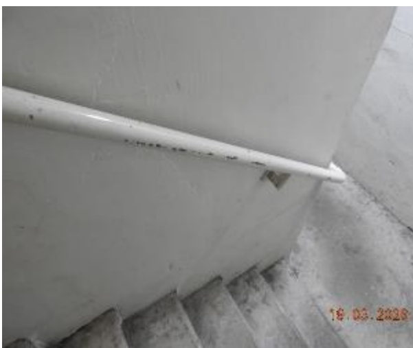
Figure 400 - General condition of level 1 fire stairs internal wall
