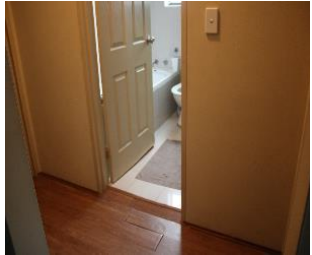
Figure 1329 - General condition of corridor internal wall
