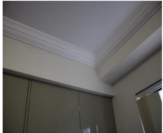
Figure 1130 - General condition of kitchen ceiling
