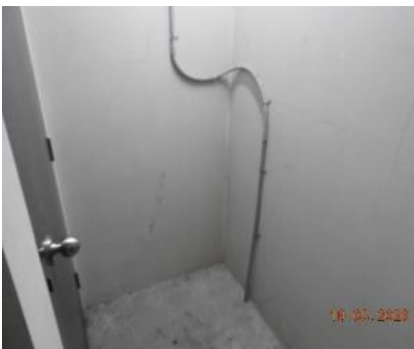
Figure 430 - General condition of level 1 fire stairs internal wall
