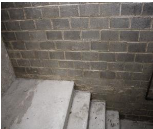
Figure 195 - General condition of B2 fire stairs internal wall
