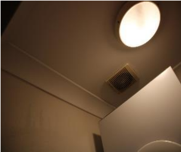
Figure 1139 - General condition of laundry ceiling
