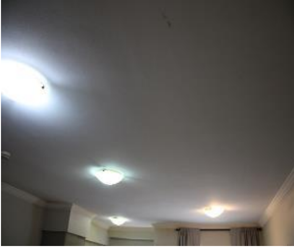
Figure 763 - General condition of open kitchen/ lounge room ceiling
