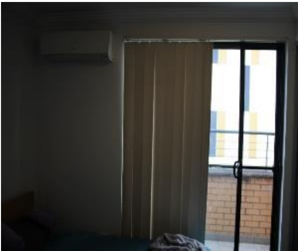
Figure 1603 - General condition of bedroom 3 internal wall
