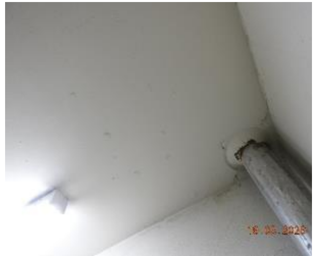
Figure 411 - General condition of level 1 fire stairs underside stairs
