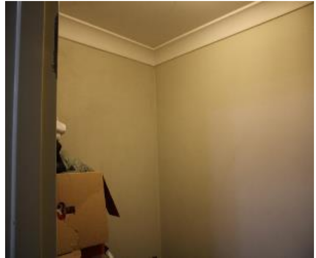
Figure 570 - General condition of laundry internal wall
