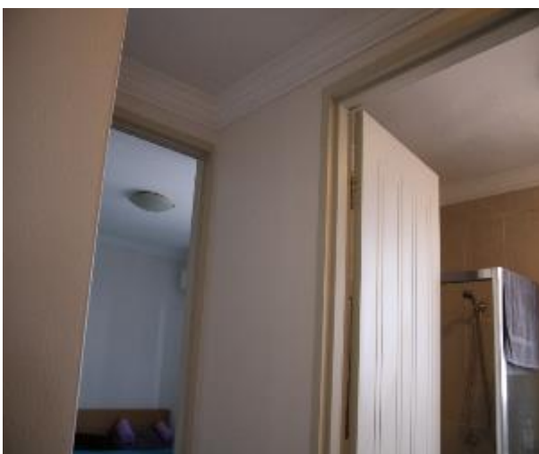
Figure 1575 - General condition of corridor internal wall
