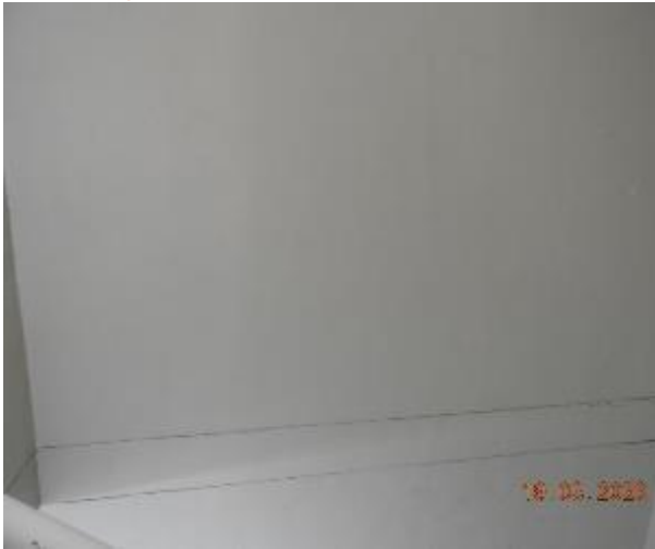
Figure 300 - General condition of level 5 fire stairs internal wall
