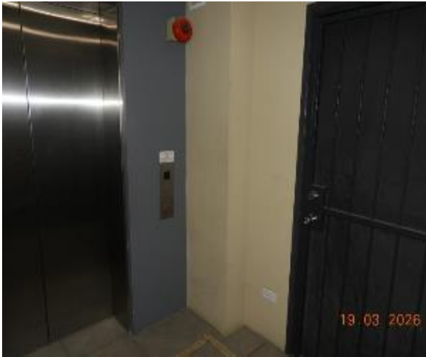
Figure 31 - General condition of level 1 common area internal wall
