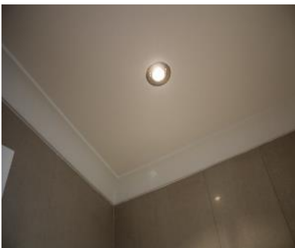
Figure 1024 - General condition of bathroom 1 ceiling
