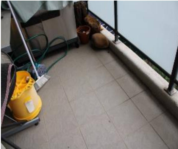
Figure 924 - General condition of balcony floor tiles
