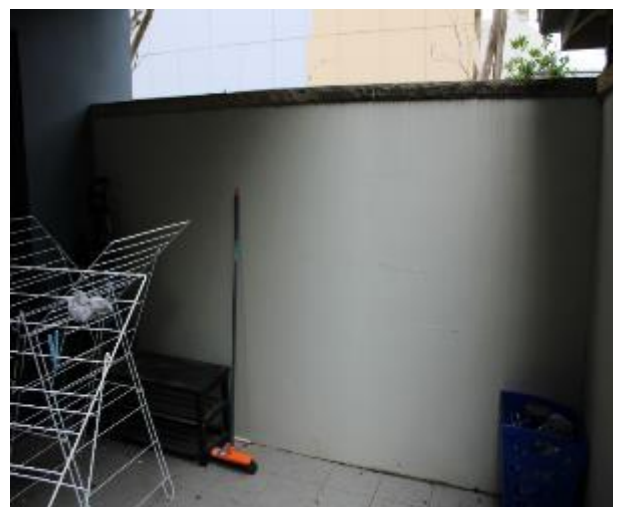
Figure 518 - General condition of courtyard external wall
