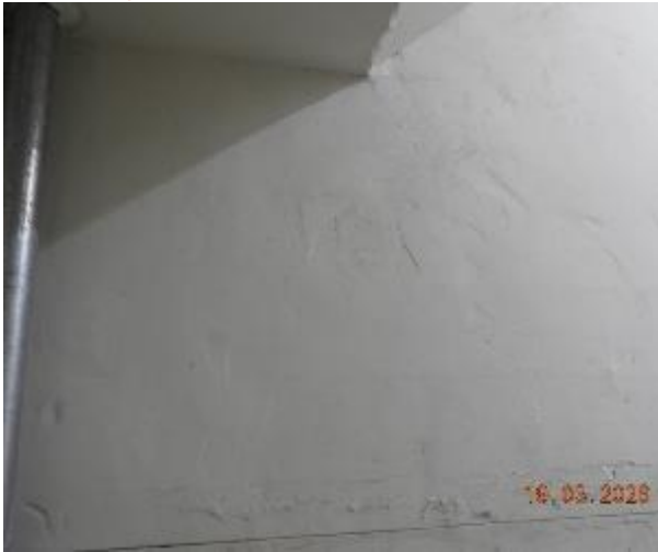
Figure 330 - General condition of level 3 fire stairs internal wall
