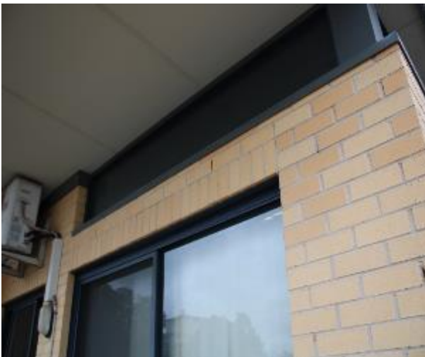
Figure 1527 - General condition of external wall
