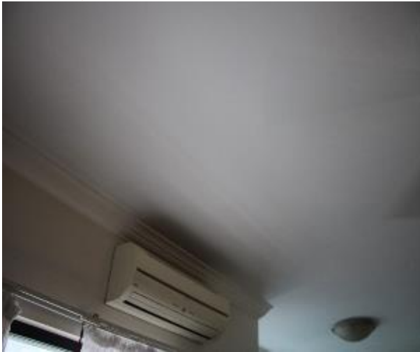
Figure 864 - General condition of bedroom 1 ceiling
