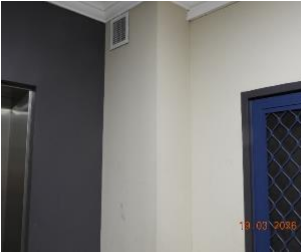
Figure 103 - General condition of level 3 common area internal wall
