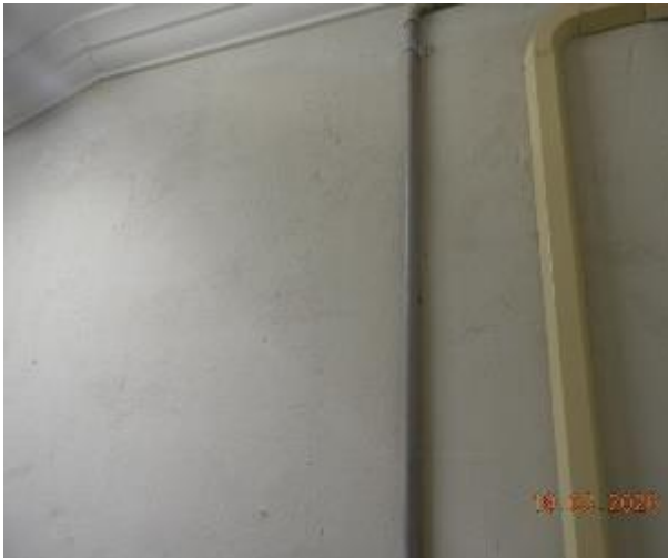
Figure 290 - General condition of level 5 fire stairs internal wall
