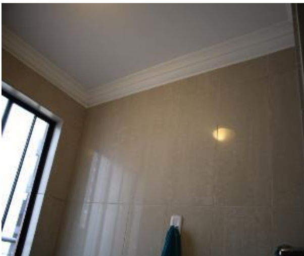
Figure 1585 - General condition of bathroom 1 internal wall
