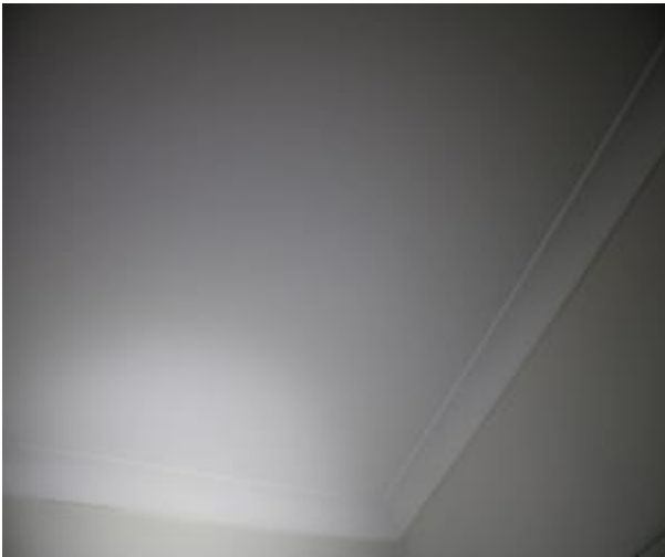
Figure 920 - General condition of bedroom 3 ceiling
