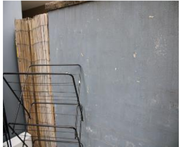
Figure 618 - General condition of courtyard external wall
