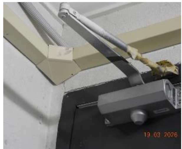
Figure 281 - Crack propagation through level 5 fire stairs internal wall
