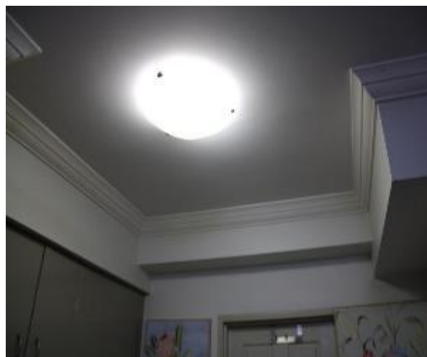
Figure 548 - General condition of open kitchen/ lounge room ceiling
