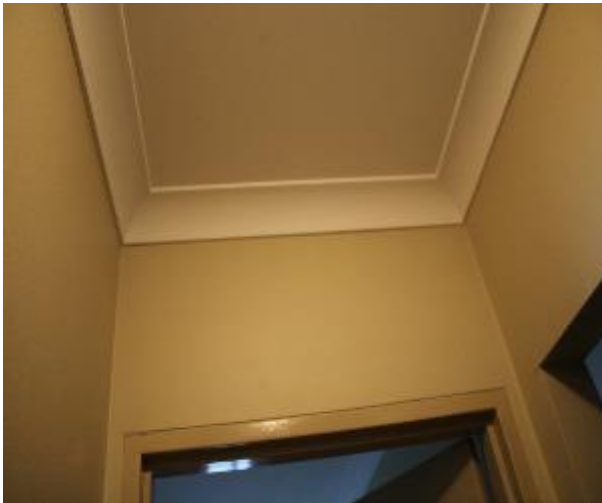
Figure 1336 - General condition of corridor internal wall
