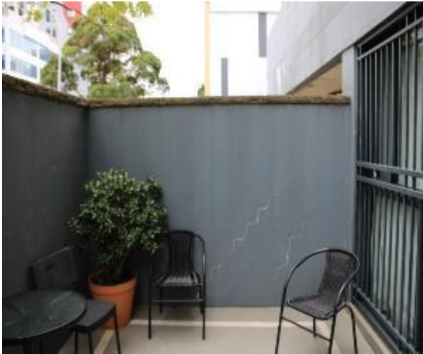
Figure 605 - General condition of courtyard external wall
