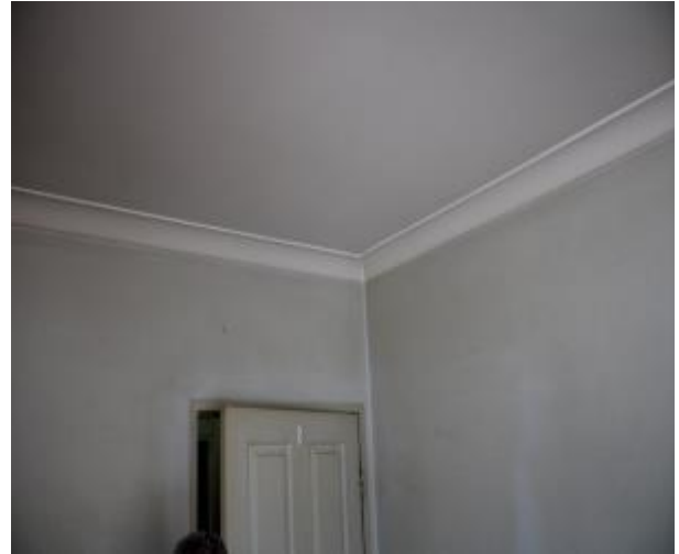
Figure 820 - General condition of study internal wall
