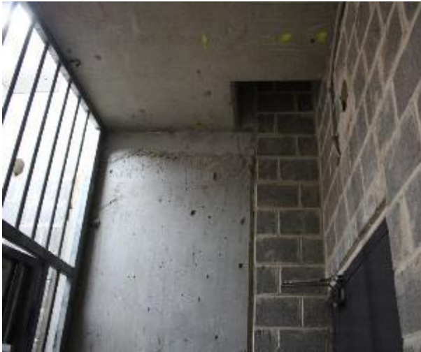
Figure 233 - General condition of B1 fire stairs internal wall
