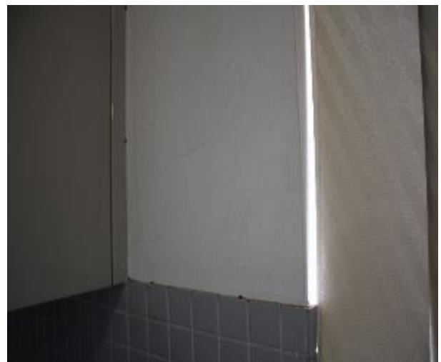
Figure 756 - General condition of open kitchen/ lounge room internal wall
