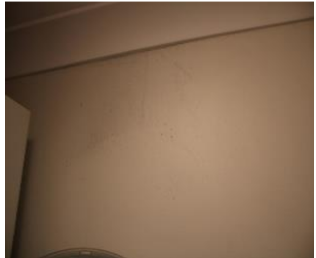
Figure 975 - Crack propagation through laundry internal wall
