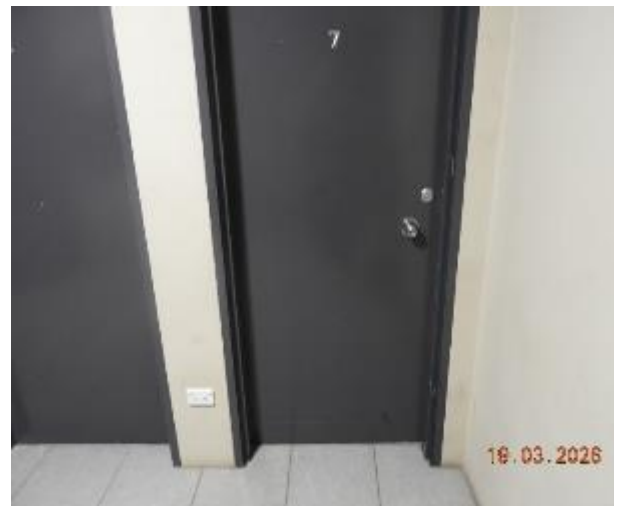
Figure 64 - General condition of level 2 common area internal wall
