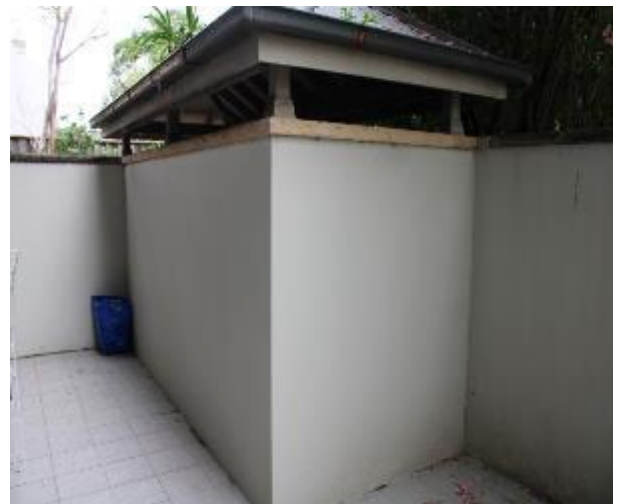
Figure 516 - General condition of courtyard external wall
