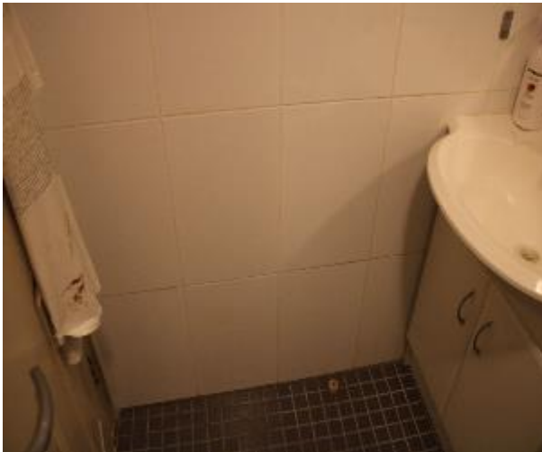
Figure 807 - General condition of ensuite bathroom internal wall
