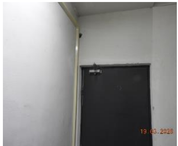
Figure 317 - General condition of level 4 fire stairs internal wall
