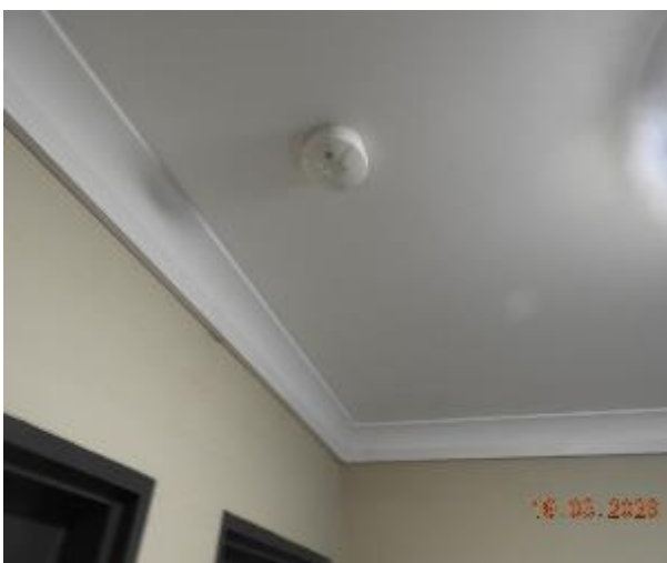
Figure 143 - General condition of level 4 common area ceiling
