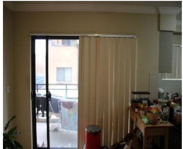
Figure 1283 - General condition of lounge room internal wall
