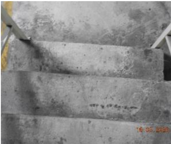
Figure 470 - General condition of basement fire stairs
