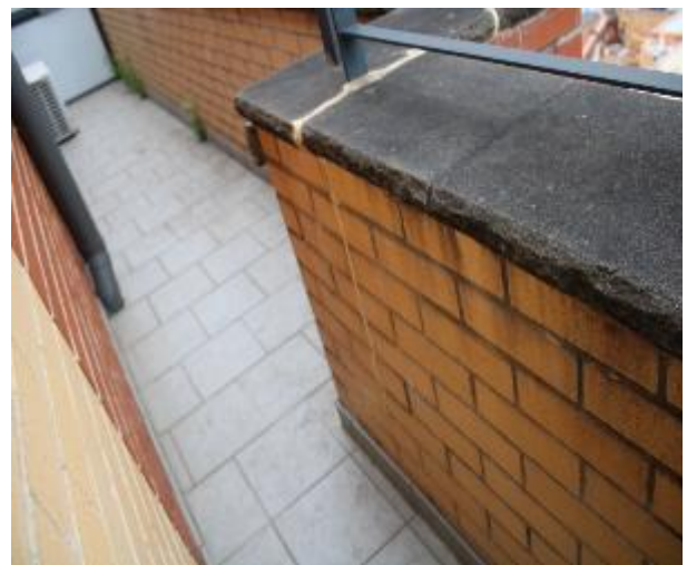
Figure 1540 - General condition of balcony balustrade
