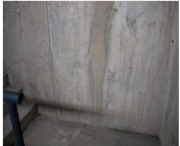
Figure 200 - General condition of B2 fire stairs internal wall
