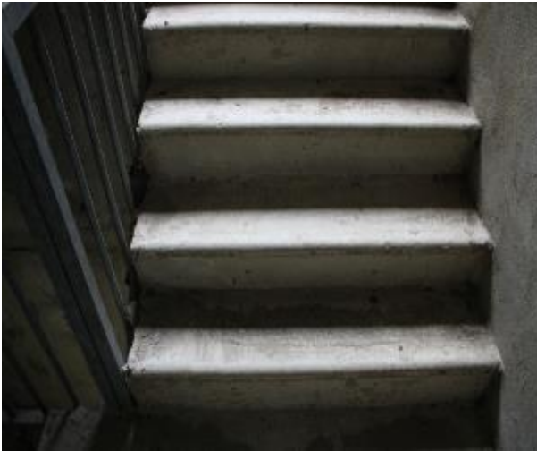
Figure 245 - General condition of level 1 fire stairs
