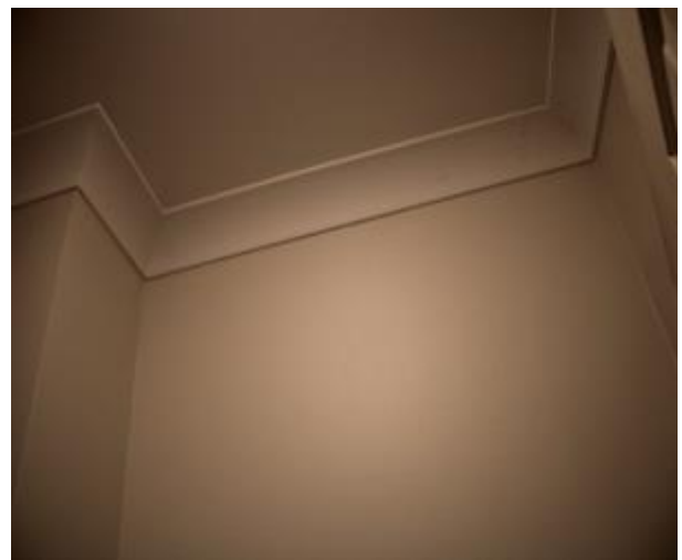
Figure 977 - General condition of laundry internal wall
