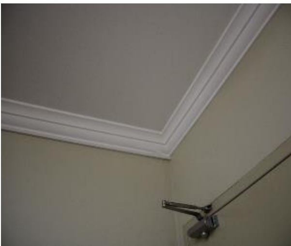
Figure 1296 - General condition of lounge room ceiling
