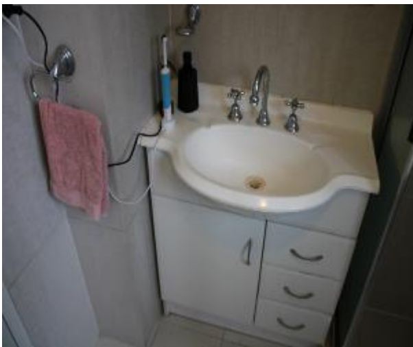
Figure 1591 - General condition of bathroom 1 internal wall
