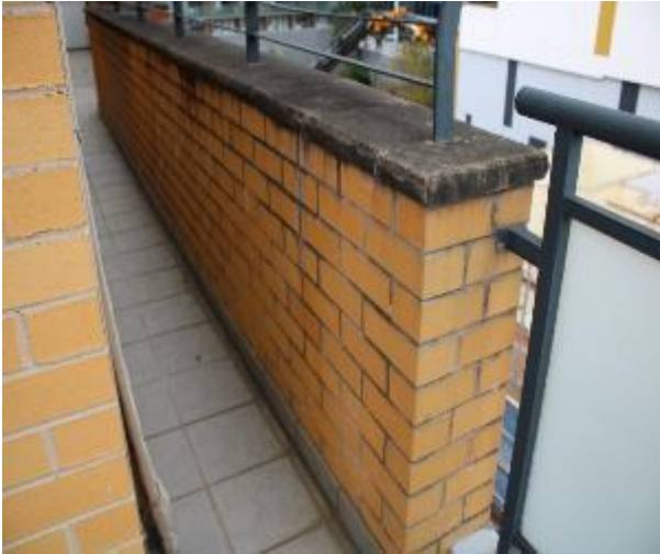
Figure 1537 - General condition of balcony balustrade
