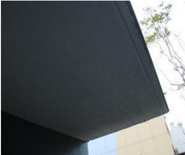
Figure 513 - General condition of balcony underside slab
