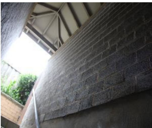
Figure 255 - General condition of level 1 fire stairs internal wall
