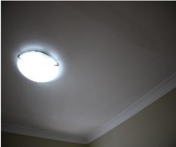
Figure 1430 - General condition of study ceiling
