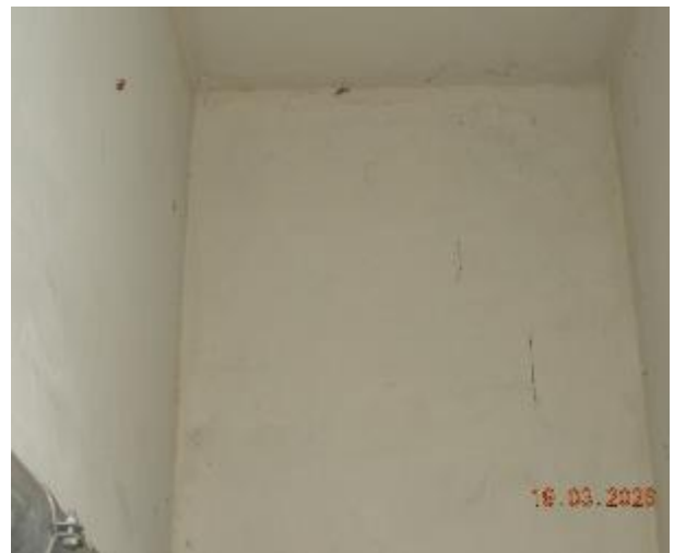
Figure 459 - General condition of basement fire stairs internal wall
