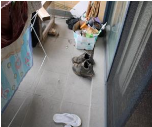
Figure 1432 - General condition of balcony floor tiles
