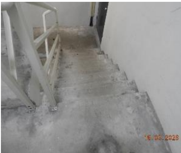
Figure 380 - General condition of level 2 fire stairs
