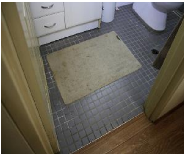
Figure 1396 - General condition of ensuite bathroom floor tiles
