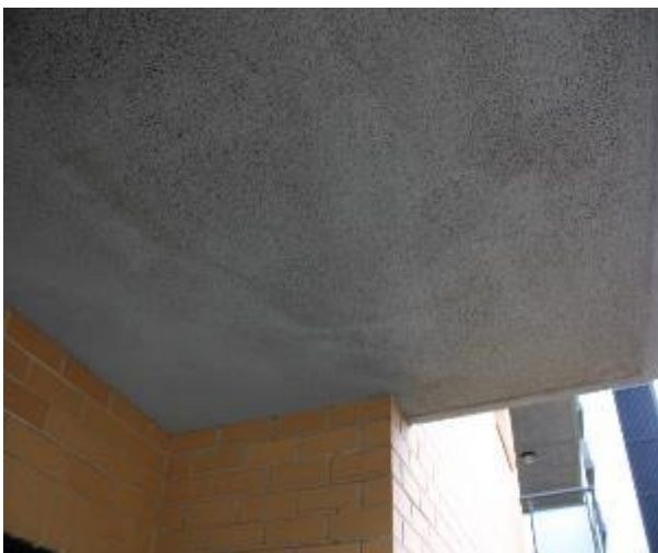
Figure 845 - General condition of balcony underside slab
