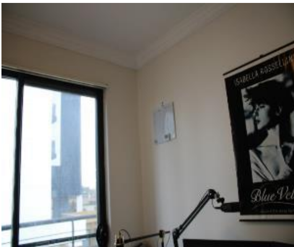
Figure 1567 - General condition of bedroom 2 internal wall
