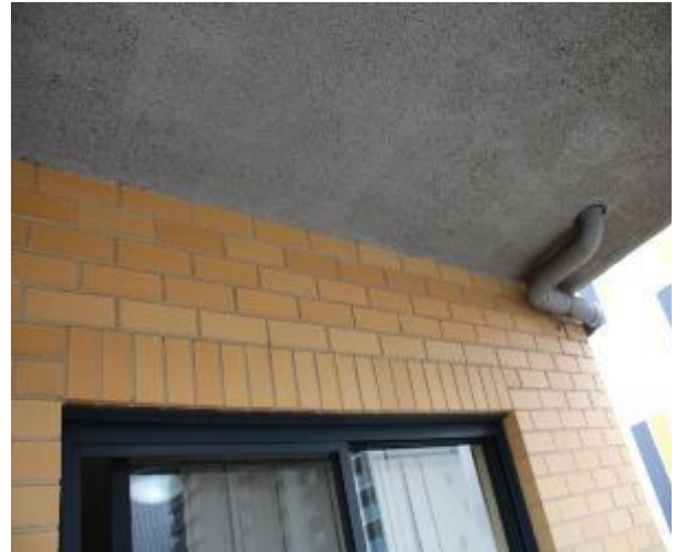
Figure 1443 - General condition of external wall
