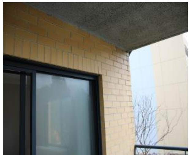
Figure 654 - General condition of external wall
