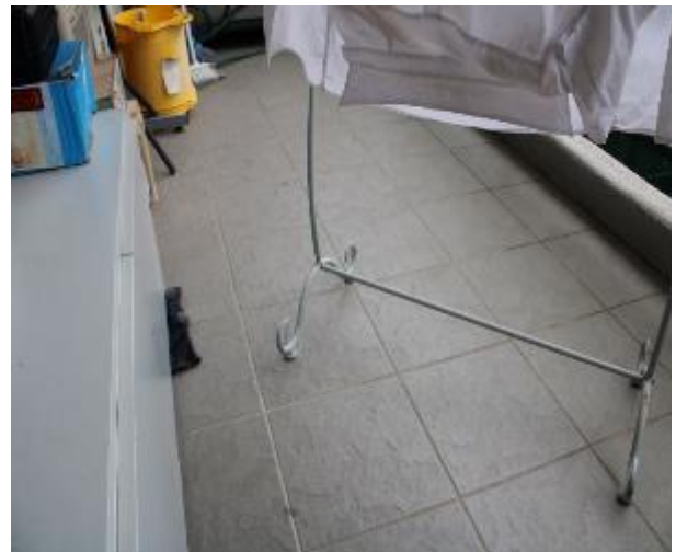
Figure 923 - General condition of balcony floor tiles
