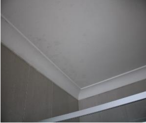
Figure 787 - General condition of bathroom 1 ceiling
