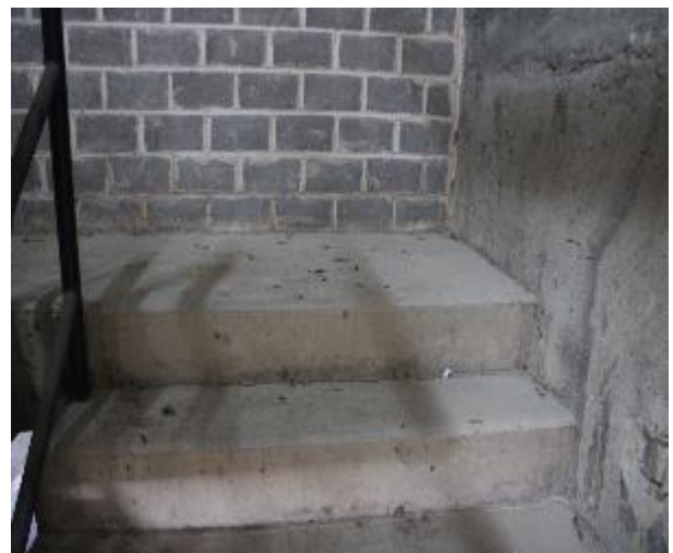
Figure 214 - General condition of B1 fire stairs
