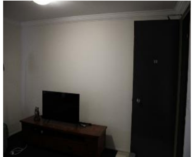
Figure 1452 - General condition of open kitchen/ lounge room internal wall
