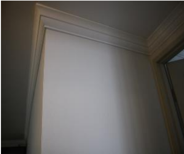
Figure 1577 - General condition of corridor internal wall
