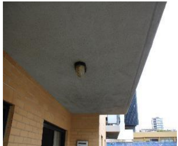
Figure 844 - General condition of balcony underside slab
