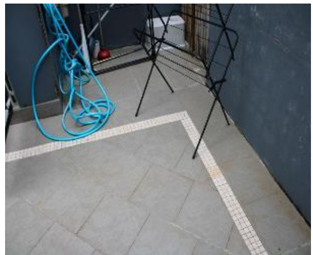
Figure 592 - General condition of courtyard floor tiles
