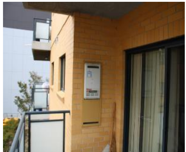
Figure 1439 - General condition of external wall
