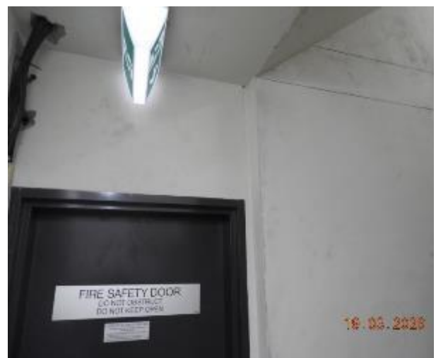
Figure 425 - General condition of level 1 fire stairs internal wall
