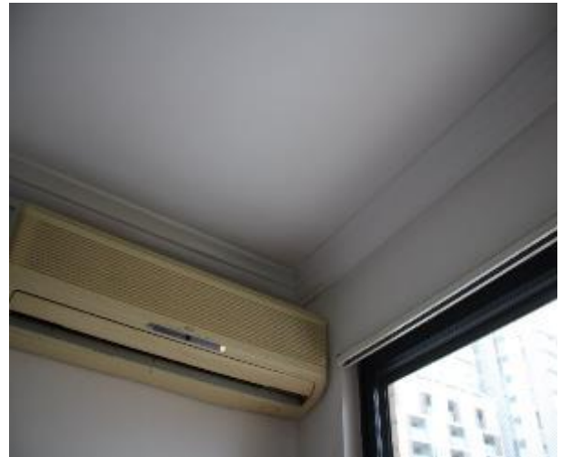
Figure 1478 - General condition of open kitchen/ lounge room ceiling
