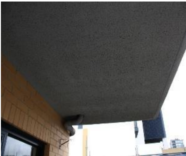
Figure 932 - General condition of balcony underside slab
