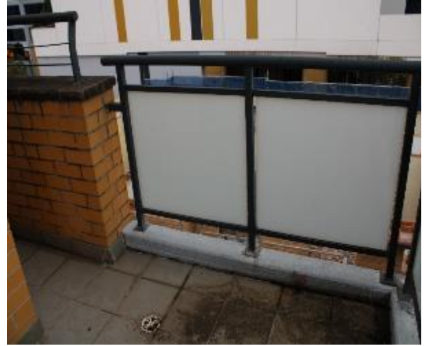
Figure 1536 - General condition of balcony balustrade
