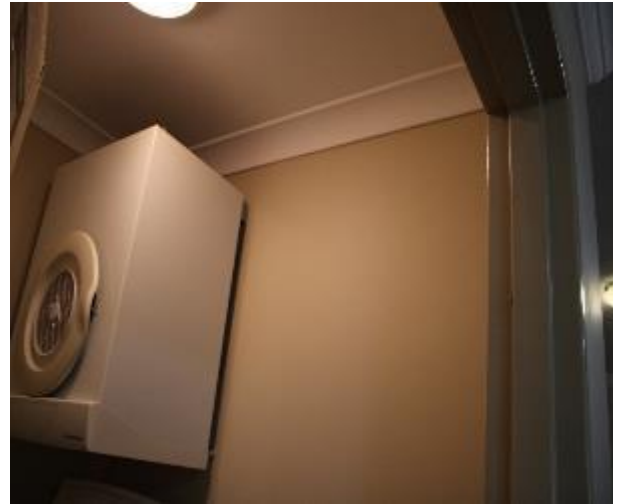
Figure 1317 - General condition of laundry internal wall
