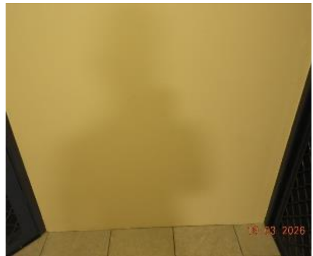
Figure 88 - General condition of level 3 common area internal wall
