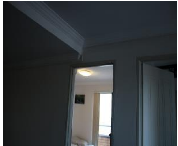
Figure 1458 - General condition of open kitchen/ lounge room internal wall
