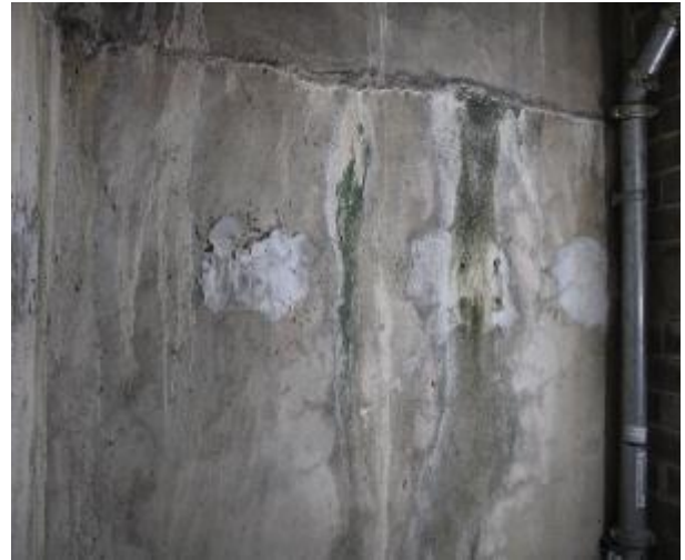
Figure 198 - General condition of B2 fire stairs internal wall
