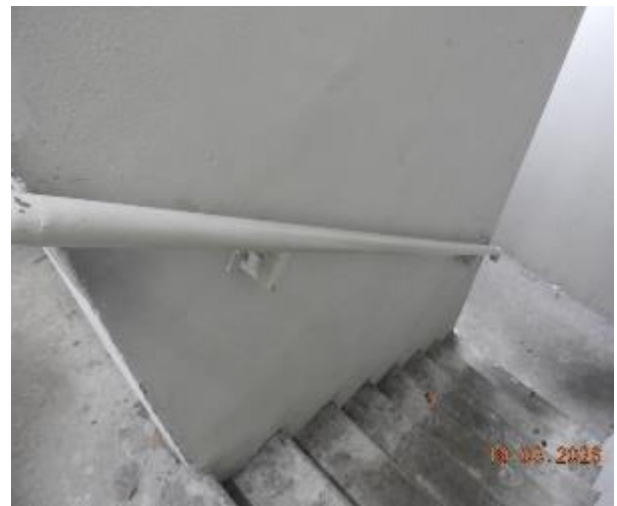
Figure 417 - General condition of level 1 fire stairs internal wall
