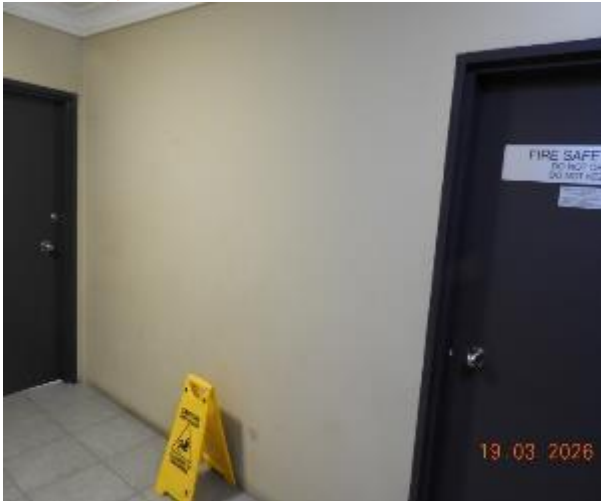
Figure 133 - General condition of level 4 common area internal wall
