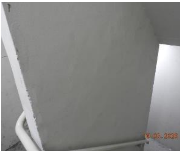
Figure 416 - General condition of level 1 fire stairs internal wall
