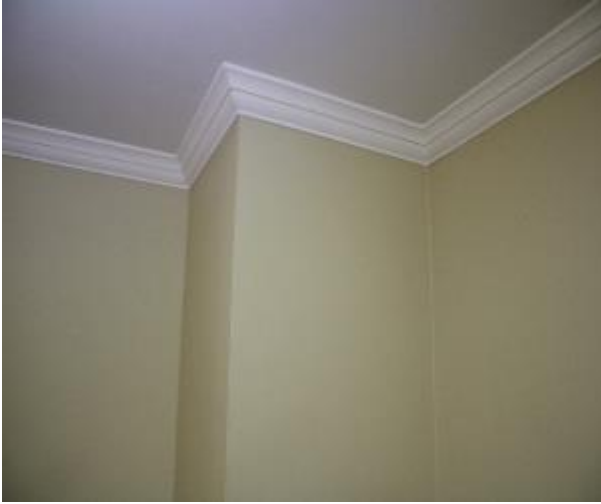
Figure 1292 - General condition of lounge room internal wall
