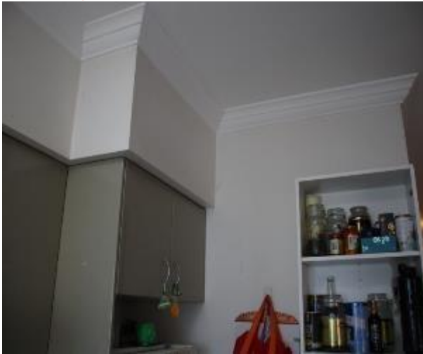
Figure 870 - General condition of kitchen internal wall
