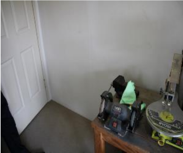
Figure 819 - General condition of study internal wall
