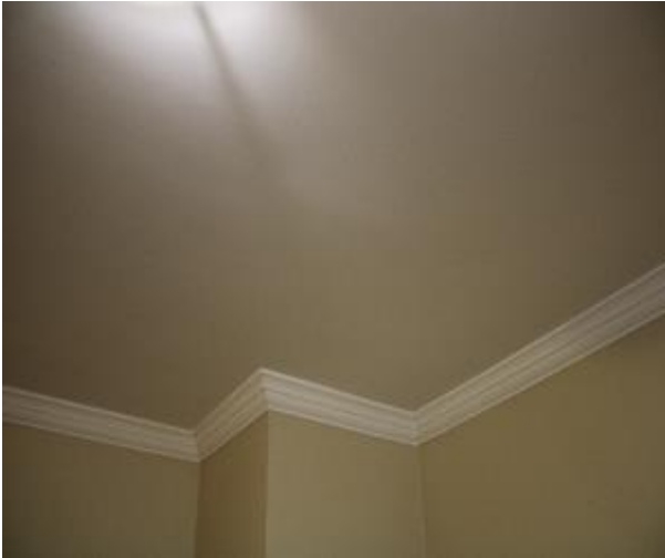
Figure 1294 - General condition of lounge room ceiling
