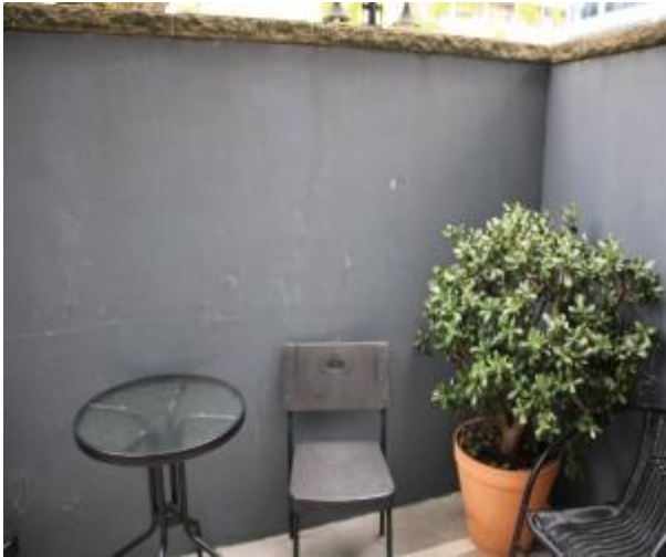
Figure 611 - General condition of courtyard external wall
