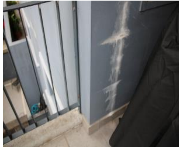
Figure 662 - General condition of external wall
