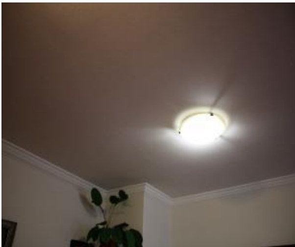
Figure 862 - General condition of bedroom 1 ceiling
