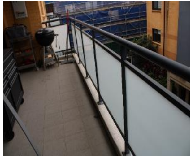
Figure 842 - General condition of balcony balustrade
