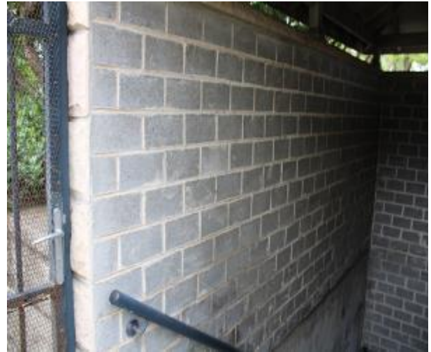
Figure 264 - General condition of level 1 fire stairs internal wall
