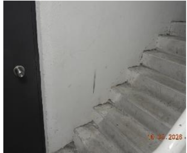
Figure 349 - General condition of level 3 fire stairs internal wall
