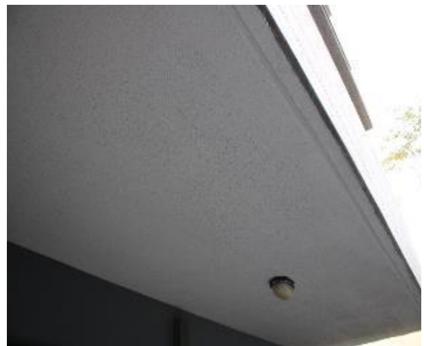
Figure 512 - General condition of balcony underside slab
