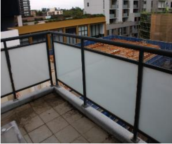
Figure 1535 - General condition of balcony balustrade
