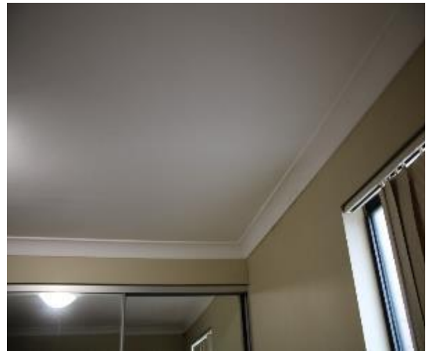
Figure 1391 - General condition of bedroom 1 ceiling
