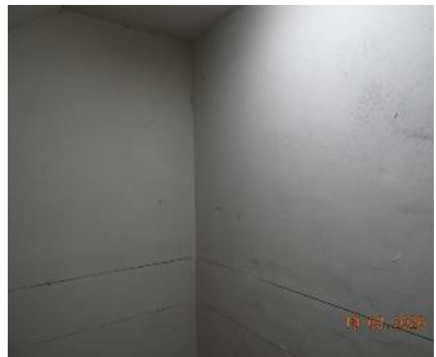
Figure 407 - General condition of level 1 fire stairs internal wall
