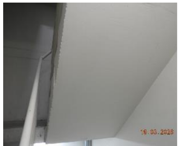
Figure 359 - General condition of level 3 fire stairs underside stairs
