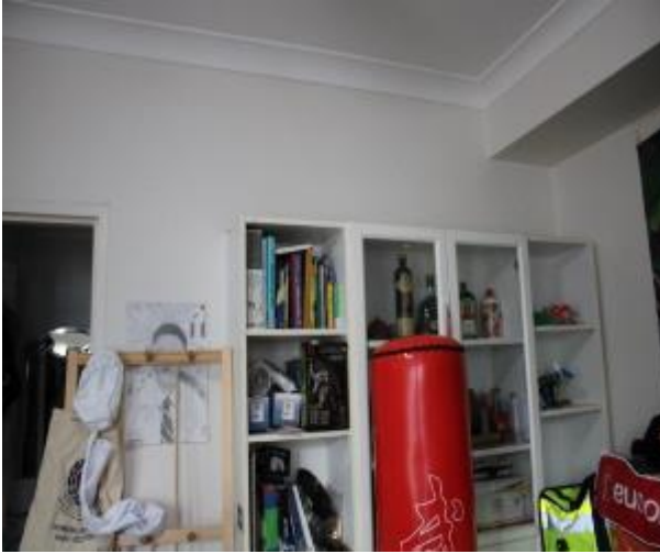
Figure 894 - General condition of bedroom 2 internal wall
