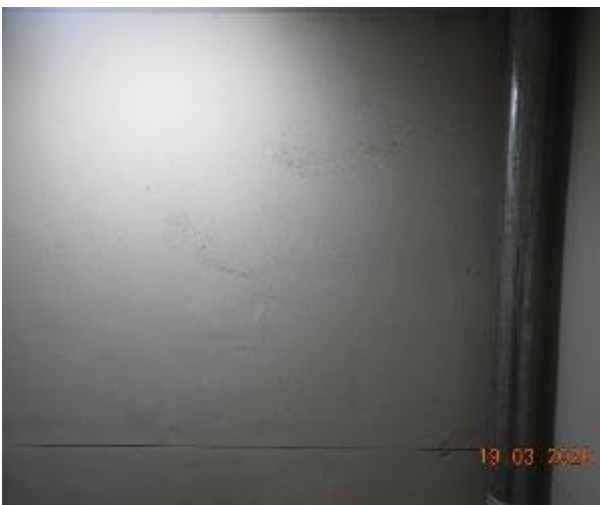
Figure 406 - General condition of level 1 fire stairs internal wall
