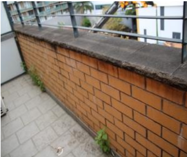
Figure 1543 - General condition of balcony balustrade
