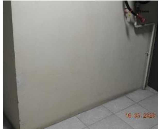
Figure 152 - General condition of level 5 common area internal wall
