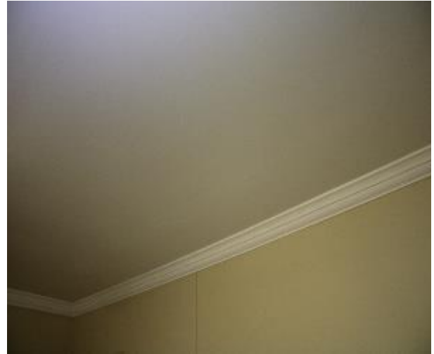
Figure 1295 - General condition of lounge room ceiling
