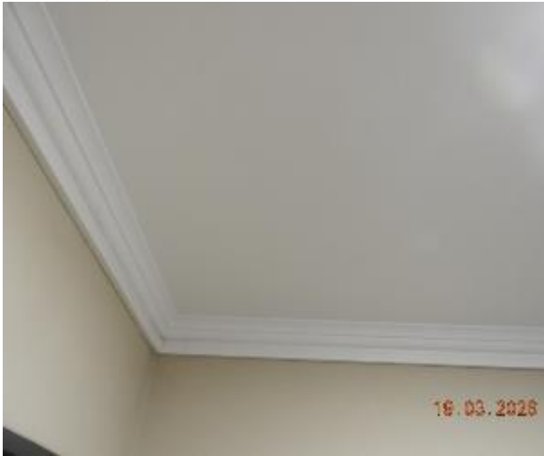
Figure 73 - General condition of level 2 common area ceiling
