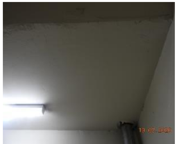
Figure 377 - General condition of level 2 fire stairs underside stairs
