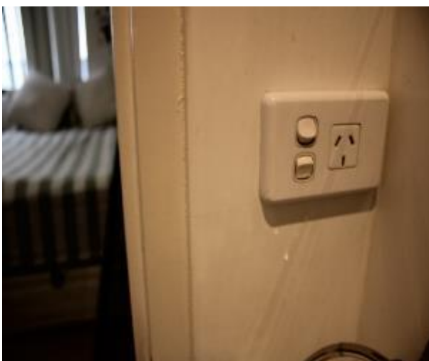
Figure 1054 - Crack propagation through ensuite bathroom internal wall
