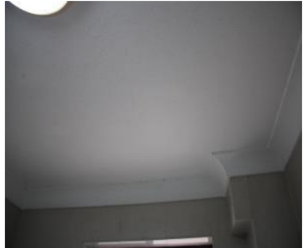
Figure 704 - General condition of bathroom 1 ceiling
