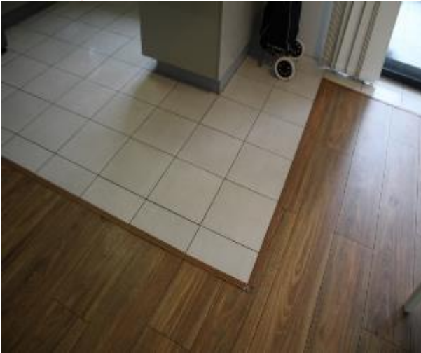
Figure 960 - General condition of kitchen floor tiles
