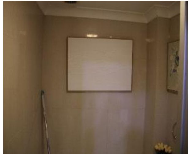
Figure 560 - General condition of bathroom 1 internal wall
