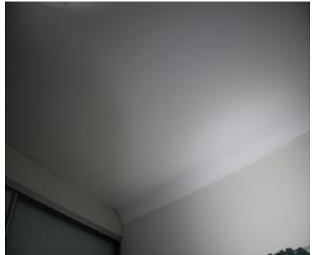
Figure 921 - General condition of bedroom 3 ceiling
