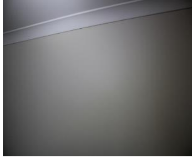
Figure 1200 - General condition of bedroom 1 internal wall
