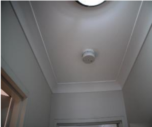
Figure 990 - General condition of corridor ceiling
