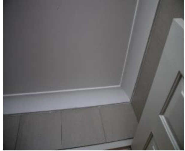
Figure 1182 - General condition of bathroom 1 ceiling
