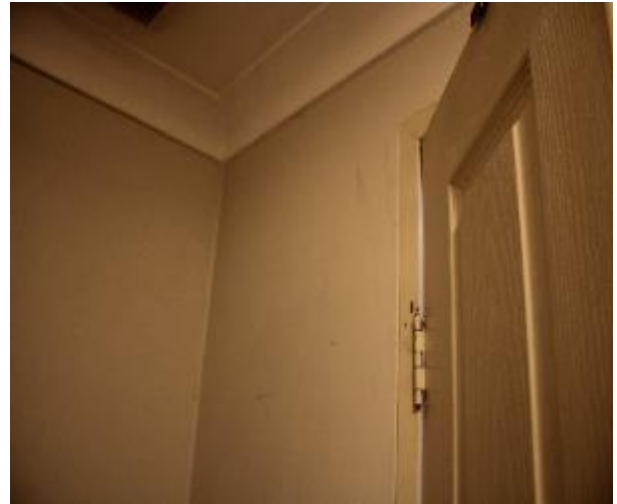
Figure 582 - General condition of laundry internal wall
