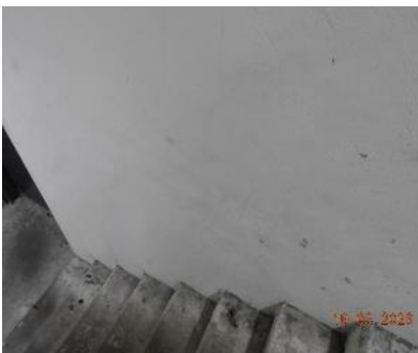
Figure 418 - General condition of level 1 fire stairs internal wall
