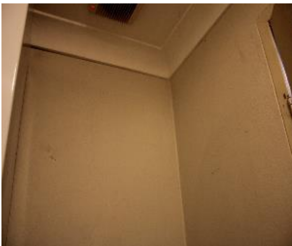
Figure 579 - General condition of laundry internal wall
