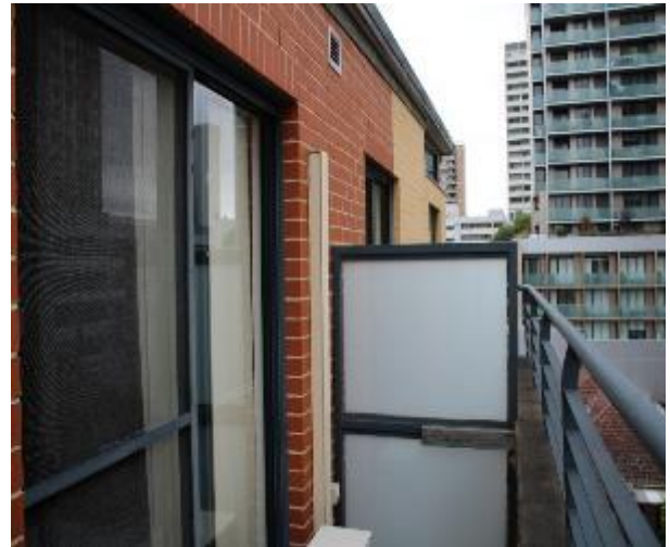
Figure 1514 - General condition of external wall
