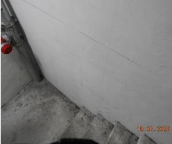
Figure 402 - General condition of level 1 fire stairs internal wall
