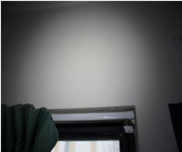
Figure 914 - General condition of bedroom 3 internal wall
