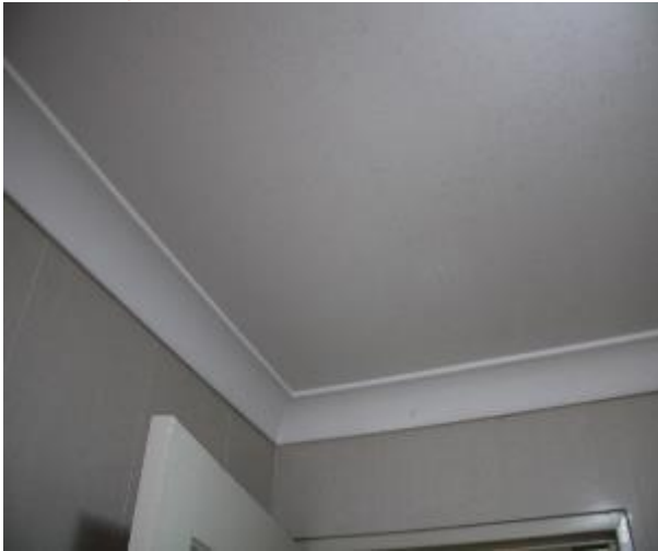
Figure 703 - General condition of bathroom 1 ceiling
