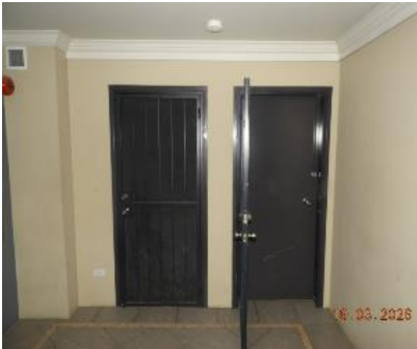
Figure 27 - General condition of level 1 common area internal wall
