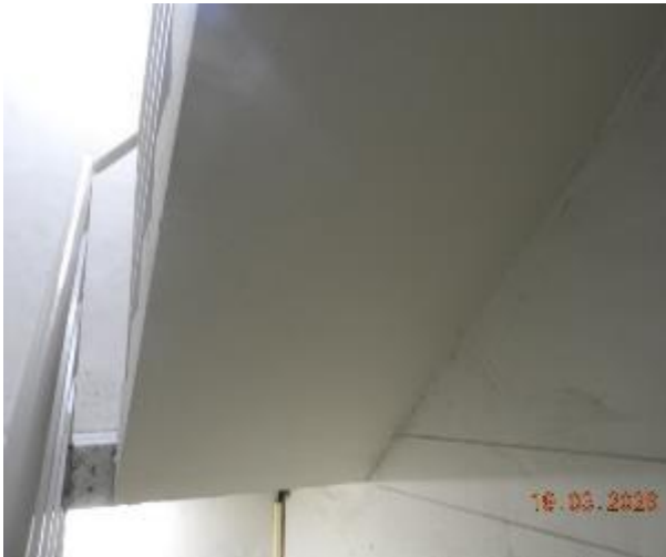
Figure 344 - General condition of level 3 fire stairs underside stairs
