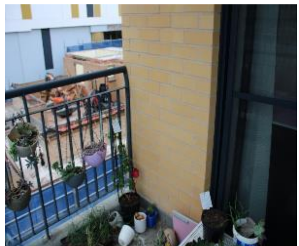
Figure 1091 - General condition of external wall
