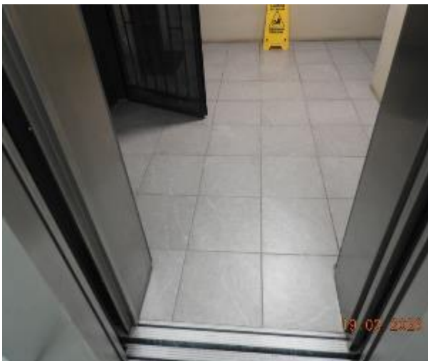
Figure 147 - General condition of level 5 common area floor tiles
