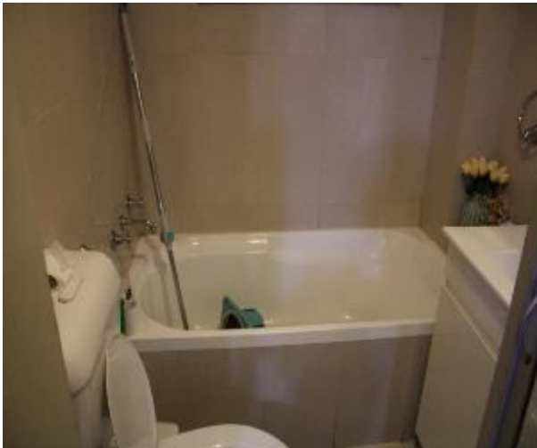
Figure 559 - General condition of bathroom 1 internal wall
