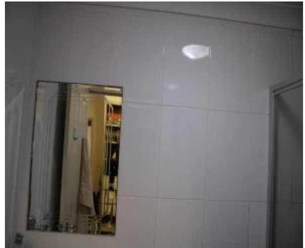
Figure 718 - General condition of ensuite bathroom internal wall
