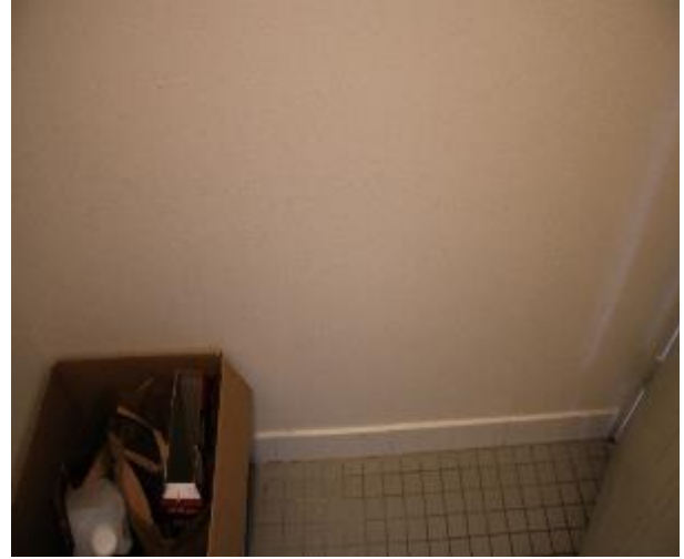
Figure 1494 - General condition of laundry internal wall
