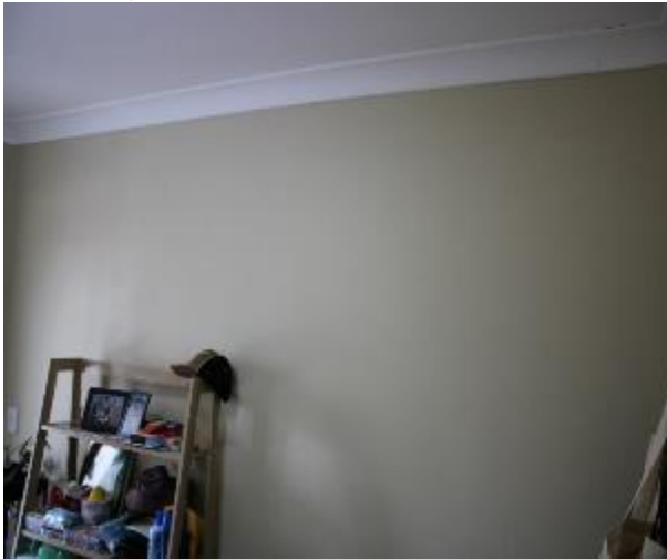
Figure 1424 - General condition of study internal wall
