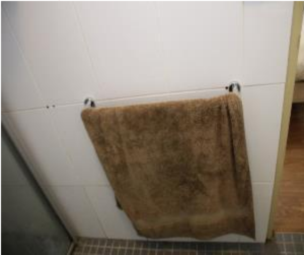
Figure 1406 - General condition of ensuite bathroom internal wall
