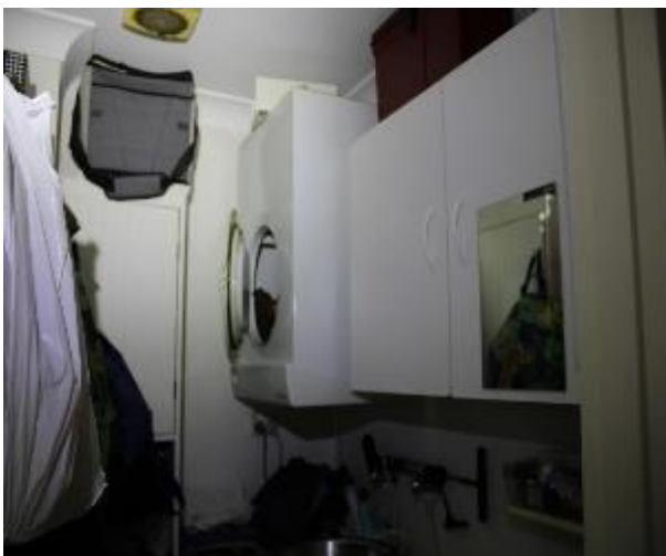
Figure 874 - General condition of laundry internal wall
