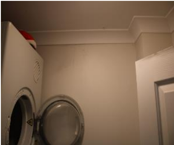
Figure 974 - General condition of laundry internal wall
