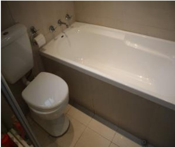
Figure 1008 - General condition of bathroom 1 internal wall
