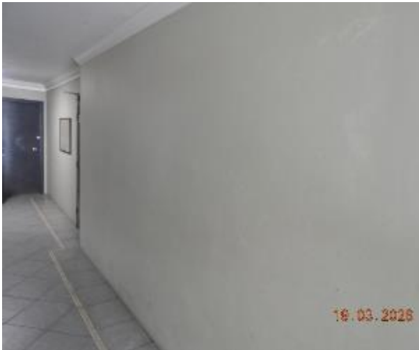
Figure 9 - General condition of level 1 common area internal wall
