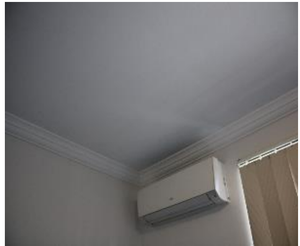
Figure 1616 - General condition of bedroom 3 ceiling
