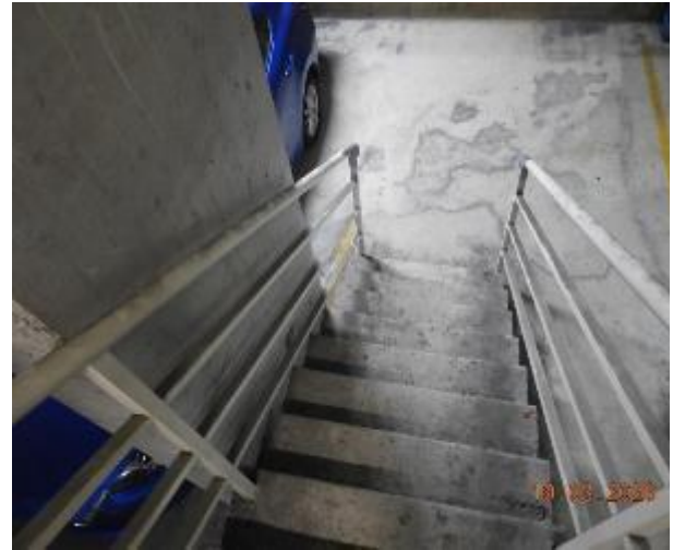
Figure 469 - General condition of basement fire stairs
