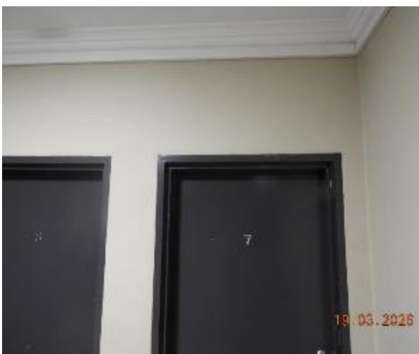
Figure 65 - General condition of level 2 common area internal wall
