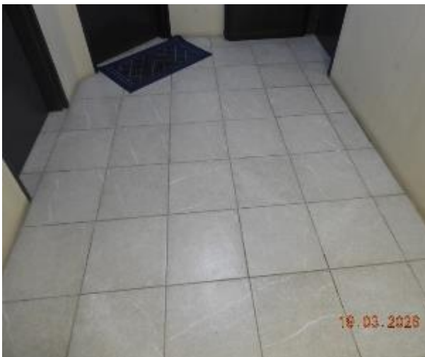
Figure 119 - General condition of level 4 common area floor tiles
