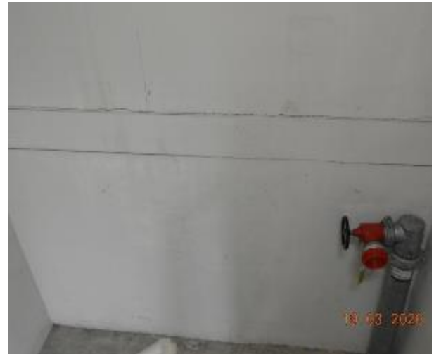
Figure 297 - General condition of level 5 fire stairs internal wall
