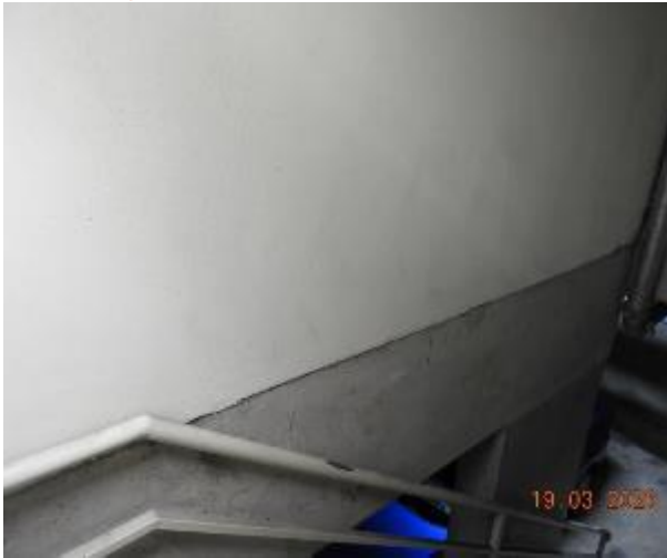
Figure 456 - General condition of basement fire stairs internal wall
