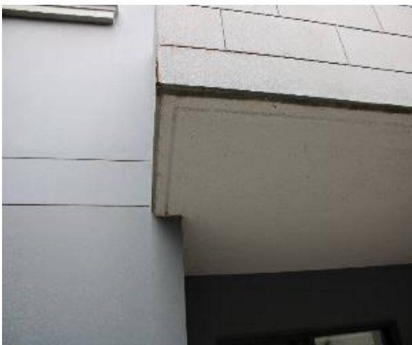
Figure 511 - General condition of balcony underside slab
