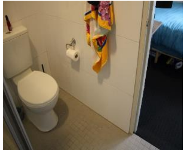
Figure 1632 - General condition of ensuite bathroom internal wall
