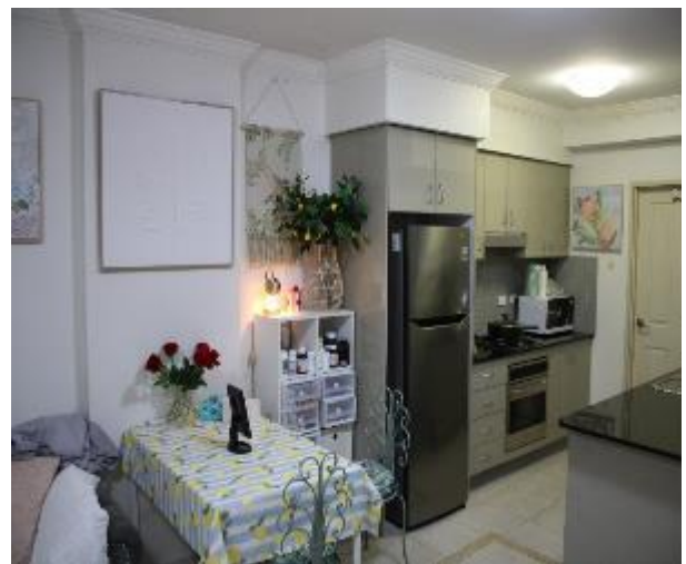
Figure 526 - General condition of open kitchen/ lounge room internal wall
