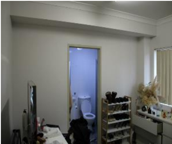
Figure 705 - General condition of dressing room internal wall
