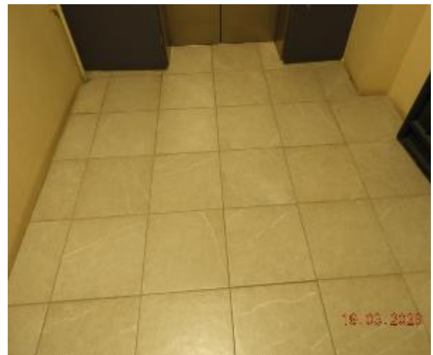
Figure 148 - General condition of level 5 common area floor tiles
