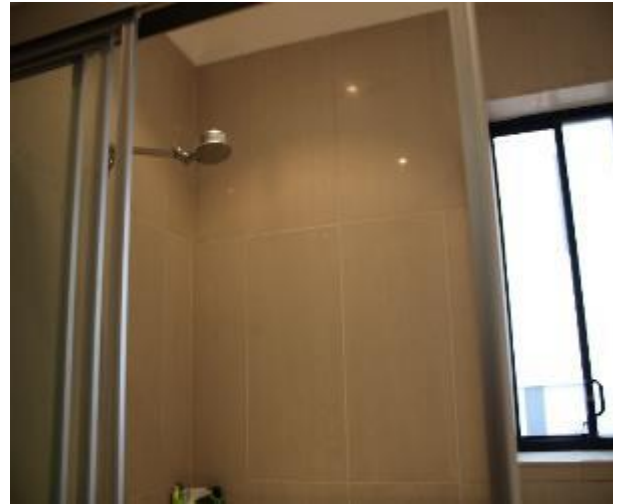
Figure 997 - General condition of bathroom 1 internal wall
