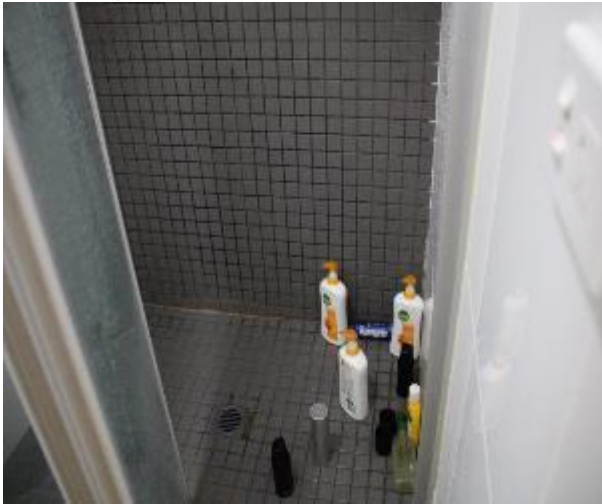
Figure 715 - General condition of ensuite bathroom internal wall
