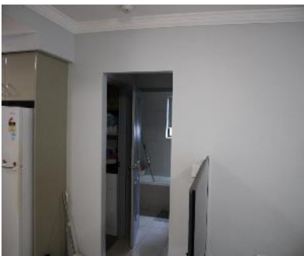
Figure 481 - General condition of open kitchen/ lounge room internal wall
