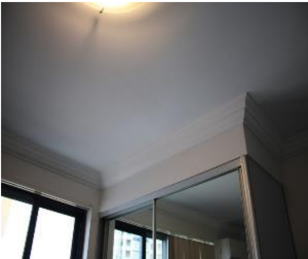
Figure 1615 - General condition of bedroom 3 ceiling
