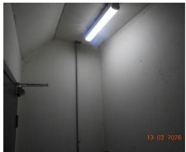
Figure 431 - General condition of level 1 fire stairs internal wall
