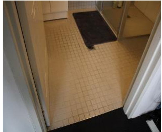
Figure 1620 - General condition of ensuite bathroom floor tiles
