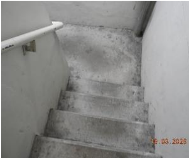
Figure 396 - General condition of level 1 fire stairs
