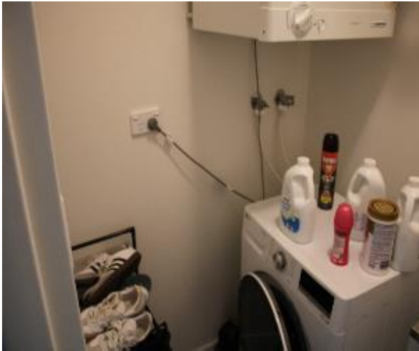
Figure 972 - General condition of laundry internal wall
