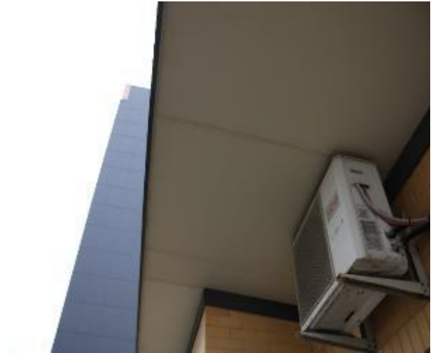
Figure 1530 - General condition of balcony underside slab
