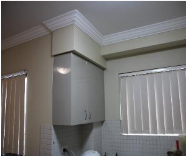
Figure 1304 - General condition of kitchen internal wall
