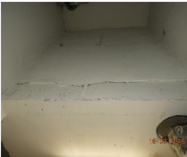
Figure 464 - General condition of basement fire stairs internal wall
