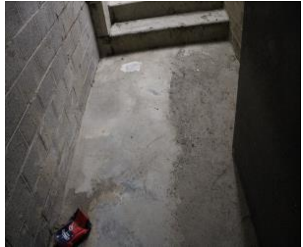
Figure 186 - General condition of B2 fire stairs concrete floor
