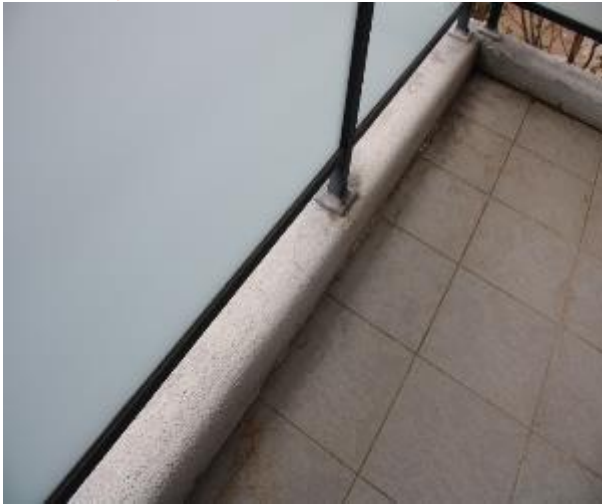
Figure 1253 - General condition of balcony floor tiles
