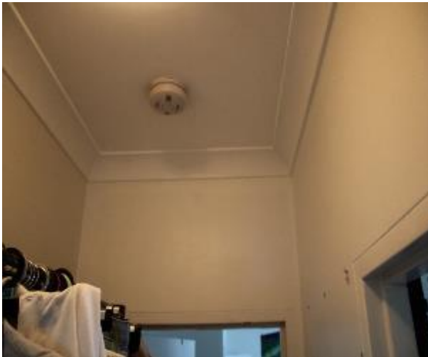
Figure 878 - General condition of corridor internal wall
