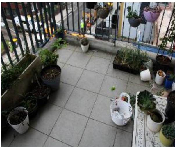
Figure 1078 - General condition of balcony floor tiles
