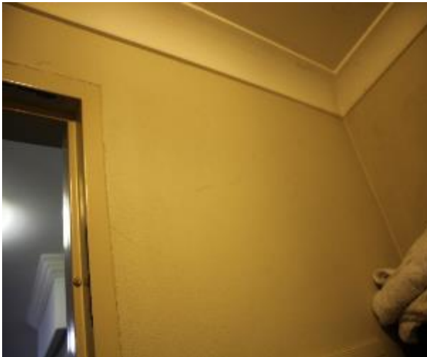
Figure 583 - General condition of laundry internal wall
