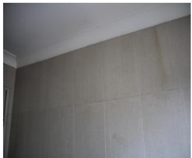
Figure 780 - General condition of bathroom 1 internal wall
