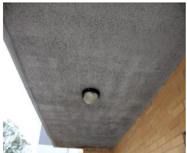
Figure 1447 - General condition of balcony underside slab
