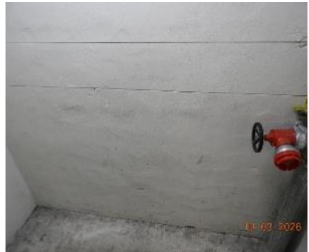
Figure 405 - General condition of level 1 fire stairs internal wall
