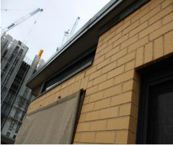
Figure 1523 - General condition of external wall
