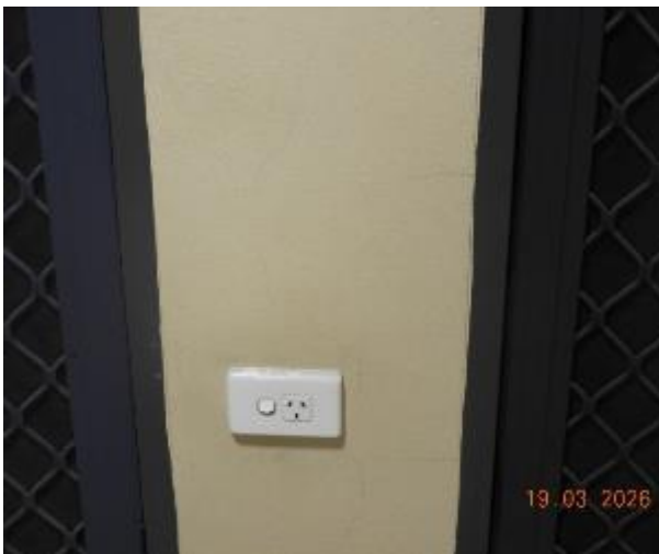
Figure 99 - Crack propagation through level 3 common area internal wall
