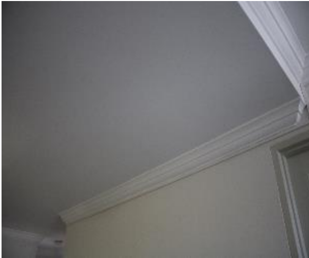
Figure 1481 - General condition of open kitchen/ lounge room ceiling
