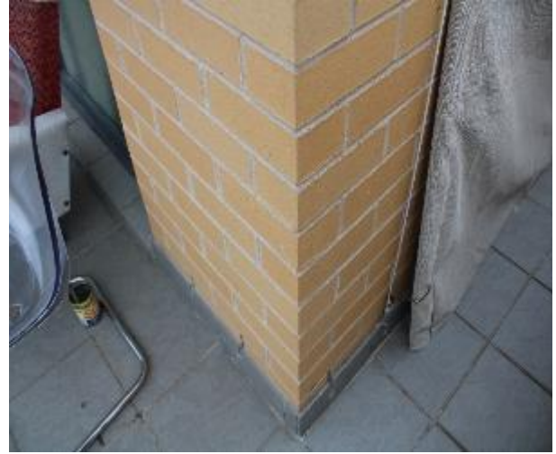
Figure 1524 - General condition of external wall
