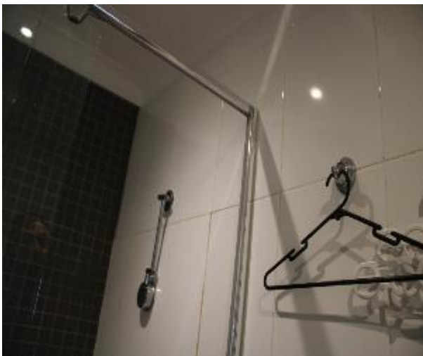
Figure 1046 - General condition of ensuite bathroom internal wall
