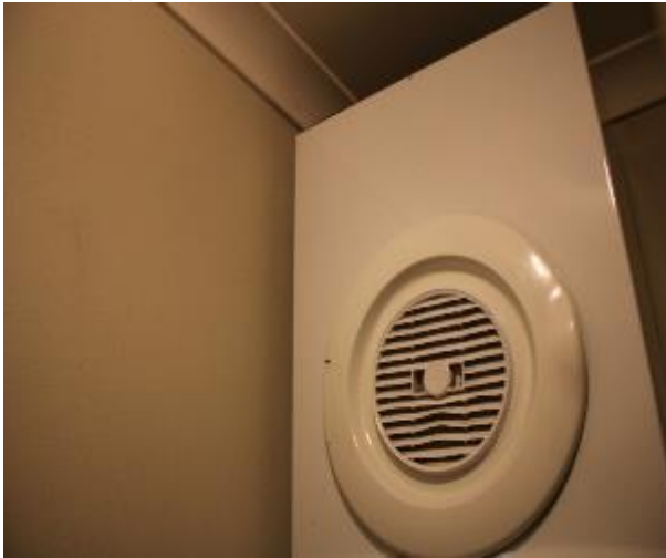
Figure 575 - General condition of laundry internal wall
