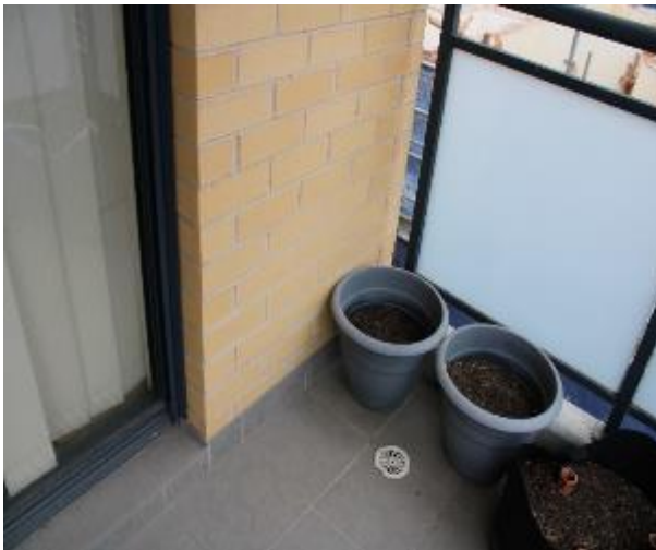
Figure 1444 - General condition of external wall
