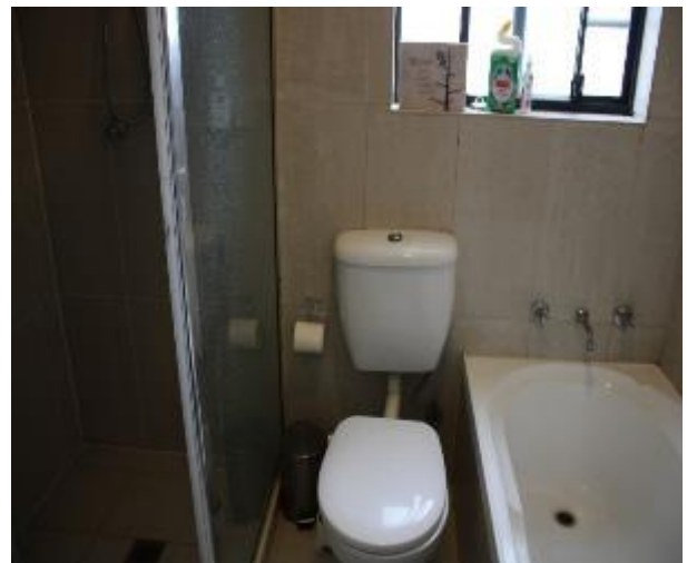
Figure 1586 - General condition of bathroom 1 internal wall
