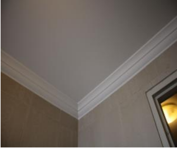
Figure 1601 - General condition of bathroom 1 ceiling
