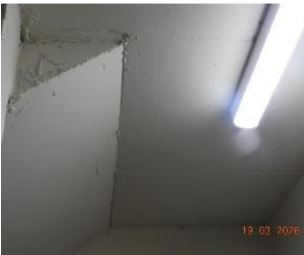
Figure 412 - General condition of level 1 fire stairs underside stairs
