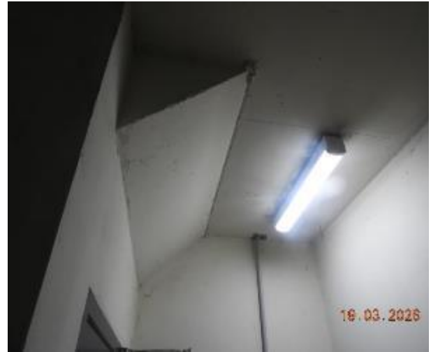
Figure 439 - General condition of level 1 fire stairs underside stairs
