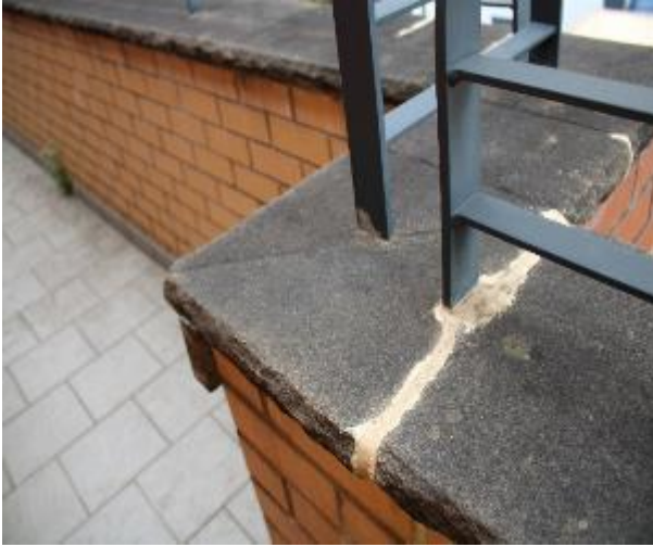
Figure 1541 - General condition of balcony balustrade
