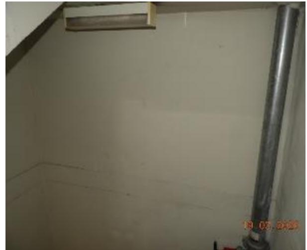
Figure 333 - General condition of level 3 fire stairs internal wall
