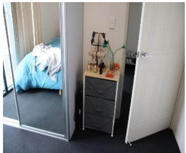
Figure 1612 - General condition of bedroom 3 internal wall
