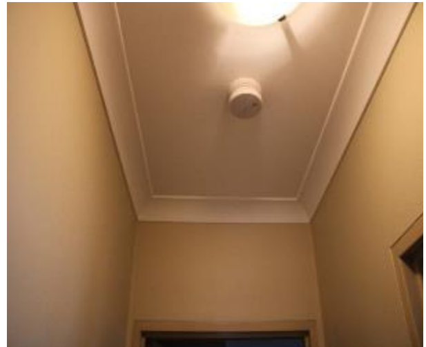
Figure 1337 - General condition of corridor ceiling
