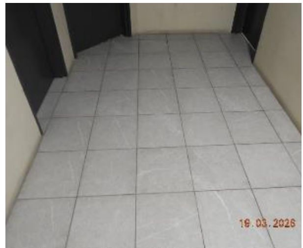
Figure 46 - General condition of level 2 common area floor tiles
