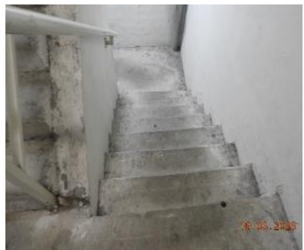
Figure 395 - General condition of level 1 fire stairs
