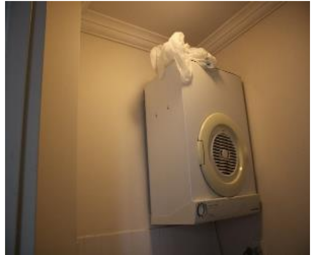
Figure 1488 - General condition of laundry internal wall
