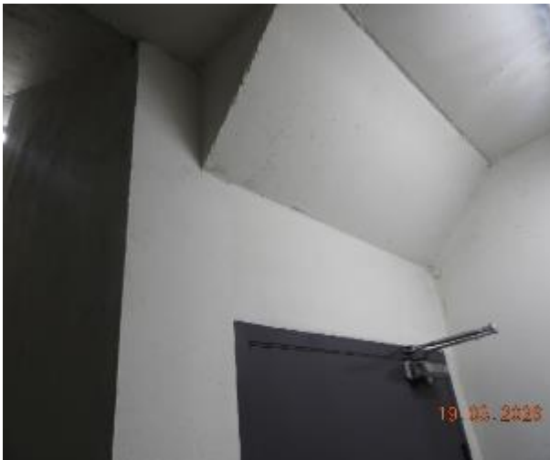
Figure 434 - General condition of level 1 fire stairs internal wall
