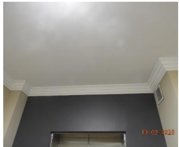
Figure 112 - General condition of level 3 common area ceiling
