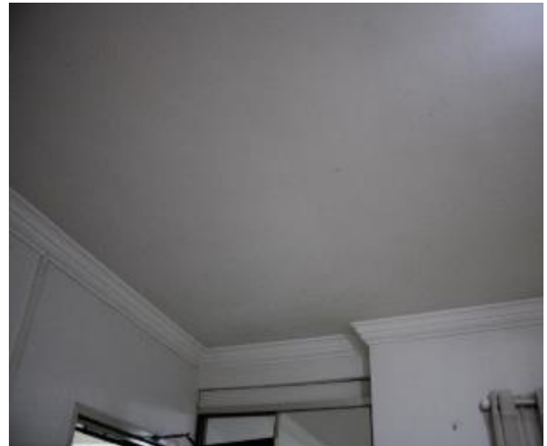
Figure 542 - General condition of open kitchen/ lounge room ceiling
