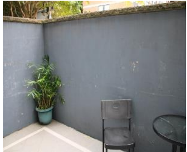
Figure 612 - General condition of courtyard external wall
