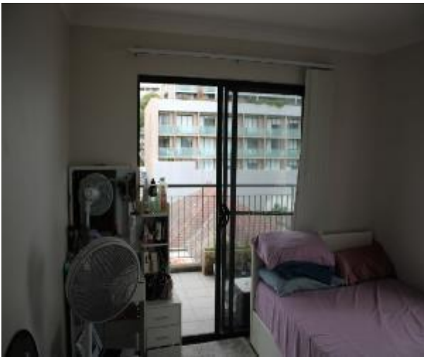
Figure 1058 - General condition of bedroom 2 internal wall
