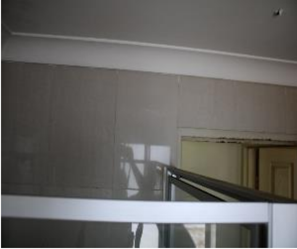
Figure 781 - General condition of bathroom 1 internal wall
