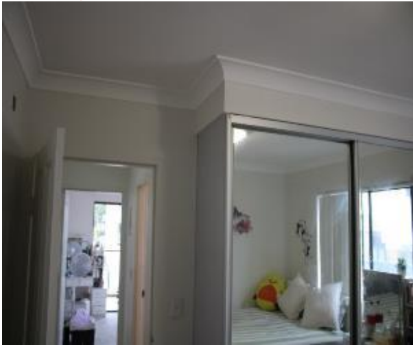
Figure 1032 - General condition of bedroom 1 internal wall
