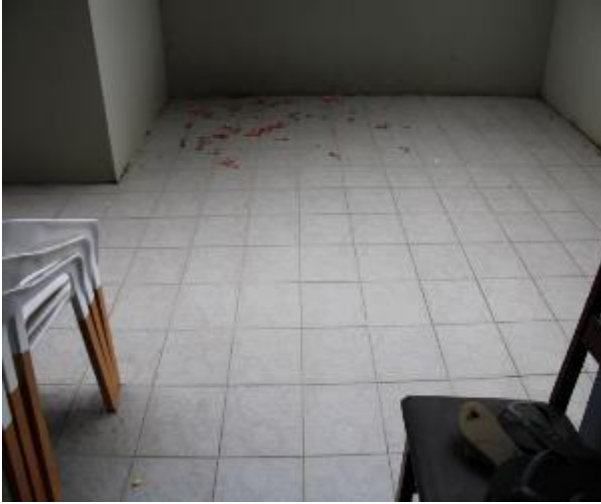
Figure 495 - General condition of courtyard floor tiles
