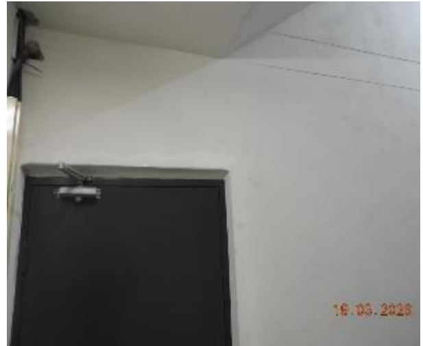
Figure 385 - General condition of level 2 fire stairs internal wall
