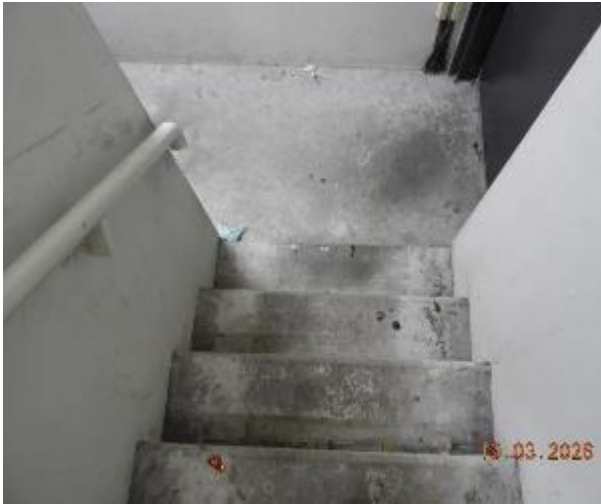
Figure 420 - General condition of level 1 fire stairs concrete floor
