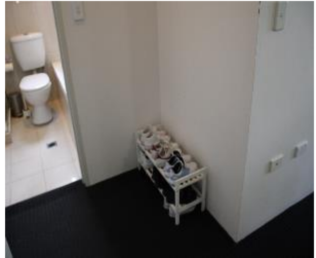
Figure 1572 - General condition of corridor internal wall
