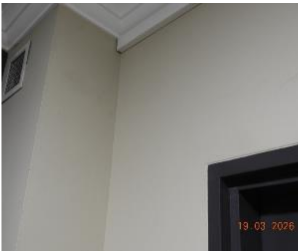
Figure 69 - General condition of level 2 common area internal wall
