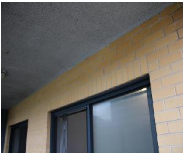
Figure 657 - General condition of external wall
