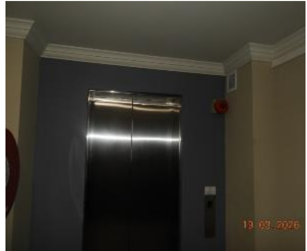
Figure 32 - General condition of level 1 common area internal wall
