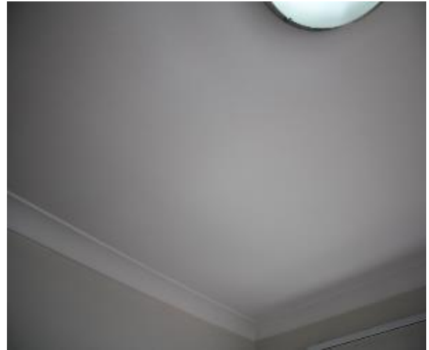
Figure 1075 - General condition of bedroom 2 ceiling
