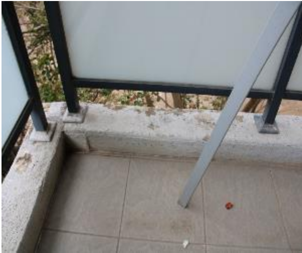
Figure 829 - General condition of balcony floor tiles
