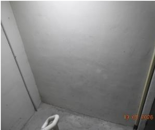
Figure 320 - General condition of level 4 fire stairs internal wall
