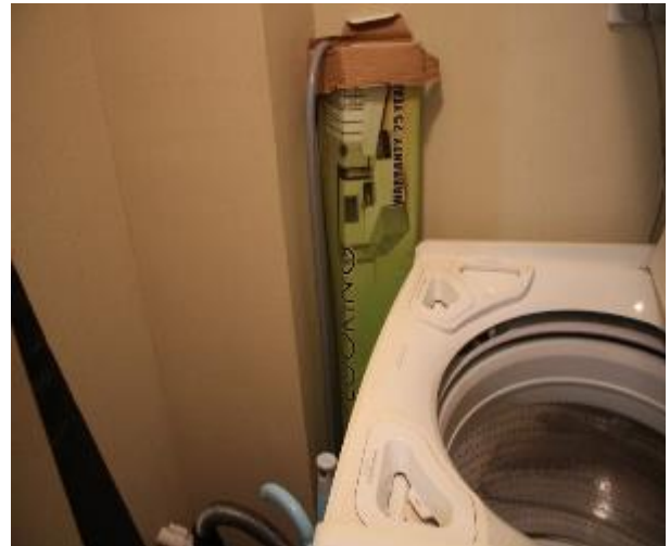
Figure 1319 - General condition of laundry internal wall
