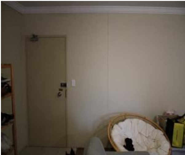
Figure 1270 - General condition of lounge room internal wall
