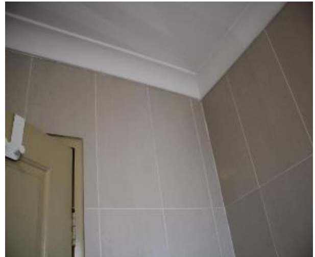
Figure 1355 - General condition of bathroom 1 internal wall
