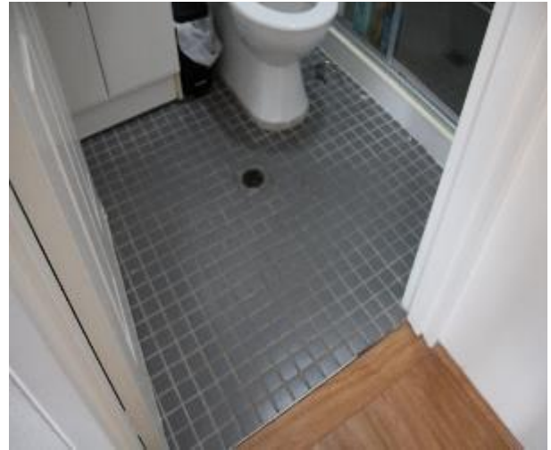
Figure 1206 - General condition of ensuite bathroom floor tiles
