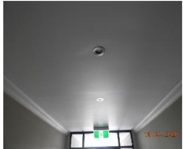
Figure 40 - General condition of level 1 common area ceiling
