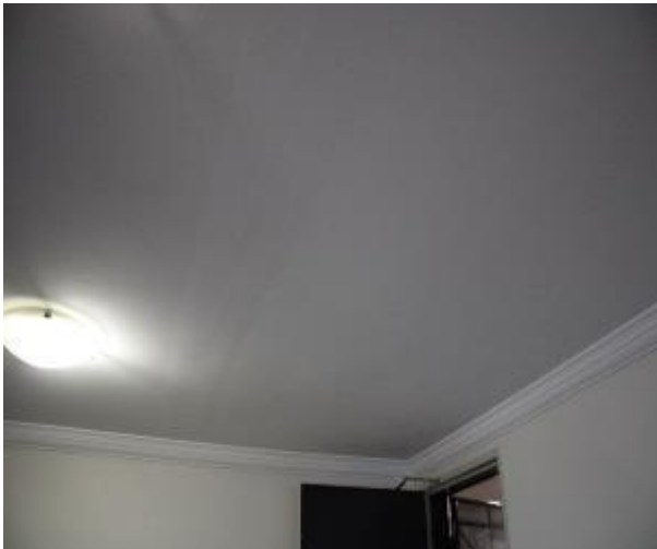
Figure 1483 - General condition of open kitchen/ lounge room ceiling
