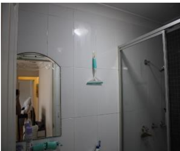
Figure 1209 - General condition of ensuite bathroom internal wall
