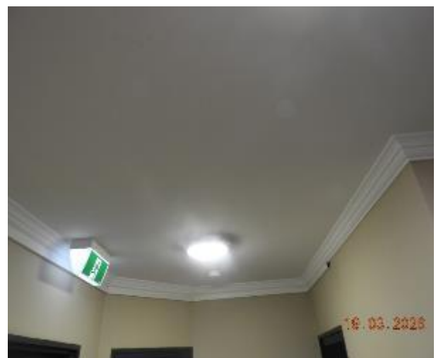
Figure 114 - General condition of level 3 common area ceiling
