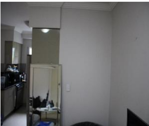
Figure 629 - General condition of lounge room internal wall
