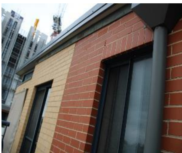
Figure 1519 - General condition of external wall
