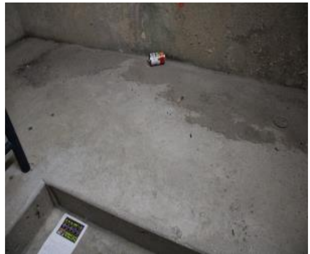
Figure 188 - General condition of B2 fire stairs concrete floor
