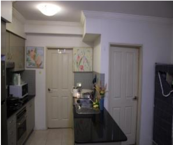
Figure 533 - General condition of open kitchen/ lounge room internal wall
