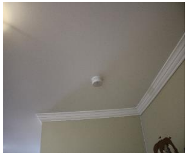
Figure 1297 - General condition of lounge room ceiling
