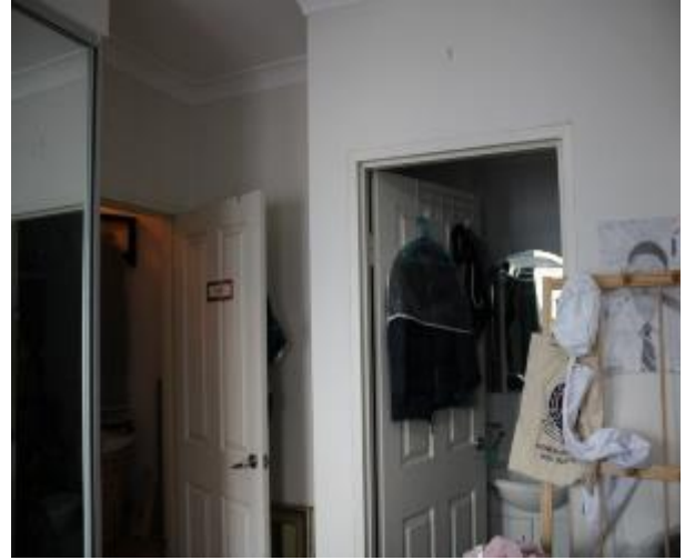
Figure 895 - General condition of bedroom 2 internal wall
