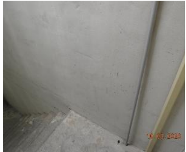
Figure 289 - General condition of level 5 fire stairs internal wall
