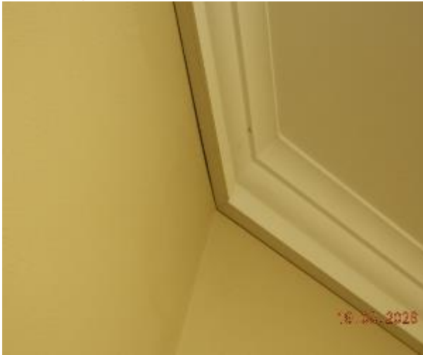
Figure 115 - General condition of level 3 common area ceiling
