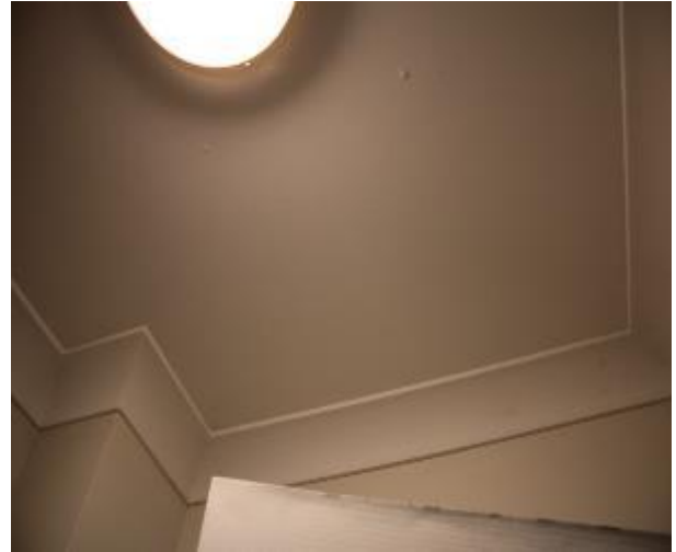
Figure 981 - General condition of laundry ceiling
