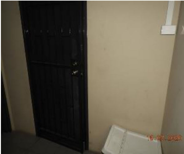
Figure 157 - General condition of level 5 common area internal wall
