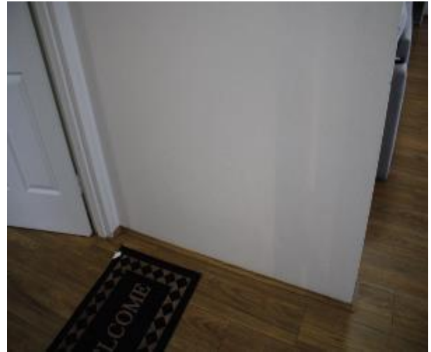
Figure 985 - General condition of corridor internal wall
