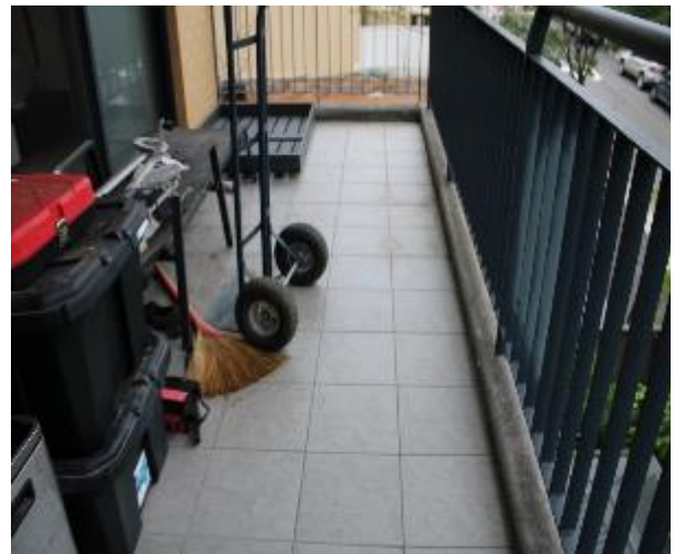
Figure 652 - General condition of balcony floor tiles
