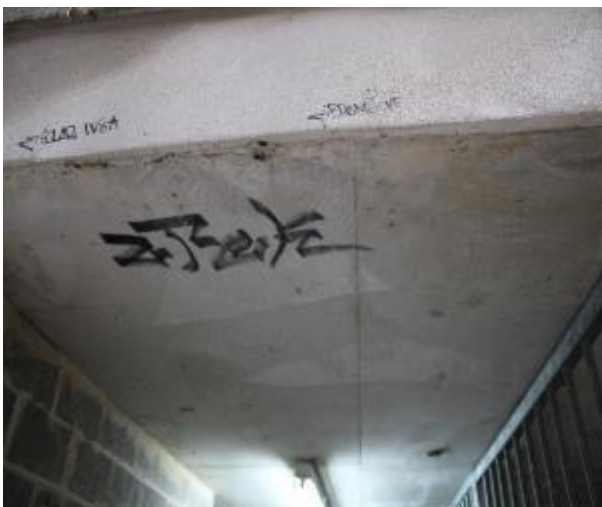
Figure 273 - General condition of fire stairs underside slab
