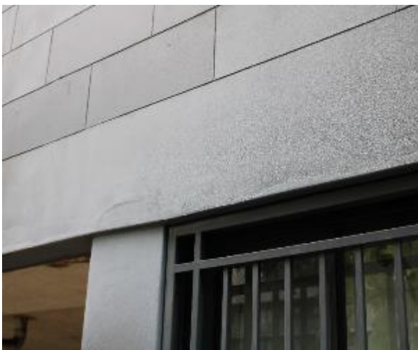
Figure 603 - General condition of external wall
