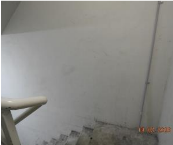
Figure 390 - General condition of level 2 fire stairs internal wall
