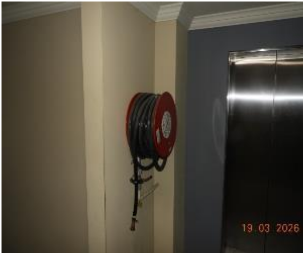
Figure 33 - General condition of level 1 common area internal wall
