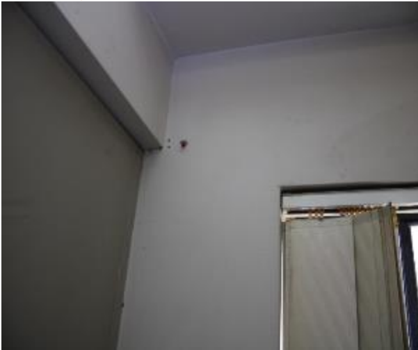
Figure 751 - General condition of open kitchen/ lounge room internal wall
