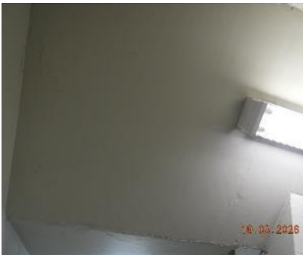
Figure 392 - General condition of level 2 fire stairs underside stairs
