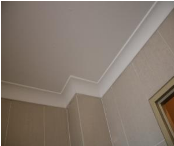
Figure 1360 - General condition of bathroom 1 ceiling
