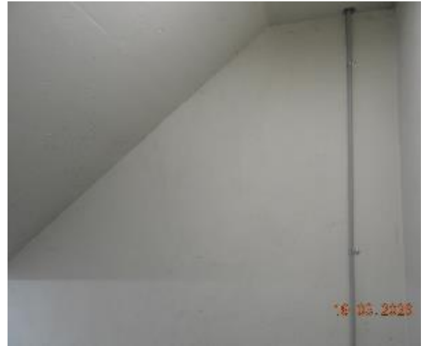
Figure 391 - General condition of level 2 fire stairs internal wall
