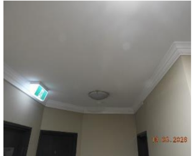
Figure 74 - General condition of level 2 common area ceiling
