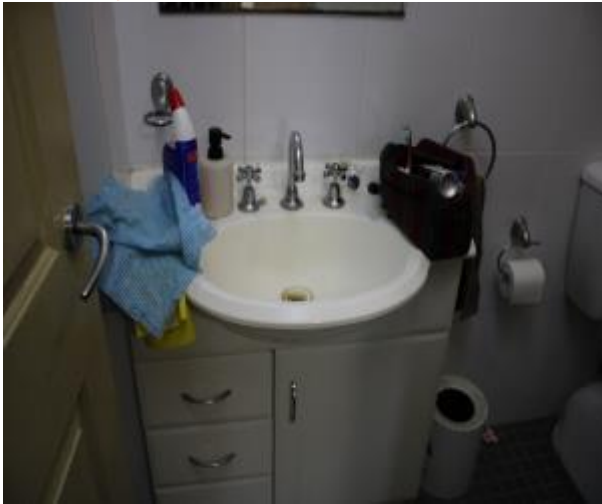
Figure 1400 - General condition of ensuite bathroom internal wall
