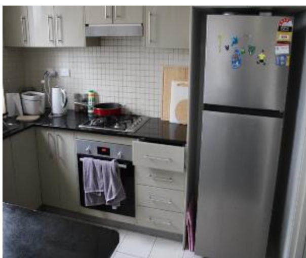
Figure 1467 - General condition of open kitchen/ lounge room internal wall
