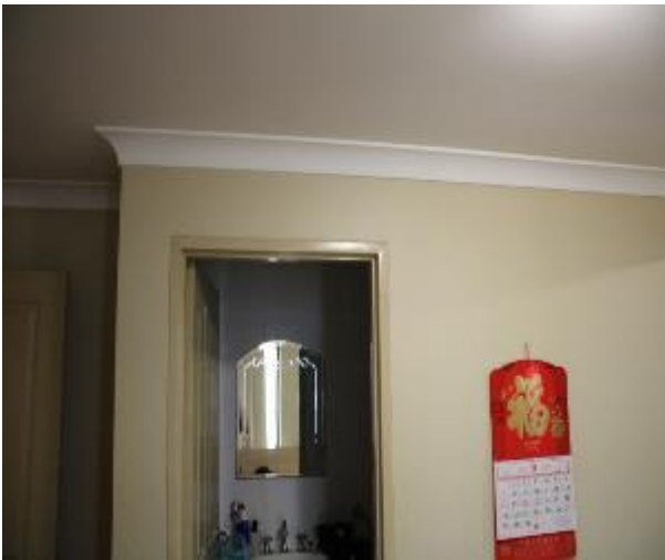
Figure 1372 - General condition of bedroom 1 internal wall
