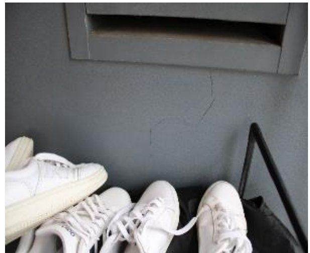
Figure 1085 - Crack propagation through external wall
