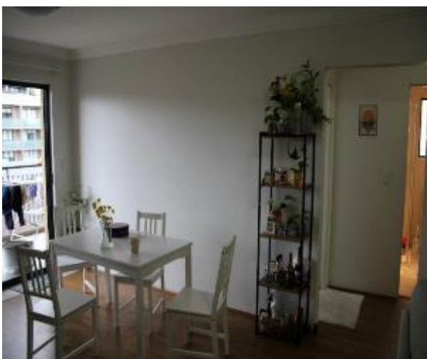
Figure 940 - General condition of lounge room internal wall
