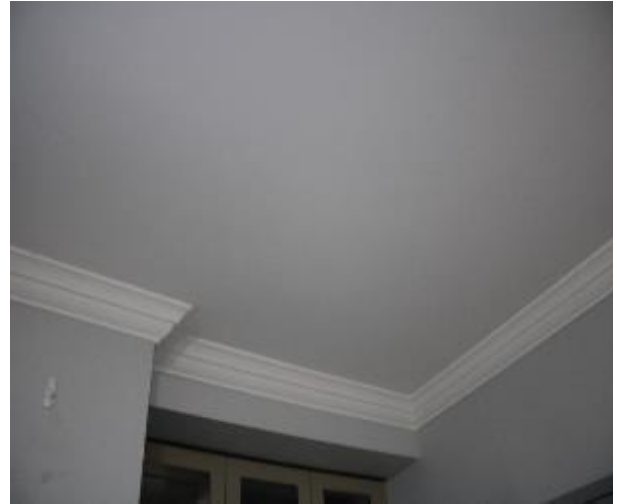
Figure 492 - General condition of open kitchen/ lounge room ceiling
