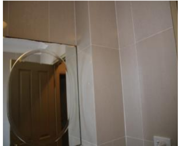
Figure 1359 - General condition of bathroom 1 internal wall
