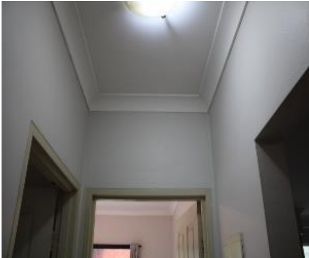
Figure 679 - General condition of corridor internal wall
