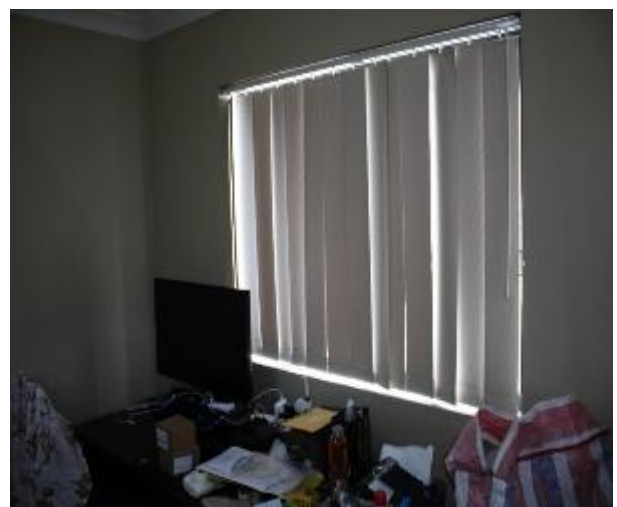
Figure 1417 - General condition of study internal wall
