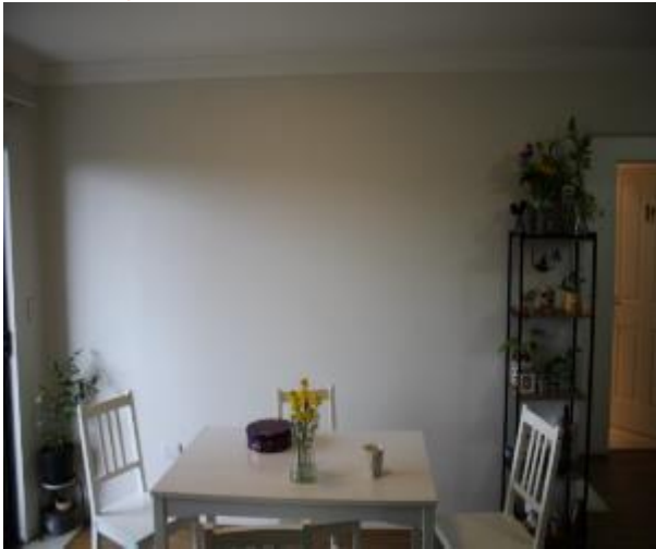
Figure 942 - General condition of lounge room internal wall
