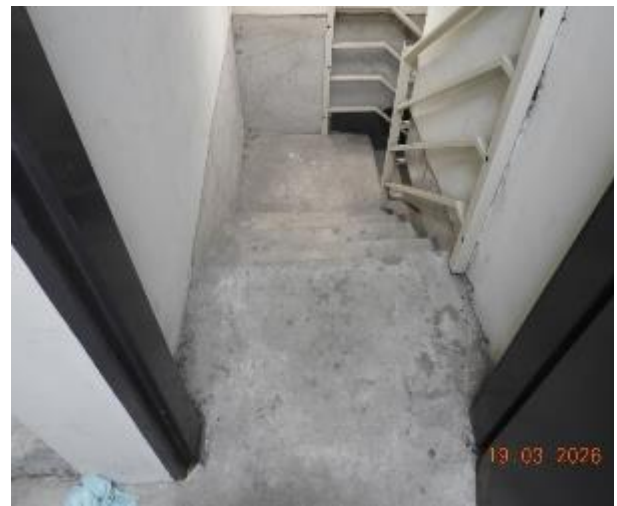
Figure 441 - General condition of basement fire stairs
