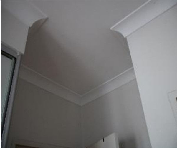
Figure 896 - General condition of bedroom 2 ceiling
