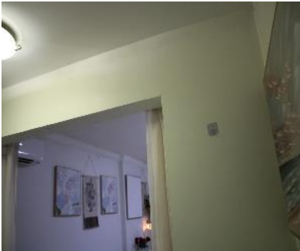
Figure 553 - General condition of bedroom 1 internal wall
