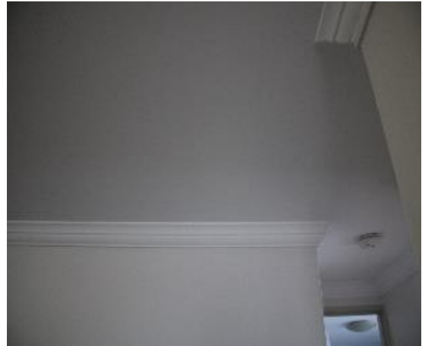
Figure 1482 - General condition of open kitchen/ lounge room ceiling
