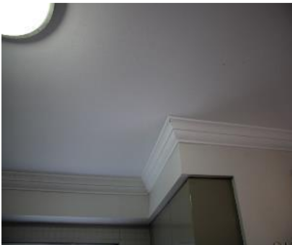
Figure 968 - General condition of kitchen ceiling
