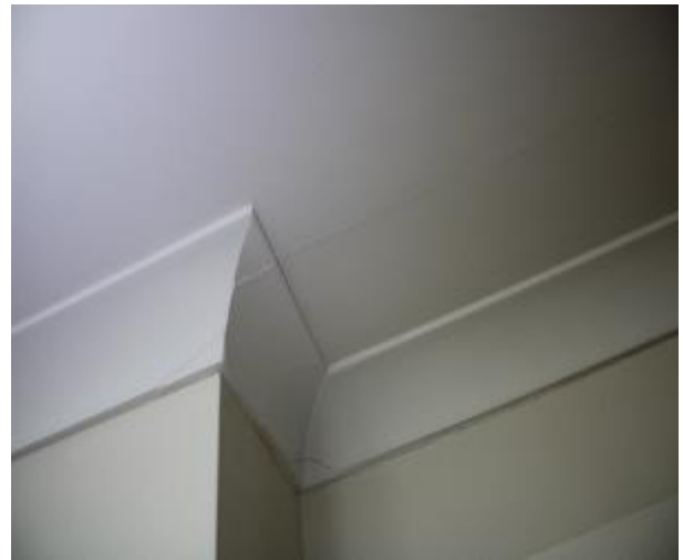
Figure 1202 - Crack propagation through bedroom 1 ceiling
