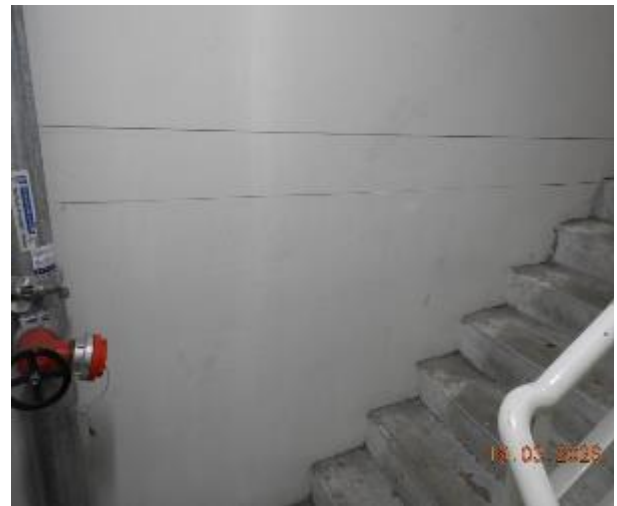
Figure 363 - General condition of level 2 fire stairs internal wall
