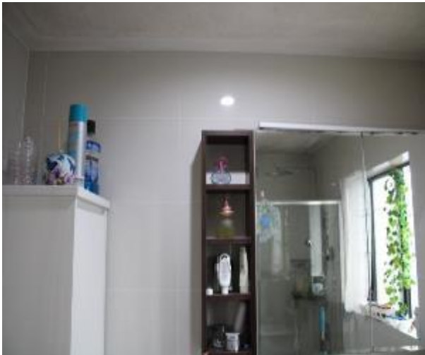
Figure 884 - General condition of bathroom 1 internal wall
