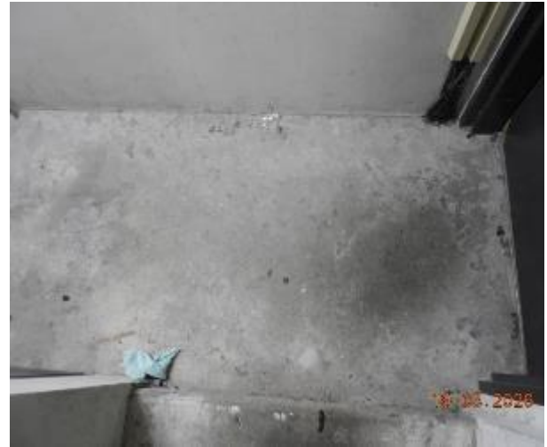
Figure 421 - General condition of level 1 fire stairs concrete floor
