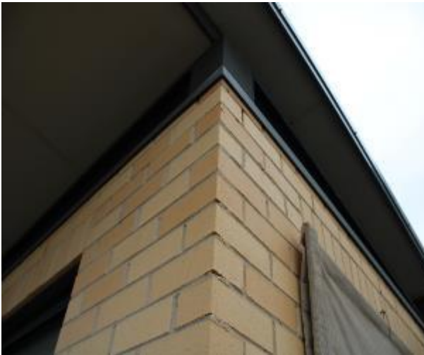
Figure 1525 - General condition of external wall
