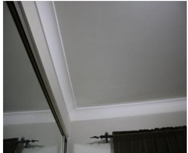
Figure 802 - General condition of bedroom 1 ceiling
