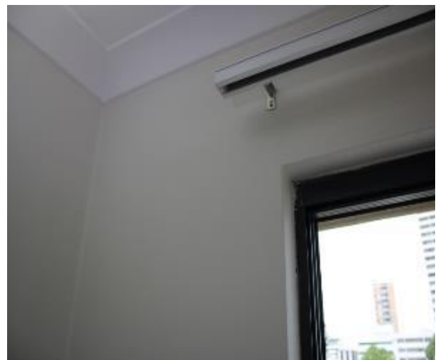
Figure 1061 - General condition of bedroom 2 internal wall
