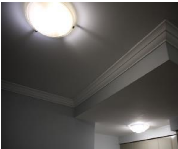
Figure 487 - General condition of open kitchen/ lounge room ceiling
