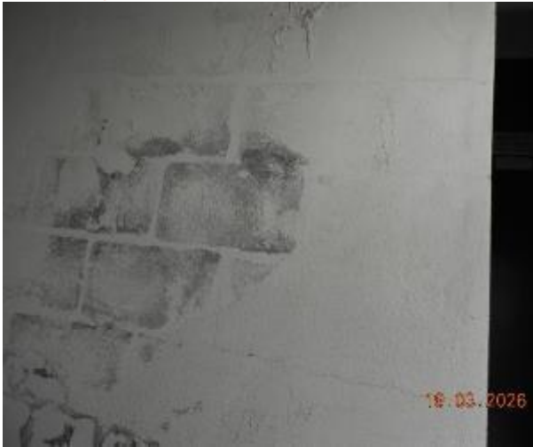
Figure 462 - General condition of basement fire stairs internal wall
