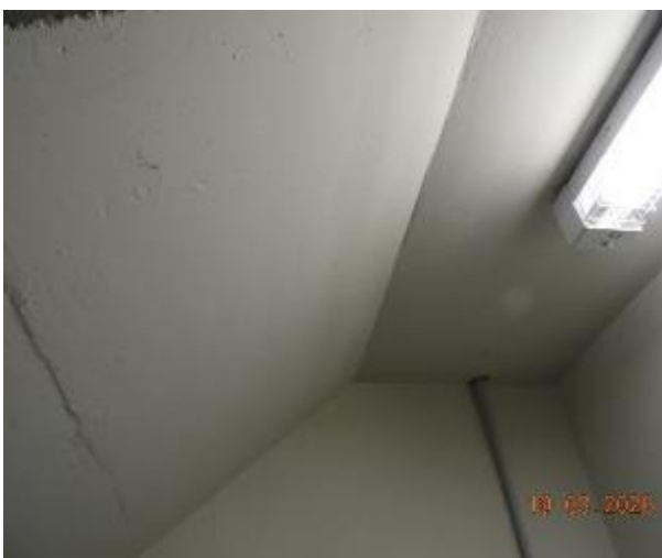
Figure 358 - General condition of level 3 fire stairs underside stairs
