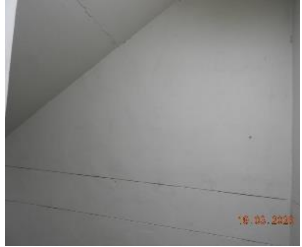
Figure 409 - General condition of level 1 fire stairs internal wall
