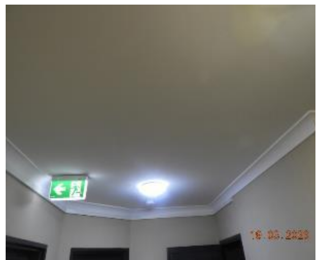
Figure 144 - General condition of level 4 common area ceiling
