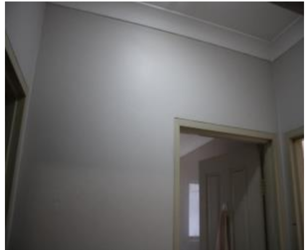
Figure 676 - General condition of corridor internal wall
