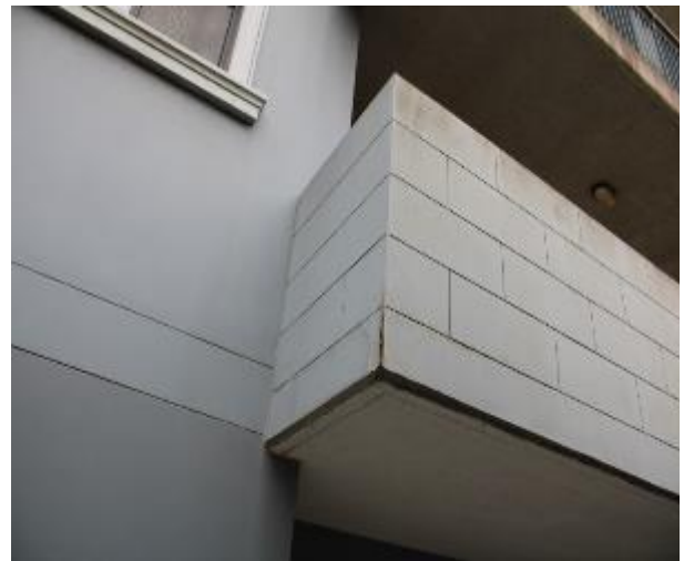
Figure 510 - General condition of external wall
