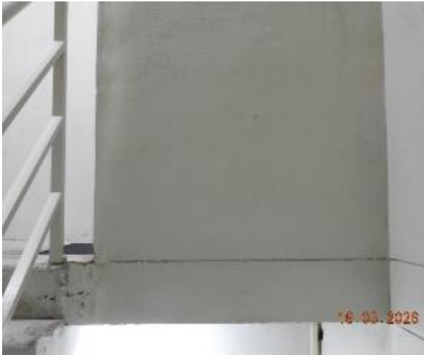
Figure 306 - General condition of level 5 fire stairs internal wall
