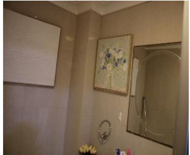
Figure 564 - General condition of bathroom 1 internal wall
