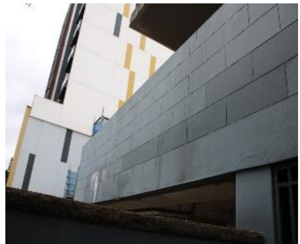
Figure 604 - General condition of external wall
