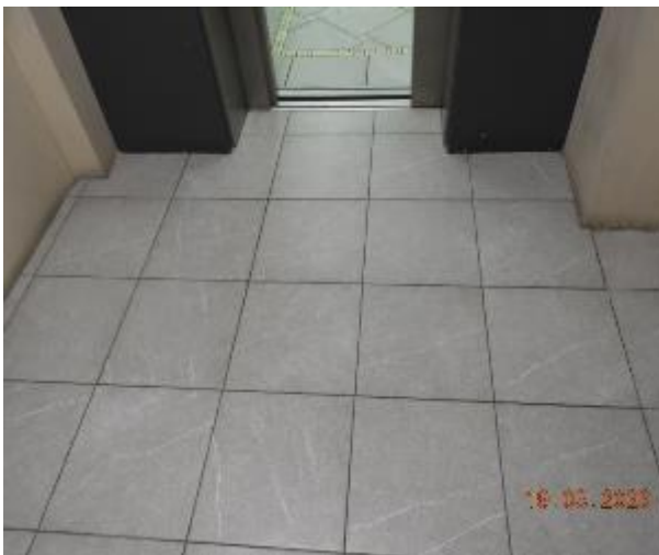
Figure 45 - General condition of level 2 common area floor tiles
