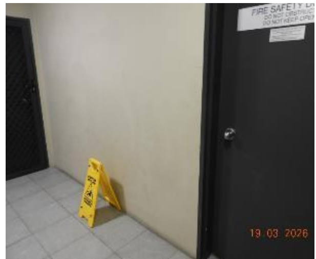
Figure 94 - General condition of level 3 common area internal wall
