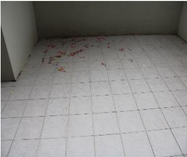
Figure 497 - General condition of courtyard floor tiles
