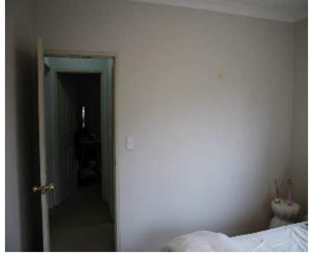
Figure 686 - General condition of bedroom 1 internal wall
