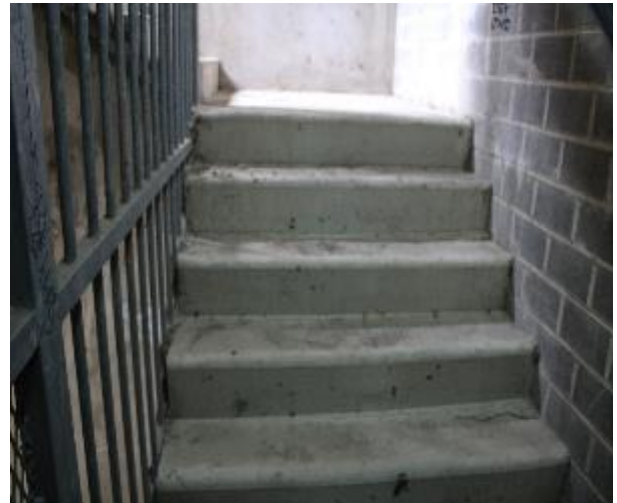
Figure 242 - General condition of level 1 fire stairs
