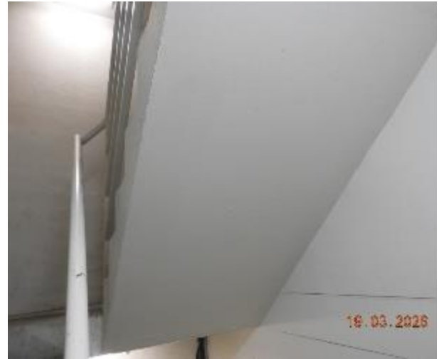
Figure 379 - General condition of level 2 fire stairs underside stairs
