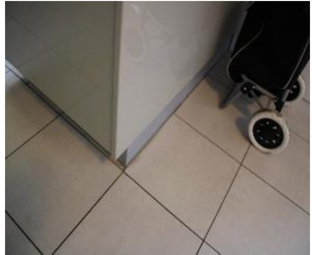
Figure 961 - General condition of kitchen floor tiles
