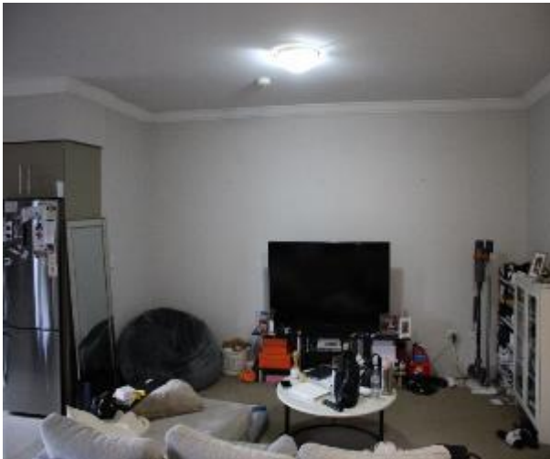
Figure 621 - General condition of lounge room internal wall
