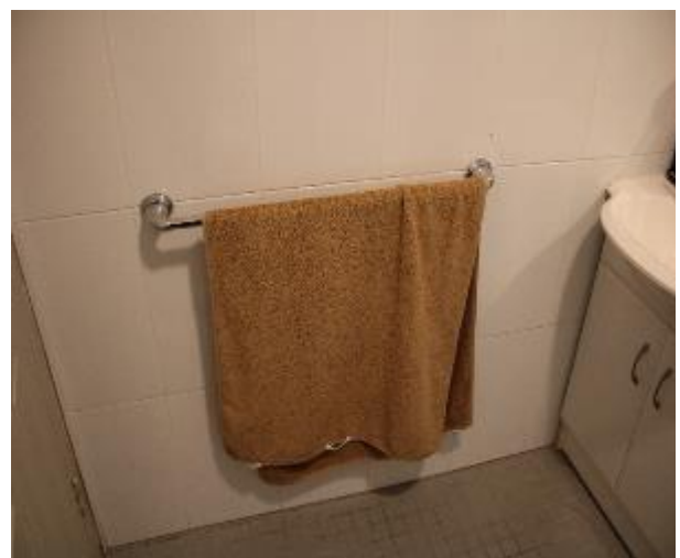
Figure 1630 - General condition of ensuite bathroom internal wall
