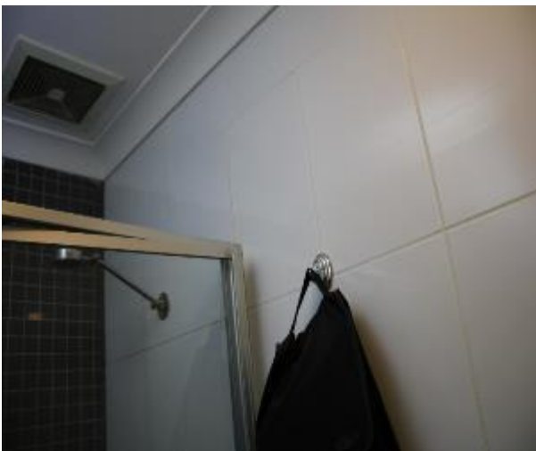
Figure 1408 - General condition of ensuite bathroom internal wall
