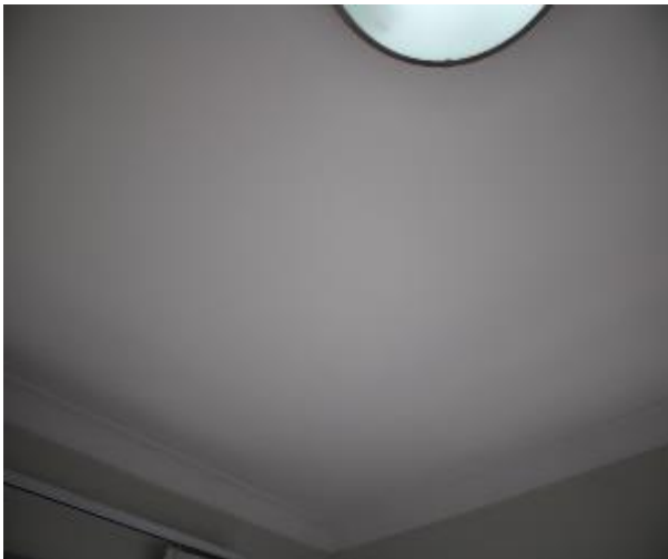
Figure 1076 - General condition of bedroom 2 ceiling
