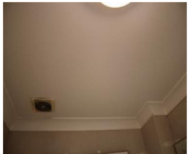
Figure 568 - General condition of bathroom 1 ceiling
