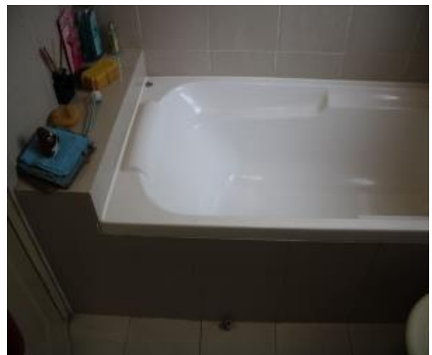
Figure 1351 - General condition of bathroom 1 internal wall
