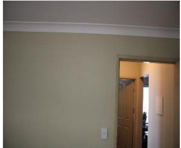
Figure 1377 - General condition of bedroom 1 internal wall
