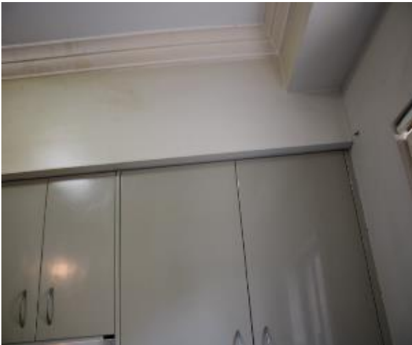
Figure 753 - General condition of open kitchen/ lounge room internal wall
