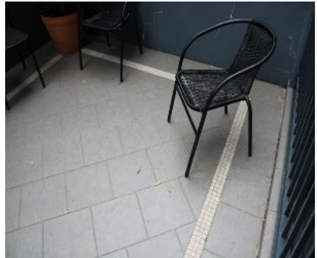
Figure 590 - General condition of courtyard floor tiles
