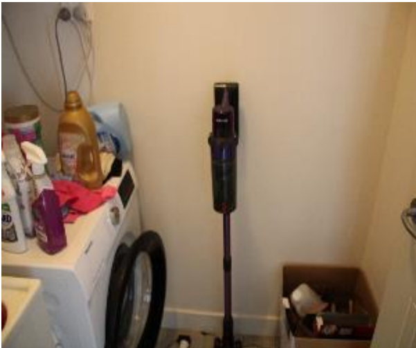
Figure 1489 - General condition of laundry internal wall
