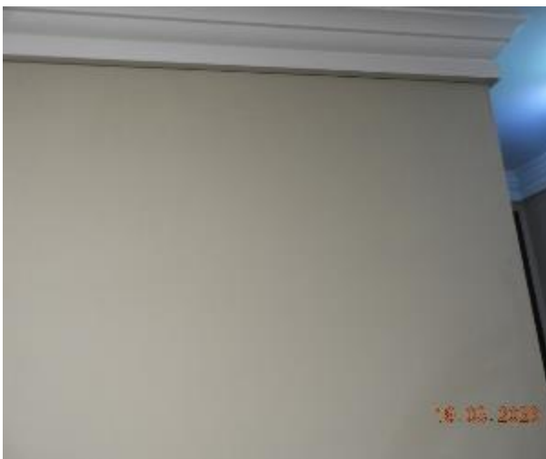
Figure 167 - General condition of level 5 common area internal wall
