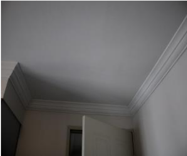
Figure 1619 - General condition of bedroom 3 ceiling
