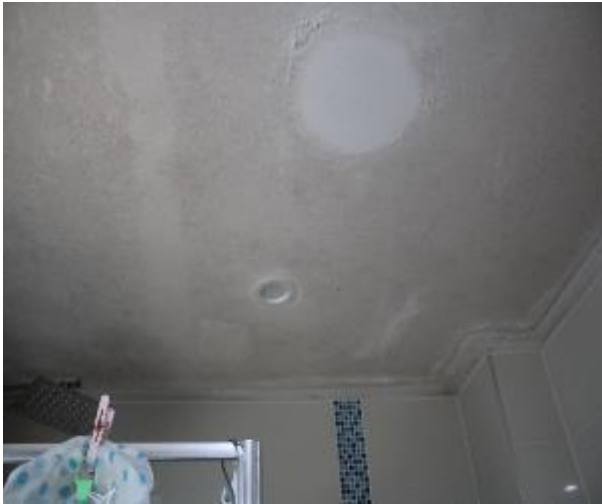
Figure 888 - General condition of bathroom 1 ceiling
