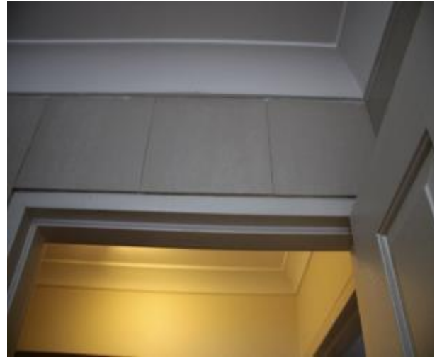
Figure 1170 - General condition of bathroom 1 internal wall
