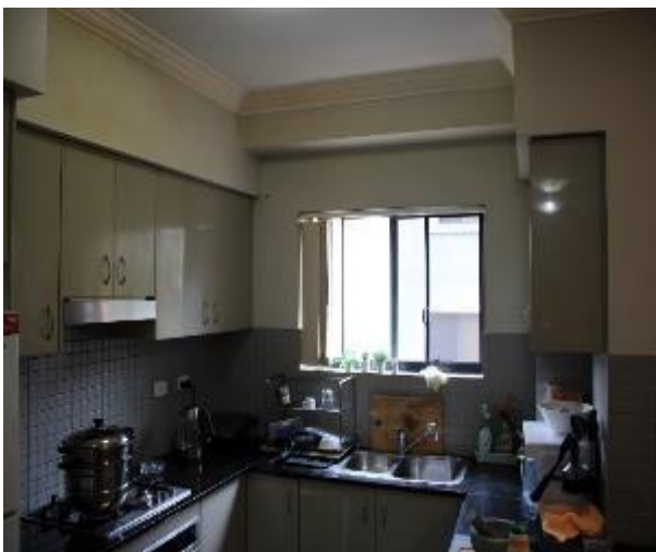
Figure 749 - General condition of open kitchen/ lounge room internal wall
