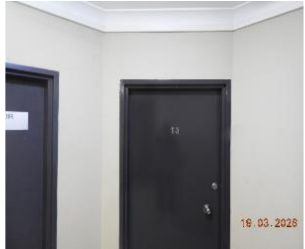
Figure 128 - General condition of level 4 common area internal wall
