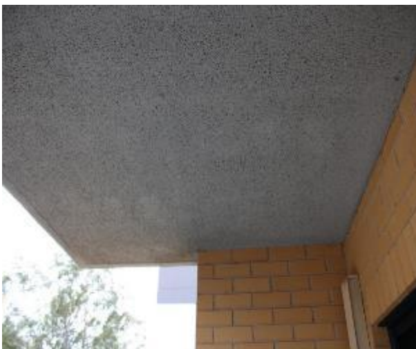
Figure 934 - General condition of balcony underside slab
