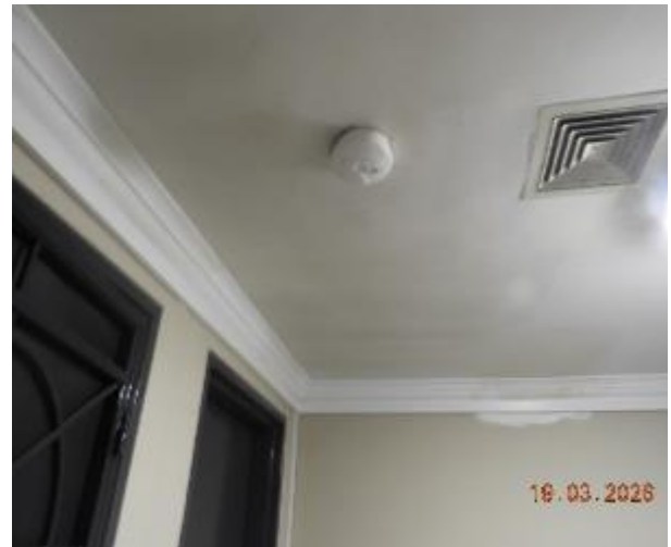
Figure 182 - General condition of level 5 common area ceiling
