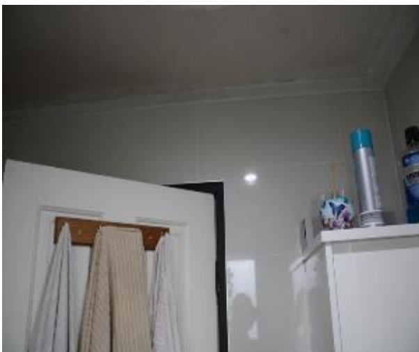
Figure 886 - General condition of bathroom 1 internal wall
