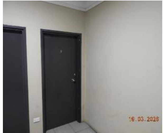
Figure 62 - General condition of level 2 common area internal wall
