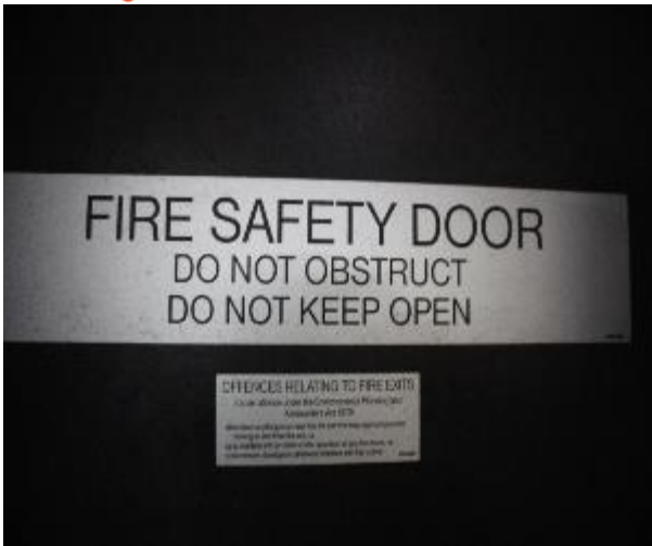
Figure 185 - The following images display the condition of the fire stairs from Basement B2 to Level 1
