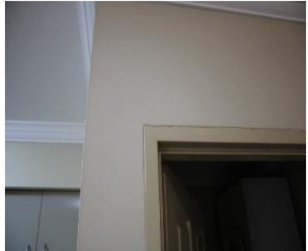
Figure 1281 - Crack propagation through lounge room internal wall
