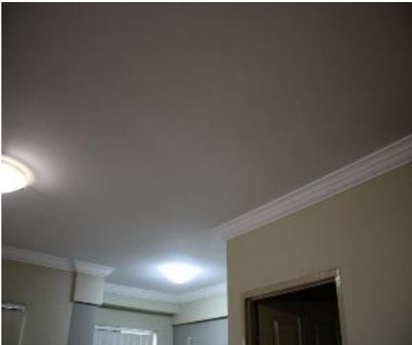
Figure 1300 - General condition of lounge room ceiling
