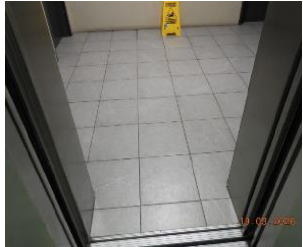
Figure 44 - General condition of level 2 common area floor tiles
