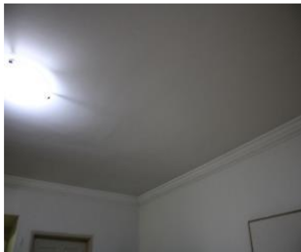
Figure 546 - General condition of open kitchen/ lounge room ceiling
