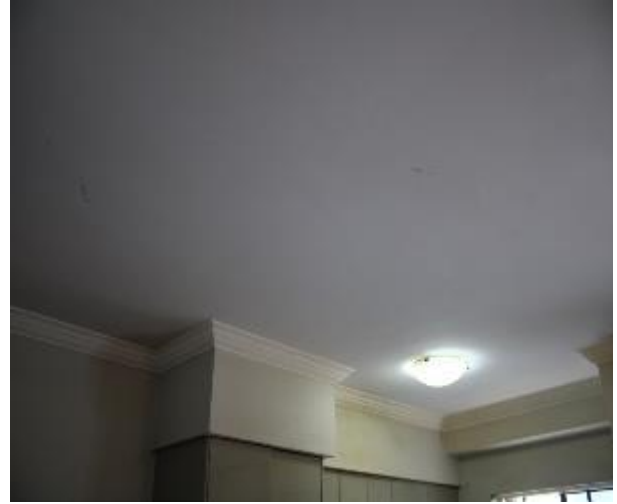
Figure 764 - General condition of open kitchen/ lounge room ceiling
