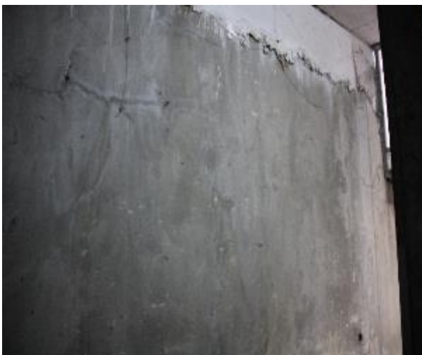
Figure 219 - General condition of B1 fire stairs internal wall
