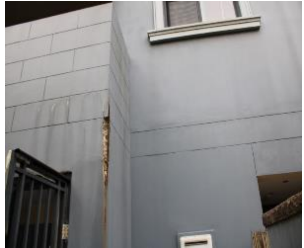
Figure 594 - General condition of external wall
