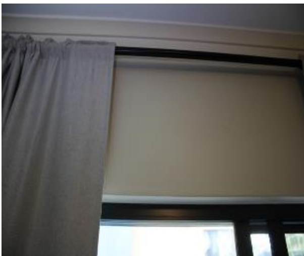
Figure 743 - General condition of open kitchen/ lounge room internal wall
