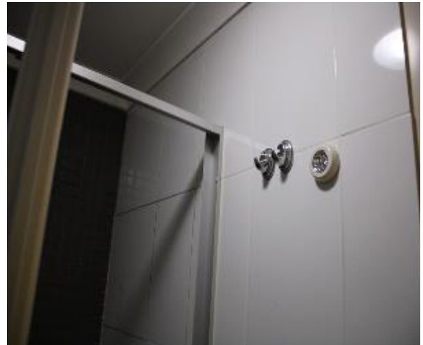
Figure 724 - General condition of ensuite bathroom internal wall
