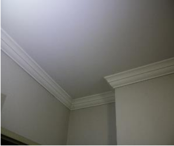
Figure 637 - General condition of lounge room ceiling
