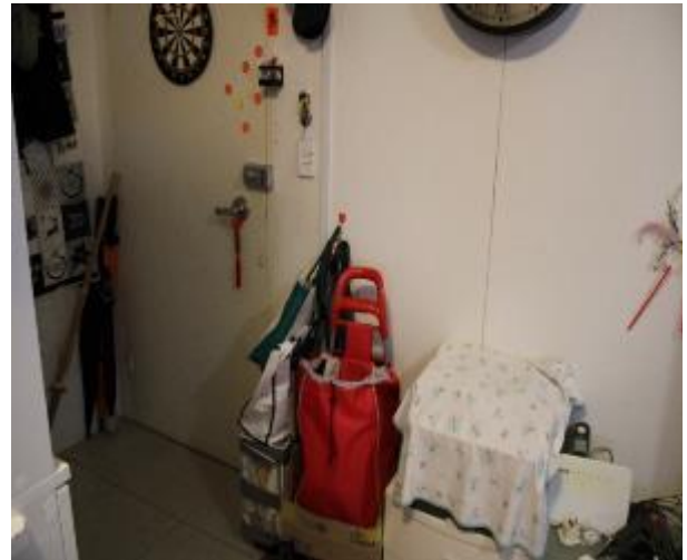
Figure 849 - General condition of bedroom 1 internal wall
