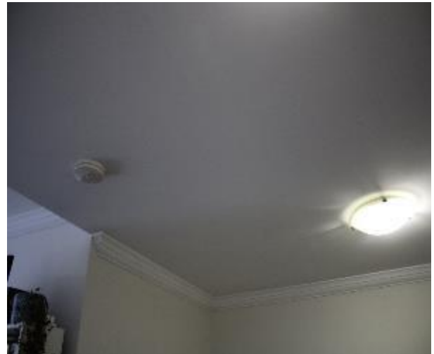
Figure 1484 - General condition of open kitchen/ lounge room ceiling
