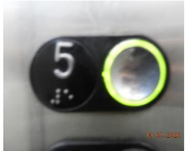
Figure 146 -The following images display the condition of Level 5 Common Area
