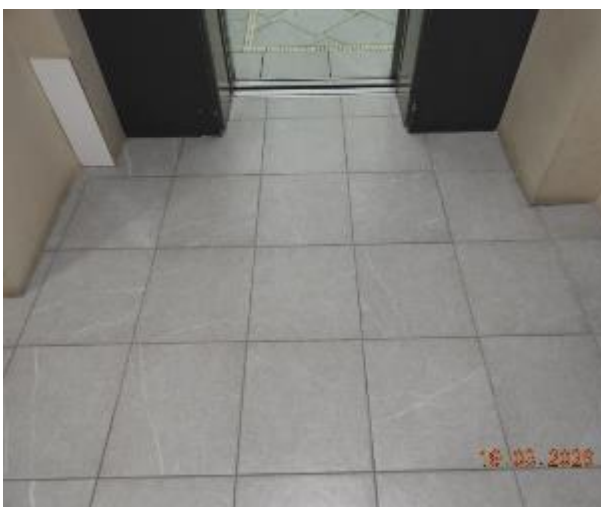
Figure 77 - General condition of level 3 common area floor tiles
