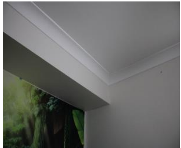
Figure 899 - General condition of bedroom 2 ceiling
