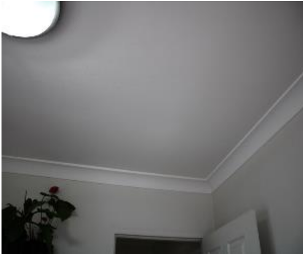
Figure 1074 - General condition of bedroom 2 ceiling
