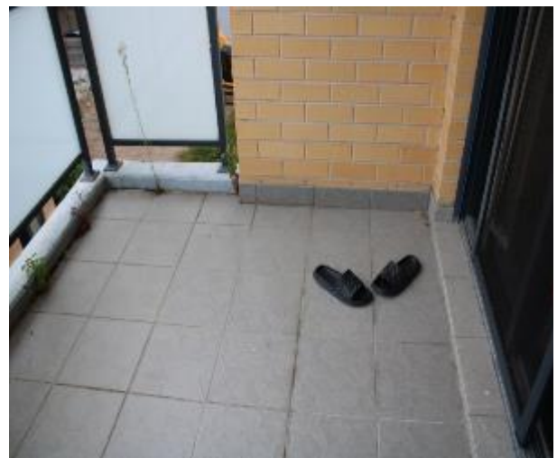
Figure 1498 - General condition of balcony floor tiles
