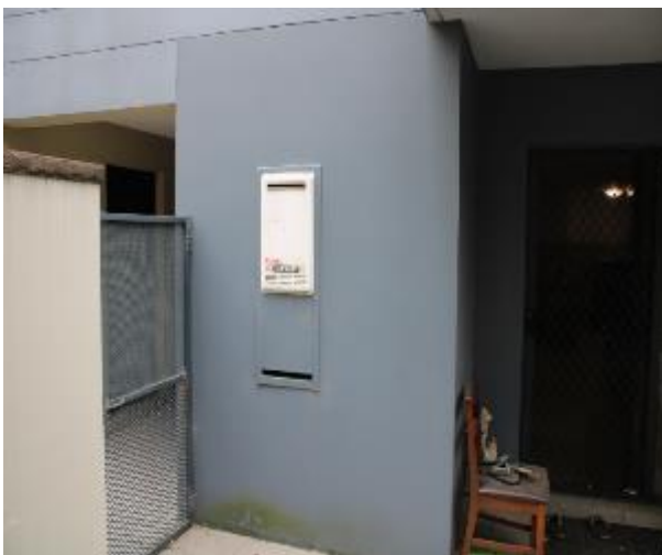
Figure 505 - General condition of external wall
