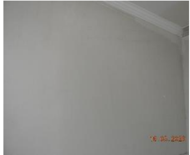
Figure 301 - General condition of level 5 fire stairs internal wall
