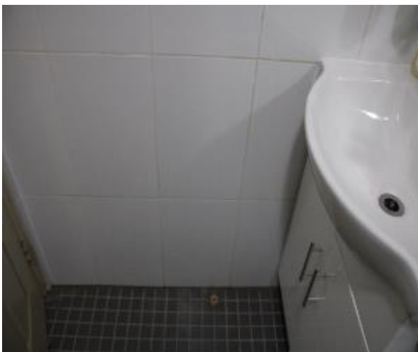
Figure 719 - General condition of ensuite bathroom internal wall
