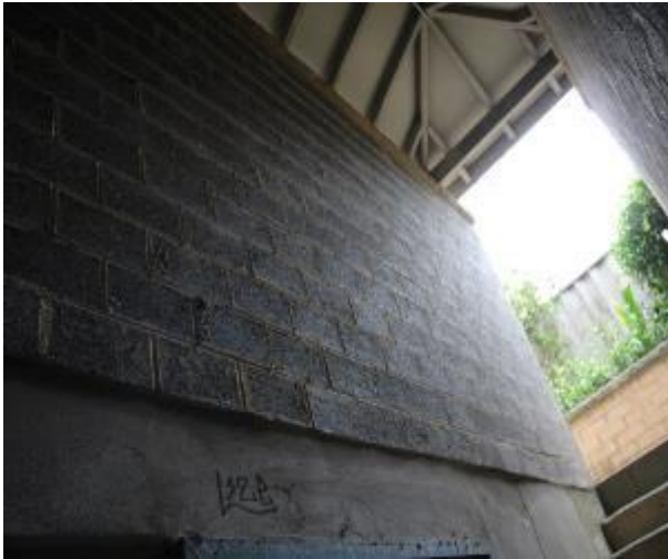
Figure 257 - General condition of level 1 fire stairs internal wall
