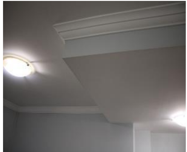
Figure 486 - General condition of open kitchen/ lounge room ceiling
