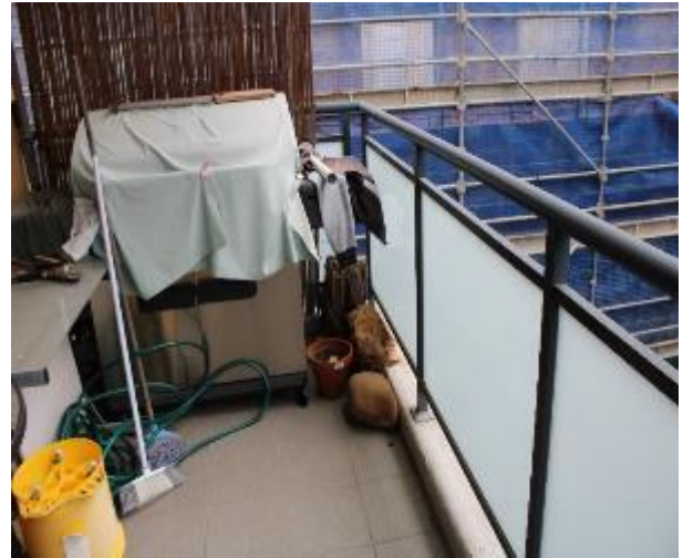
Figure 931 - General condition of balcony balustrade
