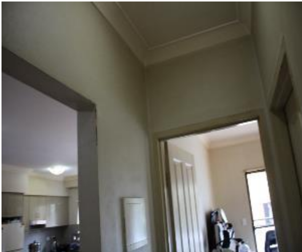
Figure 771 - General condition of corridor internal wall
