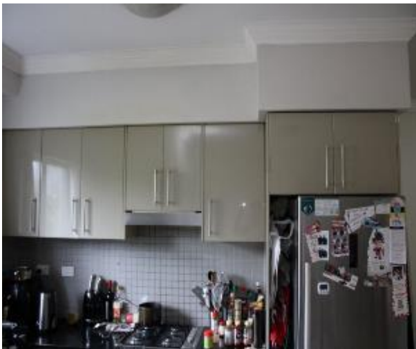
Figure 645 - General condition of kitchen internal wall
