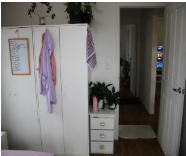
Figure 1064 - General condition of bedroom 2 internal wall
