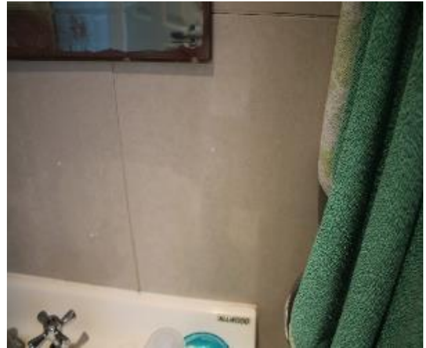
Figure 1021 - General condition of bathroom 1 internal wall
