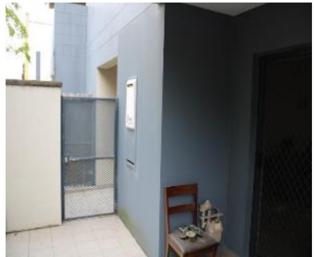
Figure 504 - General condition of external wall
