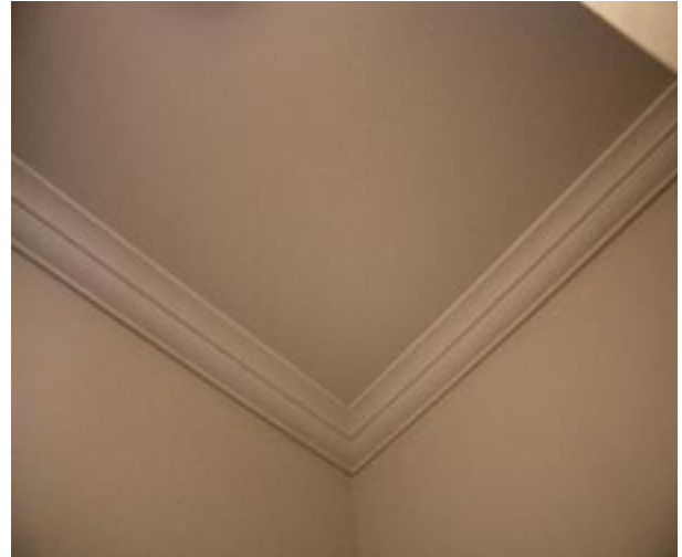
Figure 1496 - General condition of laundry ceiling
