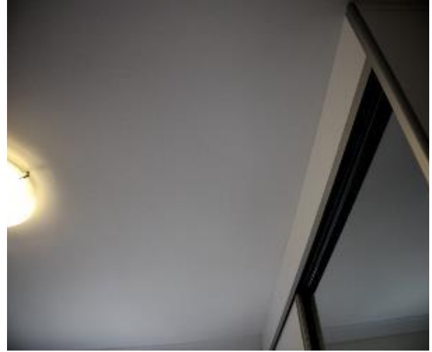
Figure 1242 - General condition of bedroom 2 ceiling
