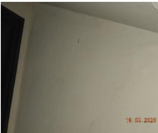
Figure 448 - General condition of basement fire stairs internal wall
