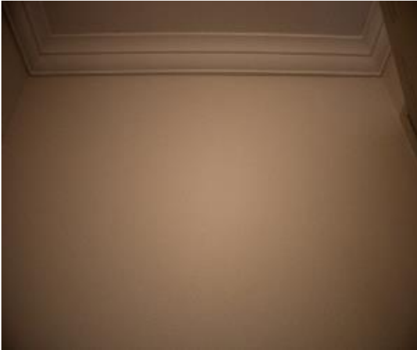
Figure 1495 - General condition of laundry internal wall
