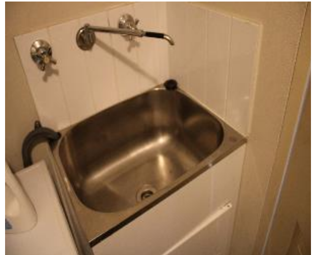
Figure 578 - General condition of laundry internal wall
