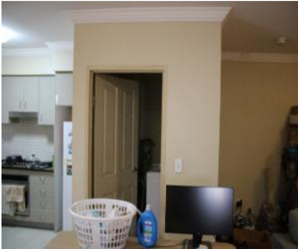
Figure 1280 - General condition of lounge room internal wall
