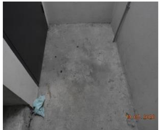
Figure 423 - General condition of level 1 fire stairs concrete floor
