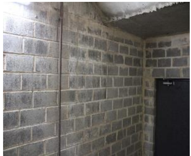
Figure 194 - General condition of B2 fire stairs internal wall
