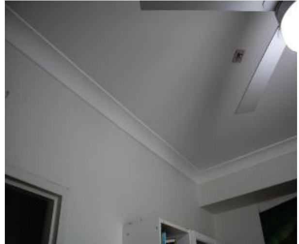
Figure 897 - General condition of bedroom 2 ceiling
