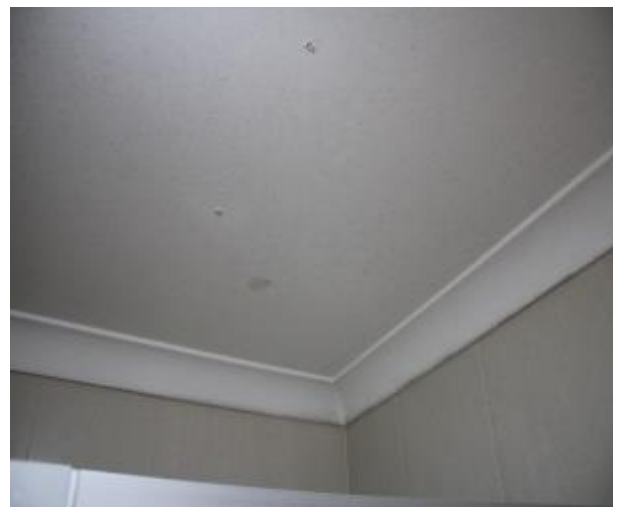
Figure 702 - General condition of bathroom 1 ceiling
