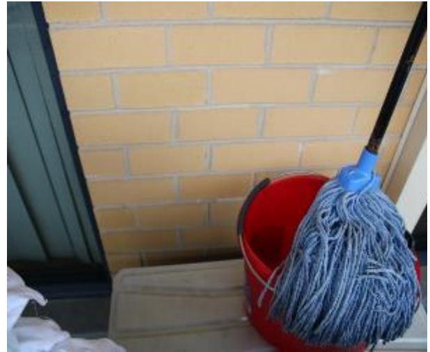
Figure 1260 - General condition of external wall
