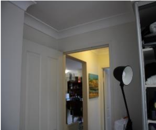
Figure 1193 - General condition of bedroom 1 internal wall
