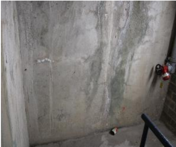
Figure 197 - General condition of B2 fire stairs internal wall
