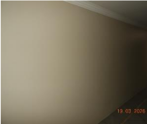
Figure 13 - General condition of level 1 common area internal wall
