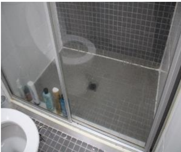
Figure 1207 - General condition of ensuite bathroom floor tiles
