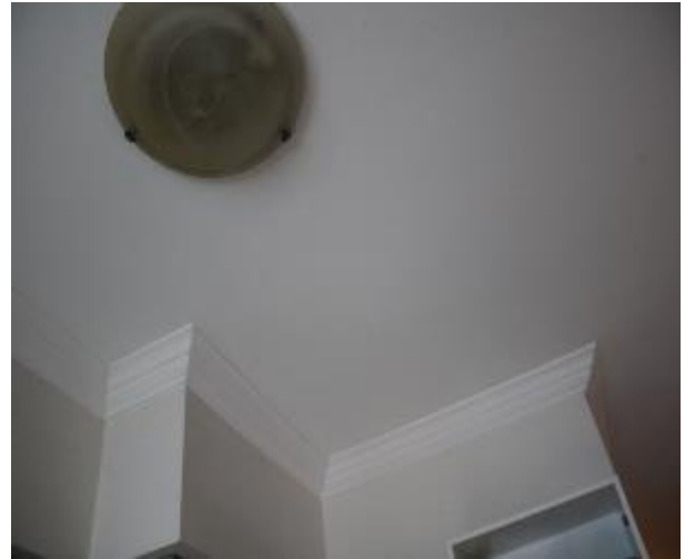
Figure 871 - General condition of kitchen ceiling
