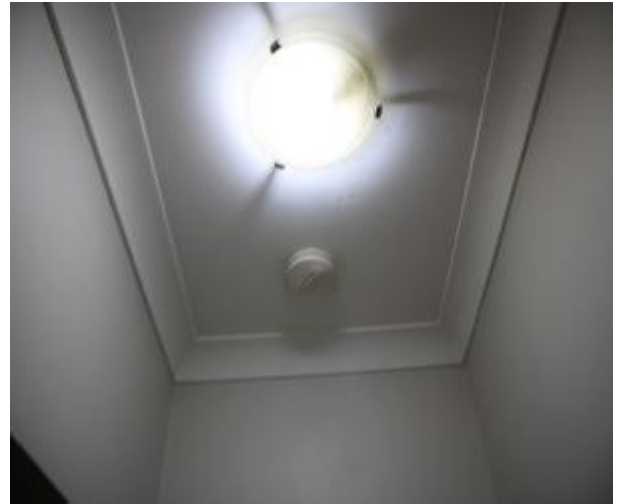
Figure 680 - General condition of corridor ceiling
