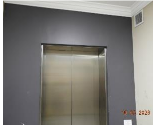
Figure 110 - General condition of level 3 common area internal wall
