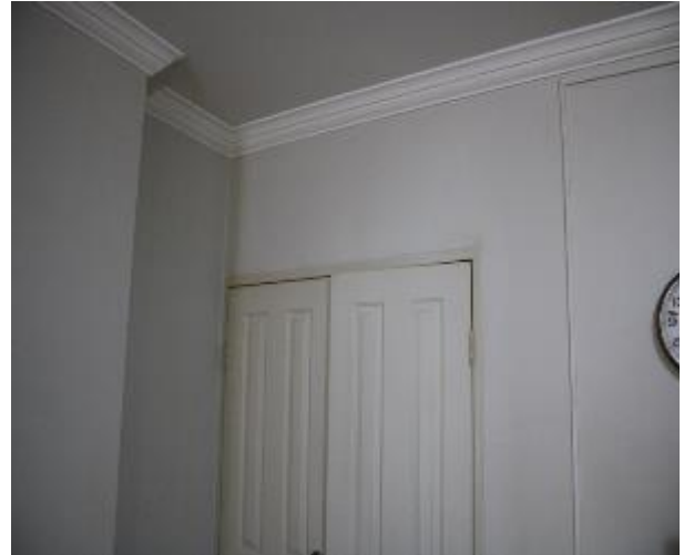
Figure 736 - General condition of open kitchen/ lounge room internal wall
