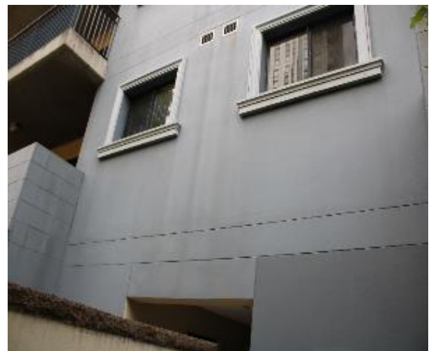
Figure 506 - General condition of external wall
