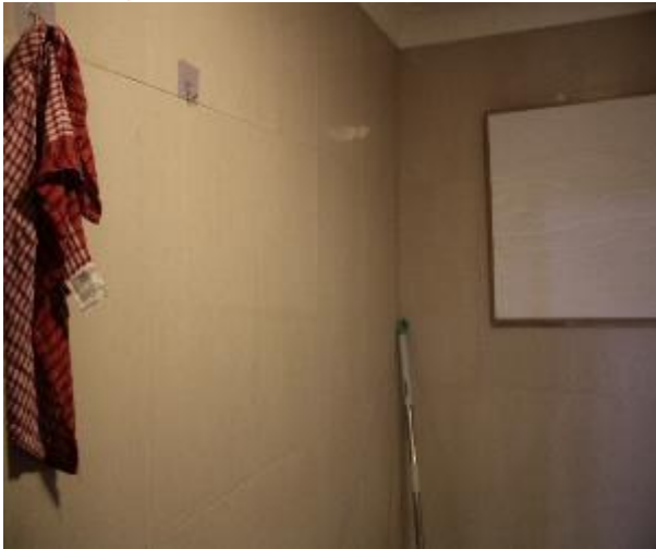
Figure 563 - General condition of bathroom 1 internal wall
