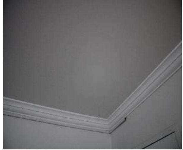
Figure 949 - General condition of lounge room ceiling
