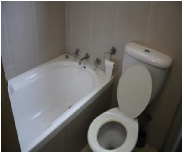
Figure 1346 - General condition of bathroom 1 internal wall
