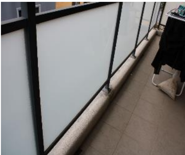
Figure 1438 - General condition of external wall
