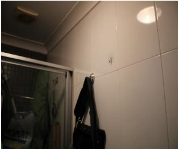
Figure 906 - General condition of ensuite bathroom internal wall
