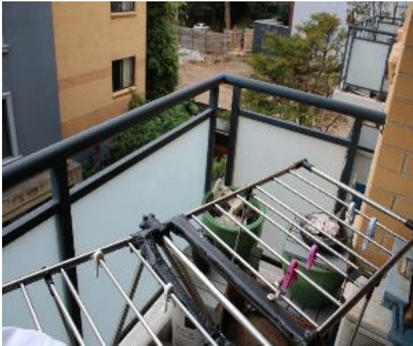
Figure 930 - General condition of balcony balustrade
