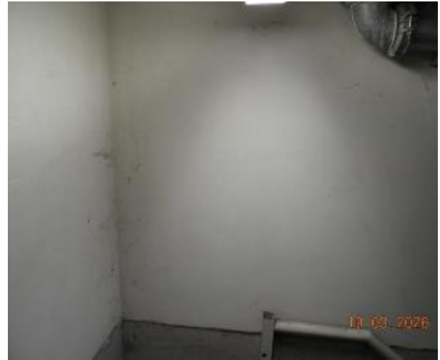
Figure 451 - General condition of basement fire stairs internal wall
