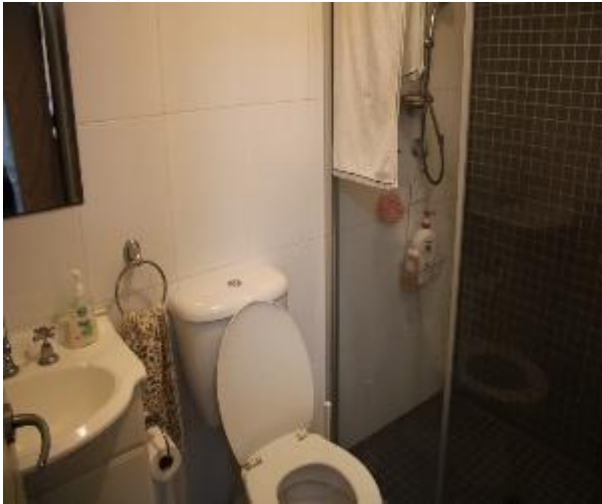
Figure 805 - General condition of ensuite bathroom internal wall
