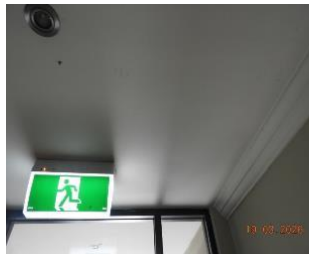
Figure 42 - General condition of level 1 common area ceiling
