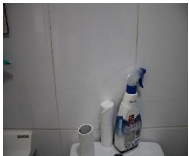
Figure 1210 - Crack propagation through ensuite bathroom internal wall
