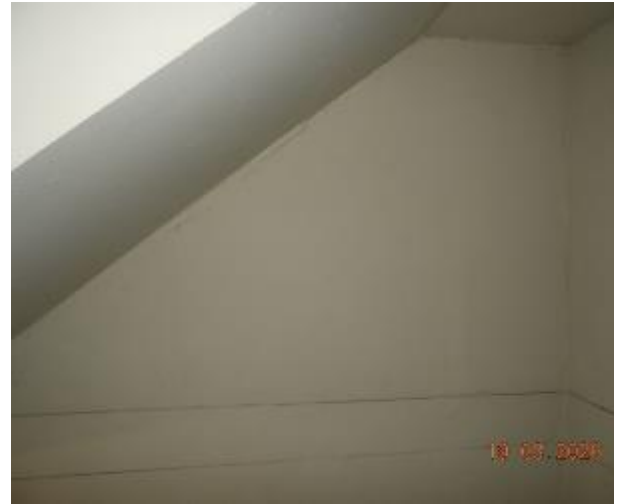
Figure 337 - General condition of level 3 fire stairs internal wall
