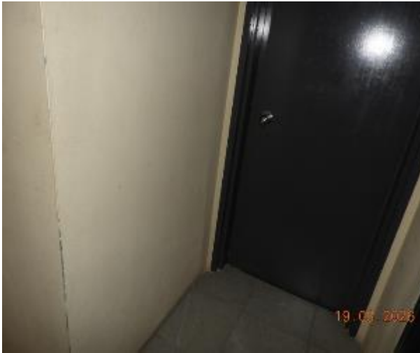
Figure 163 - General condition of level 5 common area internal wall
