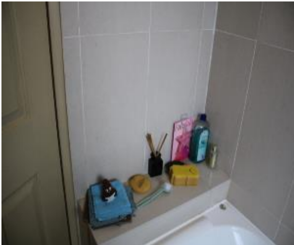
Figure 1354 - General condition of bathroom 1 internal wall
