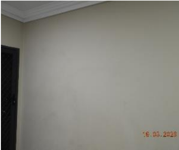
Figure 97 - General condition of level 3 common area internal wall
