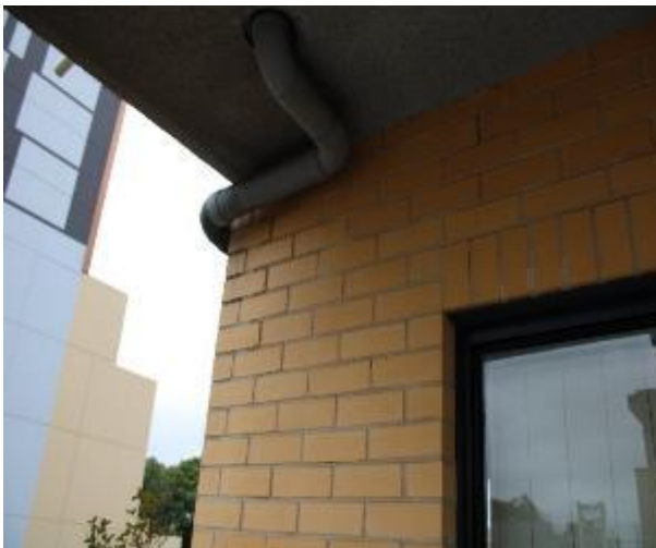
Figure 1257 - General condition of external wall
