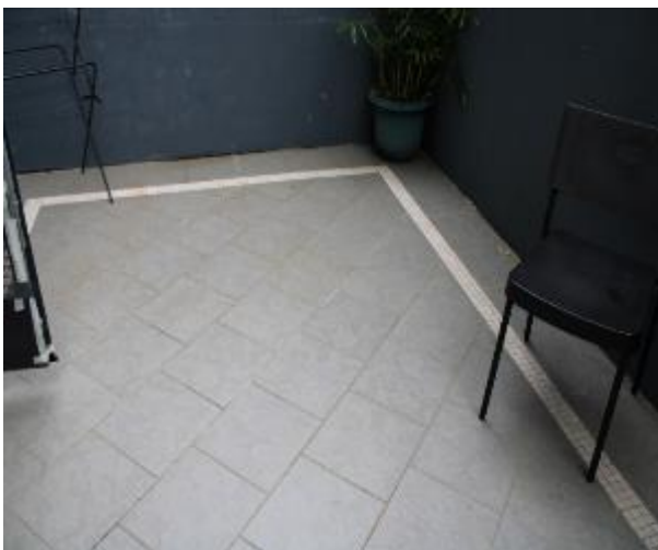
Figure 591 - General condition of courtyard floor tiles
