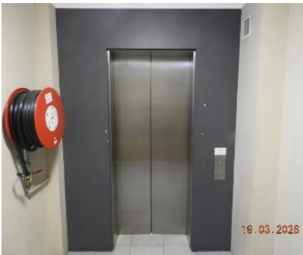
Figure 141 - General condition of level 4 common area internal wall
