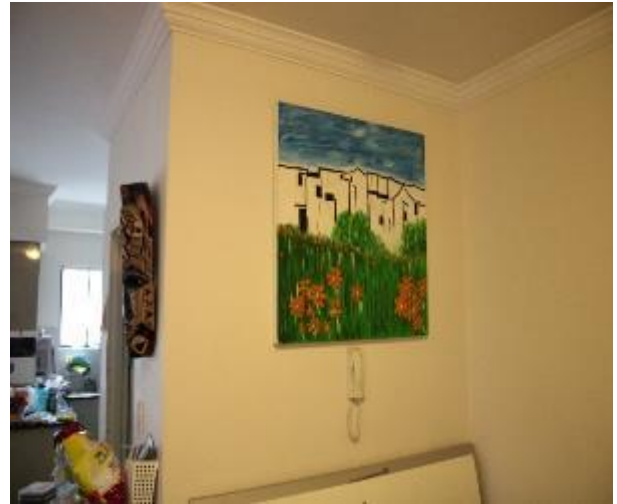
Figure 859 - General condition of bedroom 1 internal wall
