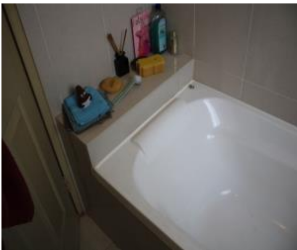
Figure 1350 - General condition of bathroom 1 internal wall
