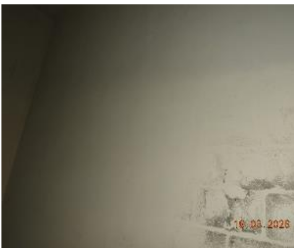
Figure 460 - General condition of basement fire stairs internal wall
