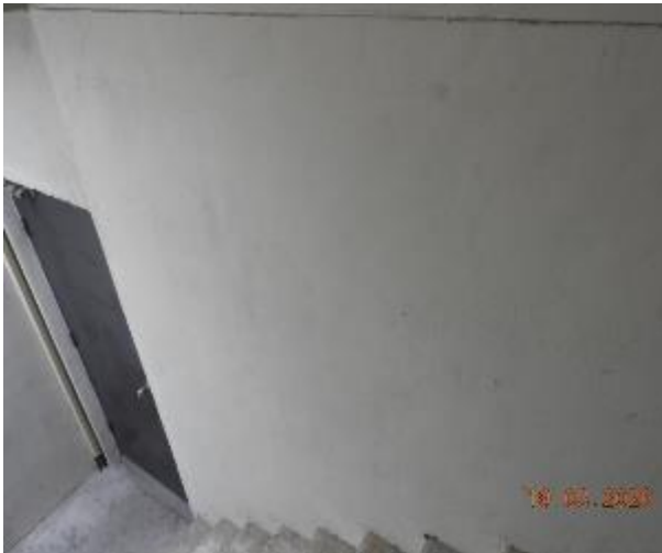
Figure 314 - General condition of level 4 fire stairs internal wall
