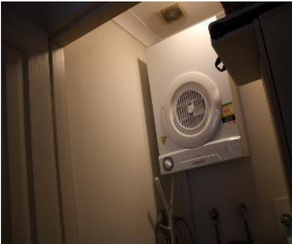
Figure 1135 - General condition of laundry internal wall
