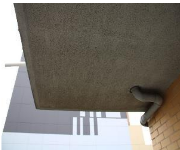
Figure 1267 - General condition of balcony underside slab
