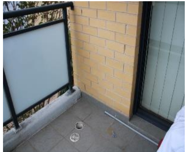
Figure 1256 - General condition of external wall
