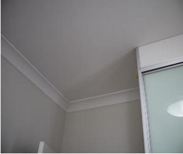
Figure 918 - General condition of bedroom 3 ceiling
