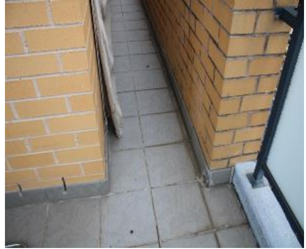
Figure 1506 - General condition of balcony floor tiles
