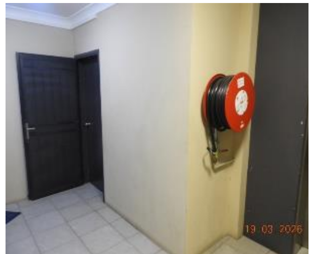
Figure 120 - General condition of level 4 common area internal wall
