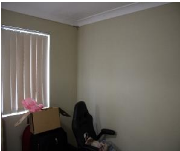
Figure 1378 - General condition of bedroom 1 internal wall
