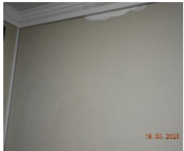
Figure 168 - General condition of level 5 common area internal wall
