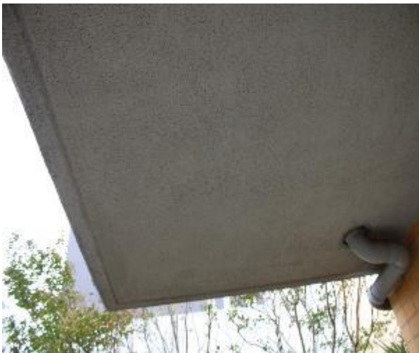
Figure 843 - General condition of balcony underside slab
