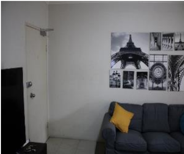
Figure 759 - General condition of open kitchen/ lounge room internal wall
