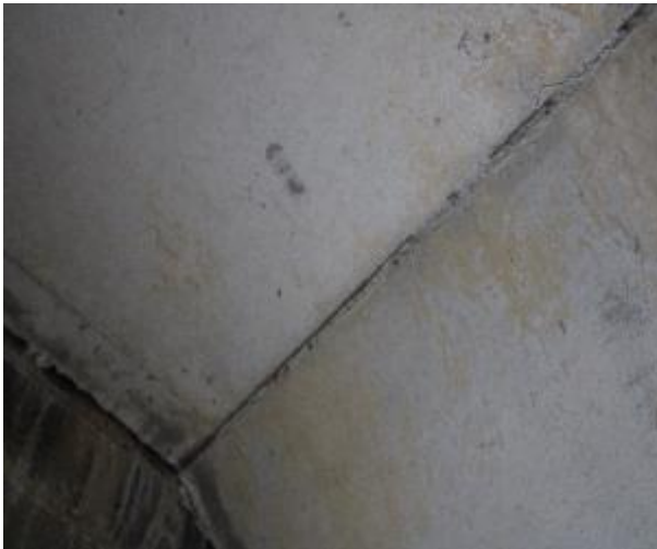
Figure 211 - General condition of B2 fire stairs underside stairs
