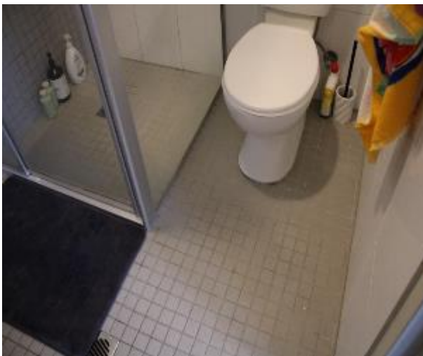
Figure 1621 - General condition of ensuite bathroom floor tiles
