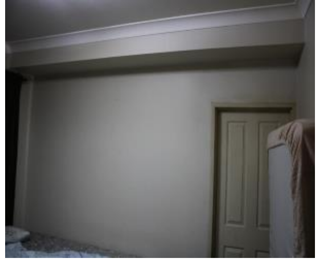
Figure 788 - General condition of bedroom 1 internal wall
