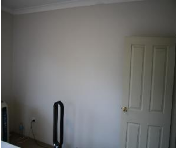
Figure 687 - General condition of bedroom 1 internal wall
