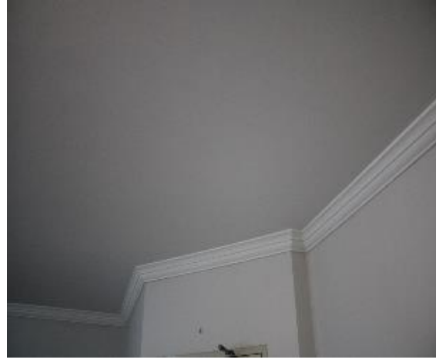
Figure 638 - General condition of lounge room ceiling
