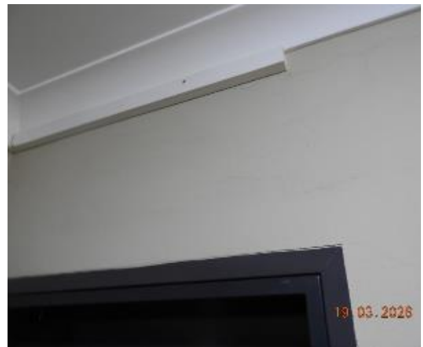
Figure 124 - General condition of level 4 common area internal wall
