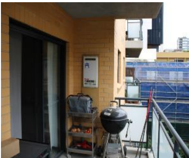
Figure 833 - General condition of external wall
