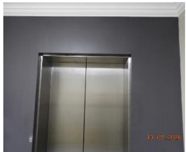
Figure 180 - General condition of level 5 common area internal wall
