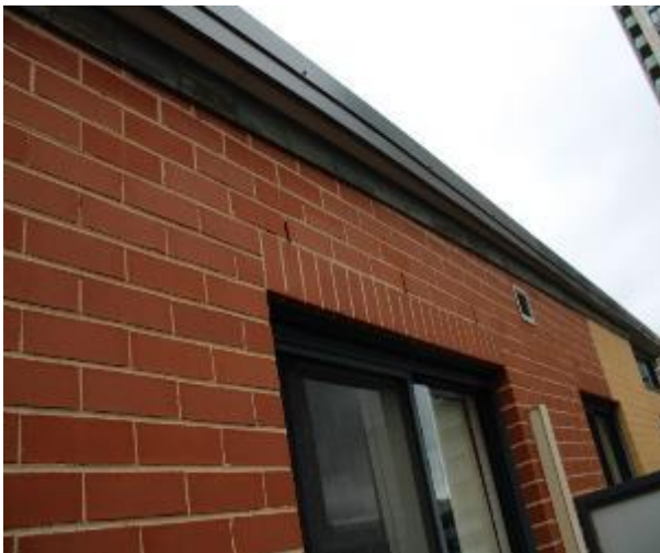
Figure 1515 - General condition of external wall
