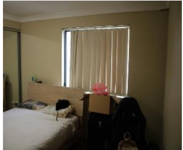
Figure 1365 - General condition of bedroom 1 internal wall
