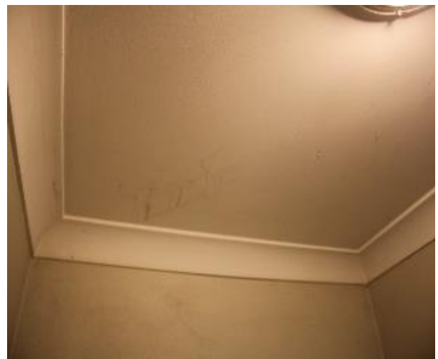
Figure 586 - General condition of laundry ceiling
