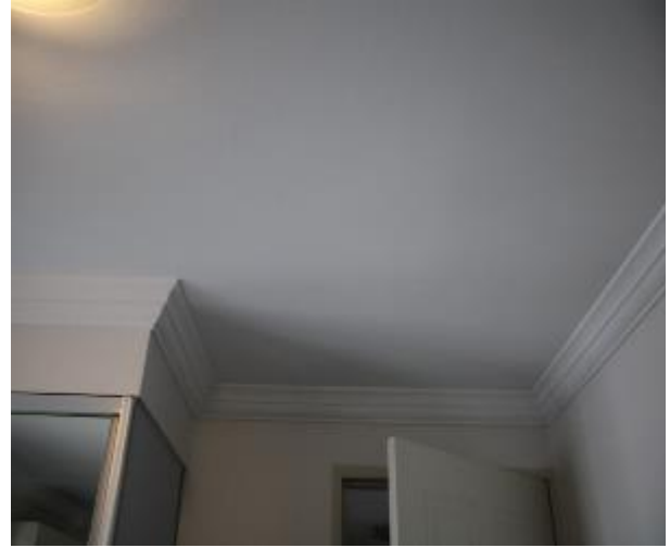
Figure 1614 - General condition of bedroom 3 ceiling
