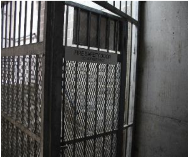
Figure 239 - General condition of level 1 fire stairs
