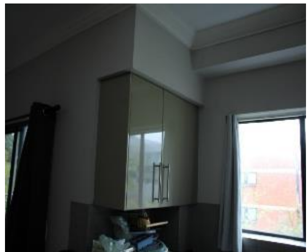
Figure 648 - General condition of kitchen internal wall
