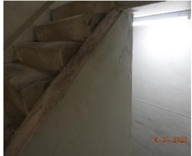
Figure 397 - General condition of level 1 fire stairs internal wall
