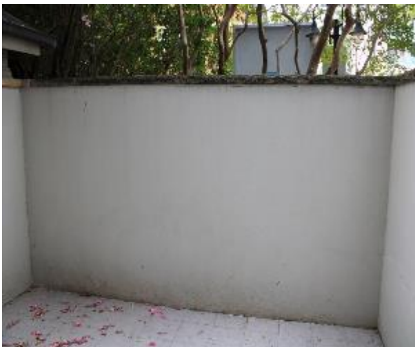
Figure 515 - General condition of courtyard external wall
