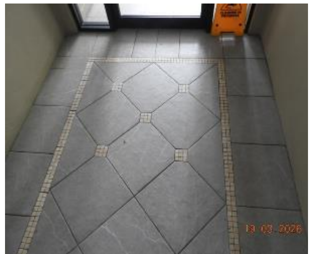
Figure 6 - General condition of level 1 common area floor tiles
