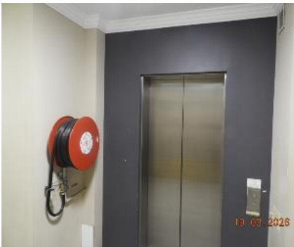
Figure 105 - General condition of level 3 common area internal wall
