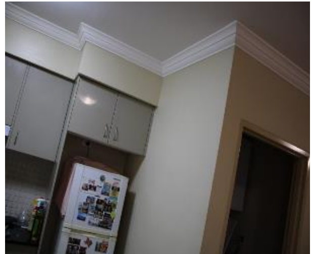
Figure 1307 - General condition of kitchen internal wall
