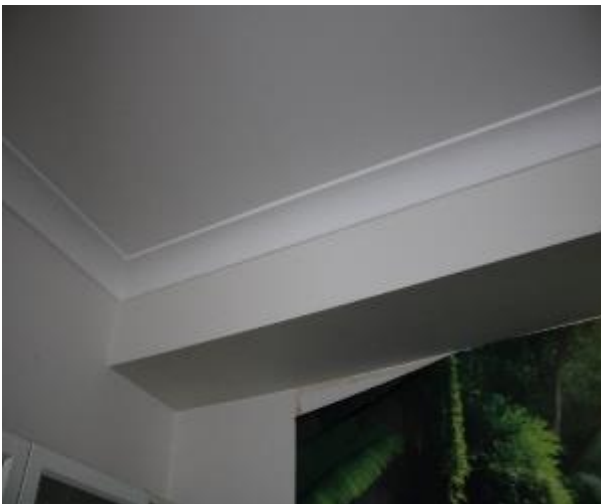
Figure 898 - General condition of bedroom 2 ceiling
