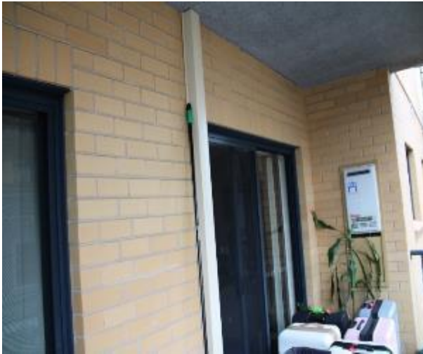
Figure 1259 - General condition of external wall
