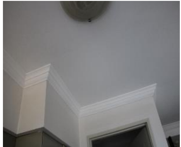
Figure 1472 - General condition of open kitchen/ lounge room ceiling
