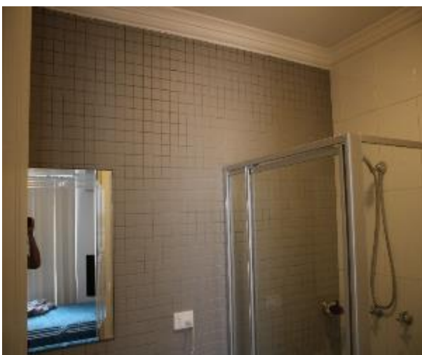
Figure 1629 - General condition of ensuite bathroom internal wall
