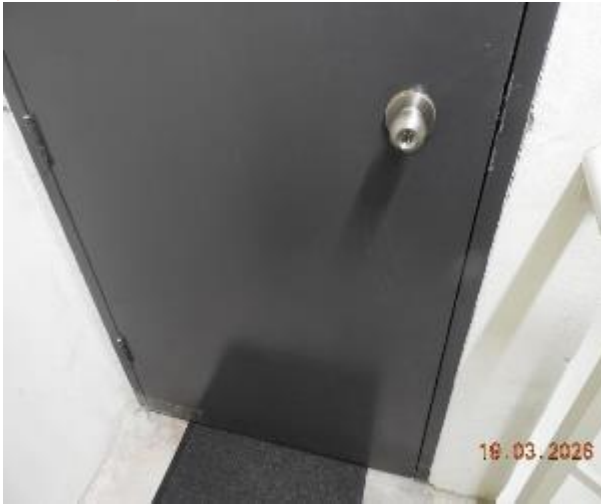
Figure 282 - General condition of level 5 fire stairs internal wall
