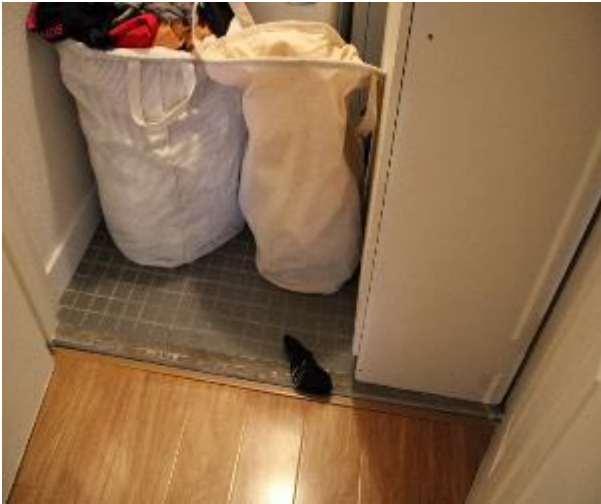
Figure 1133 - General condition of laundry floor tiles
