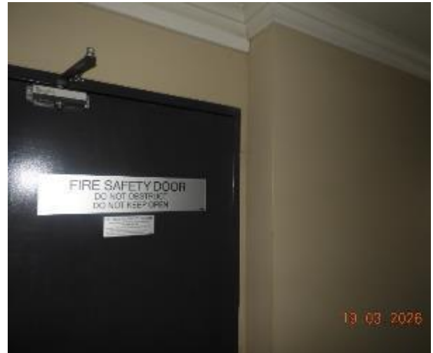
Figure 22 - General condition of level 1 common area internal wall
