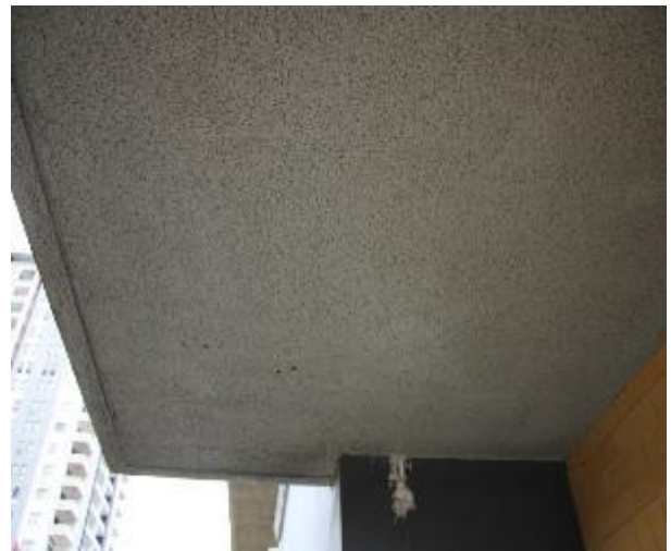
Figure 664 - General condition of balcony underside slab
