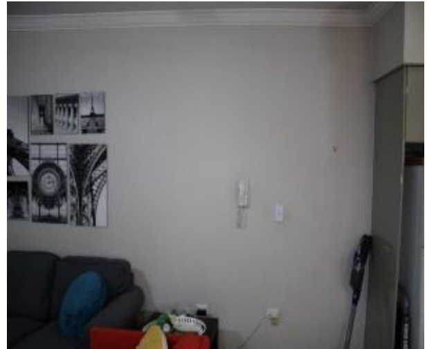
Figure 758 - General condition of open kitchen/ lounge room internal wall
