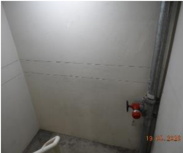
Figure 368 - General condition of level 2 fire stairs internal wall
