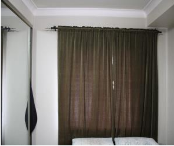
Figure 793 - General condition of bedroom 1 internal wall
