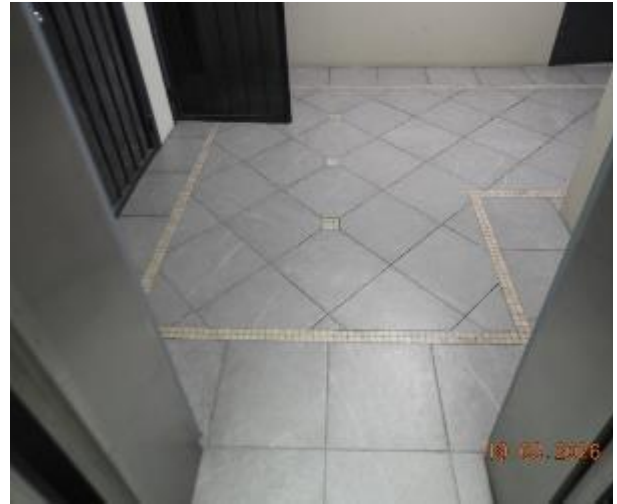
Figure 2 - General condition of level 1 common area floor tiles
