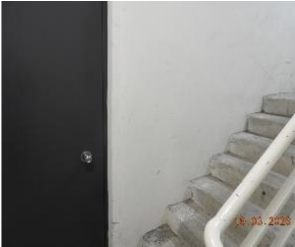
Figure 384 - General condition of level 2 fire stairs internal wall
