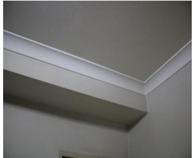
Figure 800 - General condition of bedroom 1 ceiling
