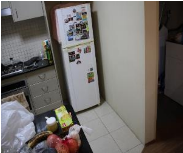
Figure 1306 - General condition of kitchen internal wall
