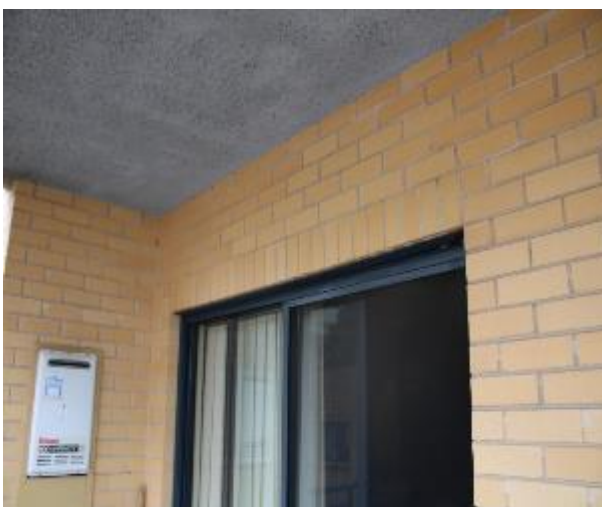
Figure 1440 - General condition of external wall
