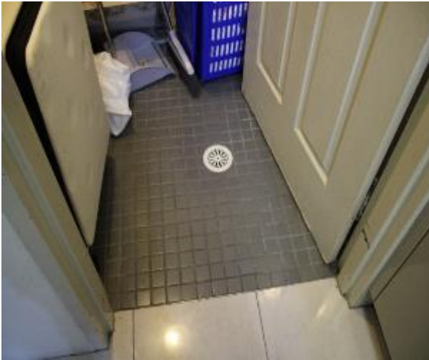
Figure 569 - General condition of laundry floor tiles
