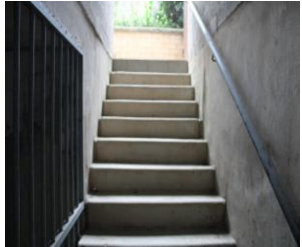
Figure 246 - General condition of level 1 fire stairs
