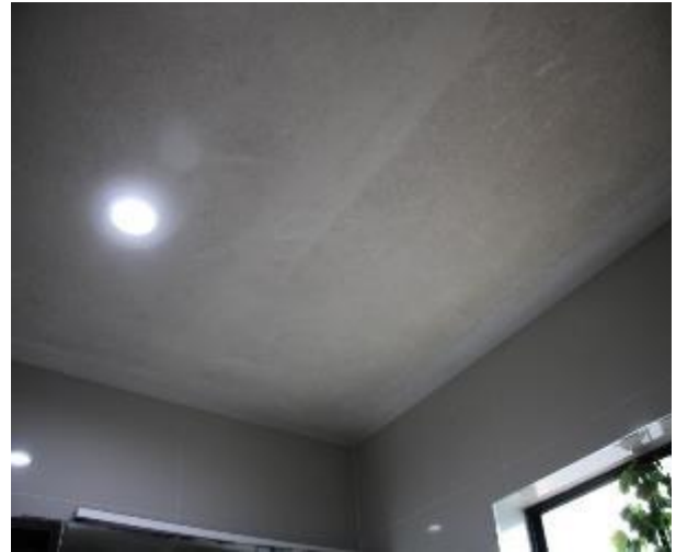
Figure 889 - General condition of bathroom 1 ceiling
