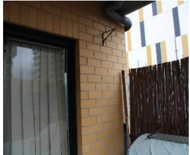
Figure 925 - General condition of external wall
