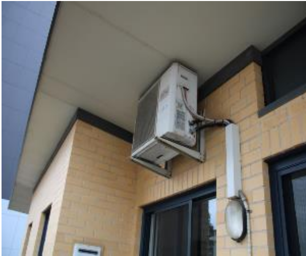
Figure 1529 - General condition of external wall
