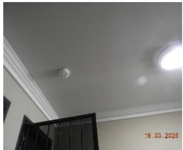
Figure 36 - General condition of level 1 common area ceiling
