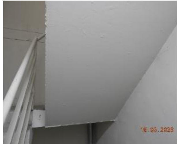
Figure 325 - General condition of level 4 fire stairs underside stairs
