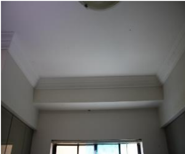
Figure 872 - General condition of kitchen ceiling
