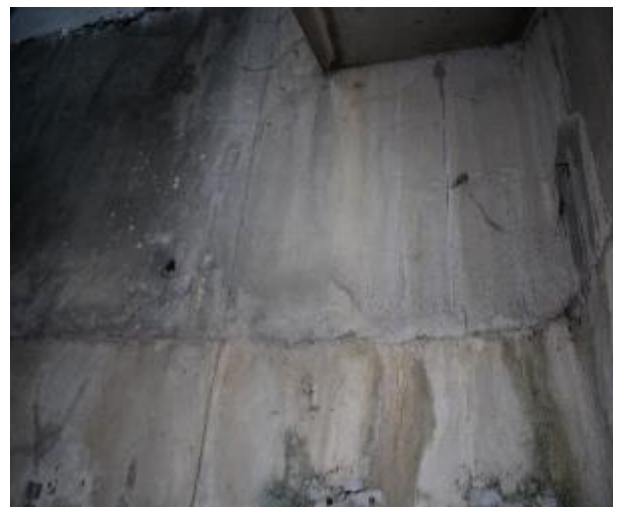
Figure 202 - General condition of B2 fire stairs internal wall
