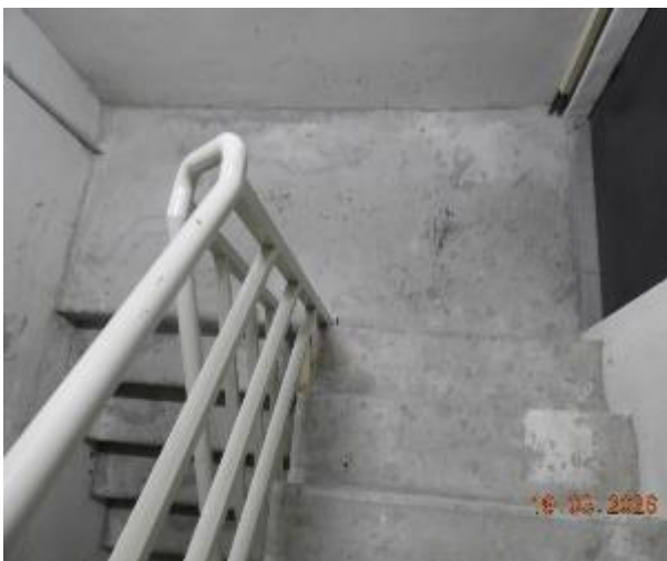
Figure 316 - General condition of level 4 fire stairs concrete floor
