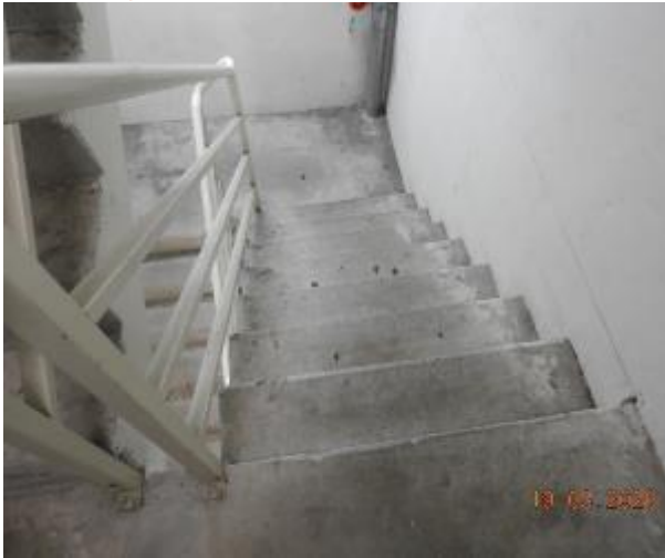
Figure 360 - General condition of level 2 fire stairs
