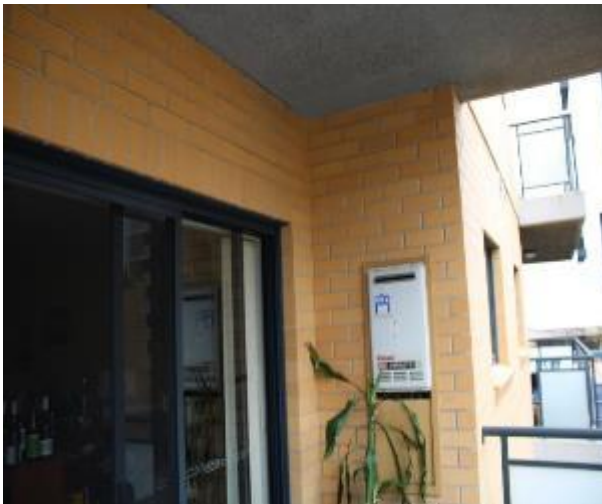
Figure 1261 - General condition of external wall
