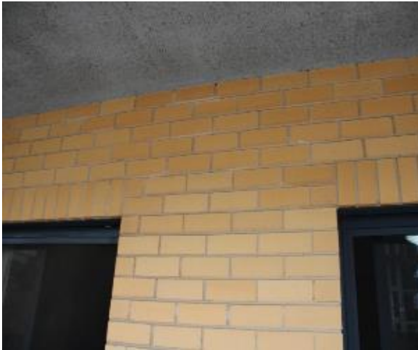
Figure 1442 - General condition of external wall
