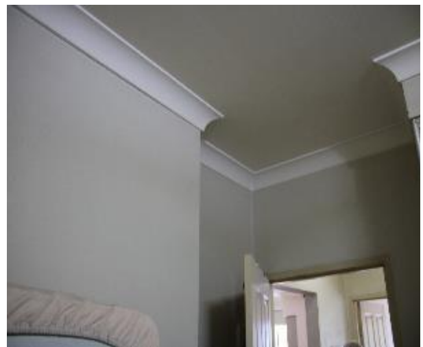
Figure 798 - General condition of bedroom 1 internal wall
