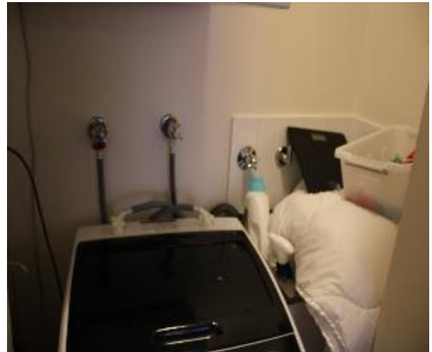
Figure 1136 - General condition of laundry internal wall
