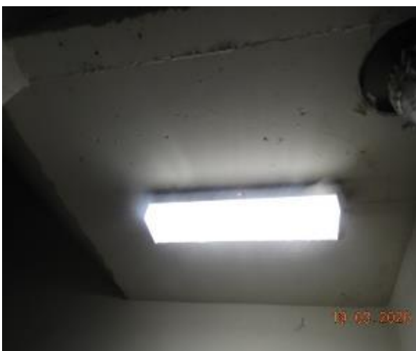
Figure 466 - General condition of basement fire stairs underside slab
