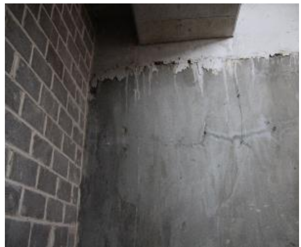
Figure 220 - General condition of B1 fire stairs internal wall
