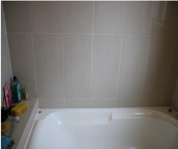
Figure 1352 - General condition of bathroom 1 internal wall
