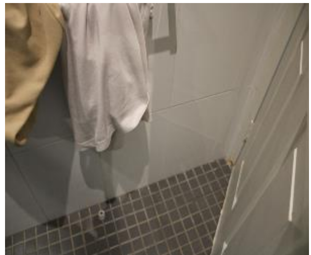
Figure 1047 - General condition of ensuite bathroom internal wall
