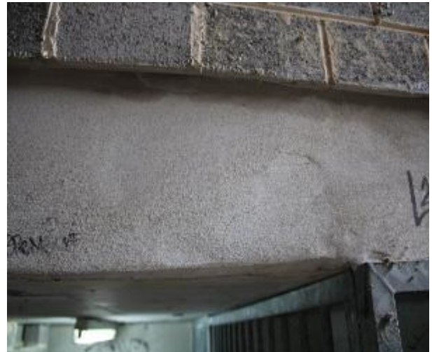
Figure 272 - Crack propagation through fire stairs underside slab
