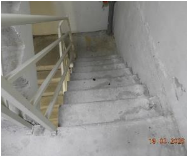
Figure 326 - General condition of level 3 fire stairs
