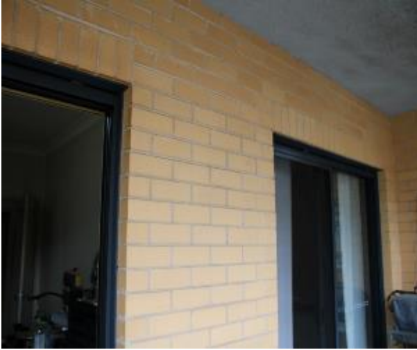
Figure 835 - General condition of external wall
