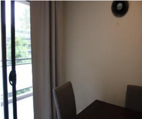
Figure 739 - General condition of open kitchen/ lounge room internal wall
