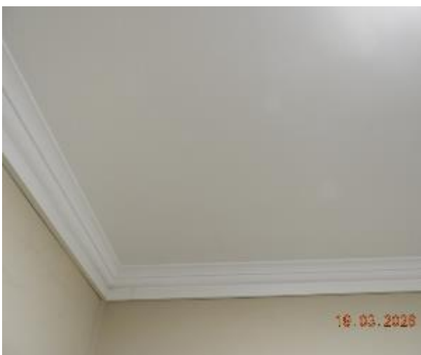
Figure 113 - General condition of level 3 common area ceiling
