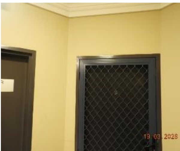
Figure 89 - General condition of level 3 common area internal wall
