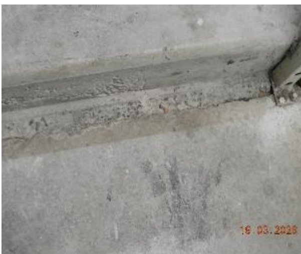
Figure 382 - General condition of level 2 fire stairs
