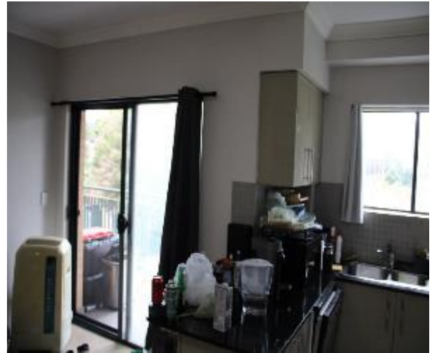
Figure 632 - General condition of lounge room internal wall
