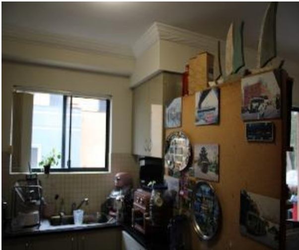
Figure 1123 - General condition of kitchen internal wall
