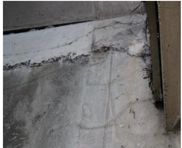
Figure 206 - General condition of B2 fire stairs internal wall
