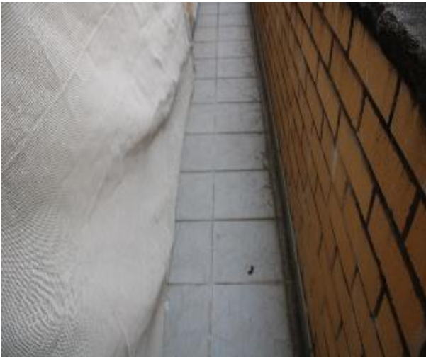
Figure 1507 - General condition of balcony floor tiles
