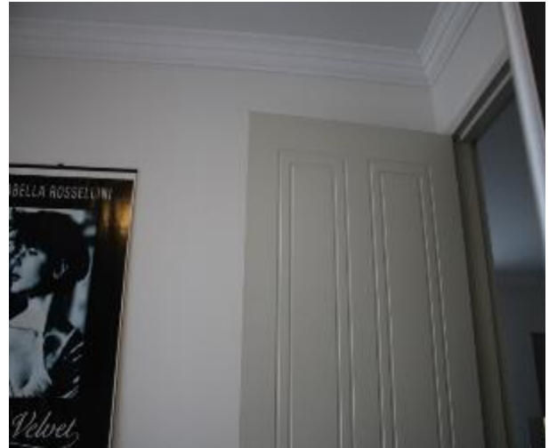
Figure 1566 - General condition of bedroom 2 internal wall
