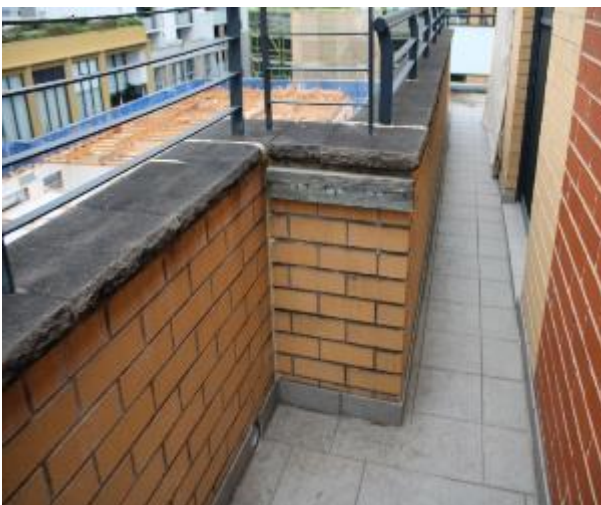
Figure 1545 - General condition of balcony balustrade
