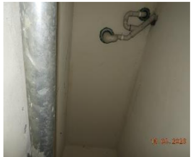
Figure 465 - General condition of basement fire stairs underside slab
