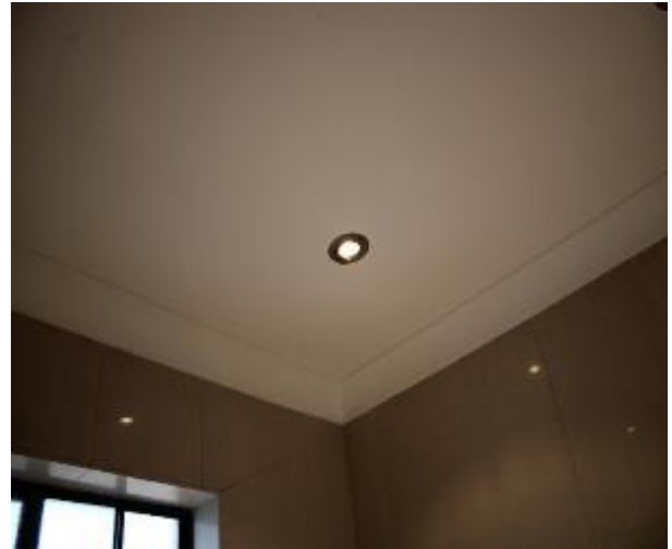
Figure 1027 - General condition of bathroom 1 ceiling
