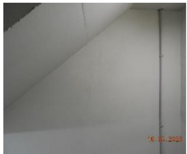
Figure 353 - General condition of level 3 fire stairs internal wall
