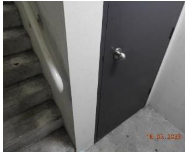
Figure 435 - General condition of level 1 fire stairs internal wall
