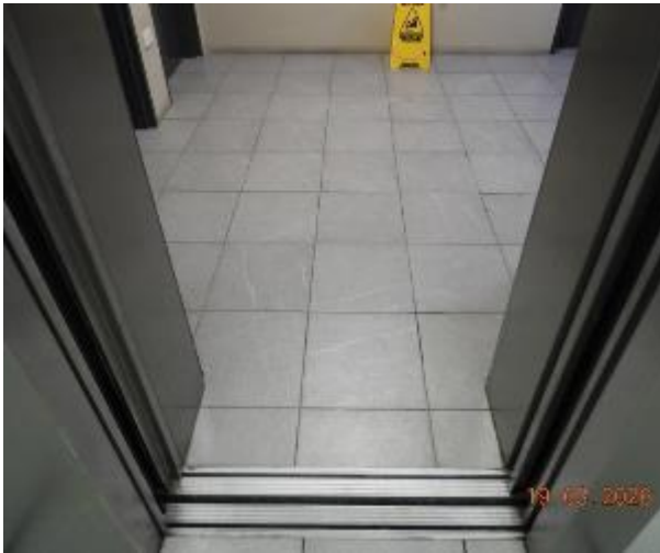
Figure 117 - General condition of level 4 common area floor tiles
