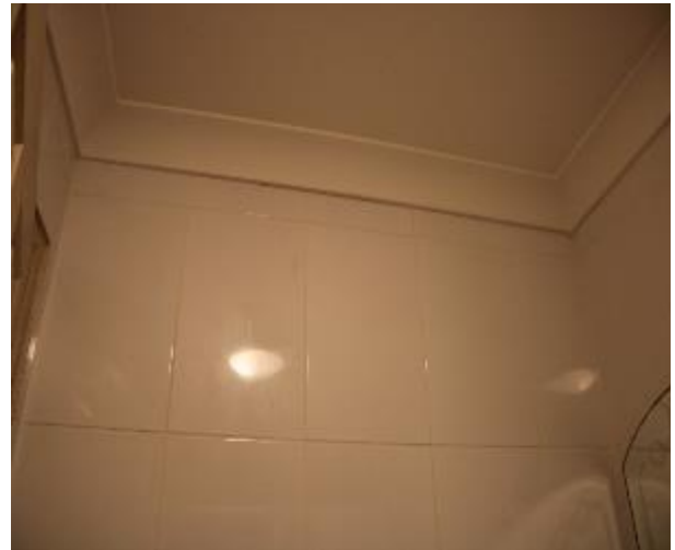
Figure 808 - General condition of ensuite bathroom internal wall
