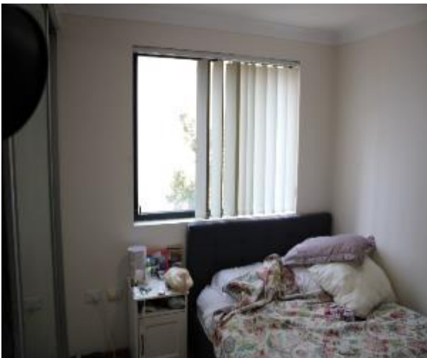
Figure 1185 - General condition of bedroom 1 internal wall
