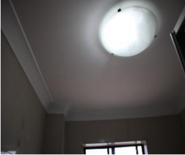
Figure 1181 - General condition of bathroom 1 ceiling
