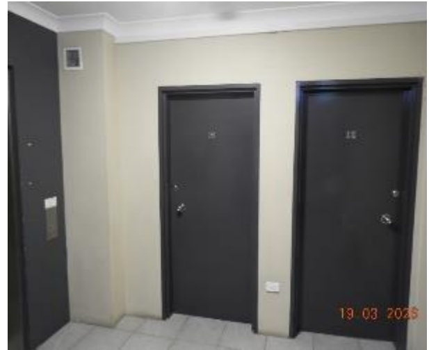
Figure 140 - General condition of level 4 common area internal wall
