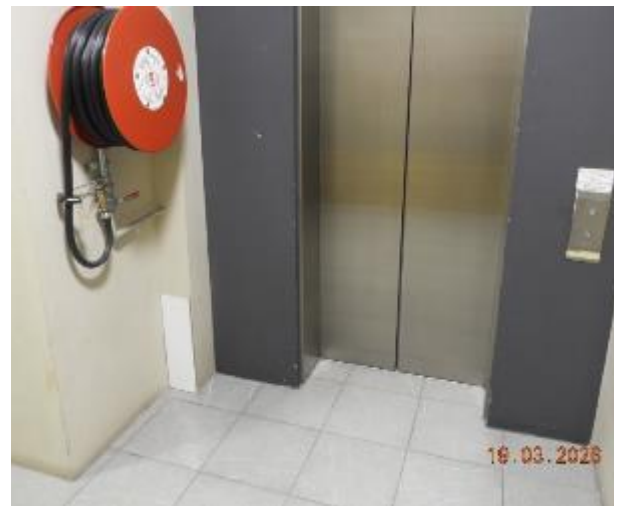
Figure 106 - General condition of level 3 common area internal wall
