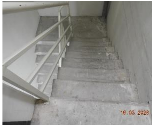
Figure 291 - General condition of level 5 fire stairs
