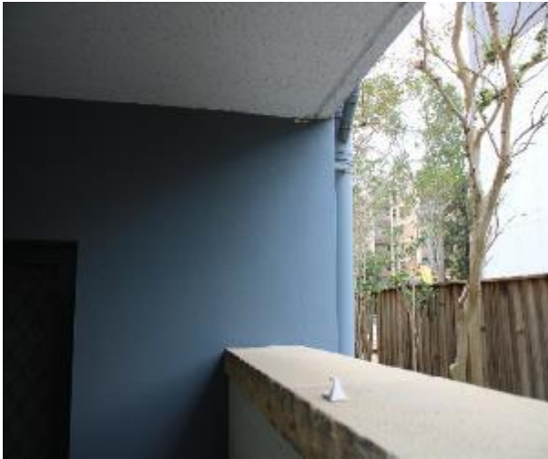
Figure 501 - General condition of external wall
