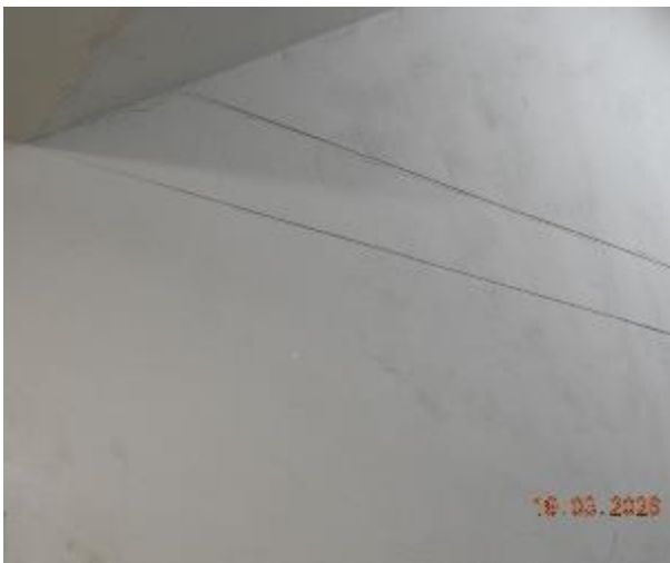
Figure 386 - General condition of level 2 fire stairs internal wall
