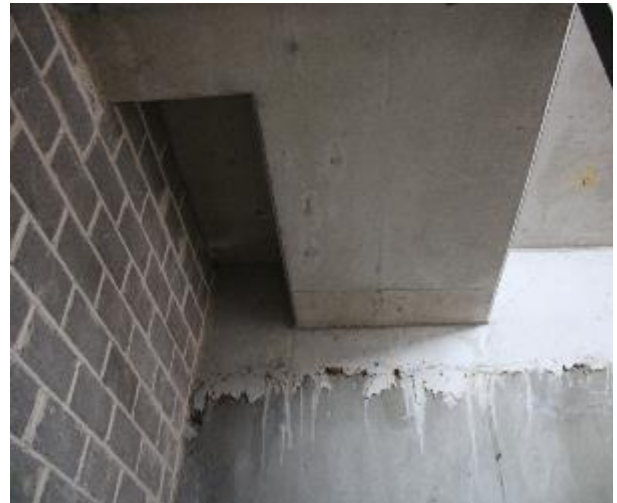
Figure 236 - General condition of B1 fire stairs underside slab
