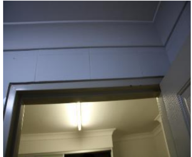
Figure 722 - General condition of ensuite bathroom internal wall
