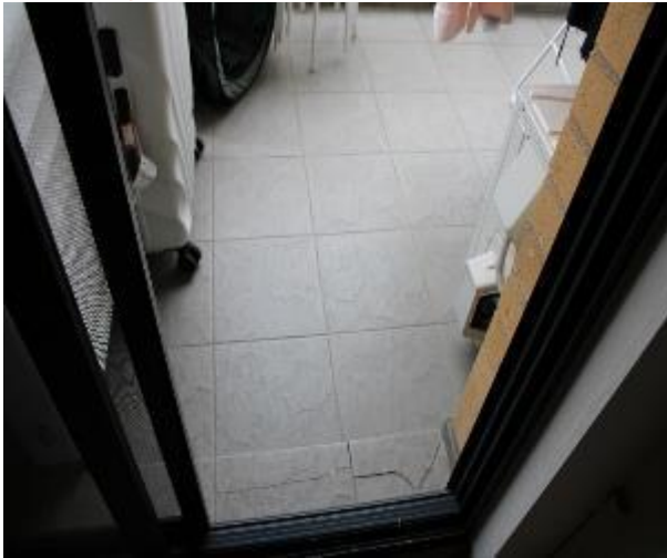
Figure 1247 - General condition of balcony floor tiles
