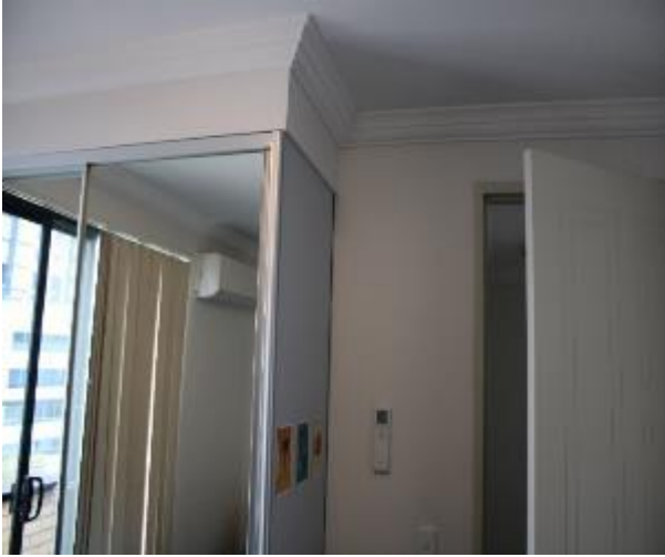
Figure 1613 - General condition of bedroom 3 internal wall
