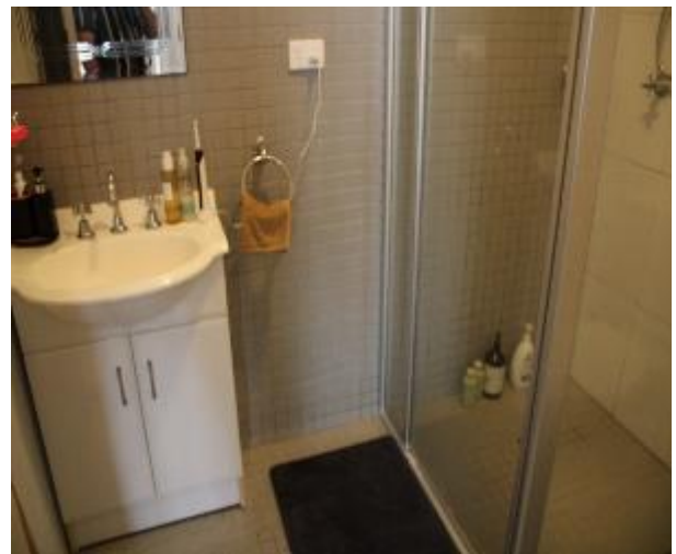
Figure 1628 - General condition of ensuite bathroom internal wall
