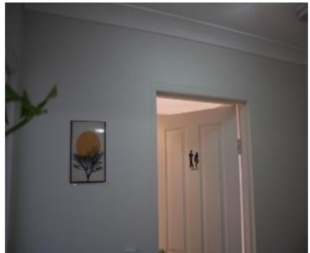
Figure 983 - General condition of corridor internal wall
