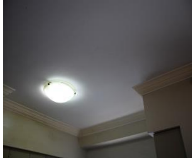
Figure 766 - General condition of open kitchen/ lounge room ceiling
