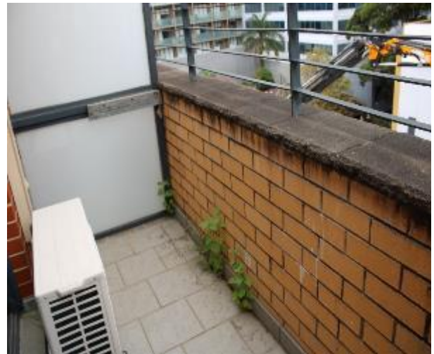
Figure 1544 - General condition of balcony balustrade
