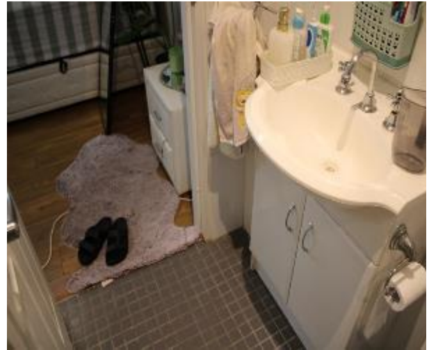
Figure 1051 - General condition of ensuite bathroom internal wall
