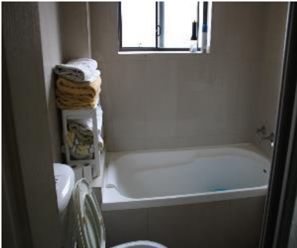
Figure 777 - General condition of bathroom 1 internal wall
