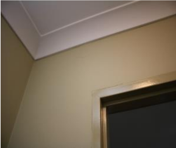
Figure 1324 - General condition of laundry internal wall
