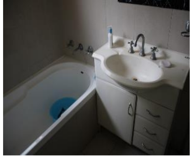
Figure 782 - General condition of bathroom 1 internal wall
