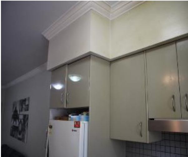
Figure 757 - General condition of open kitchen/ lounge room internal wall
