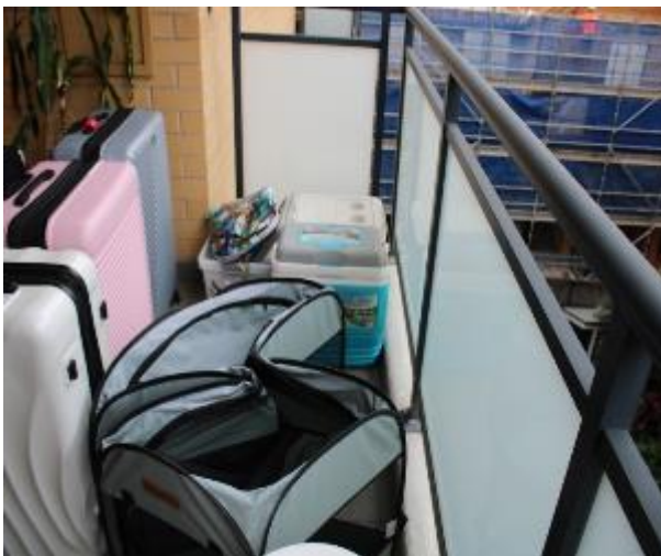
Figure 1249 - General condition of balcony floor tiles
