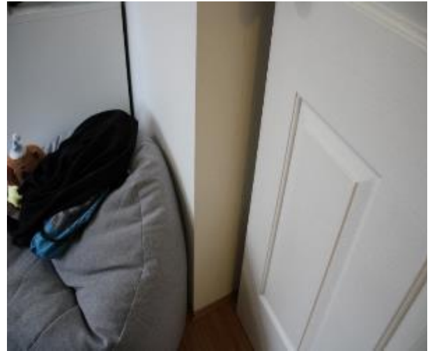
Figure 1194 - General condition of bedroom 1 internal wall
