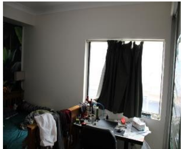
Figure 891 - General condition of bedroom 2 internal wall
