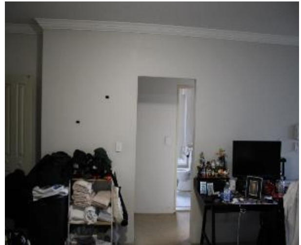
Figure 634 - General condition of lounge room internal wall
