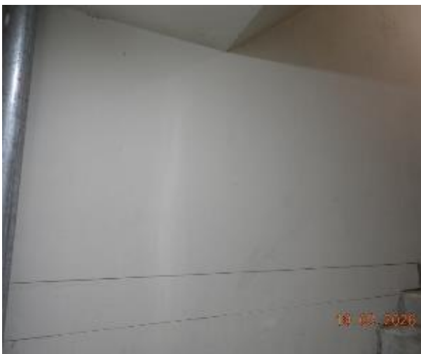
Figure 364 - General condition of level 2 fire stairs internal wall
