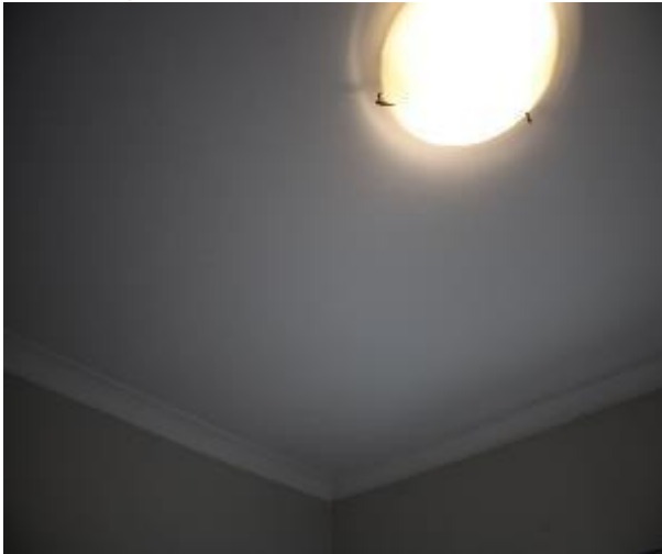
Figure 691 - General condition of bedroom 1 ceiling
