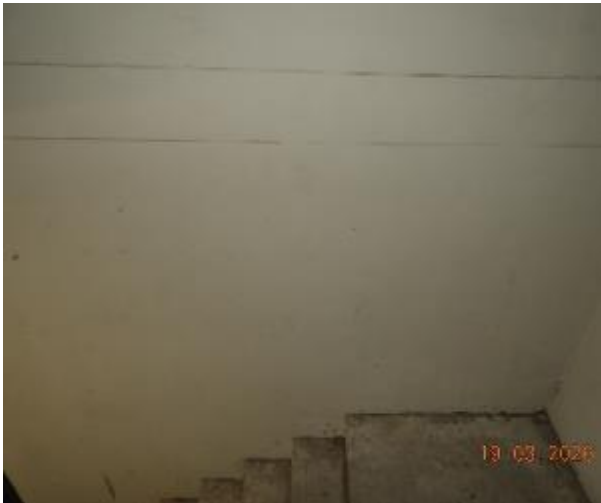
Figure 338 - General condition of level 3 fire stairs internal wall
