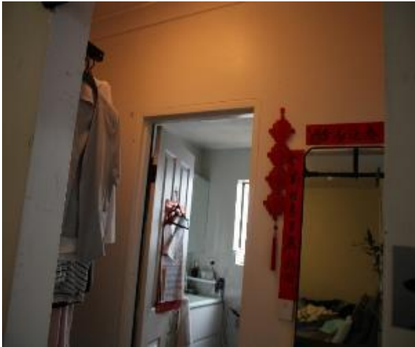
Figure 876 - General condition of corridor internal wall
