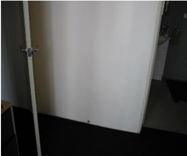
Figure 1607 - General condition of bedroom 3 internal wall
