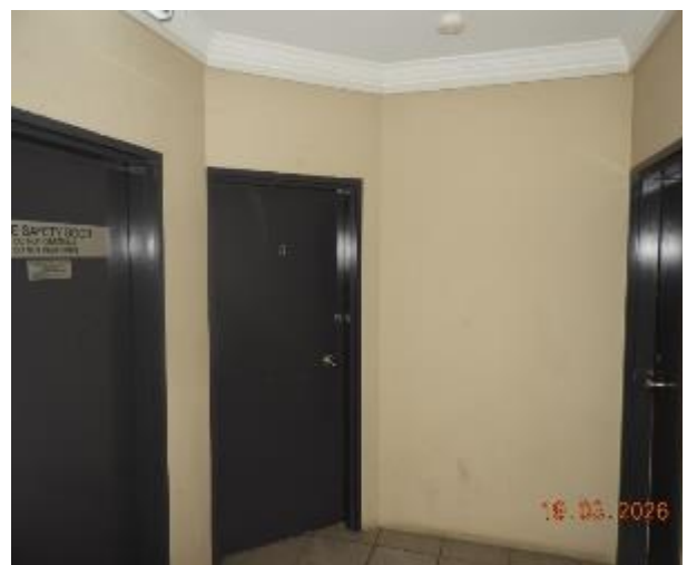
Figure 54 - General condition of level 2 common area internal wall
