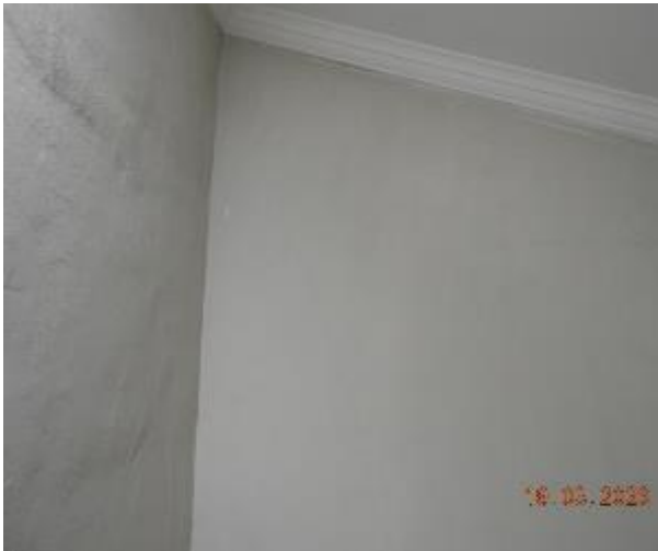
Figure 302 - General condition of level 5 fire stairs internal wall
