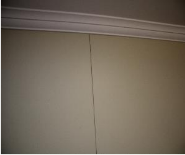
Figure 1274 - General condition of lounge room internal wall
