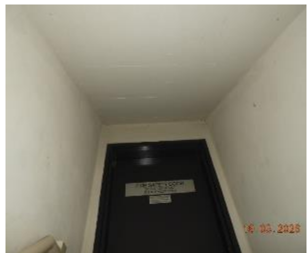
Figure 467 - General condition of basement fire stairs underside slab
