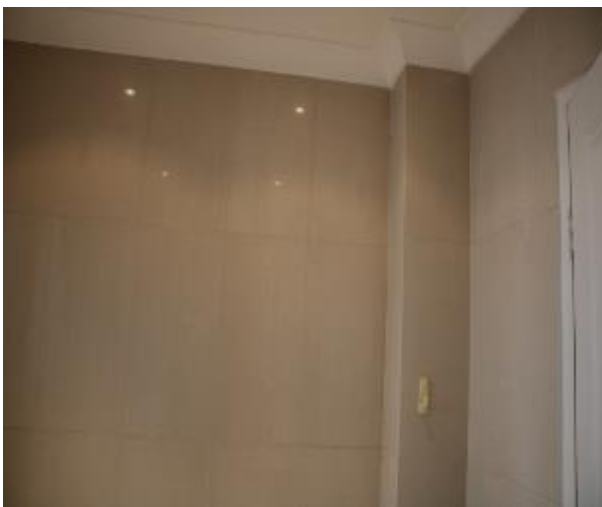
Figure 1012 - General condition of bathroom 1 internal wall
