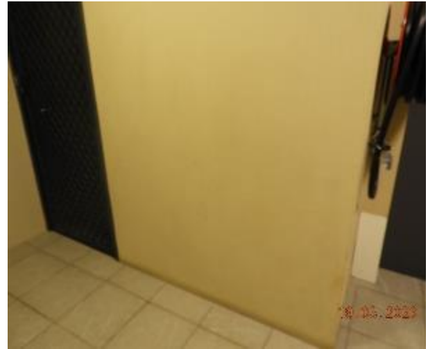
Figure 80 - General condition of level 3 common area internal wall
