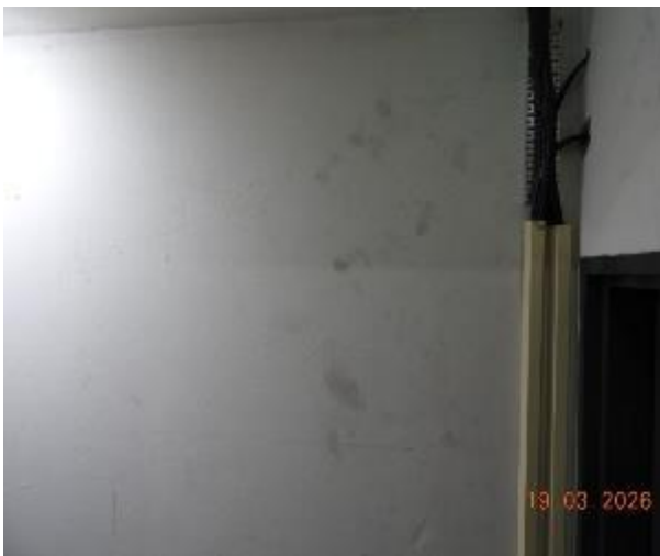
Figure 428 - General condition of level 1 fire stairs internal wall
