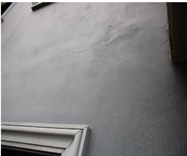
Figure 671 - General condition of external wall
