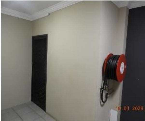
Figure 79 - General condition of level 3 common area internal wall
