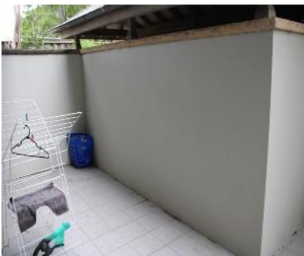
Figure 517 - General condition of courtyard external wall
