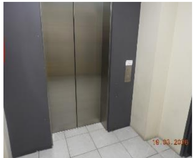
Figure 70 - General condition of level 2 common area internal wall
