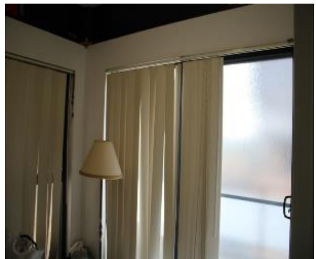
Figure 1546 - General condition of bedroom 1 internal wall
