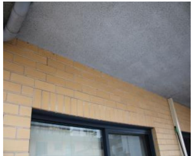
Figure 1258 - General condition of external wall
