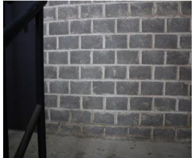
Figure 228 - General condition of B1 fire stairs internal wall
