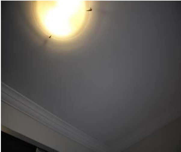
Figure 1571 - General condition of bedroom 2 ceiling
