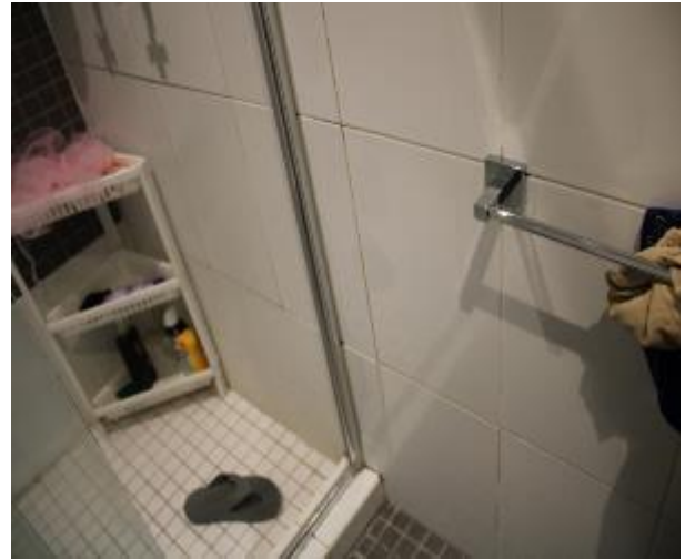
Figure 1045 - General condition of ensuite bathroom internal wall
