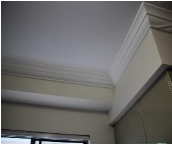
Figure 1129 - General condition of kitchen ceiling
