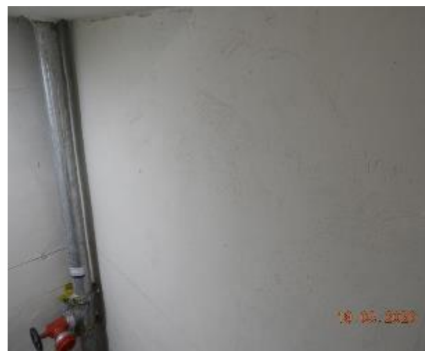
Figure 401 - General condition of level 1 fire stairs internal wall
