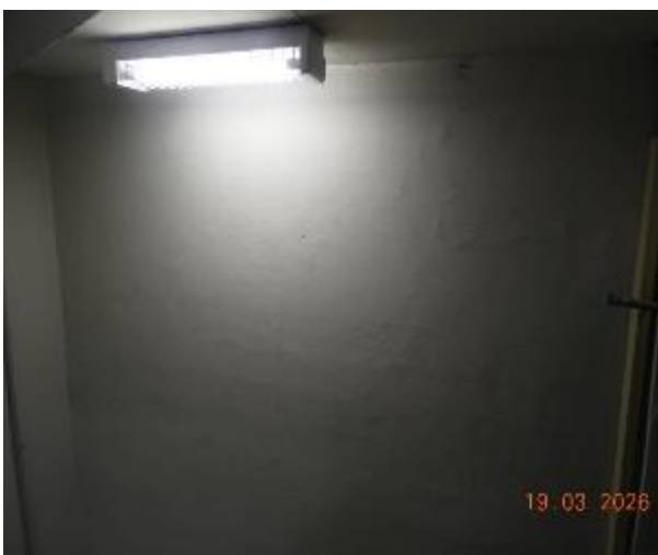
Figure 352 - General condition of level 3 fire stairs internal wall
