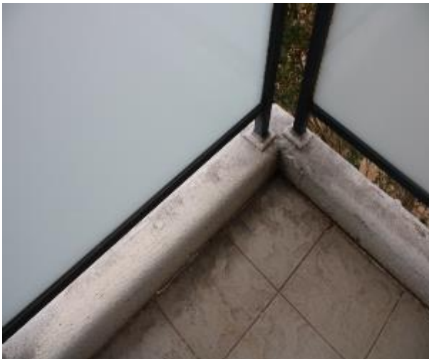
Figure 1255 - General condition of balcony floor tiles
