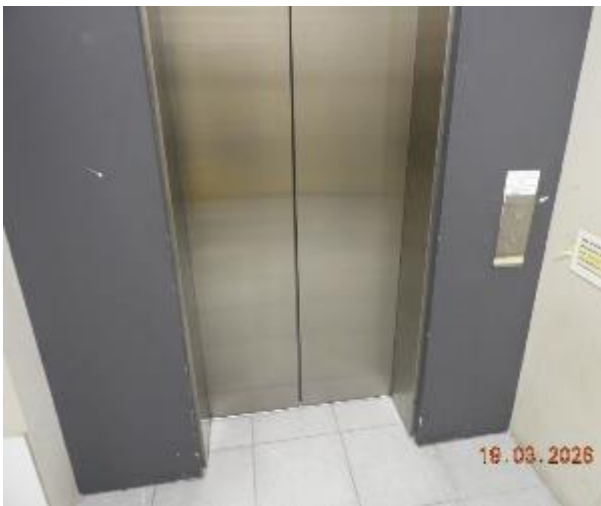
Figure 111 - General condition of level 3 common area internal wall
