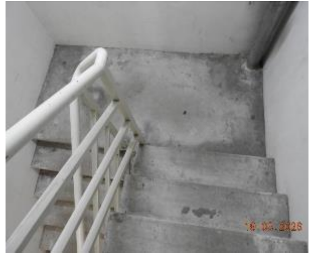
Figure 361 - General condition of level 2 fire stairs
