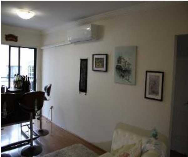
Figure 1103 - General condition of dining room internal wall
