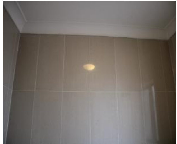
Figure 1353 - General condition of bathroom 1 internal wall
