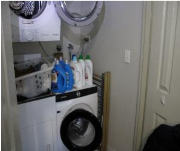
Figure 673 - General condition of laundry internal wall
