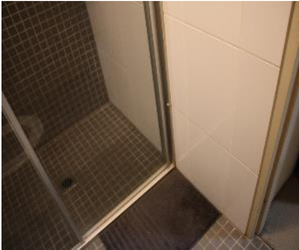
Figure 811 - General condition of ensuite bathroom internal wall
