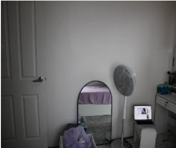
Figure 1062 - General condition of bedroom 2 internal wall
