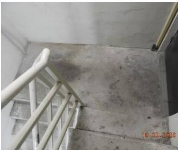
Figure 346 - General condition of level 3 fire stairs
