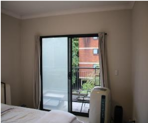
Figure 681 - General condition of bedroom 1 internal wall
