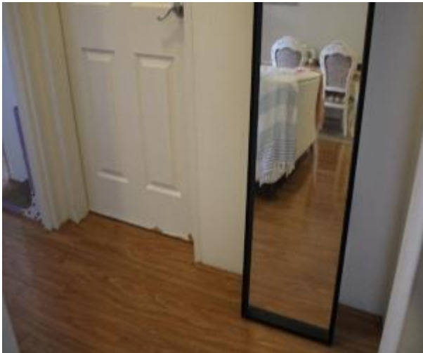
Figure 1147 - General condition of corridor internal wall
