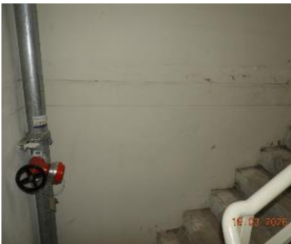
Figure 328 - General condition of level 3 fire stairs internal wall
