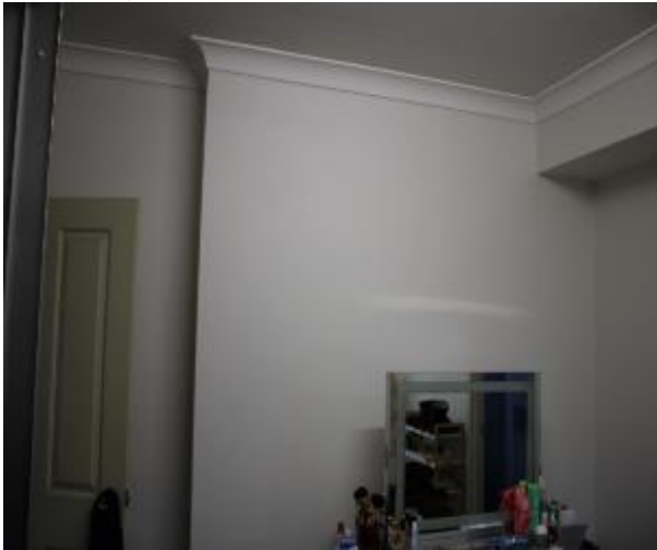
Figure 709 - General condition of dressing room internal wall
