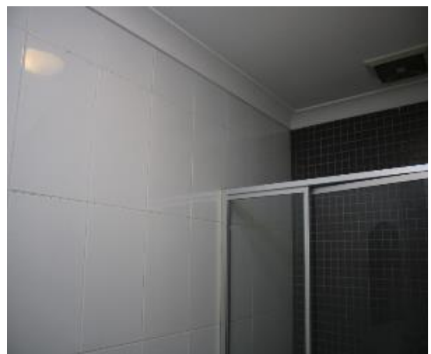
Figure 1399 - General condition of ensuite bathroom internal wall
