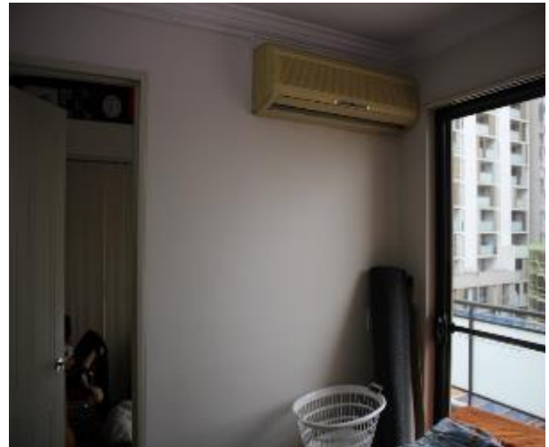
Figure 1460 - General condition of open kitchen/ lounge room internal wall
