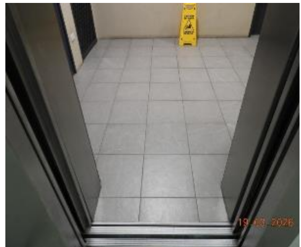
Figure 76 - General condition of level 3 common area floor tiles
