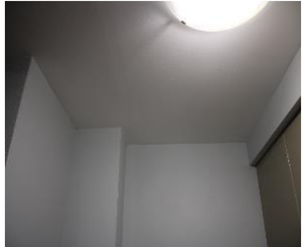
Figure 484 - General condition of open kitchen/ lounge room ceiling
