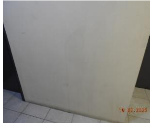
Figure 122 - General condition of level 4 common area internal wall
