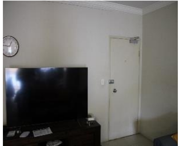
Figure 728 - General condition of open kitchen/ lounge room internal wall
