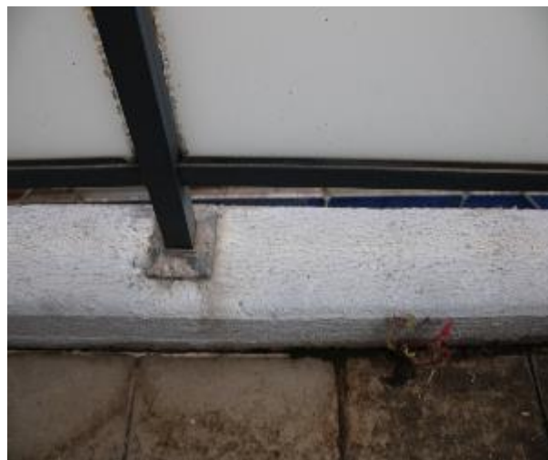
Figure 1504 - General condition of balcony floor tiles
