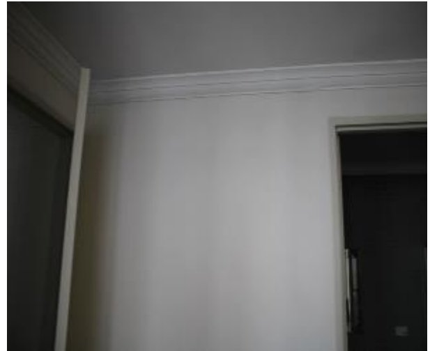
Figure 1608 - General condition of bedroom 3 internal wall
