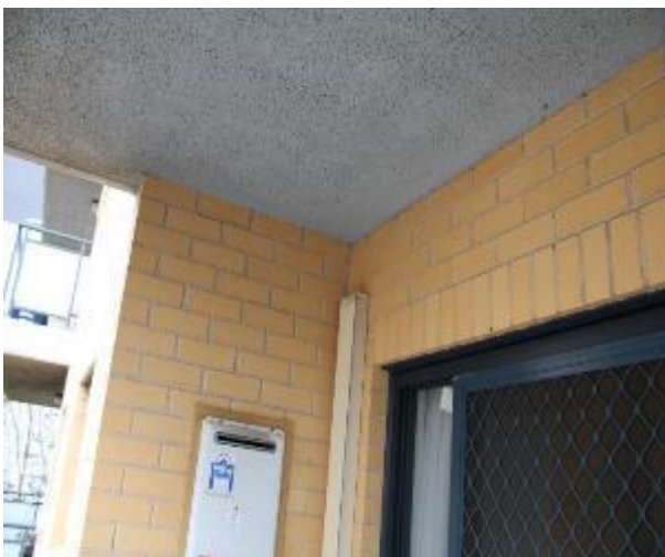
Figure 928 - General condition of external wall
