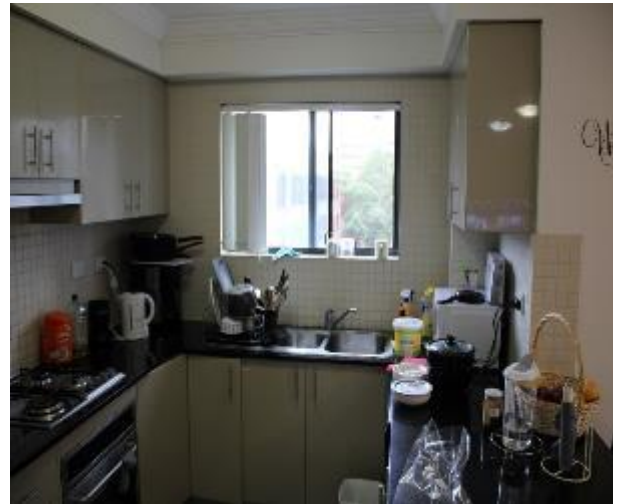
Figure 963 - General condition of kitchen internal wall
