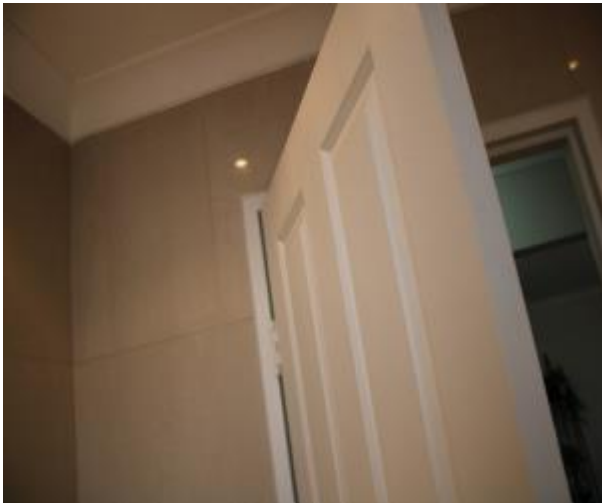
Figure 1016 - General condition of bathroom 1 internal wall
