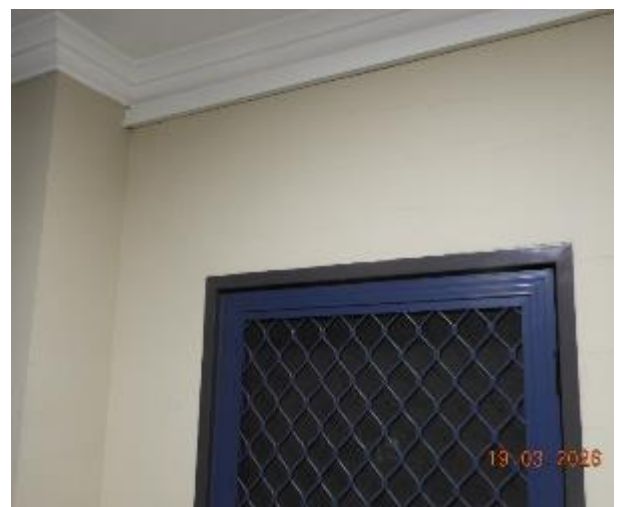
Figure 102 - General condition of level 3 common area internal wall
