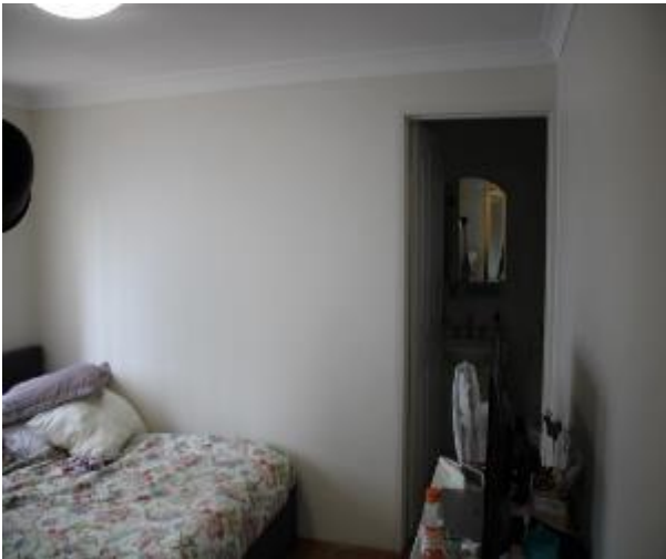
Figure 1183 - General condition of bedroom 1 internal wall
