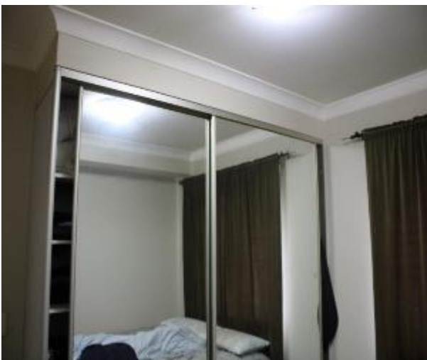
Figure 797 - General condition of bedroom 1 internal wall
