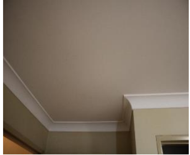
Figure 1383 - General condition of bedroom 1 ceiling
