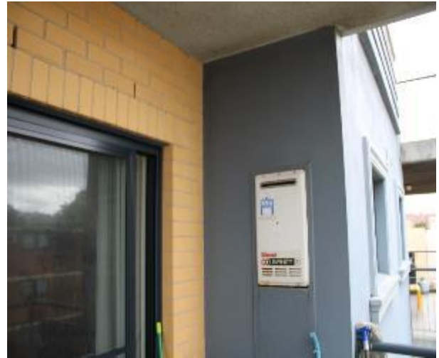
Figure 1087 - General condition of external wall
