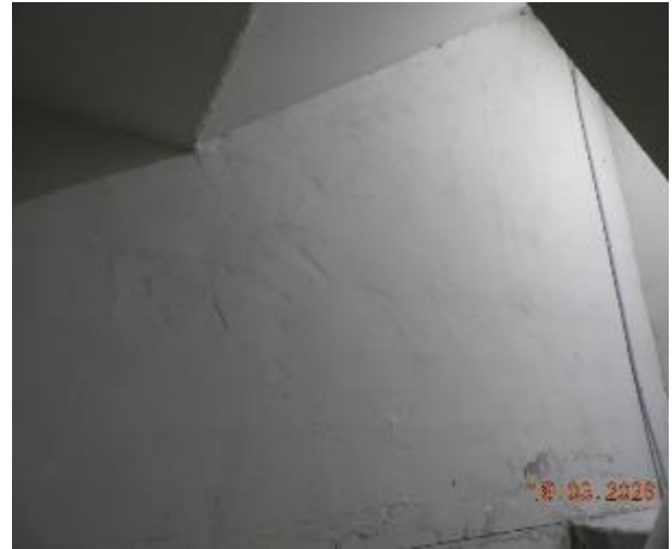
Figure 331 - General condition of level 3 fire stairs internal wall
