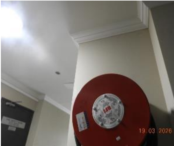
Figure 37 - General condition of level 1 common area ceiling
