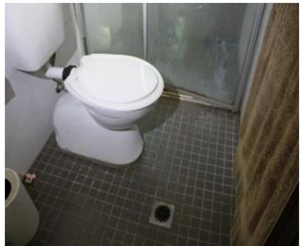
Figure 1397 - General condition of ensuite bathroom floor tiles
