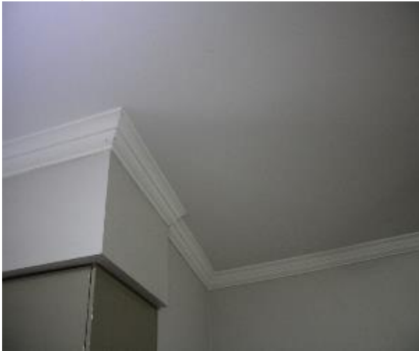
Figure 643 - General condition of lounge room ceiling
