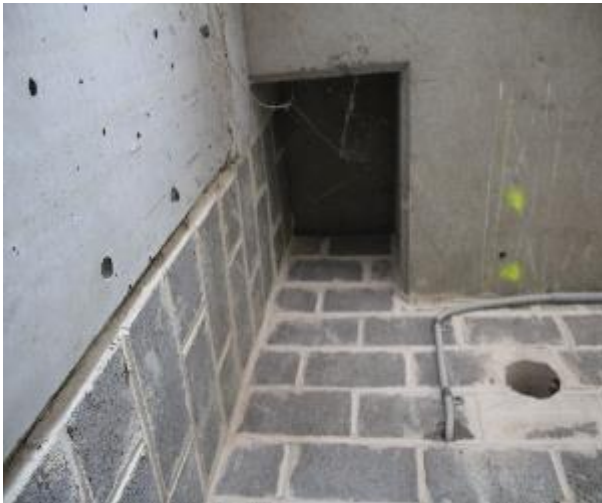
Figure 235 - General condition of B1 fire stairs underside slab
