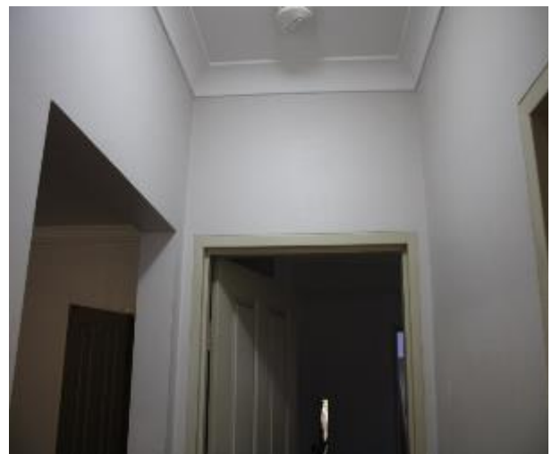
Figure 678 - General condition of corridor internal wall
