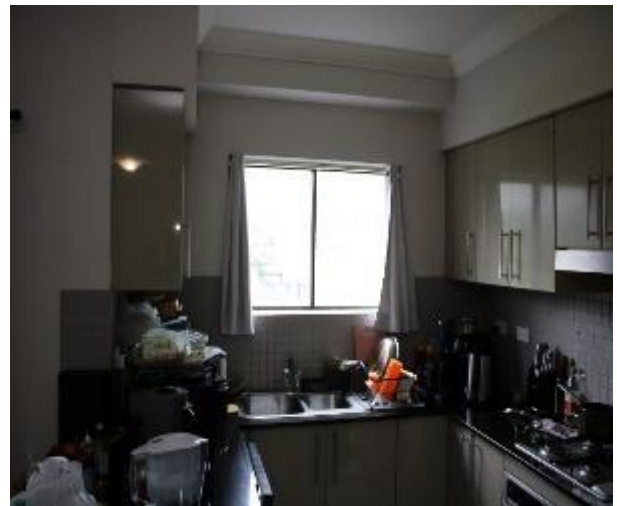
Figure 646 - General condition of kitchen internal wall
