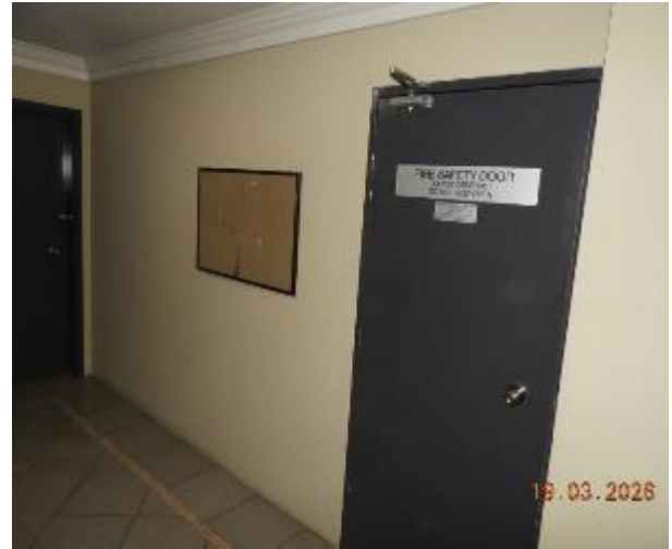
Figure 20 - General condition of level 1 common area internal wall
