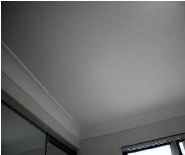
Figure 1205 - General condition of bedroom 1 ceiling
