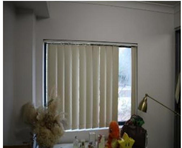
Figure 706 - General condition of dressing room internal wall
