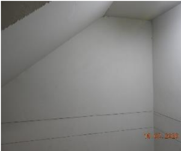
Figure 374 - General condition of level 2 fire stairs internal wall
