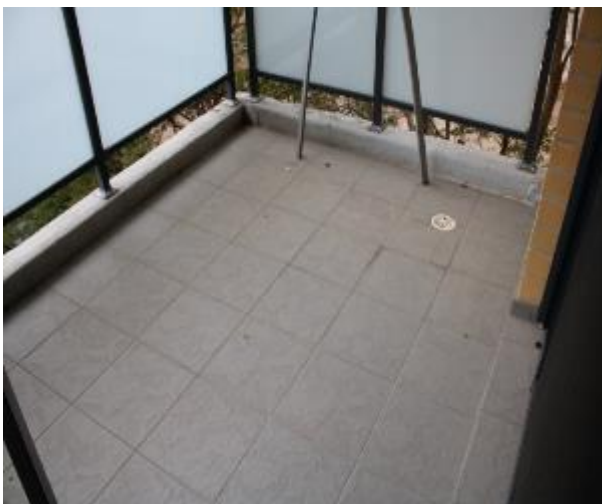
Figure 827 - General condition of balcony floor tiles
