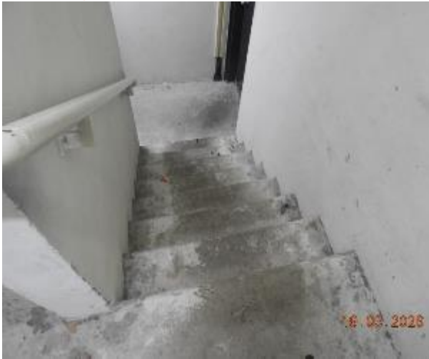
Figure 414 - General condition of level 1 fire stairs
