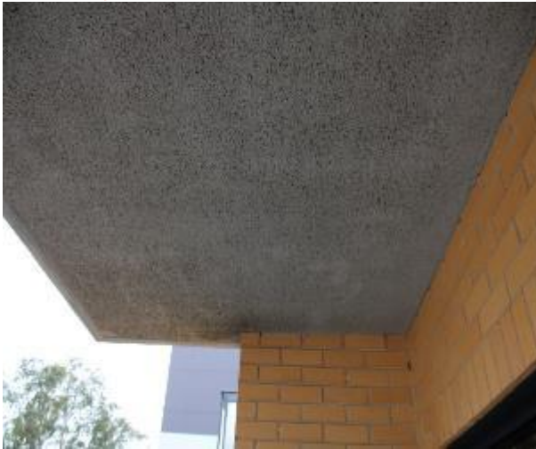
Figure 1448 - General condition of balcony underside slab
