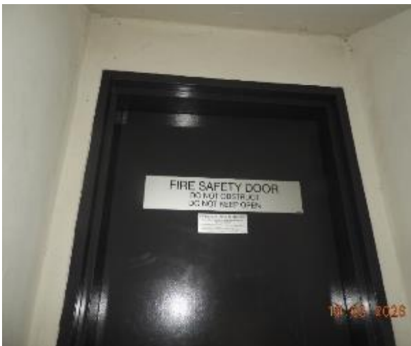
Figure 446 - General condition of basement fire stairs internal wall
