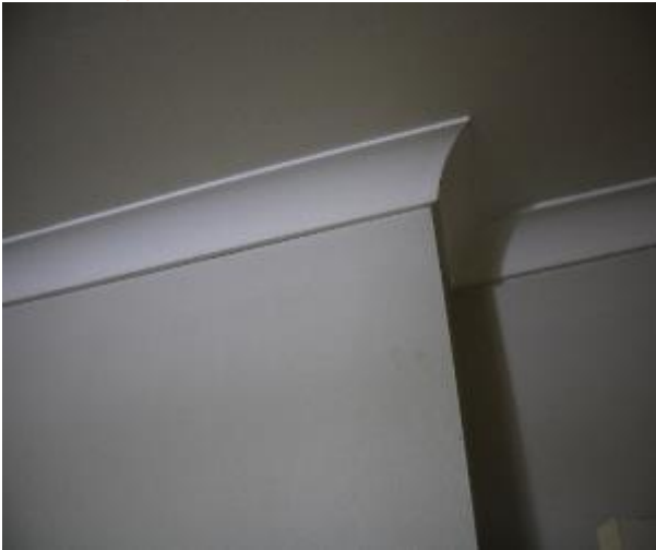
Figure 799 - General condition of bedroom 1 internal wall
