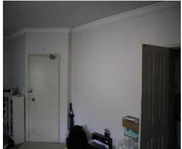
Figure 620 - General condition of lounge room internal wall
