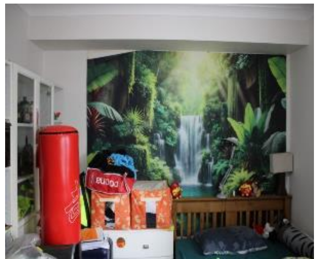
Figure 893 - General condition of bedroom 2 internal wall
