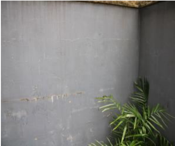
Figure 617 - General condition of courtyard external wall
