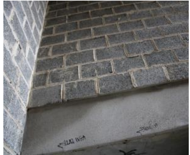
Figure 258 - General condition of level 1 fire stairs internal wall
