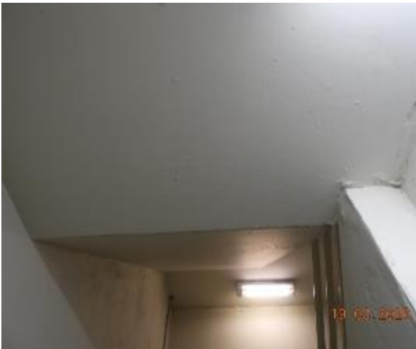
Figure 410 - General condition of level 1 fire stairs underside stairs
