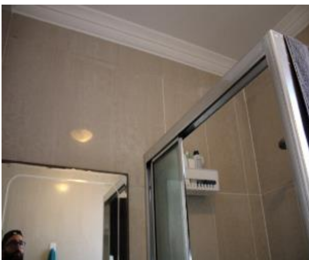
Figure 1593 - General condition of bathroom 1 internal wall
