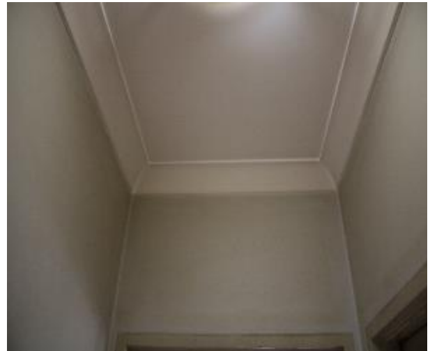
Figure 772 - General condition of corridor ceiling
