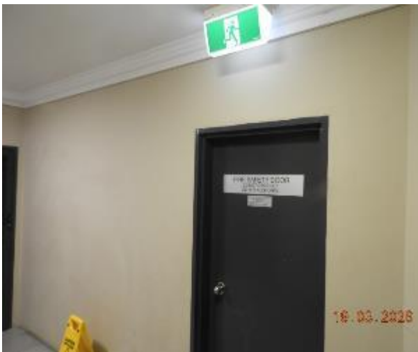
Figure 93 - General condition of level 3 common area internal wall
