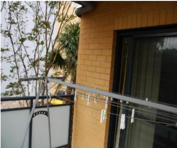
Figure 837 - General condition of external wall
