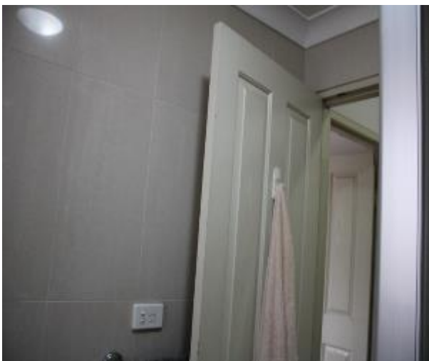
Figure 701 - General condition of bathroom 1 internal wall
