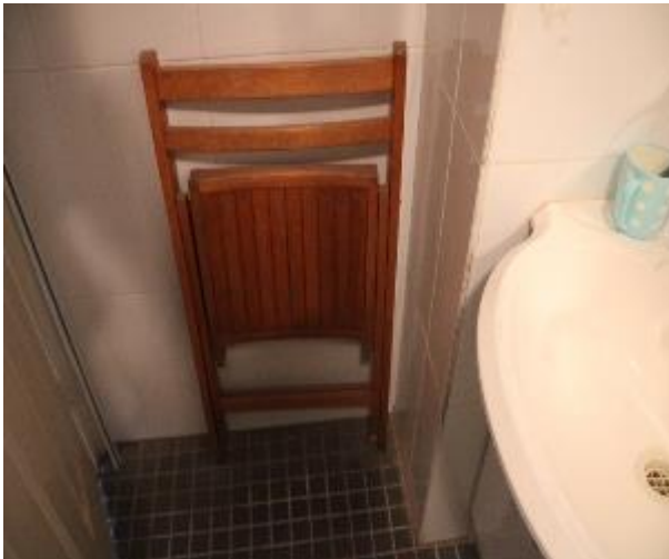
Figure 908 - General condition of ensuite bathroom internal wall
