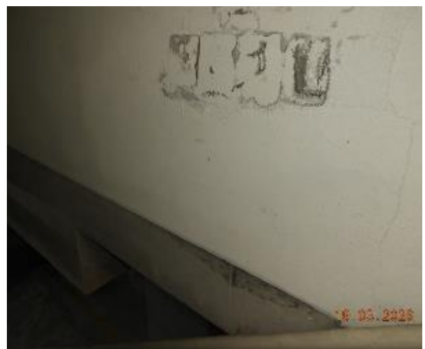
Figure 461 - General condition of basement fire stairs internal wall
