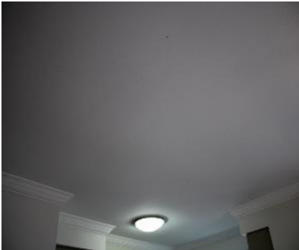
Figure 956 - General condition of lounge room ceiling
