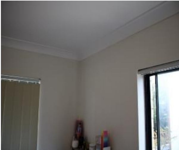
Figure 1229 - General condition of bedroom 2 internal wall
