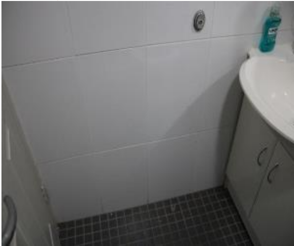
Figure 1217 - General condition of ensuite bathroom internal wall
