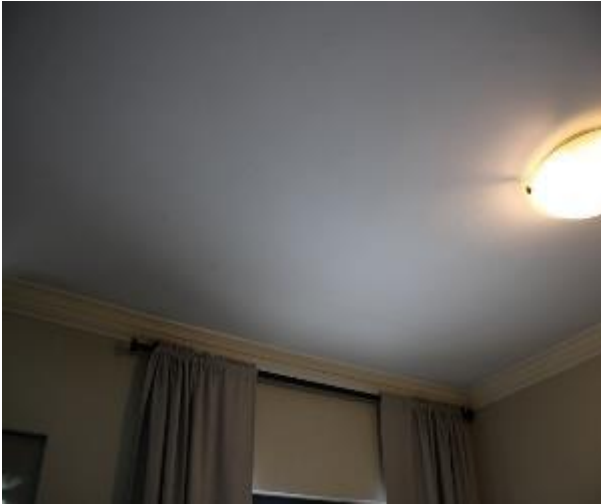
Figure 765 - General condition of open kitchen/ lounge room ceiling
