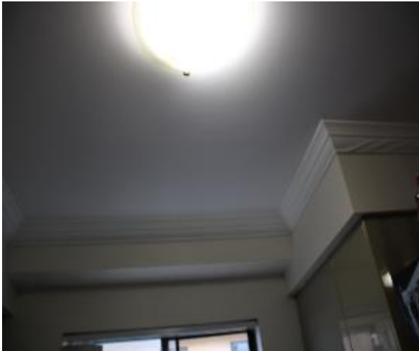
Figure 1127 - General condition of kitchen ceiling
