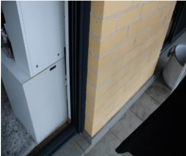
Figure 1092 - General condition of external wall
