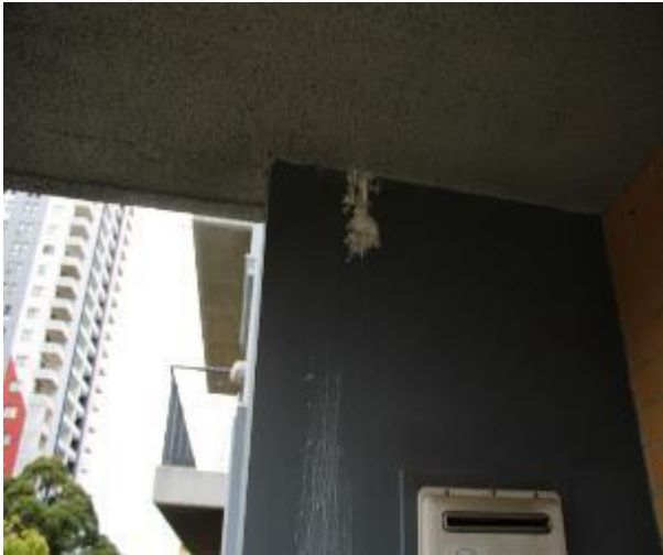
Figure 661 - General condition of external wall
