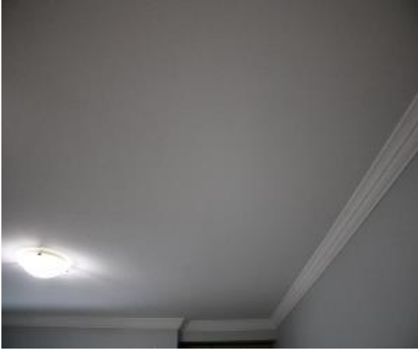
Figure 489 - General condition of open kitchen/ lounge room ceiling
