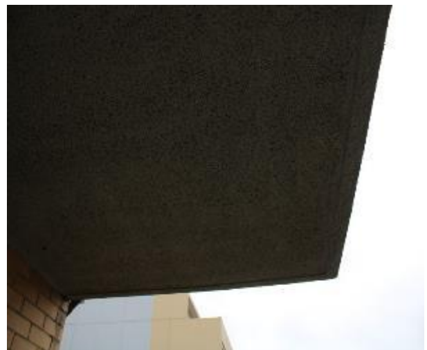
Figure 666 - General condition of balcony underside slab
