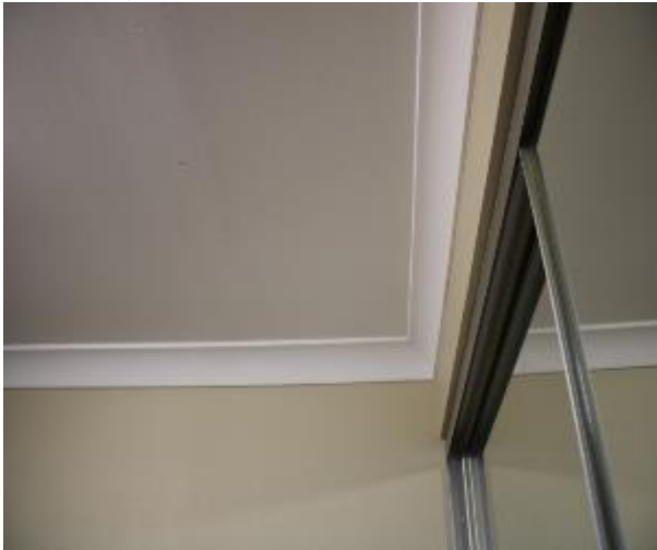
Figure 1394 - General condition of bedroom 1 ceiling
