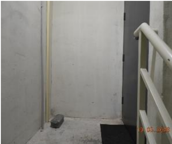
Figure 284 - General condition of level 5 fire stairs internal wall
