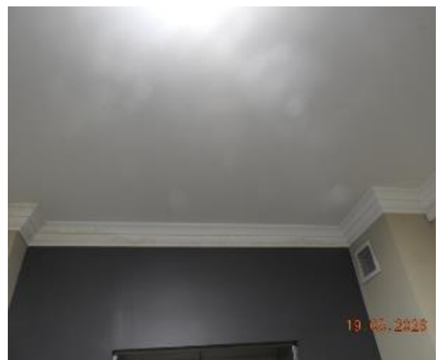
Figure 72 - General condition of level 2 common area ceiling
