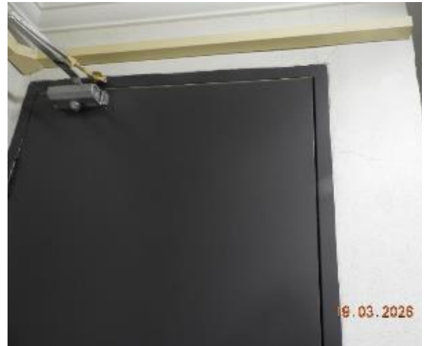
Figure 279 - General condition of level 5 fire stairs internal wall
