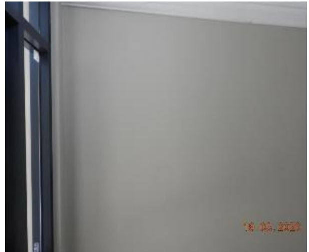
Figure 10 - General condition of level 1 common area internal wall
