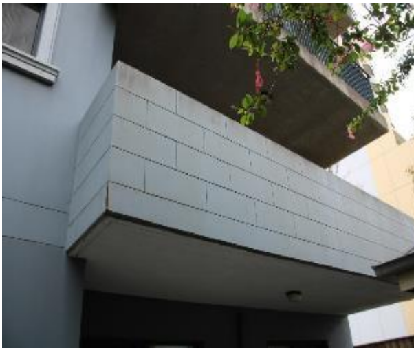
Figure 509 - General condition of external wall
