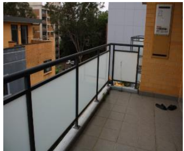
Figure 1534 - General condition of balcony balustrade
