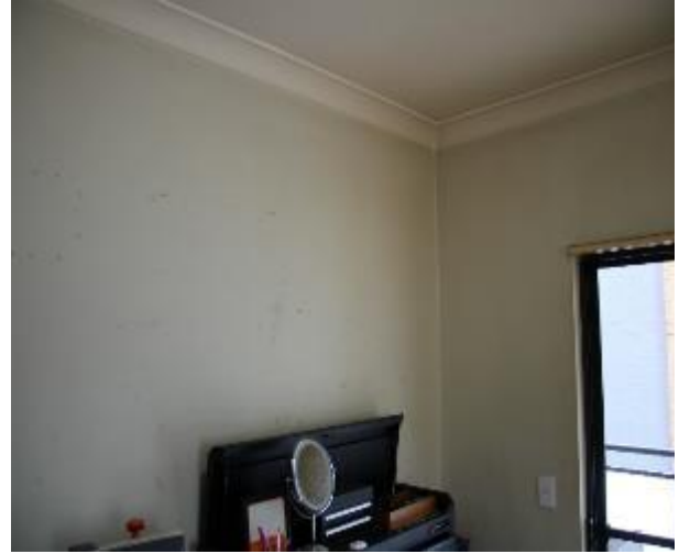
Figure 818 - General condition of study internal wall
