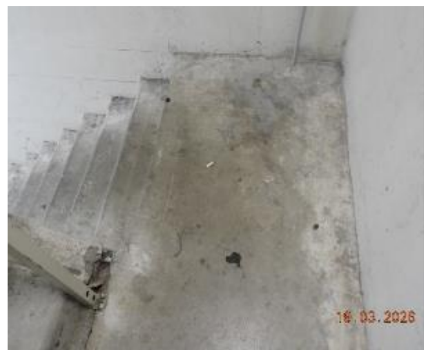
Figure 383 - General condition of level 2 fire stairs
