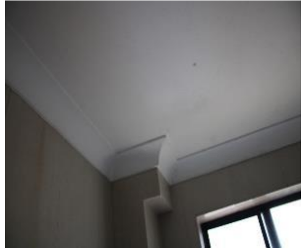
Figure 784 - General condition of bathroom 1 ceiling
