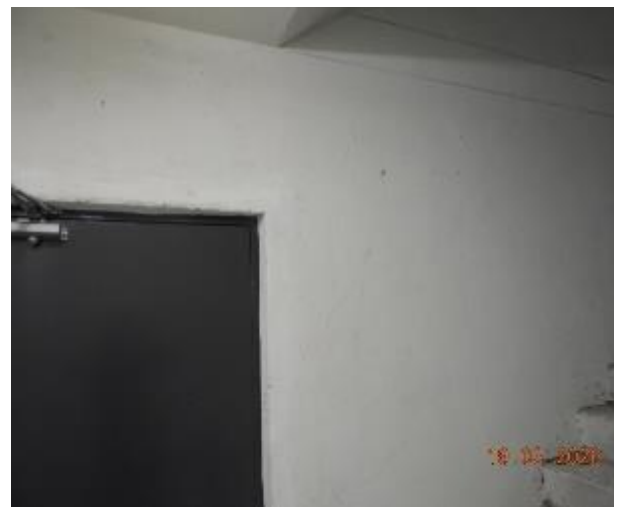
Figure 347 - General condition of level 3 fire stairs internal wall
