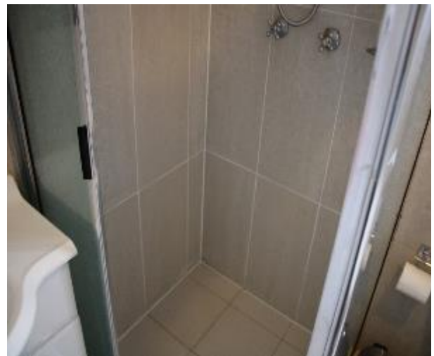
Figure 1592 - General condition of bathroom 1 internal wall
