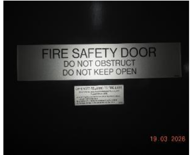
Figure 277 - The following images display the condition of the fire stairs from Level 5 to B2
