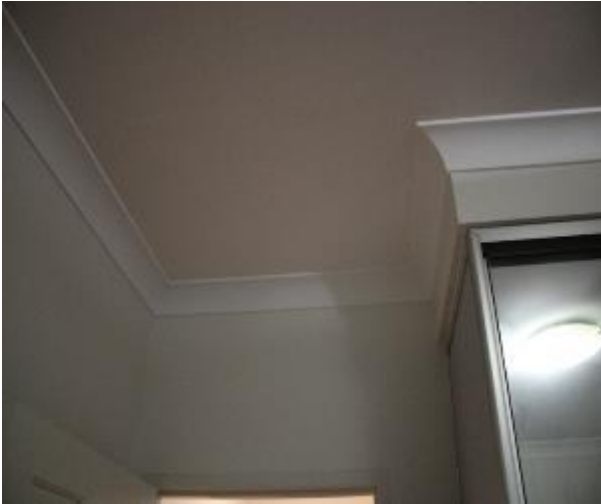
Figure 1025 - General condition of bedroom 1 ceiling
