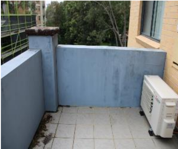
Figure 1302 - General condition of external wall
