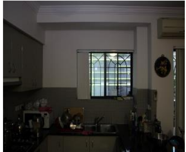
Figure 982 - General condition of kitchen internal wall
