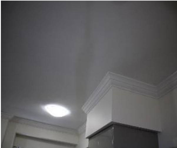
Figure 520 - General condition of open kitchen/ lounge room ceiling
