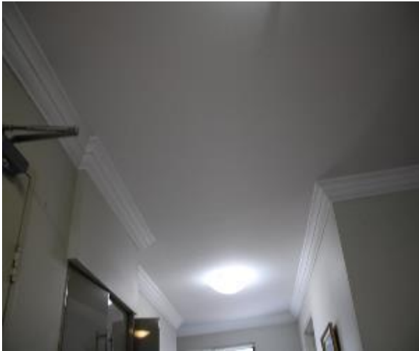
Figure 1430 - General condition of kitchen ceiling
