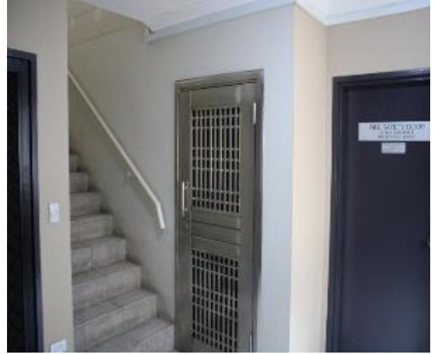
Figure 104 - General condition of level 4 common area internal wall
