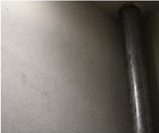
Figure 315 - General condition of level 5 to basement B2 fire stairs internal wall
