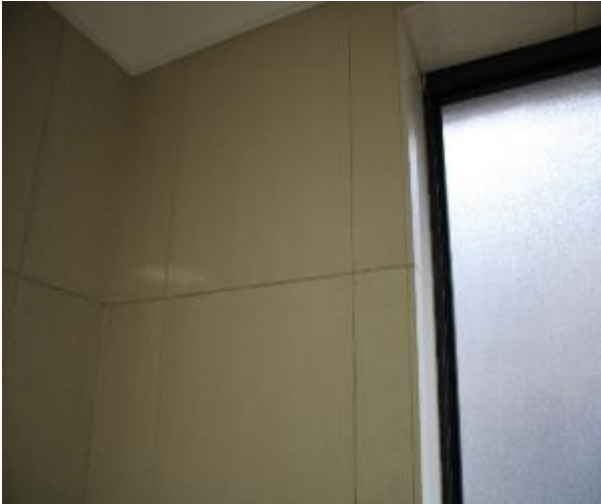
Figure 742 - General condition of bathroom 1 internal wall
