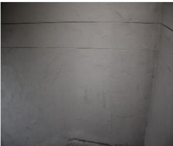
Figure 367 - General condition of level 5 to basement B2 fire stairs internal wall
