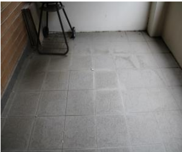
Figure 774 - General condition of balcony floor tiles
