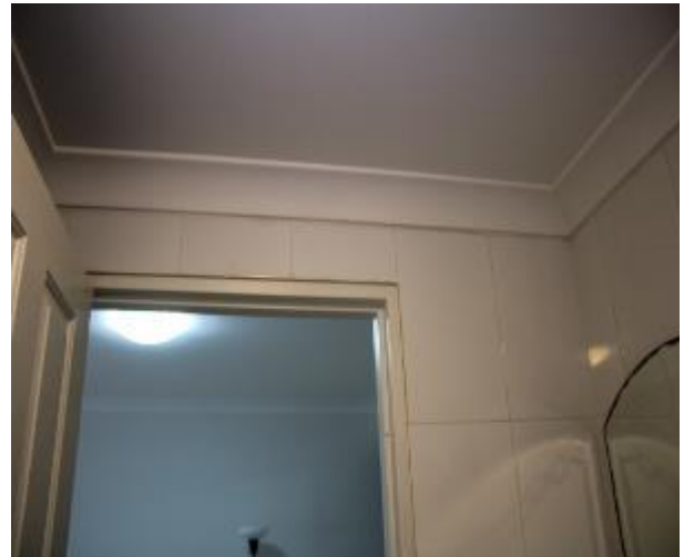
Figure 719 - General condition of ensuite bathroom internal wall
