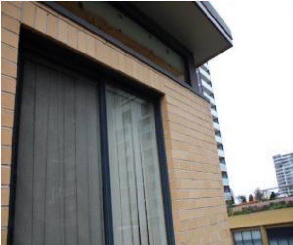
Figure 1592 - General condition of external wall
