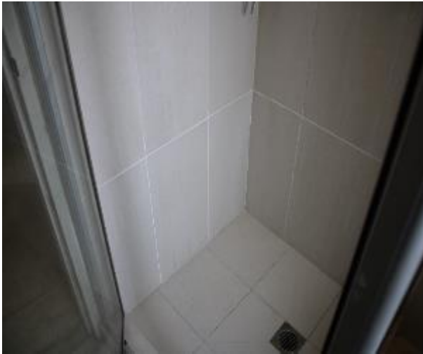
Figure 1538 - General condition of bathroom 1 internal wall
