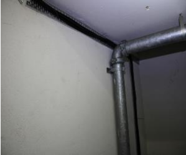
Figure 411 - General condition of level 5 to basement B2 fire stairs internal wall
