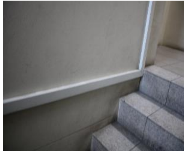
Figure 134 - General condition of staircase to level 5 common area internal wall
