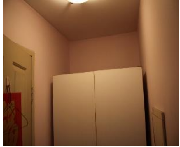
Figure 1123 - General condition of bedroom 1 internal wall
