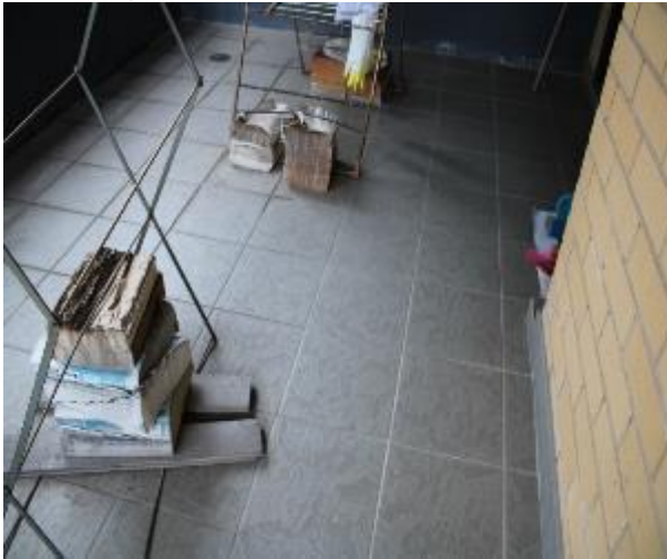
Figure 1218 - General condition of balcony 2 floor tiles
