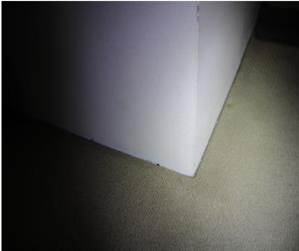
Figure 508 - General condition of open kitchen/ lounge room internal wall
