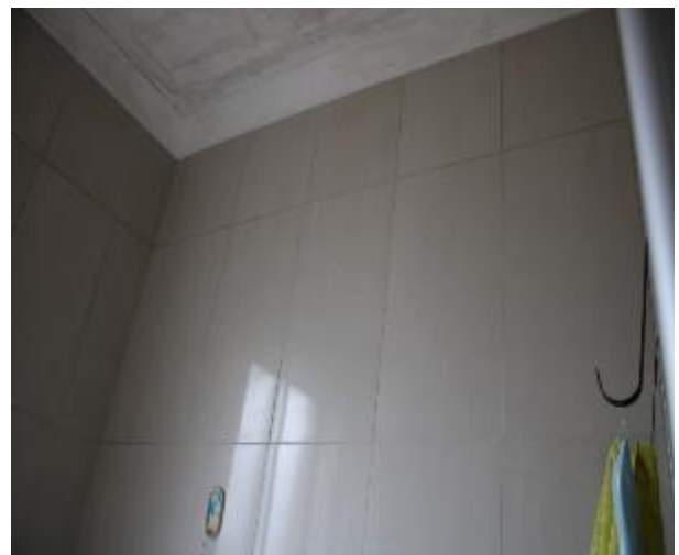
Figure 1355 - General condition of bathroom 1 internal wall
