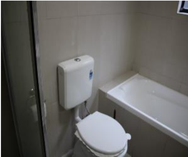
Figure 746 - General condition of bathroom 1 internal wall
