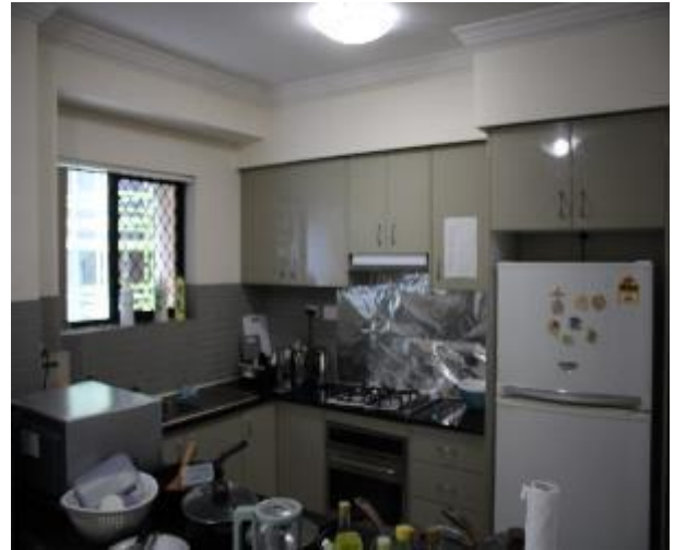
Figure 497 - General condition of open kitchen/ lounge room internal wall
