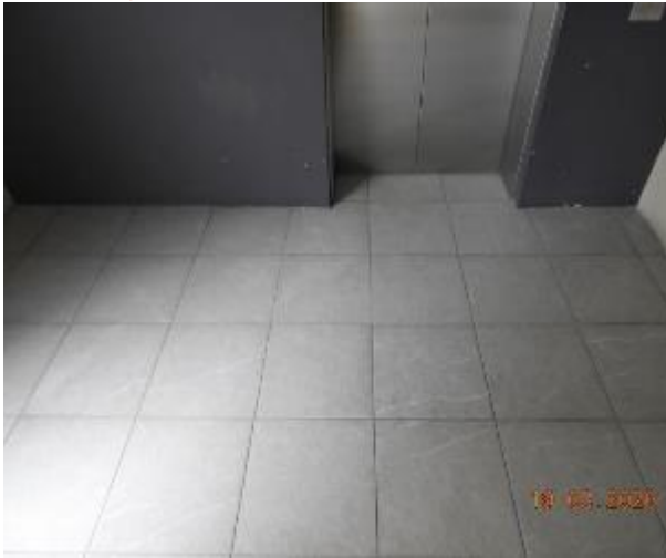
Figure 31 - General condition of level 2 common area floor tiles
