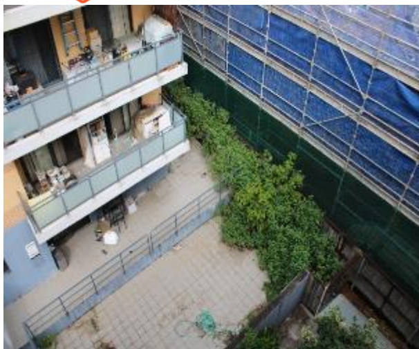
Figure 1416 - General condition of boundary as seen from Unit 28 balcony
