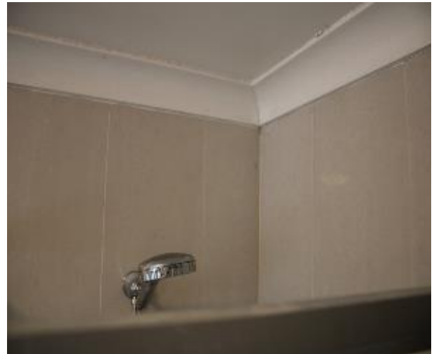
Figure 843 - General condition of bathroom 1 internal wall
