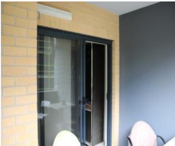
Figure 946 - General condition of external wall
