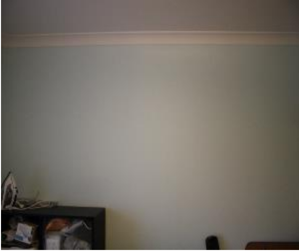
Figure 1176 - General condition of bedroom 2 internal wall
