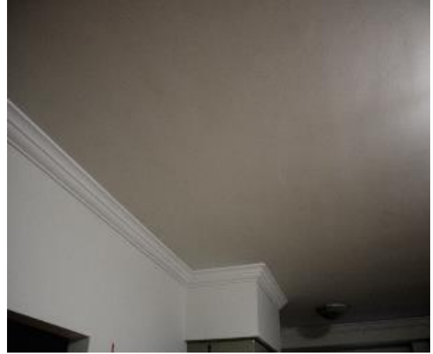
Figure 976 - General condition of lounge room ceiling
