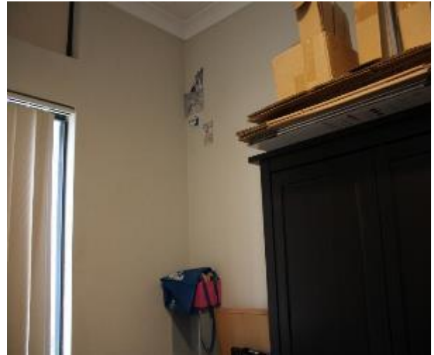
Figure 1557 - General condition of bedroom 2 internal wall
