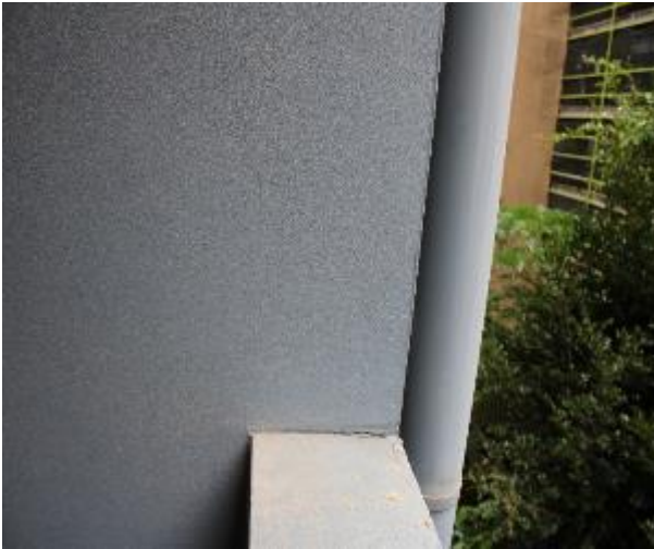
Figure 654 - General condition of external wall
