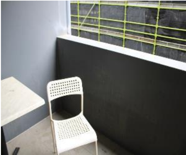
Figure 948 - General condition of external wall
