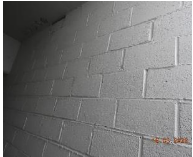
Figure 204 - General condition of B2 to Level 1 fire stairs internal wall
