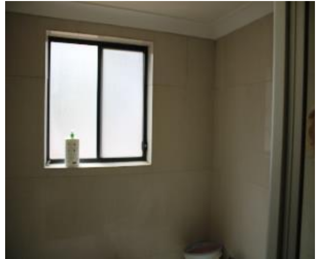
Figure 605 - General condition of bathroom 1 internal wall
