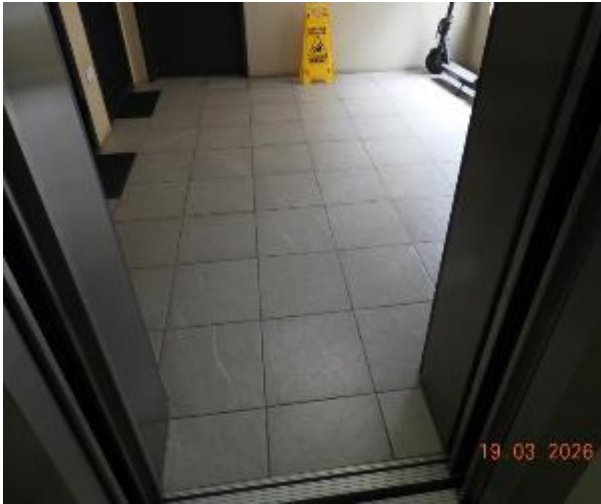
Figure 55 - General condition of level 3 common area floor tiles
