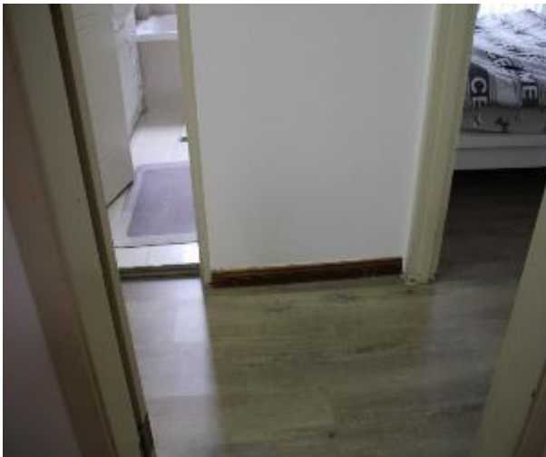
Figure 1322 - General condition of corridor internal wall
