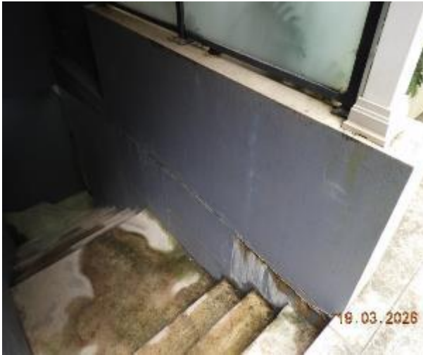
Figure 161 - General condition of B2 to Level 1 fire stairs internal wall
