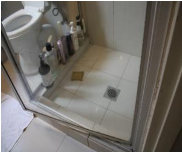
Figure 836 - General condition of bathroom 1 floor tiles
