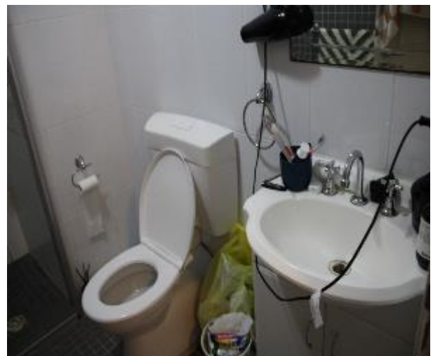
Figure 929 - General condition of ensuite bathroom internal wall
