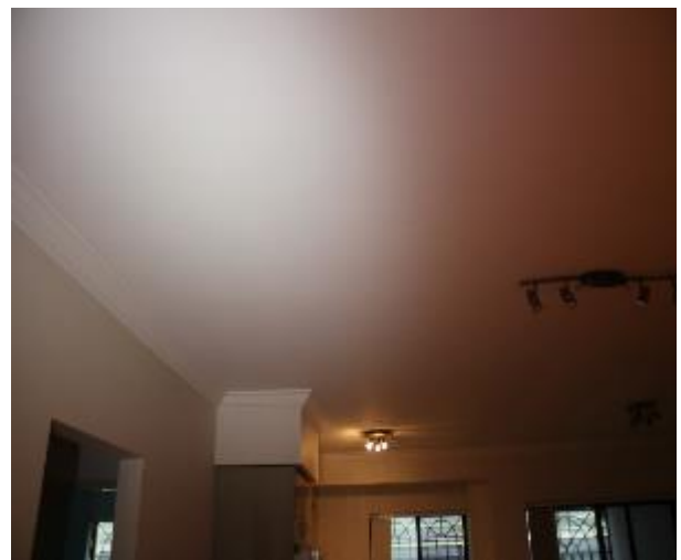
Figure 1109 - General condition of lounge room ceiling
