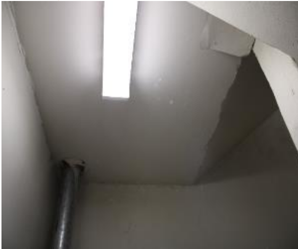
Figure 387 - General condition of level 5 to basement B2 fire stairs underside stairs
