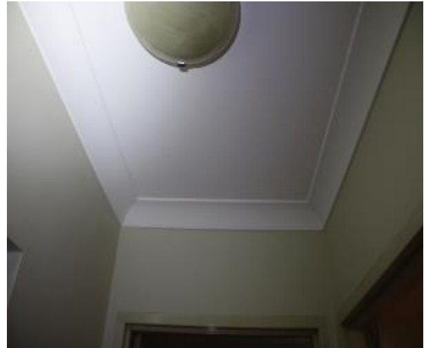
Figure 871 - General condition of corridor ceiling
