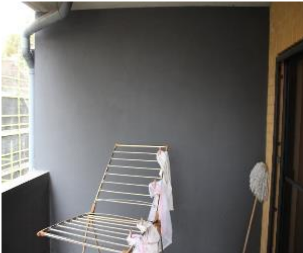
Figure 1220 - General condition of external wall
