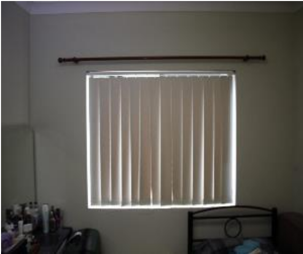
Figure 882 - General condition of bedroom 2 internal wall
