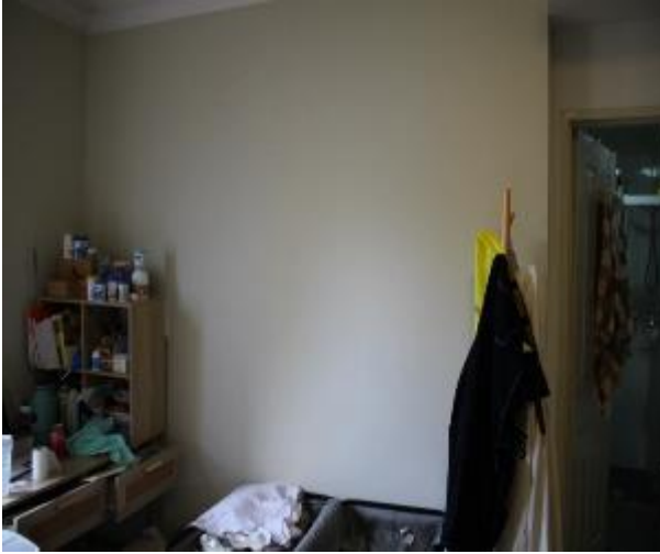
Figure 918 - General condition of bedroom 3 internal wall
