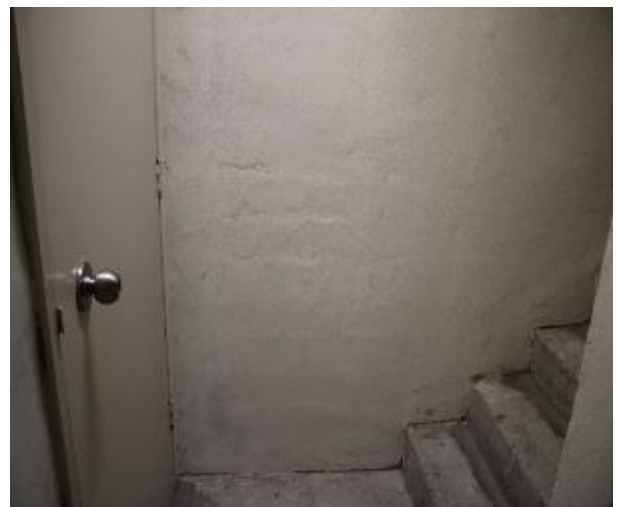
Figure 278 - General condition of level 5 to basement B2 fire stairs internal wall
