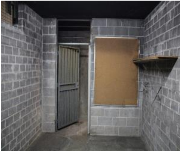
Figure 441 - General condition of basement B2 fire stairs internal wall
