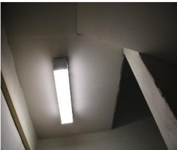
Figure 301 - General condition of level 5 to basement B2 fire stairs underside stairs
