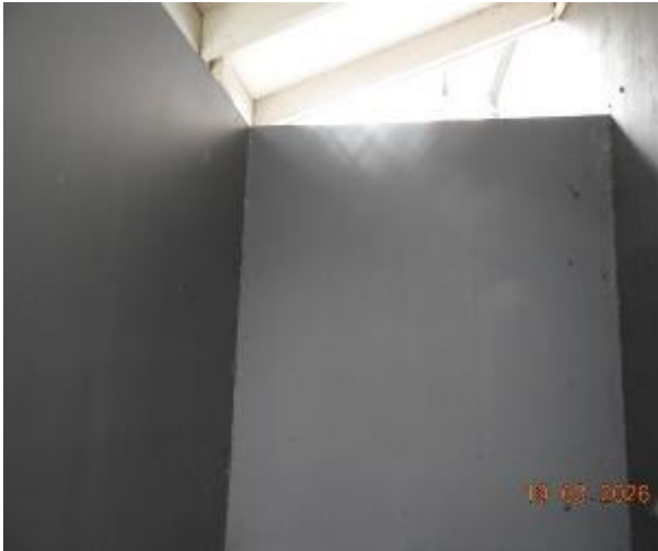
Figure 167 - General condition of B2 to Level 1 fire stairs internal wall
