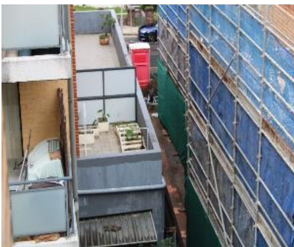
Figure 1530 - General condition of boundary as seen from Unit 29 balcony 2
