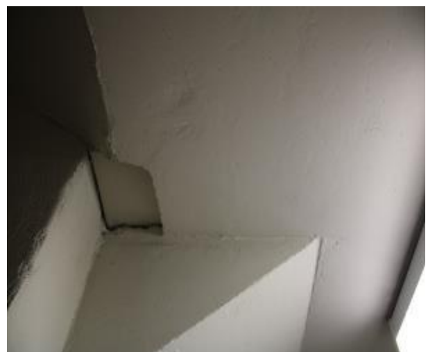
Figure 326 - General condition of level 5 to basement B2 fire stairs underside stairs
