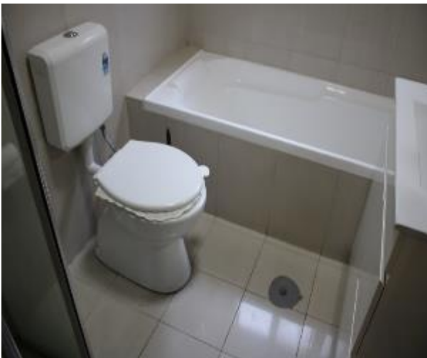
Figure 738 - General condition of bathroom 1 floor tiles
