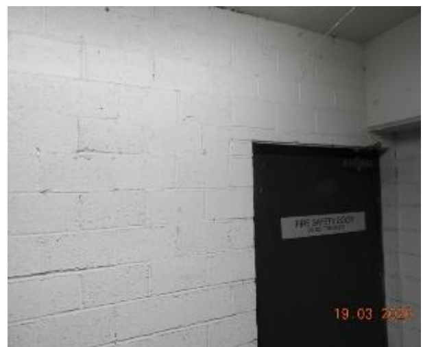
Figure 184 - General condition of B2 to Level 1 fire stairs internal wall
