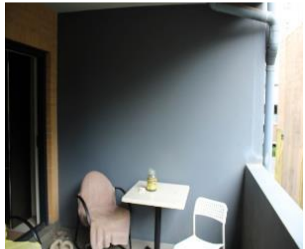
Figure 947 - General condition of external wall
