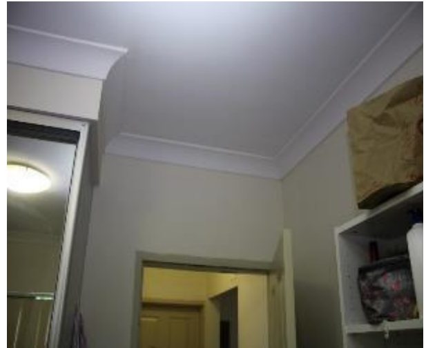
Figure 593 - General condition of bedroom 2 internal wall
