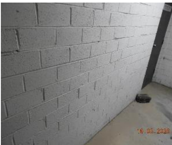
Figure 183 - General condition of B2 to Level 1 fire stairs internal wall
