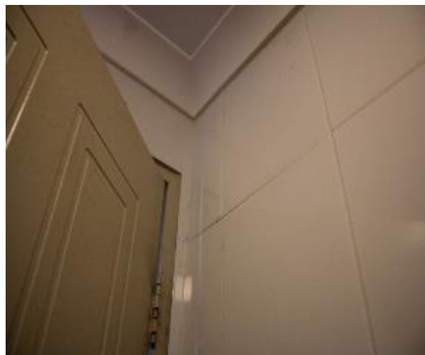
Figure 1503 - General condition of ensuite bathroom internal wall
