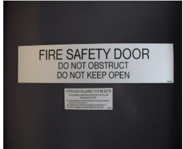
Figure 220 - The following images display the condition of the fire stairs from Level 5 to Basement B2
