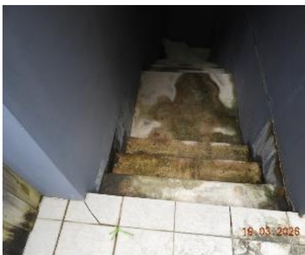
Figure 157 - General condition of B2 to Level 1 fire stairs
