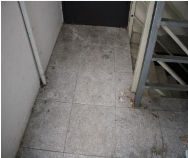
Figure 393 - General condition of level 5 to basement B2 fire stairs
