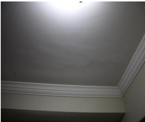
Figure 830 - General condition of open kitchen/ lounge room ceiling
