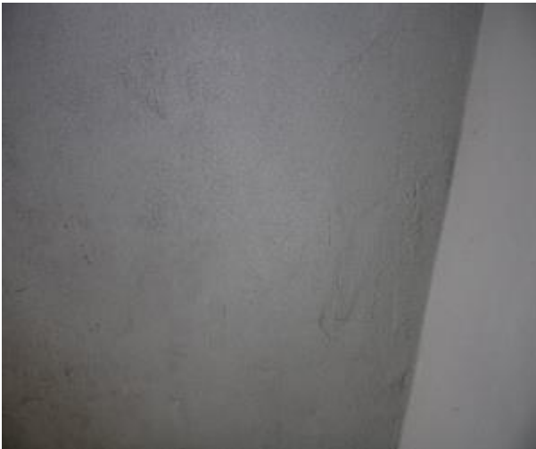
Figure 263 - General condition of level 5 to basement B2 fire stairs internal wall
