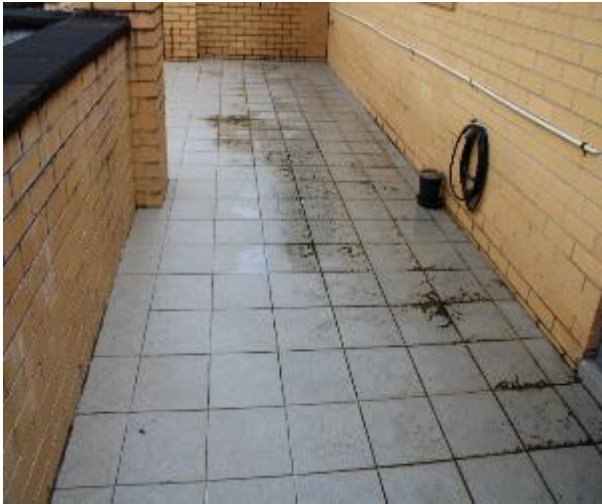
Figure 1392 - General condition of balcony 3 floor tiles
