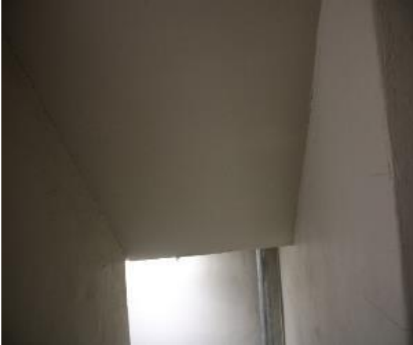
Figure 303 - General condition of level 5 to basement B2 fire stairs underside stairs
