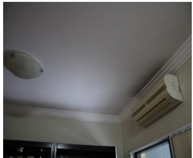
Figure 831 - General condition of open kitchen/ lounge room ceiling
