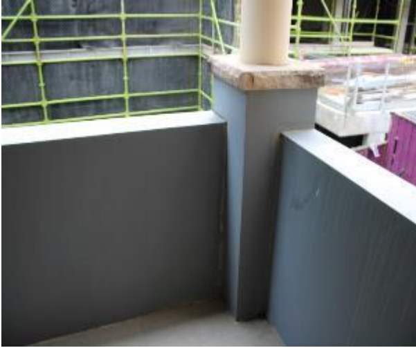
Figure 646 - General condition of external wall
