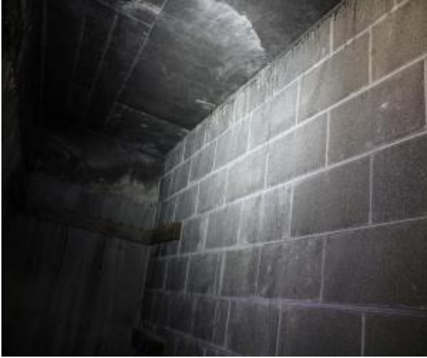
Figure 477 - General condition of basement B2 fire stairs internal wall
