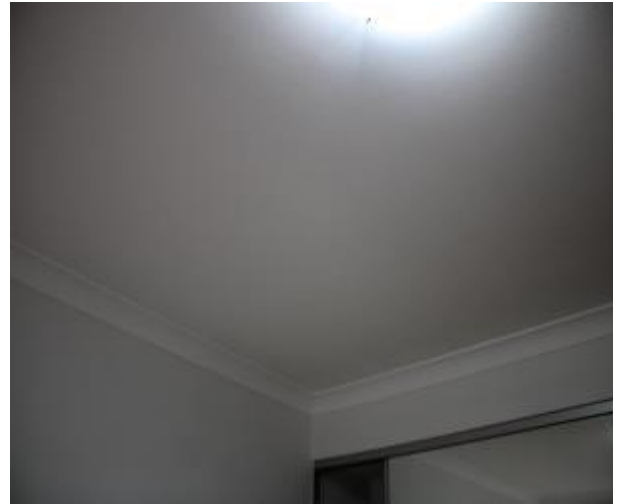
Figure 705 - General condition of bedroom 1 ceiling
