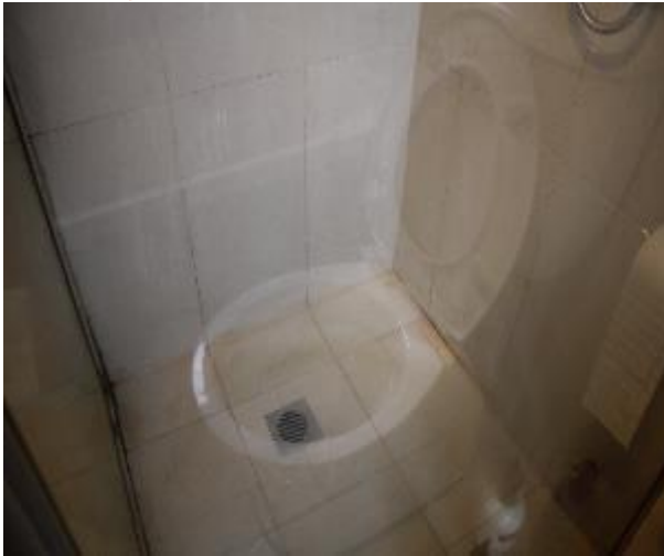
Figure 1188 - General condition of bathroom 1 internal wall
