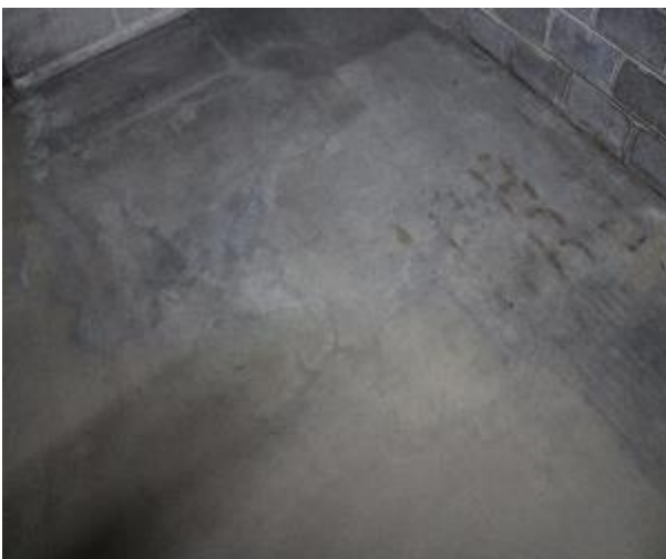
Figure 439 - General condition of basement B2 fire stairs pavement slab
