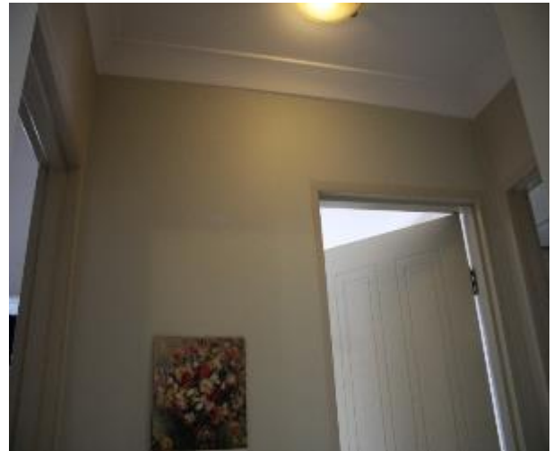
Figure 1463 - General condition of corridor internal wall
