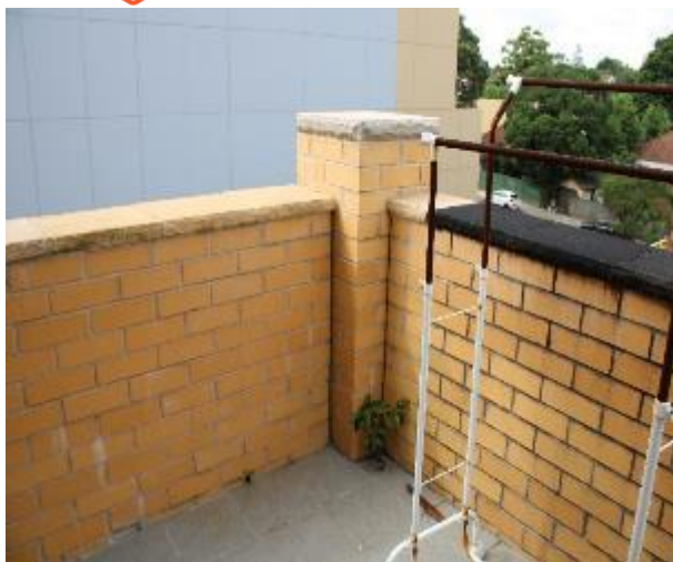
Figure 1404 - General condition of external wall
