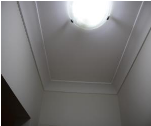
Figure 989 - General condition of corridor ceiling
