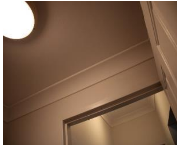
Figure 695 - General condition of laundry internal wall
