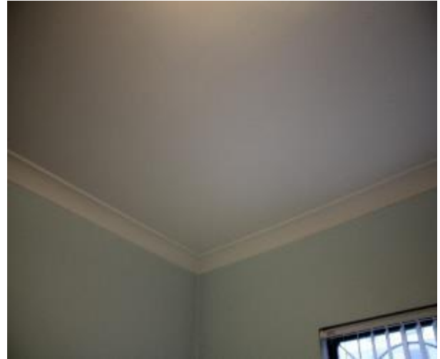
Figure 1179 - General condition of bedroom 2 ceiling
