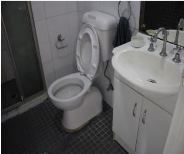
Figure 562 - General condition of ensuite bathroom internal wall
