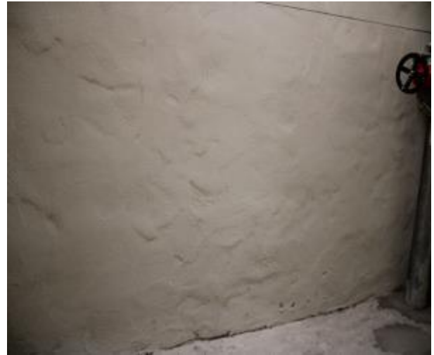
Figure 310 - General condition of level 5 to basement B2 fire stairs internal wall
