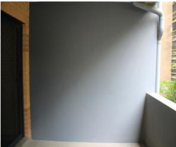
Figure 650 - General condition of external wall
