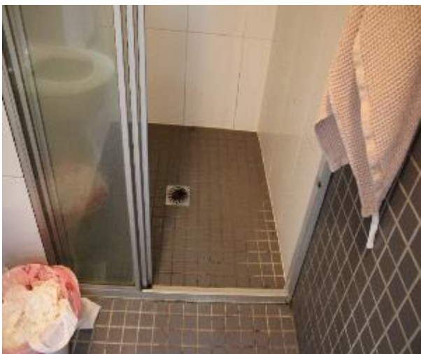
Figure 708 - General condition of ensuite bathroom floor tiles
