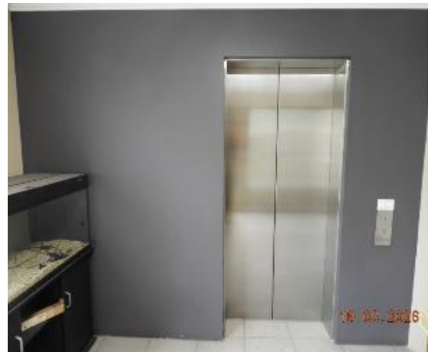
Figure 58 - General condition of level 3 common area internal wall
