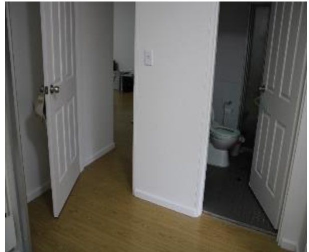
Figure 701 - General condition of bedroom 1 internal wall
