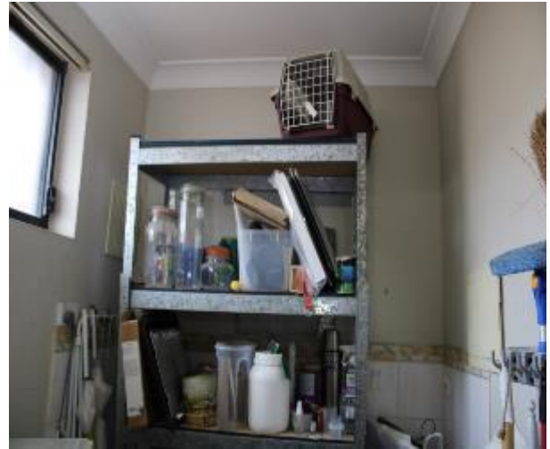
Figure 1437 - General condition of laundry internal wall
