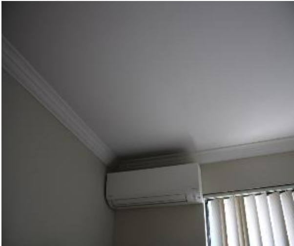
Figure 1460 - General condition of lounge room ceiling
