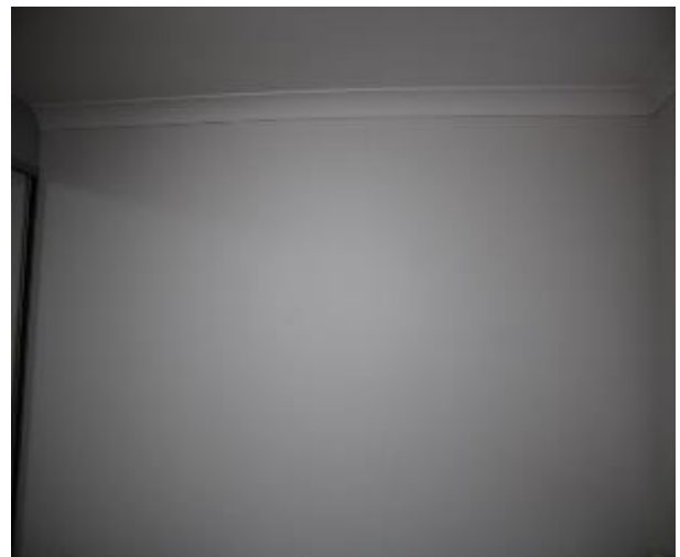
Figure 761 - General condition of bedroom 3 internal wall
