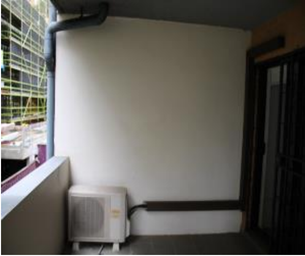
Figure 782 - General condition of external wall
