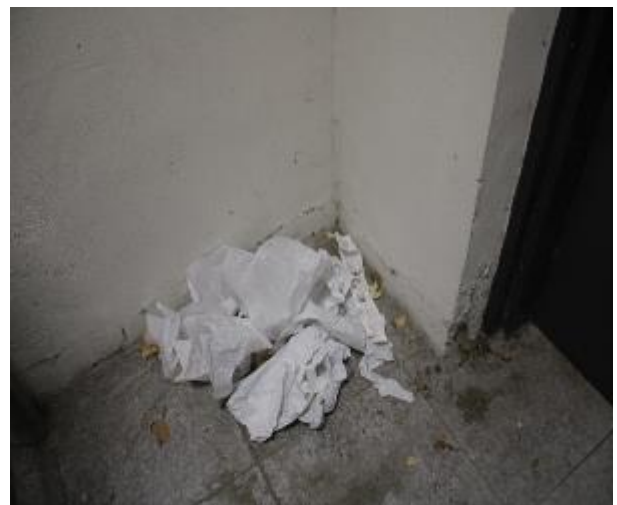
Figure 398 - General condition of level 5 to basement B2 fire stairs internal wall
