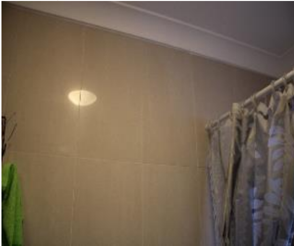
Figure 1041 - General condition of bathroom 1 internal wall
