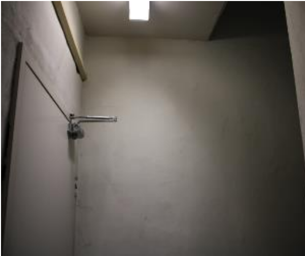
Figure 279 - General condition of level 5 to basement B2 fire stairs internal wall
