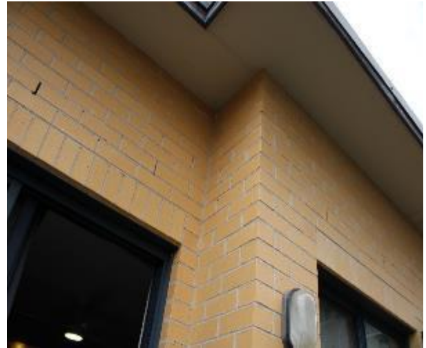
Figure 1575 - General condition of external wall
