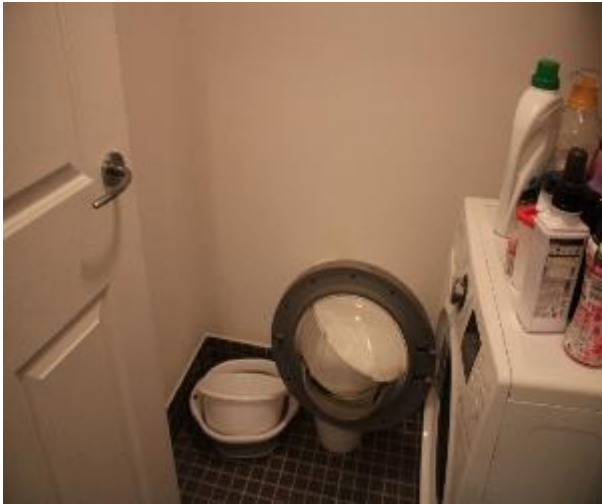
Figure 692 - General condition of laundry internal wall
