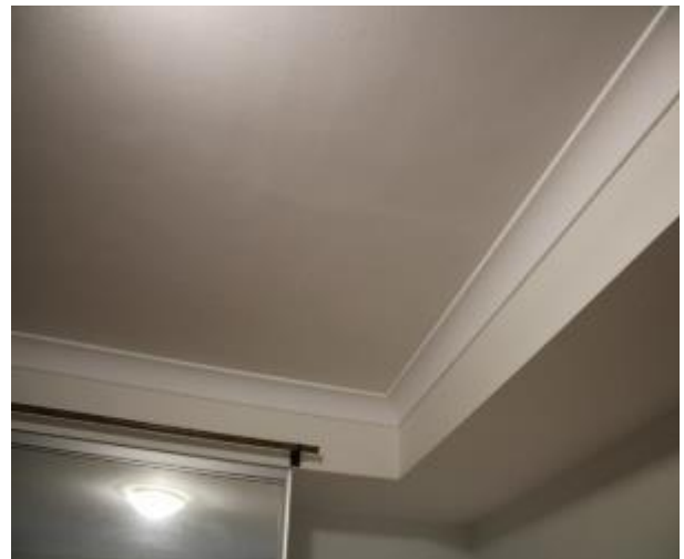
Figure 998 - General condition of study ceiling
