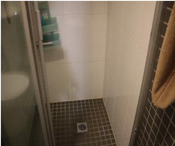
Figure 1007 - General condition of ensuite bathroom internal wall
