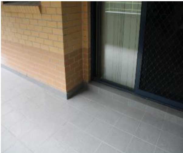
Figure 642 - General condition of external wall
