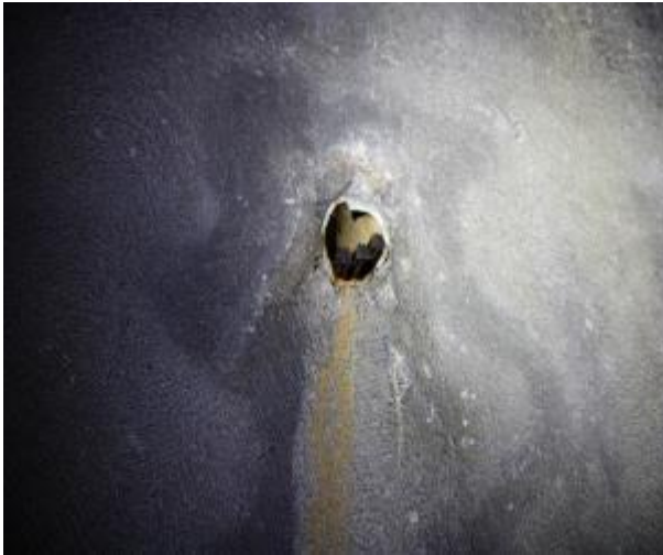
Figure 465 - General condition of basement B2 fire stairs internal wall
