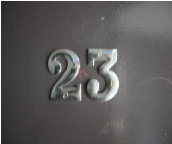
Figure 662 - The following images display the condition of Unit 23
