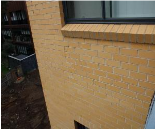
Figure 1320 - General condition of external wall
