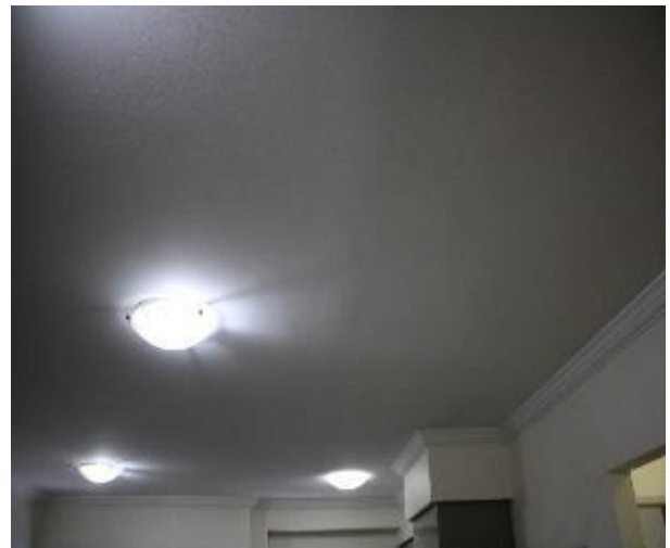
Figure 519 - General condition of open kitchen/ lounge room ceiling
