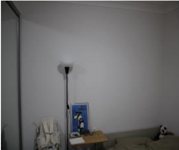
Figure 728 - General condition of bedroom 2 internal wall
