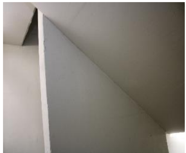
Figure 296 - General condition of level 5 to basement B2 fire stairs internal wall
