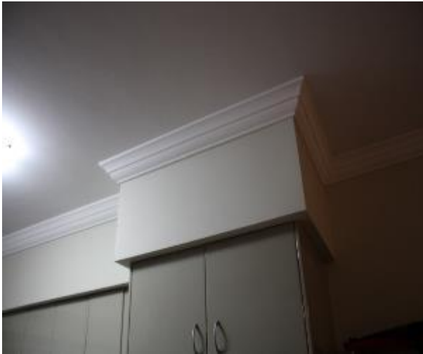
Figure 828 - General condition of open kitchen/ lounge room ceiling
