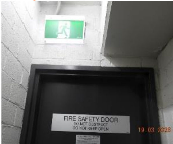
Figure 197 - General condition of B2 to Level 1 fire stairs internal wall
