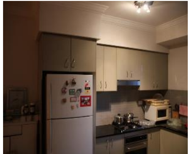
Figure 1113 - General condition of kitchen internal wall
