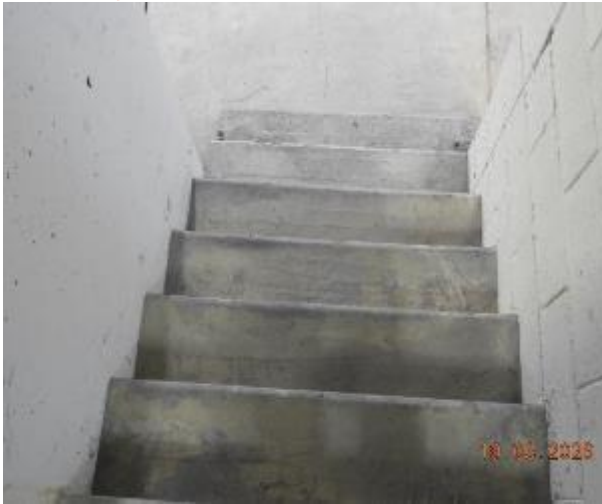
Figure 215 - General condition of B2 to Level 1 fire stairs
