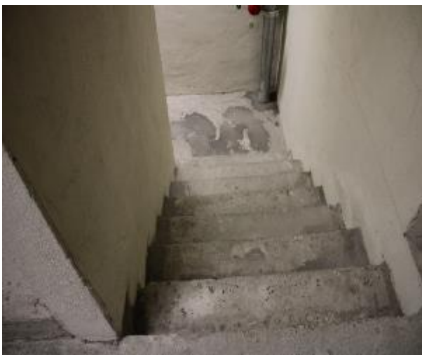
Figure 277 - General condition of level 5 to basement B2 fire stairs
