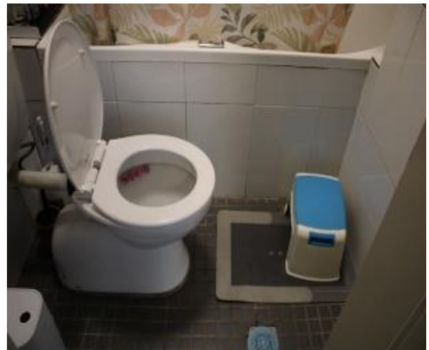
Figure 1373 - General condition of ensuite bathroom floor tiles
