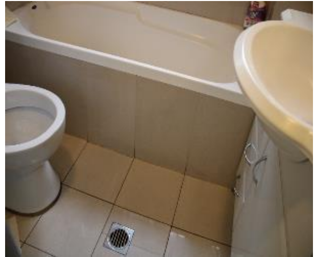
Figure 1183 - General condition of bathroom 1 floor tiles
