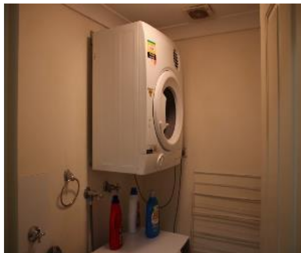
Figure 533 - General condition of laundry internal wall
