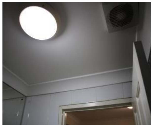
Figure 573 - General condition of ensuite bathroom ceiling
