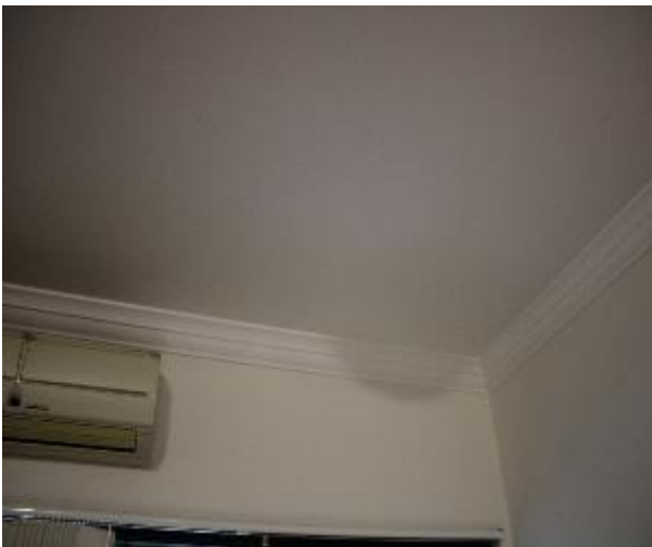
Figure 979 - General condition of lounge room ceiling
