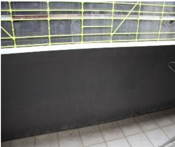
Figure 1238 - General condition of external wall
