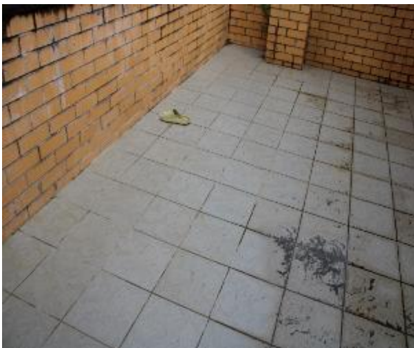
Figure 1394 - General condition of balcony 3 floor tiles
