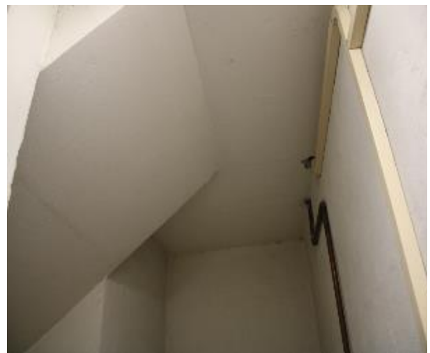
Figure 302 - General condition of level 5 to basement B2 fire stairs underside stairs
