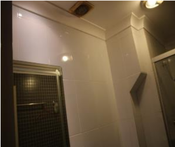
Figure 1146 - General condition of ensuite bathroom internal wall
