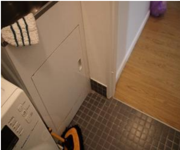
Figure 694 - General condition of laundry internal wall
