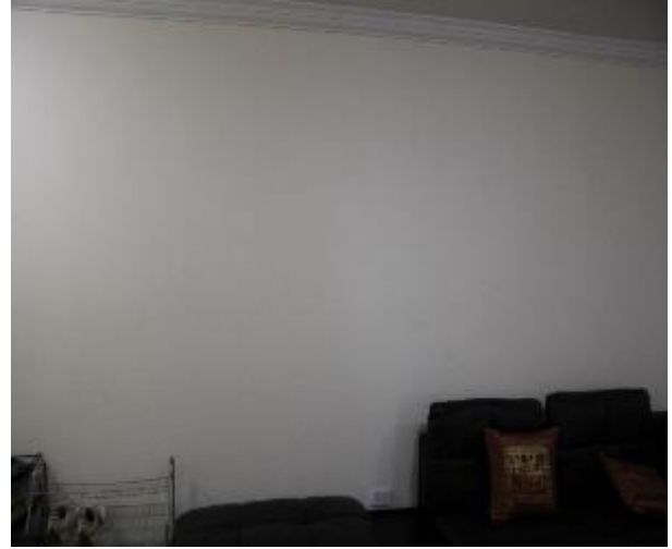
Figure 491 - General condition of open kitchen/ lounge room internal wall
