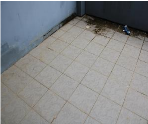
Figure 1292 - General condition of balcony floor tiles
