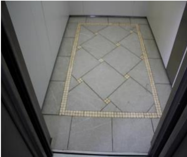
Figure 25 - General condition of level 1 common area floor tiles
