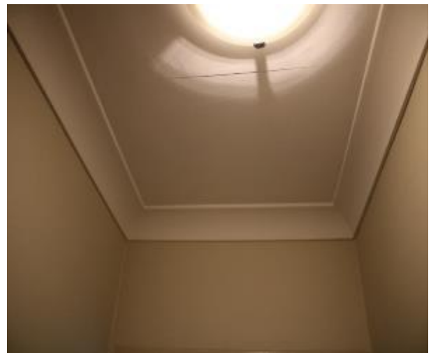
Figure 903 - General condition of corridor ceiling
