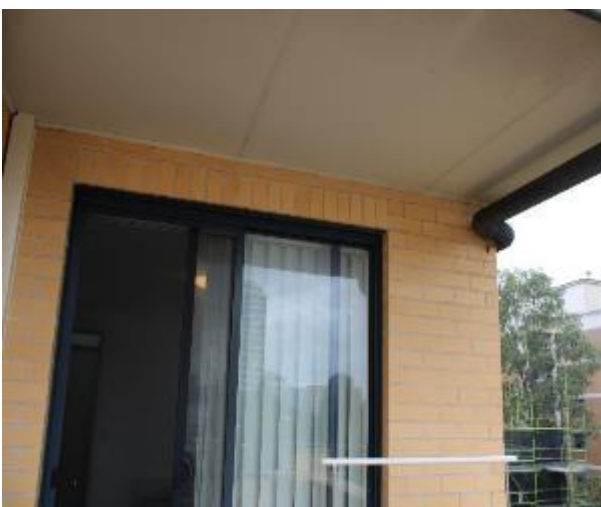
Figure 1402 - General condition of external wall
