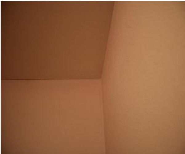
Figure 1136 - General condition of bedroom 1 ceiling
