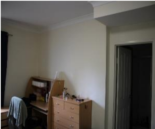
Figure 552 - General condition of bedroom 1 internal wall
