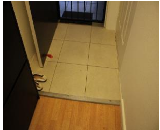
Figure 964 - General condition of entry floor tiles
