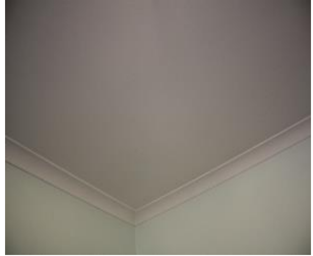
Figure 1207 - General condition of study ceiling
