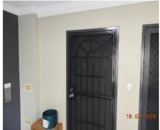
Figure 74 - General condition of level 3 common area internal wall
