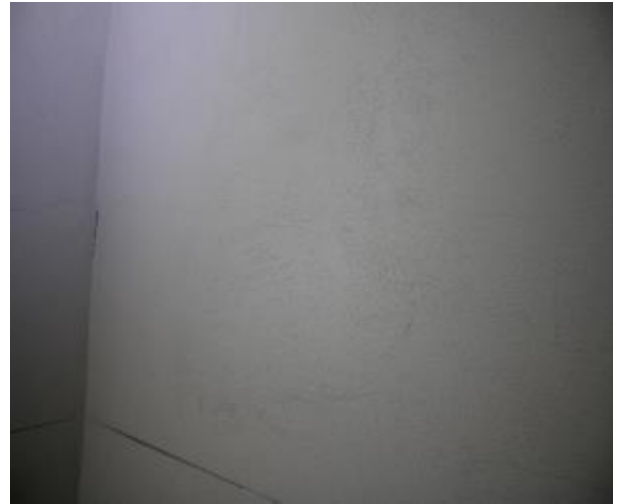
Figure 262 - General condition of level 5 to basement B2 fire stairs internal wall
