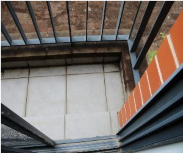
Figure 1386 - General condition of balcony 2 floor tiles
