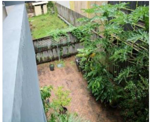
Figure 797 - General condition of boundary fence as seen from Unit 23 balcony
