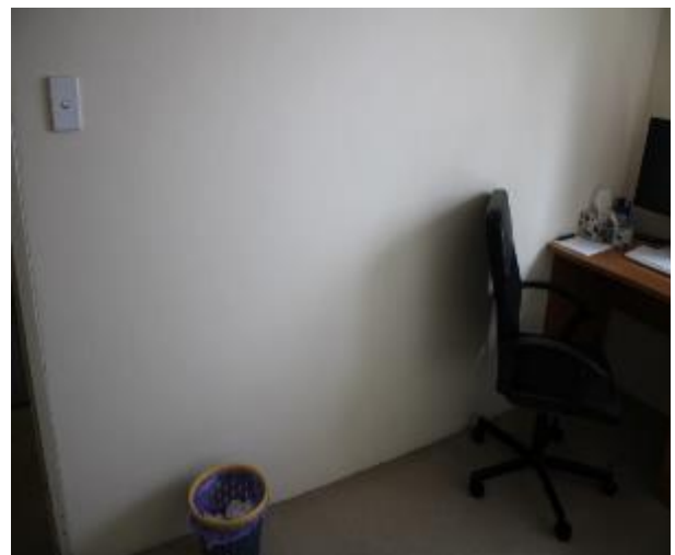
Figure 627 - General condition of bedroom 3 internal wall
