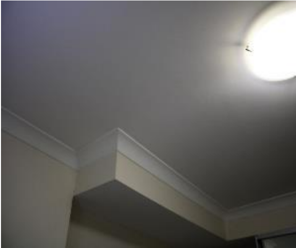
Figure 558 - General condition of bedroom 1 ceiling
