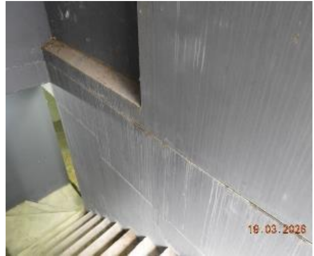
Figure 162 - General condition of B2 to Level 1 fire stairs internal wall
