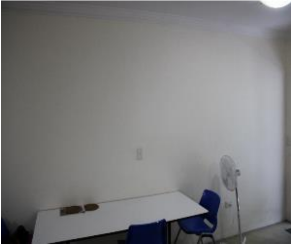
Figure 492 - General condition of open kitchen/ lounge room internal wall
