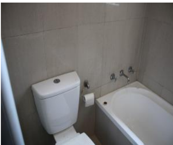
Figure 1536 - General condition of bathroom 1 internal wall
