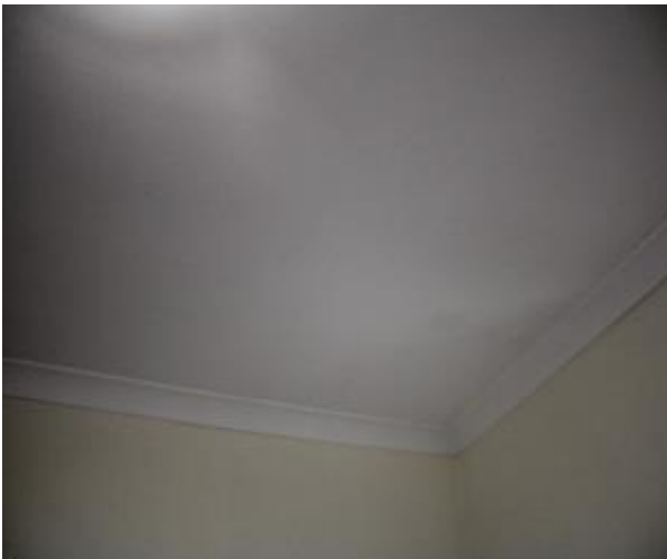
Figure 600 - General condition of bedroom 2 ceiling
