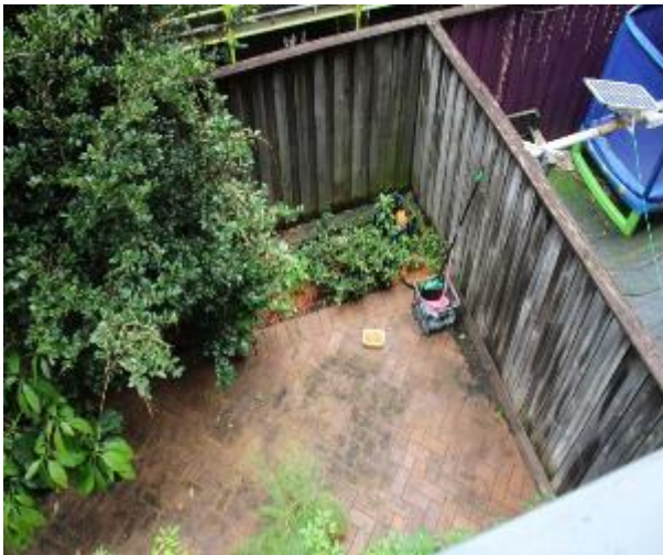
Figure 796 - General condition of boundary fence as seen from Unit 23 balcony
