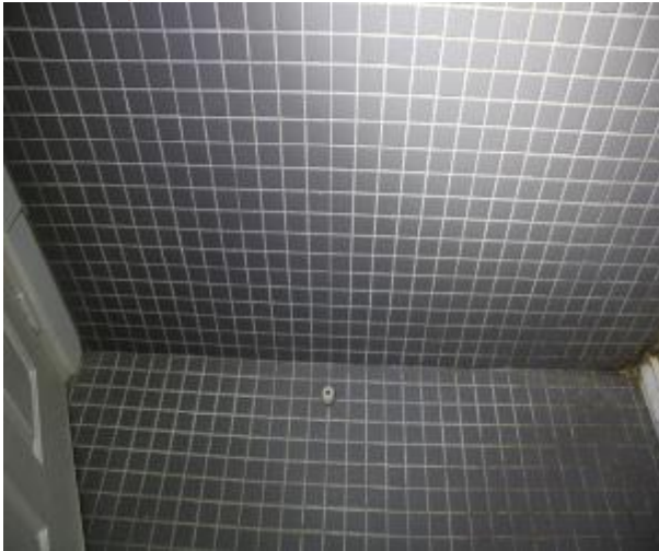
Figure 568 - General condition of ensuite bathroom internal wall
