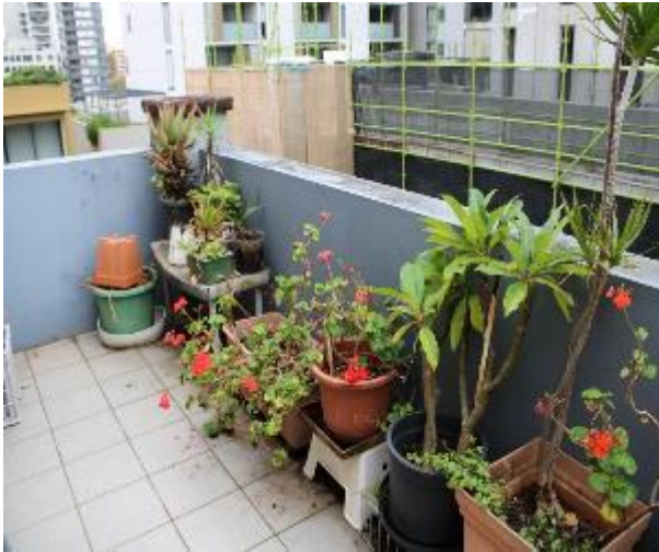
Figure 1586 - General condition of external wall
