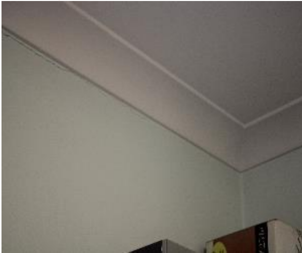
Figure 1200 - General condition of study internal wall
