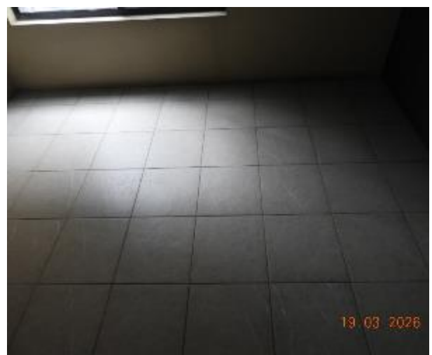
Figure 30 - General condition of level 2 common area floor tiles
