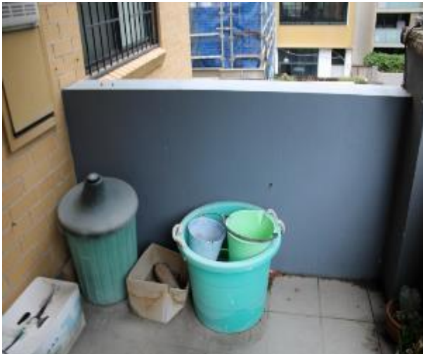
Figure 1073 - General condition of external wall
