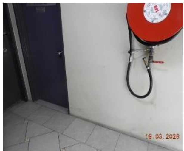
Figure 18 - General condition of level 1 common area internal wall
