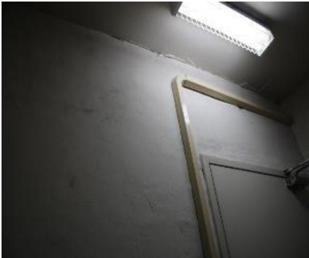
Figure 233 - General condition of level 5 to basement B2 fire stairs internal wall
