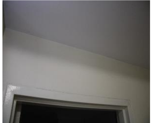
Figure 559 - General condition of bedroom 1 ceiling
