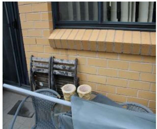
Figure 1571 - General condition of external wall
