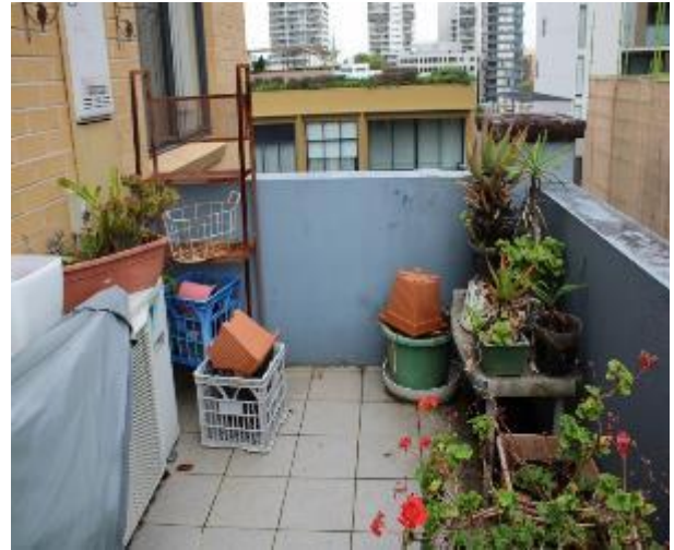
Figure 1587 - General condition of external wall
