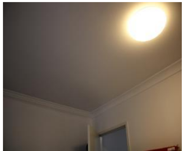
Figure 1289 - General condition of bedroom 1 ceiling
