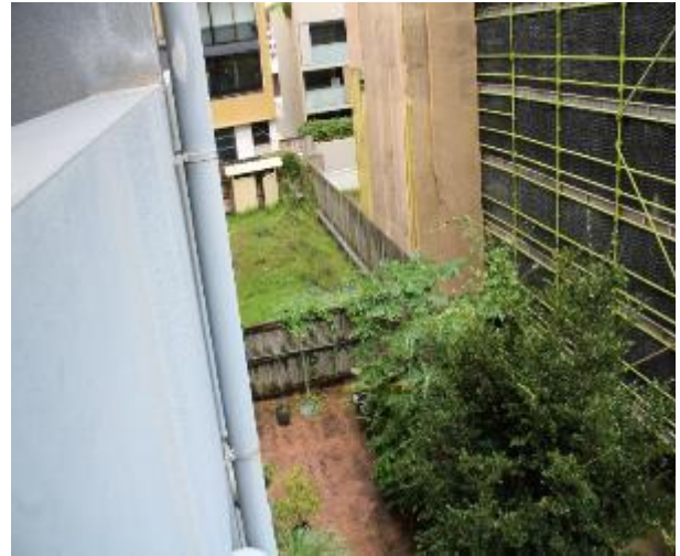
Figure 961 - General condition of boundary fence as seen from Unit 24 balcony
