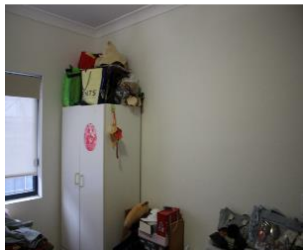
Figure 1052 - General condition of bedroom 2 internal wall
