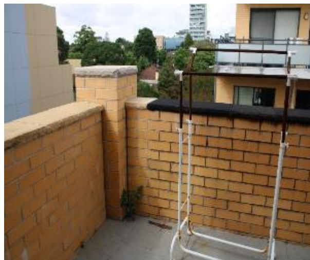
Figure 1405 - General condition of external wall
