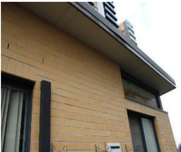
Figure 1570 - General condition of external wall
