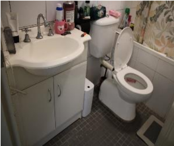
Figure 1374 - General condition of ensuite bathroom internal wall
