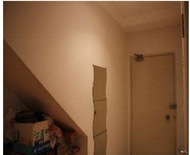
Figure 1083 - General condition of lounge room internal wall
