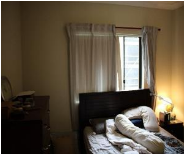
Figure 854 - General condition of bedroom 1 internal wall
