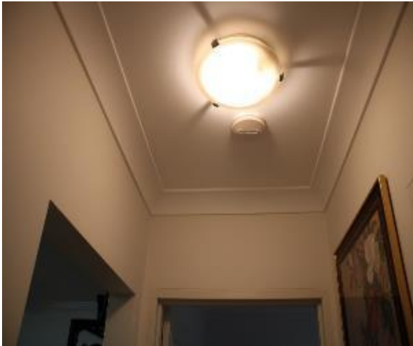
Figure 1017 - General condition of corridor ceiling
