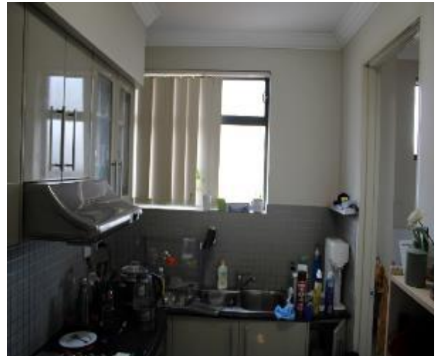
Figure 1421 - General condition of kitchen internal wall
