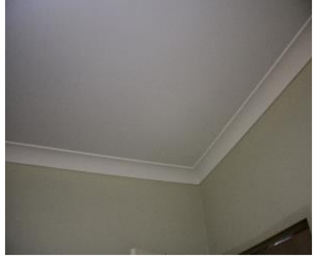
Figure 889 - General condition of bedroom 2 ceiling
