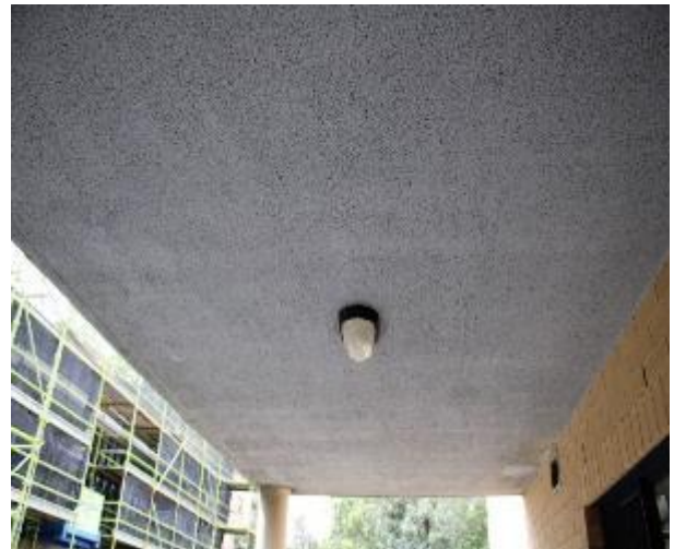
Figure 659 - General condition of balcony underside slab
