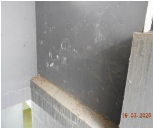
Figure 163 - General condition of B2 to Level 1 fire stairs internal wall
