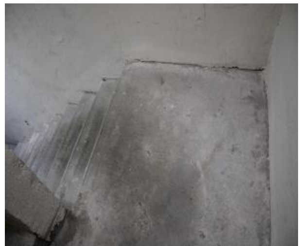
Figure 356 - General condition of level 5 to basement B2 fire stairs
