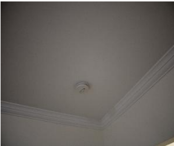
Figure 518 - General condition of open kitchen/ lounge room ceiling
