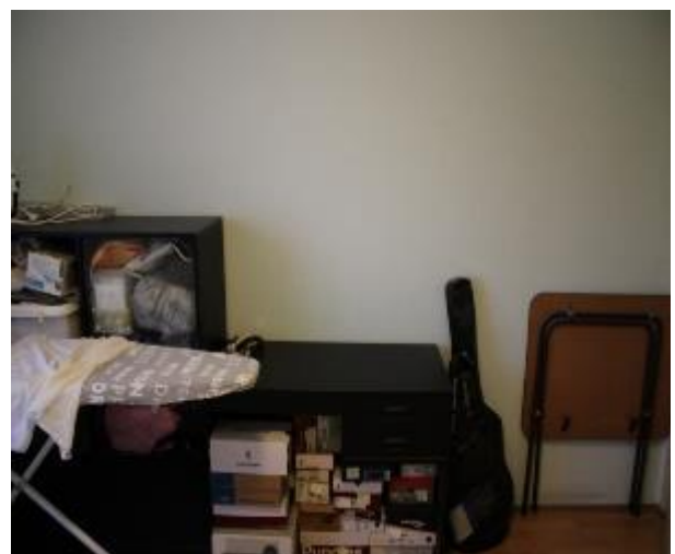
Figure 1175 - General condition of bedroom 2 internal wall
