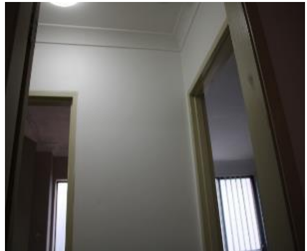
Figure 1323 - General condition of corridor internal wall
