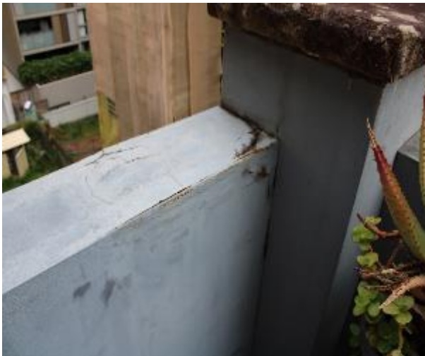
Figure 1588 - General condition of external wall
