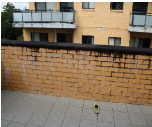
Figure 1408 - General condition of external wall
