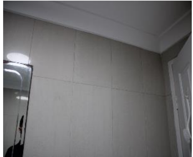
Figure 753 - General condition of bathroom 1 internal wall
