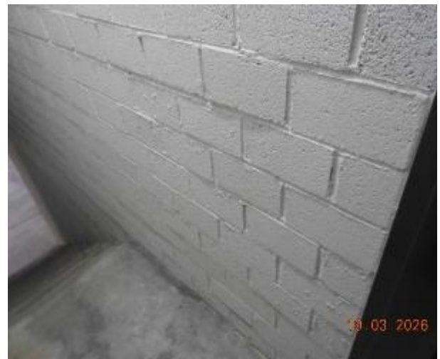
Figure 200 - General condition of B2 to Level 1 fire stairs internal wall
