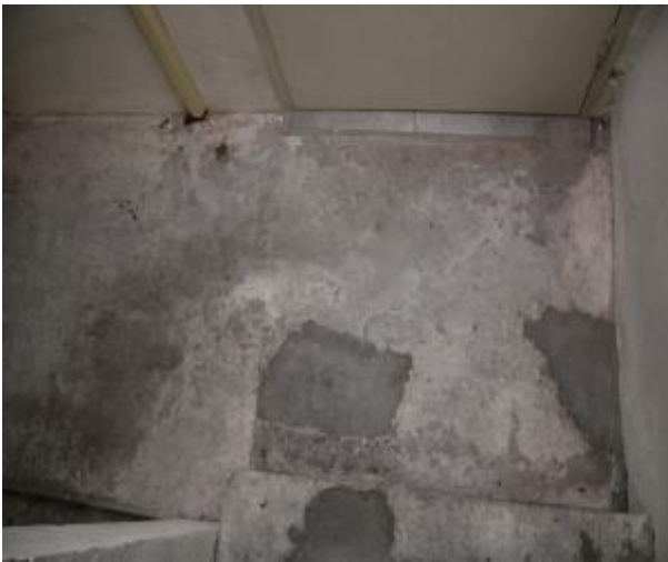
Figure 329 - General condition of level 5 to basement B2 fire stairs
