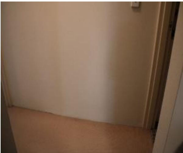
Figure 892 - General condition of corridor internal wall
