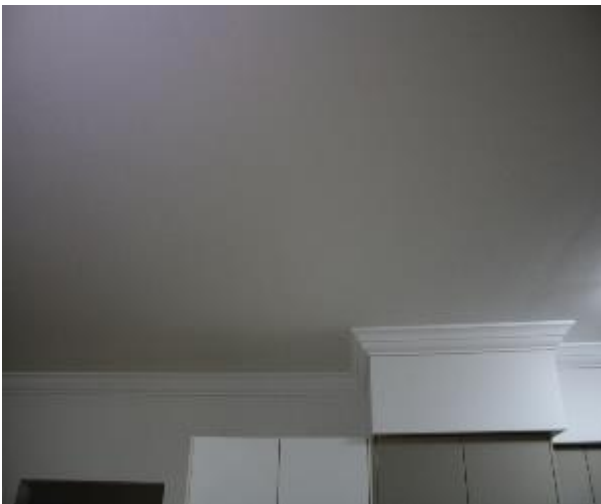
Figure 684 - General condition of kitchen ceiling
