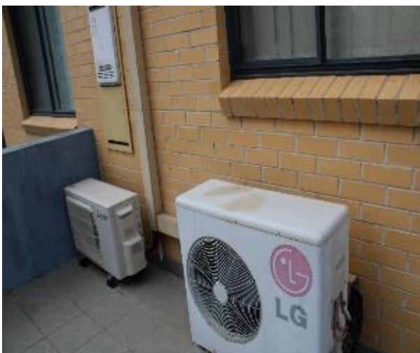
Figure 1300 - General condition of external wall
