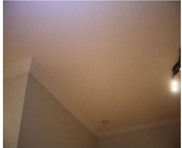
Figure 1107 - General condition of lounge room ceiling
