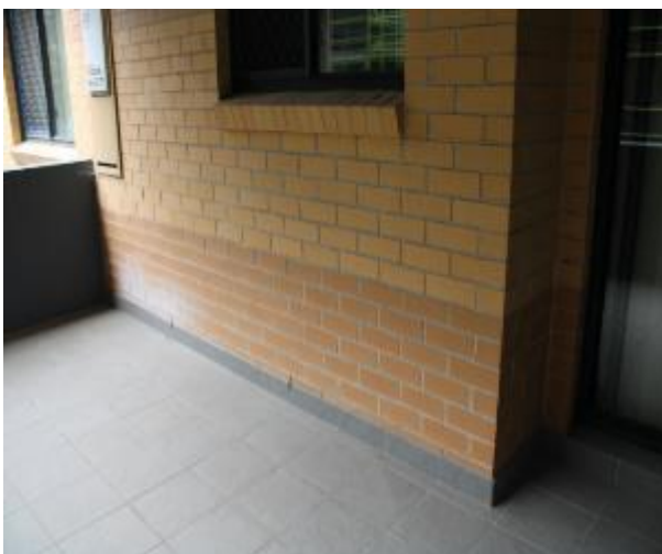
Figure 638 - General condition of external wall
