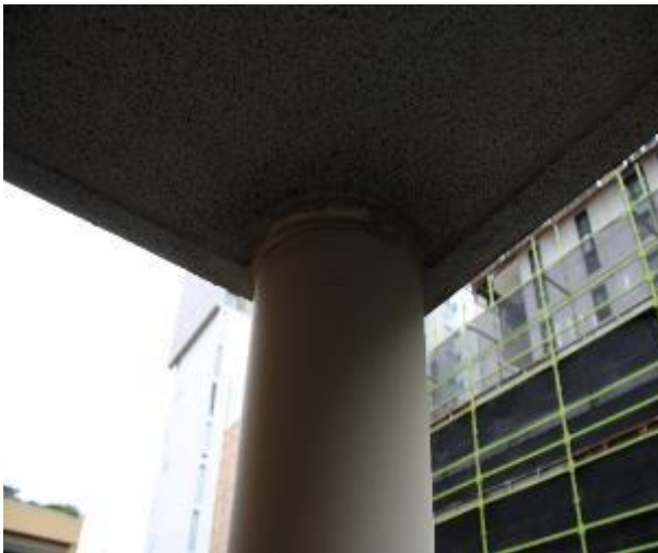
Figure 790 - General condition of external wall
