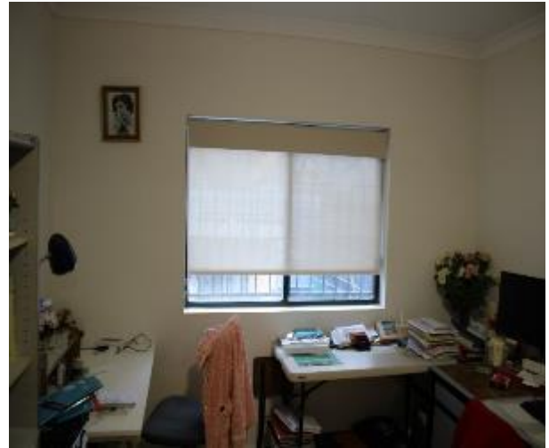
Figure 994 - General condition of study internal wall
