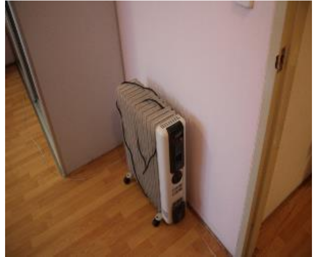
Figure 1125 - General condition of bedroom 1 internal wall
