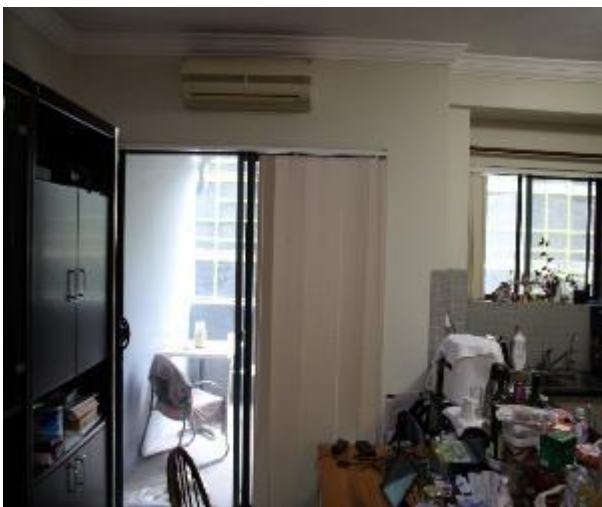
Figure 814 - General condition of open kitchen/ lounge room internal wall
