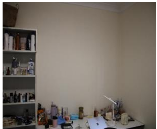
Figure 591 - General condition of bedroom 2 internal wall
