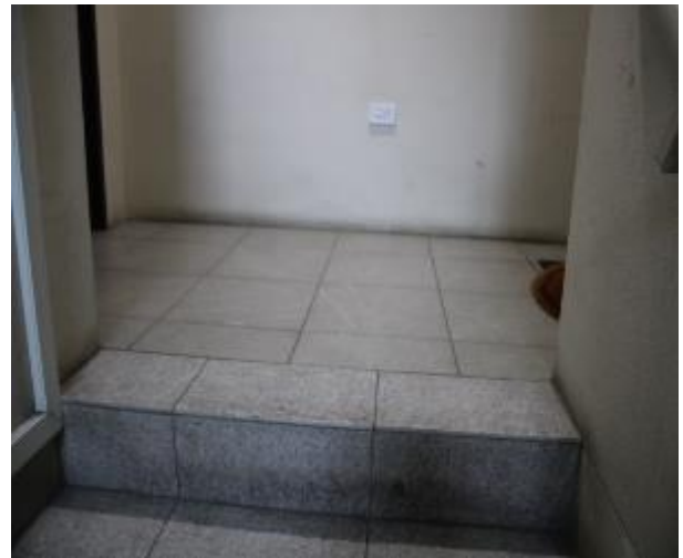
Figure 136 - General condition of level 5 common area floor tiles
