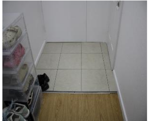
Figure 663 - General condition of entry floor tiles
