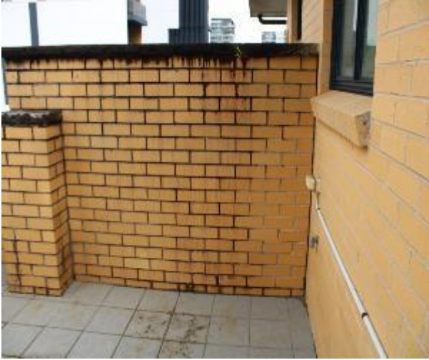
Figure 1410 - General condition of external wall
