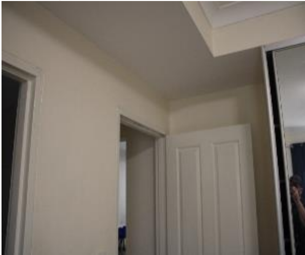
Figure 550 - General condition of bedroom 1 internal wall
