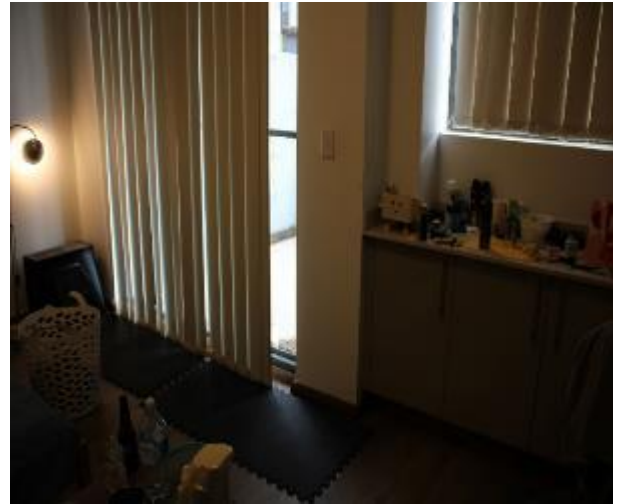
Figure 1285 - General condition of bedroom 1 internal wall
