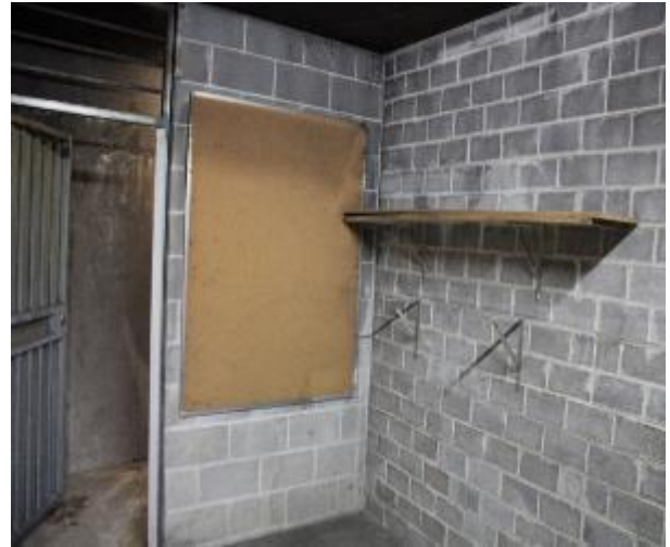
Figure 442 - General condition of basement B2 fire stairs internal wall
