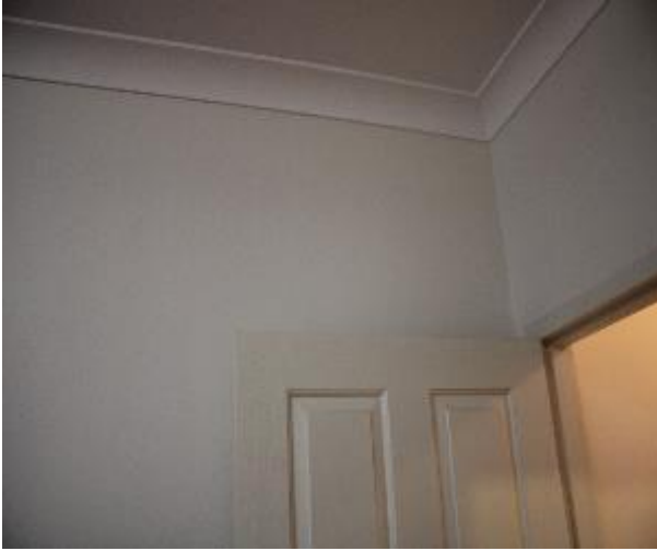
Figure 1023 - General condition of bedroom 1 internal wall
