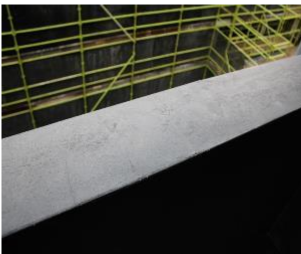
Figure 1222 - Crack propagation through external wall
