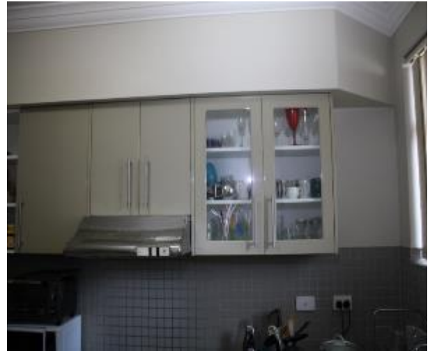
Figure 1425 - General condition of kitchen internal wall
