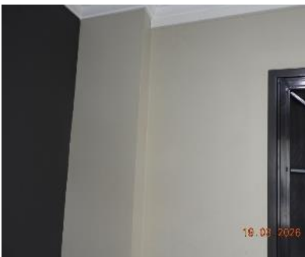
Figure 77 - General condition of level 3 common area internal wall
