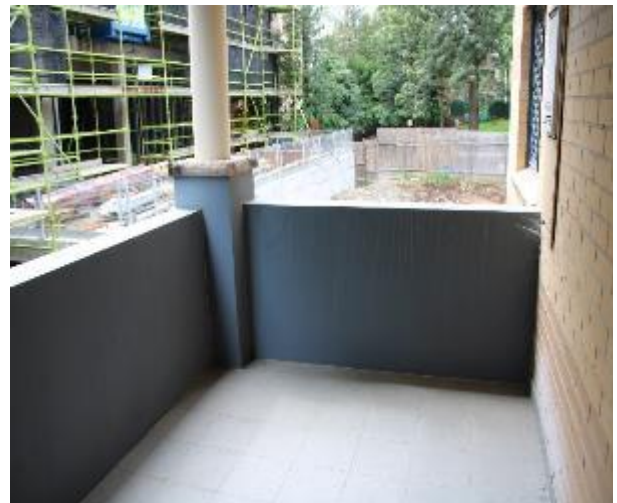
Figure 645 - General condition of external wall
