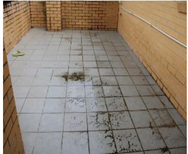
Figure 1393 - General condition of balcony 3 floor tiles
