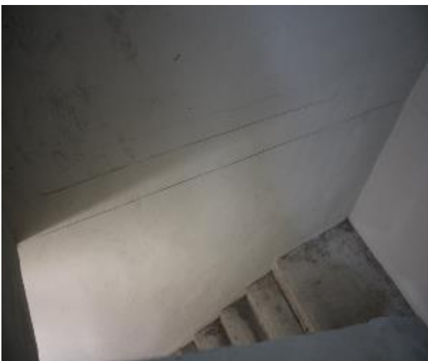
Figure 253 - General condition of level 5 to basement B2 fire stairs internal wall
