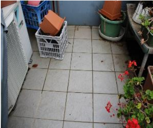
Figure 1568 - General condition of balcony 3 floor tiles
