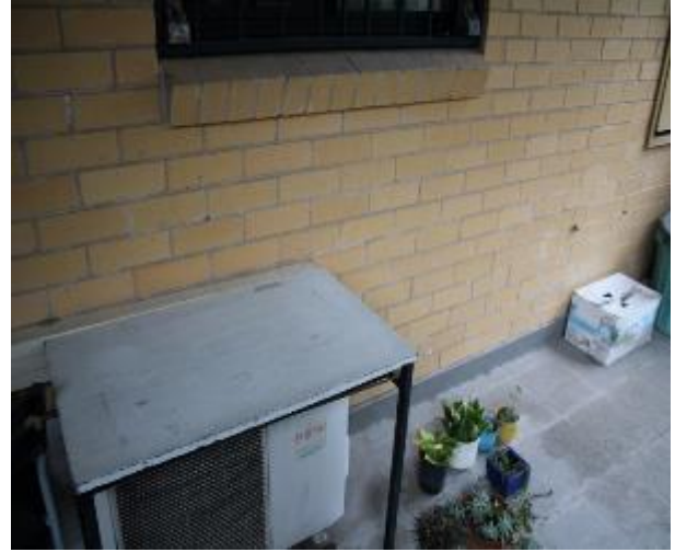
Figure 1060 - General condition of external wall
