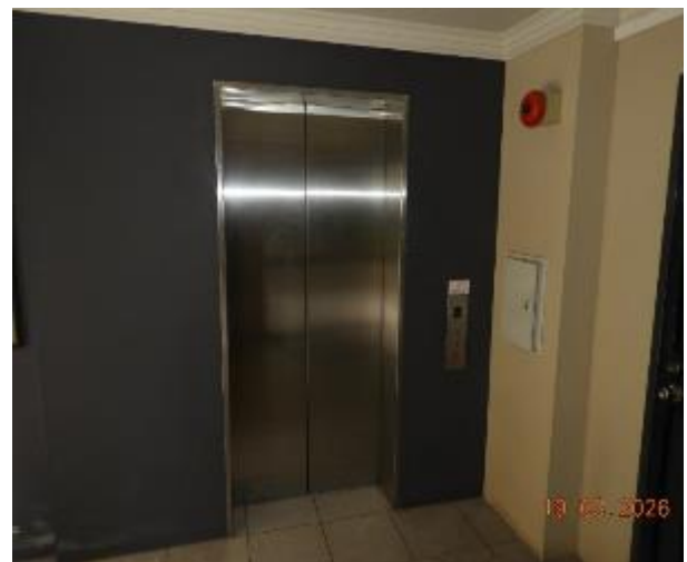
Figure 6 - General condition of level 1 common area internal wall
