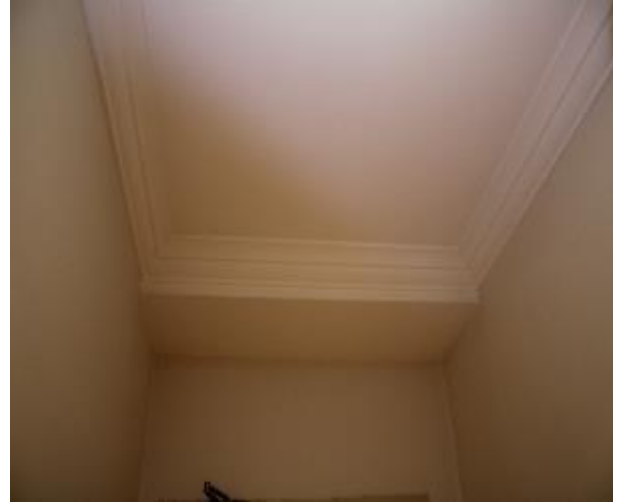
Figure 1105 - General condition of lounge room ceiling
