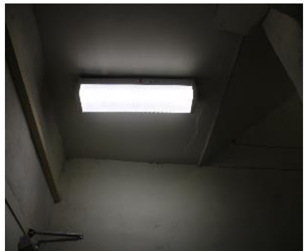
Figure 350 - General condition of level 5 to basement B2 fire stairs underside stairs
