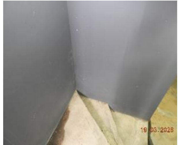
Figure 174 - General condition of B2 to Level 1 fire stairs internal wall
