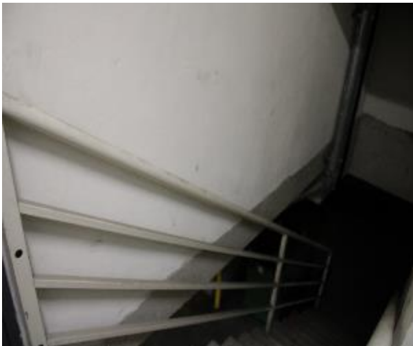
Figure 407 - General condition of level 5 to basement B2 fire stairs internal wall
