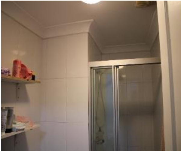
Figure 710 - General condition of ensuite bathroom internal wall
