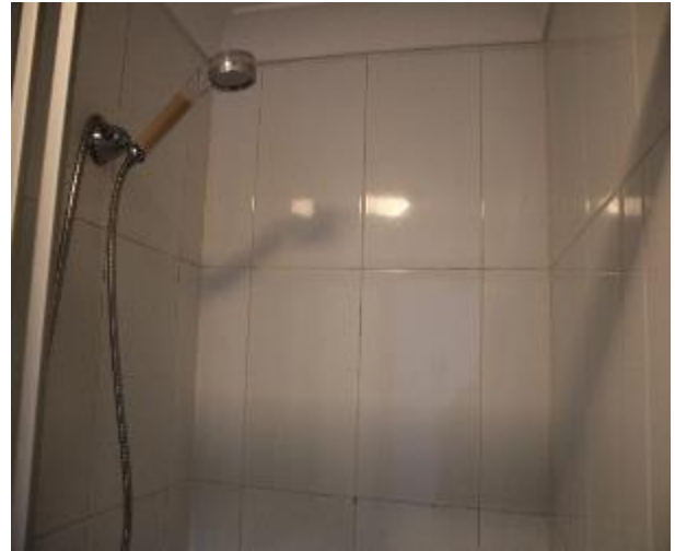
Figure 717 - General condition of ensuite bathroom internal wall
