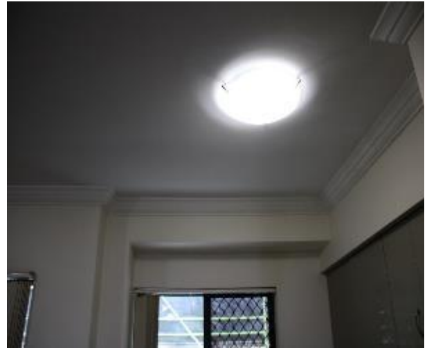
Figure 521 - General condition of open kitchen/ lounge room ceiling
