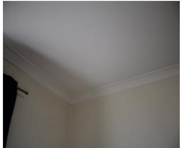
Figure 553 - General condition of bedroom 1 ceiling
