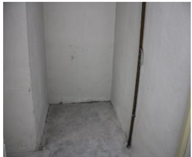
Figure 336 - General condition of level 5 to basement B2 fire stairs internal wall
