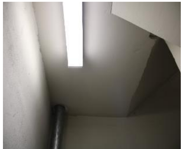
Figure 324 - General condition of level 5 to basement B2 fire stairs underside stairs
