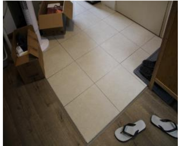
Figure 1249 - General condition of kitchen floor tiles
