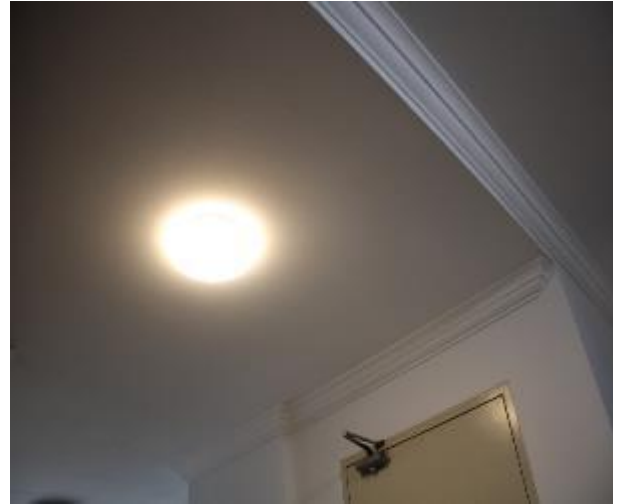
Figure 1257 - General condition of kitchen ceiling
