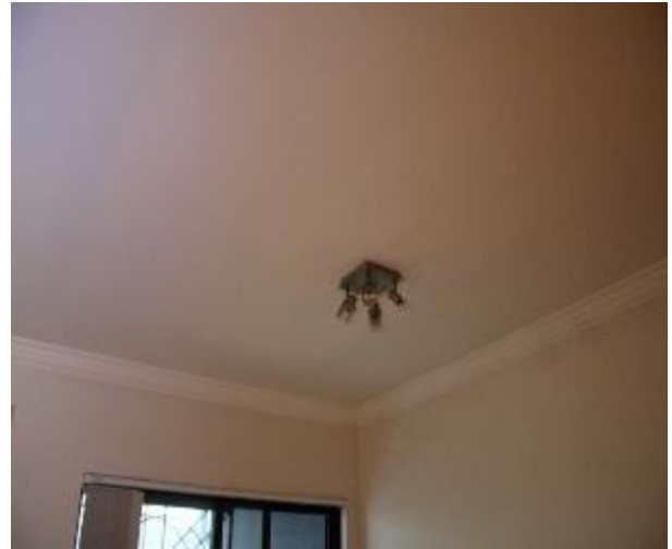
Figure 1111 - General condition of lounge room ceiling
