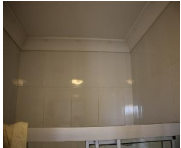
Figure 1499 - General condition of ensuite bathroom internal wall
