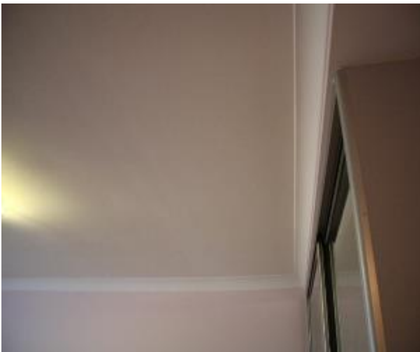
Figure 1138 - General condition of bedroom 1 ceiling
