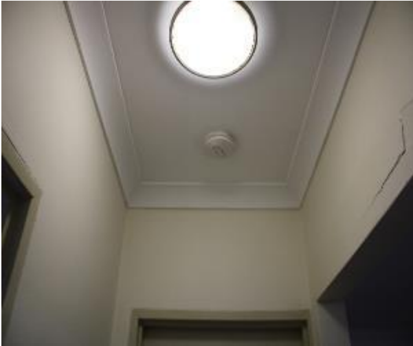
Figure 582 - General condition of corridor ceiling
