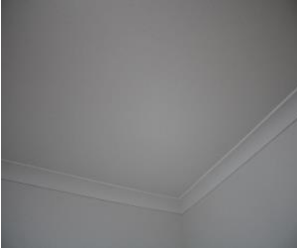
Figure 734 - General condition of bedroom 2 ceiling
