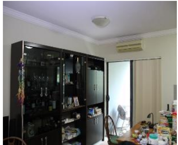
Figure 813 - General condition of open kitchen/ lounge room internal wall
