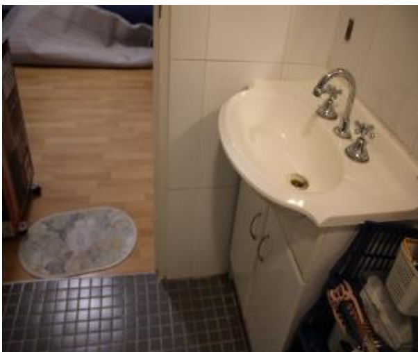
Figure 1009 - General condition of ensuite bathroom internal wall
