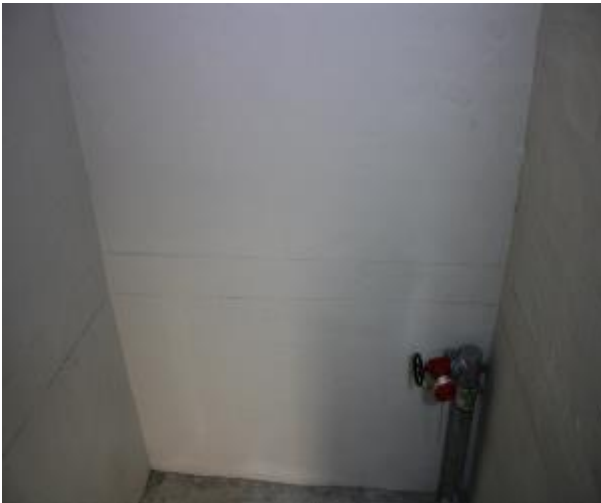
Figure 251 - General condition of level 5 to basement B2 fire stairs internal wall
