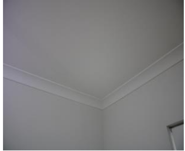
Figure 735 - General condition of bedroom 2 ceiling
