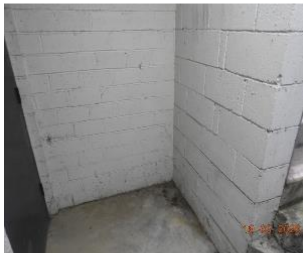
Figure 186 - General condition of B2 to Level 1 fire stairs internal wall
