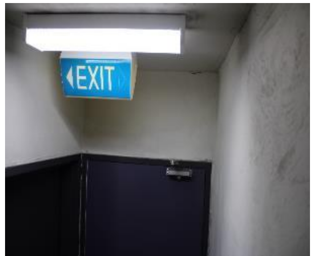
Figure 384 - General condition of level 5 to basement B2 fire stairs internal wall
