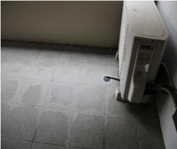
Figure 772 - General condition of balcony floor tiles
