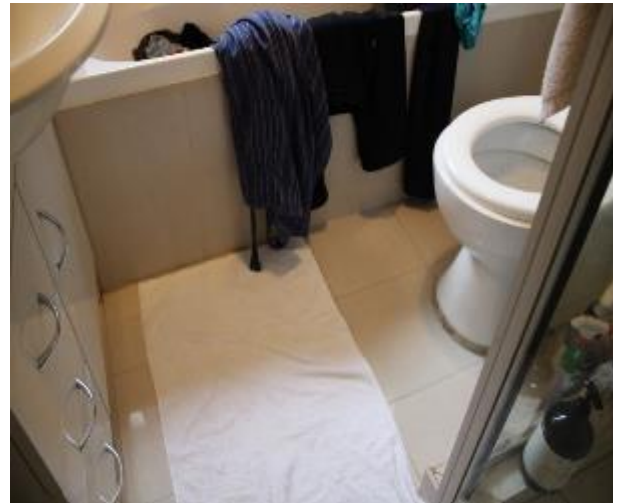
Figure 837 - General condition of bathroom 1 floor tiles
