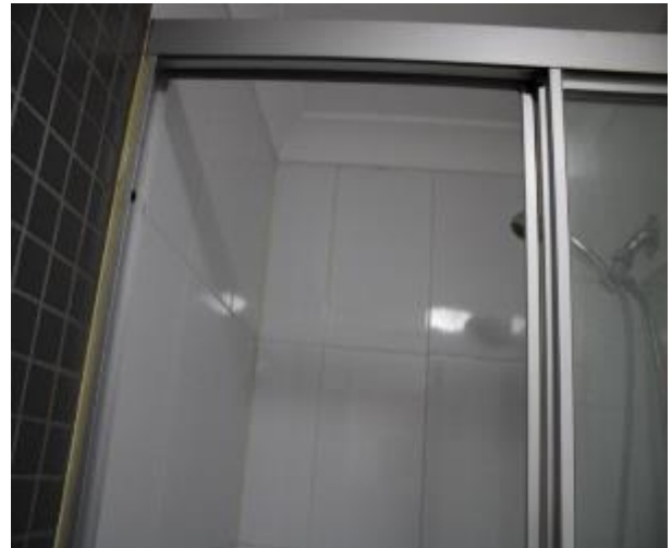
Figure 571 - General condition of ensuite bathroom internal wall
