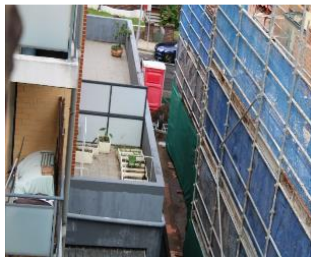
Figure 1531 - General condition of boundary as seen from Unit 29 balcony 2
