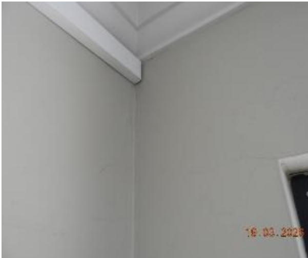
Figure 15 - General condition of level 1 common area internal wall
