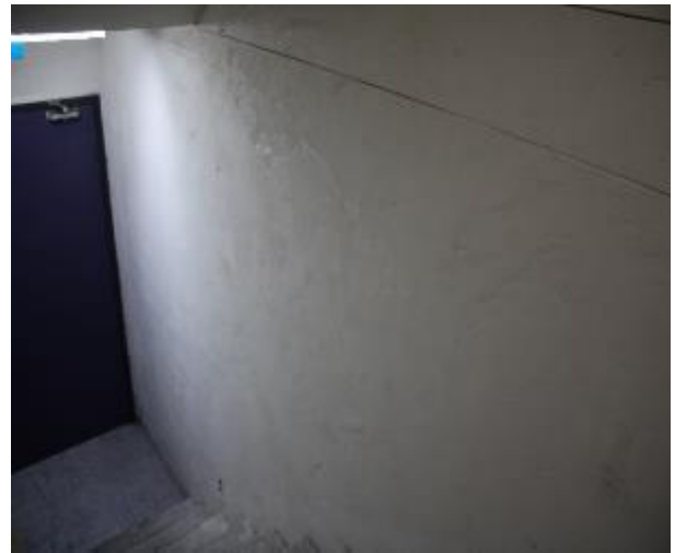
Figure 372 - General condition of level 5 to basement B2 fire stairs internal wall
