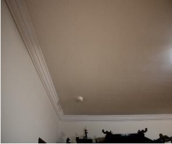
Figure 975 - General condition of lounge room ceiling
