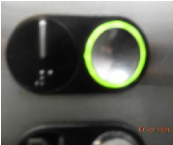
Figure 1 - The following images display the condition of Level 1 Common Area
