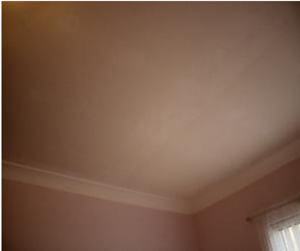
Figure 1140 - General condition of bedroom 1 ceiling
