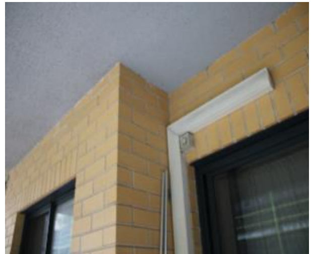
Figure 945 - General condition of external wall
