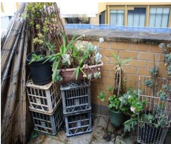
Figure 1524 - General condition of external wall
