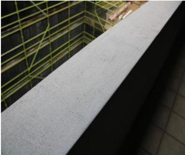
Figure 1242 - Crack propagation through external wall
