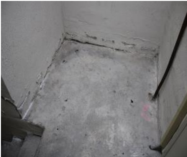
Figure 221 - General condition of level 5 to basement B2 fire stairs
