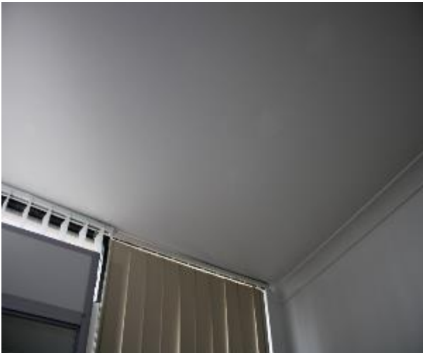
Figure 1342 - General condition of study ceiling
