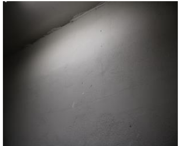
Figure 366 - General condition of level 5 to basement B2 fire stairs internal wall
