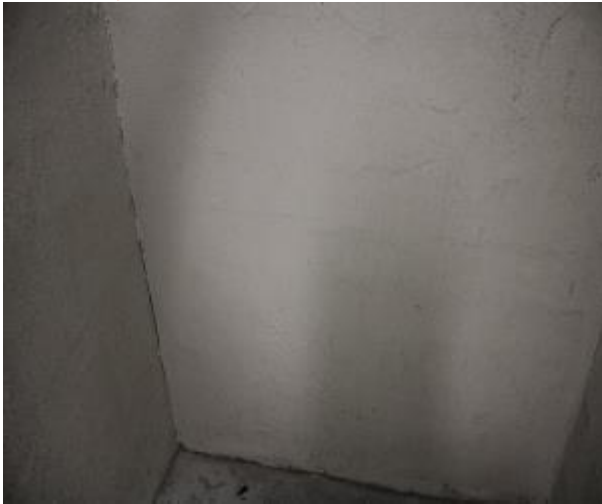
Figure 291 - General condition of level 5 to basement B2 fire stairs internal wall
