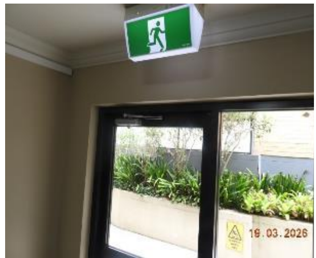
Figure 12 - General condition of level 1 common area internal wall
