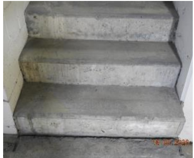
Figure 218 - General condition of B2 to Level 1 fire stairs
