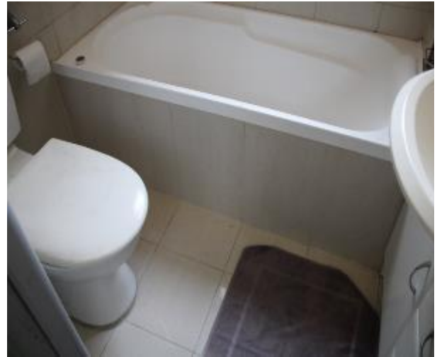
Figure 1533 - General condition of bathroom 1 floor tiles
