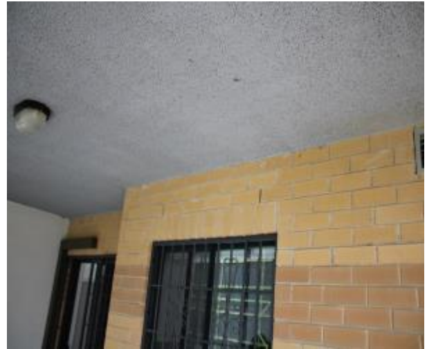
Figure 777 - General condition of external wall
