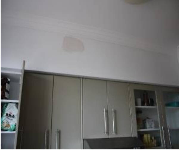
Figure 1254 - General condition of kitchen internal wall
