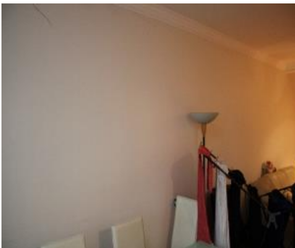
Figure 1102 - General condition of lounge room internal wall
