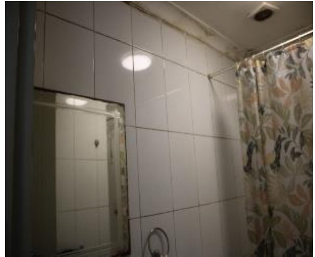
Figure 1375 - General condition of ensuite bathroom internal wall
