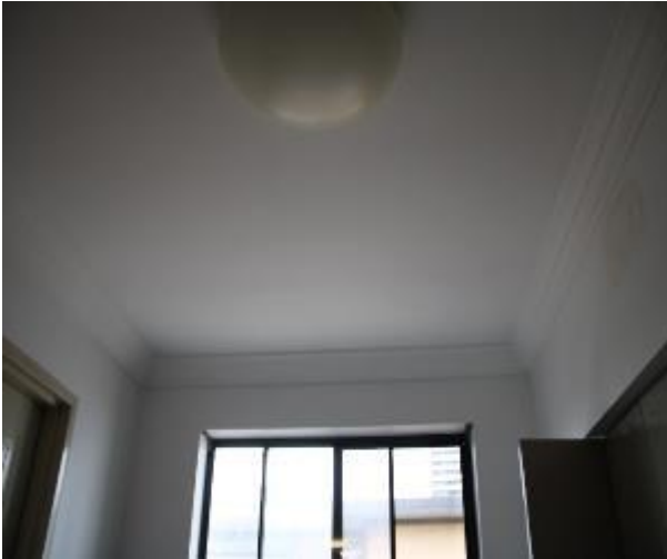
Figure 1256 - General condition of kitchen ceiling
