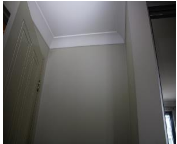
Figure 1481 - General condition of bedroom 1 internal wall
