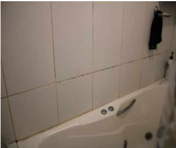
Figure 1376 - General condition of ensuite bathroom internal wall
