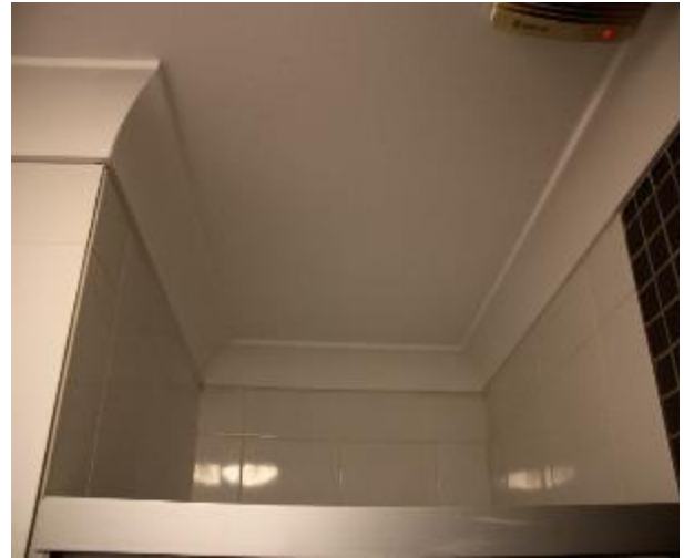
Figure 1012 - General condition of ensuite bathroom ceiling
