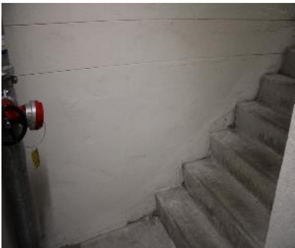
Figure 359 - General condition of level 5 to basement B2 fire stairs internal wall
