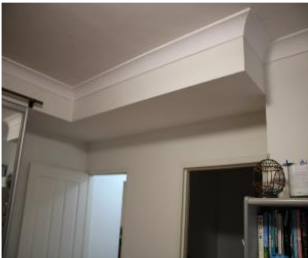
Figure 997 - General condition of study internal wall
