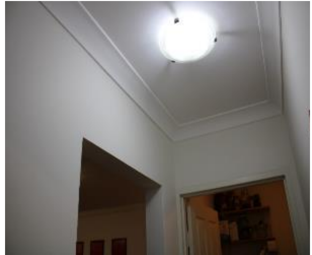
Figure 988 - General condition of corridor internal wall
