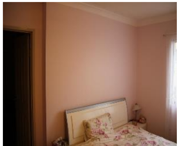
Figure 1133 - General condition of bedroom 1 internal wall
