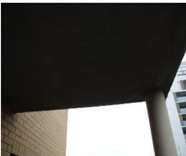
Figure 1246 - General condition of balcony underside slab
