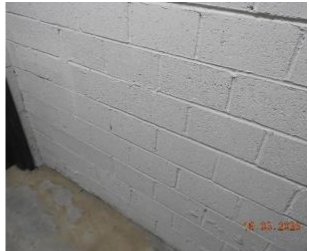
Figure 198 - General condition of B2 to Level 1 fire stairs internal wall
