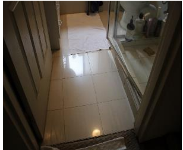
Figure 835 - General condition of bathroom 1 floor tiles
