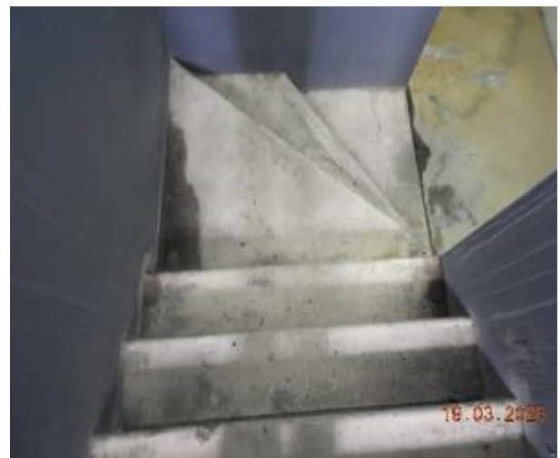
Figure 172 - General condition of B2 to Level 1 fire stairs
