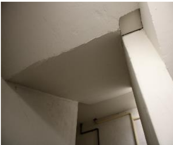
Figure 323 - General condition of level 5 to basement B2 fire stairs underside stairs
