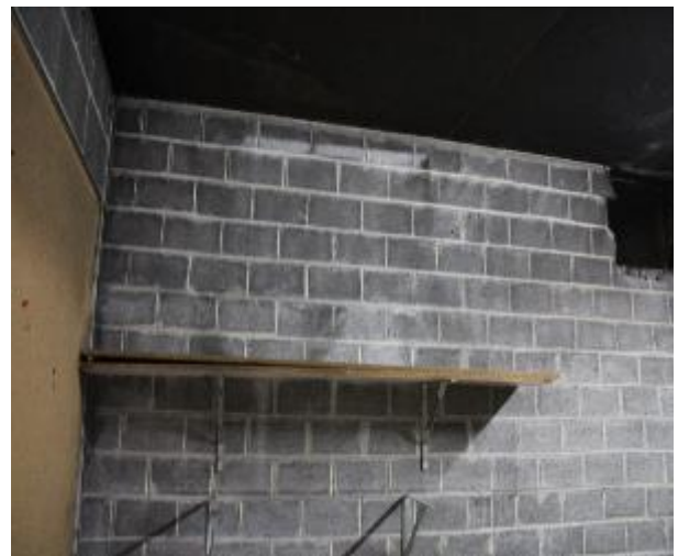
Figure 444 - General condition of basement B2 fire stairs internal wall
