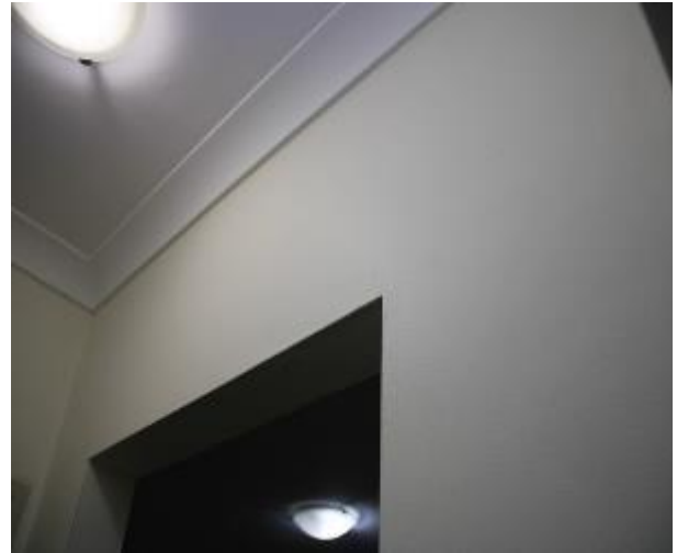
Figure 527 - General condition of corridor internal wall
