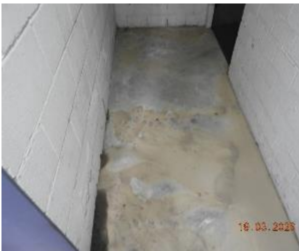
Figure 177 - General condition of B2 to Level 1 fire stairs pavement slab
