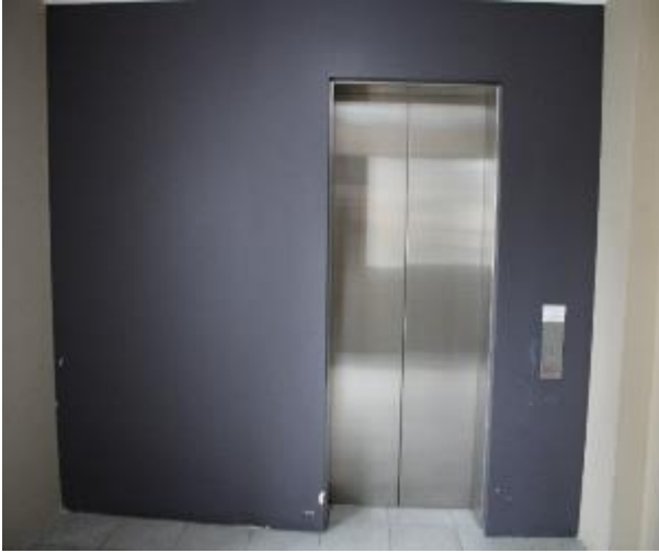
Figure 91 - General condition of level 4 common area internal wall
