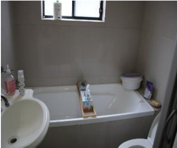
Figure 604 - General condition of bathroom 1 internal wall
