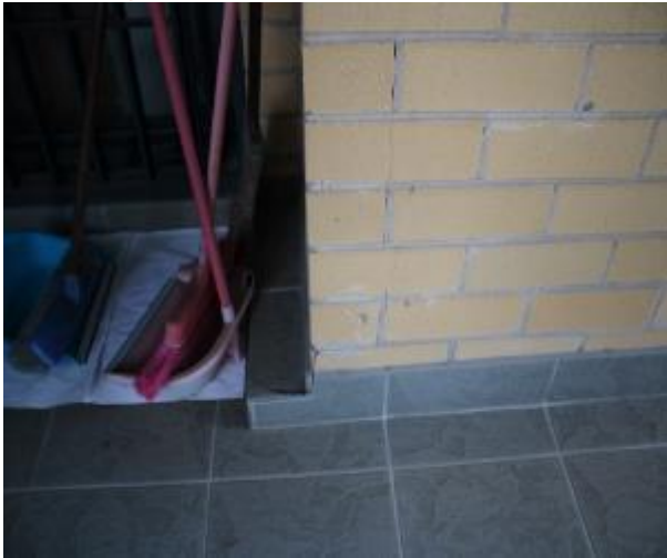
Figure 1230 - Crack propagation through external wall
