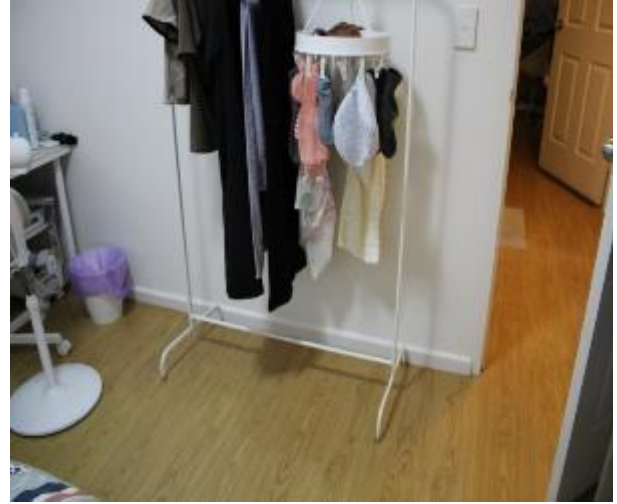
Figure 765 - General condition of bedroom 3 internal wall
