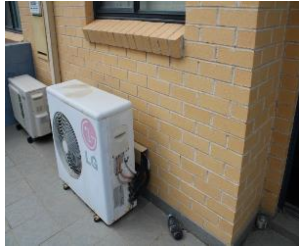
Figure 1297 - General condition of external wall
