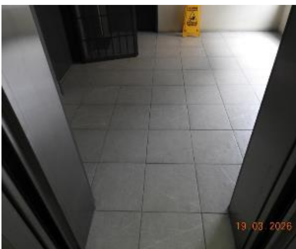
Figure 29 - General condition of level 2 common area floor tiles
