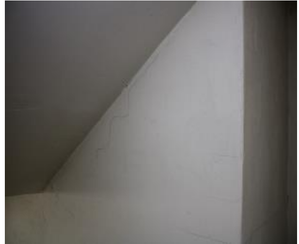
Figure 300 - General condition of level 5 to basement B2 fire stairs internal wall
