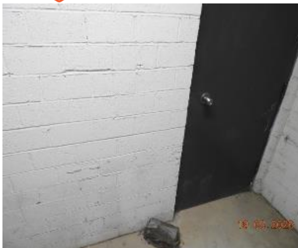
Figure 185 - General condition of B2 to Level 1 fire stairs internal wall
