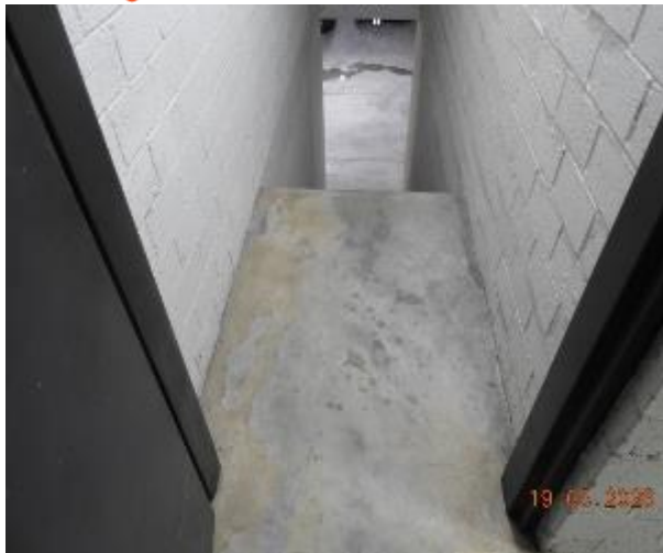
Figure 191 - General condition of B2 to Level 1 fire stairs pavement slab
