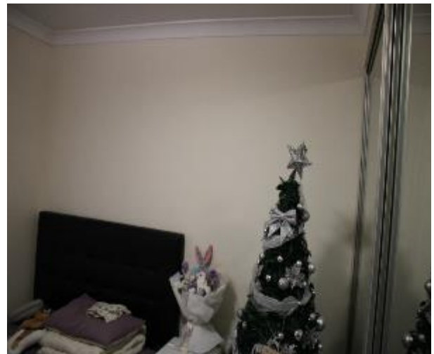
Figure 585 - General condition of bedroom 2 internal wall
