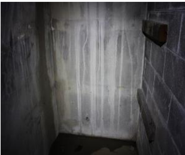
Figure 473 - General condition of basement B2 fire stairs internal wall
