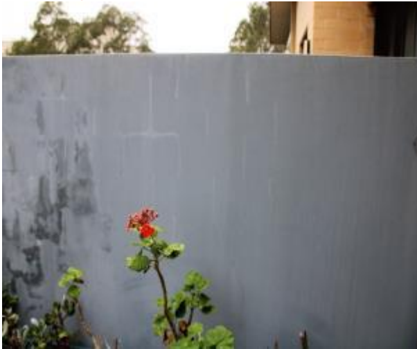
Figure 1580 - General condition of external wall
