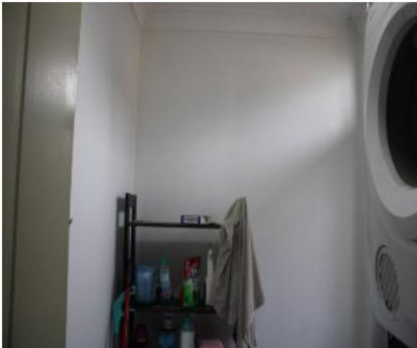
Figure 1262 - General condition of laundry internal wall
