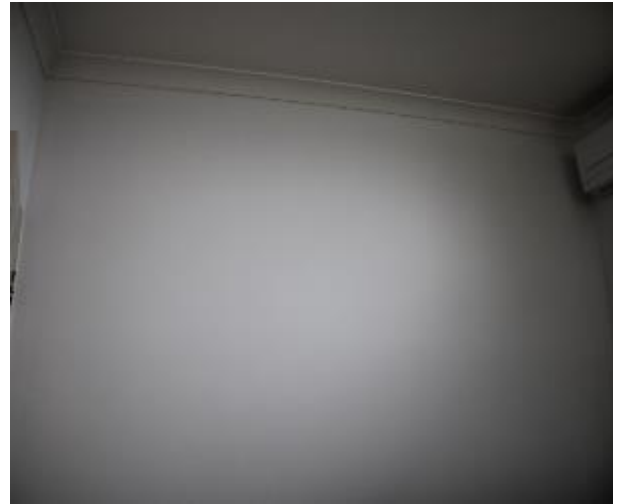
Figure 1333 - General condition of study internal wall
