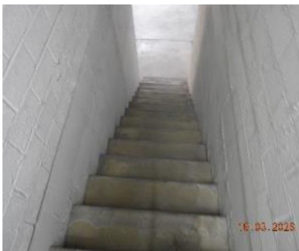
Figure 213 - General condition of B2 to Level 1 fire stairs
