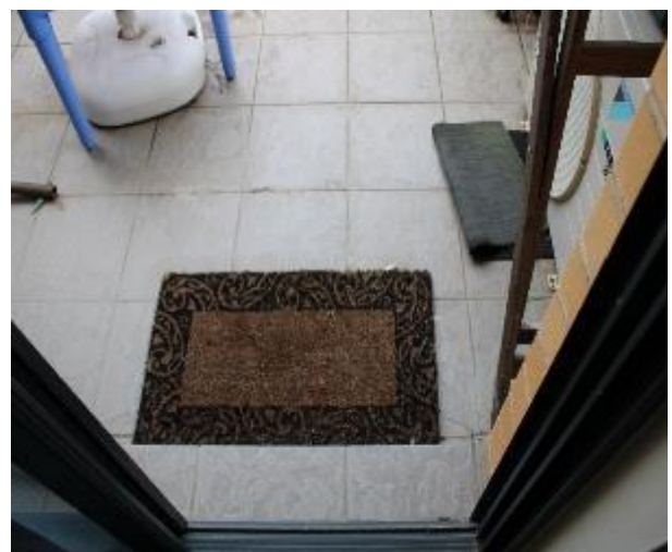
Figure 1513 - General condition of balcony 2 floor tiles
