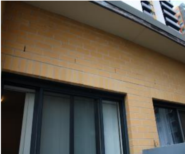
Figure 1296 - General condition of external wall
