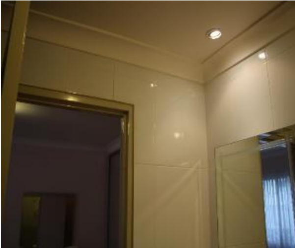
Figure 1154 - General condition of ensuite bathroom internal wall
