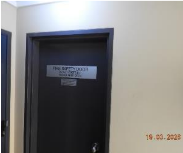
Figure 43 - General condition of level 2 common area internal wall
