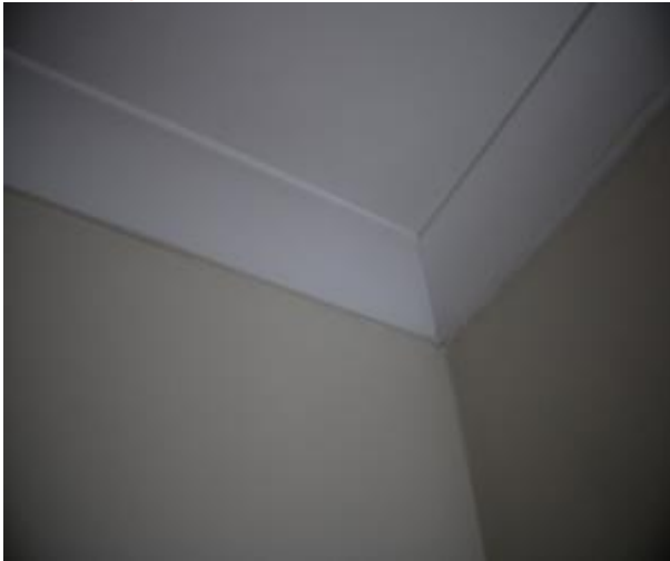
Figure 634 - General condition of bedroom 3 ceiling
