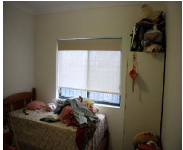
Figure 1048 - General condition of bedroom 2 internal wall
