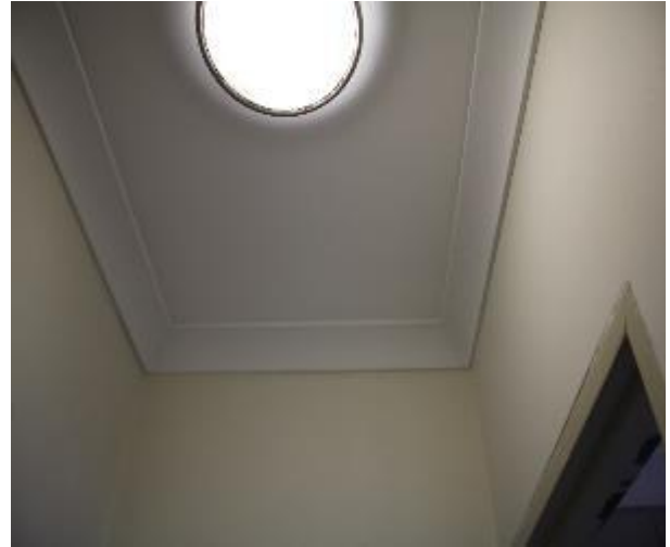
Figure 583 - General condition of corridor ceiling
