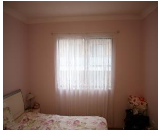
Figure 1131 - General condition of bedroom 1 internal wall
