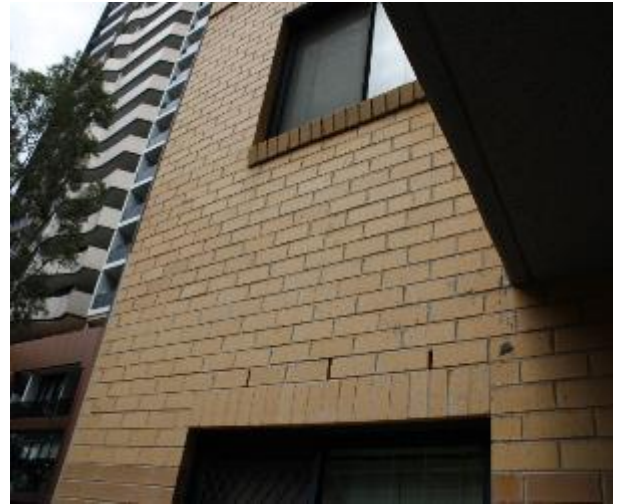
Figure 641 - General condition of external wall
