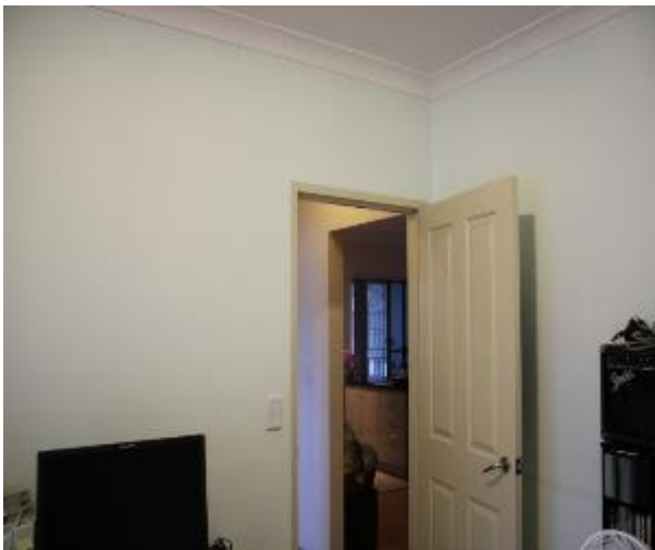
Figure 1202 - General condition of study internal wall
