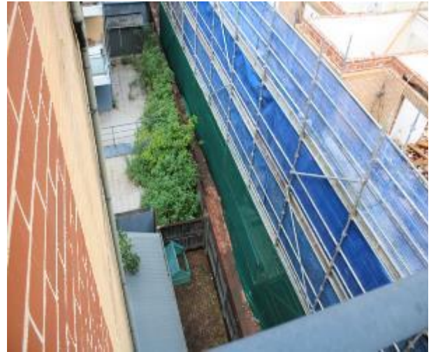
Figure 1509 - General condition of boundary as seen from Unit 29 balcony 1
