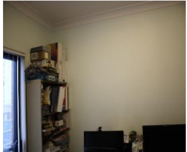
Figure 1201 - General condition of study internal wall
