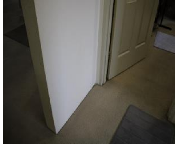
Figure 577 - General condition of corridor internal wall
