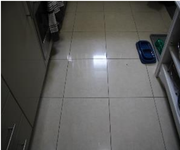
Figure 1420 - General condition of kitchen floor tiles
