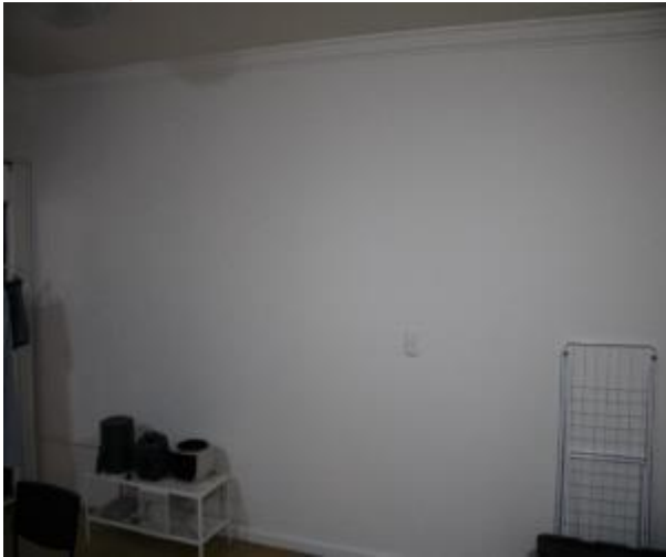
Figure 668 - General condition of kitchen internal wall
