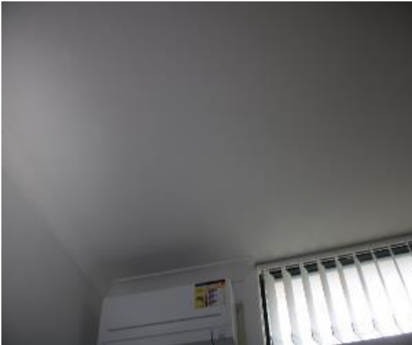
Figure 1340 - General condition of study ceiling
