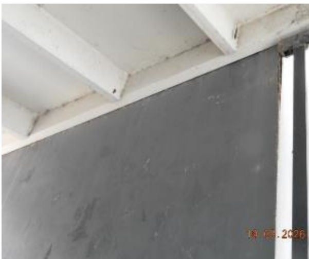
Figure 165 - General condition of B2 to Level 1 fire stairs internal wall
