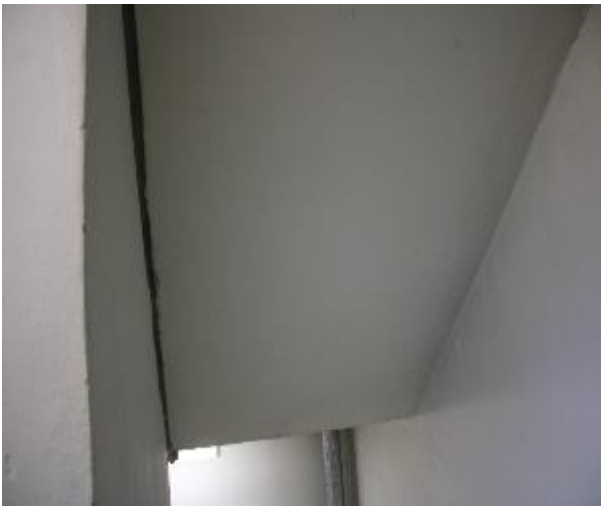
Figure 353 - General condition of level 5 to basement B2 fire stairs underside stairs
