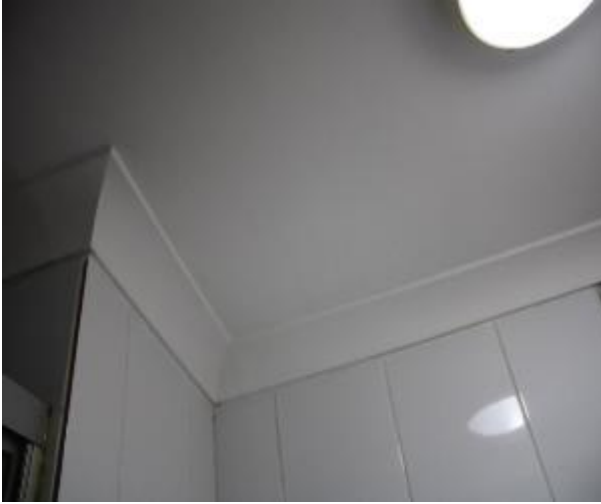
Figure 574 - General condition of ensuite bathroom ceiling
