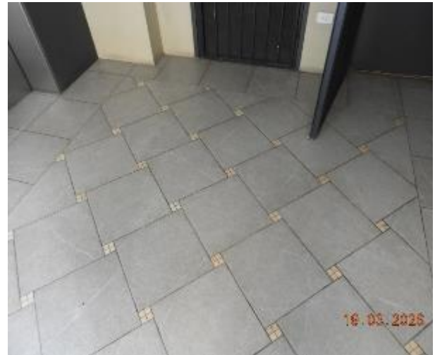
Figure 4 - General condition of level 1 common area floor tiles
