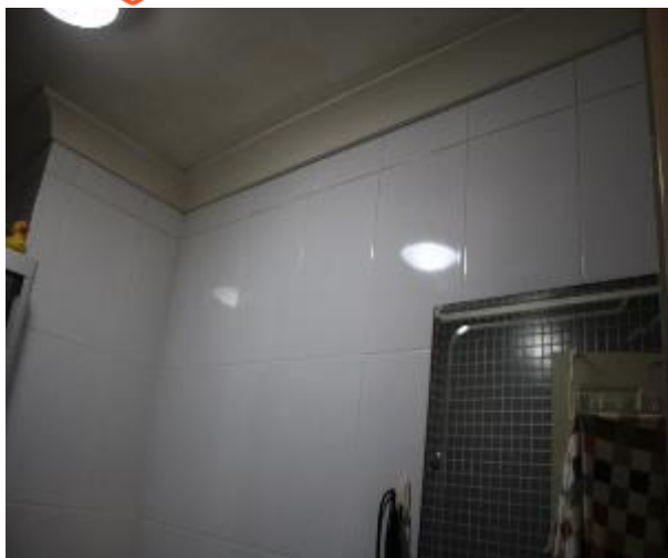
Figure 930 - General condition of ensuite bathroom internal wall
