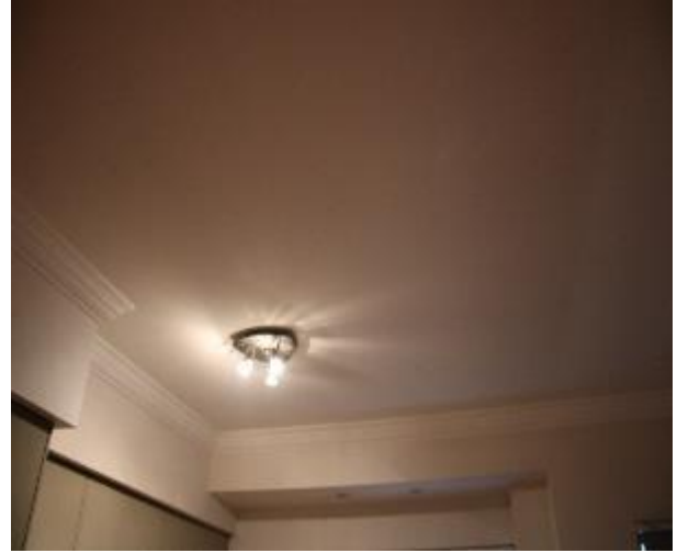
Figure 1117 - General condition of kitchen ceiling
