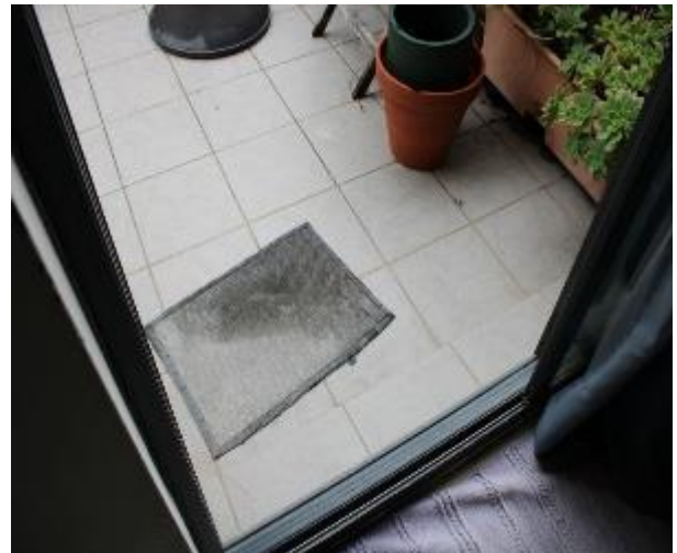
Figure 1565 - General condition of balcony 3 floor tiles
