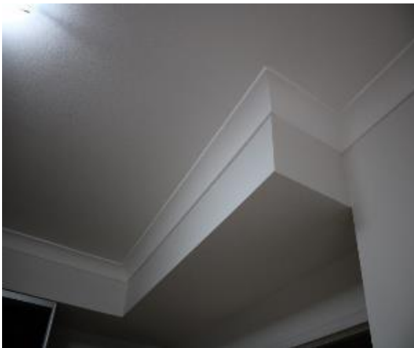
Figure 706 - General condition of bedroom 1 ceiling
