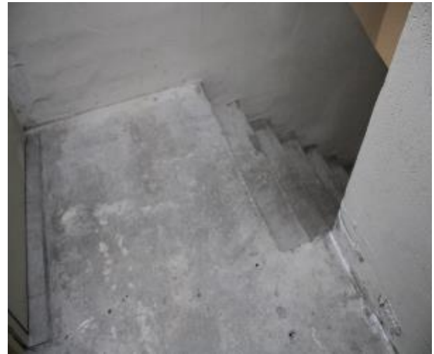
Figure 222 - General condition of level 5 to basement B2 fire stairs
