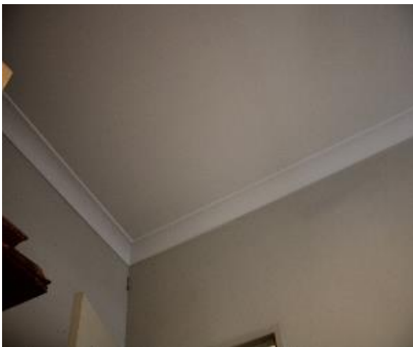
Figure 1558 - General condition of bedroom 2 ceiling
