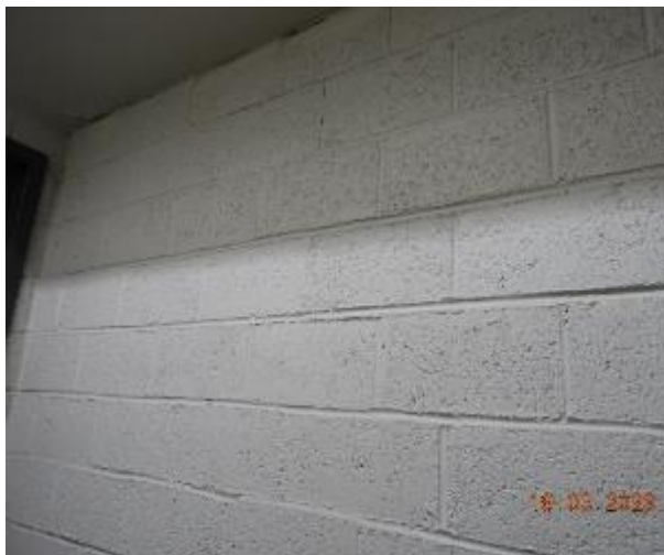
Figure 199 - General condition of B2 to Level 1 fire stairs internal wall
