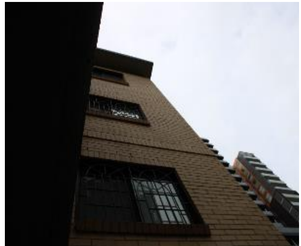
Figure 803 - General condition of external wall
