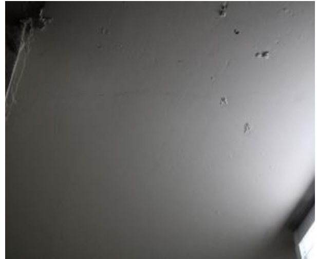
Figure 244 - General condition of level 5 to basement B2 fire stairs underside slab
