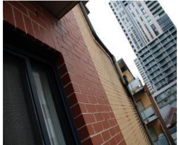
Figure 1213 - General condition of external wall
