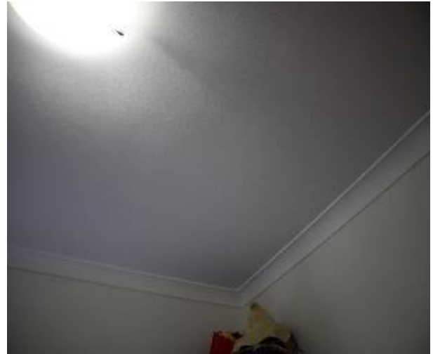
Figure 1054 - General condition of bedroom 2 ceiling
