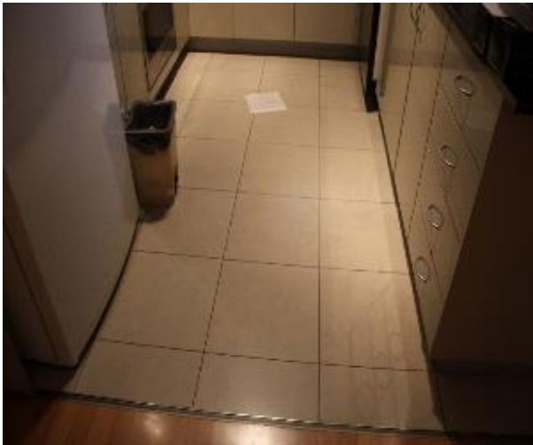
Figure 1112 - General condition of kitchen floor tiles
