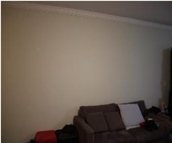
Figure 812 - General condition of open kitchen/ lounge room internal wall
