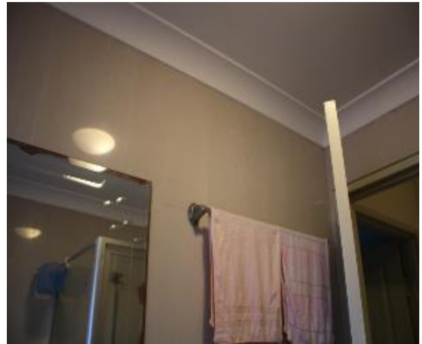
Figure 1191 - General condition of bathroom 1 internal wall
