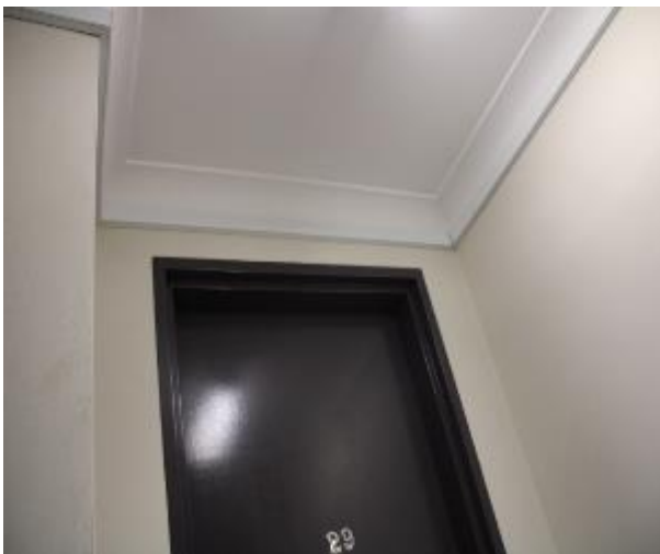
Figure 141 - General condition of level 5 common area internal wall
