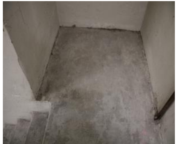
Figure 330 - General condition of level 5 to basement B2 fire stairs
