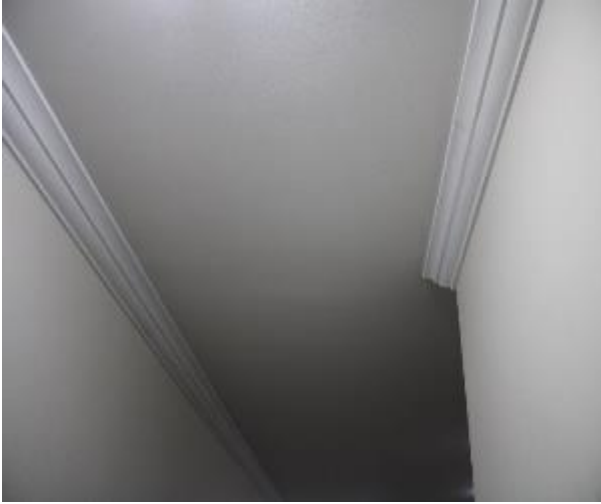
Figure 514 - General condition of open kitchen/ lounge room ceiling
