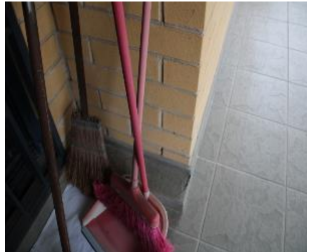
Figure 1233 - General condition of external wall
