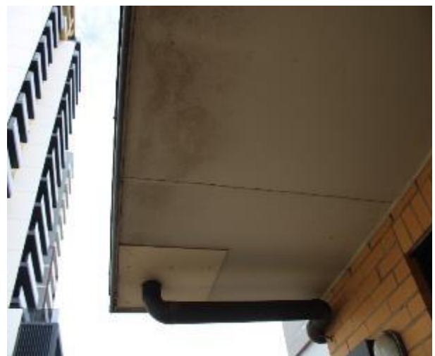
Figure 1525 - General condition of balcony underside slab
