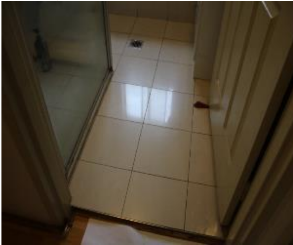
Figure 1182 - General condition of bathroom 1 floor tiles
