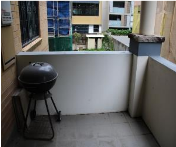
Figure 788 - General condition of external wall
