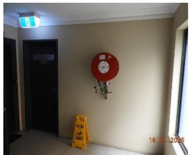
Figure 42 - General condition of level 2 common area internal wall
