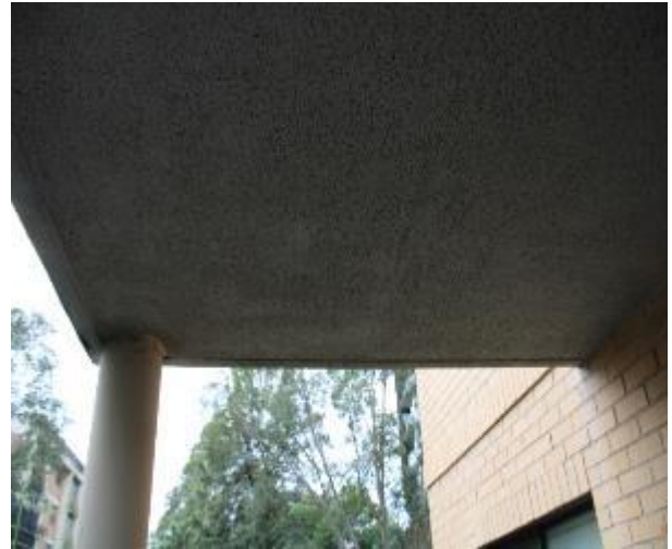
Figure 955 - General condition of balcony underside slab
