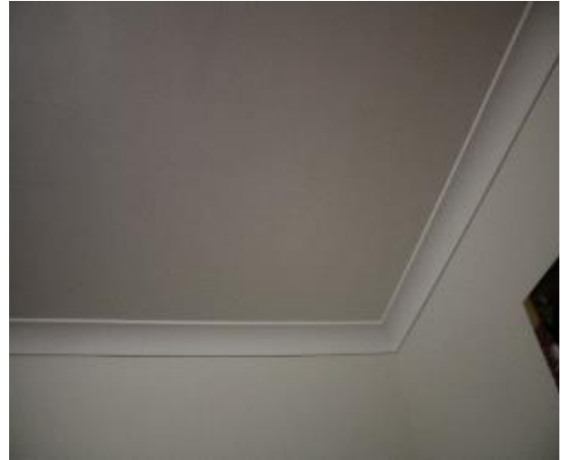
Figure 1026 - General condition of bedroom 1 ceiling
