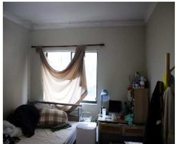
Figure 909 - General condition of bedroom 3 internal wall
