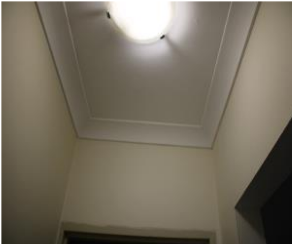
Figure 528 - General condition of corridor ceiling
