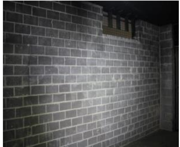
Figure 448 - General condition of basement B2 fire stairs internal wall
