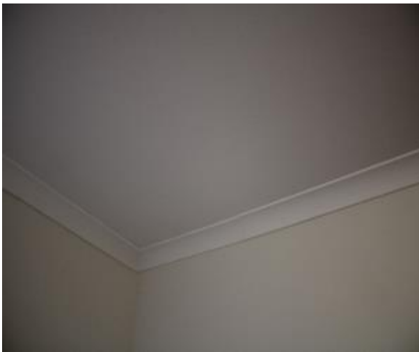
Figure 1001 - General condition of study ceiling
