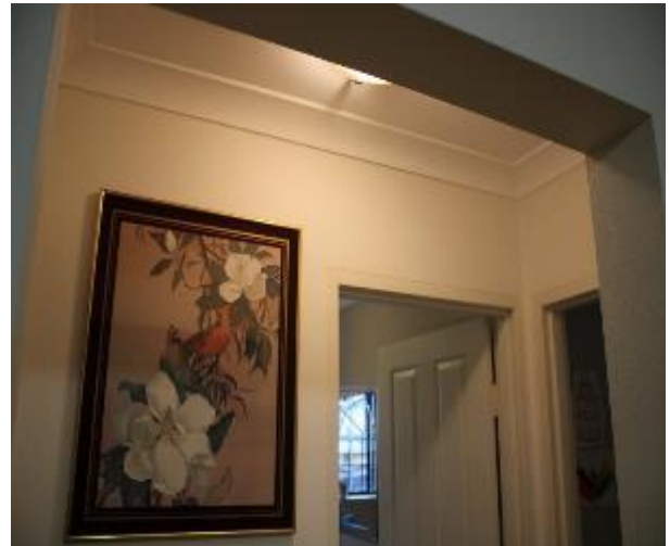
Figure 1014 - General condition of corridor internal wall
