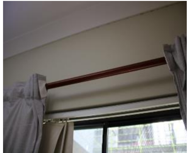
Figure 855 - General condition of bedroom 1 internal wall
