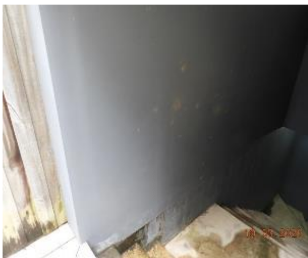
Figure 159 - General condition of B2 to Level 1 fire stairs internal wall
