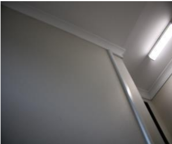
Figure 135 - General condition of staircase to level 5 common area internal wall
