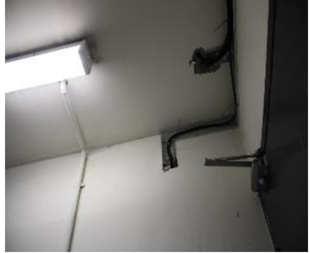
Figure 430 - General condition of level 5 to basement B2 fire stairs underside stairs
