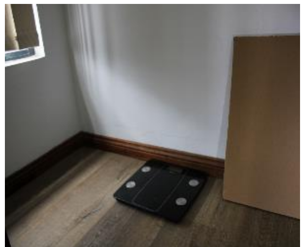
Figure 1337 - General condition of study internal wall
