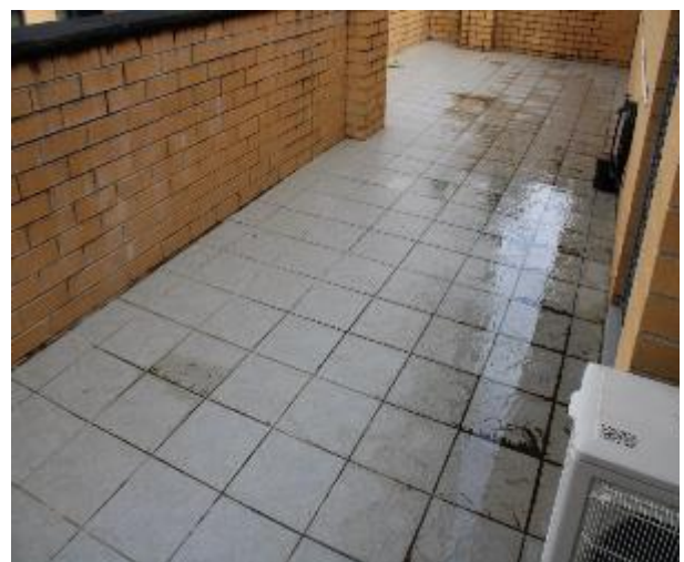
Figure 1391 - General condition of balcony 3 floor tiles
