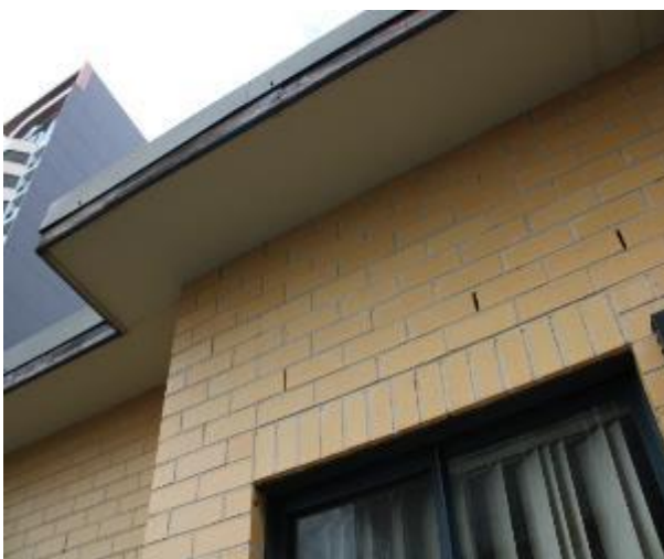
Figure 1572 - General condition of external wall
