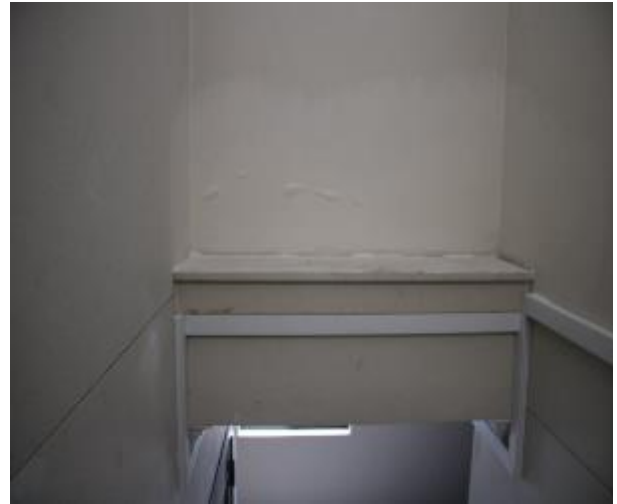
Figure 128 - General condition of staircase to level 5 common area internal wall
