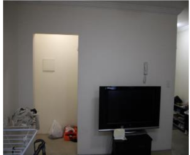
Figure 505 - General condition of open kitchen/ lounge room internal wall
