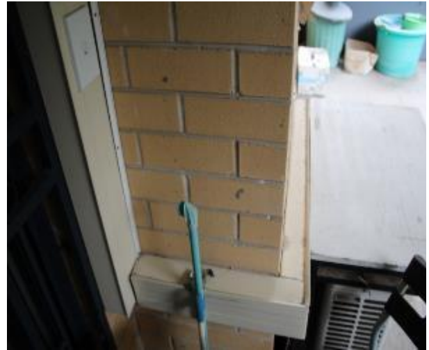
Figure 1066 - General condition of external wall
