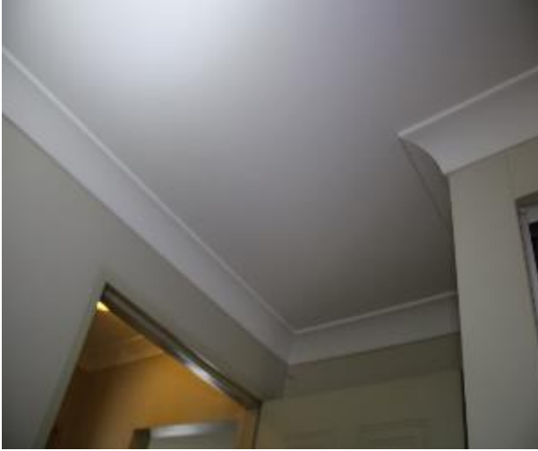
Figure 1484 - General condition of bedroom 1 ceiling
