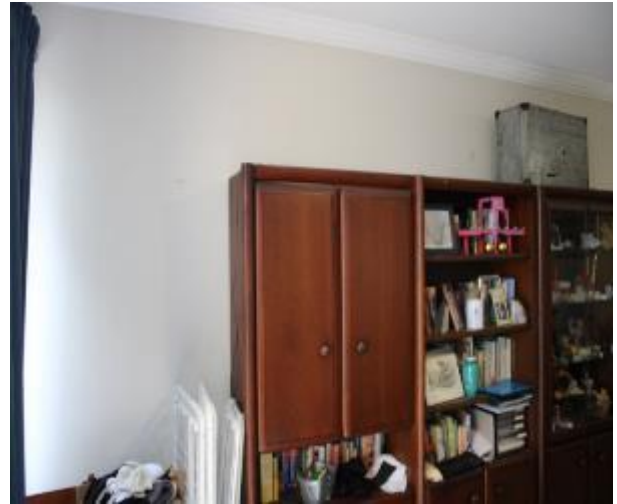
Figure 1455 - General condition of lounge room internal wall
