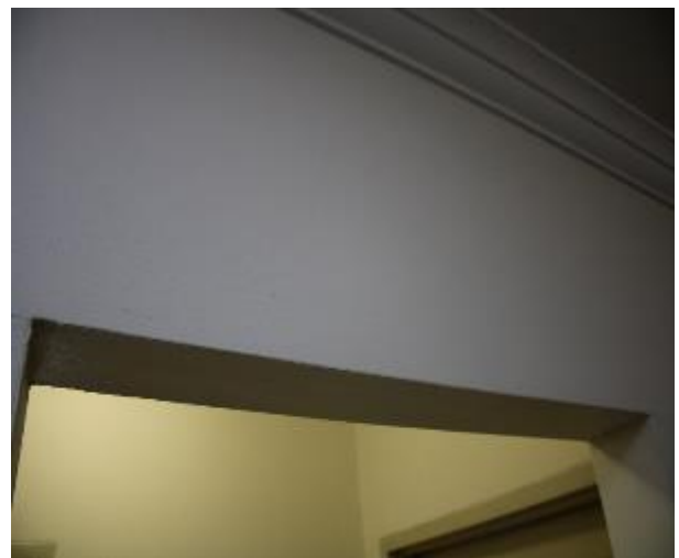
Figure 501 - General condition of open kitchen/ lounge room internal wall
