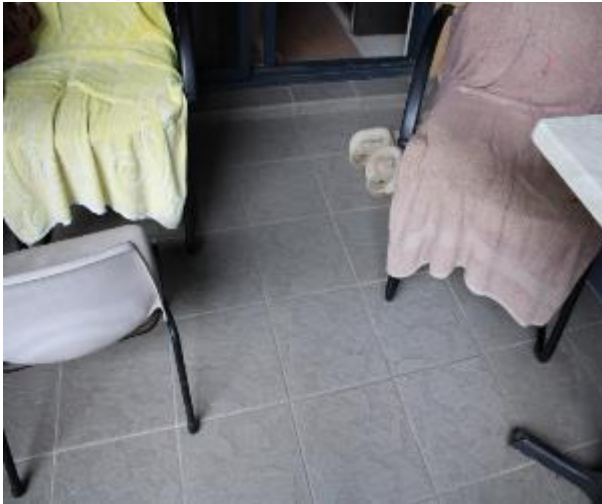
Figure 936 - General condition of balcony floor tiles
