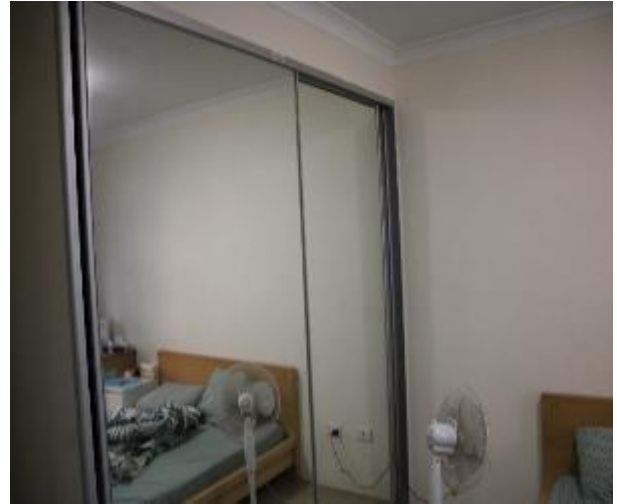
Figure 547 - General condition of bedroom 1 internal wall
