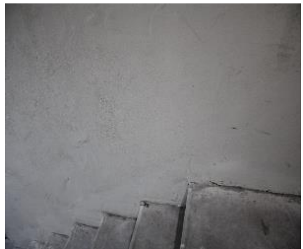
Figure 374 - General condition of level 5 to basement B2 fire stairs internal wall
