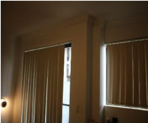
Figure 1286 - General condition of bedroom 1 internal wall
