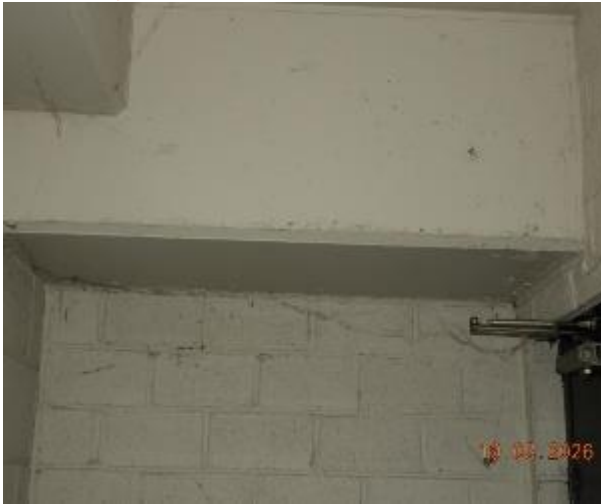
Figure 179 - General condition of B2 to Level 1 fire stairs internal wall
