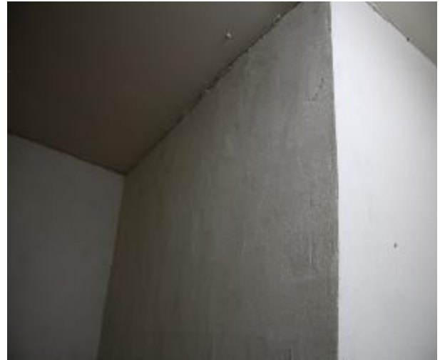
Figure 250 - General condition of level 5 to basement B2 fire stairs internal wall
