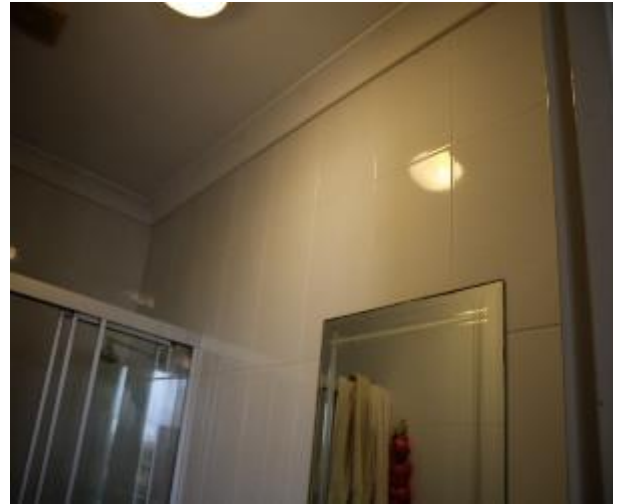
Figure 1497 - General condition of ensuite bathroom internal wall
