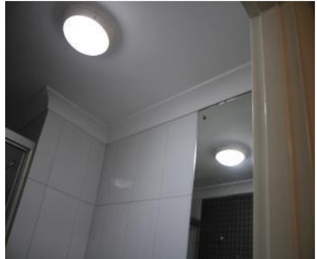
Figure 563 - General condition of ensuite bathroom internal wall
