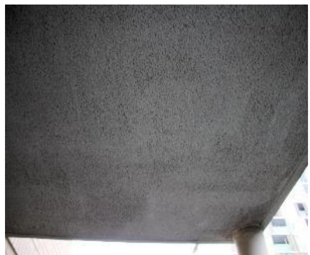
Figure 1076 - General condition of balcony underside slab
