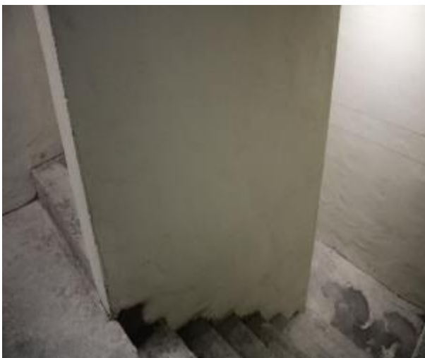
Figure 295 - General condition of level 5 to basement B2 fire stairs internal wall
