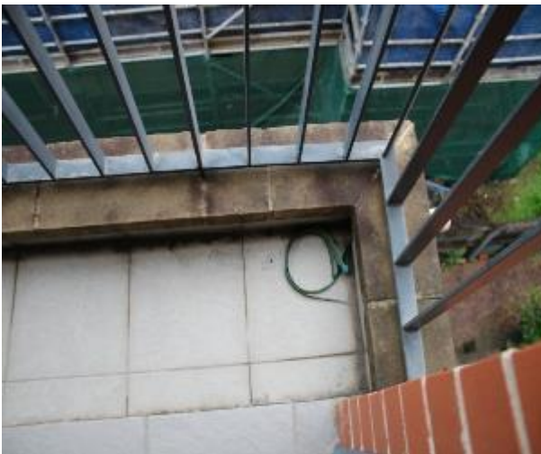
Figure 1210 - General condition of balcony floor tiles
