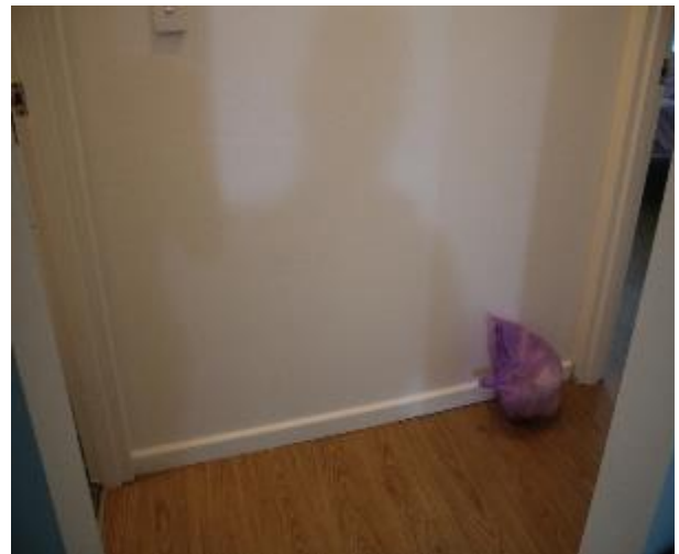
Figure 685 - General condition of corridor internal wall
