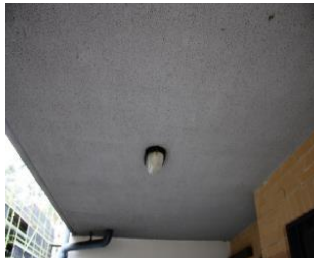
Figure 793 - General condition of balcony underside slab
