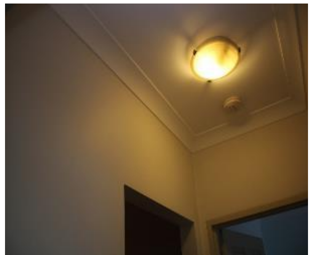
Figure 1163 - General condition of corridor internal wall
