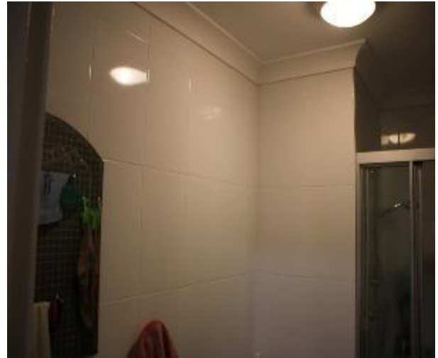
Figure 1006 - General condition of ensuite bathroom internal wall
