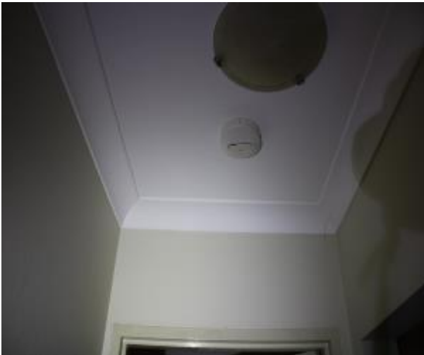
Figure 872 - General condition of corridor ceiling
