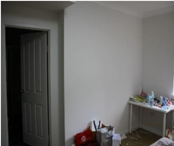
Figure 700 - General condition of bedroom 1 internal wall
