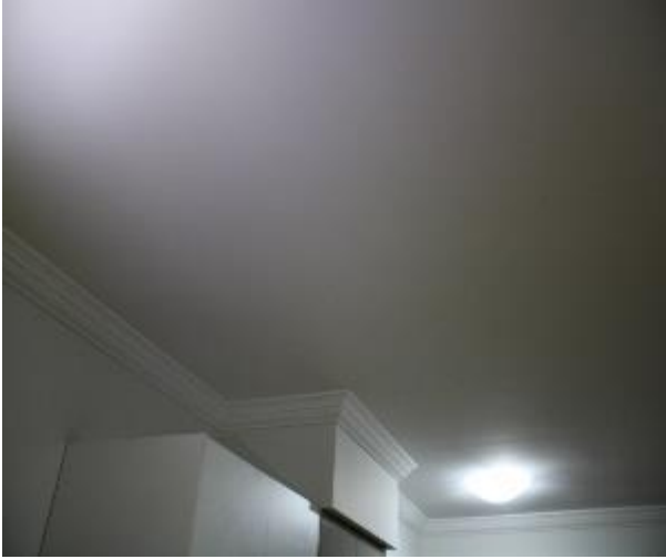
Figure 680 - General condition of kitchen ceiling
