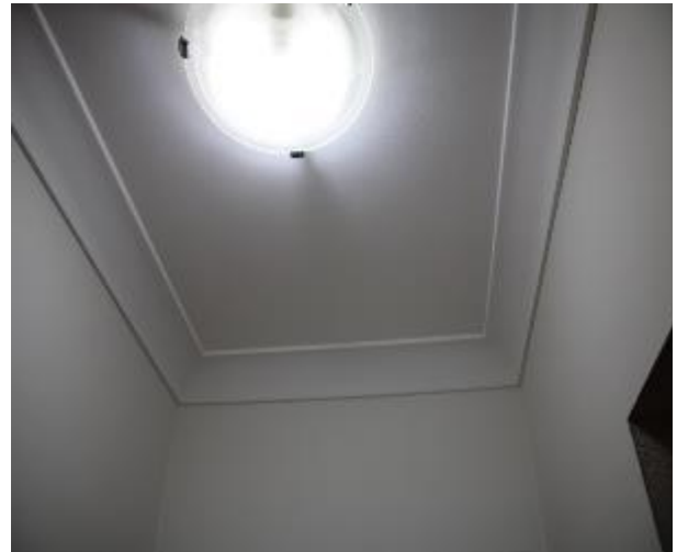
Figure 990 - General condition of corridor ceiling
