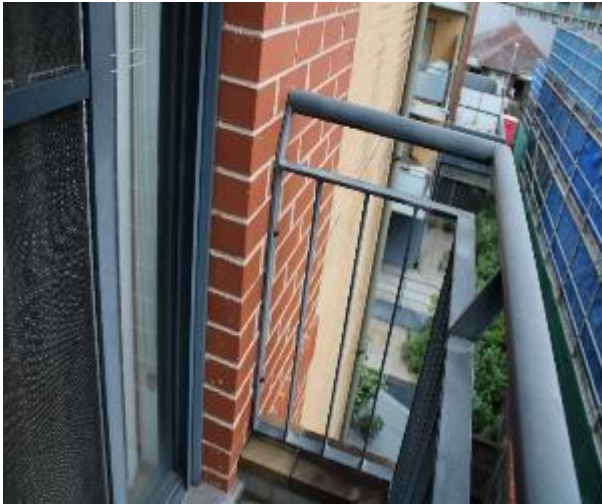
Figure 1212 - General condition of external wall
