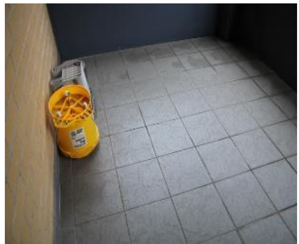
Figure 1217 - General condition of balcony 2 floor tiles
