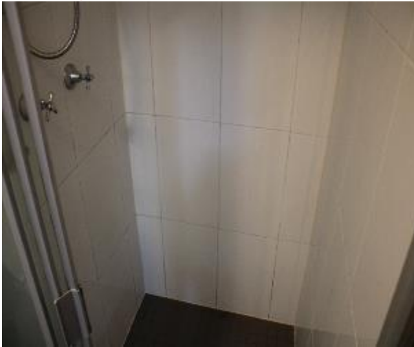
Figure 716 - General condition of ensuite bathroom internal wall
