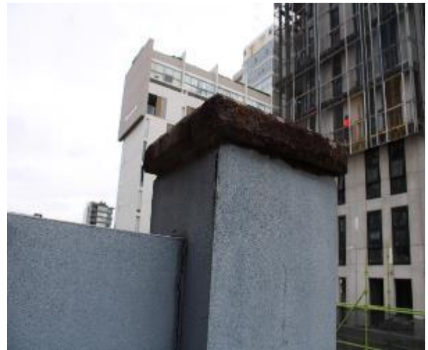
Figure 1311 - General condition of external wall
