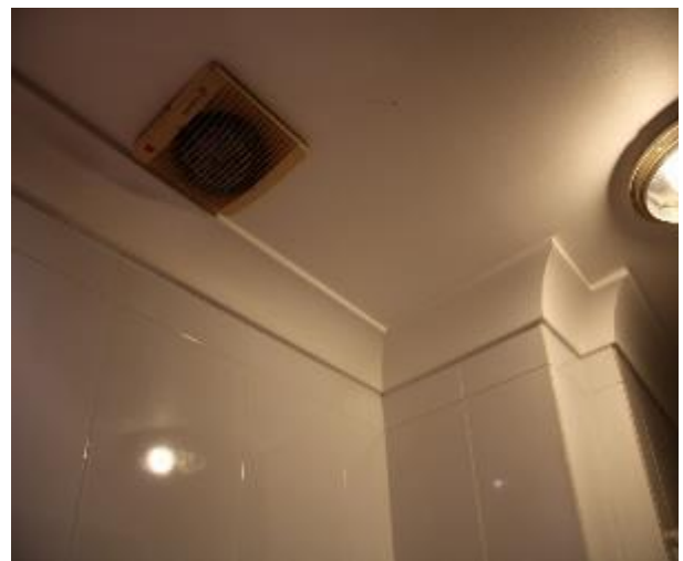
Figure 1157 - General condition of ensuite bathroom ceiling
