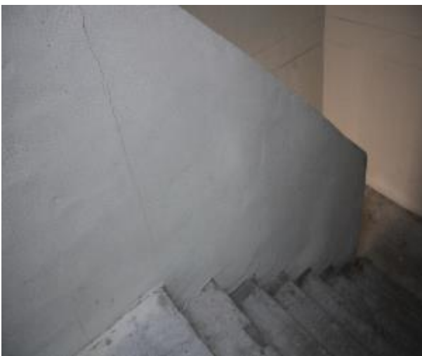
Figure 241 - General condition of level 5 to basement B2 fire stairs internal wall
