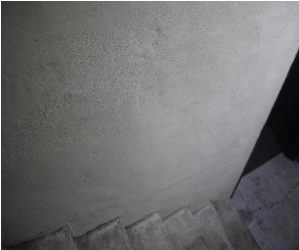
Figure 381 - General condition of level 5 to basement B2 fire stairs internal wall
