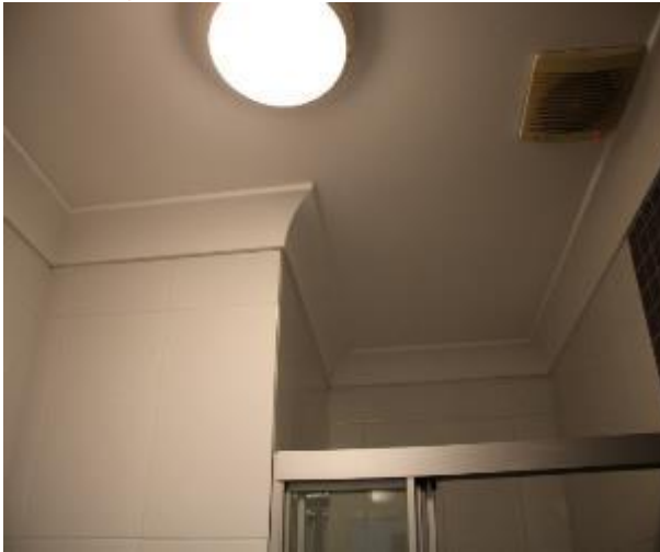
Figure 1011 - General condition of ensuite bathroom ceiling
