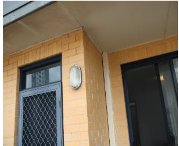
Figure 1399 - General condition of external wall
