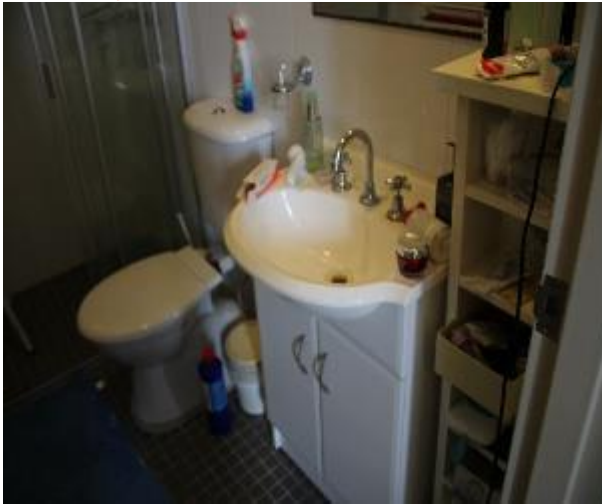
Figure 1496 - General condition of ensuite bathroom internal wall
