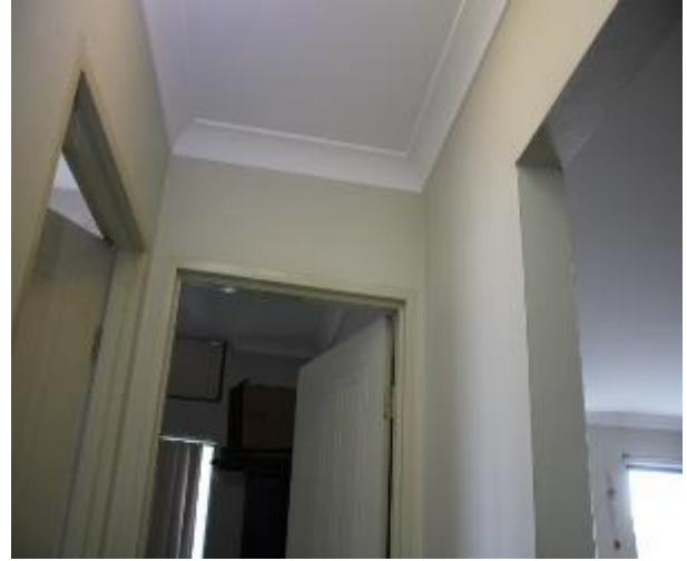
Figure 1467 - General condition of corridor internal wall
