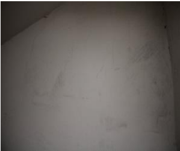
Figure 371 - General condition of level 5 to basement B2 fire stairs internal wall
