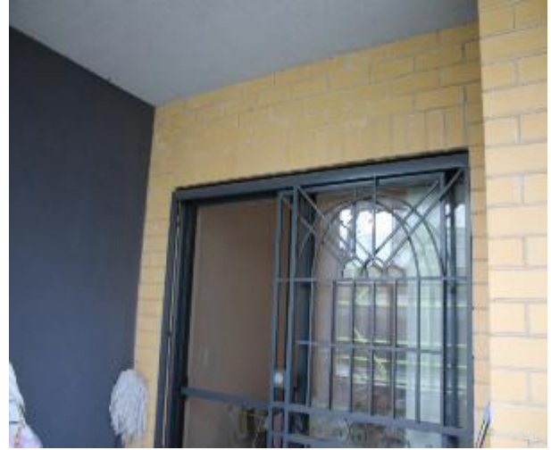
Figure 1225 - General condition of external wall
