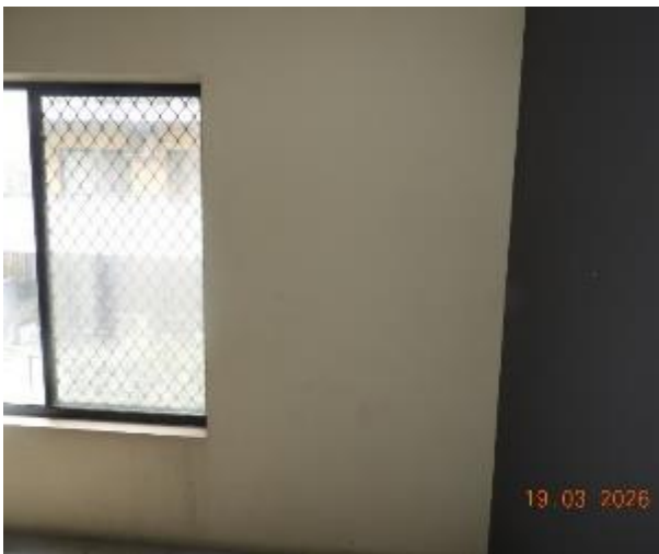
Figure 33 - General condition of level 2 common area internal wall
