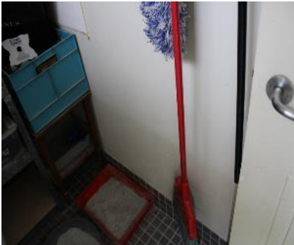
Figure 1438 - General condition of laundry internal wall
