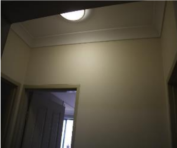
Figure 576 - General condition of corridor internal wall
