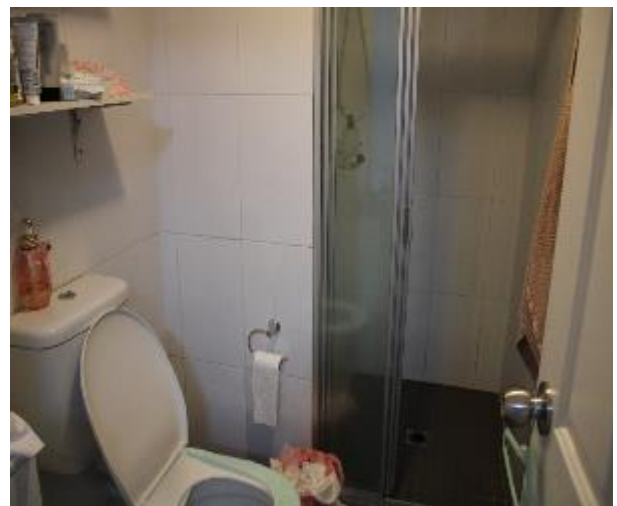
Figure 709 - General condition of ensuite bathroom internal wall
