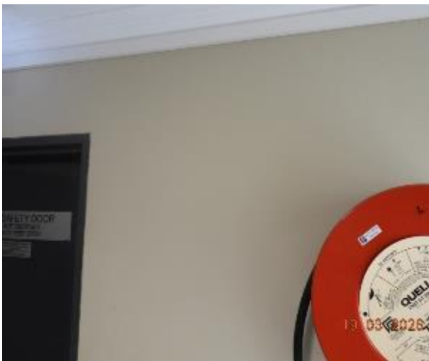
Figure 69 - General condition of level 3 common area internal wall
