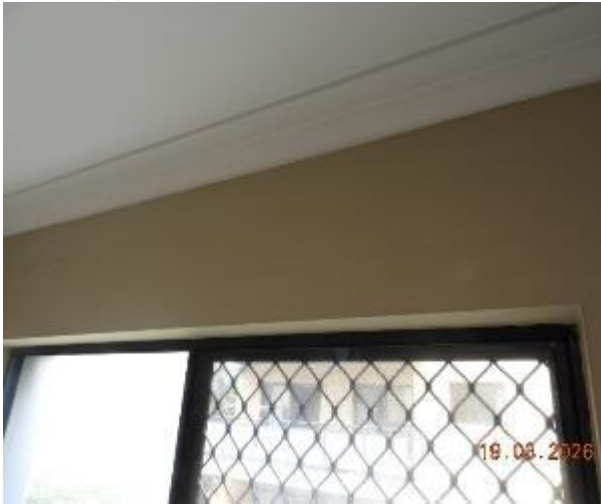
Figure 61 - General condition of level 3 common area internal wall
