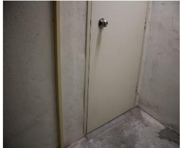
Figure 334 - General condition of level 5 to basement B2 fire stairs internal wall
