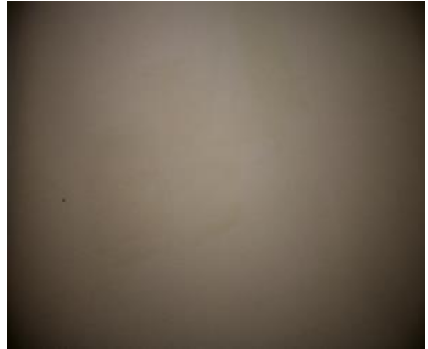
Figure 539 - General condition of laundry internal wall
