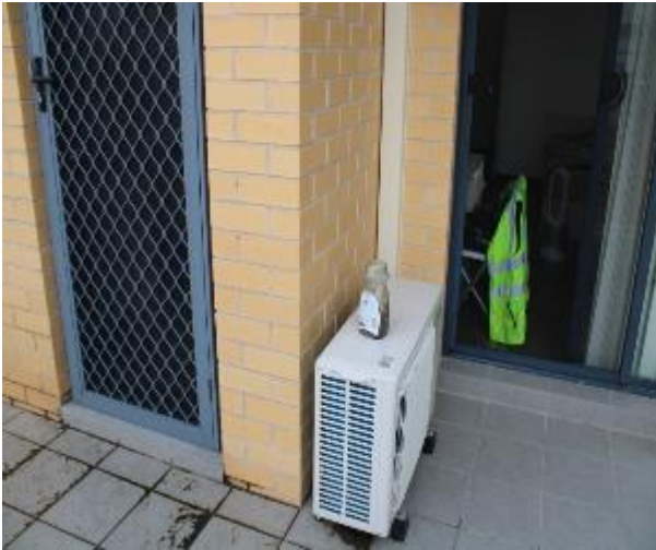
Figure 1398 - General condition of external wall
