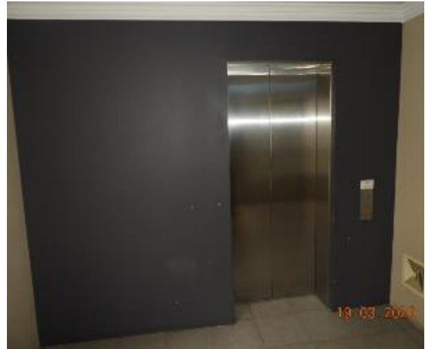
Figure 32 - General condition of level 2 common area internal wall
