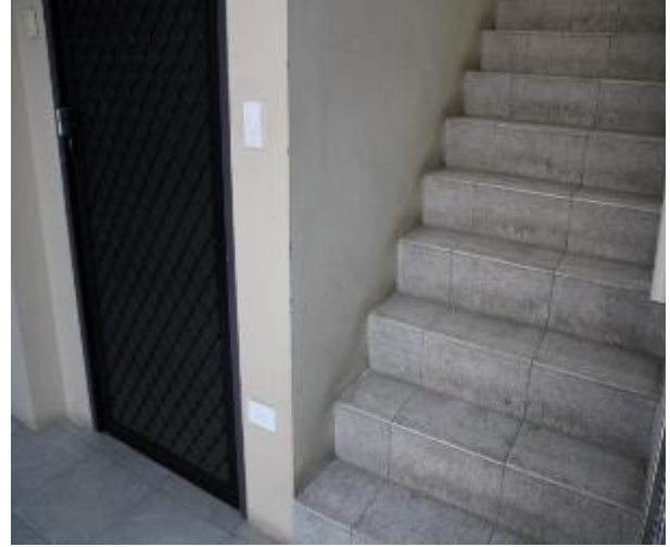
Figure 116 - General condition of staircase to level 5 common area internal wall
