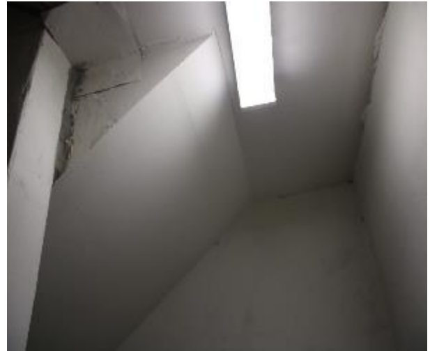
Figure 388 - General condition of level 5 to basement B2 fire stairs underside stairs
