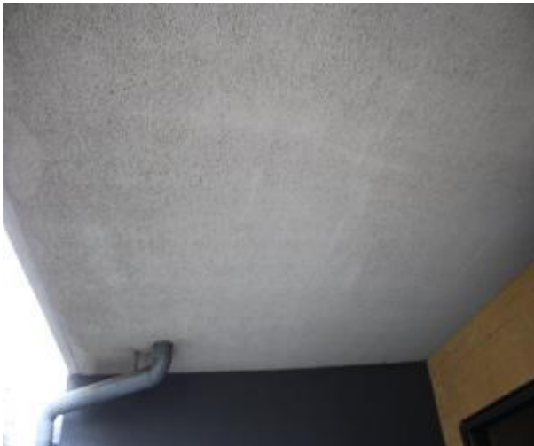
Figure 1244 - General condition of balcony underside slab
