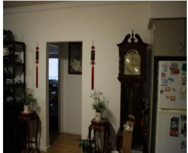
Figure 970 - General condition of lounge room internal wall
