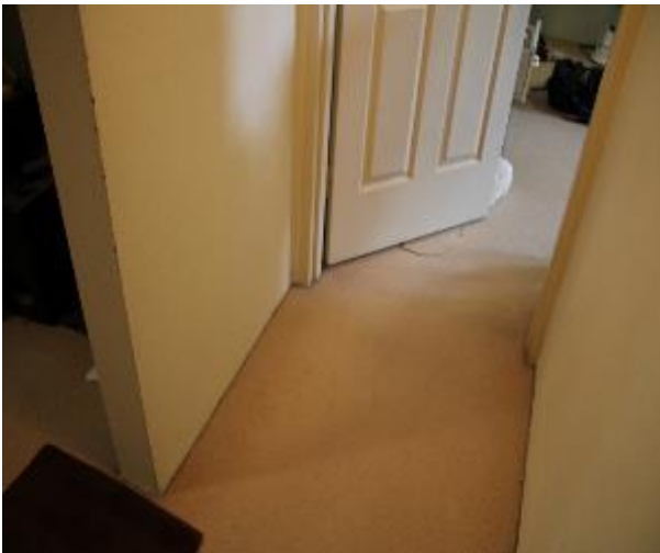
Figure 896 - General condition of corridor internal wall
