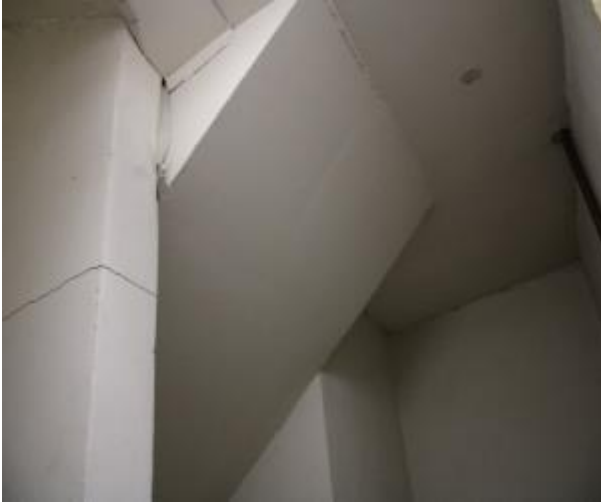
Figure 351 - General condition of level 5 to basement B2 fire stairs underside stairs
