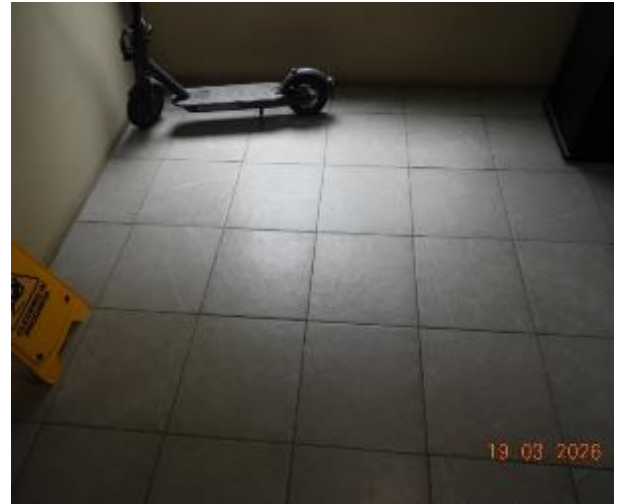
Figure 56 - General condition of level 3 common area floor tiles
