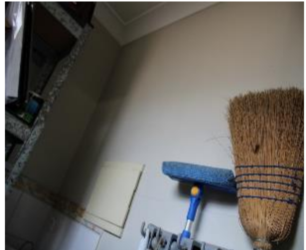
Figure 1439 - General condition of laundry internal wall
