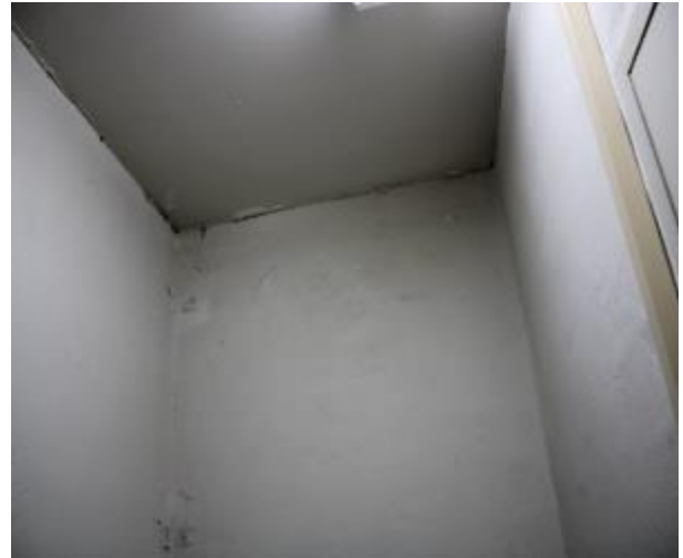
Figure 226 - General condition of level 5 to basement B2 fire stairs internal wall
