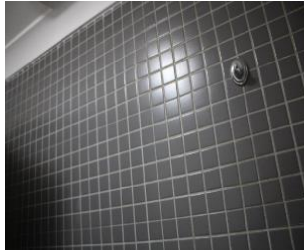
Figure 569 - General condition of ensuite bathroom internal wall
