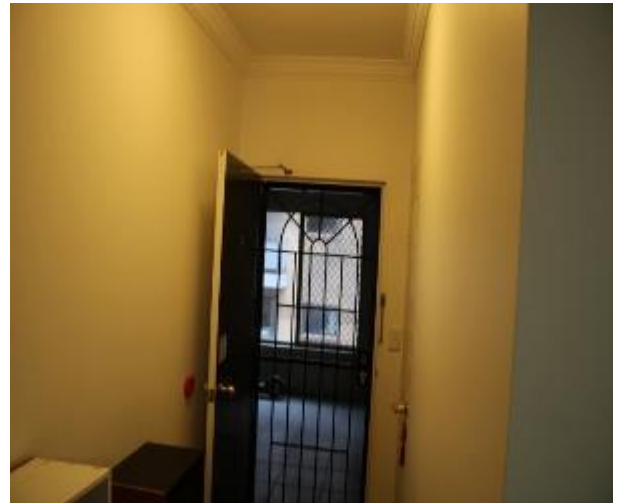
Figure 966 - General condition of lounge room internal wall
