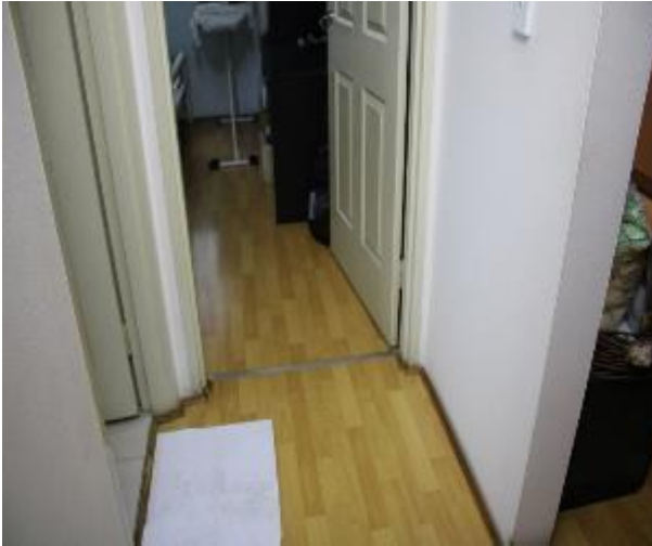
Figure 1160 - General condition of corridor internal wall
