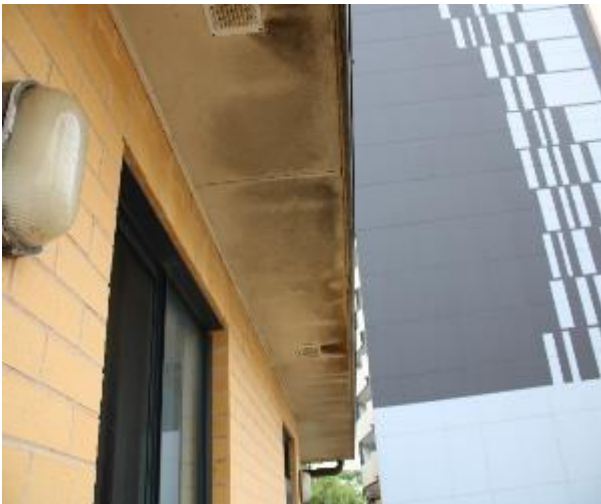
Figure 1412 - General condition of balcony underside slab
