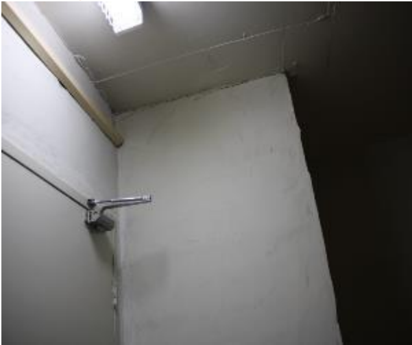
Figure 237 - General condition of level 5 to basement B2 fire stairs internal wall
