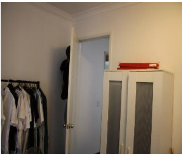
Figure 1282 - General condition of bedroom 1 internal wall
