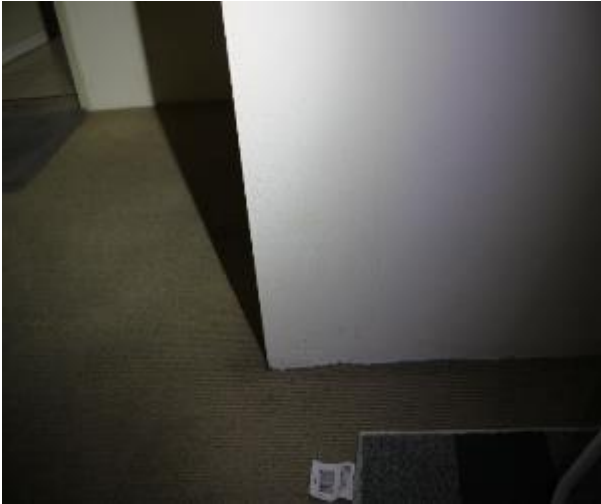
Figure 504 - General condition of open kitchen/ lounge room internal wall
