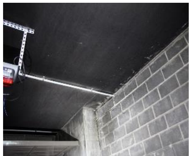
Figure 452 - General condition of basement B2 fire stairs underside slab
