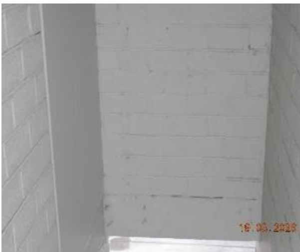
Figure 207 - General condition of B2 to Level 1 fire stairs internal wall
