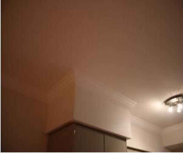
Figure 1116 - General condition of kitchen ceiling
