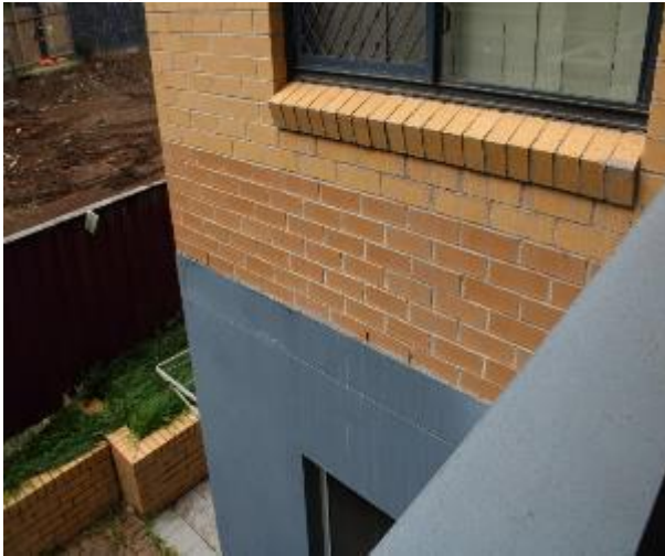
Figure 640 - General condition of external wall
