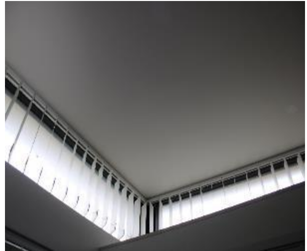
Figure 1341 - General condition of study ceiling
