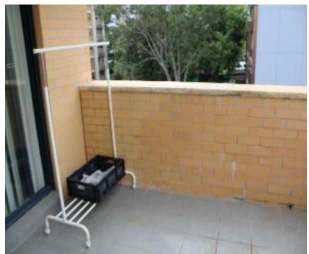
Figure 1403 - General condition of external wall
