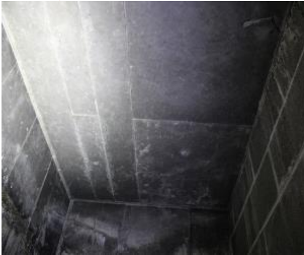
Figure 483 – General condition of basement B2 fire stairs underside slab
