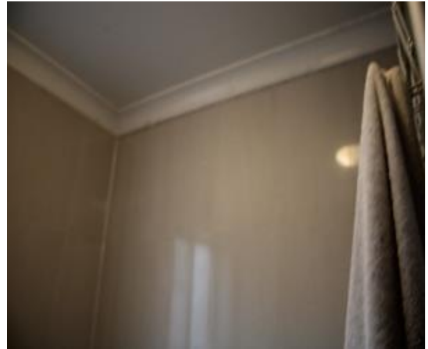
Figure 841 - General condition of bathroom 1 internal wall
