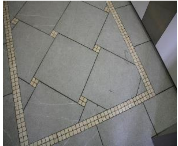
Figure 26 - General condition of level 1 common area floor tiles
