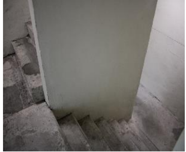
Figure 346 - General condition of level 5 to basement B2 fire stairs internal wall
