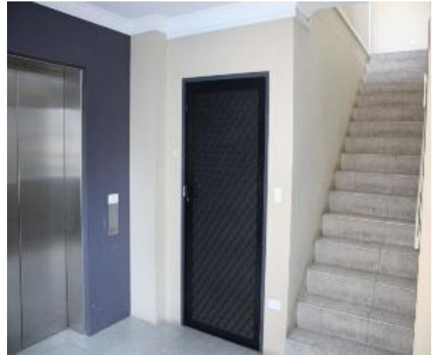
Figure 86 - General condition of level 4 common area internal wall
