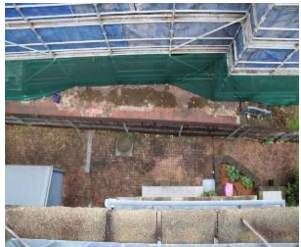
Figure 1511 - General condition of boundary as seen from Unit 29 balcony 1
