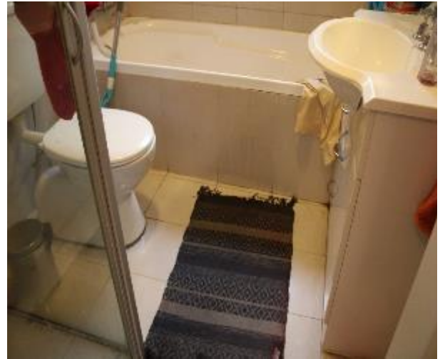
Figure 1030 - General condition of bathroom 1 floor tiles
