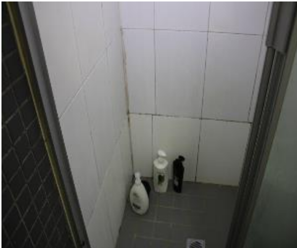
Figure 570 - General condition of ensuite bathroom internal wall
