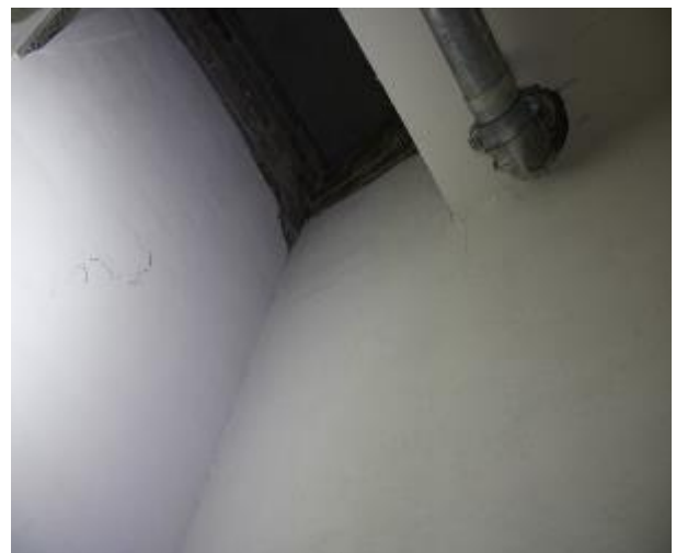
Figure 416 - General condition of level 5 to basement B2 fire stairs internal wall
