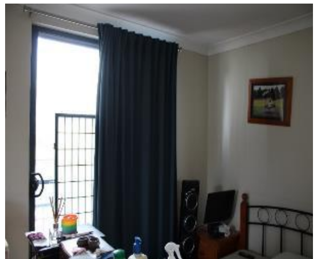
Figure 1483 - General condition of bedroom 1 internal wall
