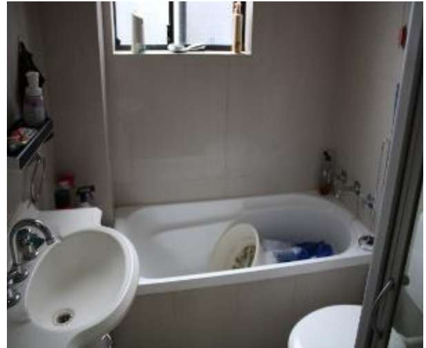
Figure 1345 - General condition of bathroom 1 internal wall
