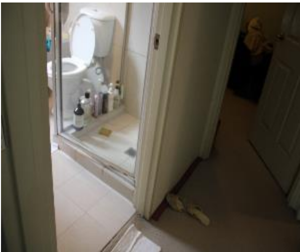
Figure 868 - General condition of corridor internal wall
