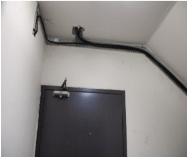
Figure 405 - General condition of level 5 to basement B2 fire stairs internal wall
