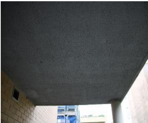
Figure 792 - General condition of balcony underside slab
