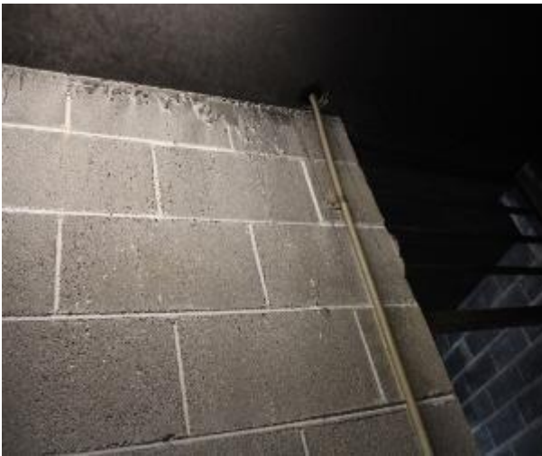
Figure 479 - General condition of basement B2 fire stairs internal wall
