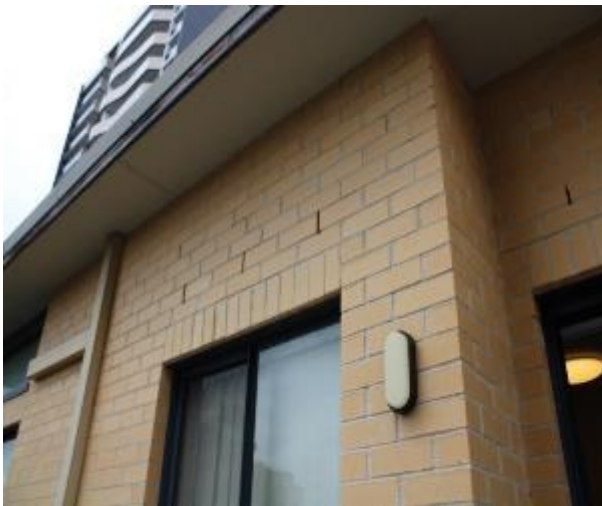
Figure 1298 - General condition of external wall
