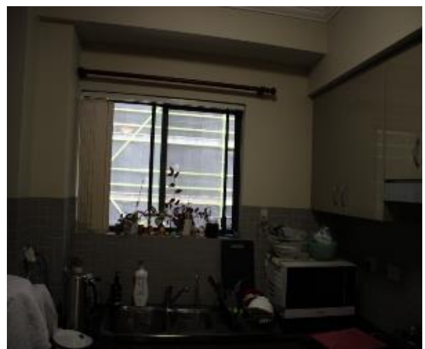
Figure 833 - General condition of kitchen internal wall
