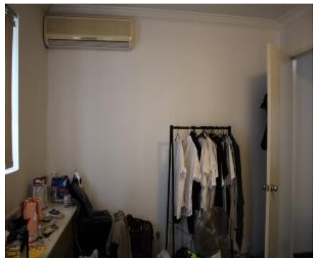
Figure 1283 - General condition of bedroom 1 internal wall
