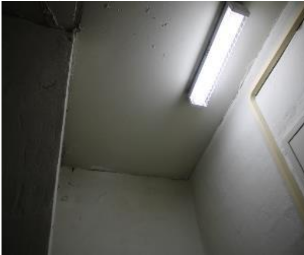
Figure 243 - General condition of level 5 to basement B2 fire stairs underside slab
