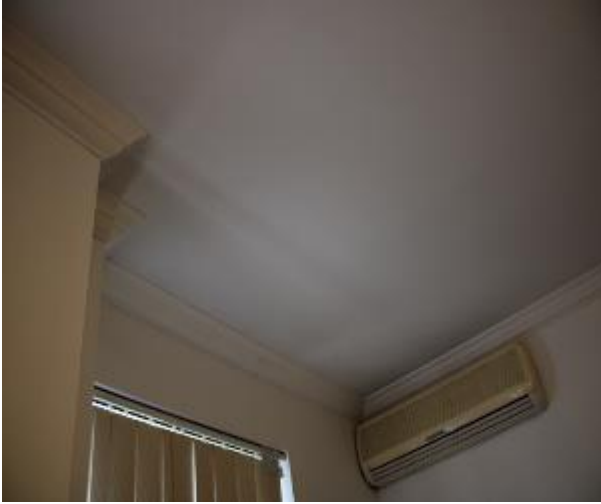
Figure 1290 - General condition of bedroom 1 ceiling
