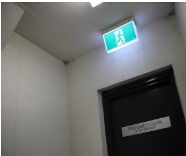
Figure 397 - General condition of level 5 to basement B2 fire stairs internal wall
