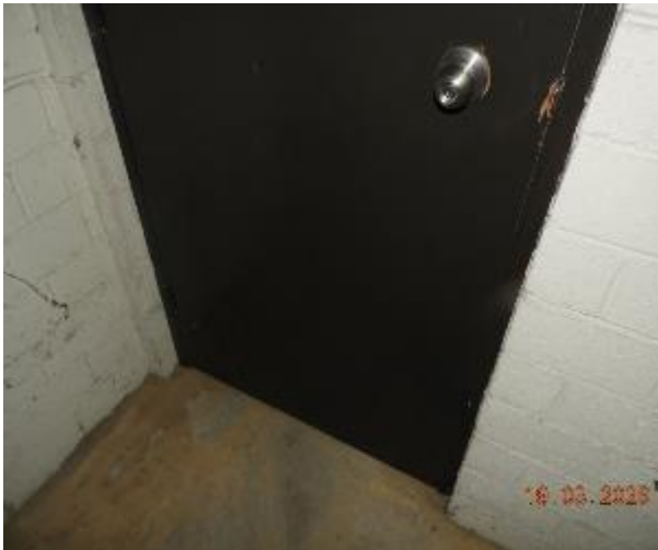
Figure 181 - General condition of B2 to Level 1 fire stairs internal wall
