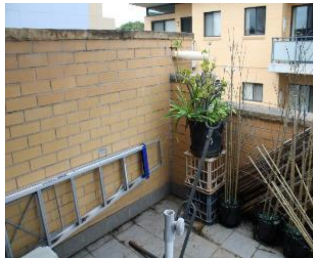
Figure 1517 - General condition of external wall
