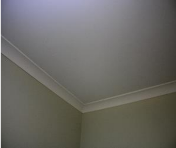
Figure 890 - General condition of bedroom 2 ceiling
