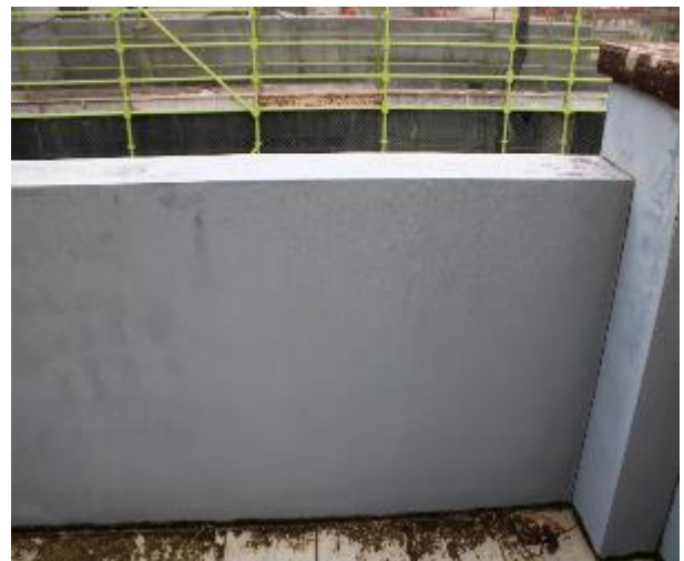
Figure 1305 - General condition of external wall
