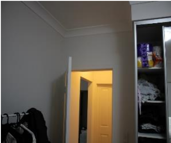
Figure 730 - General condition of bedroom 2 internal wall
