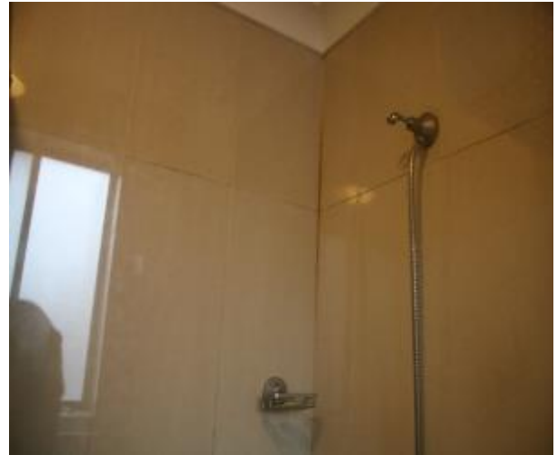
Figure 1189 - General condition of bathroom 1 internal wall
