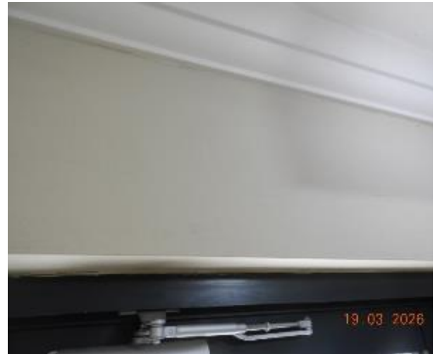
Figure 16 - General condition of level 1 common area internal wall
