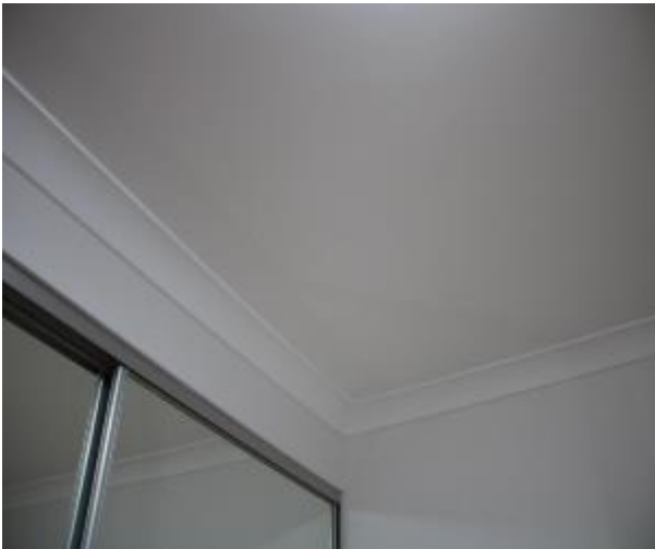
Figure 736 - General condition of bedroom 2 ceiling
