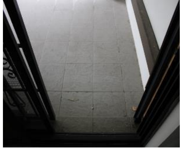
Figure 771 - General condition of balcony floor tiles
