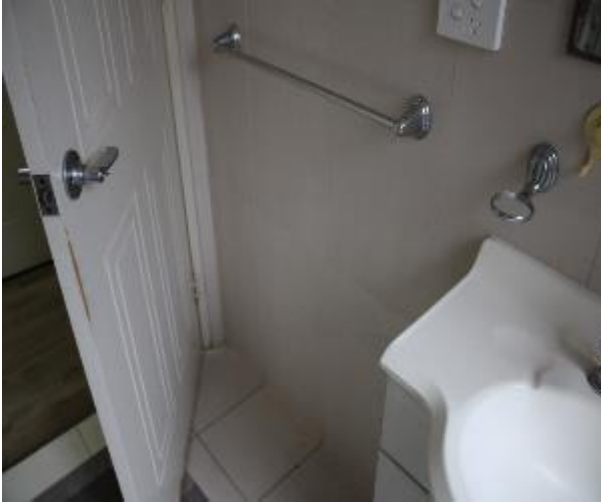
Figure 1350 - General condition of bathroom 1 internal wall
