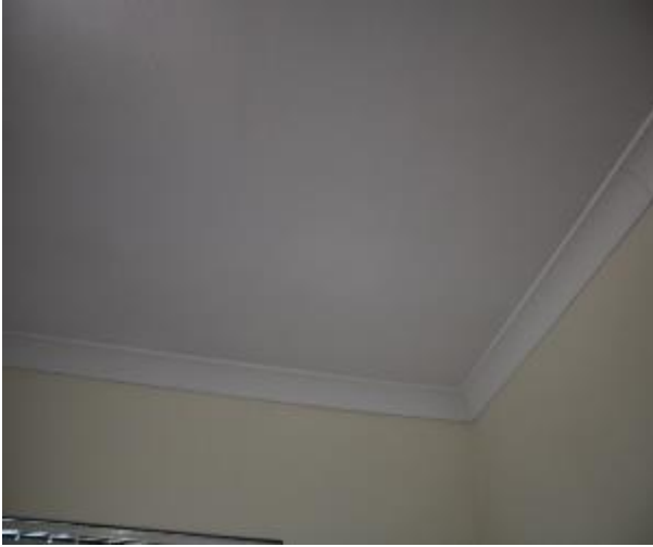
Figure 598 - General condition of bedroom 2 ceiling
