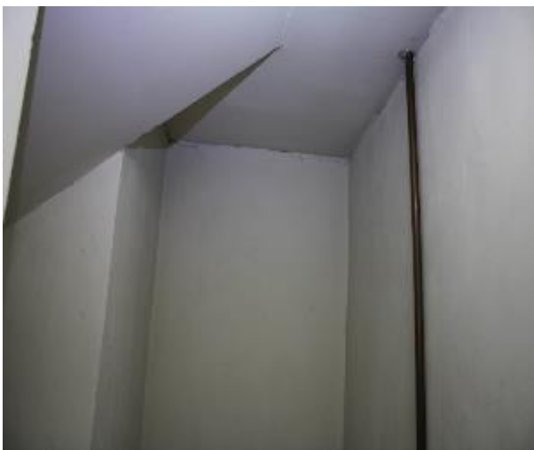
Figure 337 - General condition of level 5 to basement B2 fire stairs internal wall
