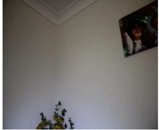
Figure 1024 - General condition of bedroom 1 internal wall
