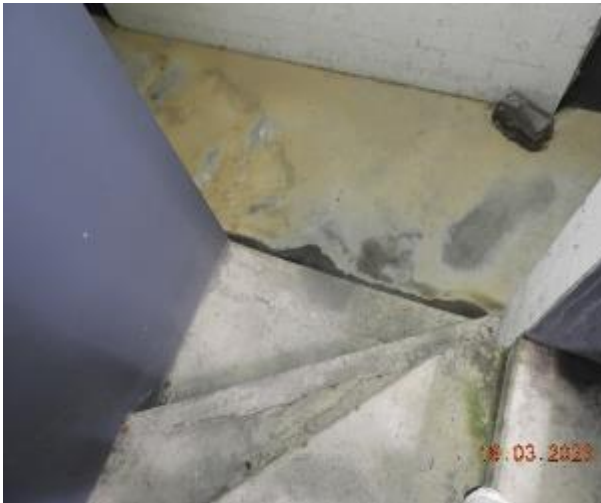
Figure 175 - General condition of B2 to Level 1 fire stairs pavement slab
