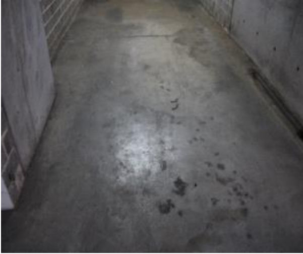
Figure 435 - General condition of basement B2 fire stairs pavement slab
