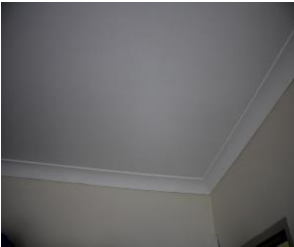
Figure 630 - General condition of bedroom 3 ceiling
