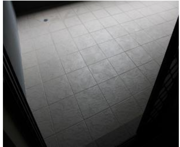
Figure 635 - General condition of balcony floor tiles
