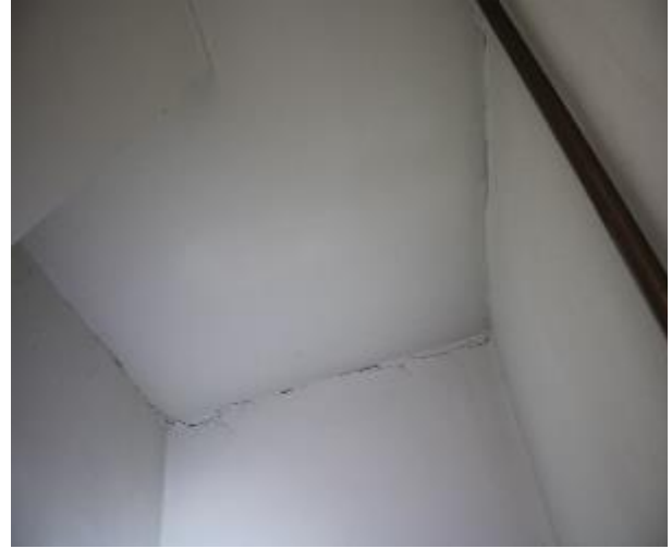
Figure 352 - General condition of level 5 to basement B2 fire stairs underside stairs
