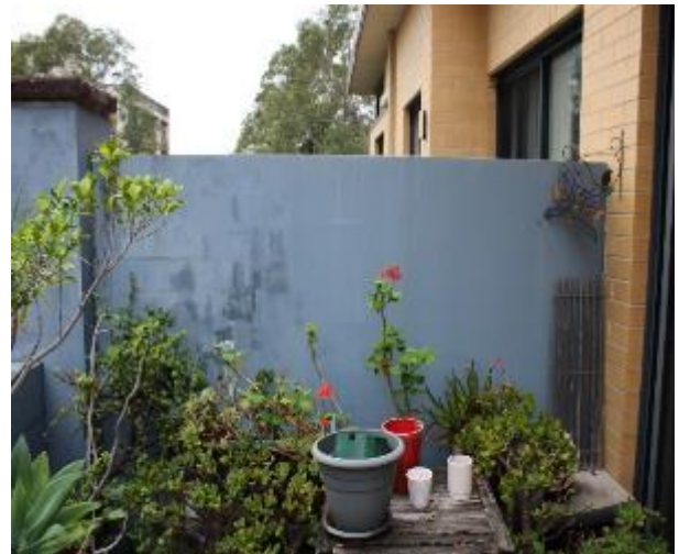
Figure 1577 - General condition of external wall
