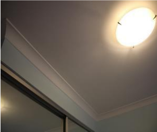
Figure 1178 - General condition of bedroom 2 ceiling
