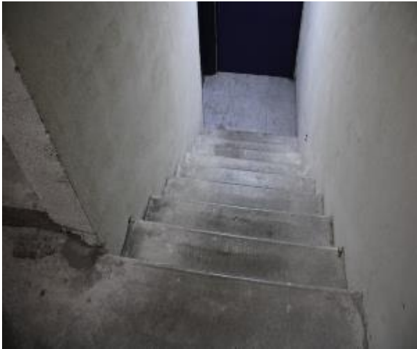
Figure 357 - General condition of level 5 to basement B2 fire stairs
