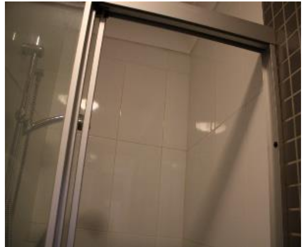
Figure 1008 - General condition of ensuite bathroom internal wall
