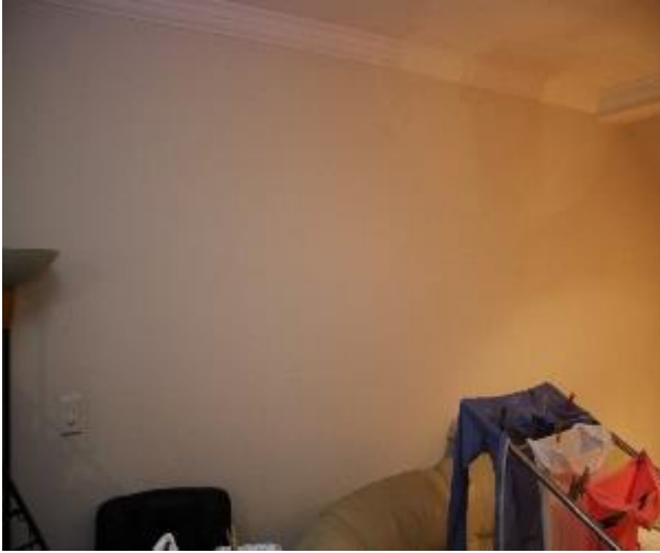
Figure 1104 - General condition of lounge room internal wall
