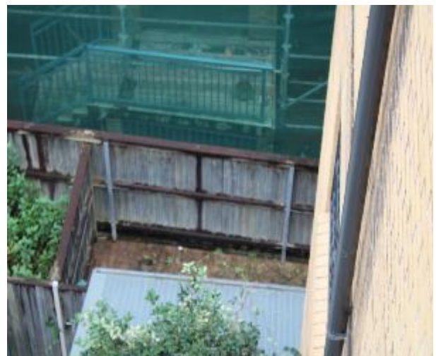
Figure 1415 - General condition of boundary as seen from Unit 28 balcony
