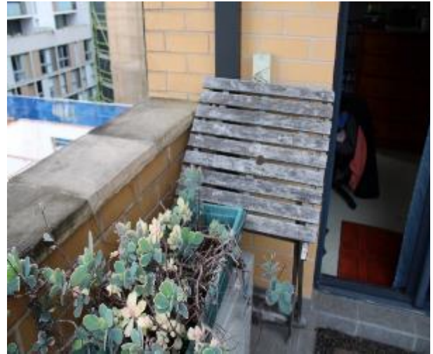
Figure 1521 - General condition of external wall
