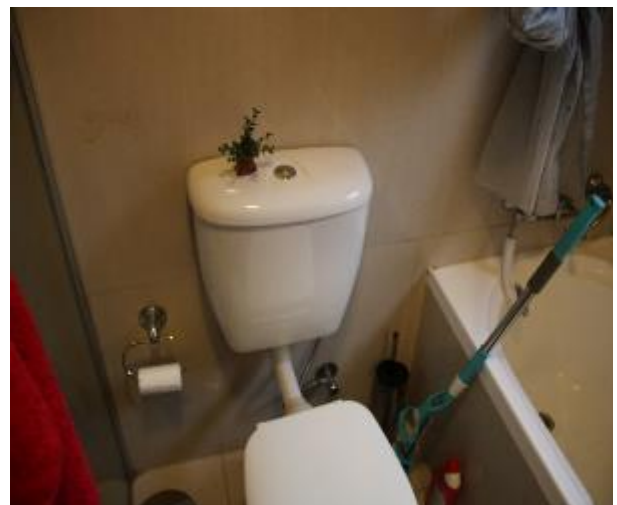
Figure 1040 - General condition of bathroom 1 internal wall
