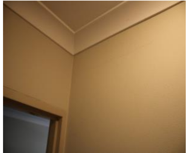
Figure 895 - General condition of corridor internal wall
