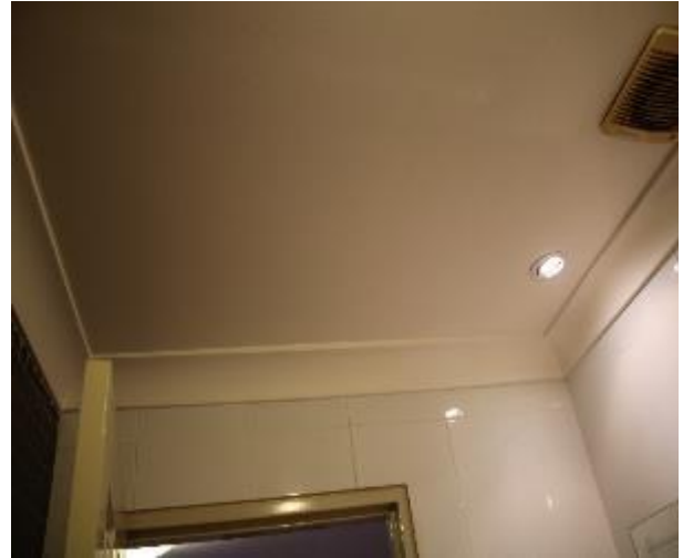
Figure 1155 - General condition of ensuite bathroom ceiling
