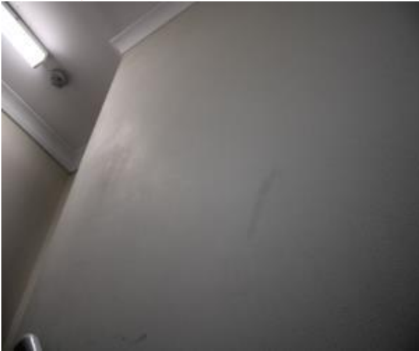
Figure 133 - General condition of staircase to level 5 common area internal wall
