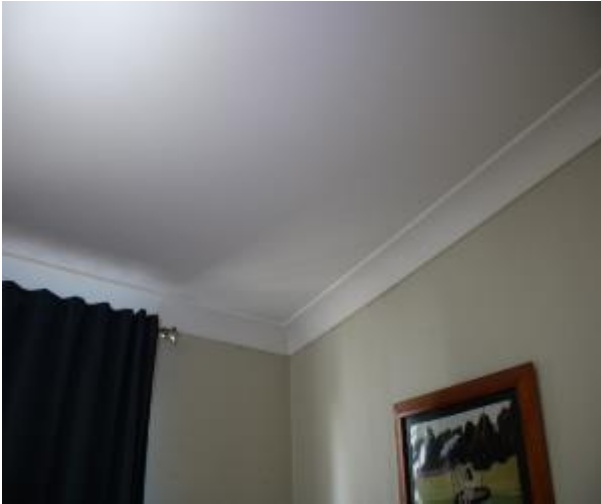
Figure 1486 - General condition of bedroom 1 ceiling
