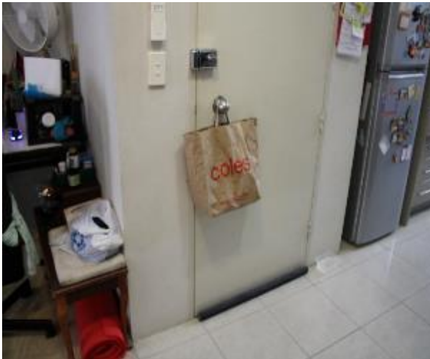
Figure 1426 - General condition of kitchen internal wall
