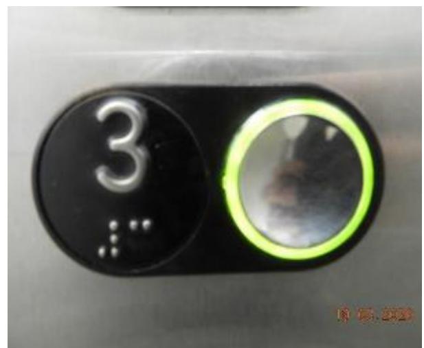
Figure 54 -The following images display the condition of Level 3 Common Area
