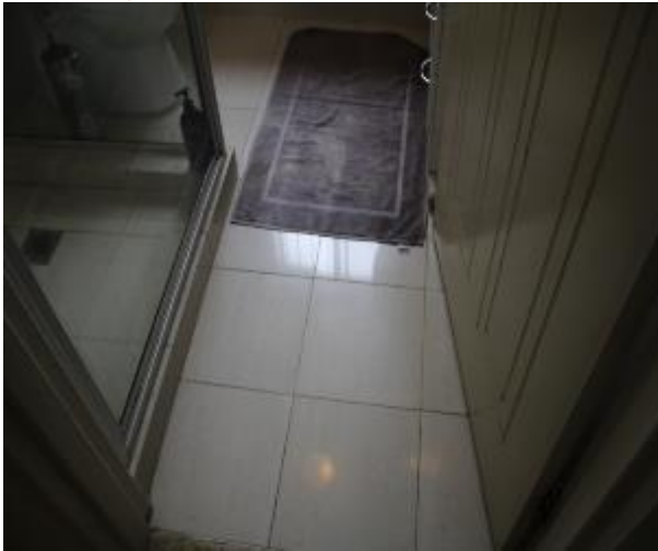
Figure 1532 - General condition of bathroom 1 floor tiles
