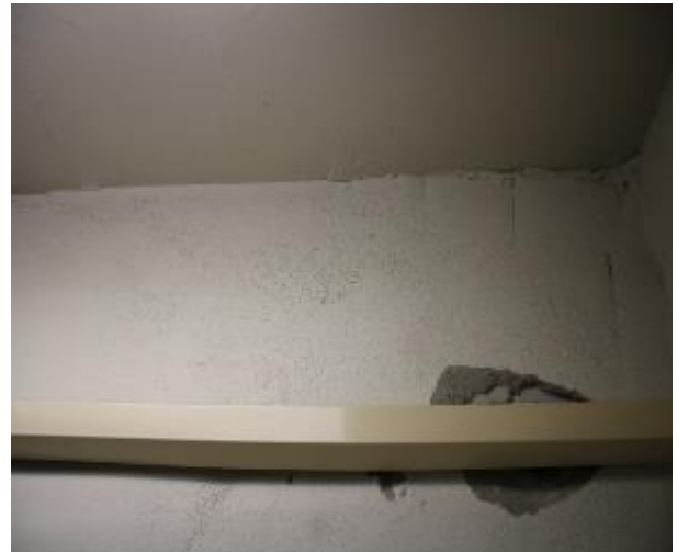
Figure 282 - General condition of level 5 to basement B2 fire stairs internal wall
