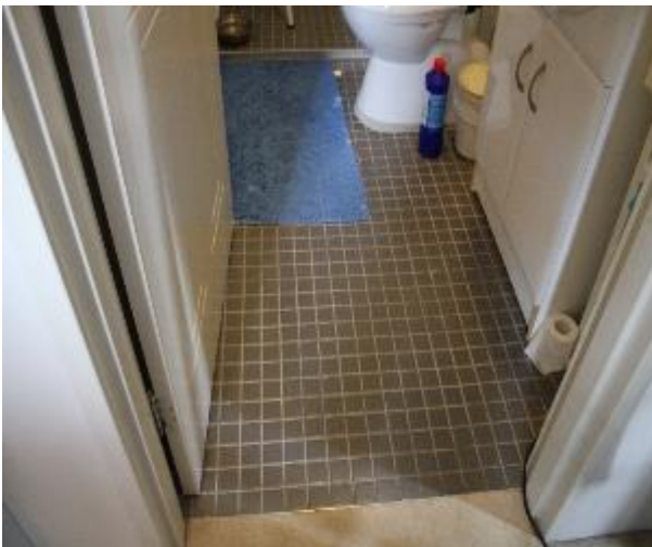
Figure 1494 - General condition of ensuite bathroom floor tiles
