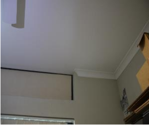
Figure 1562 - General condition of bedroom 2 ceiling
