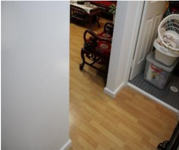
Figure 987 - General condition of corridor internal wall
