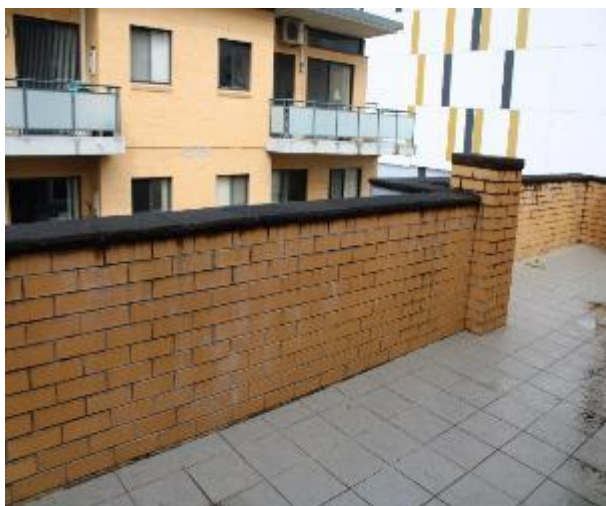
Figure 1406 - General condition of external wall
