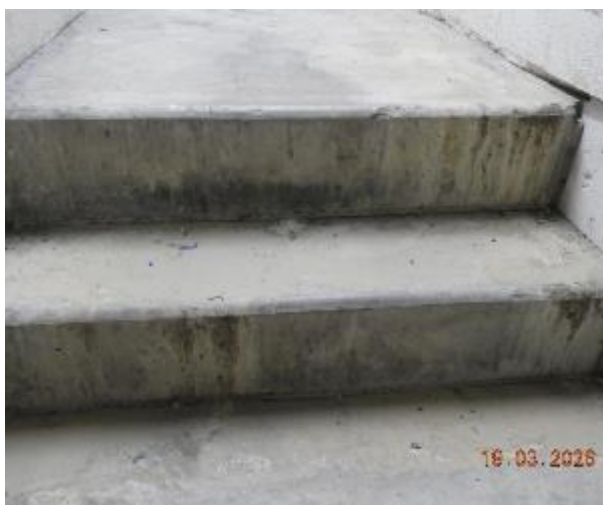
Figure 195 - General condition of B2 to Level 1 fire stairs
