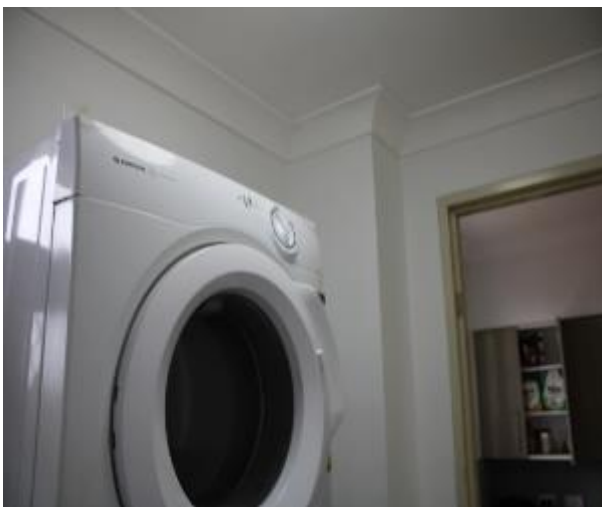
Figure 1264 - General condition of laundry internal wall
