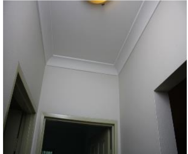
Figure 1161 - General condition of corridor internal wall
