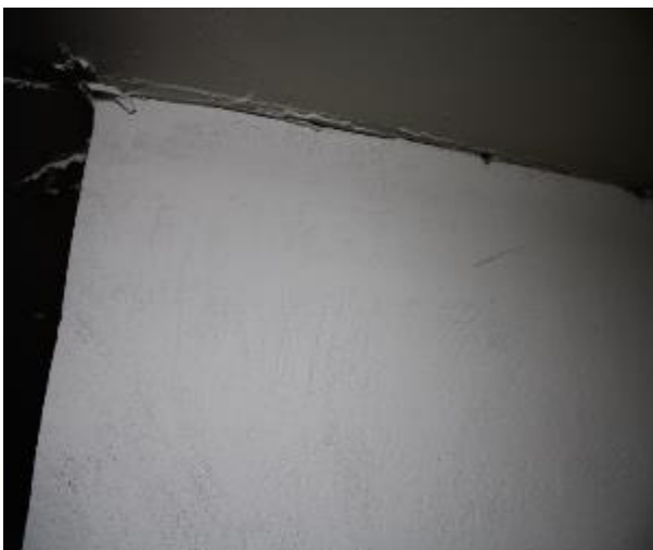
Figure 229 - General condition of level 5 to basement B2 fire stairs internal wall
