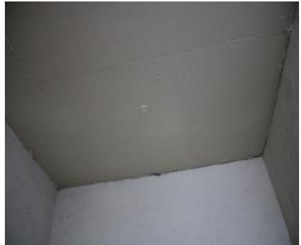
Figure 246 - General condition of level 5 to basement B2 fire stairs underside slab
