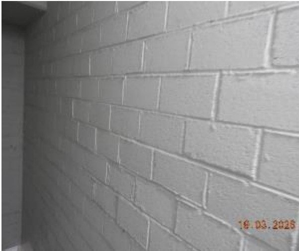
Figure 203 - General condition of B2 to Level 1 fire stairs internal wall
