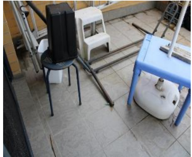
Figure 1515 - General condition of balcony 2 floor tiles
