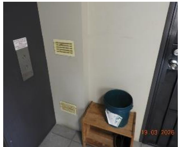
Figure 76 - General condition of level 3 common area internal wall
