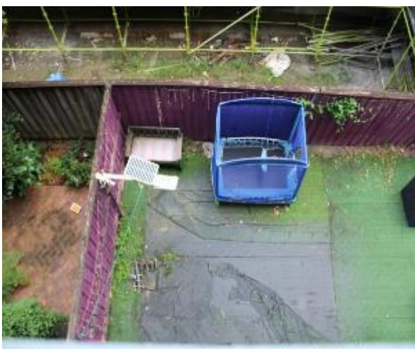
Figure 958 - General condition of boundary fence as seen from Unit 24 balcony
