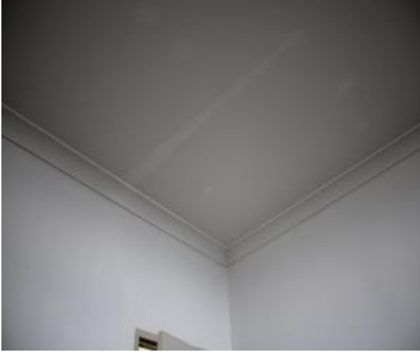
Figure 1338 - General condition of study ceiling
