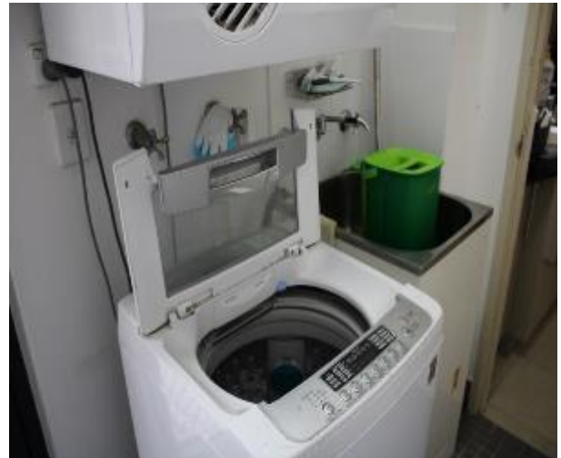
Figure 1263 - General condition of laundry internal wall
