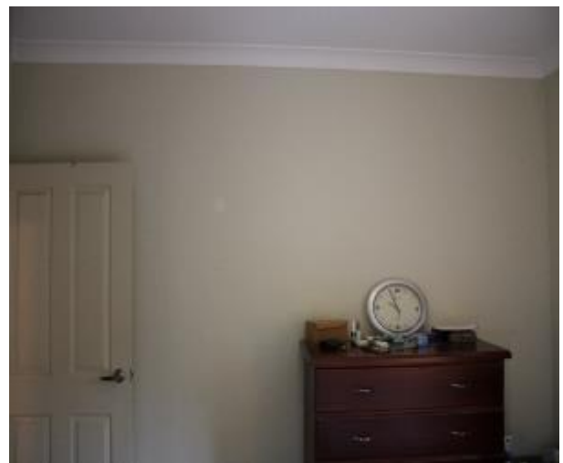
Figure 857 - General condition of bedroom 1 internal wall
