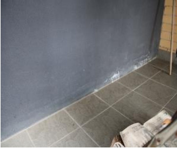
Figure 1224 - General condition of external wall
