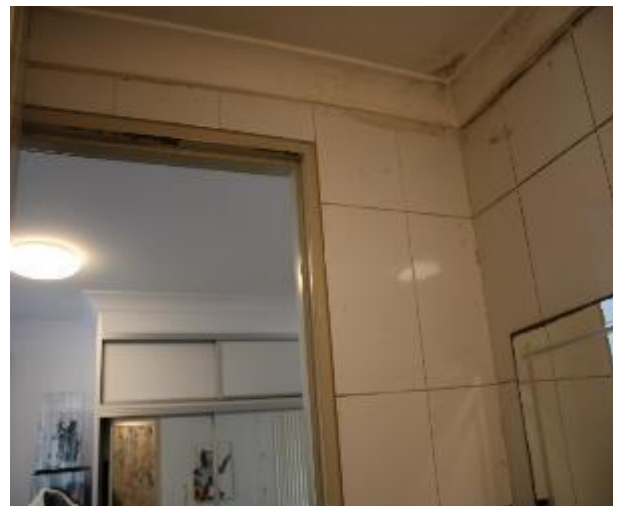
Figure 1383 - General condition of ensuite bathroom internal wall
