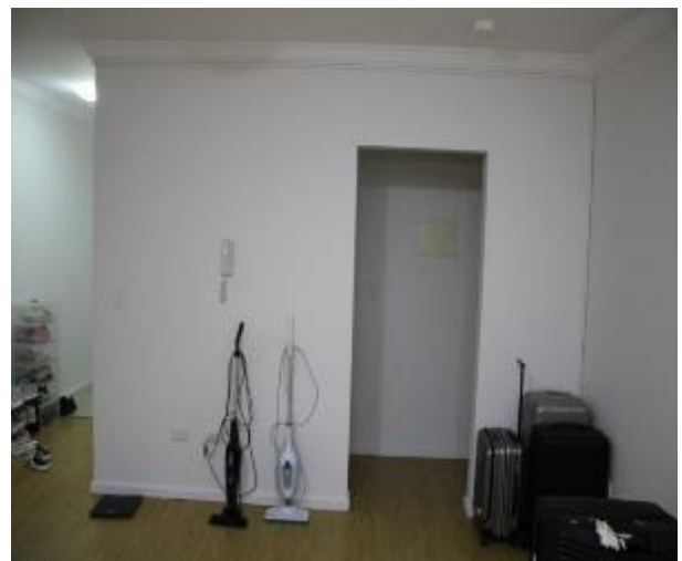
Figure 673 - General condition of kitchen internal wall
