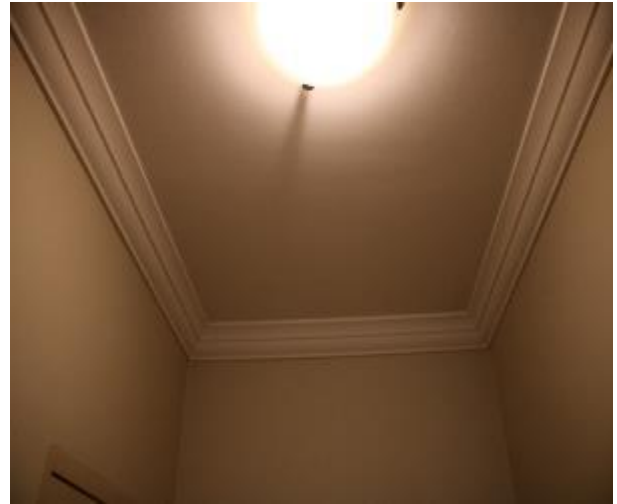
Figure 823 - General condition of open kitchen/ lounge room ceiling
