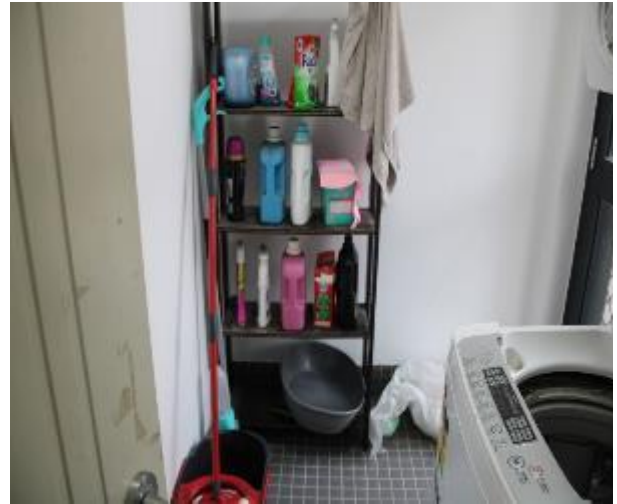
Figure 1261 - General condition of laundry internal wall
