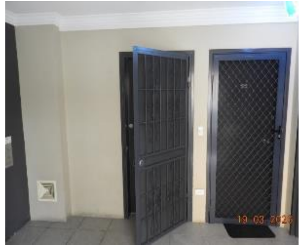
Figure 44 - General condition of level 2 common area internal wall
