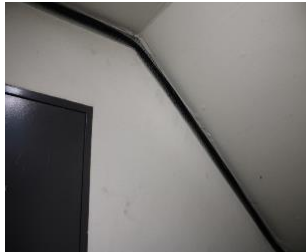
Figure 408 - General condition of level 5 to basement B2 fire stairs internal wall
