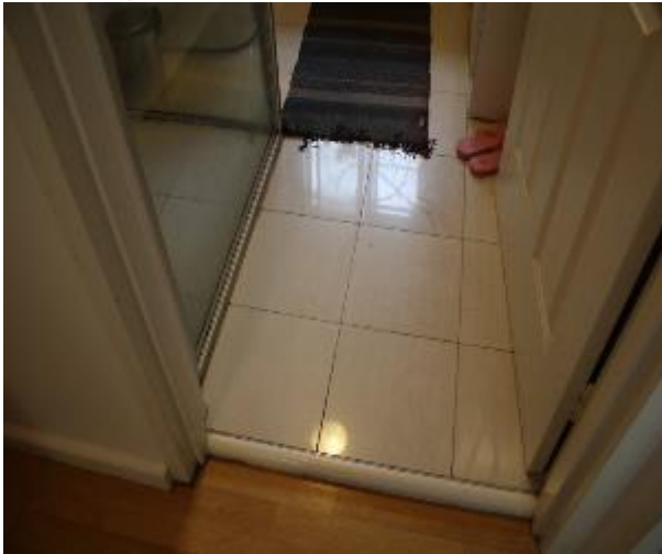
Figure 1029 - General condition of bathroom 1 floor tiles
