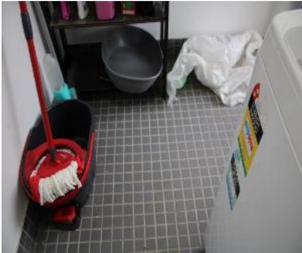
Figure 1260 - General condition of laundry floor tiles
