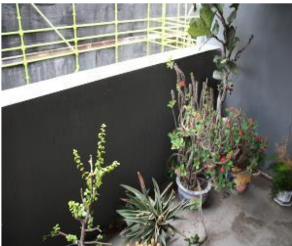
Figure 1069 - General condition of external wall
