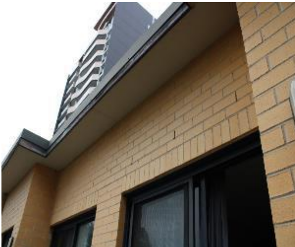
Figure 1576 - General condition of external wall
