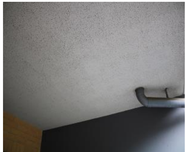
Figure 957 - General condition of balcony underside slab
