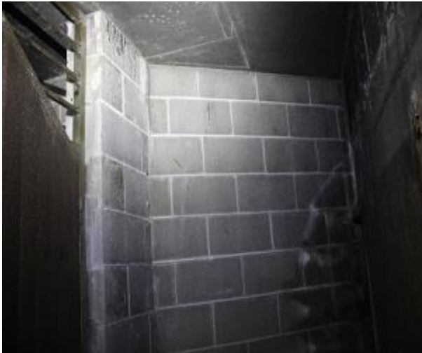
Figure 459 - General condition of basement B2 fire stairs internal wall
