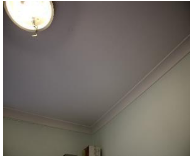
Figure 1209 - General condition of study ceiling
