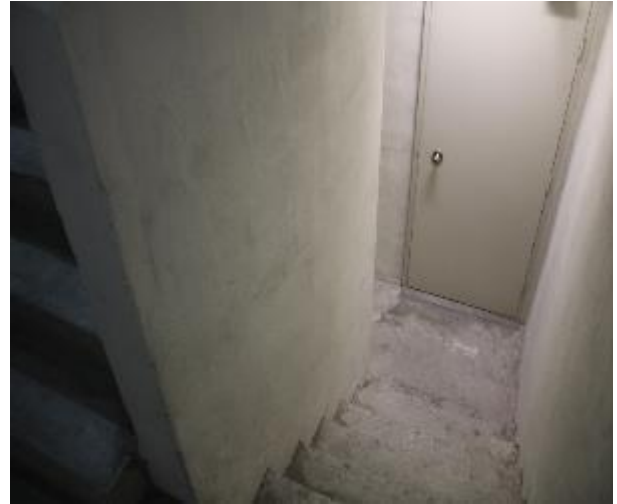
Figure 270 - General condition of level 5 to basement B2 fire stairs internal wall
