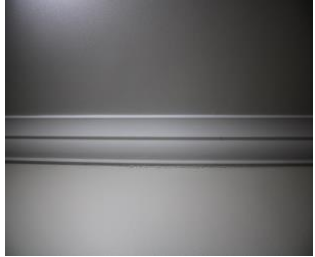
Figure 515 - Crack propagation through open kitchen/ lounge room ceiling
