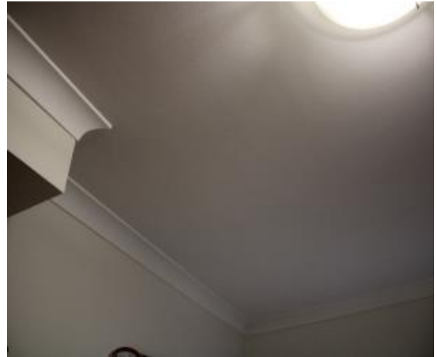
Figure 1000 - General condition of study ceiling
