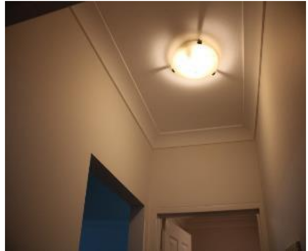
Figure 687 - General condition of corridor ceiling
