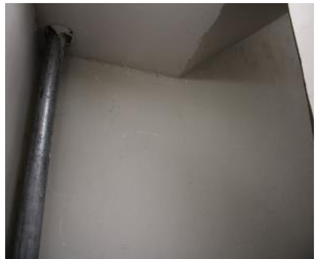
Figure 360 - General condition of level 5 to basement B2 fire stairs internal wall
