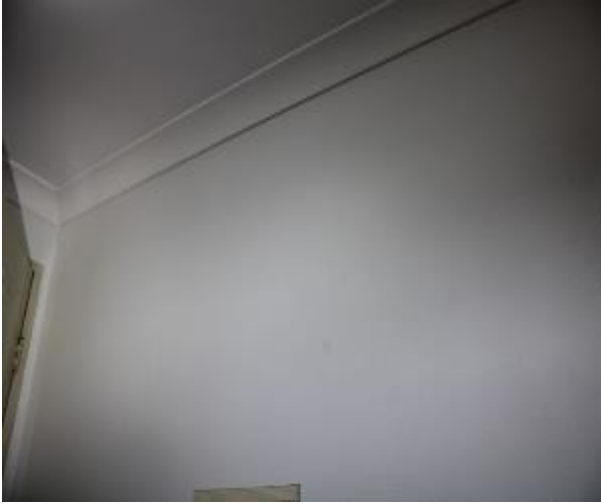
Figure 1266 - General condition of laundry internal wall
