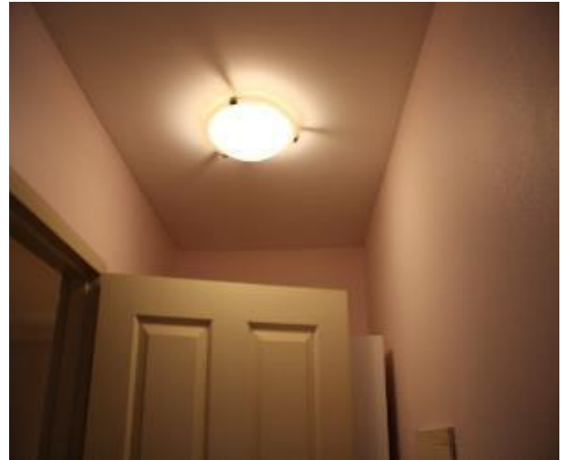
Figure 1135 - General condition of bedroom 1 ceiling
