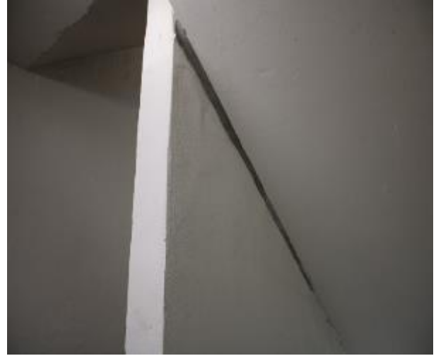
Figure 376 - General condition of level 5 to basement B2 fire stairs internal wall
