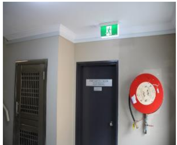
Figure 100 - General condition of level 4 common area internal wall
