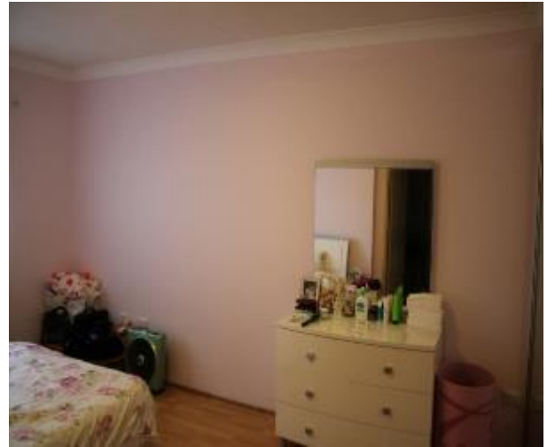
Figure 1129 - General condition of bedroom 1 internal wall
