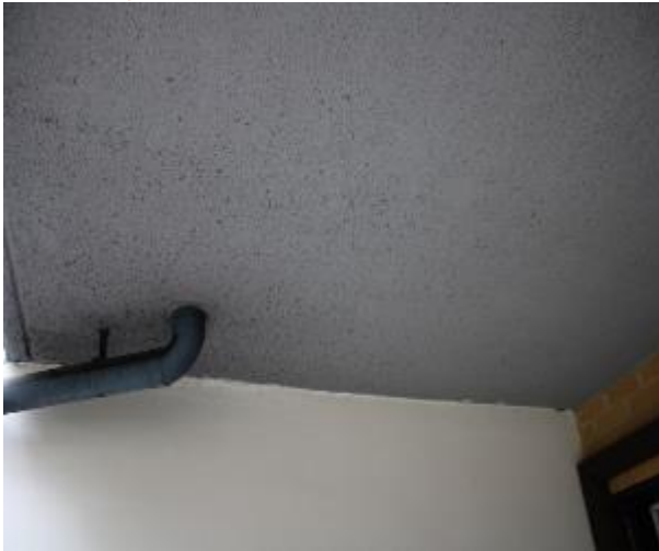
Figure 794 - General condition of balcony underside slab
