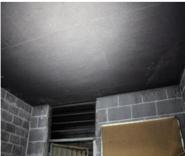
Figure 449 - General condition of basement B2 fire stairs underside slab
