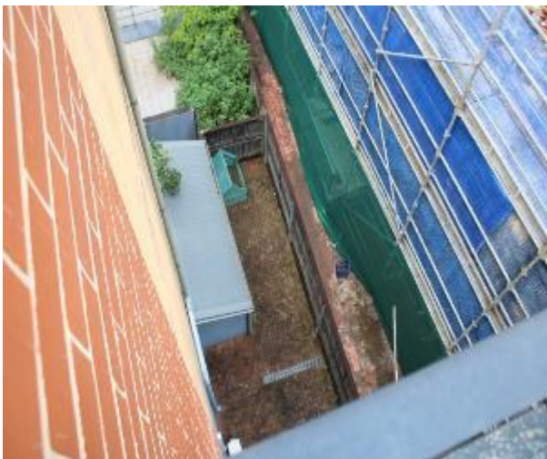
Figure 1510 - General condition of boundary as seen from Unit 29 balcony 1
