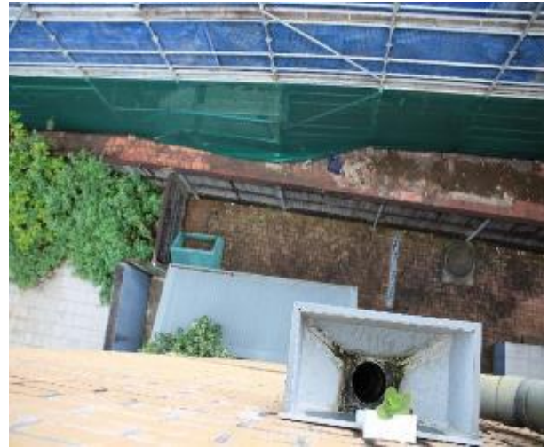
Figure 1527 - General condition of boundary as seen from Unit 29 balcony 2
