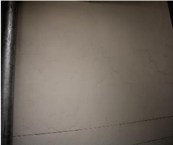
Figure 309 - General condition of level 5 to basement B2 fire stairs internal wall
