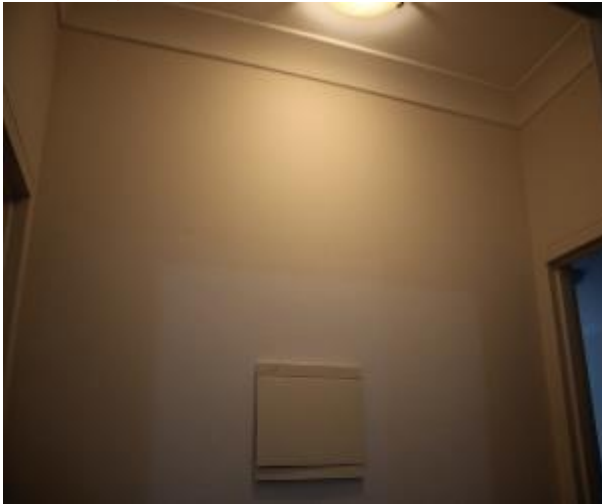
Figure 686 - General condition of corridor internal wall
