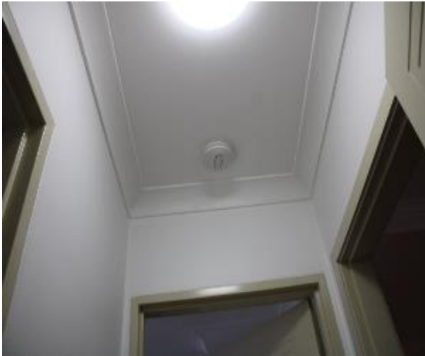
Figure 1326 - General condition of corridor ceiling
