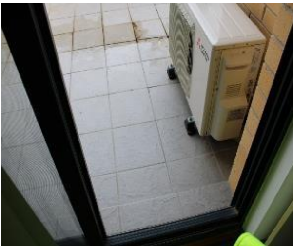
Figure 1388 - General condition of balcony 3 floor tiles
