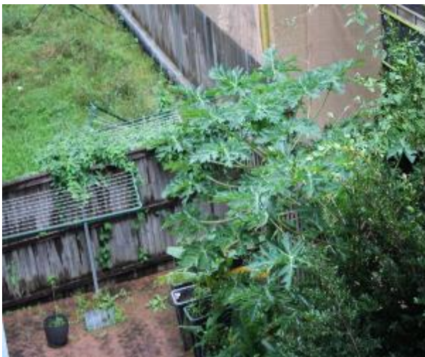
Figure 962 - General condition of boundary fence as seen from Unit 24 balcony
