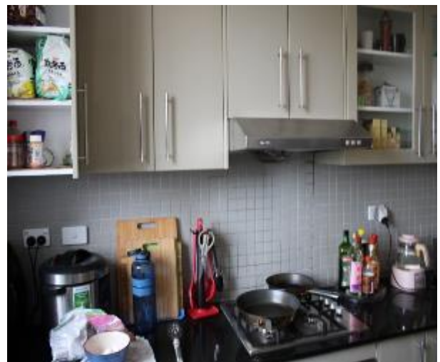
Figure 1253 - General condition of kitchen internal wall
