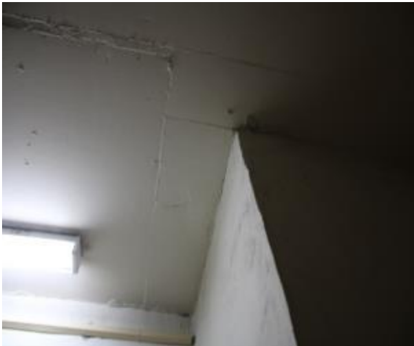
Figure 245 - General condition of level 5 to basement B2 fire stairs underside slab
