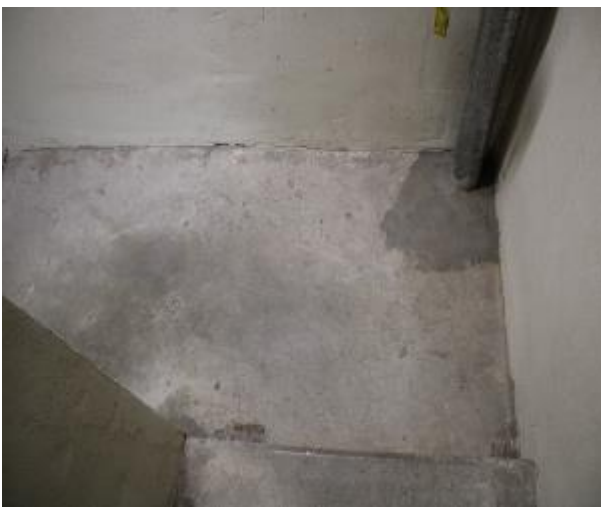
Figure 355 - General condition of level 5 to basement B2 fire stairs
