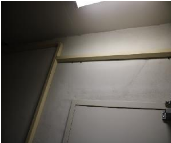
Figure 281 - General condition of level 5 to basement B2 fire stairs internal wall
