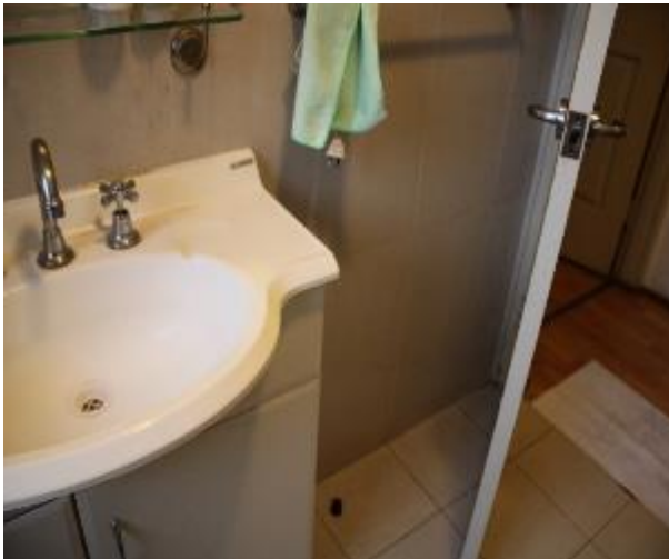
Figure 1190 - General condition of bathroom 1 internal wall
