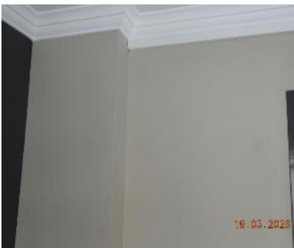
Figure 47 - General condition of level 2 common area internal wall
