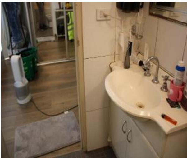
Figure 1382 - General condition of ensuite bathroom internal wall
