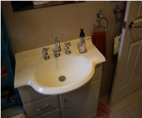
Figure 1043 - General condition of bathroom 1 internal wall
