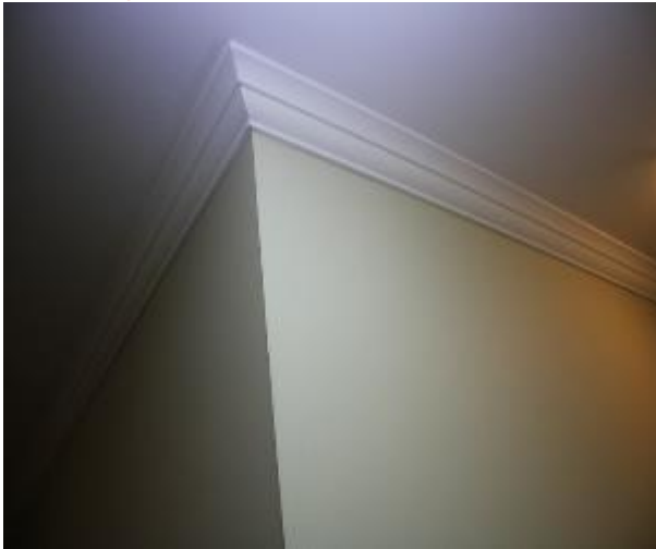
Figure 822 - General condition of open kitchen/ lounge room internal wall
