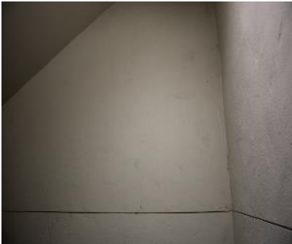
Figure 317 - General condition of level 5 to basement B2 fire stairs internal wall
