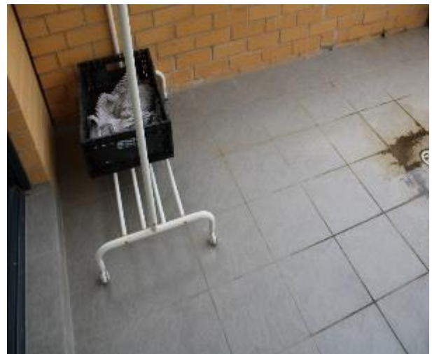
Figure 1389 - General condition of balcony 3 floor tiles
