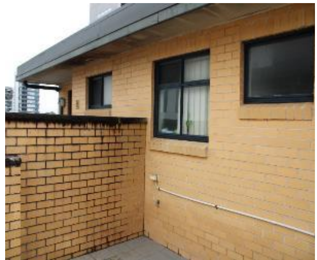
Figure 1395 - General condition of external wall
