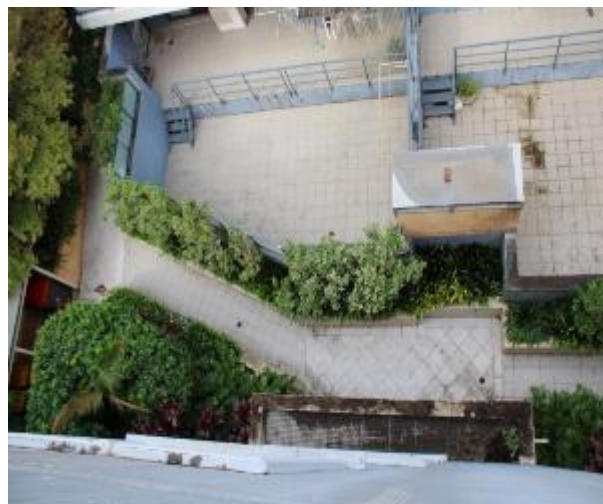
Figure 1417 - General condition of boundary as seen from Unit 28 balcony
