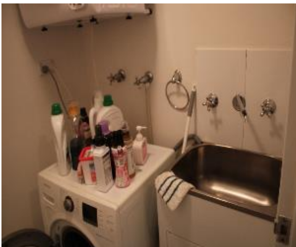
Figure 690 - General condition of laundry internal wall
