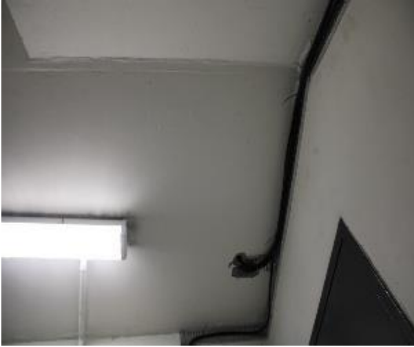
Figure 429 - General condition of level 5 to basement B2 fire stairs underside stairs
