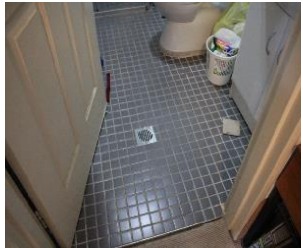
Figure 927 - General condition of ensuite bathroom floor tiles
