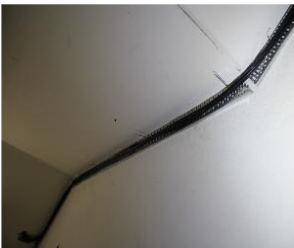
Figure 427 - General condition of level 5 to basement B2 fire stairs underside stairs
