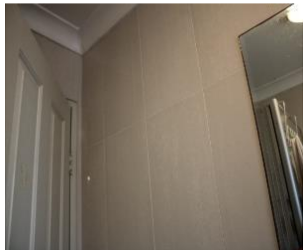
Figure 845 - General condition of bathroom 1 internal wall
