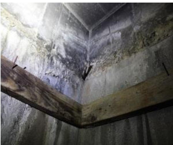
Figure 475 - General condition of basement B2 fire stairs internal wall
