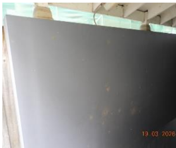
Figure 160 - General condition of B2 to Level 1 fire stairs internal wall
