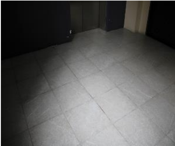
Figure 85 - General condition of level 4 common area floor tiles
