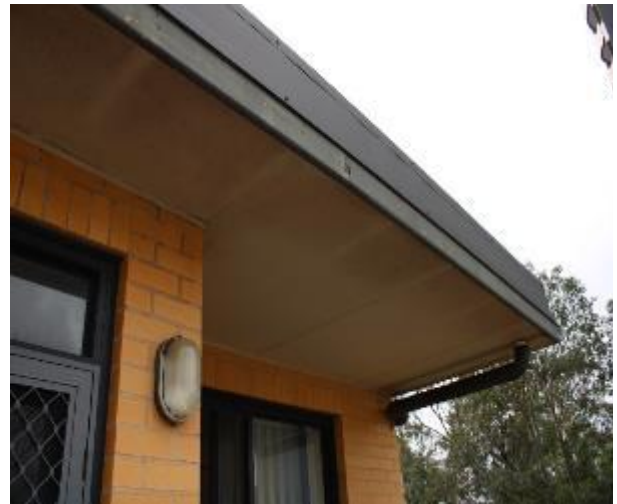
Figure 1413 - General condition of balcony underside slab
