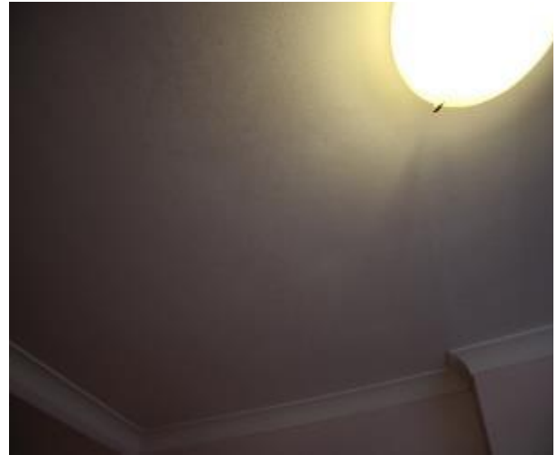
Figure 1141 - General condition of bedroom 1 ceiling
