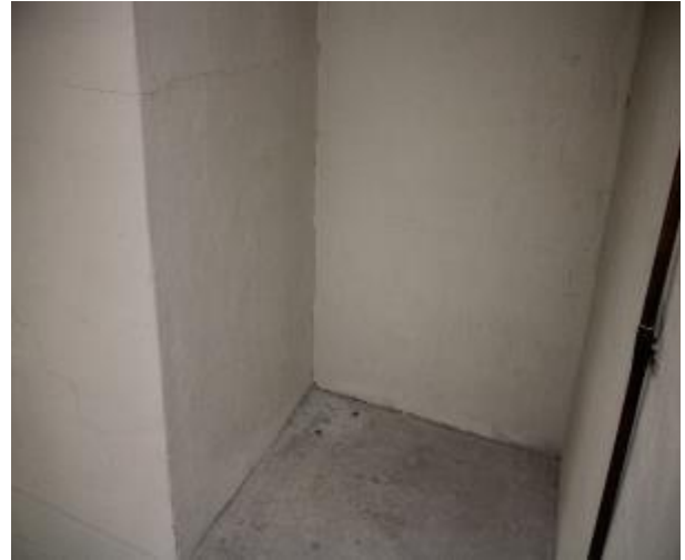
Figure 288 - General condition of level 5 to basement B2 fire stairs internal wall
