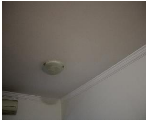
Figure 978 - General condition of lounge room ceiling
