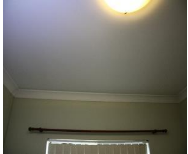
Figure 891 - General condition of bedroom 2 ceiling
