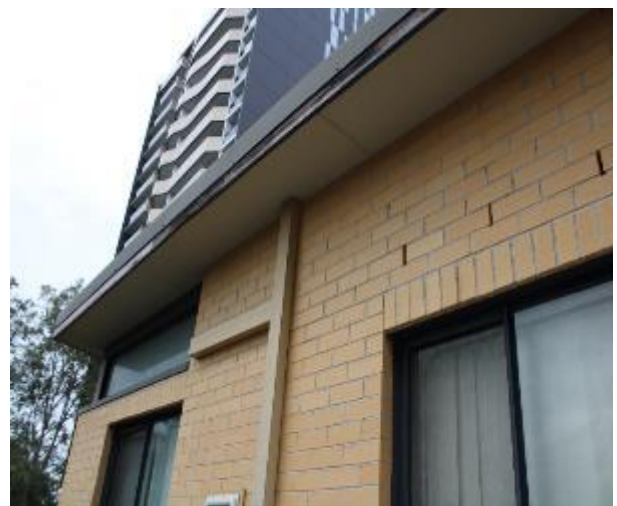
Figure 1301 - General condition of external wall
