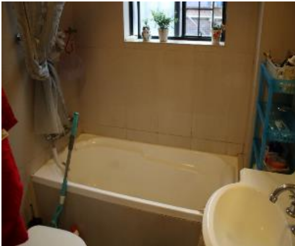
Figure 1031 - General condition of bathroom 1 internal wall
