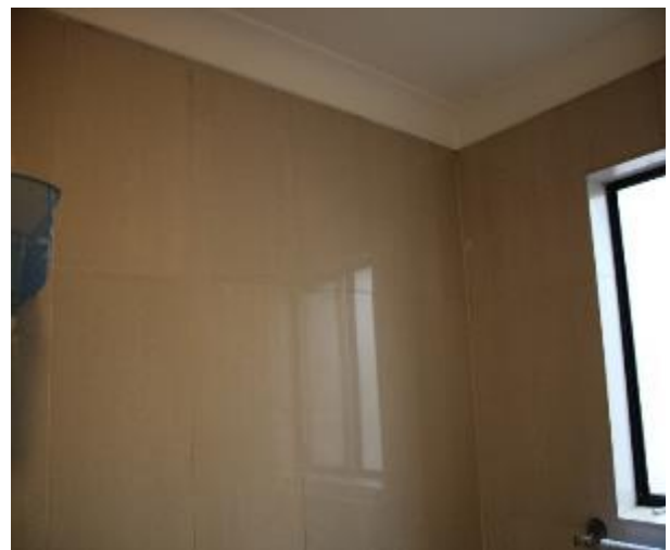
Figure 1187 - General condition of bathroom 1 internal wall
