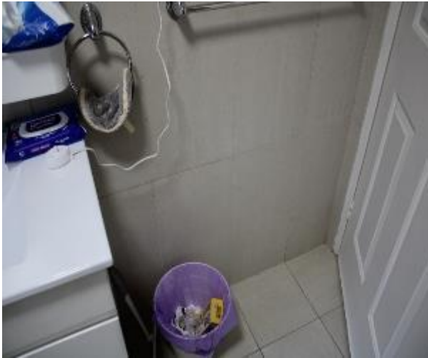
Figure 752 - General condition of bathroom 1 internal wall
