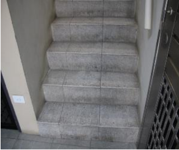
Figure 115 - General condition of staircase to level 5 common area
