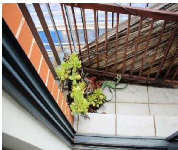
Figure 1507 - General condition of balcony 1 floor tiles
