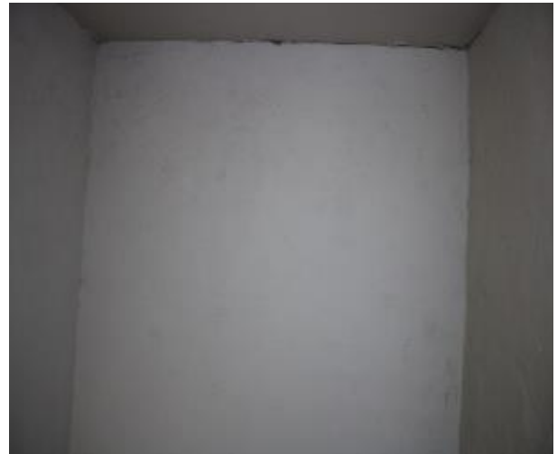
Figure 252 - General condition of level 5 to basement B2 fire stairs internal wall
