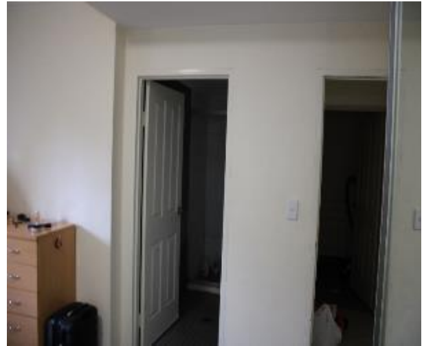
Figure 551 - General condition of bedroom 1 internal wall
