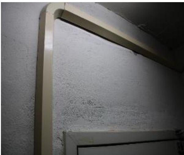
Figure 235 - General condition of level 5 to basement B2 fire stairs internal wall
