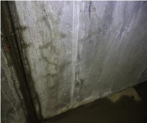
Figure 471 - General condition of basement B2 fire stairs internal wall
