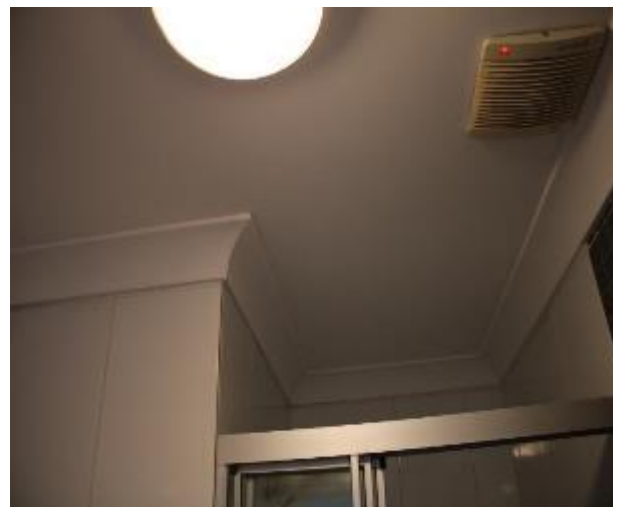
Figure 721 - General condition of ensuite bathroom ceiling
