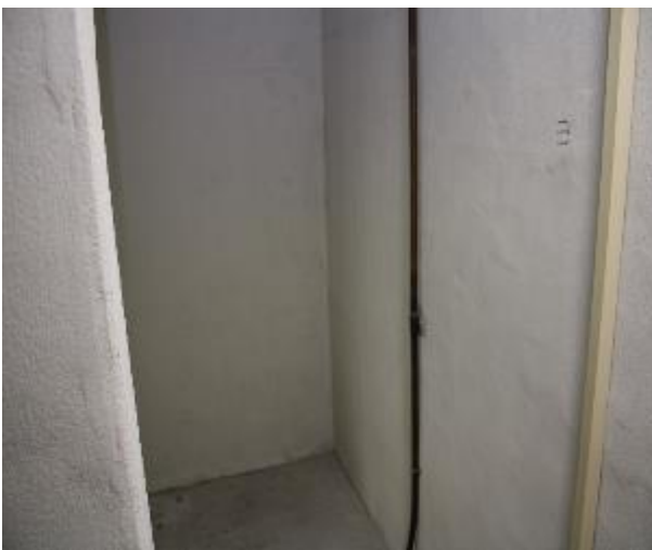
Figure 283 - General condition of level 5 to basement B2 fire stairs internal wall
