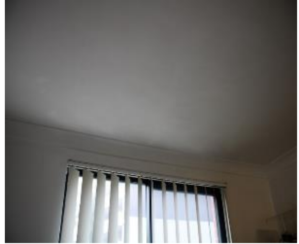
Figure 1369 - General condition of bedroom 2 ceiling
