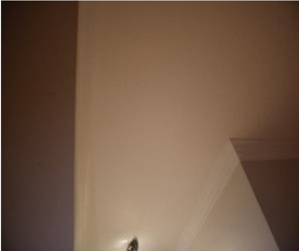
Figure 1106 - General condition of lounge room ceiling
