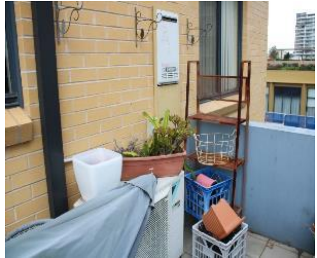
Figure 1569 - General condition of external wall
