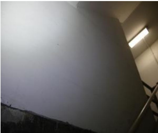
Figure 419 - General condition of level 5 to basement B2 fire stairs internal wall
