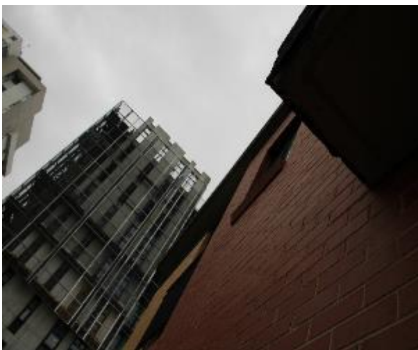
Figure 1216 - General condition of external wall
