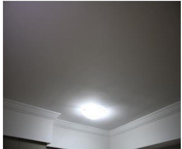
Figure 683 - General condition of kitchen ceiling
