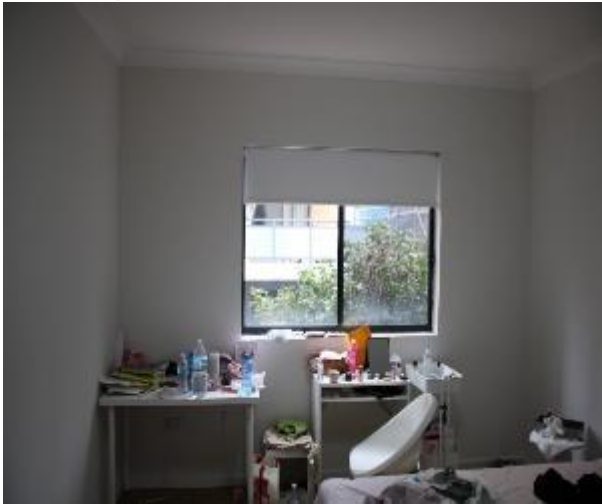
Figure 698 - General condition of bedroom 1 internal wall
