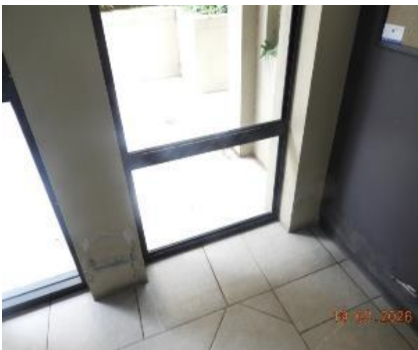
Figure 11 - General condition of level 1 common area internal wall
