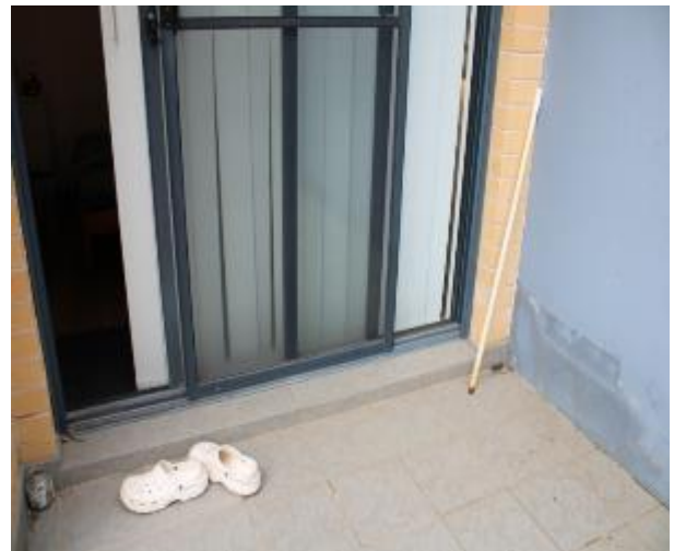
Figure 1295 - General condition of external wall
