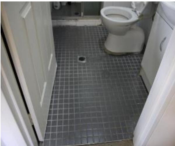
Figure 560 - General condition of ensuite bathroom floor tiles
