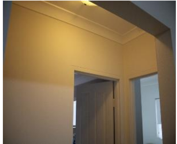
Figure 723 - General condition of corridor internal wall
