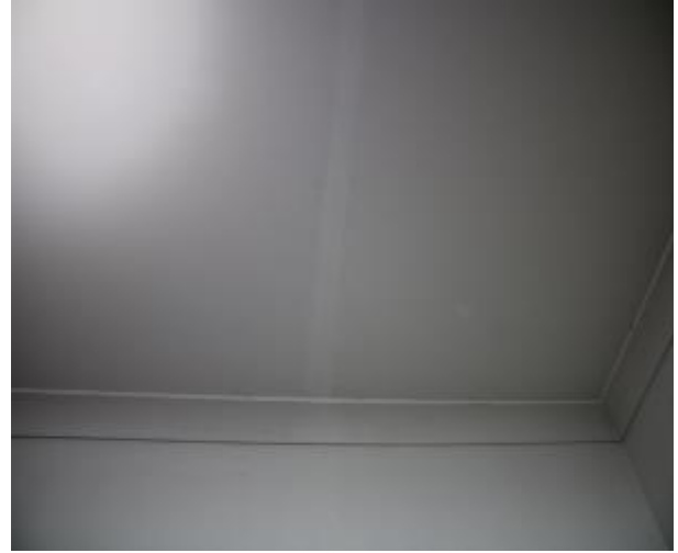
Figure 1339 - General condition of study ceiling
