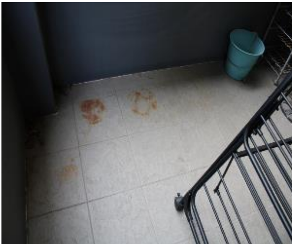
Figure 938 - General condition of balcony floor tiles
