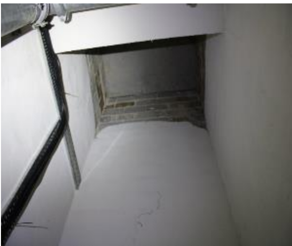
Figure 415 - General condition of level 5 to basement B2 fire stairs internal wall
