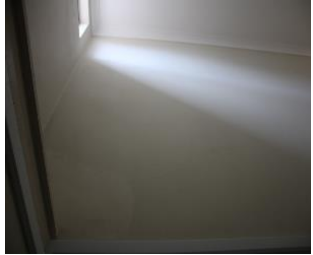
Figure 122 - General condition of staircase to level 5 common area internal wall
