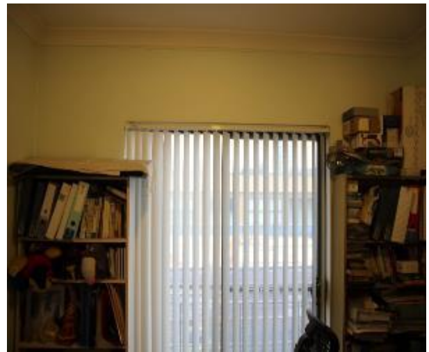
Figure 1197 - General condition of study internal wall
