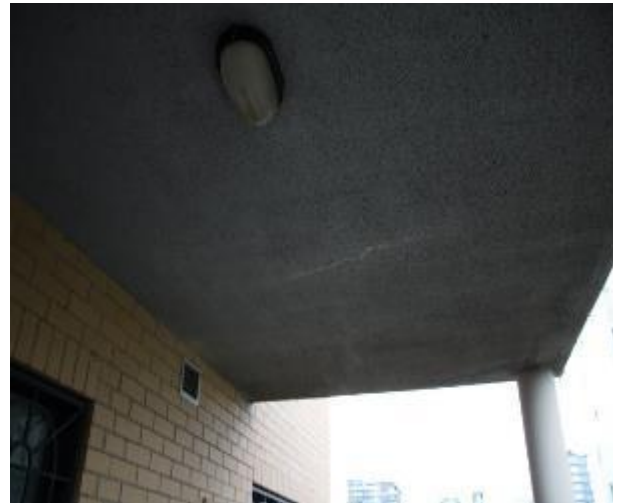
Figure 1245 - General condition of balcony underside slab
