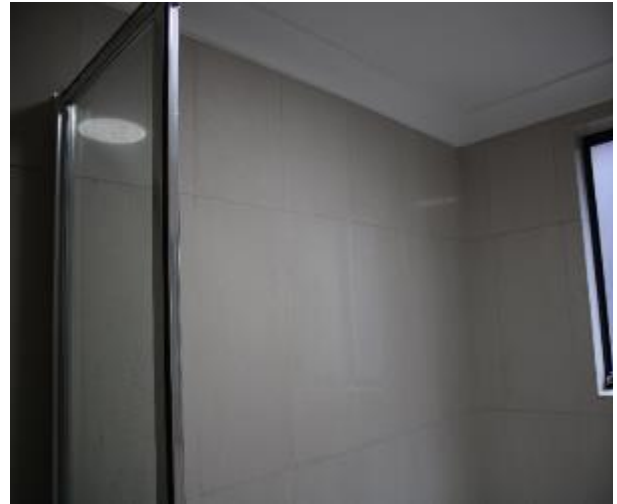
Figure 747 - General condition of bathroom 1 internal wall
