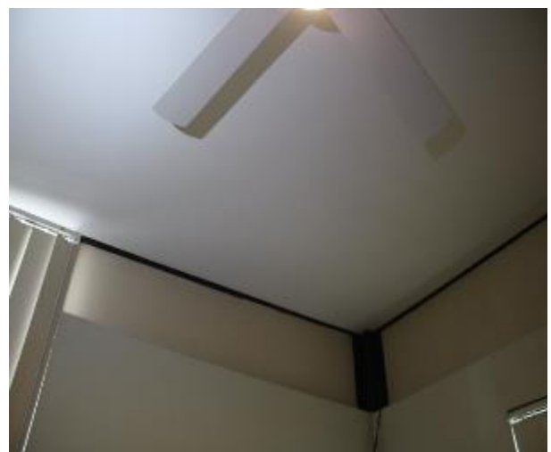
Figure 1561 - General condition of bedroom 2 ceiling
