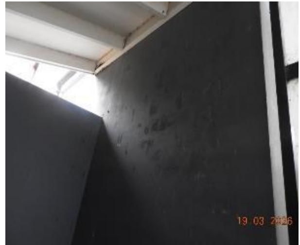
Figure 164 - General condition of B2 to Level 1 fire stairs internal wall
