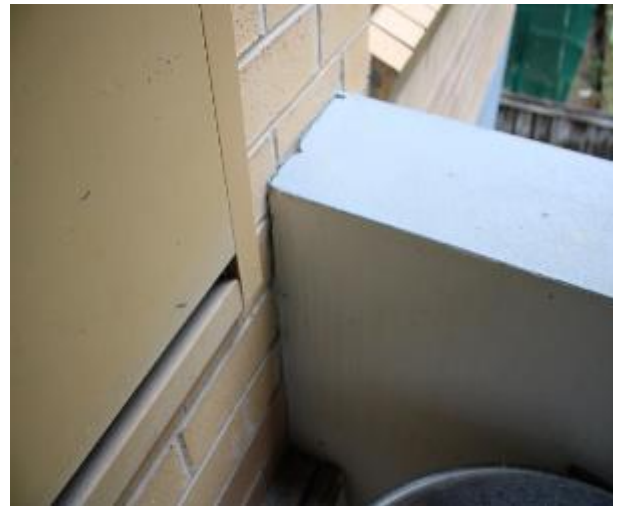
Figure 791 - General condition of external wall
