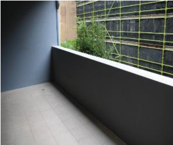
Figure 648 - General condition of external wall
