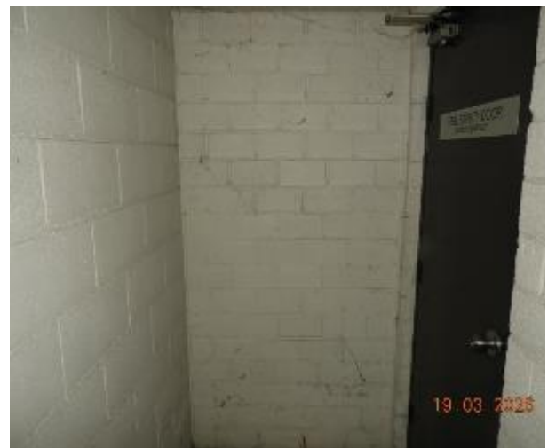
Figure 178 - General condition of B2 to Level 1 fire stairs internal wall
