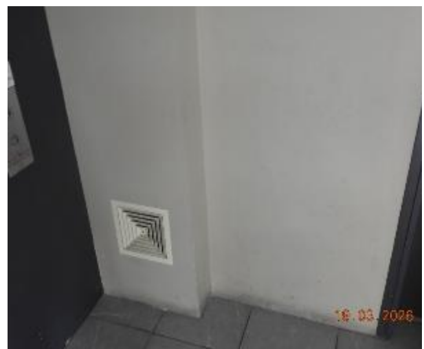
Figure 48 - General condition of level 2 common area internal wall
