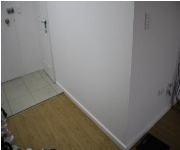
Figure 664 - General condition of kitchen internal wall
