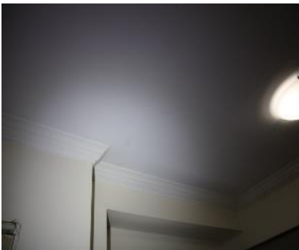
Figure 524 - General condition of open kitchen/ lounge room ceiling
