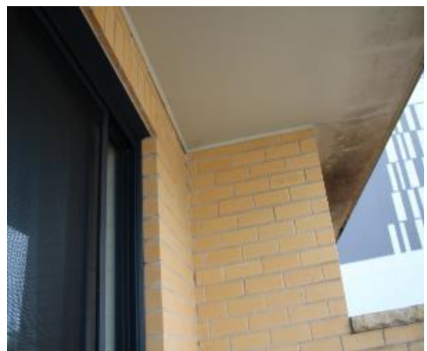
Figure 1519 - General condition of external wall
