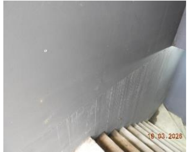
Figure 168 - General condition of B2 to Level 1 fire stairs internal wall
