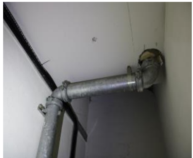
Figure 426 - General condition of level 5 to basement B2 fire stairs underside stairs
