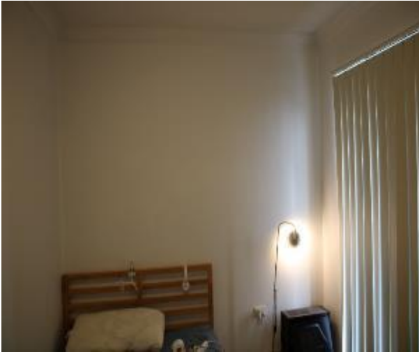
Figure 1280 - General condition of bedroom 1 internal wall
