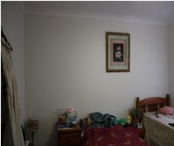
Figure 1049 - General condition of bedroom 2 internal wall
