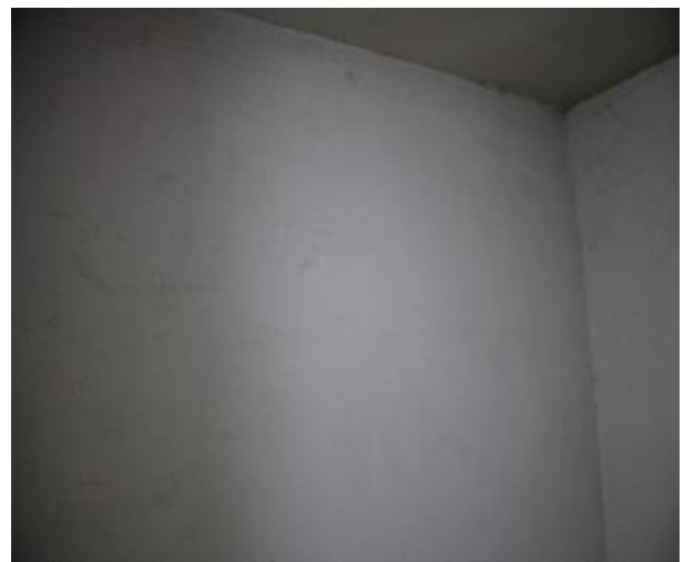
Figure 254 - General condition of level 5 to basement B2 fire stairs internal wall
