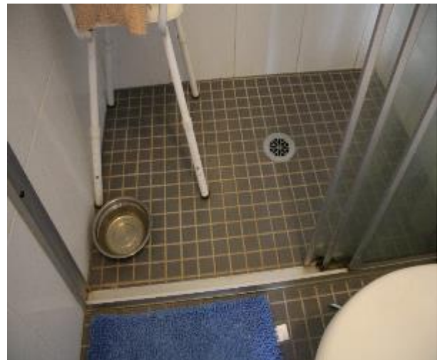
Figure 1495 - General condition of ensuite bathroom floor tiles
