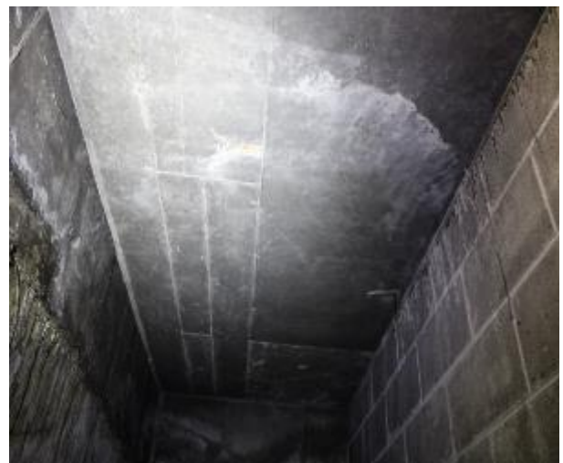
Figure 482 - General condition of basement B2 fire stairs underside slab
