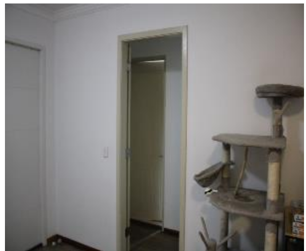
Figure 1271 - General condition of dining room internal wall
