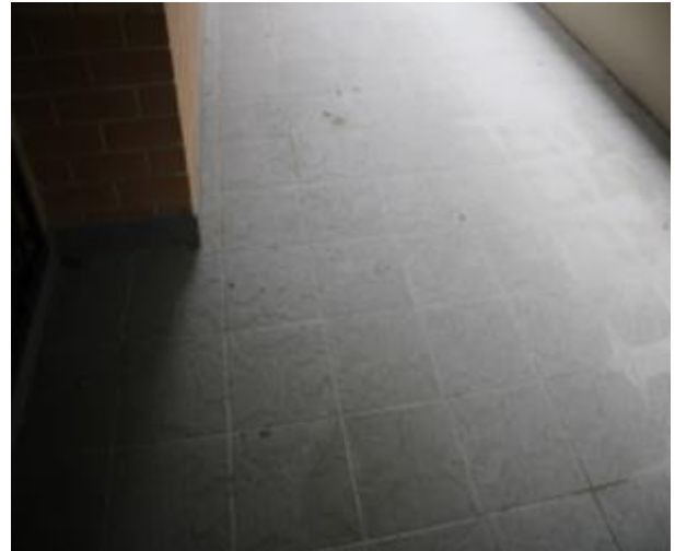
Figure 773 - General condition of balcony floor tiles
