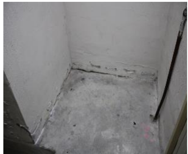
Figure 224 - General condition of level 5 to basement B2 fire stairs
