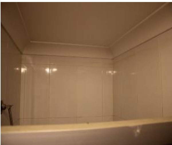
Figure 1150 - General condition of ensuite bathroom internal wall
