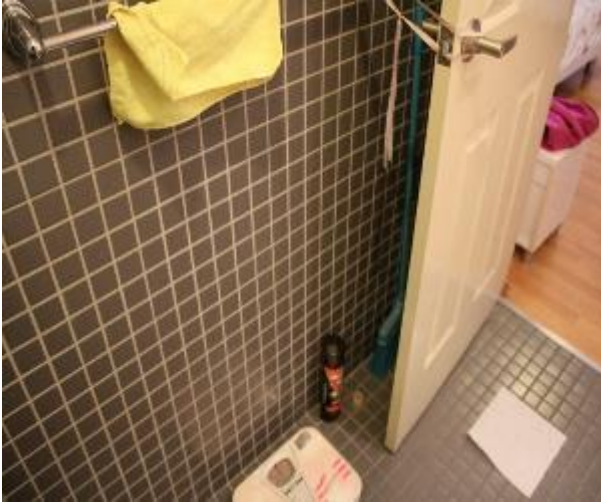
Figure 1152 - General condition of ensuite bathroom internal wall
