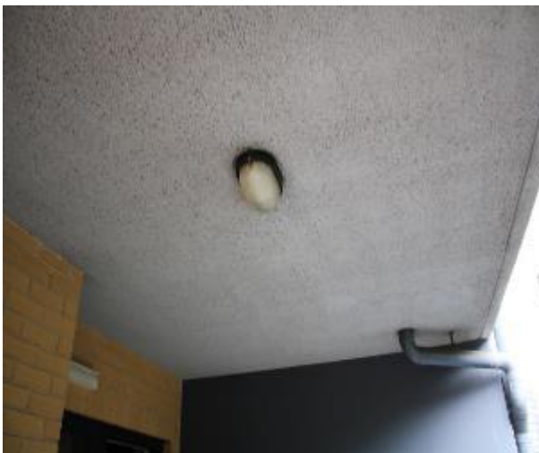
Figure 956 - General condition of balcony underside slab
