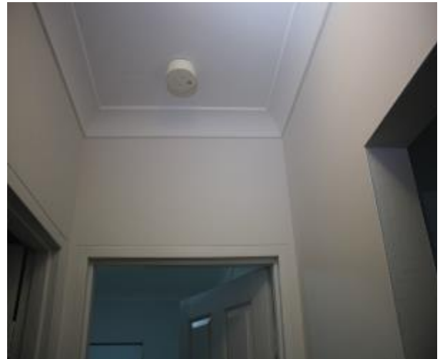
Figure 725 - General condition of corridor internal wall
