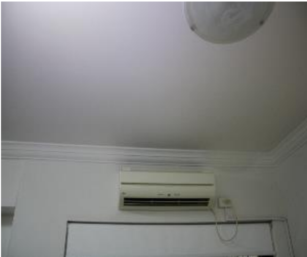
Figure 682 - General condition of kitchen ceiling
