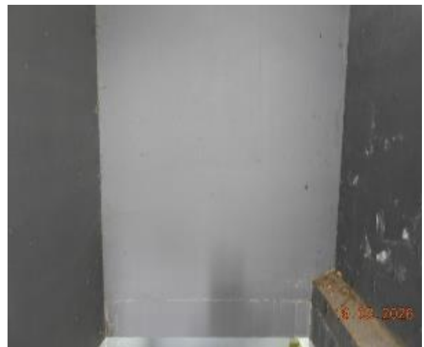
Figure 166 - General condition of B2 to Level 1 fire stairs internal wall
