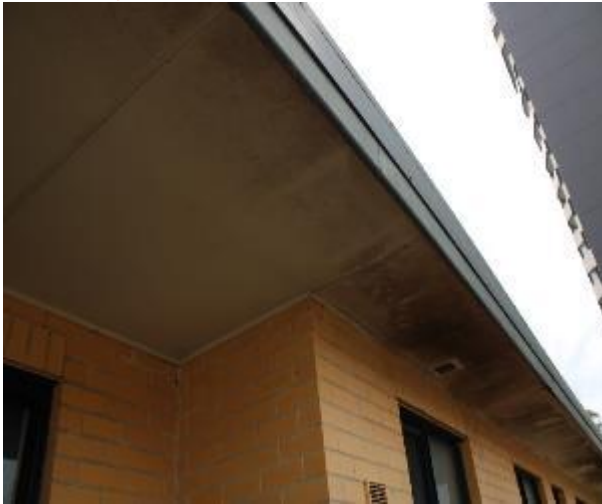
Figure 1526 - General condition of balcony underside slab
