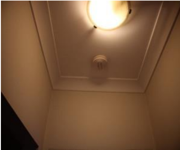
Figure 1164 - General condition of corridor ceiling
