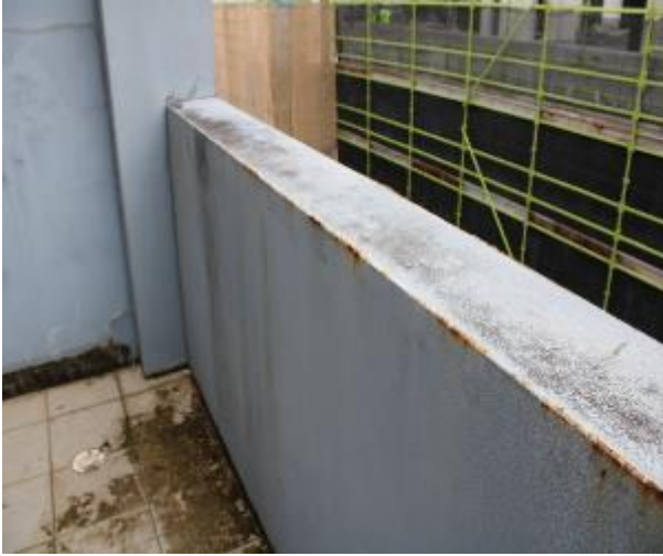
Figure 1308 - General condition of external wall
