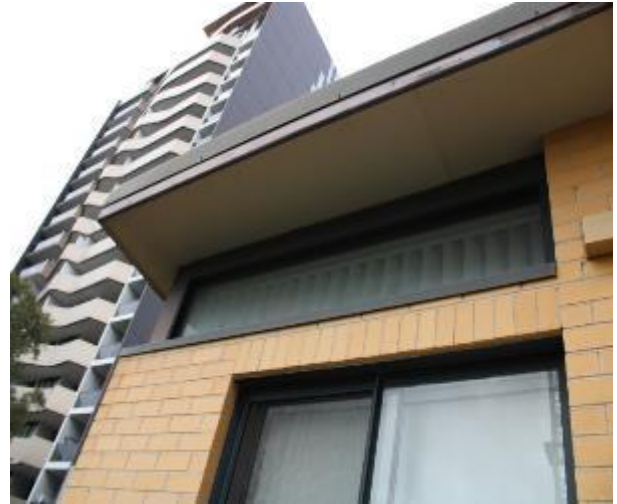
Figure 1321 - General condition of external wall
