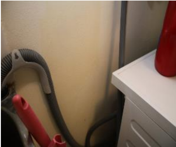
Figure 538 - General condition of laundry internal wall
