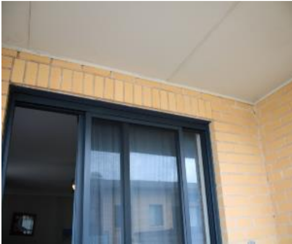
Figure 1520 - General condition of external wall
