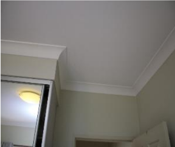
Figure 860 - General condition of bedroom 1 ceiling
