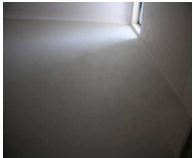
Figure 126 - General condition of staircase to level 5 common area internal wall
