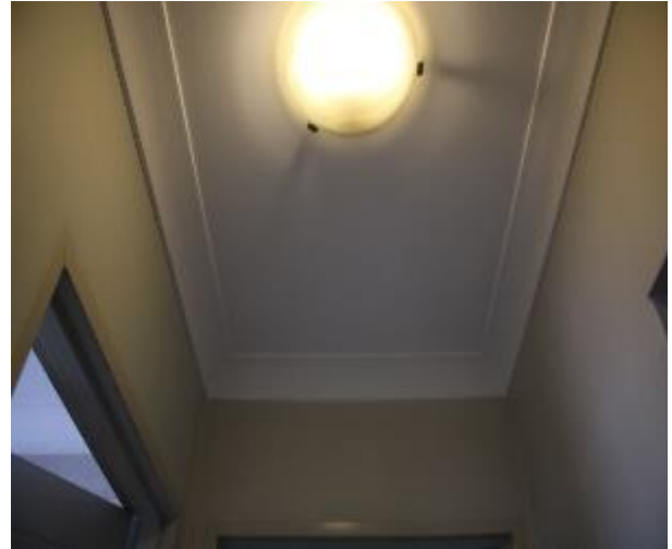
Figure 1469 - General condition of corridor ceiling
