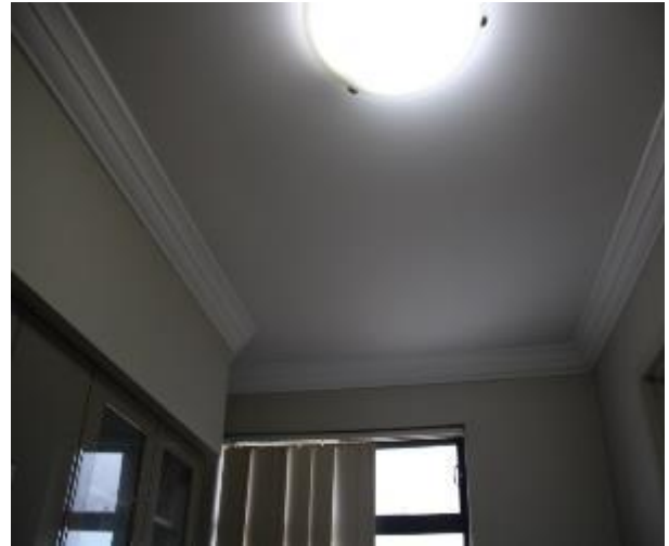
Figure 1431 - General condition of kitchen ceiling
