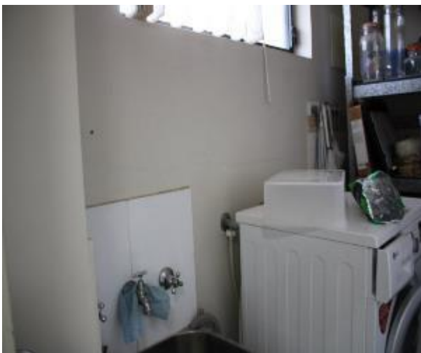
Figure 1434 - General condition of laundry internal wall
