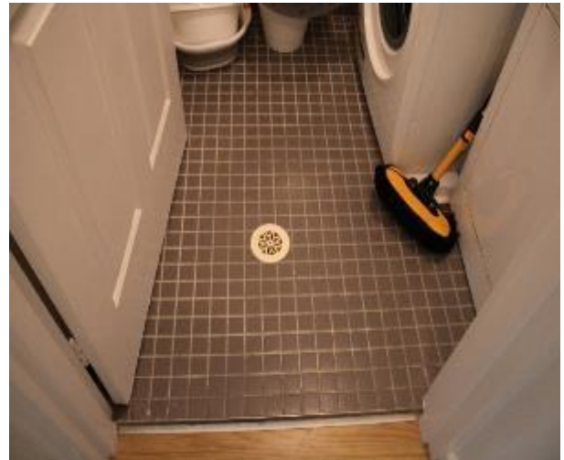
Figure 689 - General condition of laundry floor tiles
