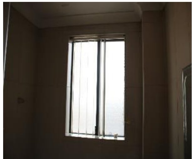
Figure 1535 - General condition of bathroom 1 internal wall
