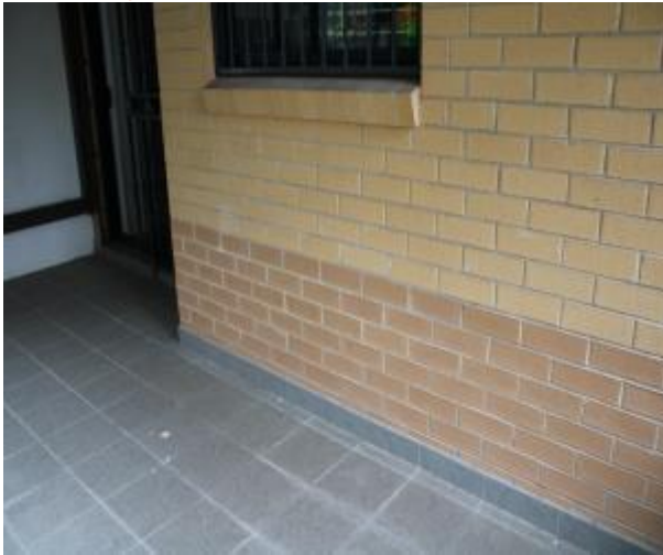
Figure 776 - General condition of external wall
