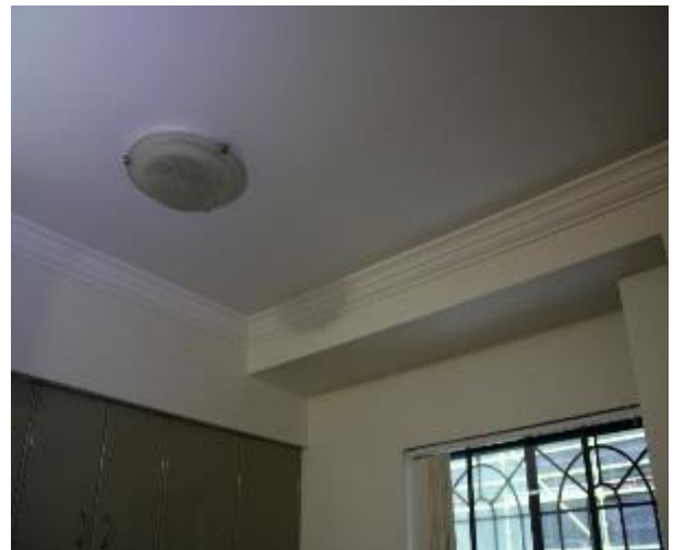
Figure 980 - General condition of lounge room ceiling
