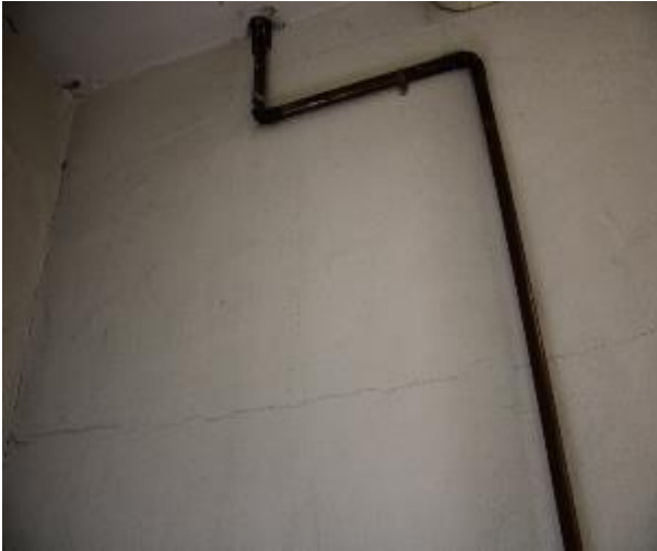
Figure 287 - General condition of level 5 to basement B2 fire stairs internal wall
