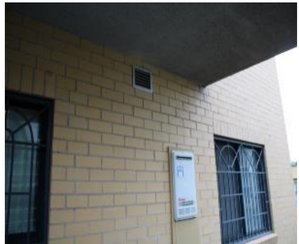
Figure 1229 - General condition of external wall
