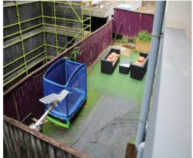
Figure 795 - General condition of boundary fence as seen from Unit 23 balcony
