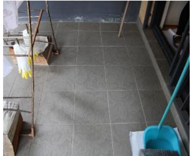
Figure 1219 - General condition of balcony 2 floor tiles
