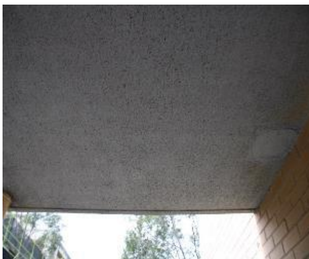
Figure 660 - General condition of balcony underside slab
