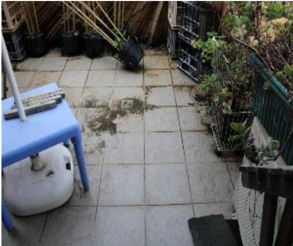
Figure 1514 - General condition of balcony 2 floor tiles
