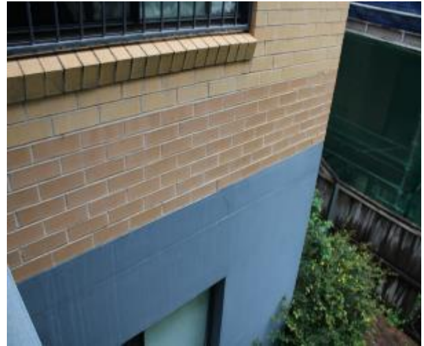
Figure 801 - General condition of external wall
