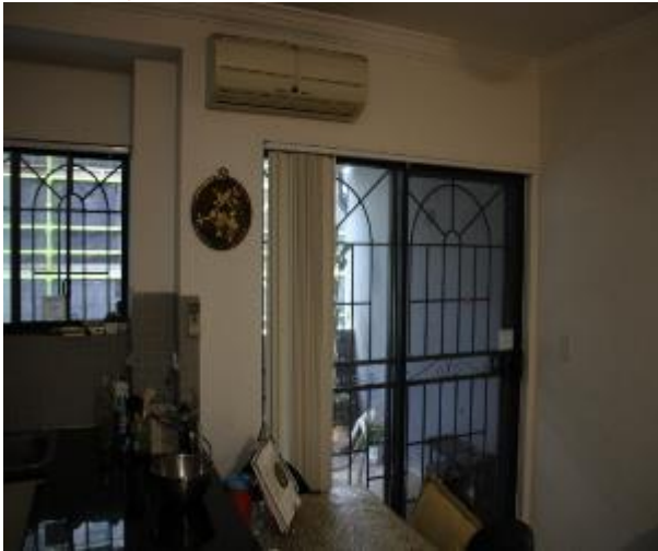
Figure 969 - General condition of lounge room internal wall
