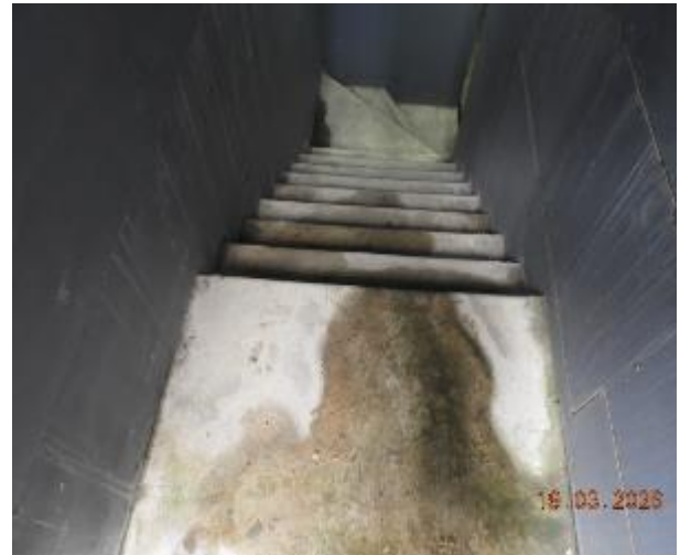
Figure 170 - General condition of
