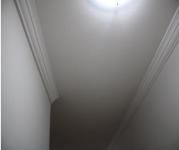
Figure 676 - General condition of kitchen ceiling
