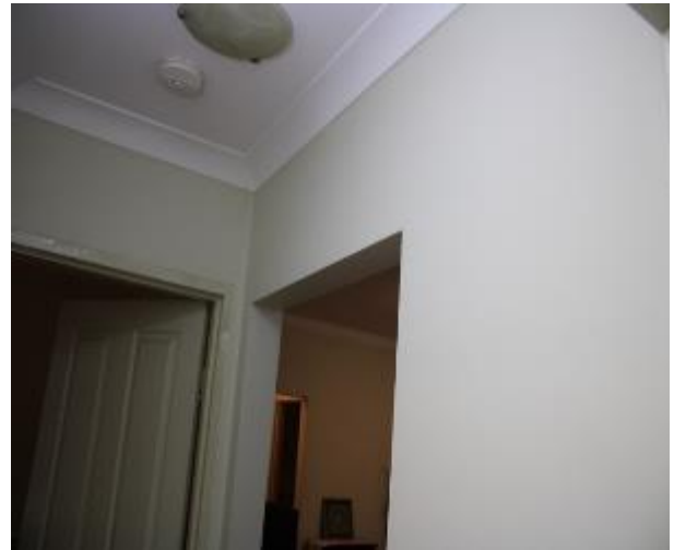
Figure 867 - General condition of corridor internal wall
