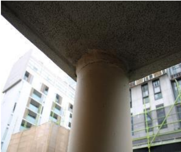
Figure 1077 - General condition of balcony underside slab
