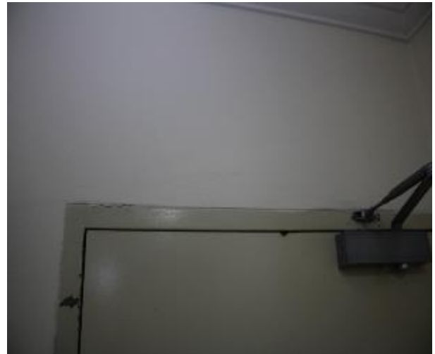
Figure 487 - Crack propagation through open kitchen/ lounge room internal wall
