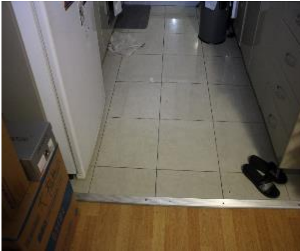
Figure 981 - General condition of kitchen floor tiles
