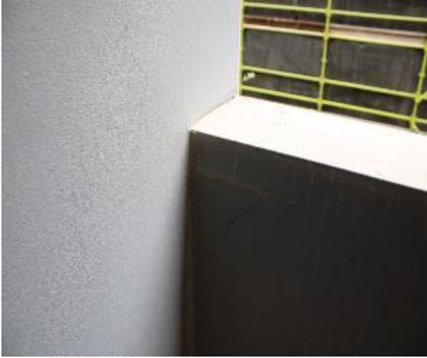
Figure 652 - General condition of external wall
