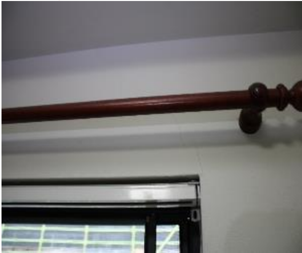
Figure 834 - Crack propagation through kitchen internal wall
