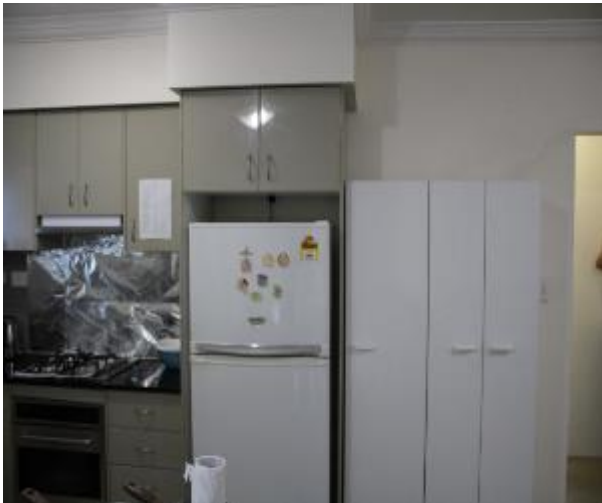
Figure 498 - General condition of open kitchen/ lounge room internal wall
