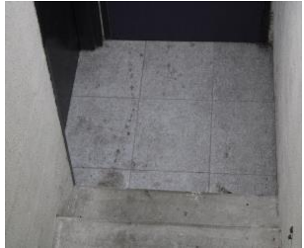
Figure 358 - General condition of level 5 to basement B2 fire stairs
