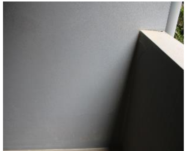
Figure 651 - General condition of external wall
