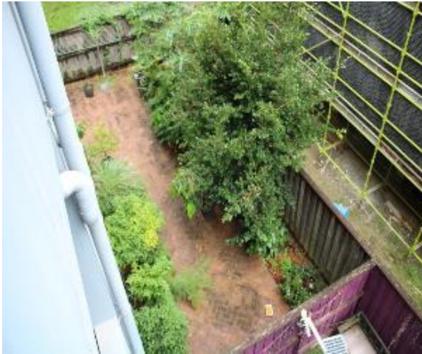
Figure 960 - General condition of boundary fence as seen from Unit 24 balcony
