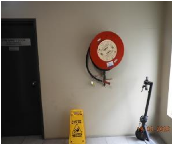
Figure 67 - General condition of level 3 common area internal wall
