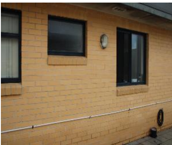
Figure 1396 - General condition of external wall
