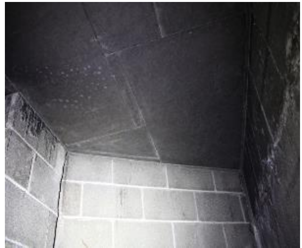
Figure 480 - General condition of basement B2 fire stairs underside slab
