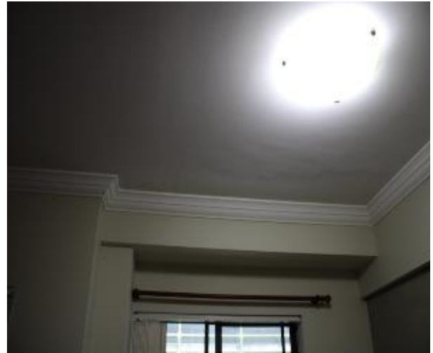
Figure 829 - General condition of open kitchen/ lounge room ceiling
