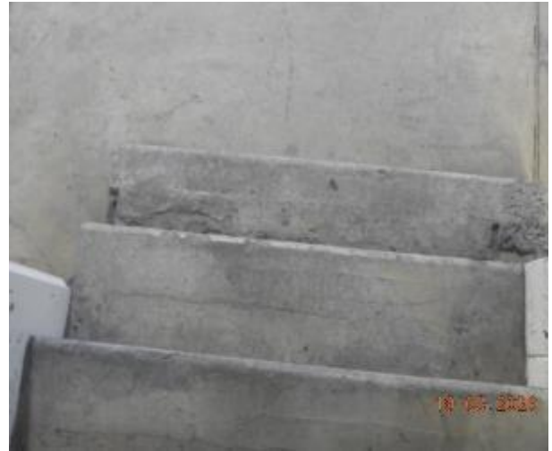
Figure 216 - General condition of B2 to Level 1 fire stairs
