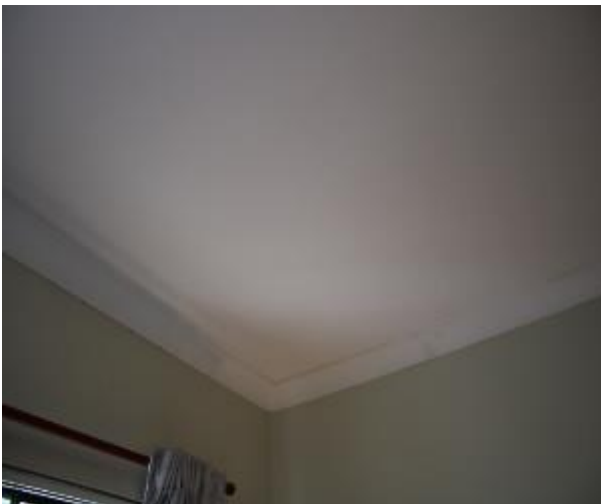
Figure 862 - General condition of bedroom 1 ceiling
