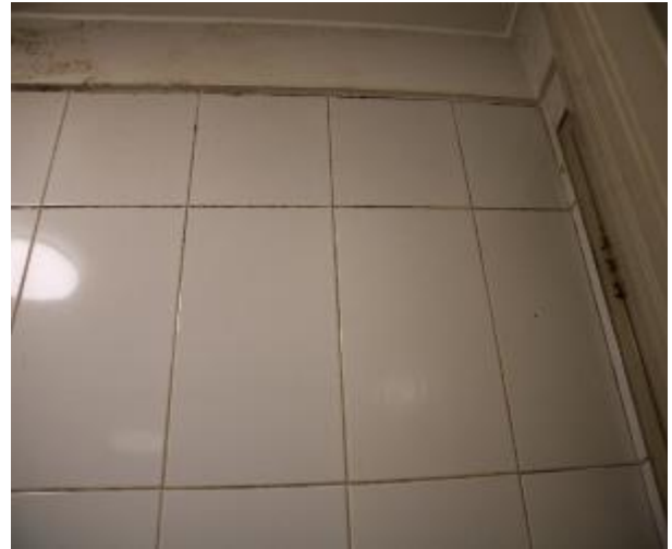
Figure 1381 - General condition of ensuite bathroom internal wall
