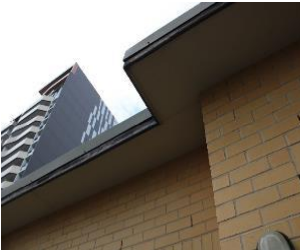
Figure 1594 - General condition of eave
