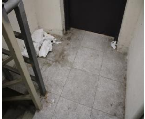
Figure 394 - General condition of level 5 to basement B2 fire stairs
