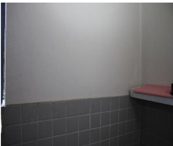
Figure 1422 - General condition of kitchen internal wall
