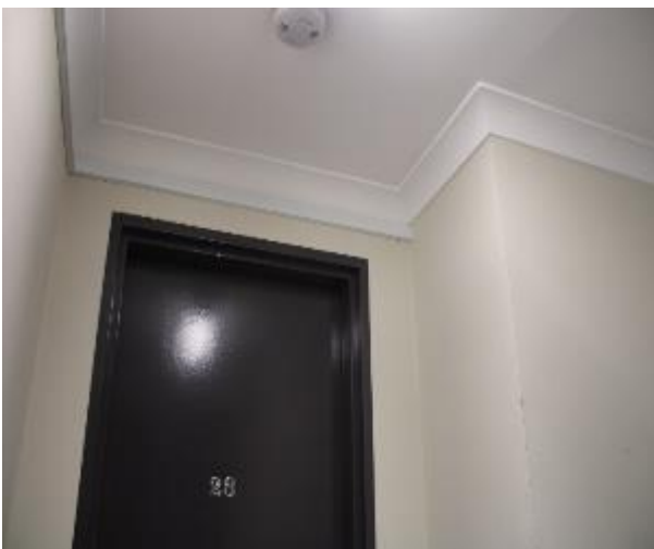
Figure 149 - General condition of level 5 common area internal wall
