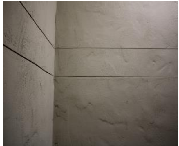
Figure 312 - General condition of level 5 to basement B2 fire stairs internal wall
