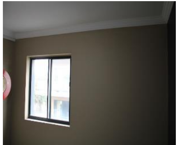
Figure 94 - General condition of level 4 common area internal wall
