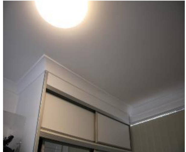
Figure 1371 - General condition of bedroom 2 ceiling
