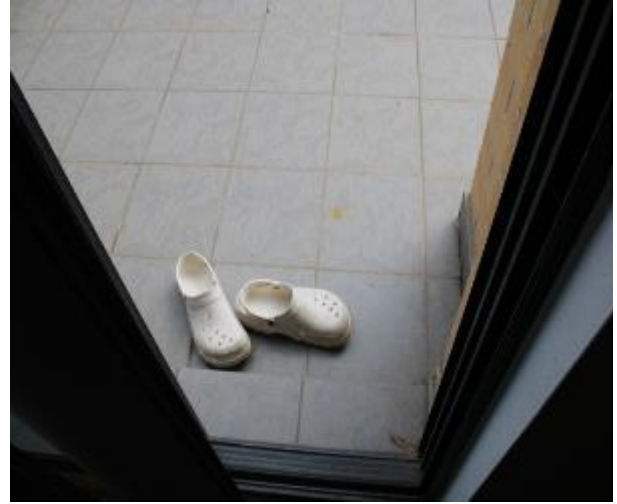
Figure 1291 - General condition of balcony floor tiles
