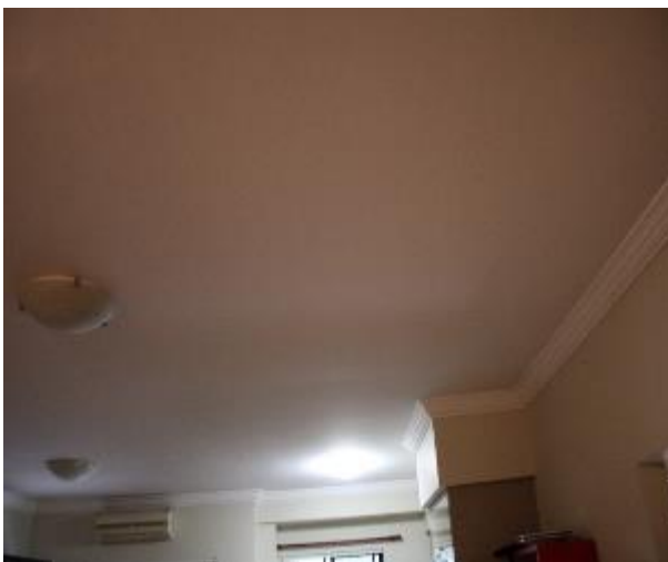
Figure 826 - General condition of open kitchen/ lounge room ceiling
