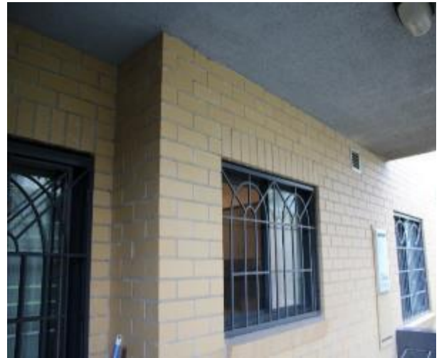
Figure 1227 - General condition of external wall
