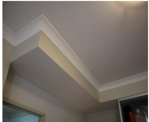
Figure 921 - General condition of bedroom 3 ceiling
