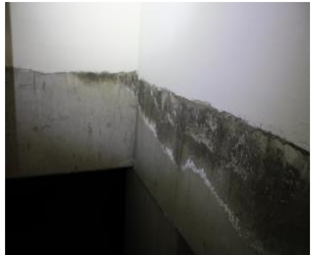
Figure 414 - General condition of level 5 to basement B2 fire stairs internal wall
