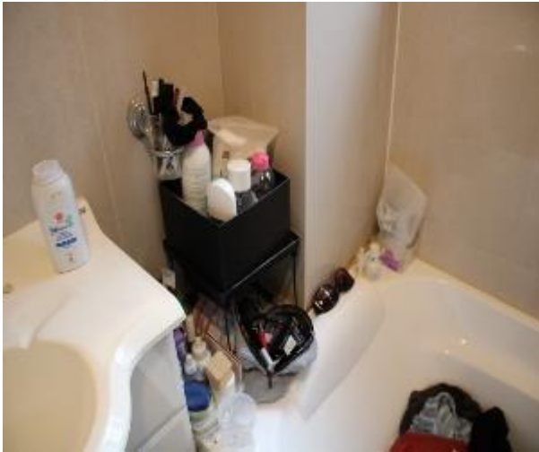
Figure 846 - General condition of bathroom 1 internal wall
