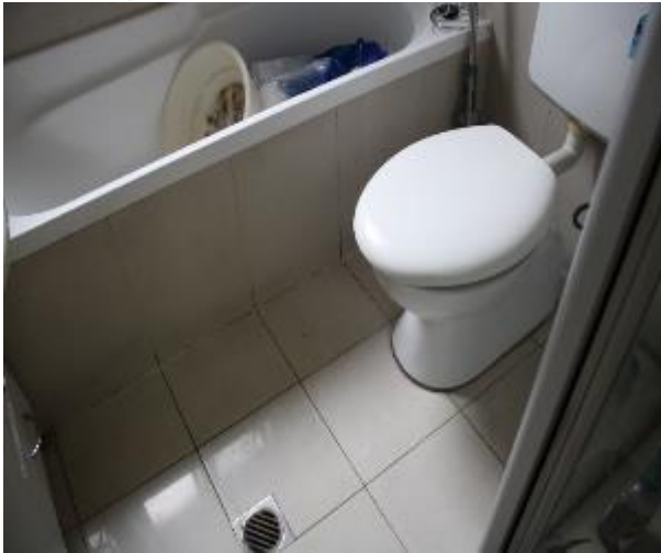
Figure 1344 - General condition of bathroom 1 floor tiles
