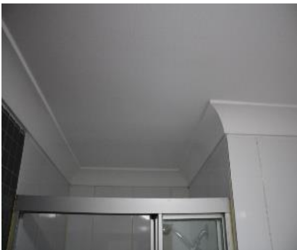
Figure 572 - General condition of ensuite bathroom ceiling
