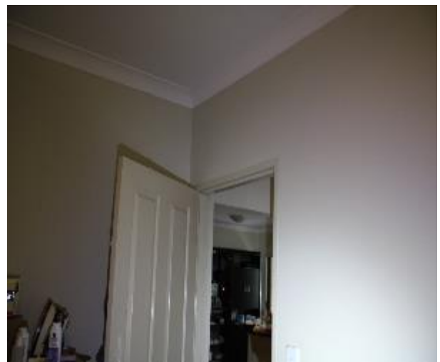
Figure 887 - General condition of bedroom 2 internal wall
