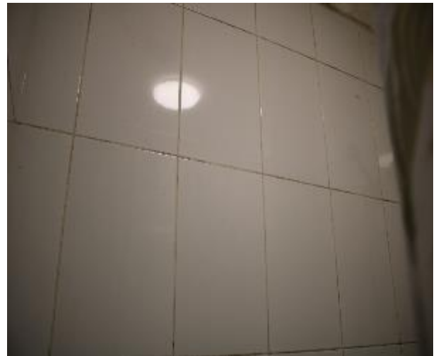
Figure 1377 - General condition of ensuite bathroom internal wall
