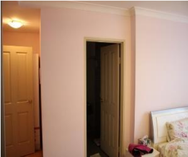
Figure 1134 - General condition of bedroom 1 internal wall
