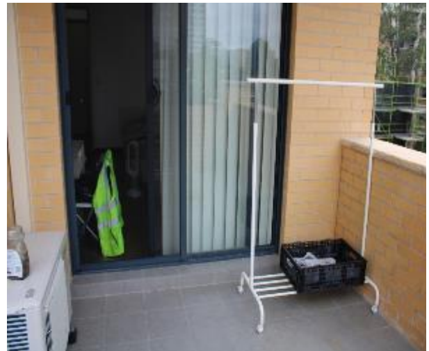
Figure 1401 - General condition of external wall
