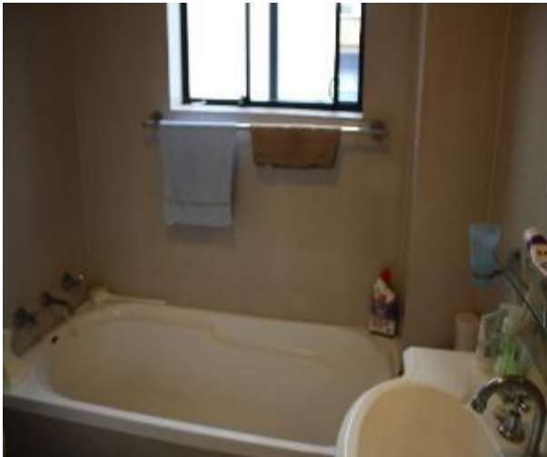
Figure 1184 - General condition of bathroom 1 internal wall
