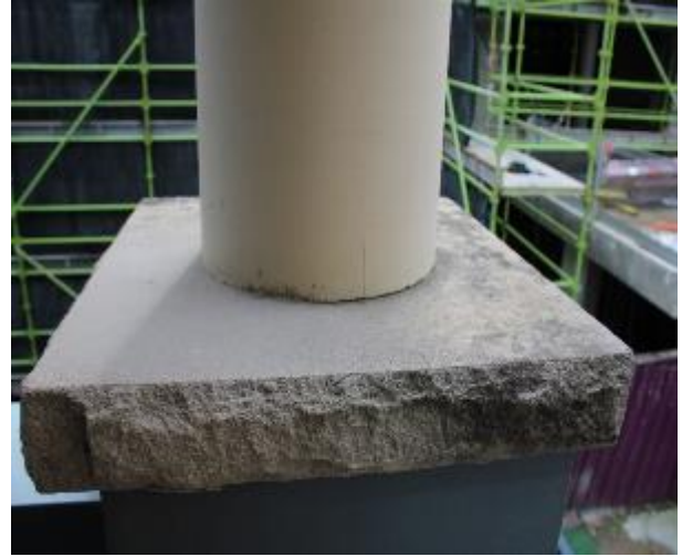
Figure 647 - General condition of external wall
