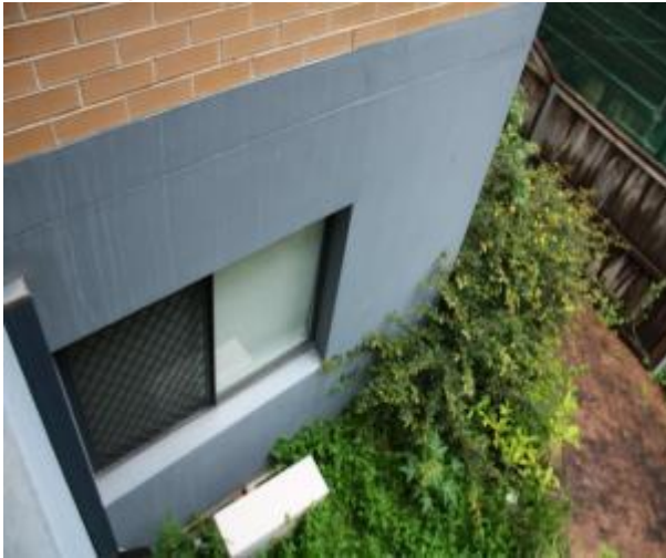
Figure 800 - General condition of external wall
