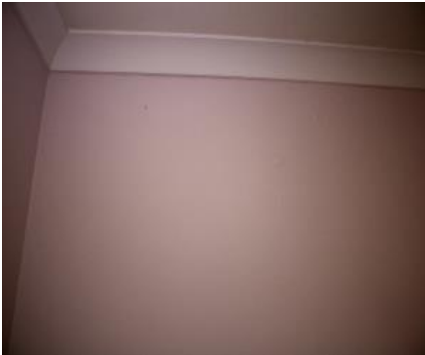
Figure 1130 - General condition of bedroom 1 internal wall
