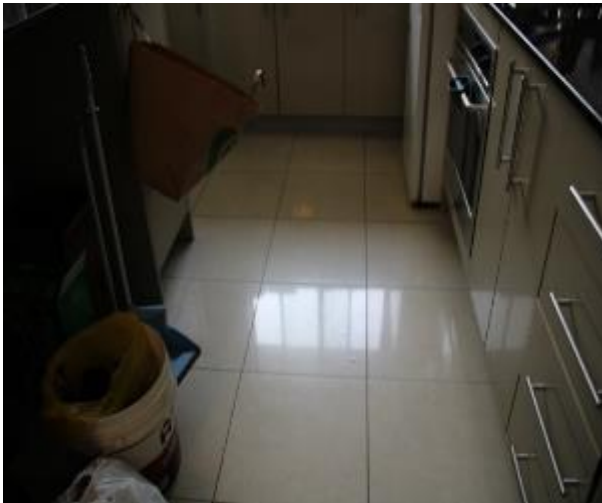
Figure 1250 - General condition of kitchen floor tiles
