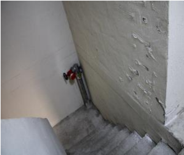
Figure 249 - General condition of level 5 to basement B2 fire stairs internal wall
