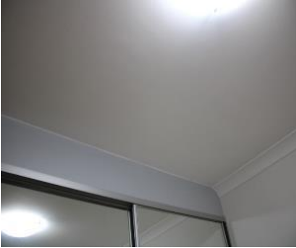
Figure 770 - General condition of bedroom 3 ceiling
