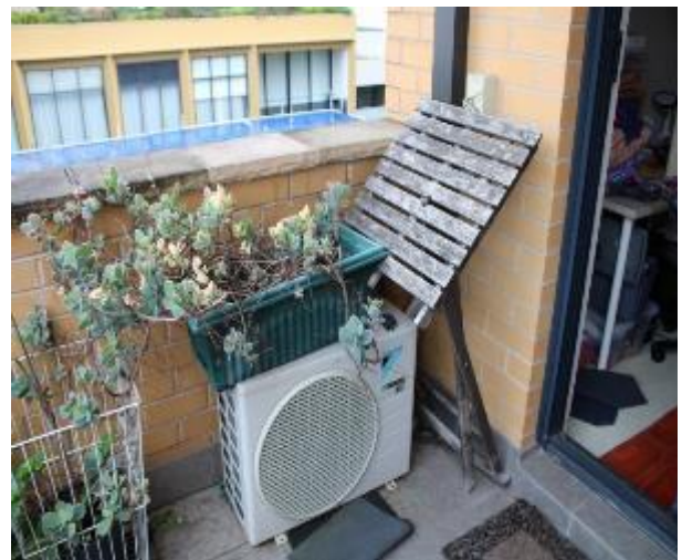
Figure 1523 - General condition of external wall
