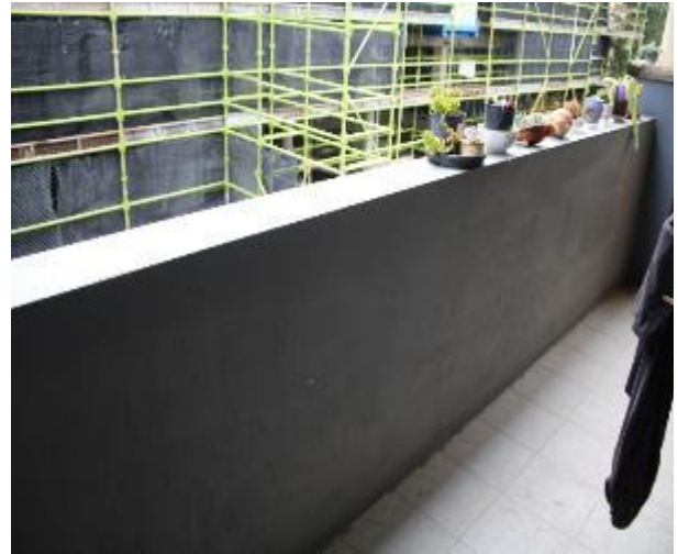
Figure 949 - General condition of external wall
