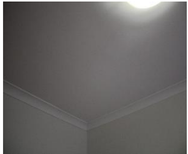
Figure 1056 - General condition of bedroom 2 ceiling
