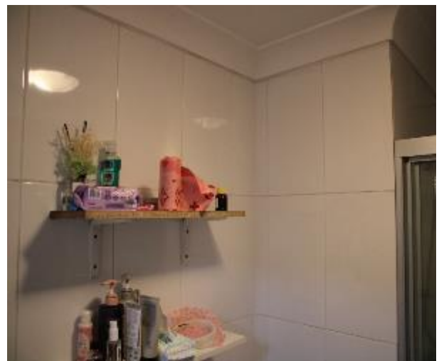
Figure 715 - General condition of ensuite bathroom internal wall
