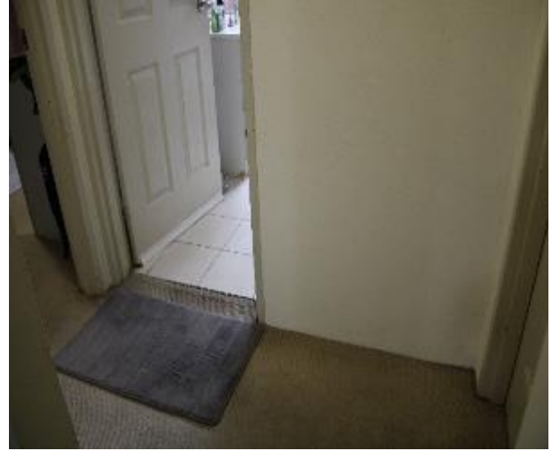
Figure 575 - General condition of corridor internal wall
