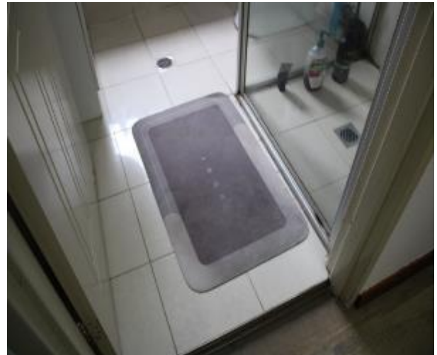
Figure 1343 - General condition of bathroom 1 floor tiles
