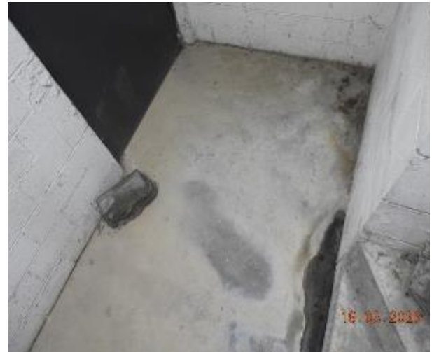
Figure 176 - General condition of B2 to Level 1 fire stairs pavement slab
