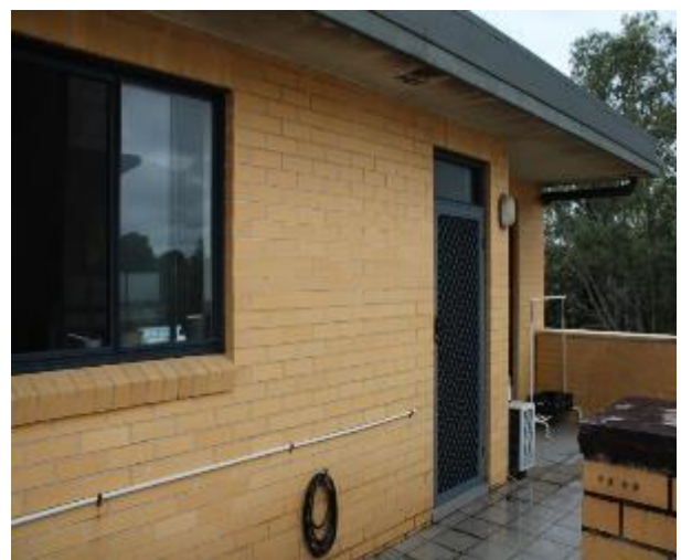
Figure 1397 - General condition of external wall
