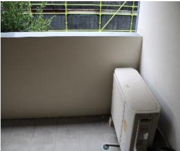
Figure 784 - General condition of external wall
