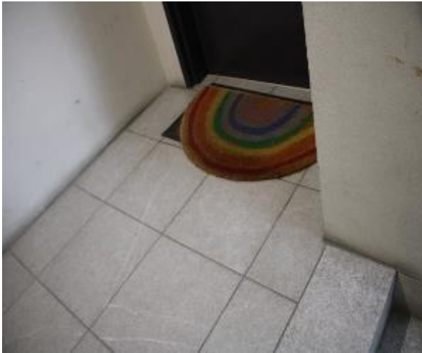
Figure 139 - General condition of level 5 common area floor tiles
