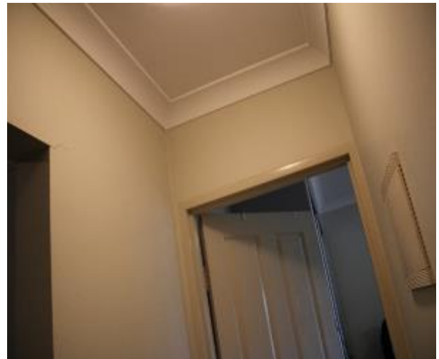
Figure 897 - General condition of corridor internal wall
