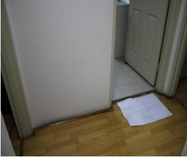
Figure 1158 - General condition of corridor internal wall
