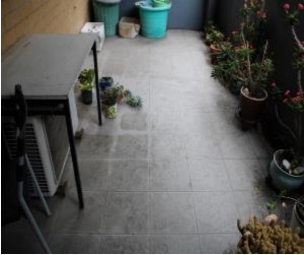
Figure 1059 - General condition of balcony floor tiles
