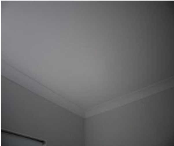
Figure 704 - General condition of bedroom 1 ceiling
