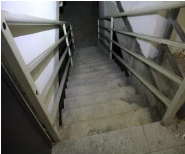
Figure 395 - General condition of level 5 to basement B2 fire stairs
