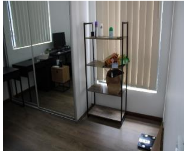
Figure 1327 - General condition of study internal wall
