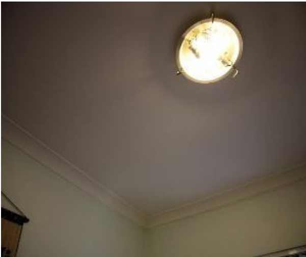
Figure 1208 - General condition of study ceiling
