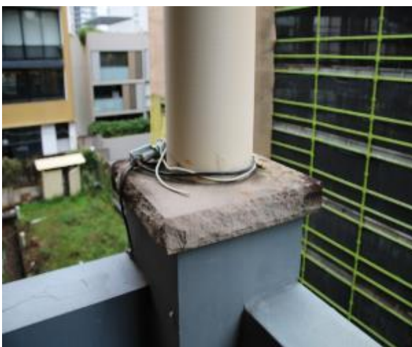
Figure 1075 - General condition of external wall
