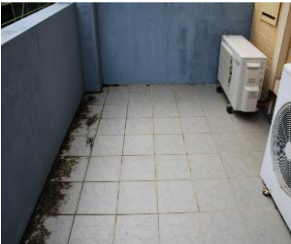
Figure 1294 - General condition of balcony floor tiles
