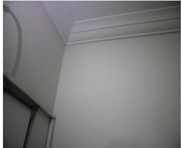
Figure 669 - General condition of kitchen internal wall
