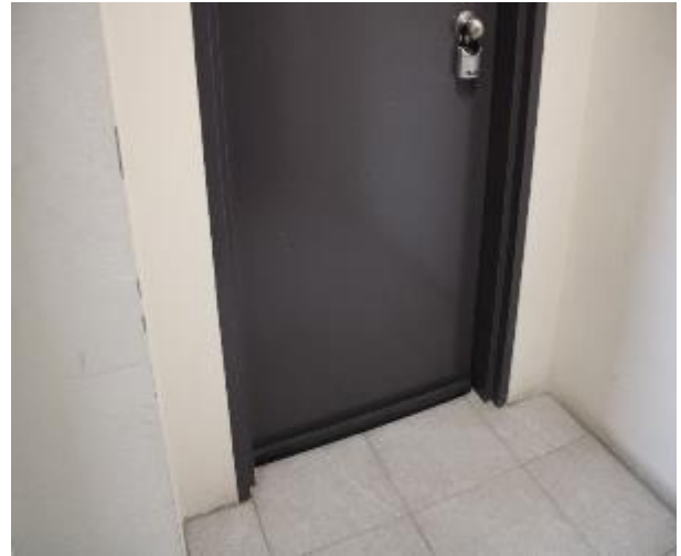
Figure 140 - General condition of level 5 common area internal wall
