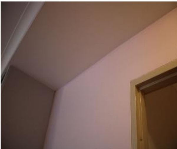
Figure 1126 - General condition of bedroom 1 internal wall
