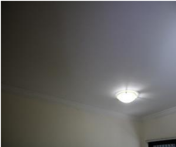
Figure 522 - General condition of open kitchen/ lounge room ceiling
