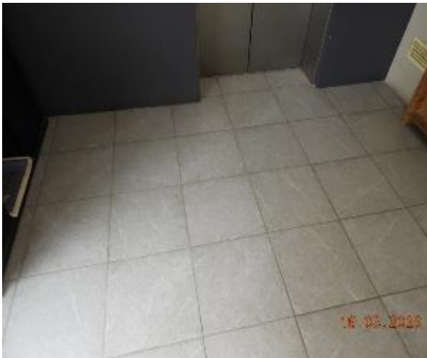
Figure 57 - General condition of level 3 common area floor tiles
