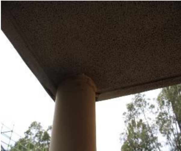
Figure 954 - General condition of balcony underside slab
