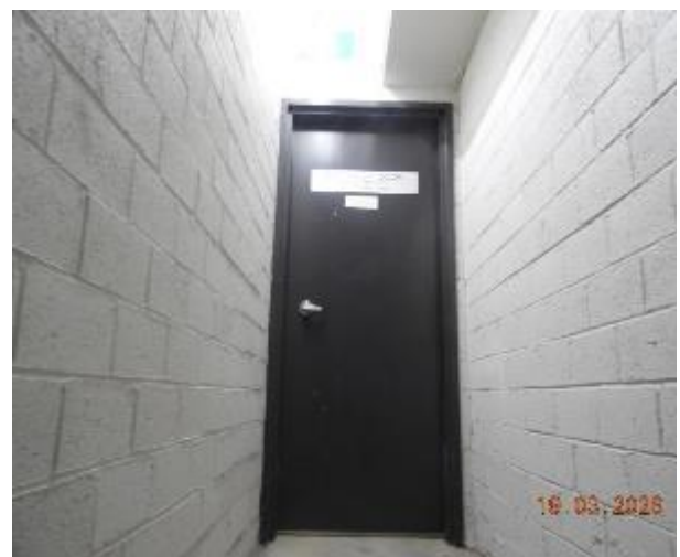
Figure 196 - General condition of B2 to Level 1 fire stairs internal wall
