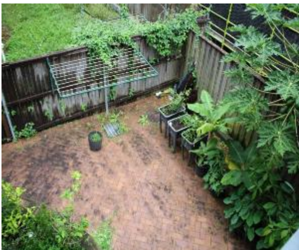
Figure 798 - General condition of boundary fence as seen from Unit 23 balcony
