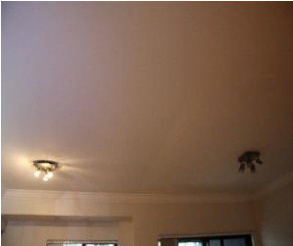
Figure 1110 - General condition of lounge room ceiling
