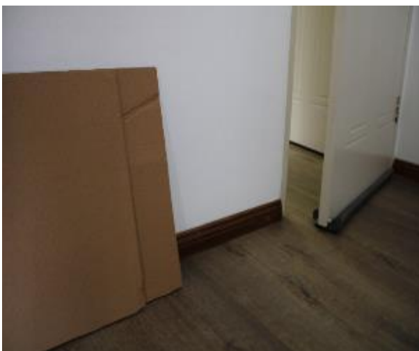
Figure 1336 - General condition of study internal wall
