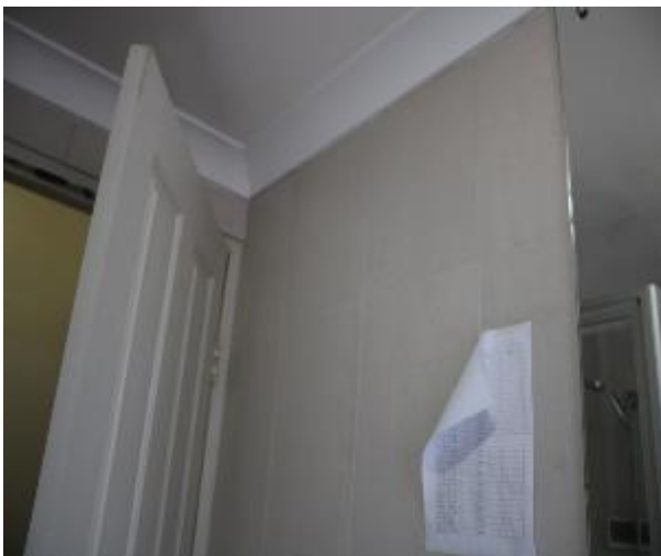
Figure 612 - General condition of bathroom 1 internal wall
