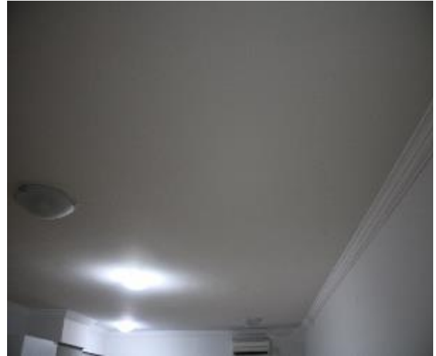
Figure 677 - General condition of kitchen ceiling
