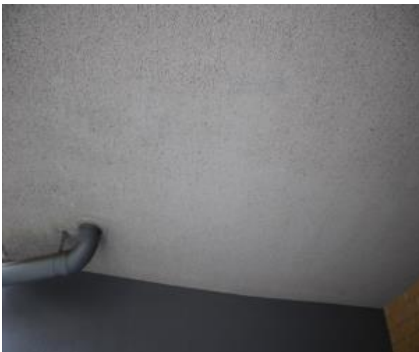
Figure 1079 - General condition of balcony underside slab
