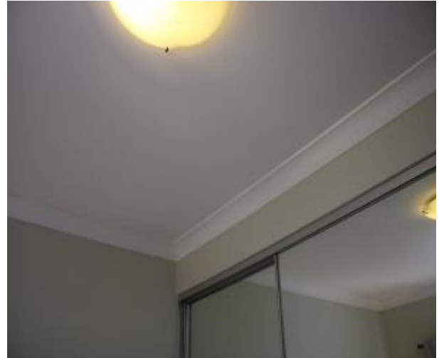
Figure 861 - General condition of bedroom 1 ceiling
