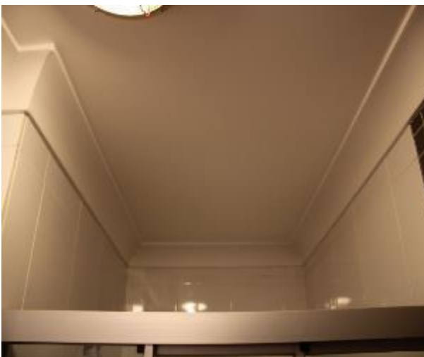
Figure 1156 - General condition of ensuite bathroom ceiling
