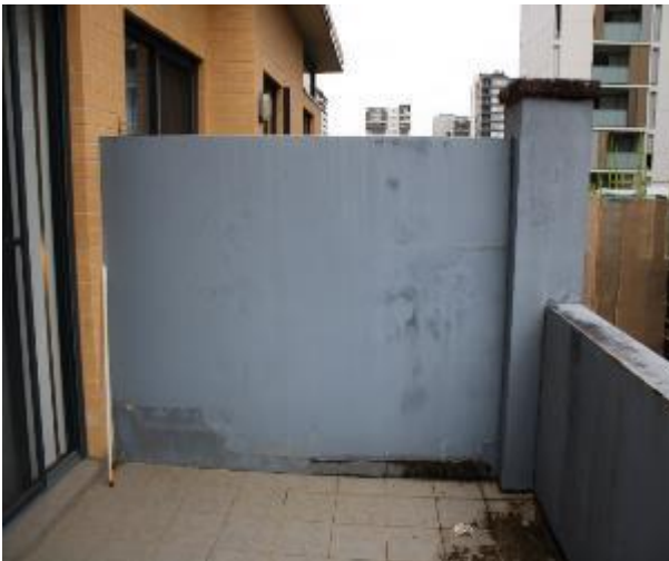
Figure 1310 - General condition of external wall
