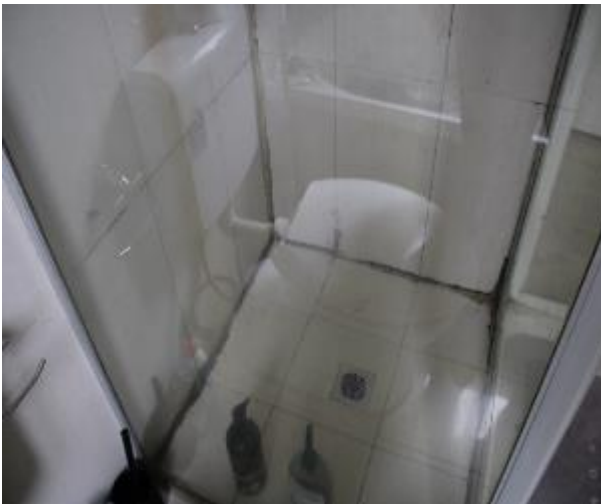
Figure 1352 - General condition of bathroom 1 internal wall
