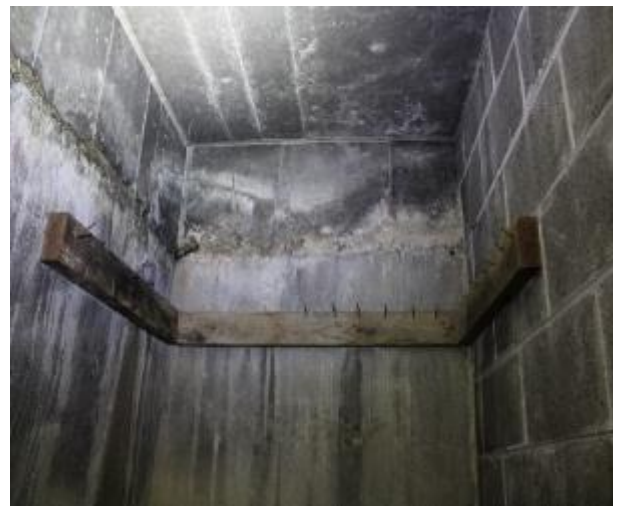
Figure 474 - General condition of basement B2 fire stairs internal wall
