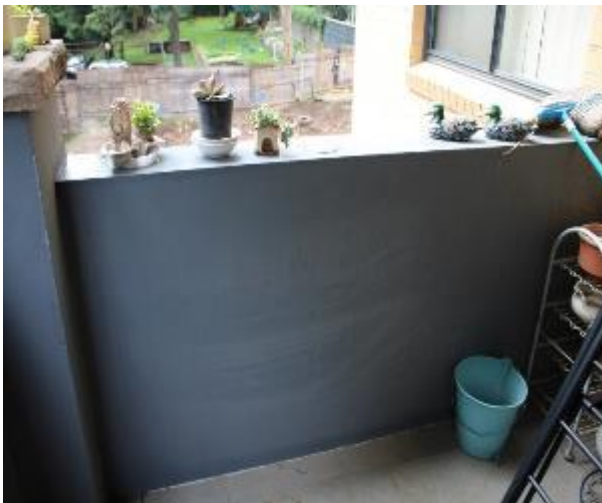
Figure 952 - General condition of external wall
