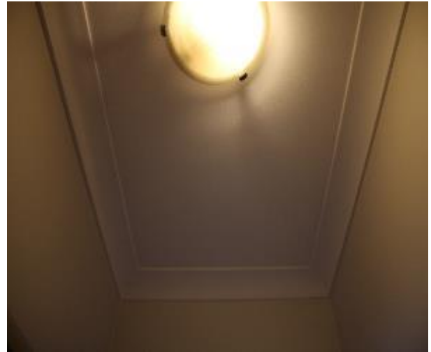
Figure 1165 - General condition of corridor ceiling
