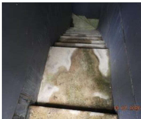
Figure 158 - General condition of B2 to Level 1 fire stairs
