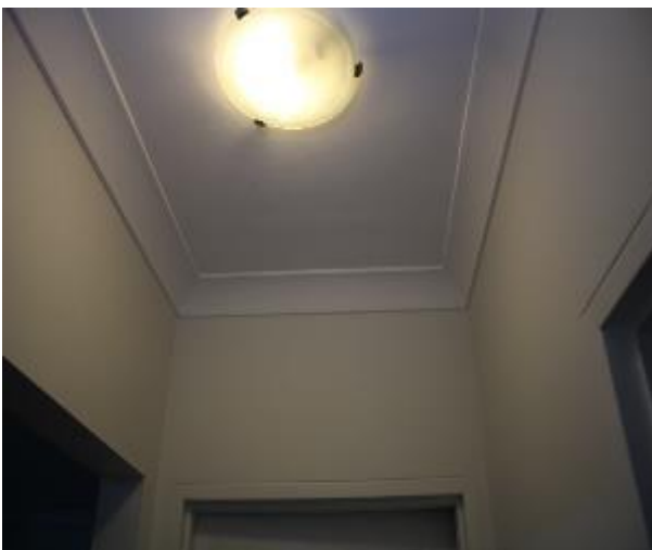
Figure 726 - General condition of corridor ceiling
