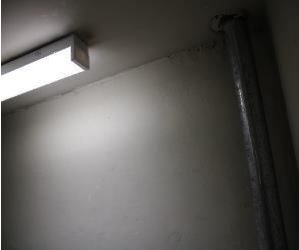
Figure 363 - General condition of level 5 to basement B2 fire stairs internal wall
