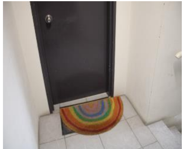
Figure 148 - General condition of level 5 common area internal wall
