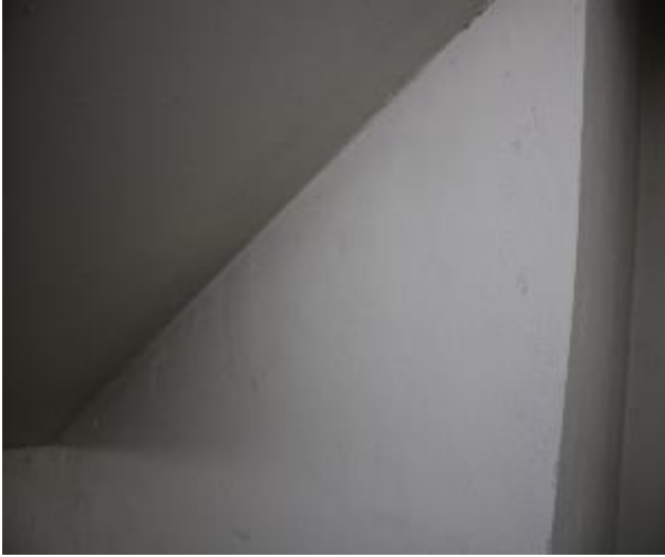
Figure 345 - General condition of level 5 to basement B2 fire stairs internal wall
