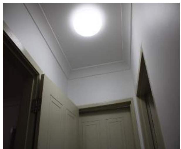
Figure 1325 - General condition of corridor ceiling
