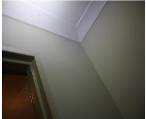
Figure 907 - General condition of laundry internal wall
