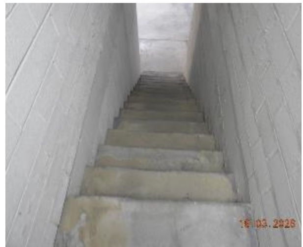
Figure 194 - General condition of B2 to Level 1 fire stairs
