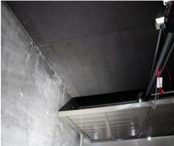
Figure 453 - General condition of basement B2 fire stairs underside slab
