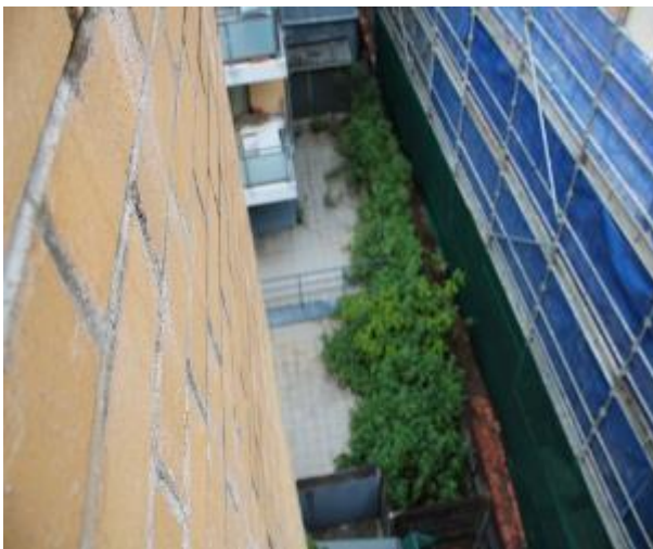
Figure 1528 - General condition of boundary as seen from Unit 29 balcony 2
