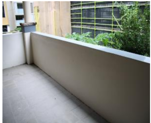
Figure 787 - General condition of external wall
