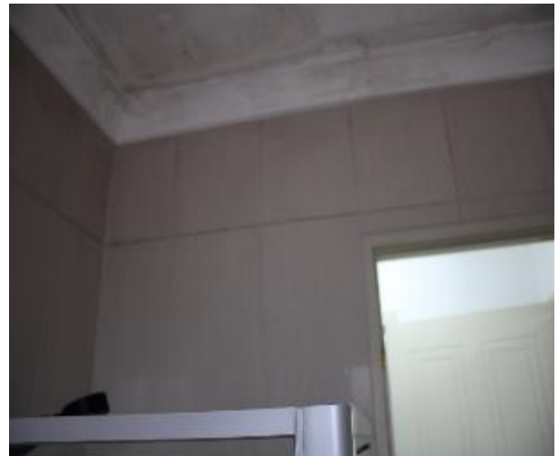
Figure 1353 - General condition of bathroom 1 internal wall
