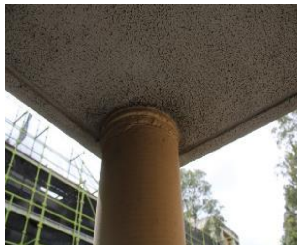
Figure 661 - General condition of balcony underside slab
