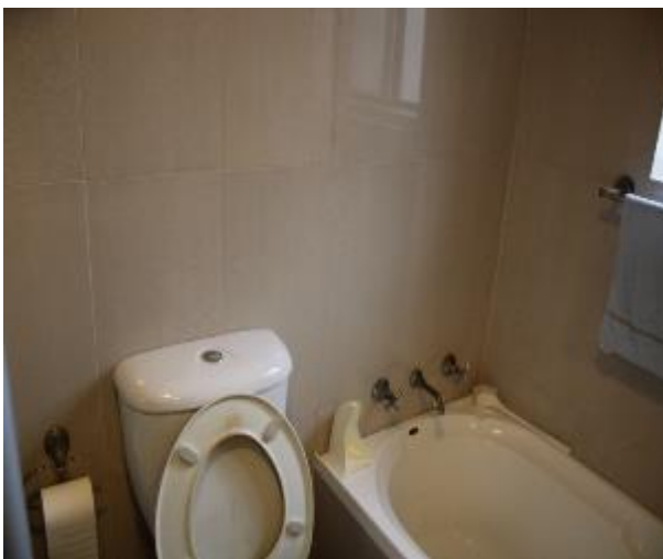
Figure 1186 - General condition of bathroom 1 internal wall
