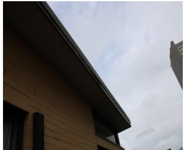
Figure 1595 - General condition of eave
