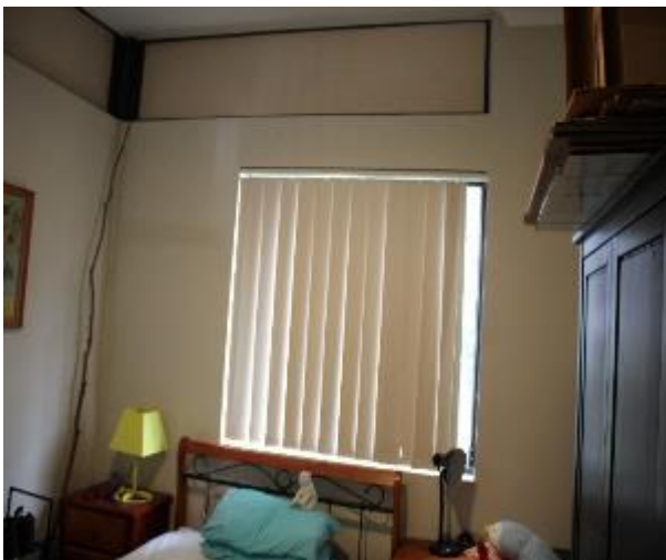
Figure 1546 - General condition of bedroom 2 internal wall
