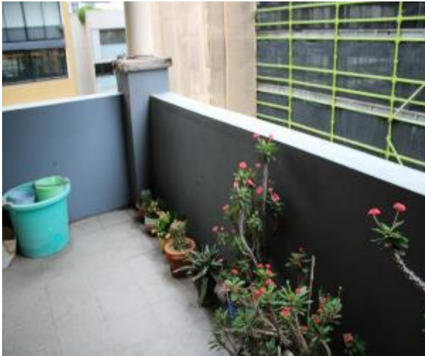
Figure 1071 - General condition of external wall
