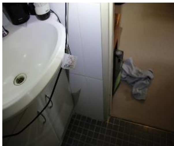
Figure 933 - General condition of ensuite bathroom internal wall
