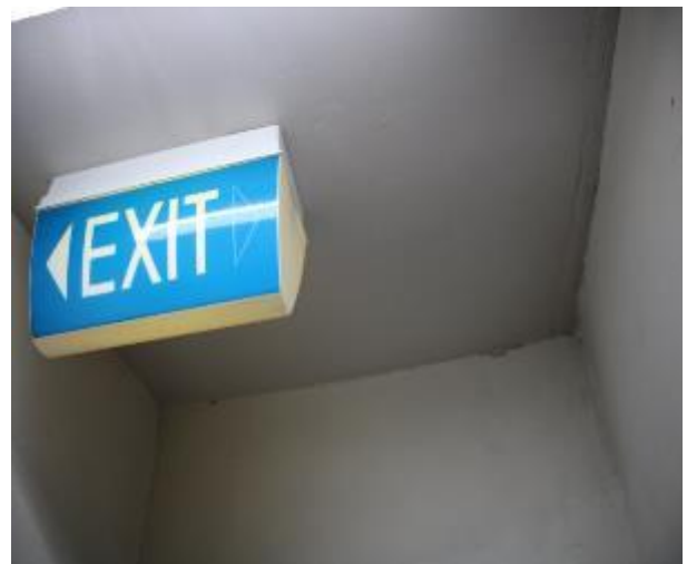
Figure 390 - General condition of level 5 to basement B2 fire stairs underside stairs
