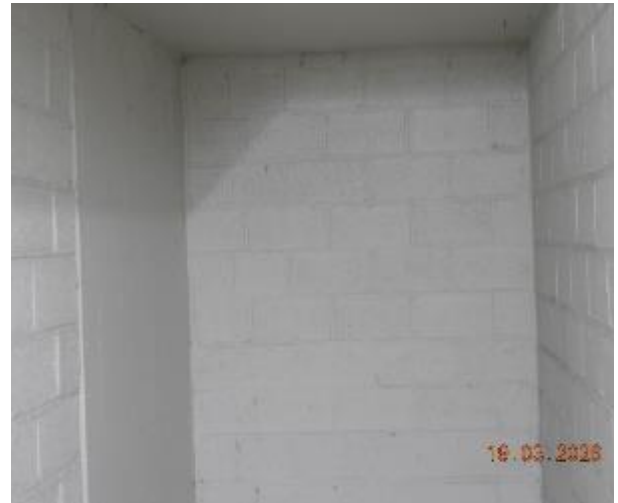
Figure 206 - General condition of B2 to Level 1 fire stairs internal wall
