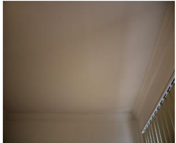
Figure 1287 - General condition of bedroom 1 ceiling
