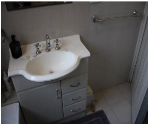
Figure 1540 - General condition of bathroom 1 internal wall
