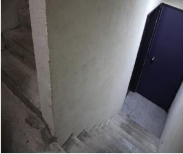
Figure 375 - General condition of level 5 to basement B2 fire stairs internal wall
