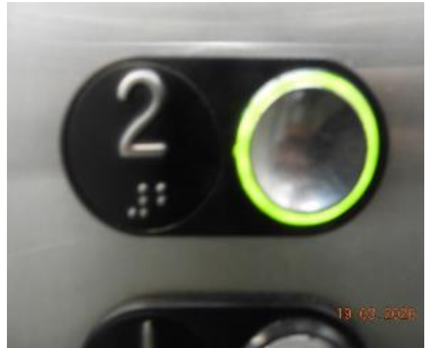
Figure 28 -The following images display the condition of level 2 Common Area
