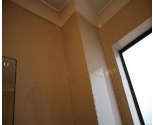
Figure 847 - General condition of bathroom 1 internal wall
