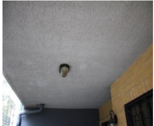
Figure 1078 - General condition of balcony underside slab
