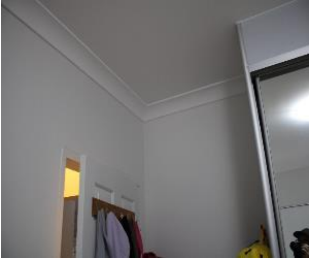
Figure 764 - General condition of bedroom 3 internal wall
