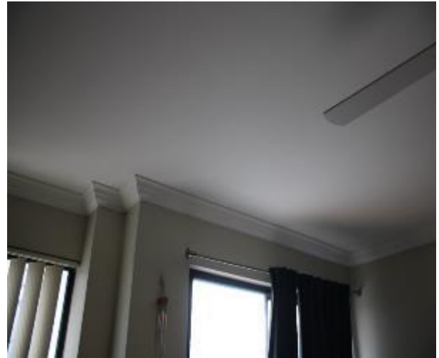
Figure 1461 - General condition of lounge room ceiling
