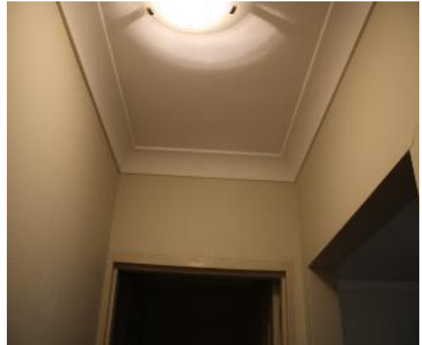
Figure 901 - General condition of corridor internal wall
