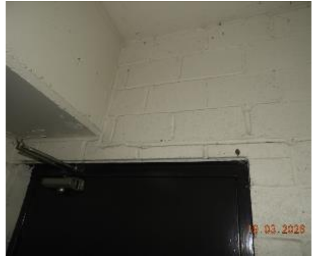
Figure 180 - General condition of B2 to Level 1 fire stairs internal wall
