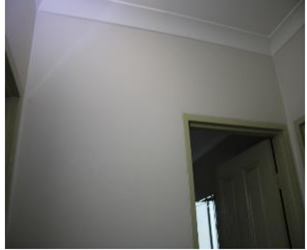
Figure 1159 - General condition of corridor internal wall
