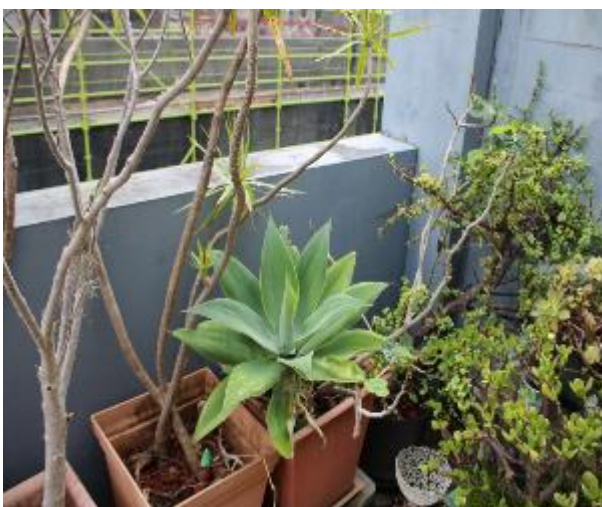
Figure 1584 - General condition of external wall
