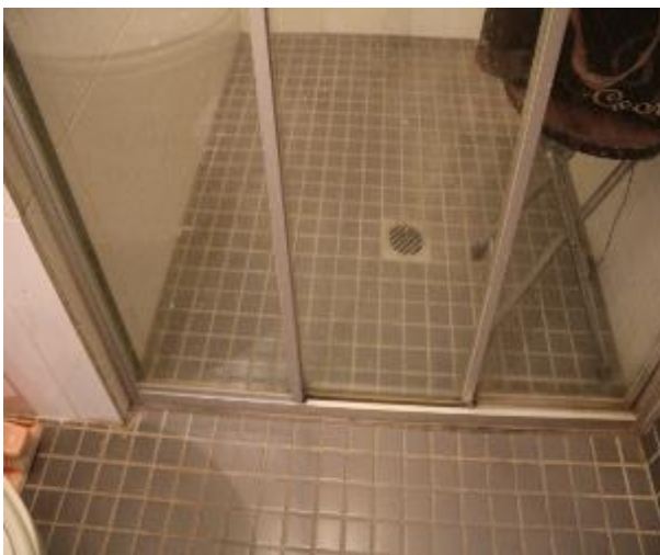
Figure 1144 - General condition of ensuite bathroom floor tiles
