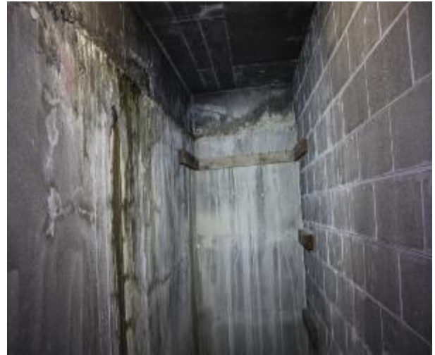
Figure 466 - General condition of basement B2 fire stairs internal wall
