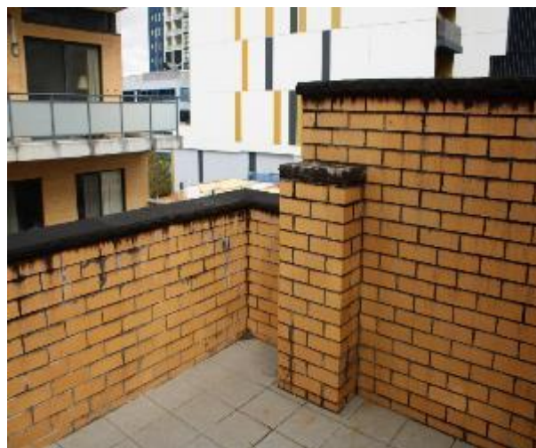
Figure 1409 - General condition of external wall
