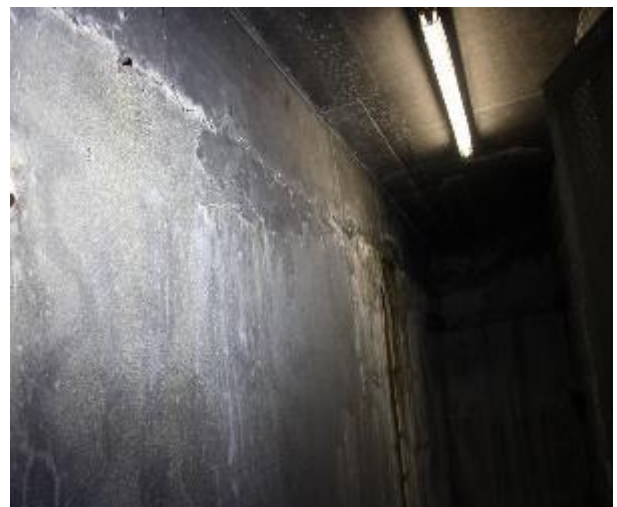
Figure 464 - General condition of basement B2 fire stairs internal wall
