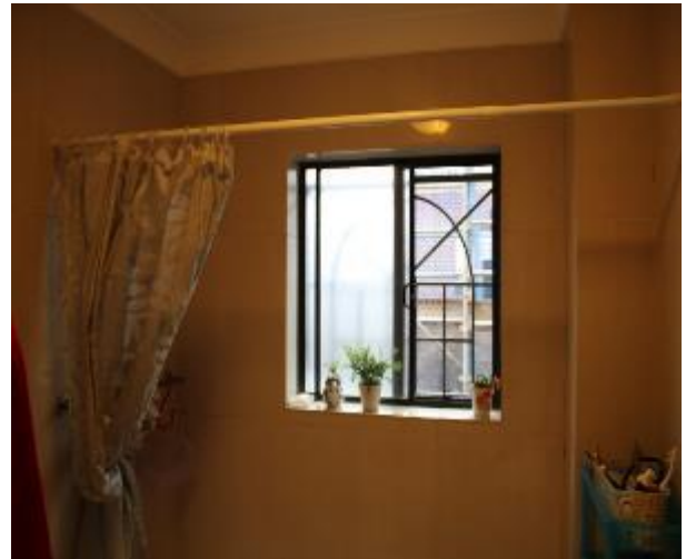
Figure 1032 - General condition of bathroom 1 internal wall
