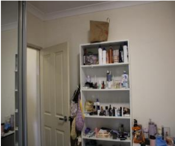
Figure 592 - General condition of bedroom 2 internal wall
