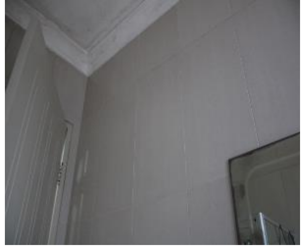
Figure 1351 - General condition of bathroom 1 internal wall
