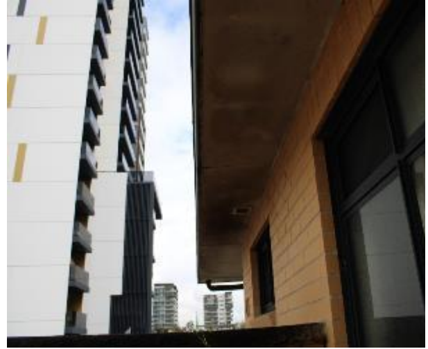
Figure 1411 - General condition of balcony underside slab
