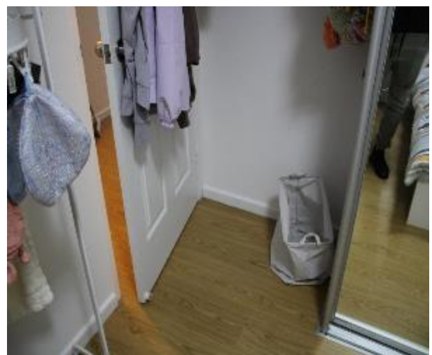
Figure 763 - General condition of bedroom 3 internal wall
