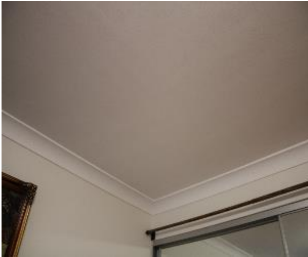
Figure 999 - General condition of study ceiling
