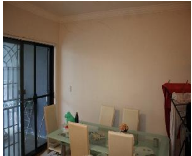
Figure 1099 - General condition of lounge room internal wall
