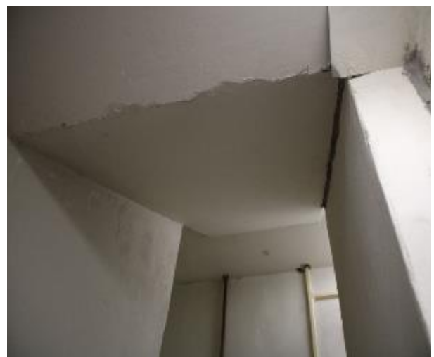
Figure 386 - General condition of level 5 to basement B2 fire stairs underside stairs
