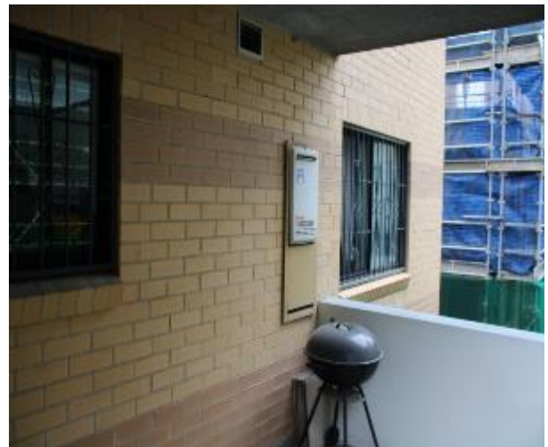
Figure 775 - General condition of external wall
