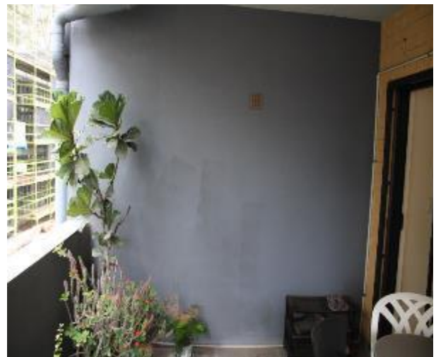
Figure 1068 - General condition of external wall
