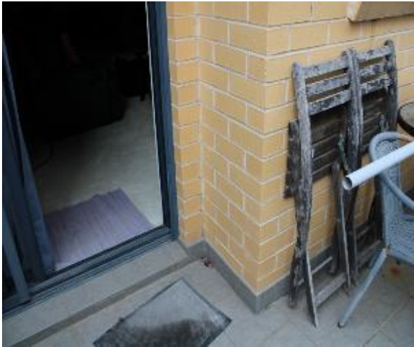
Figure 1574 - General condition of external wall
