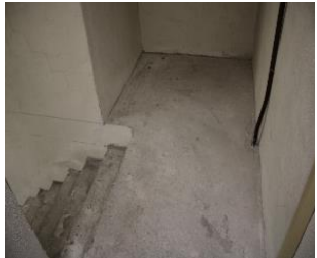
Figure 276 - General condition of level 5 to basement B2 fire stairs
