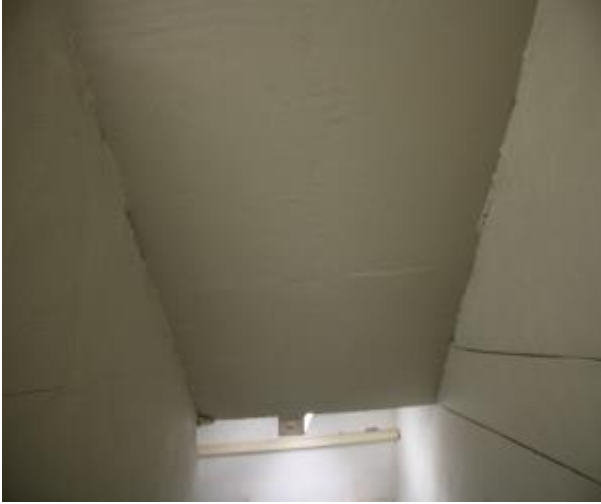
Figure 327 - General condition of level 5 to basement B2 fire stairs underside stairs
