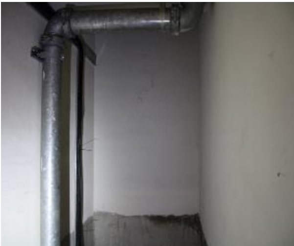
Figure 413 - General condition of level 5 to basement B2 fire stairs internal wall
