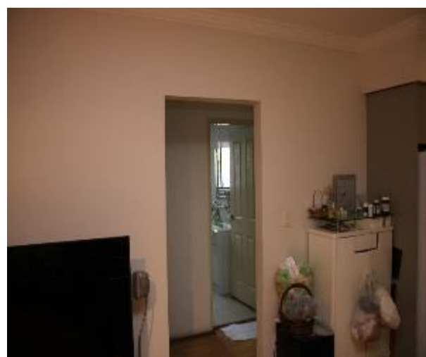
Figure 1097 - General condition of lounge room internal wall
