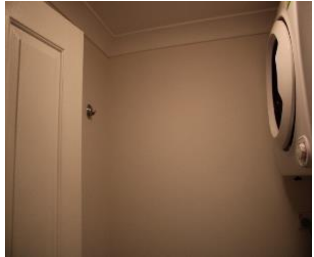
Figure 693 - General condition of laundry internal wall
