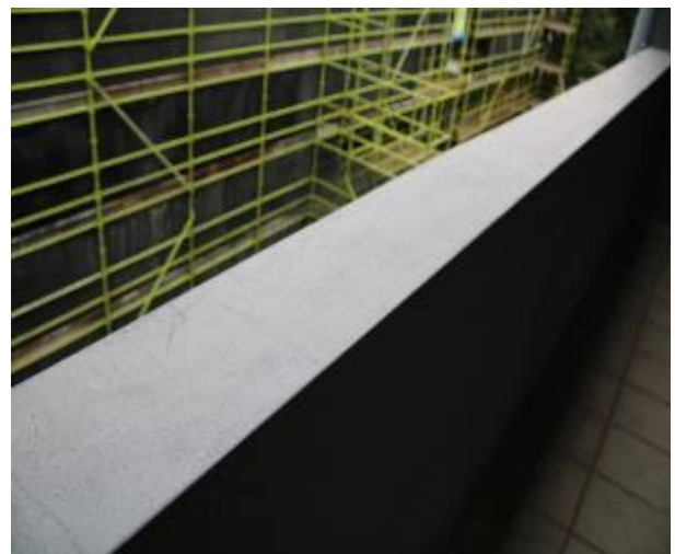
Figure 1241 - General condition of external wall
