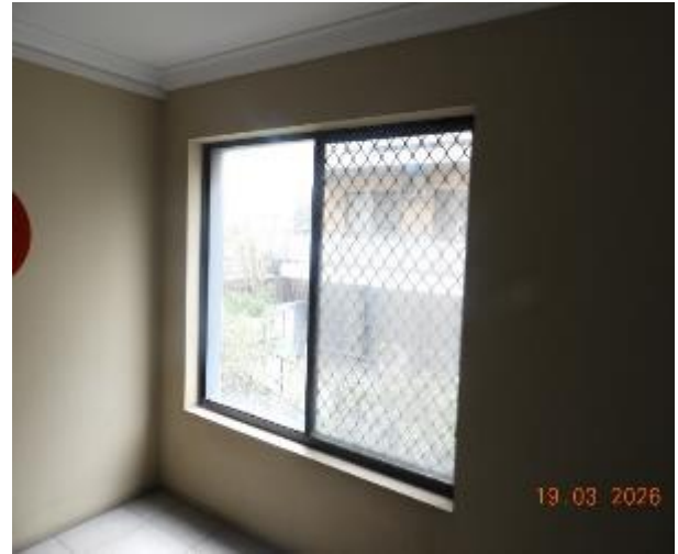
Figure 38 - General condition of level 2 common area internal wall
