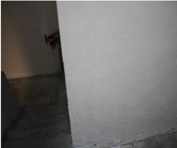
Figure 231 - General condition of level 5 to basement B2 fire stairs internal wall
