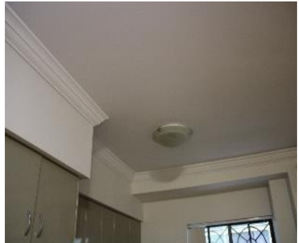
Figure 984 - General condition of kitchen ceiling
