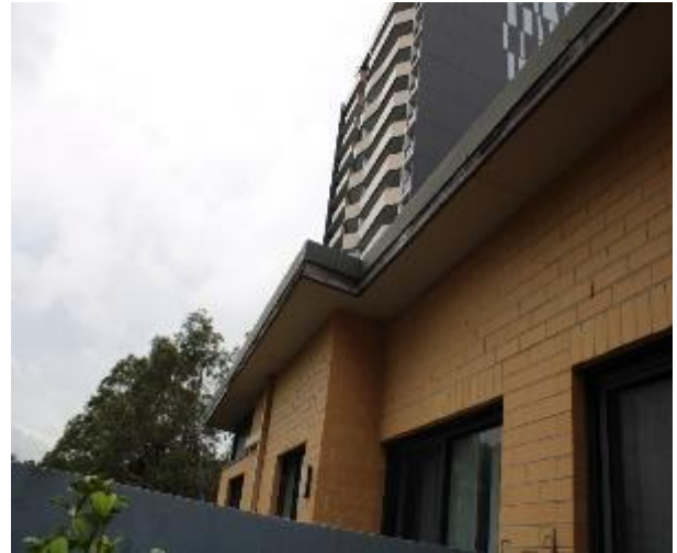
Figure 1593 - General condition of eave
