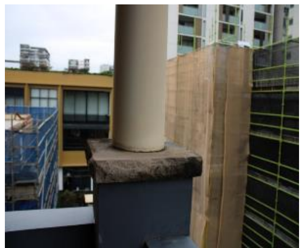
Figure 1247 - General condition of external wall
