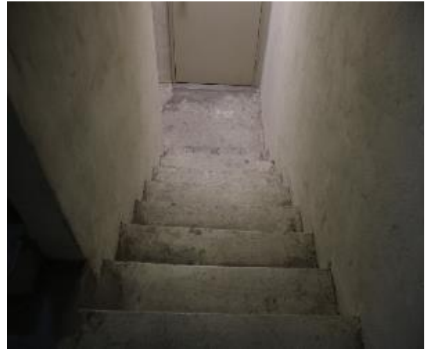
Figure 274 - General condition of level 5 to basement B2 fire stairs
