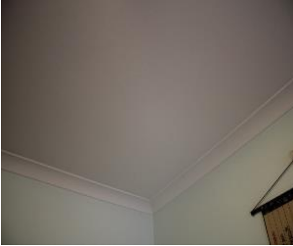
Figure 1206 - General condition of study ceiling
