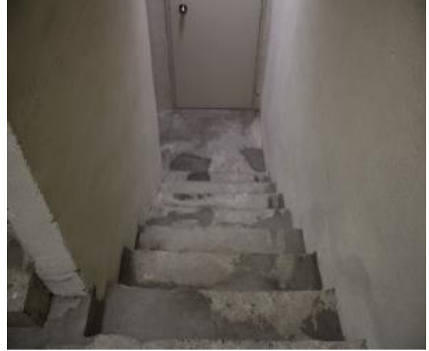
Figure 328 - General condition of level 5 to basement B2 fire stairs
