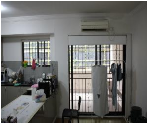
Figure 670 - General condition of kitchen internal wall
