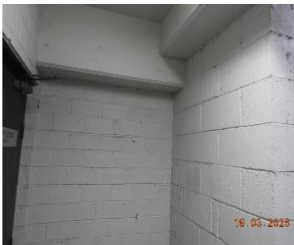
Figure 187 - General condition of B2 to Level 1 fire stairs internal wall
