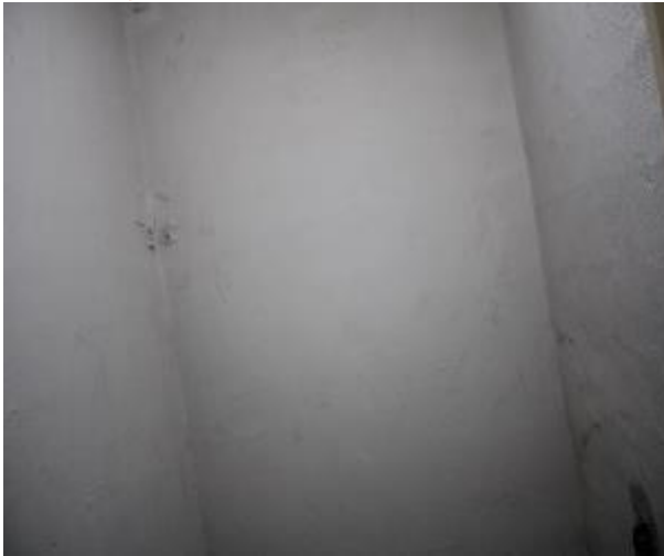
Figure 225 - General condition of level 5 to basement B2 fire stairs internal wall
