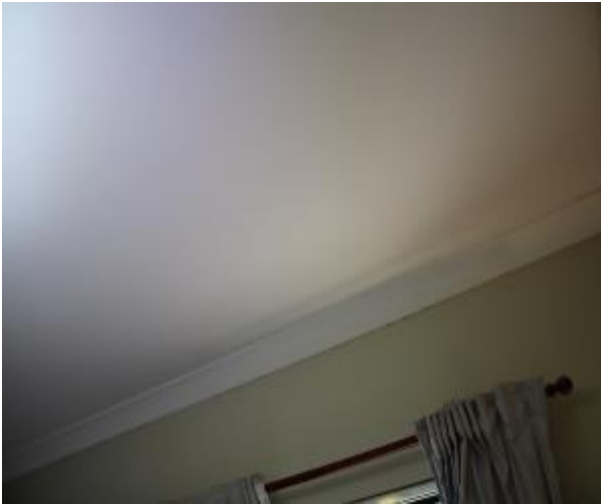
Figure 864 - General condition of bedroom 1 ceiling
