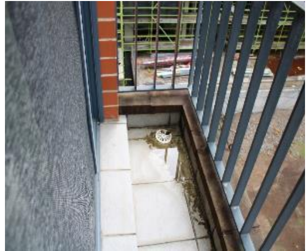
Figure 1387 - General condition of balcony 2 floor tiles
