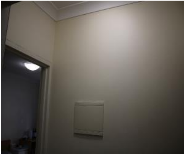
Figure 526 - General condition of corridor internal wall
