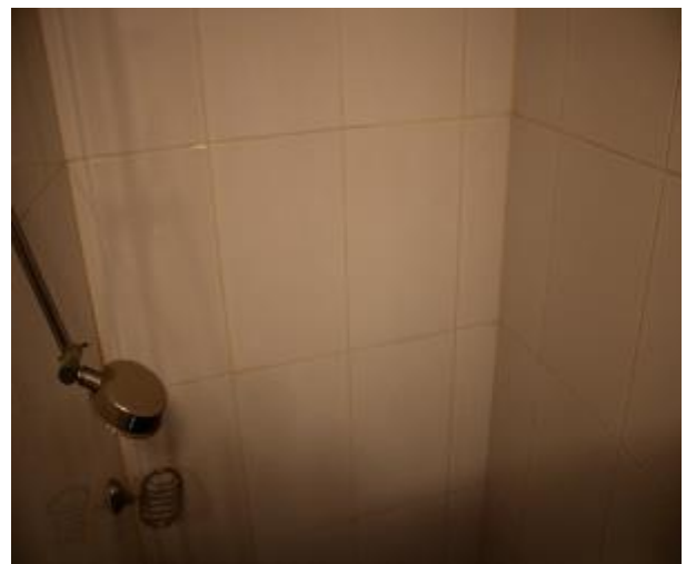
Figure 1151 - General condition of ensuite bathroom internal wall
