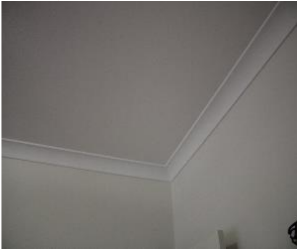
Figure 1053 - General condition of bedroom 2 ceiling
