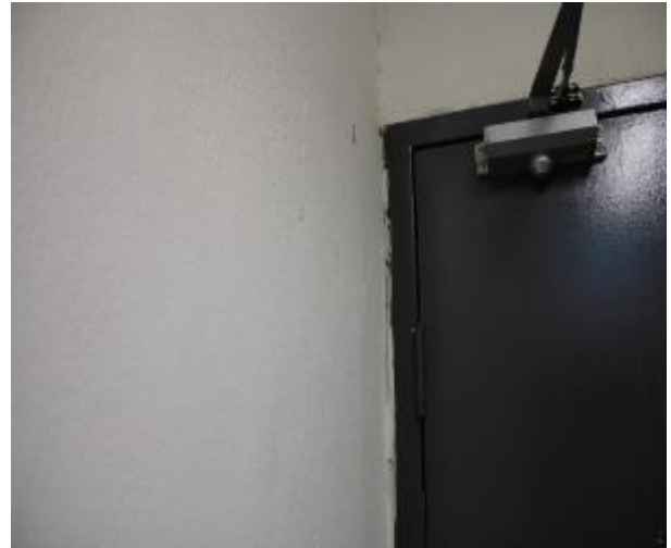
Figure 406 - General condition of level 5 to basement B2 fire stairs internal wall
