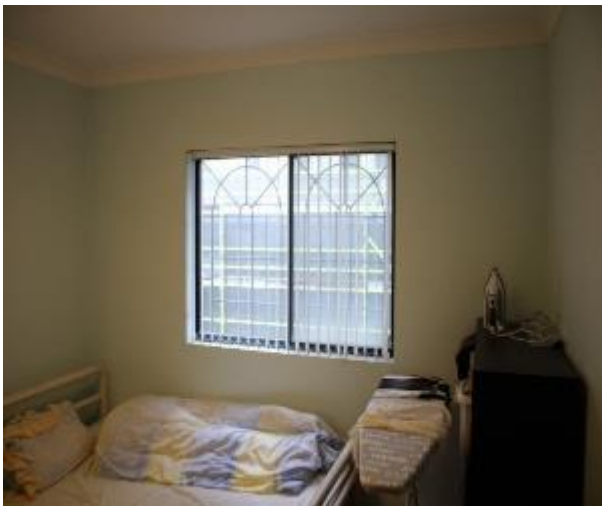
Figure 1166 - General condition of bedroom 2 internal wall
