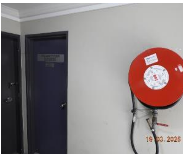
Figure 17 - General condition of level 1 common area internal wall
