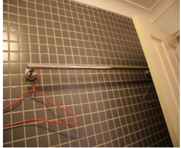
Figure 1153 - General condition of ensuite bathroom internal wall
