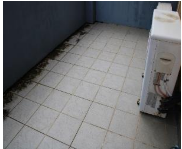
Figure 1293 - General condition of balcony floor tiles
