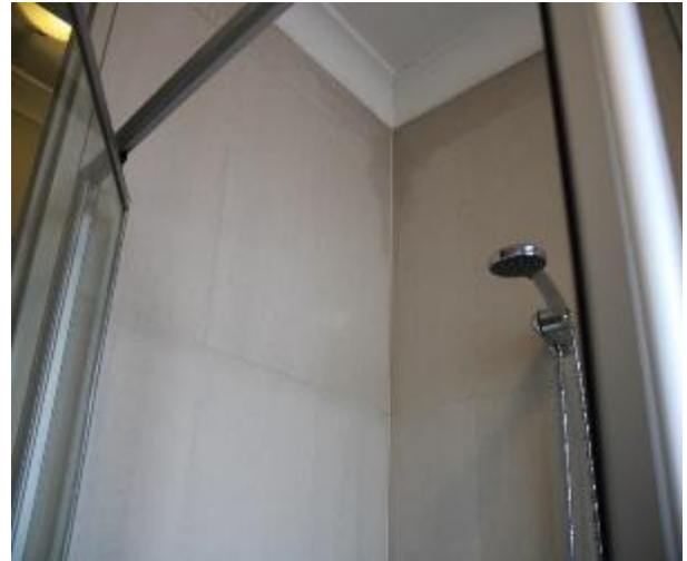
Figure 1539 - General condition of bathroom 1 internal wall
