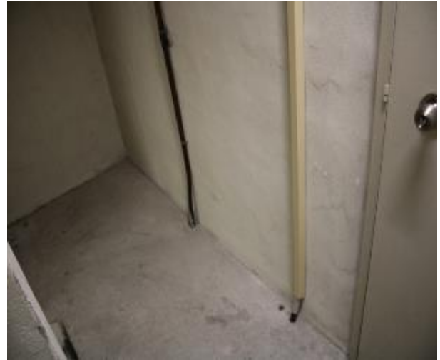
Figure 280 - General condition of level 5 to basement B2 fire stairs internal wall
