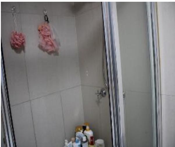
Figure 748 - General condition of bathroom 1 internal wall
