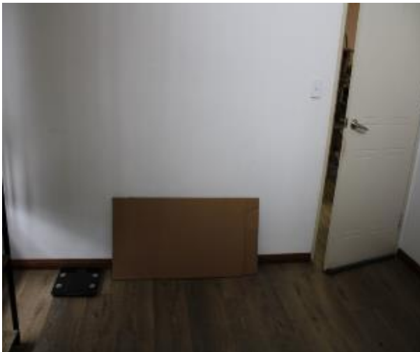
Figure 1334 - General condition of study internal wall
