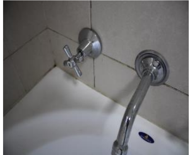
Figure 743 - Crack propagation through bathroom 1 internal wall
