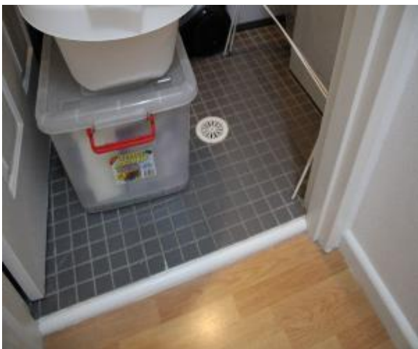
Figure 991 - General condition of laundry floor tiles
