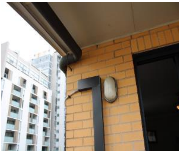
Figure 1522 - General condition of external wall
