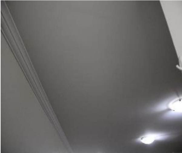
Figure 516 - General condition of open kitchen/ lounge room ceiling
