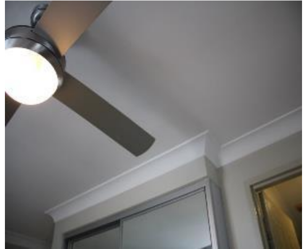
Figure 1493 - General condition of bedroom 1 ceiling
