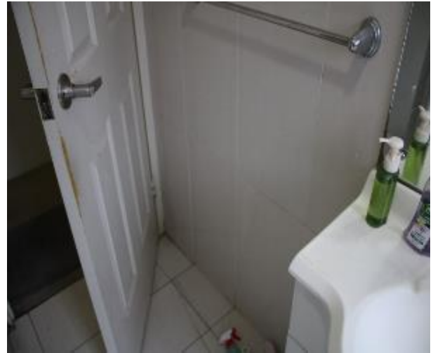
Figure 611 - General condition of bathroom 1 internal wall
