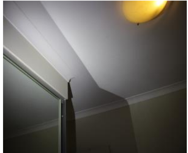
Figure 865 - General condition of bedroom 1 ceiling
