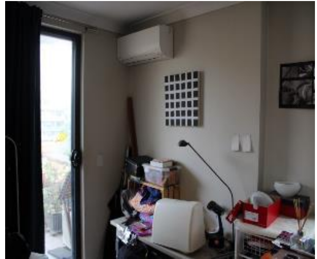
Figure 1473 - General condition of bedroom 1 internal wall
