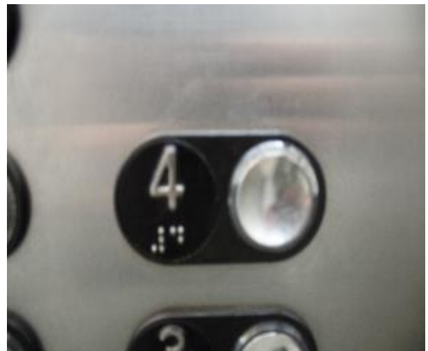
Figure 82 -The following images display the condition of Level 4 & 5 Common Area
