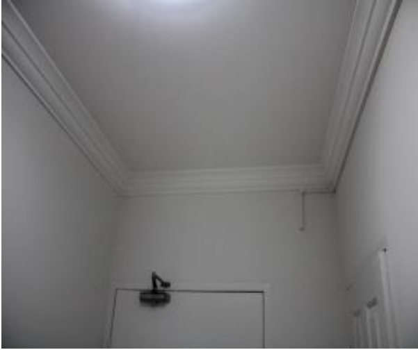
Figure 674 - General condition of kitchen ceiling
