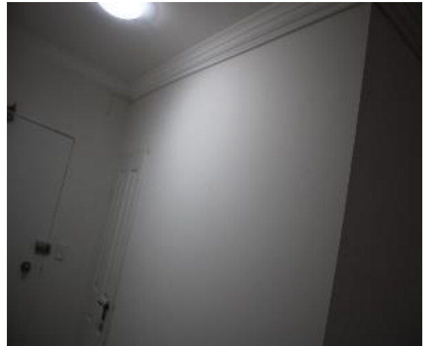
Figure 665 - General condition of kitchen internal wall
