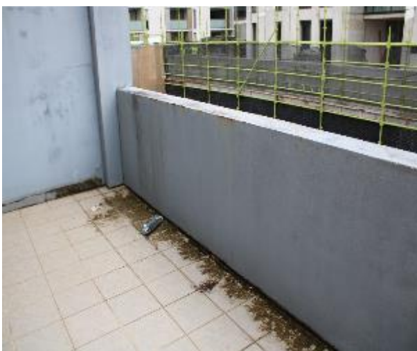
Figure 1306 - General condition of external wall
