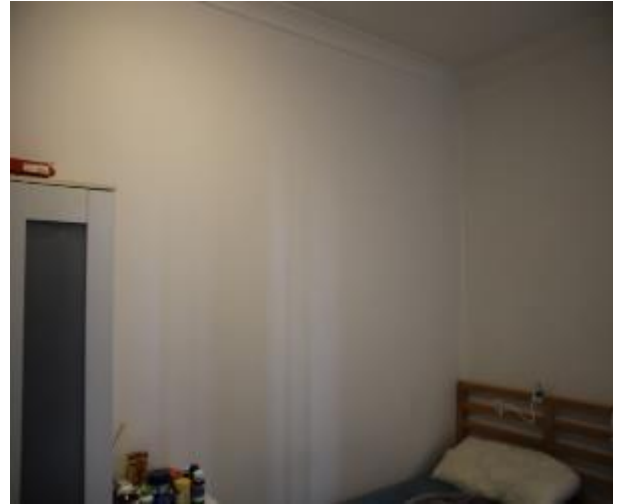
Figure 1281 - General condition of bedroom 1 internal wall
