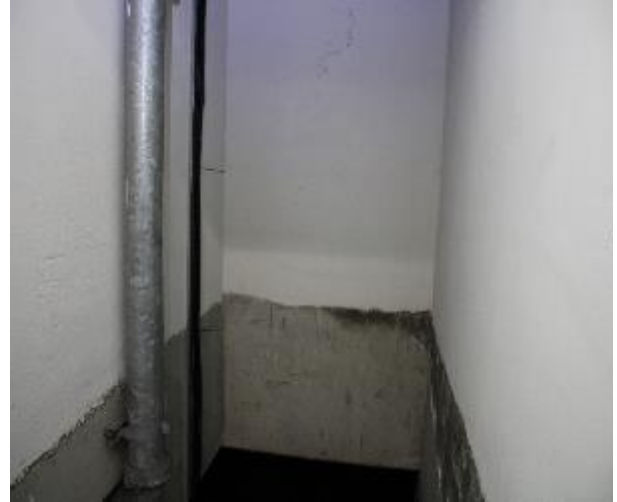
Figure 412 - General condition of level 5 to basement B2 fire stairs internal wall
