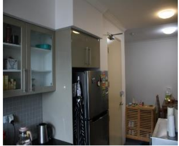
Figure 1255 - General condition of kitchen internal wall
