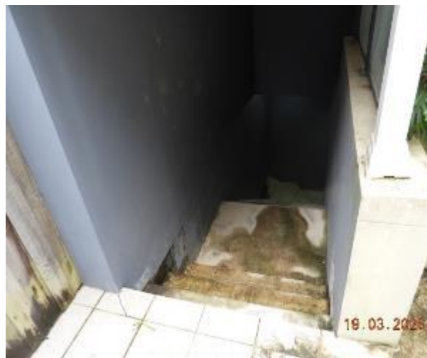
Figure 156 - General condition of B2 to Level 1 fire stairs
