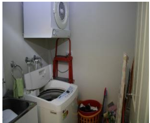
Figure 905 - General condition of laundry internal wall
