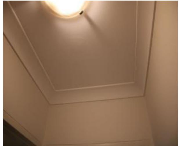
Figure 1018 - General condition of corridor ceiling
