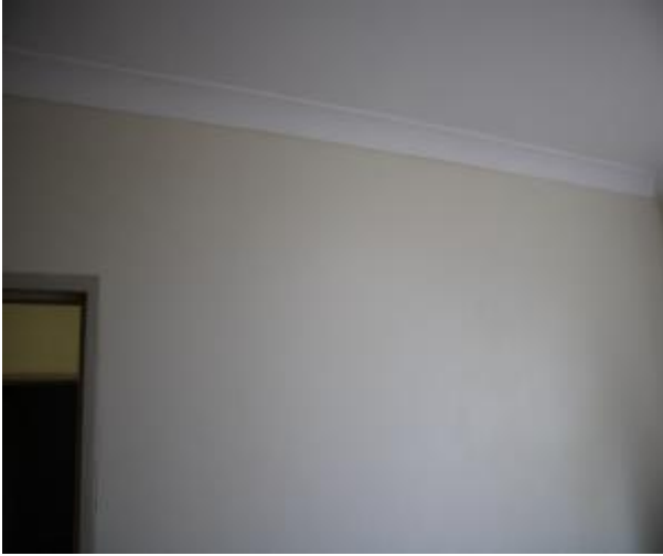
Figure 628 - General condition of bedroom 3 internal wall
