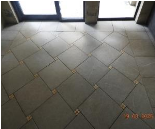
Figure 3 - General condition of level 1 common area floor tiles
