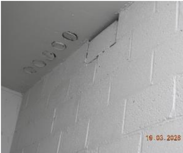
Figure 205 - General condition of B2 to Level 1 fire stairs internal wall
