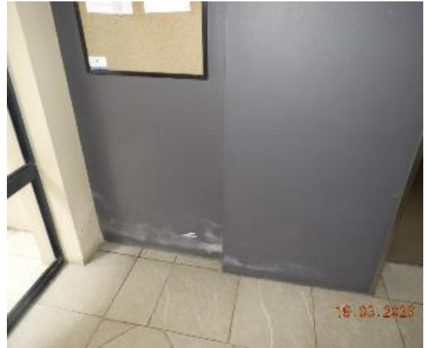
Figure 8 - General condition of level 1 common area internal wall
