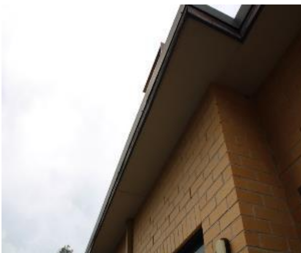
Figure 1318 - General condition of external wall
