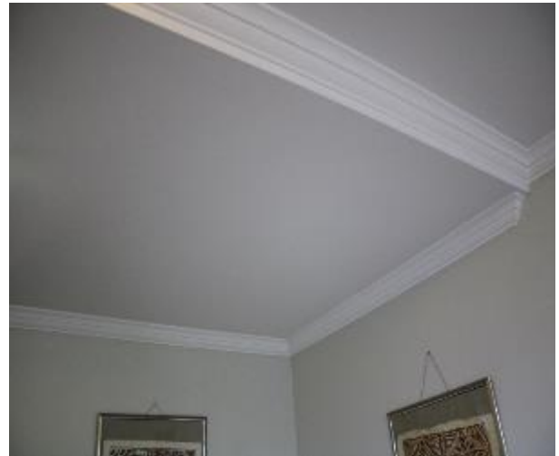
Figure 1457 - General condition of lounge room ceiling
