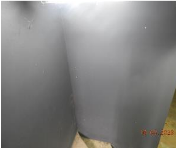
Figure 173 - General condition of B2 to Level 1 fire stairs internal wall
