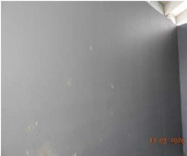
Figure 169 - General condition of B2 to Level 1 fire stairs internal wall
