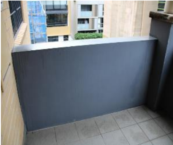
Figure 1236 - General condition of external wall
