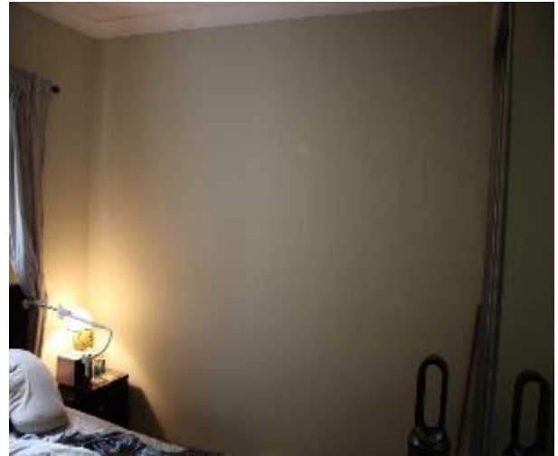
Figure 853 - General condition of bedroom 1 internal wall
