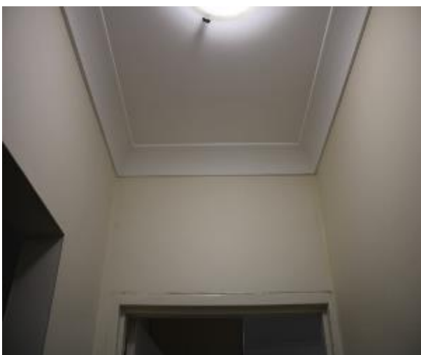
Figure 530 - General condition of corridor ceiling
