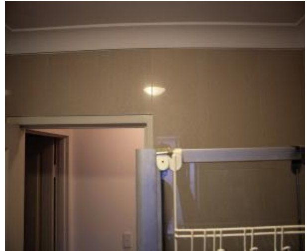
Figure 1042 - General condition of bathroom 1 internal wall
