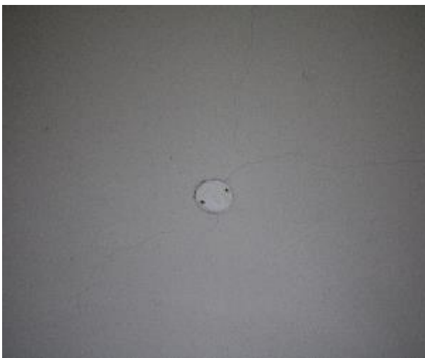
Figure 247 - Crack propagation through level 5 to basement B2 fire stairs underside slab
