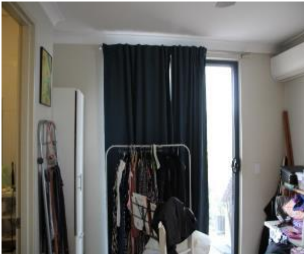
Figure 1474 - General condition of bedroom 1 internal wall
