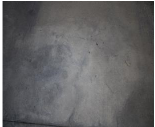
Figure 438 - General condition of basement B2 fire stairs pavement slab
