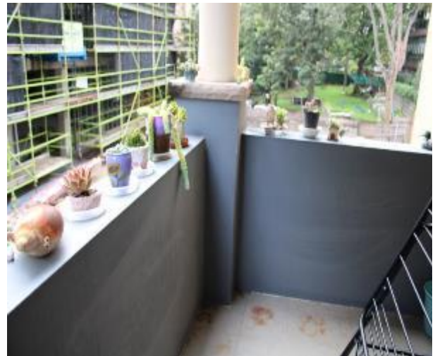
Figure 951 - General condition of external wall
