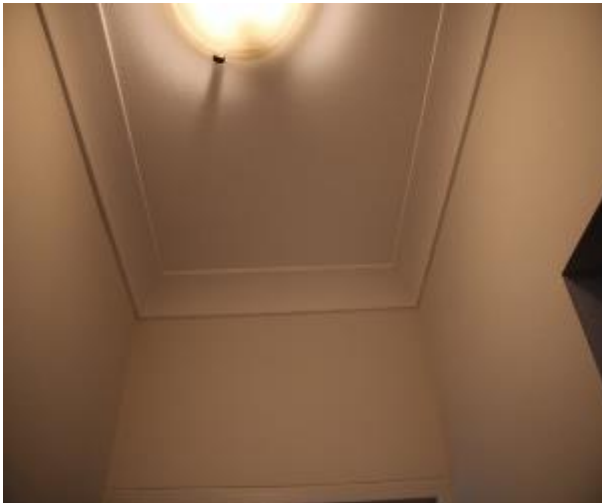
Figure 688 - General condition of corridor ceiling
