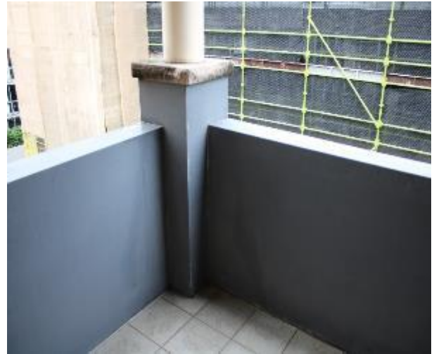
Figure 1237 - General condition of external wall
