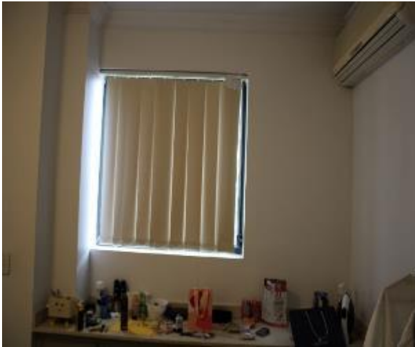
Figure 1284 - General condition of bedroom 1 internal wall
