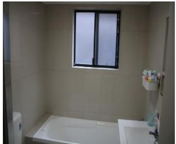
Figure 739 - General condition of bathroom 1 internal wall
