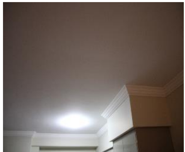
Figure 827 - General condition of open kitchen/ lounge room ceiling
