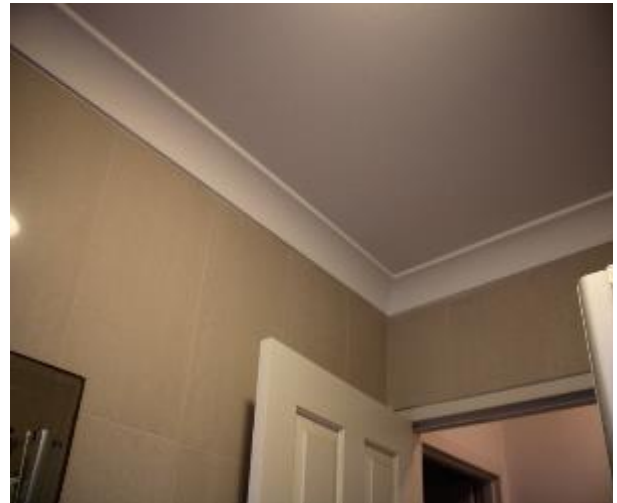
Figure 1044 - General condition of bathroom 1 internal wall
