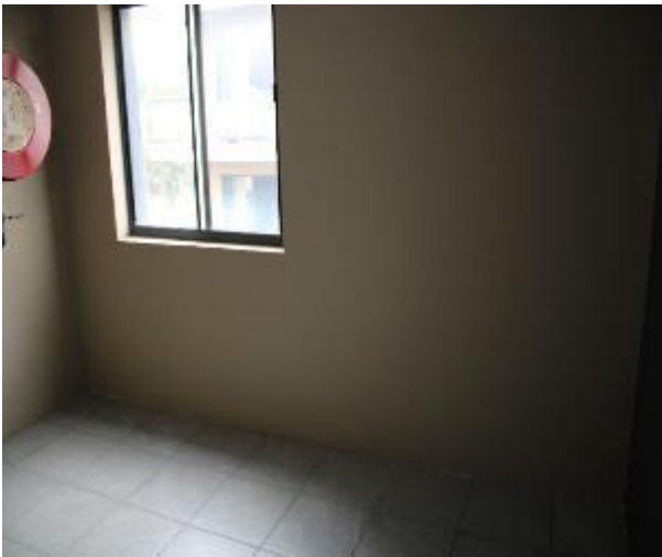
Figure 93 - General condition of level 4 common area internal wall
