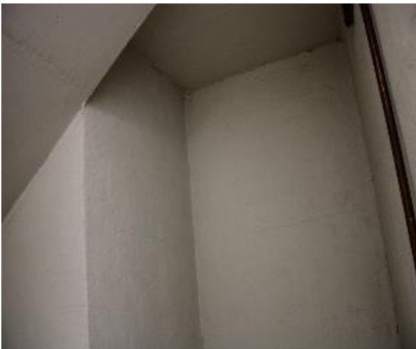
Figure 289 - General condition of level 5 to basement B2 fire stairs internal wall
