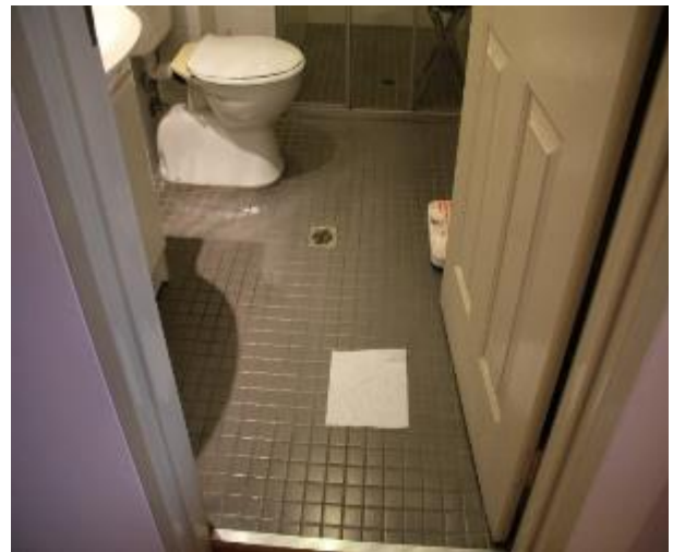
Figure 1143 - General condition of ensuite bathroom floor tiles
