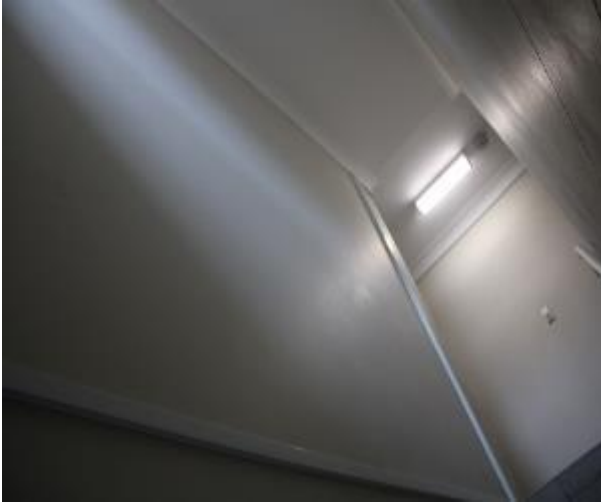
Figure 121 - General condition of staircase to level 5 common area internal wall
