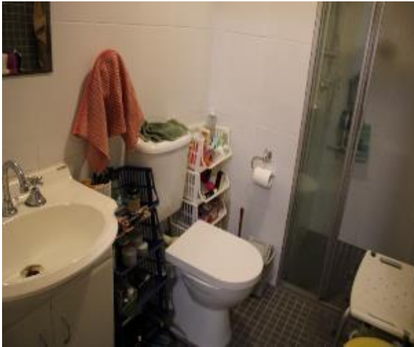
Figure 1005 - General condition of ensuite bathroom internal wall
