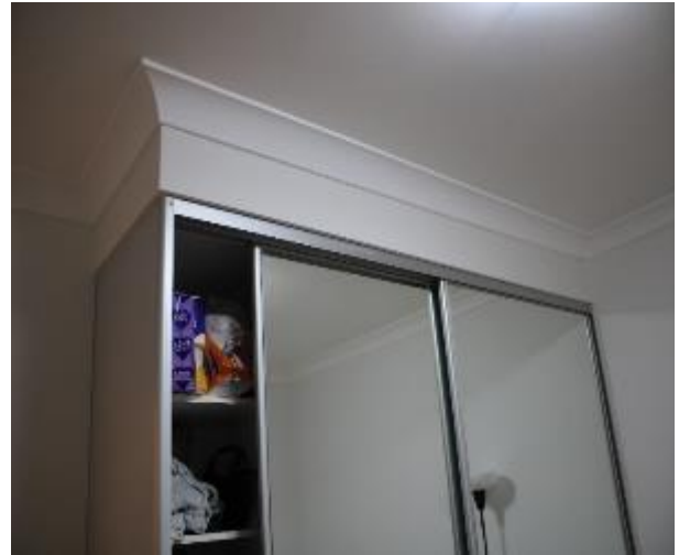
Figure 729 - General condition of bedroom 2 internal wall
