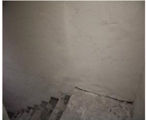
Figure 316 - General condition of level 5 to basement B2 fire stairs internal wall
