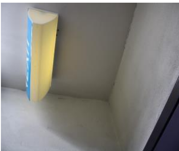
Figure 391 - General condition of level 5 to basement B2 fire stairs underside stairs
