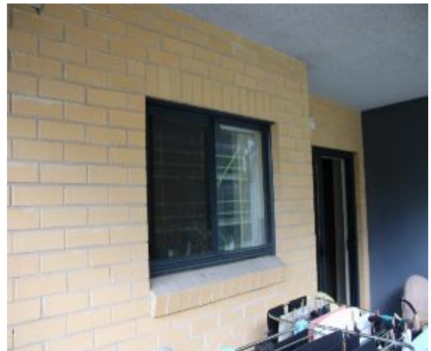
Figure 941 - General condition of external wall
