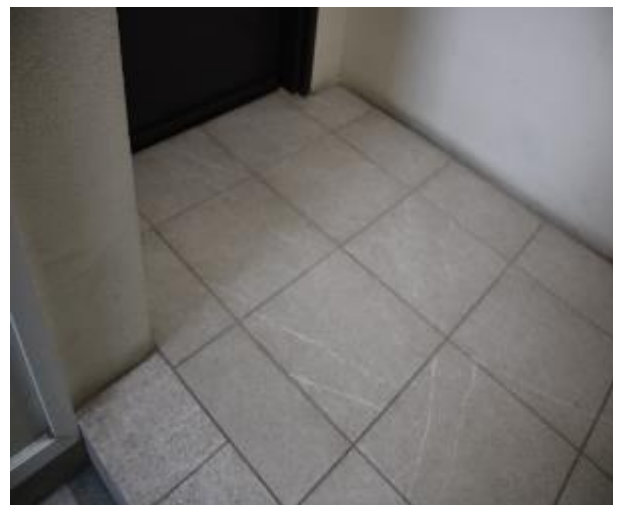
Figure 138 - General condition of level 5 common area floor tiles
