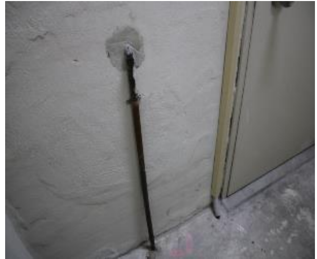
Figure 232 - General condition of level 5 to basement B2 fire stairs internal wall
