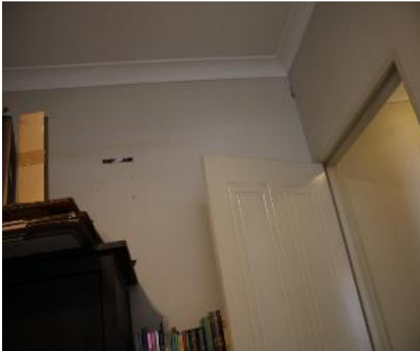
Figure 1556 - General condition of bedroom 2 internal wall
