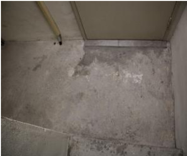
Figure 275 - General condition of level 5 to basement B2 fire stairs
