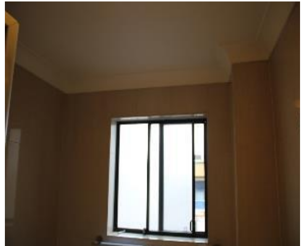
Figure 1185 - General condition of bathroom 1 internal wall
