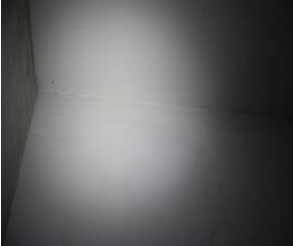
Figure 269 - General condition of level 5 to basement B2 fire stairs internal wall
