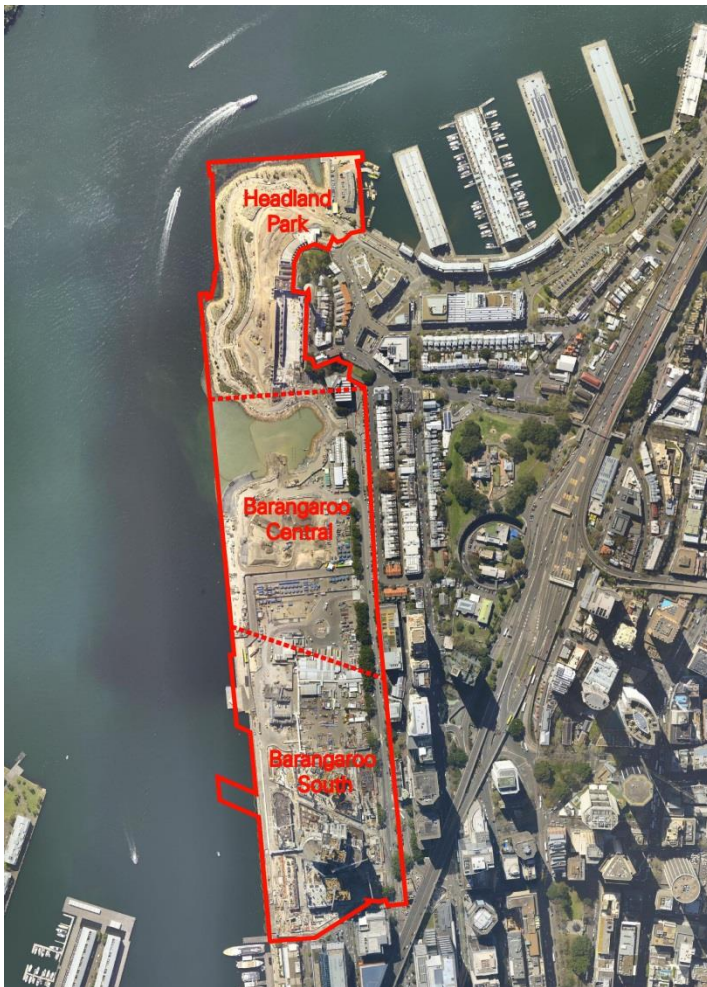
Figure 1 – Barangaroo site locational context and precincts
