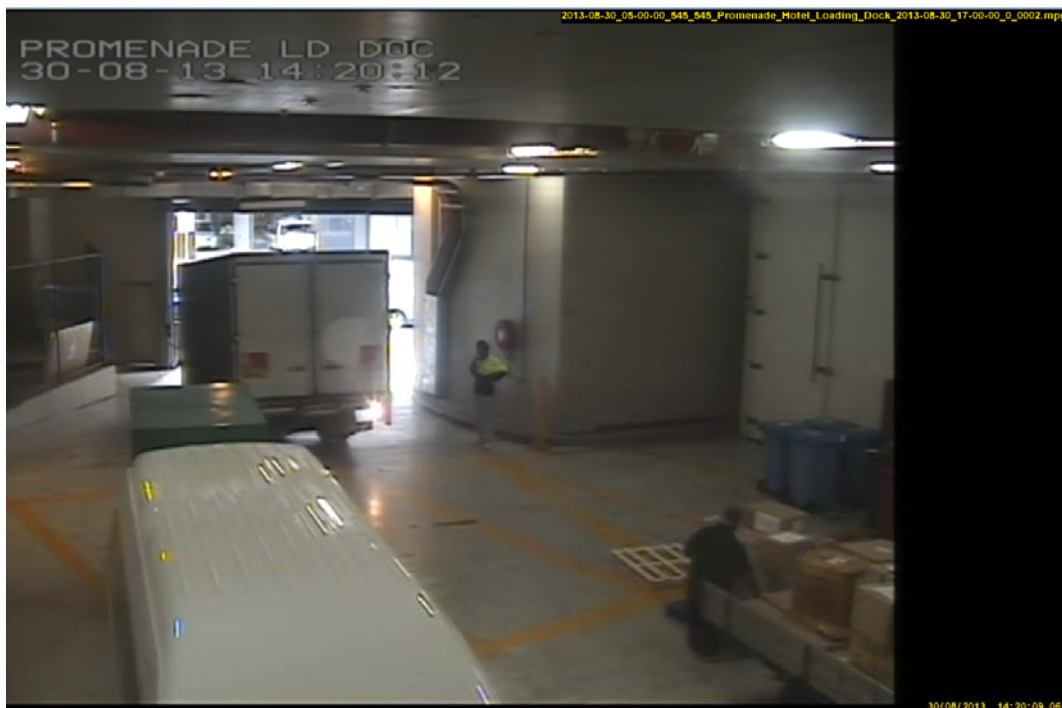
Figure 21 Crown Promenade Loading Dock
