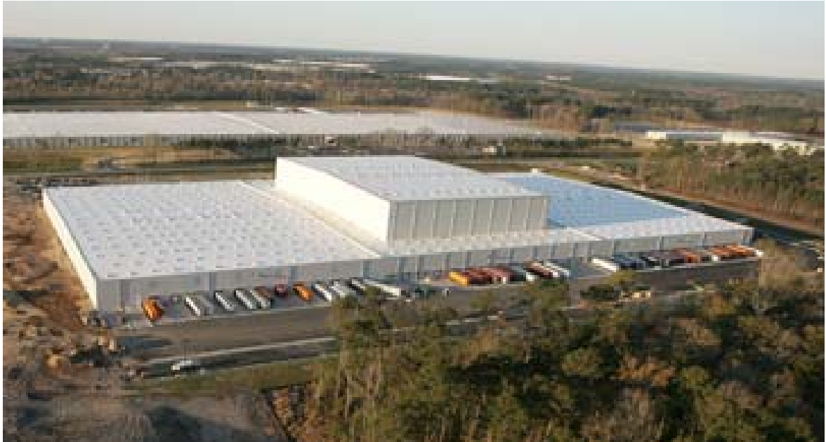
Figure 4.7: Highbay Warehouse, USA
