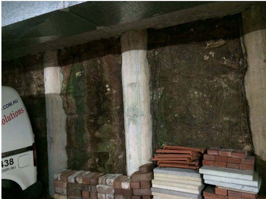
Photo 3: Northern wall – 3 of 5
