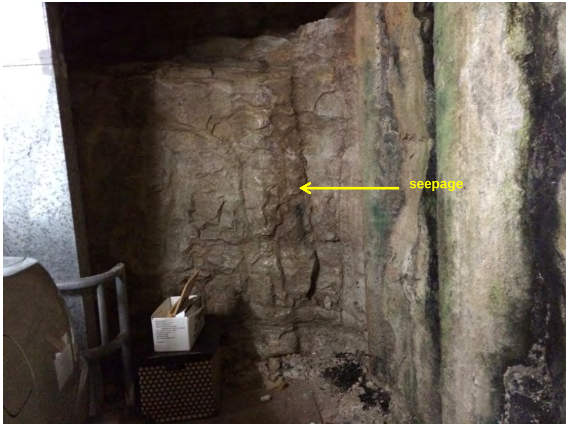
Photo 9: Southern wall western end – 1 of 3
