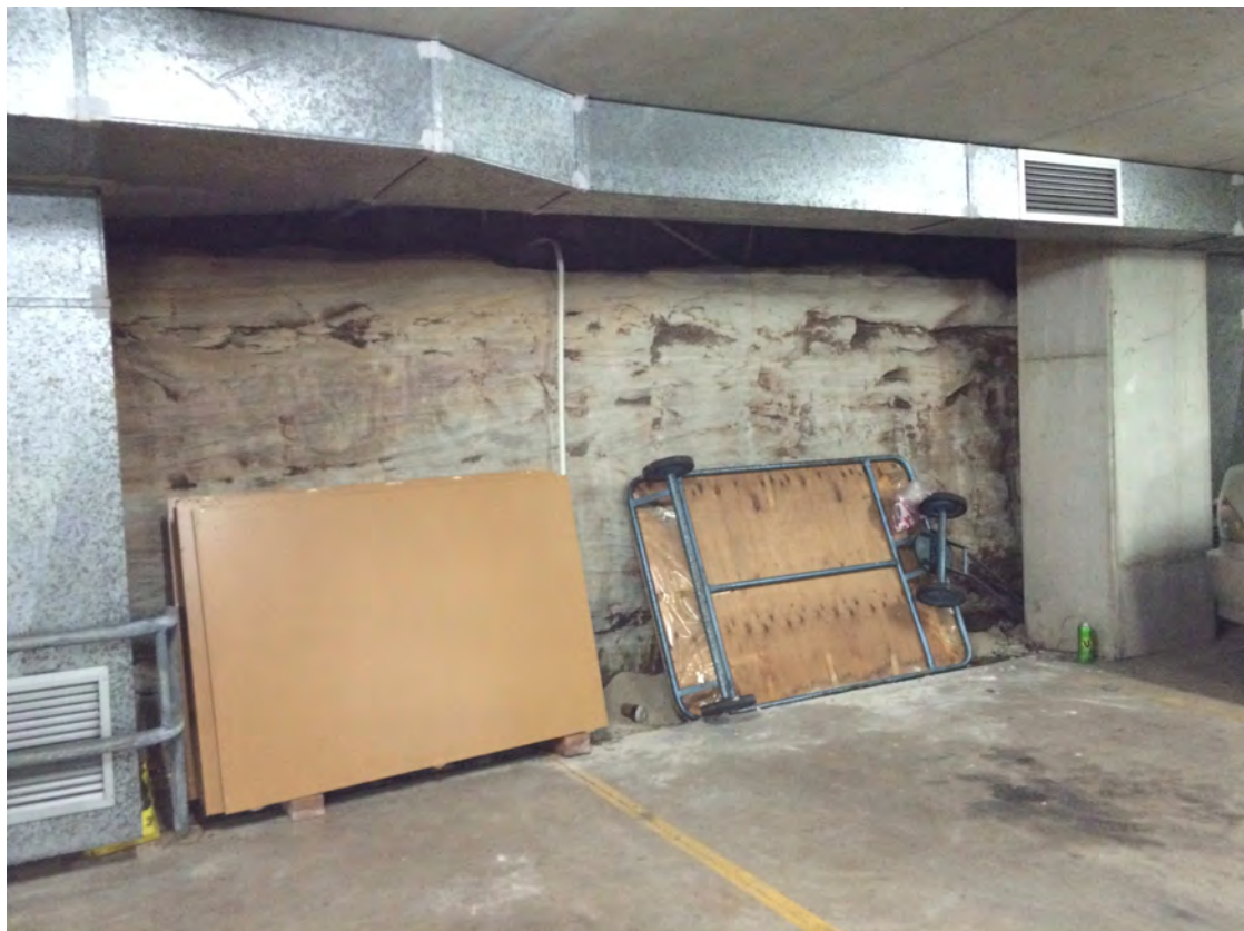
Photo 10: Southern wall – 2 of 3
