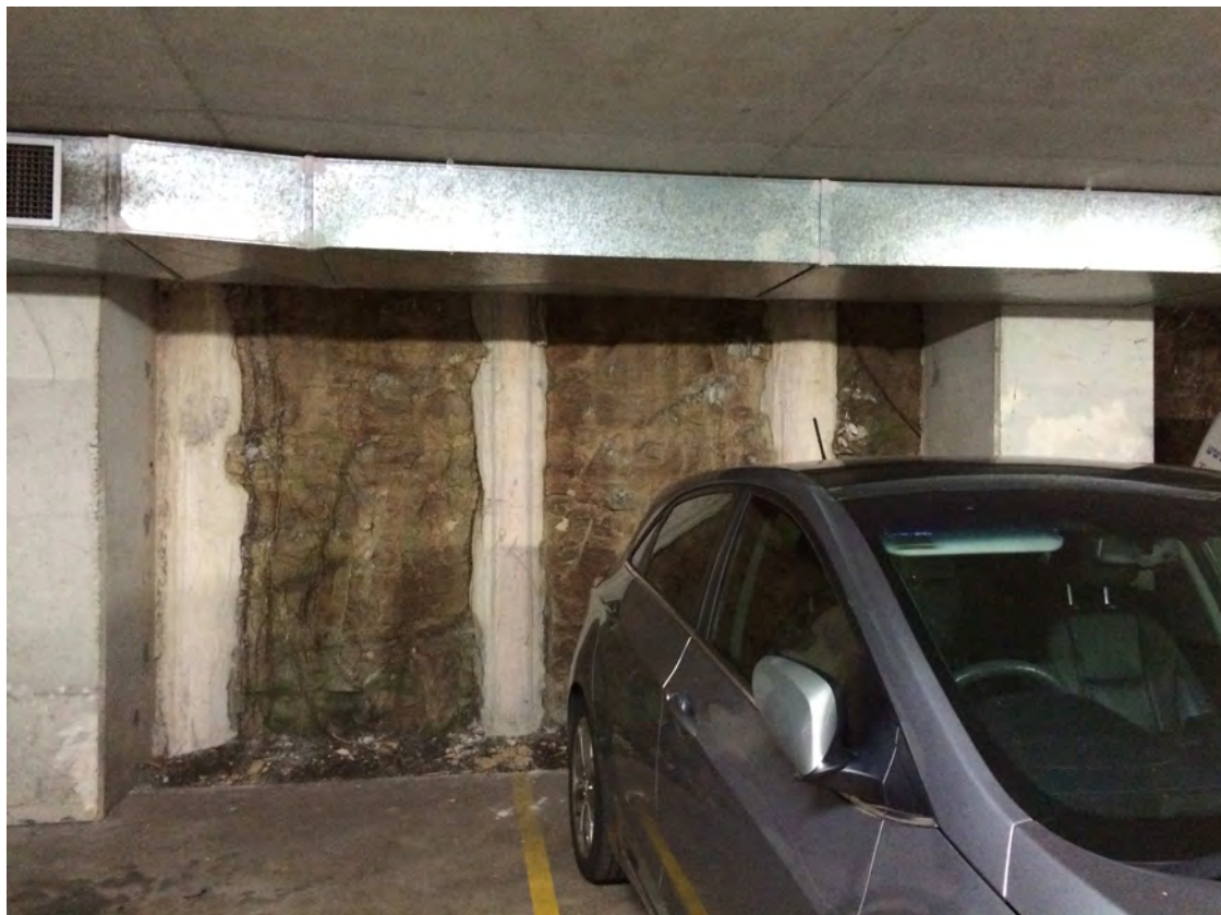
Photo 4: Northern wall – 4 of 5
