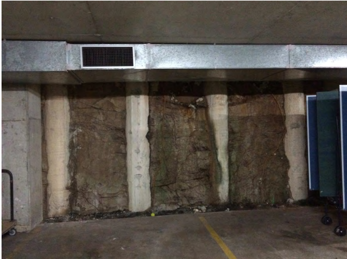
Photo 5: Northern wall near the western end– 5 of 5
