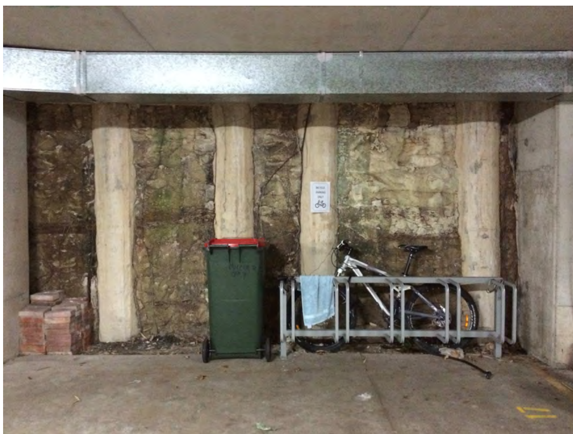
Photo 1: Northern wall – 2 of 5
