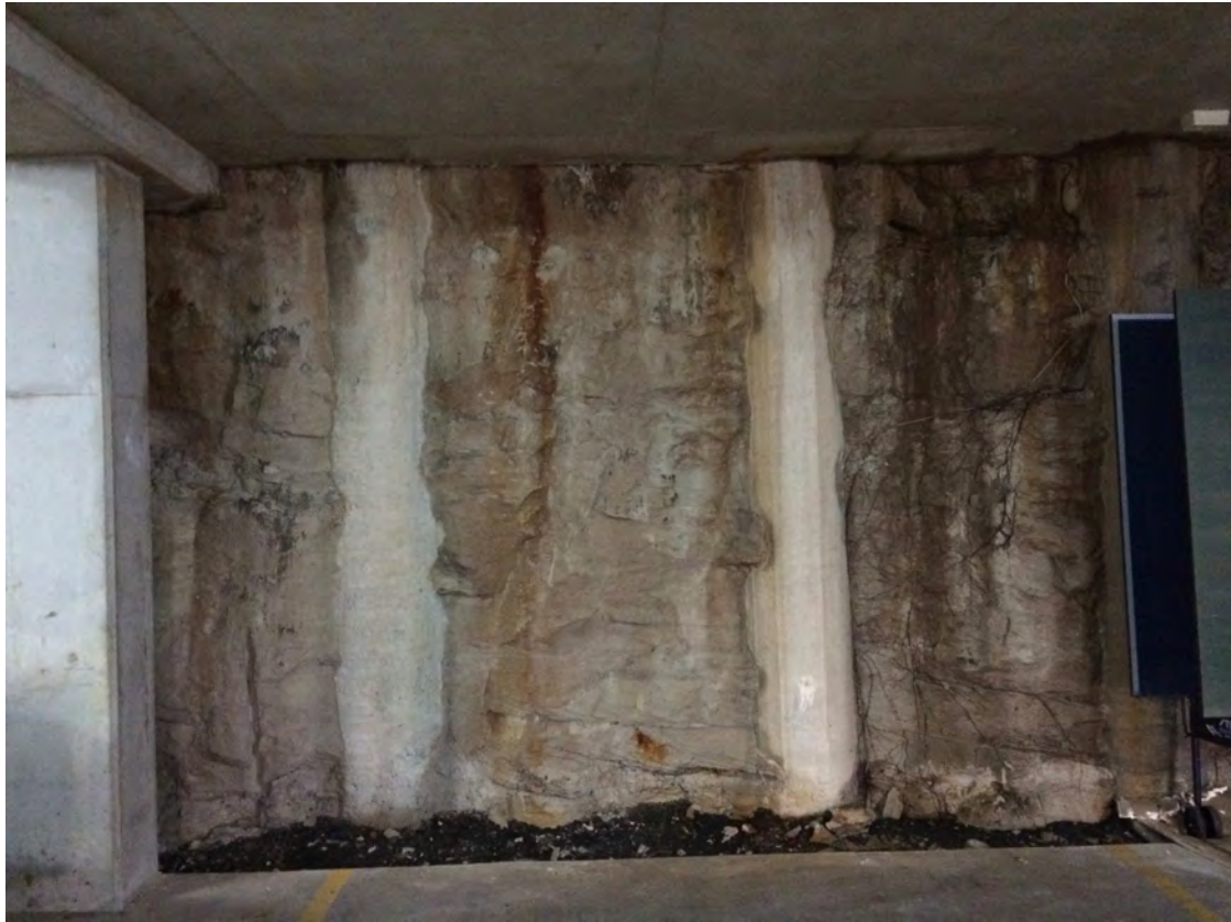
Photo 7: Western wall – 2 of 3
