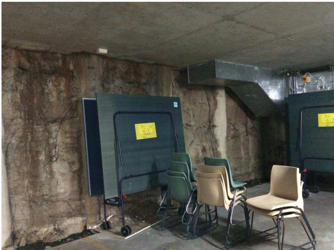
Photo 6: Western wall northern end– 1 of 3
