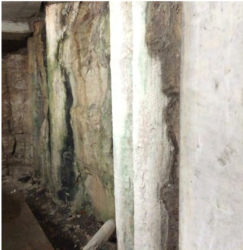
Photo 8: Western wall southern end – 3 of 3
