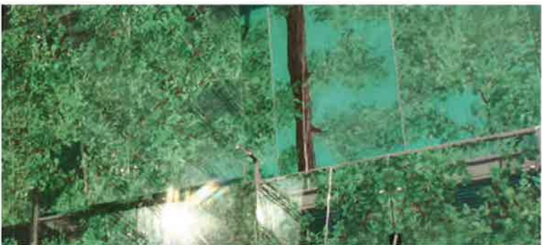
GL1-LAMINATED GLASS WITH INTERLAYER TO NORTHERN GLASS WALL FOR BOUNDARY SETBACK. DESIGN OF INTERLAYER TBC IMAGE SHOWN AS EXAMPLE ONLY.
