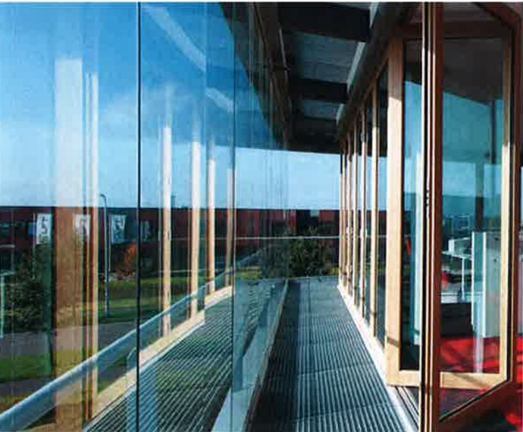
GCL-CLEAR GLASS WHERE POSSIBLE IT IS THE DESIGN INTENTION FOR GLASS TO BE CLEAR AND FRAMES TO BE THIN AND ELEGANTLY DETAILED.
