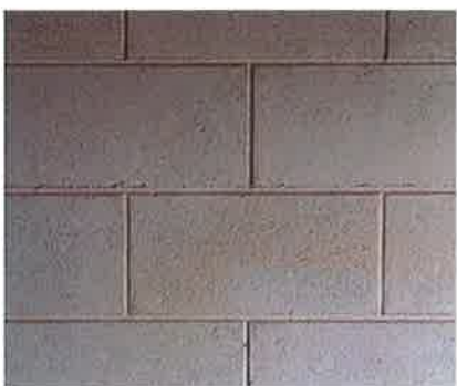
BLRP-BLOCKWORK RENDERED & PAINTED.
