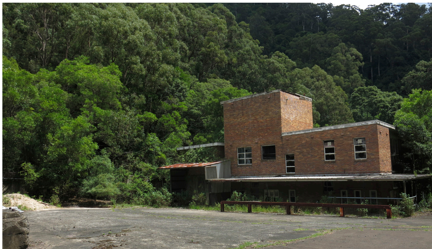
Workshop Concrete Pad
