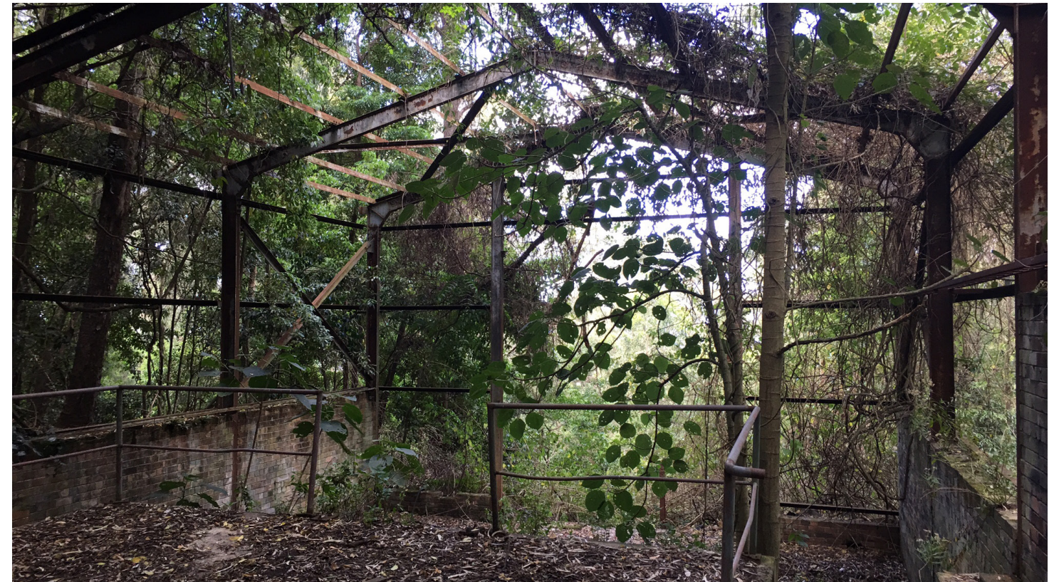
Coal Conveyor Gantry
