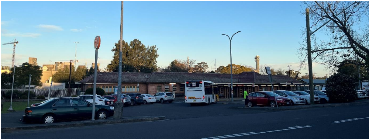
Figure 5.4: Bomaderry Station, Meroo Street, Bomaderry
