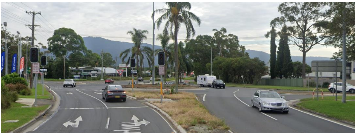
Figure 5.3: View north on Princes Highway of roundabout intersection with Moss Vale Road/Cambewarra Road
