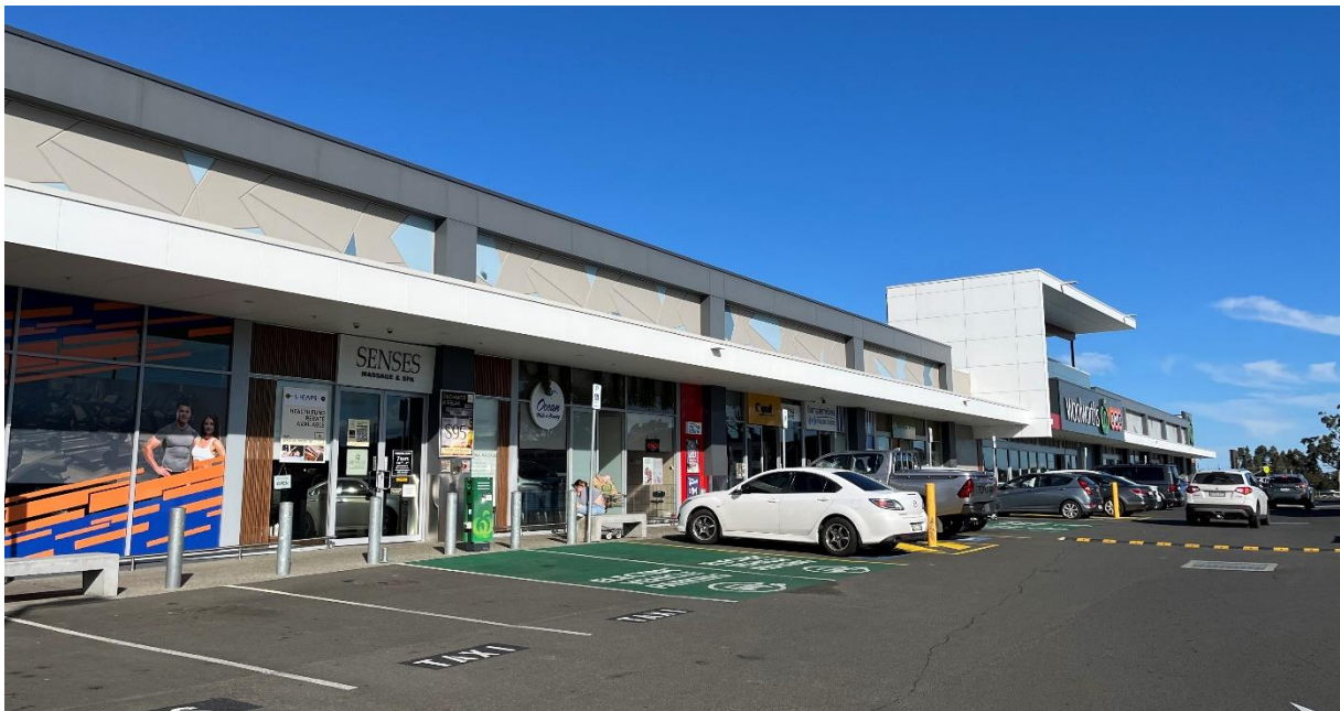
Figure 5.6: Bomaderry Woolworths Shopping Strip, Princes Highway & Cambewarra Road
