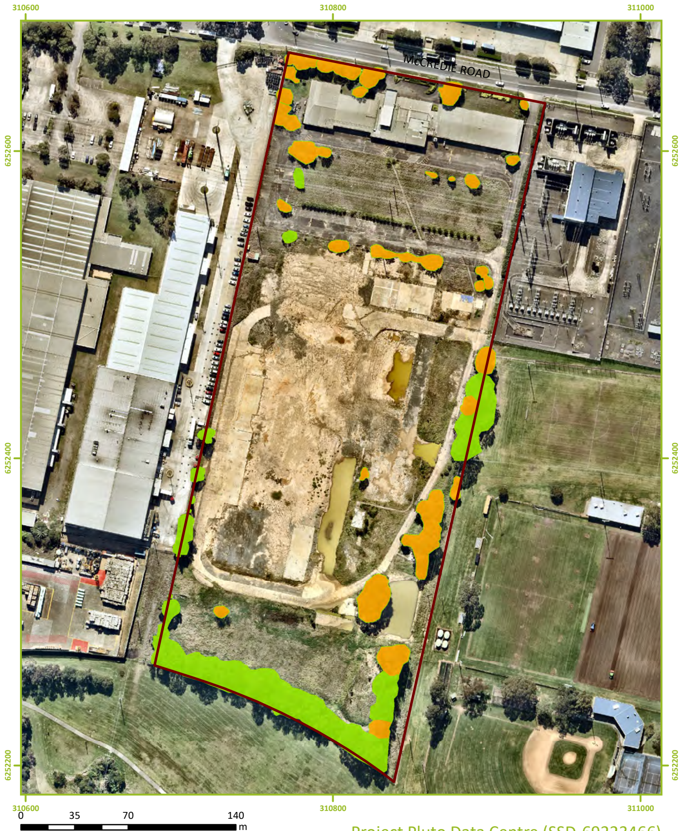
Project Pluto Data Centre (SSD-69223466)
