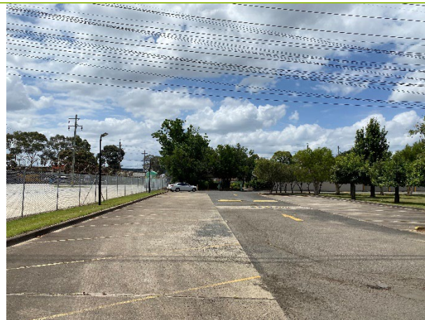
Photo 6. Car park landscaping (western end of northern site portion)
