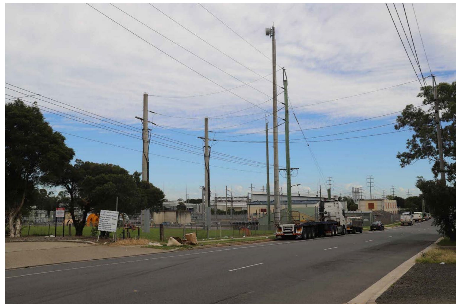
Figure 13 Viewpoint 02 existing view.
