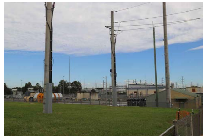
Photo 7. View south-west from 120 McCredie Road.
