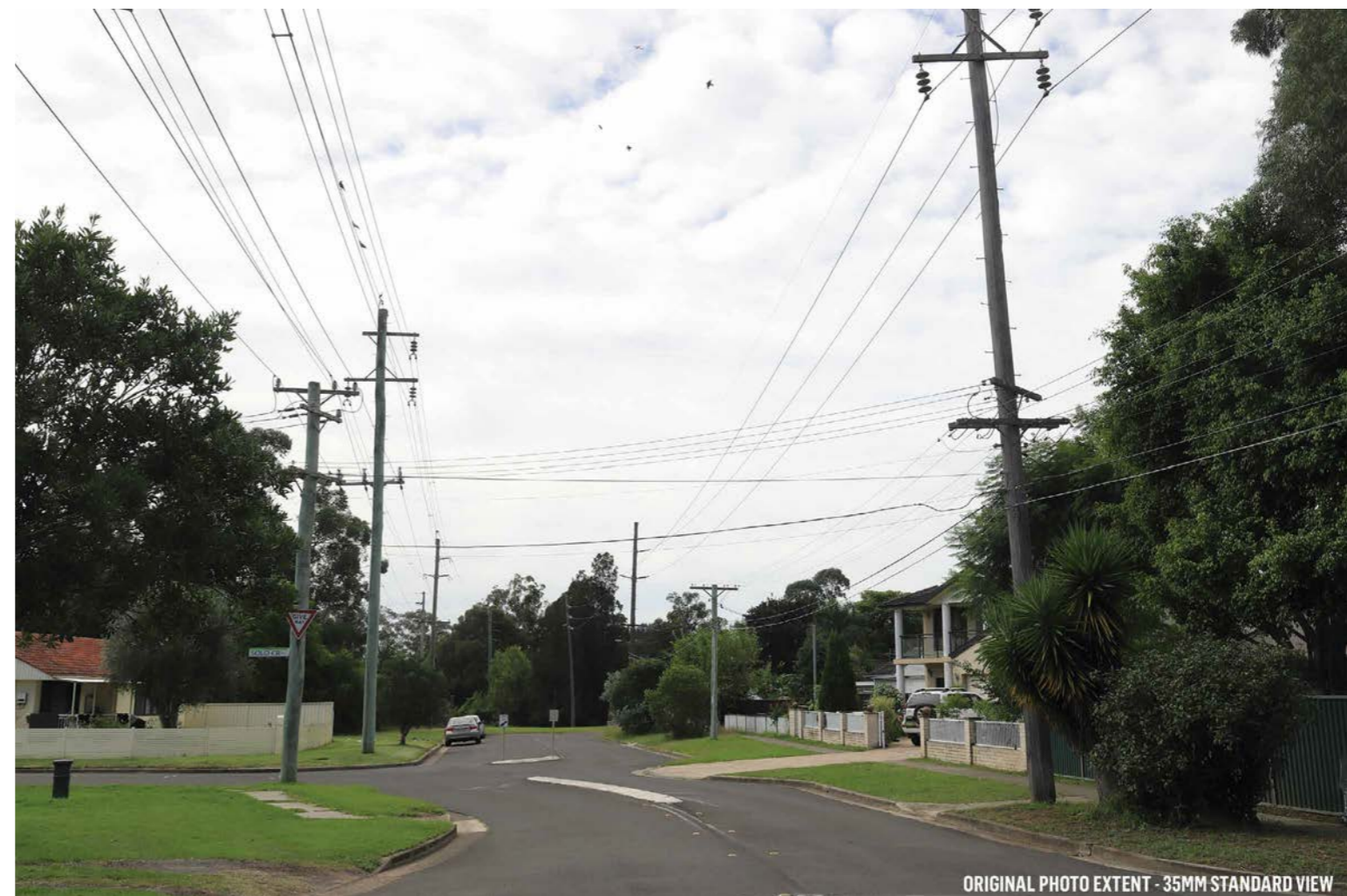
Figure 25 Viewpoint 06 existing view.
