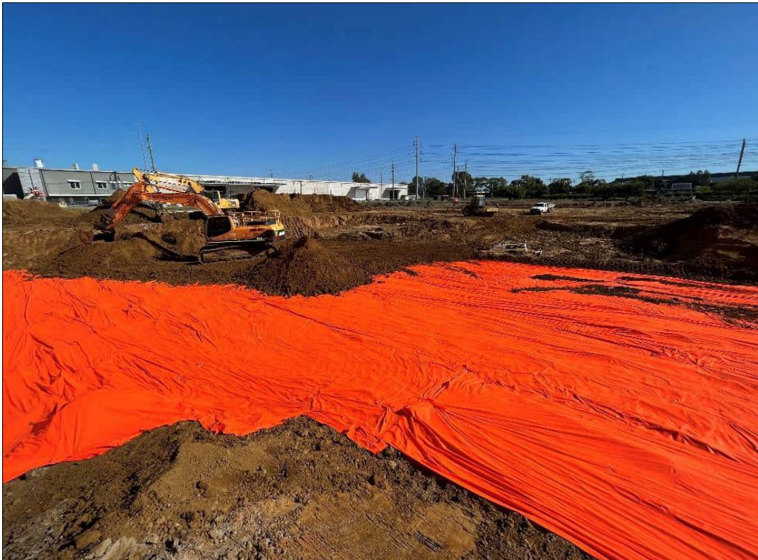
Photo 1: Orange, Mesh Geotextile Marker Layer Present Overlaying Asbestos Containment Cell
