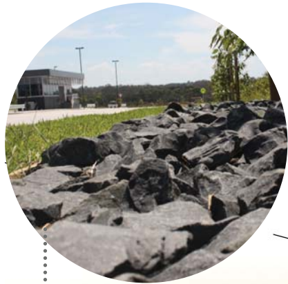
Ballast under road barrier between kerb and turf
