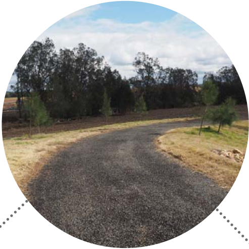
Spray seal maintenance road 4m for Fire Service, 3m for basin and biodiversity
