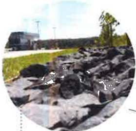
Ballast under road barrier between kerb and turf
