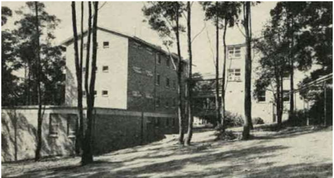
Figure 49: The Nurses' Home, showing bridge connections between the two wings and the Nurses' Training School (Source: Hospitals' Association Journal, May 1967, page 3)
