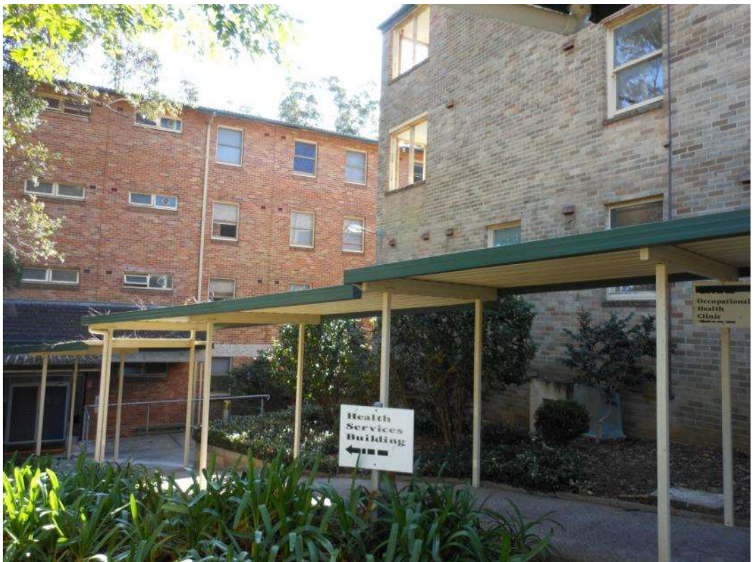
Figure 11: The older portion of the hospital, now used for education and training.
