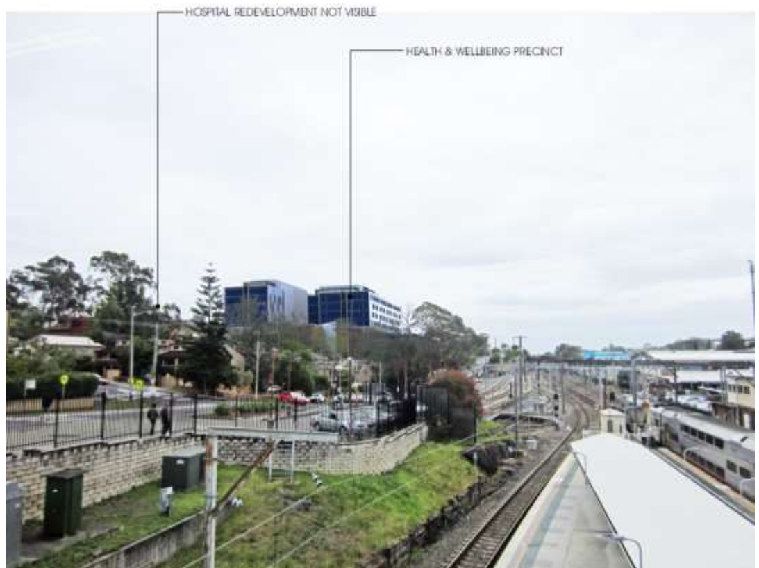
Figure 60: Gosford Train Station - Comparative view of the Approved (top) and s96 modification (bottom) view towards North. Note that only the proposed Health & Wellbeing Precinct is visible from this aspect. (Source: Fitzpatrick + Partners)
