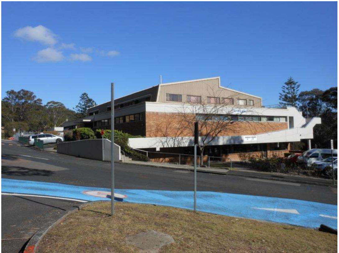
Figure 10: Health Services Building (adjacent to Racecourse Road), viewed from internal hospital road
