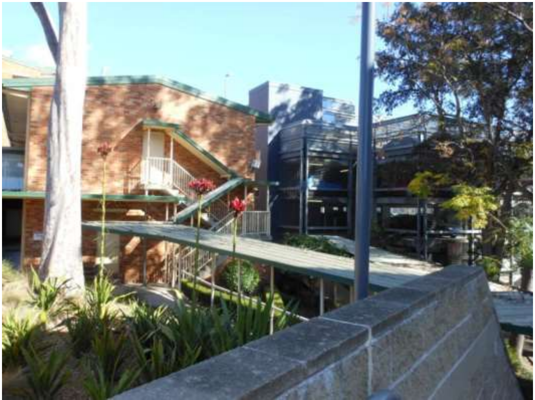
Figure 18: Administrative buildings associated with the main hospital building
