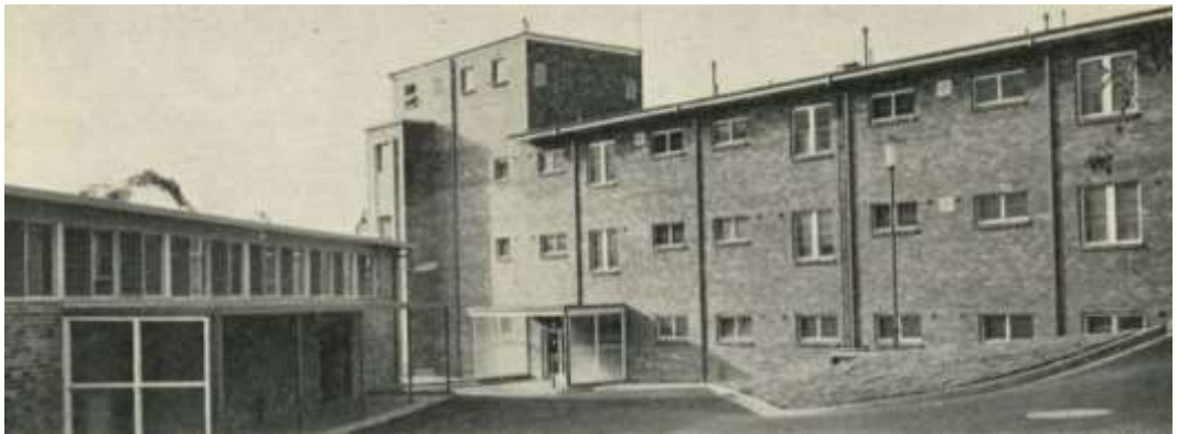
Figure 48: Rear of Hospital, showing entrance to Casualty Section, and, on left, the Laundry (Source: Hospitals' Association Journal, May 1967, page 3)
