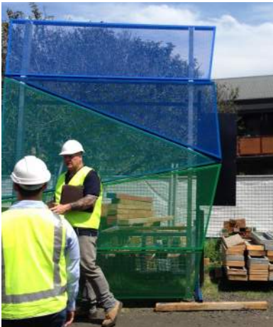
B PERFORATED METAL FACADE
