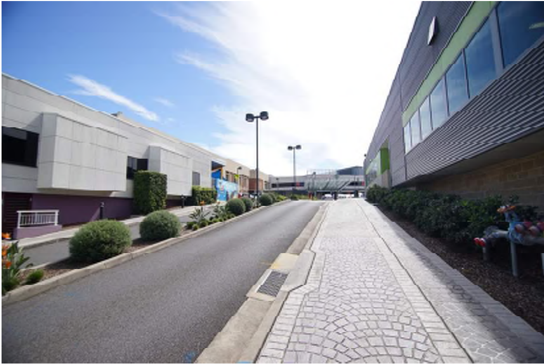
1 Beane Street leading up to the Main Entrance of Gosford Hospital
