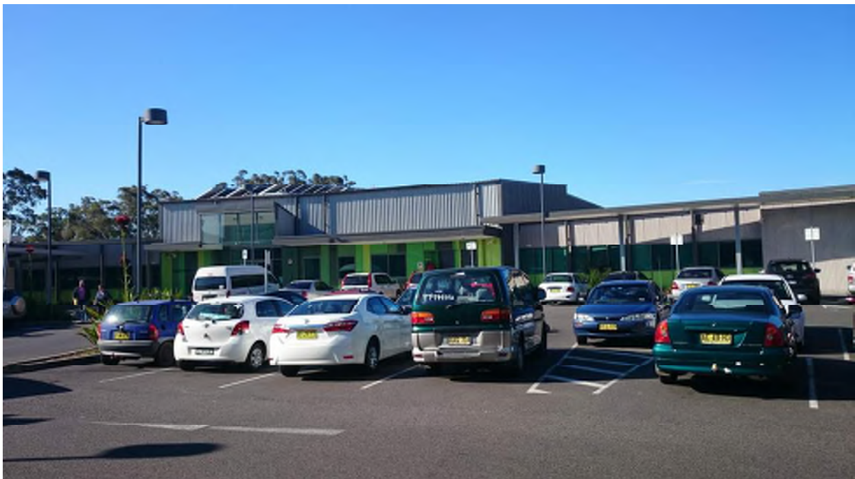
6 Existing New Mental Health Building Opposite Main Entrance
