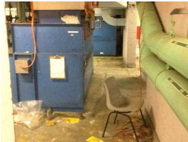
Photo No: J128740-001-MAND-Photo004 Result: SMF - Positive Building/Level: Main Building-All Levels Room/Location: All areas-Throughout Feature/Material: On Ground-Insulation Material
