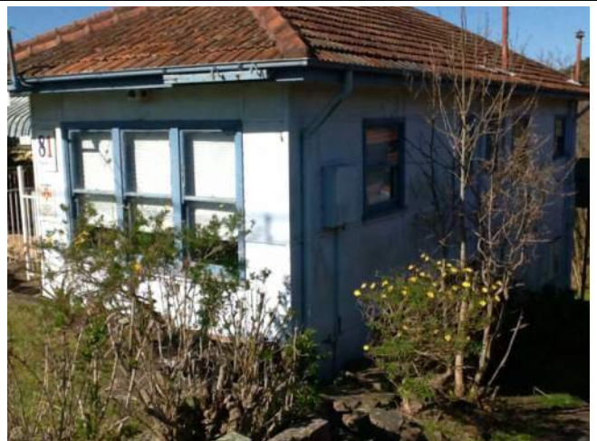
Photo No: J128740-002-ABOR-Photo014 Result: Lead (Paint) - Presumed Positive Building/Level: Main Building-Ground Level Room/Location: Surroundings- Feature/Material: Wall-Paint System/s
