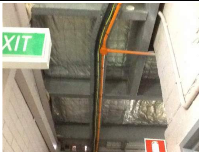
Photo No: J128740-001-MAND-Photo006 Result: SMF - Positive Building/Level: Main Building-Level Three Room/Location: All areas-Throughout Feature/Material: Roof Lining-Sarking Insulation
