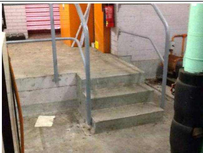
Photo No: J128740-001-MAND-Photo007 Result: Lead (Dust) - Positive Building/Level: Main Building-Level Three Room/Location: All areas-Various Throughout Feature/Material: All surfaces-Accumulated Dust
