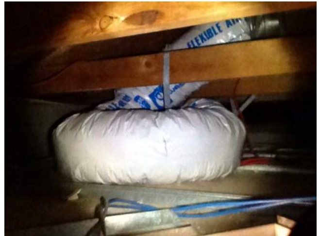
Photo No: J128740-001-MAND-Photo029 Result: SMF - Positive Building/Level: Main Building-Levels One & Two Room/Location: Various Rooms-Ceiling Space Feature/Material: Flexible Ductwork Insulation-Insulation Material
