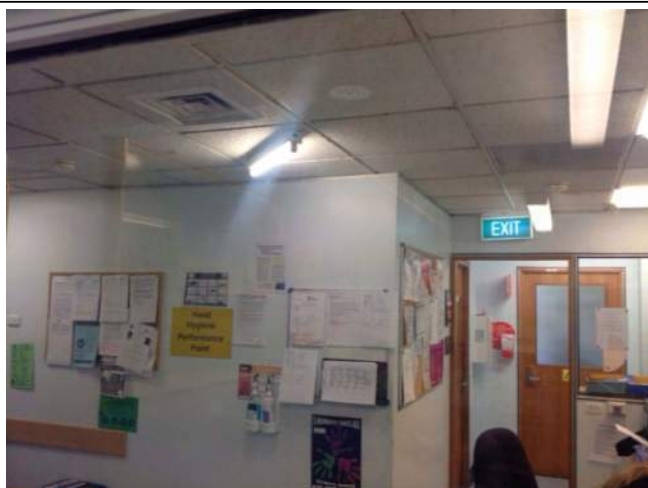
Photo No: J128740-003-HEAL-Photo001 Result: SMF - Presumed Positive Building/Level: Health Services Building-Level One Room/Location: Dental Surgery 1, 2, 3, 4 & 5, Laboratory, Stores and Reception Area- Feature/Material: Ceiling Tiles-Compressed Ceiling Tiles
