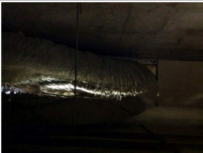
Photo No: J128740-003-HEAL-Photo045 Result: SMF - Presumed Positive Building/Level: Health Services Building-Level One Room/Location: Throughout Level-Ceiling Space Feature/Material: Flexible Ductwork Insulation-Insulation Material
