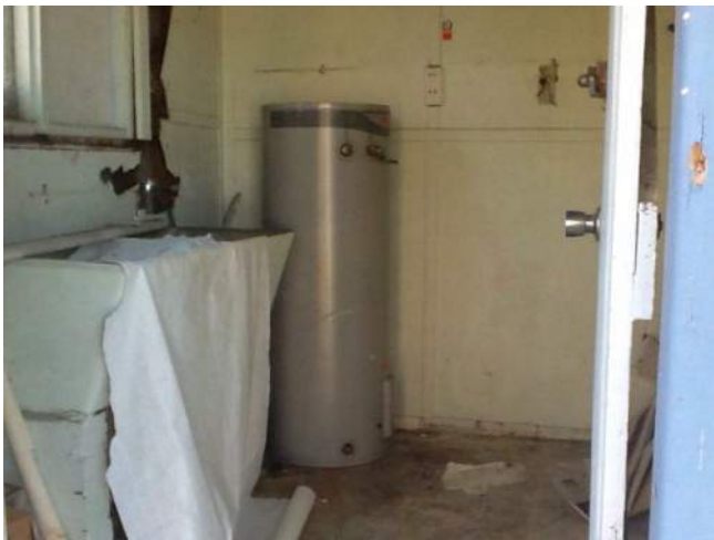
Photo No: J128740-002-ABOR-Photo018 Result: SMF - Presumed Positive Building/Level: Main Building-Basement Room/Location: Laundry (adjacent Toilets)- Feature/Material: Hot Water Heater-Insulation Material
