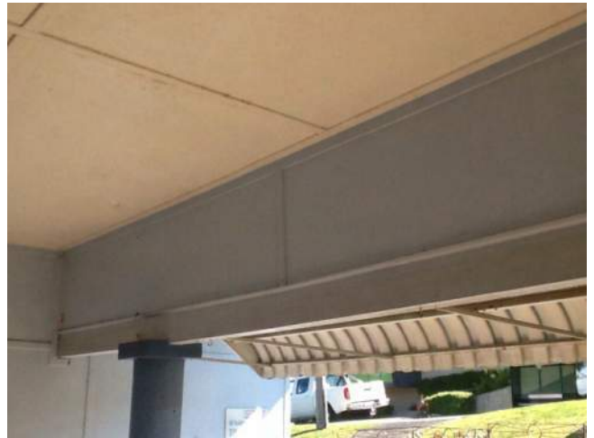
Photo No: J128740-002-ABOR-Photo012 Result: Asbestos - Presumed Positive Building/Level: Main Building-Ground Level Room/Location: Front Porch- Feature/Material: Infill Panels - High Level-Fibre Cement Sheetting
