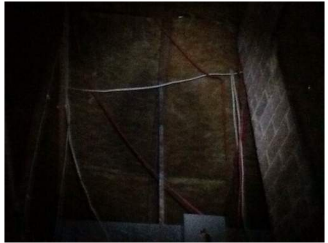
Photo No: J128740-001-MAND-Photo021 Result: SMF - Positive Building/Level: Main Building-Level Two Room/Location: Roof Space-Throughout Feature/Material: Roof Lining-Insulation Material
