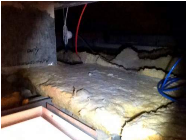
Photo No: J128740-001-MAND-Photo034 Result: SMF - Positive Building/Level: Main Building-Levels One & Two Room/Location: Ceiling Space-Variou Throughout Feature/Material: Insulation-Insulation Batts
