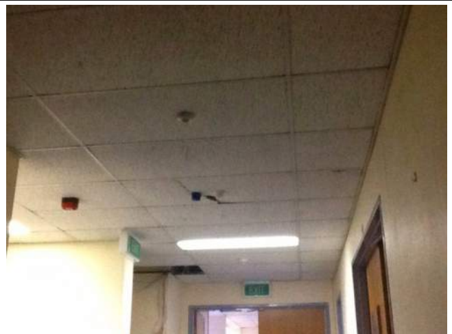
Photo No: J128740-001-MAND-Photo011 Result: SMF - Positive Building/Level: Main Building-Levels One & Two Room/Location: Various Rooms-Throughout Feature/Material: Ceiling Tiles-Compressed Ceiling Tiles
