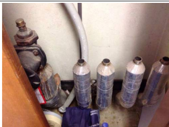
Photo No: J128740-003-HEAL-Photo017 Result: SMF - Presumed Positive Building/Level: Health Services Building-Level Three Room/Location: Human Resources-Reception Desk, Header Cupboard Feature/Material: Pipework Insulation-Insulation Material
