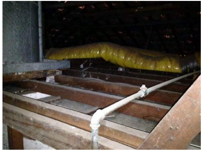
Photo No: J128740-002-ABOR-Photo008 Result: SMF - Positive Building/Level: Main Building-Ground Level Room/Location: Roof Space-Throughout Feature/Material: Flexible Ductwork Insulation-Insulation Material
