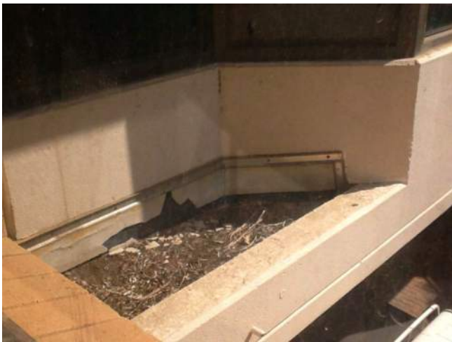
Photo No: J128740-001-MAND-Photo024 Result: Asbestos - Presumed Positive Building/Level: Main Building-Level Two Room/Location: Main Entrance-Adjacent Door Feature/Material: Wall Cladding-Fibre Cement Sheetting
