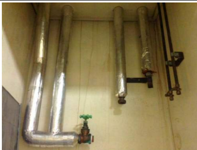
Photo No: J128740-003-HEAL-Photo002 Result: SMF - Presumed Positive Building/Level: Health Services Building-Level One Room/Location: Corridor between Dentist and Library-Header Cupboard Feature/Material: Pipework Insulation-Insulation Material
