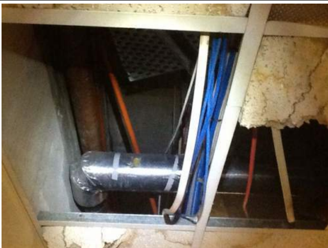
Photo No: J128740-001-MAND-Photo033 Result: SMF - Positive Building/Level: Main Building-Levels One & Two Room/Location: Various Rooms-Ceiling Space Feature/Material: Pipework Insulation-Insulation Material
