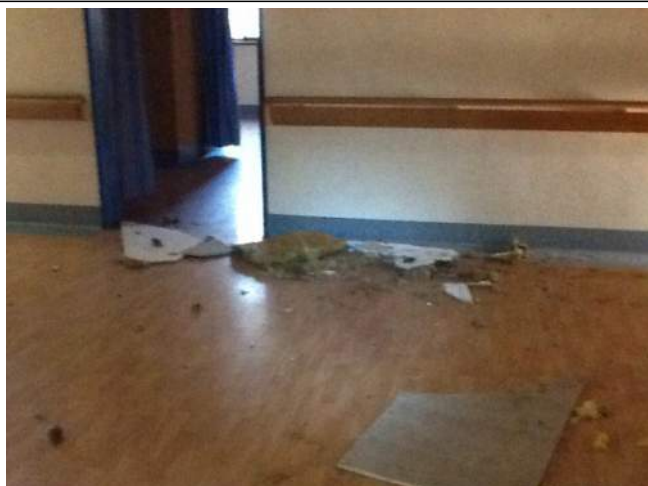
Photo No: J128740-001-MAND-Photo035 Result: SMF - Positive Building/Level: Main Building-Levels One & Two Room/Location: Various Rooms-Throughout Feature/Material: On Ground-Insulation Batt's
