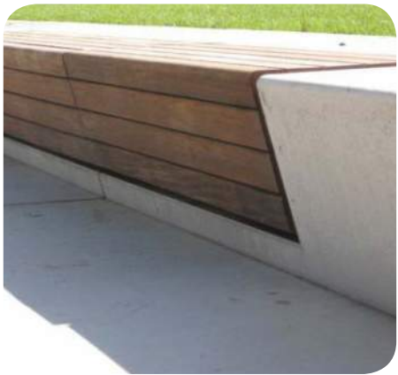
Concrete benche seating with composite timber inlays
