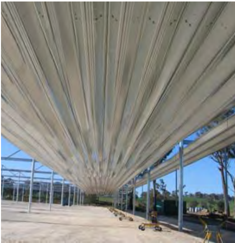
I METAL ROOFING
