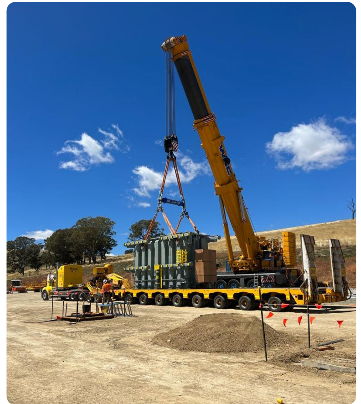
Left: Proposed transport equipment. Above: ARES transporting a 120-ton transformer on a platform trailer.
