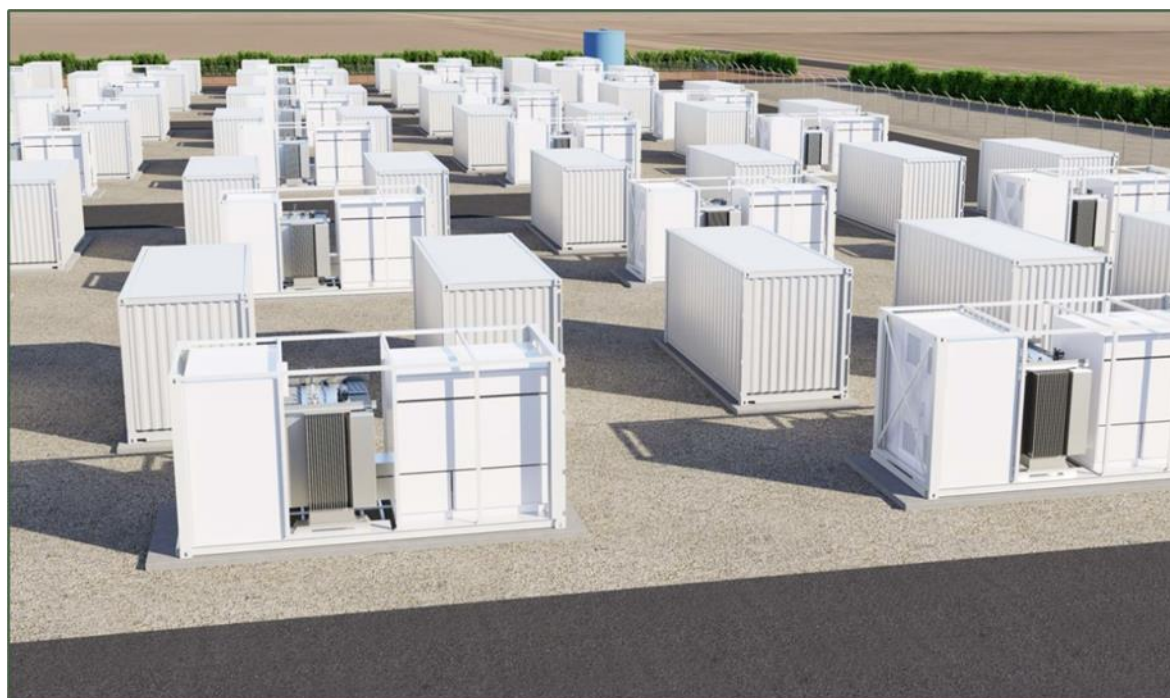
Figure 4 Indicative Image of BESS Modules
