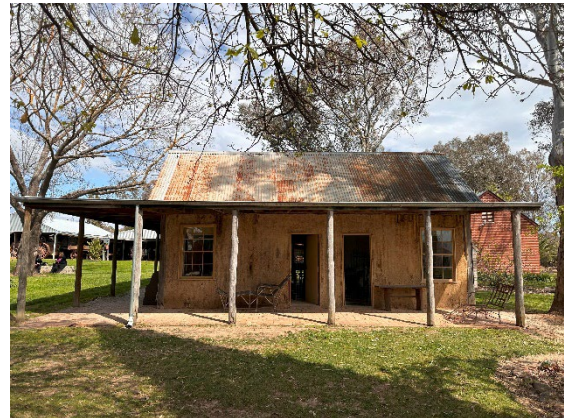
Figure 14 – Wattle & Daub Cottage (Wagner’s Store)
