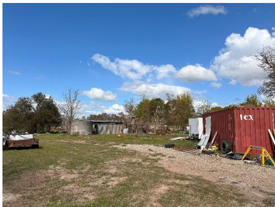
Figure 9 – Existing structures on site
