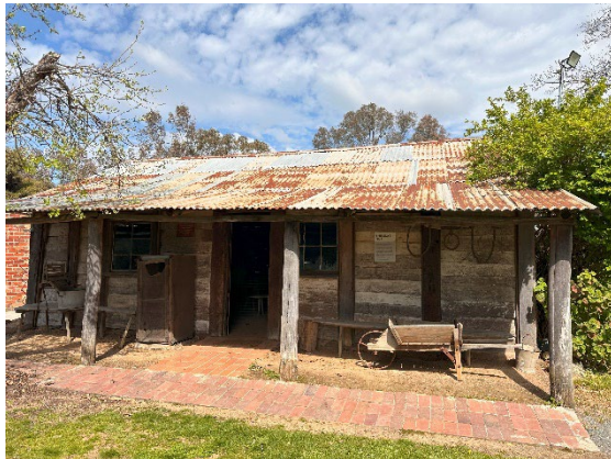
Figure 13 – Slab Hut (Wagner’s Store)
