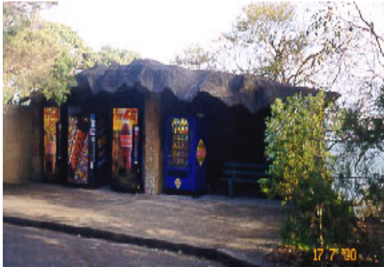
Figure 7.49 The former shelter exhibiting the use of ferro-cement to create a 'grotto' effect.
