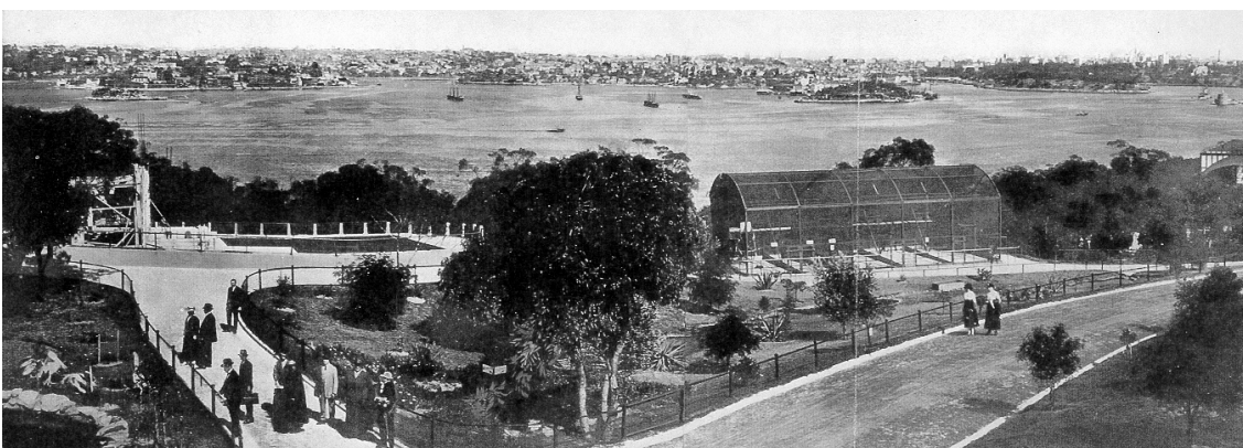
Figure 3.7 View south from Taronga Zoo across the harbour. In the right of the photo notice the caged bird exhibit, examples of which remain on-site. The path layout was a deliberate scheme, designed to draw the visitor along to each exhibit.
