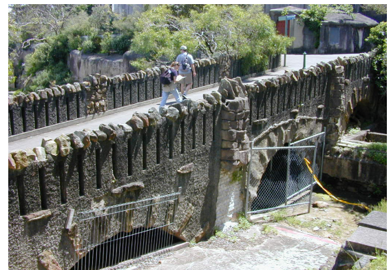
Figure 7.52 The use of small stones to give a rustic charm to the Rustic Bridge.
