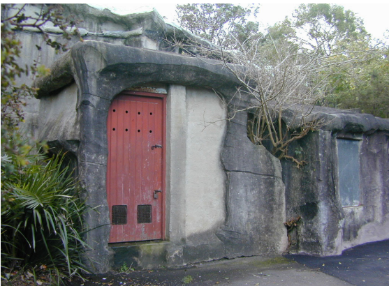
Figure 7.47 The Aquarium Building and its coating of ferro-cement to create a 'grotto' effect.
