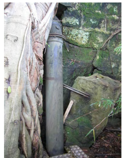
Figure 2.35 West end of wall 63L showing stormwater pipe and damage caused by fig tree roots.
