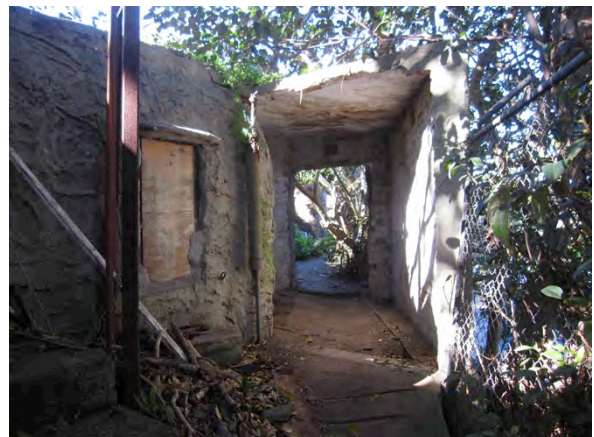
Figure 2.51 Rough openings made in the walls of the den over the Aboriginal site. Source: Jean Rice
