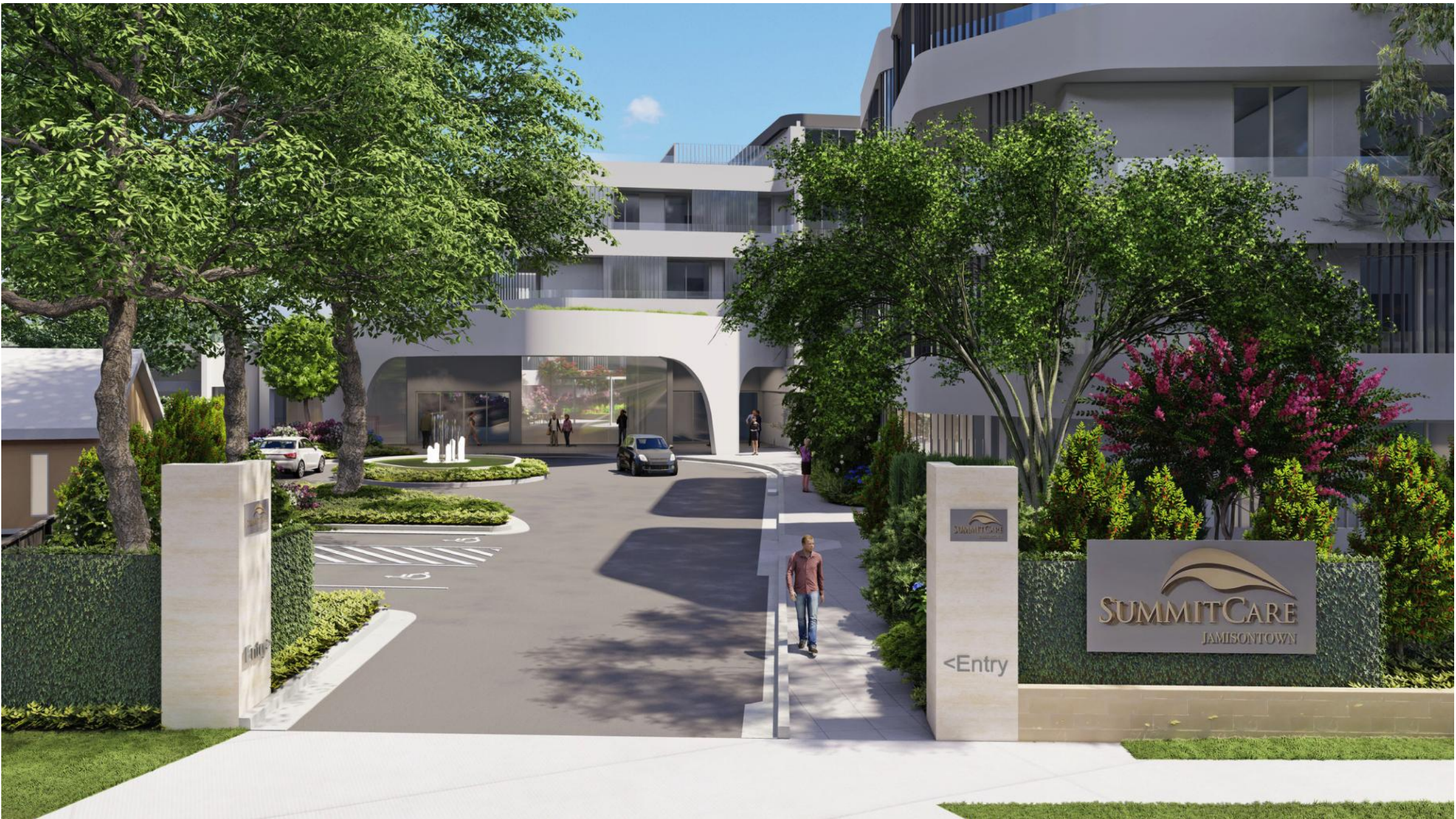
View of McNaughton Street Main Entrance
