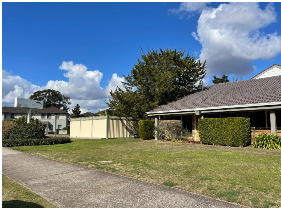
Figure 6: Existing unit, from Jamison Road South side looking East (source: The Planning Studio)
