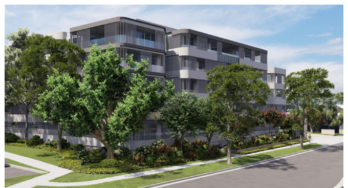
Figure 10: View from Harris Street looking towards Building A (Source: Arterra)
