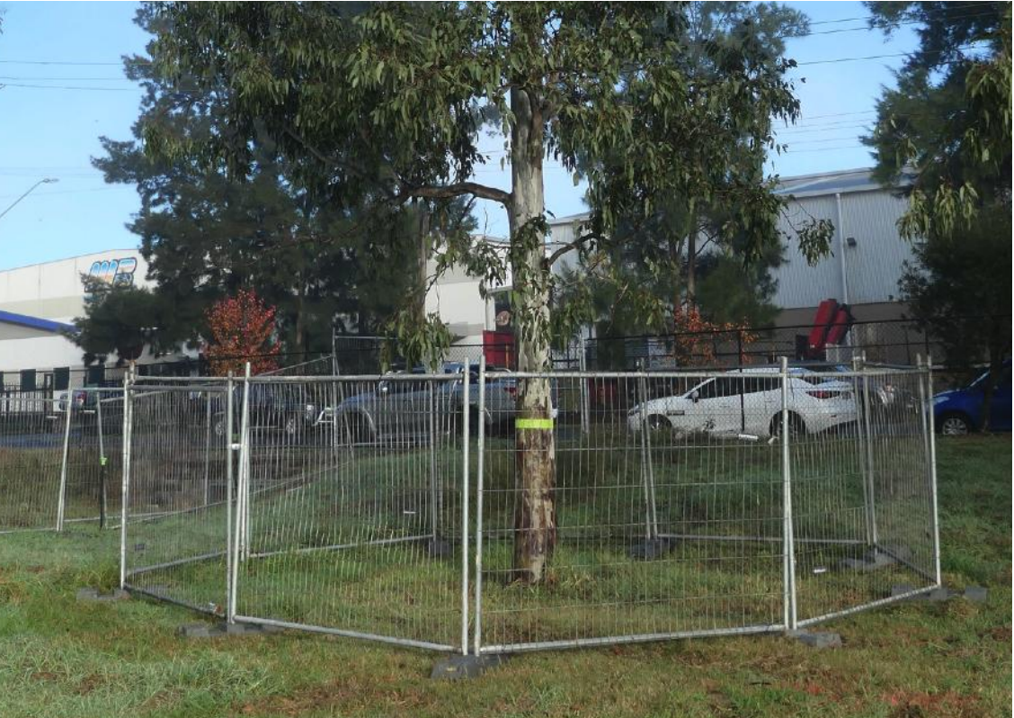
Example image of acceptable tree protection fencing measures to be applied. (1.8m high rigid metal fencing with appropriate lateral bracing)
