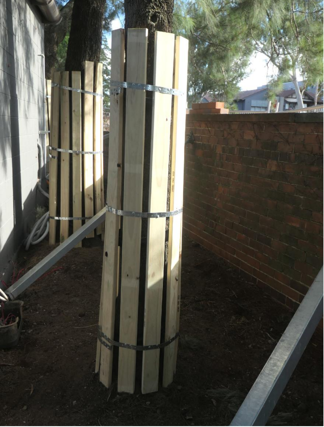
Example image of acceptable trunk protection battens
