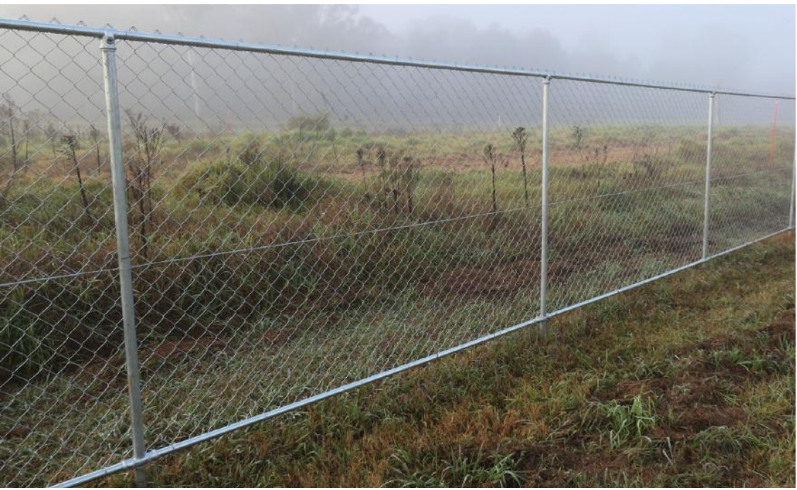
Example image of acceptable tree protection fencing measures to be applied. (1.8m high chainlink fencing with posts driven into ground)
