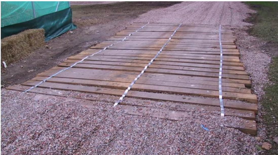
Figure 16 – Example of acceptable Tree Protection Area ground protection (Photo: Arterra)
