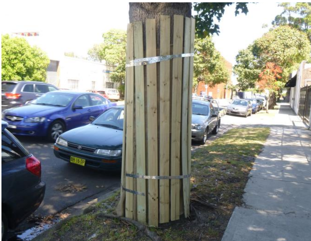
Figure 17 – Example of acceptable Trunk Protection batten installation. (Photo: Arterra)
