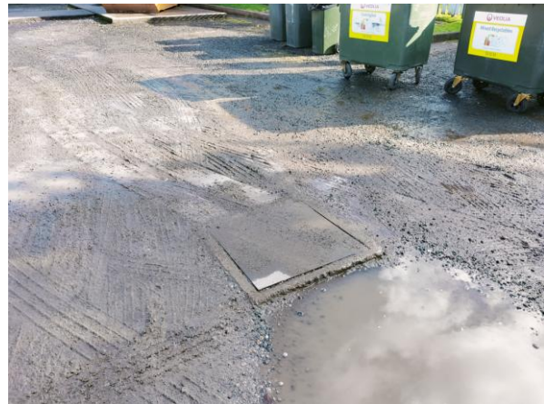
Figure 4.4 Evidence of subsurface services were observed.
