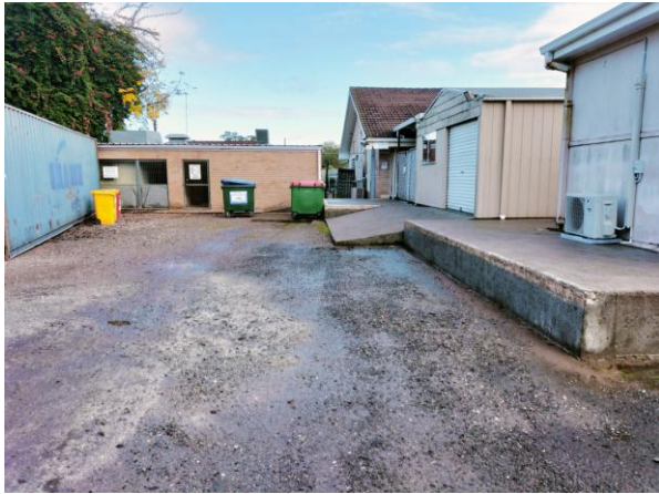
Figure 4.1 West-facing photo at the rear of SummitCare Penrith. Most of the study area is covered by hard surfaces, such as buildings and concrete, making evaluation of subsurface conditions difficult.
