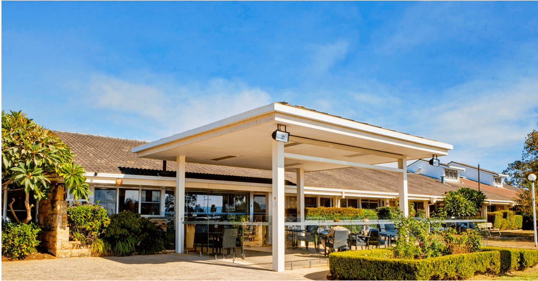
Figure 3: Existing aged care facility (SummitCare Penrith)
