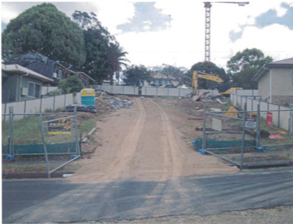
Photograph 17: View north towards 26 Dalziell Street
