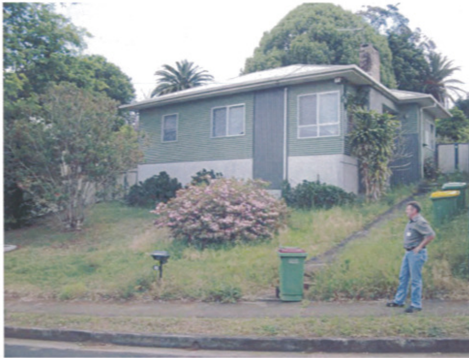
Photograph 15: View north towards the frontage of 24 Dalziell Street
