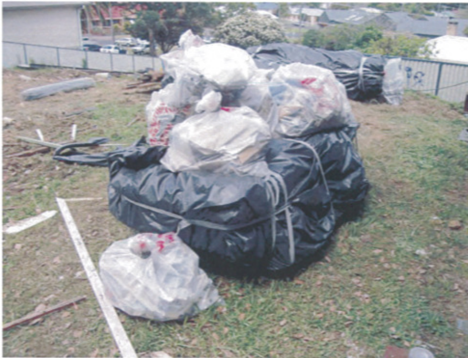
Photograph 19: Double-bagged ACM sheeting removed from the building under demolition
