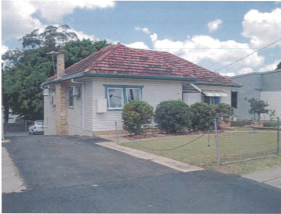
Photograph 1: View southwest towards the frontage of 61 Uralba Street
