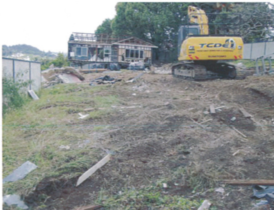
Photograph 18: View west from the eastern boundary of 26 Dalziell Street
