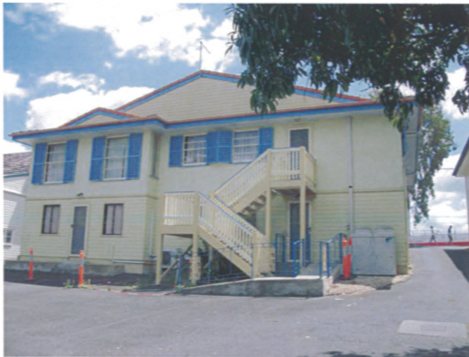
Photograph 10: View north towards the rear of 69 Uralba Street
