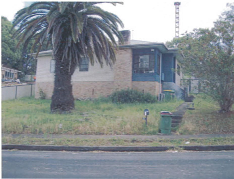
Photograph 13: View north towards 28 Dalziell Street
