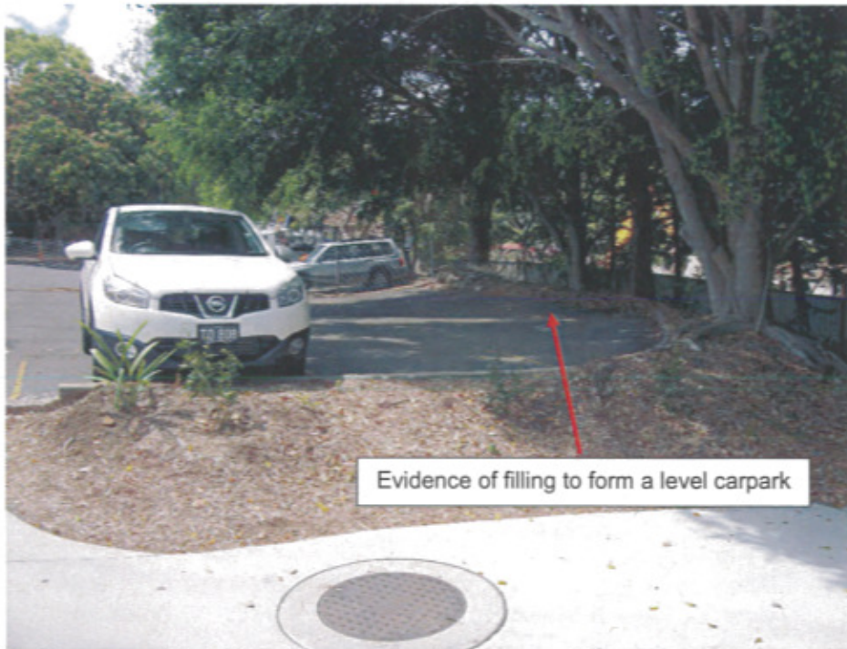
Photograph 6: Rear carpark of 61 Uralba Street and evidence of filling to form a level platform
