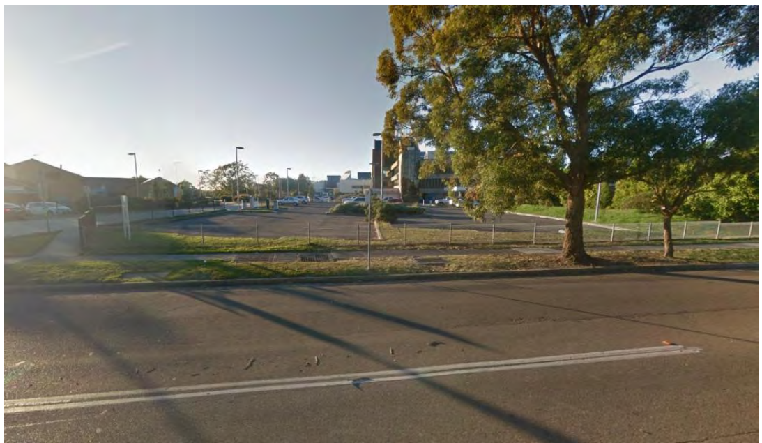
Figure 12 View of the site from Kareena Road. The carpark in the foreground forms part of the development zone (Source: Google)
