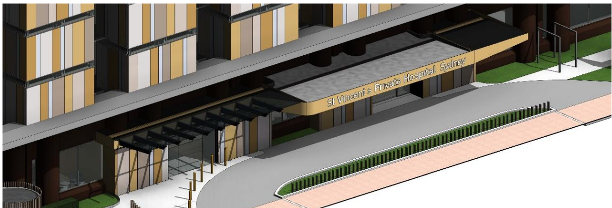
Figure 4 Indicative 3D view of awning extension
