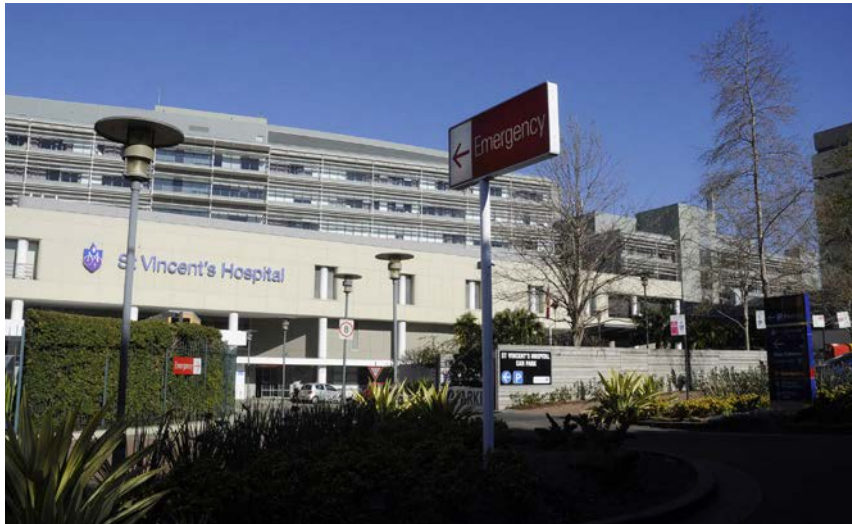
SVHS and forecourt off Victoria Street
