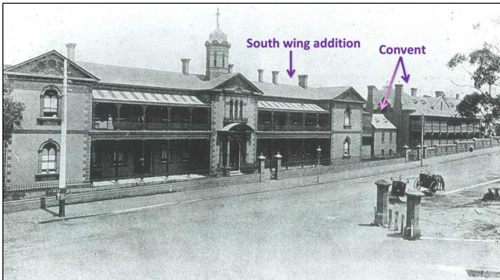
Figure 21: 1905 photograph showing the south wing addition to the hospital (Whitaker 2007:38).
