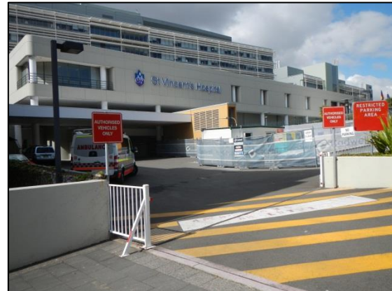
Figure 43: Ambulance parking area in front of the Aikenhead Building.
