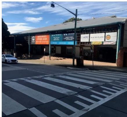
View of 15-17 Blaxland Road from Blaxland Road looking north-east
