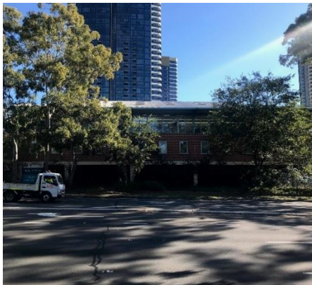
View of 15-17 Blaxland Road from Concord Road looking west
