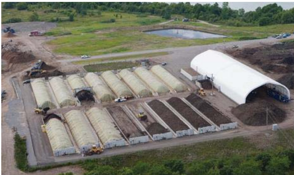
Figure 111 Example design of membrane cover (GORE and associates, 2013)
