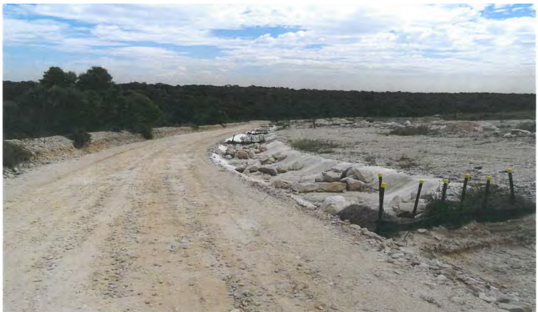
Figure 2.2 Lined drain along western perimeter haul road with siltation traps
