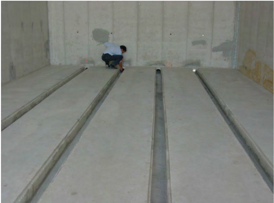
Photo 6.1 Example of aerated composting bunker floor
