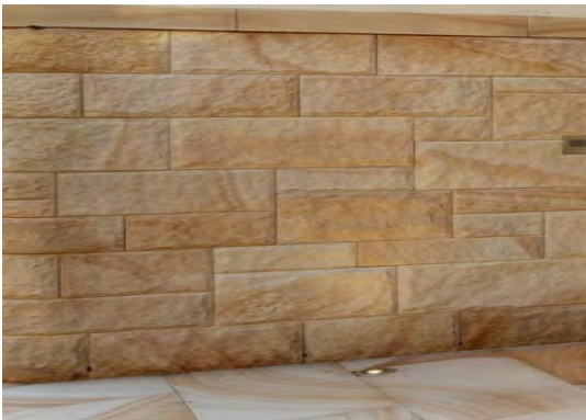
Sandstone external all finishes
