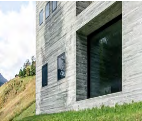
Earthy Tones to facade.
