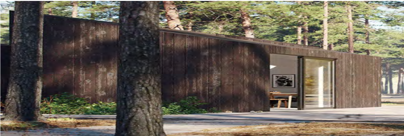
Low Scale building nestled in landscaping and nature - Loenen Pavilion by KAAN
