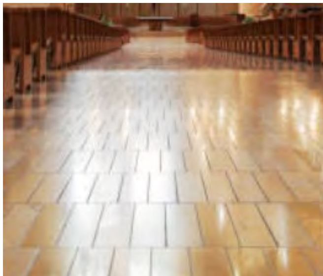
Floors internal chapel Sandstone floor tiles durable & easily maintained
