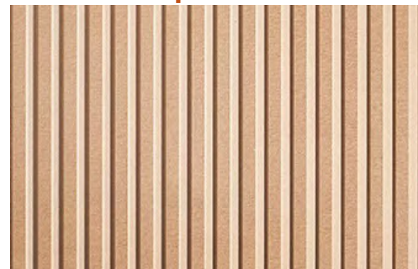
Timber Cladding on the ceiling
