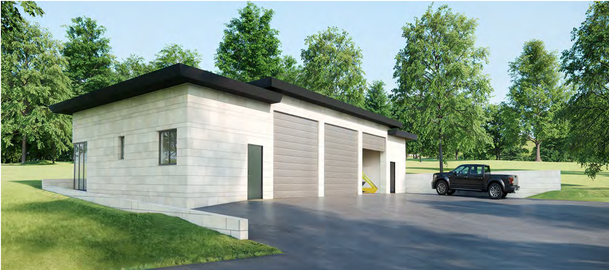
Nestle Building with Nature using darker tones thereby making building submissive and blending in with surrounding landscape settings
