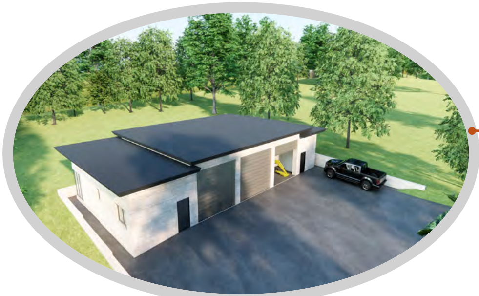
Step Roof designed to accommodated maintenance machines
