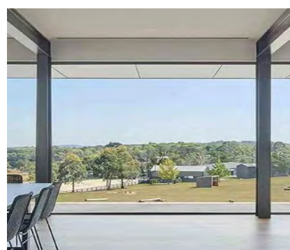
Full Height Glazing to maximise natural lighting internally
