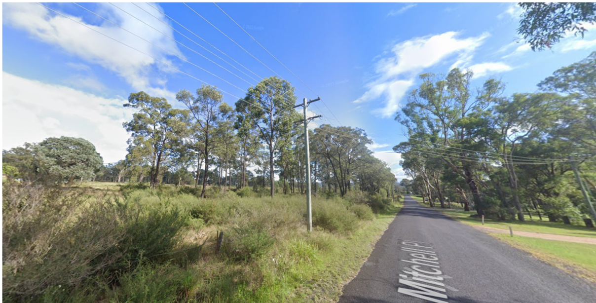
Image 3 – Existing Low Voltage Overhead Powerline Crossing Mitchell Place.
