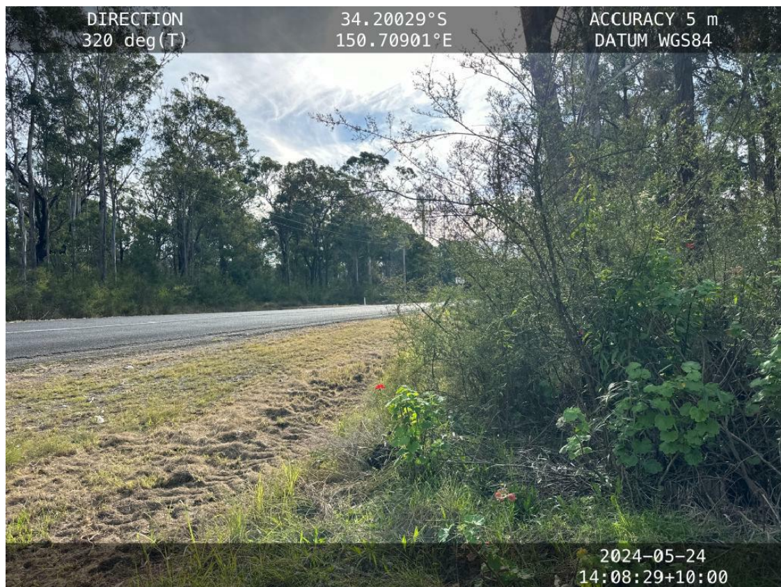
Figure 1-4 – Douglas Park Drive to the west (Source: TBE)
